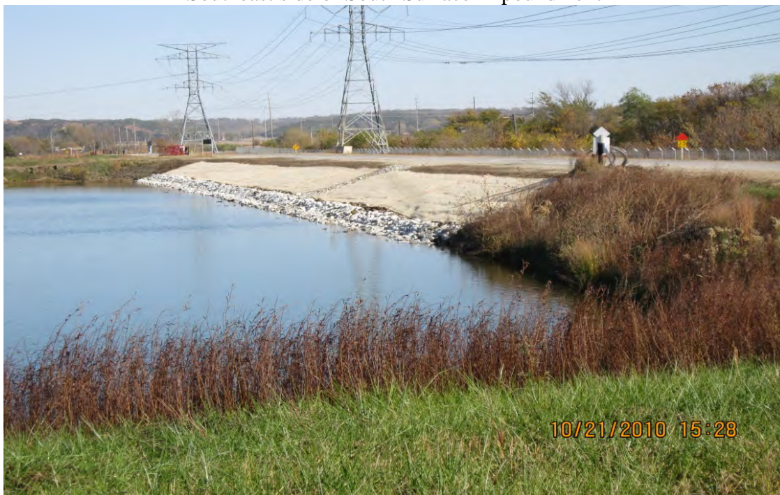
Photo 7 – Placed rip-rap to protect wave erosion action Southeast side of South Surface Impoundment
