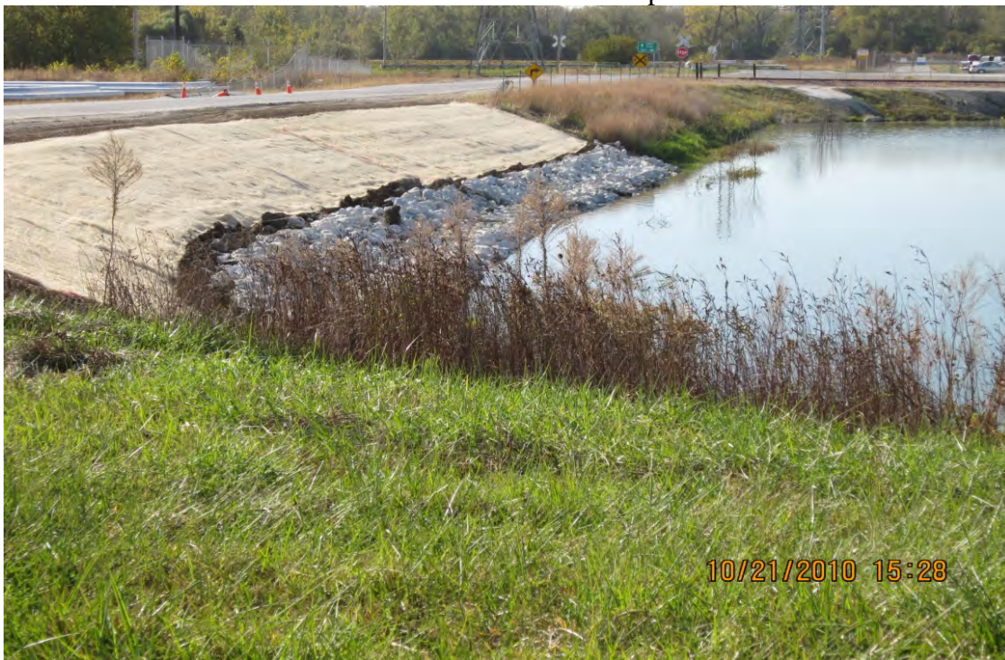
Photo 6 – Placed rip-rap to protect wave erosion action Southwest side of South Surface Impoundment
