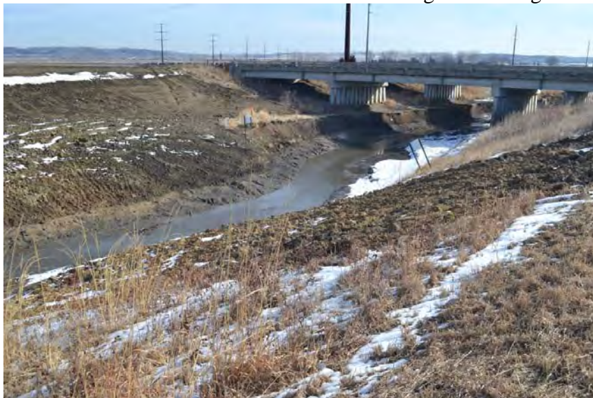
Photo 2 – Same area with final cover over slough area and graded
