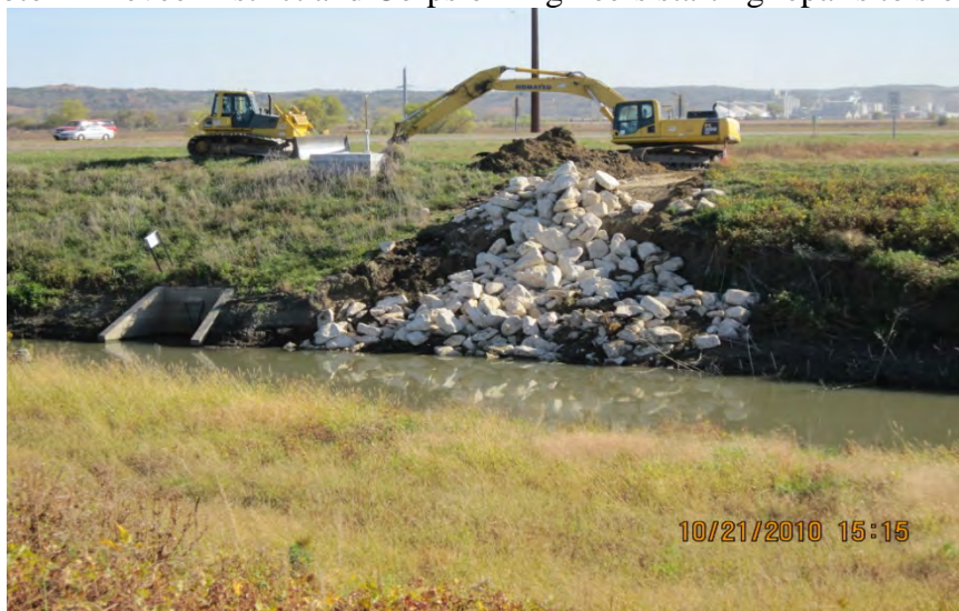
Photo 1 - Levee District and Corps of Engineers starting repairs to slough
