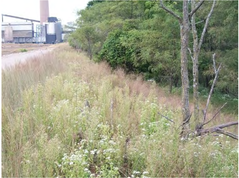
Figure 5.2.3b: Downstream/Outside Slope of Northern Portion of Embankment.
