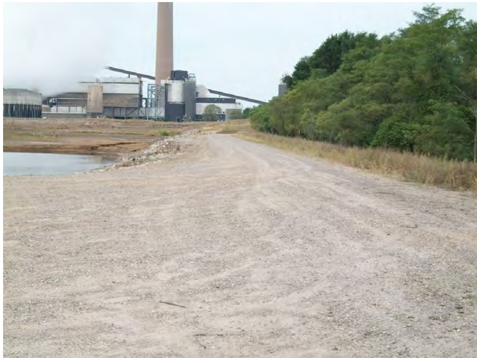
Figure 5.2.1: Crest of Bottom Ash Pond dike.
