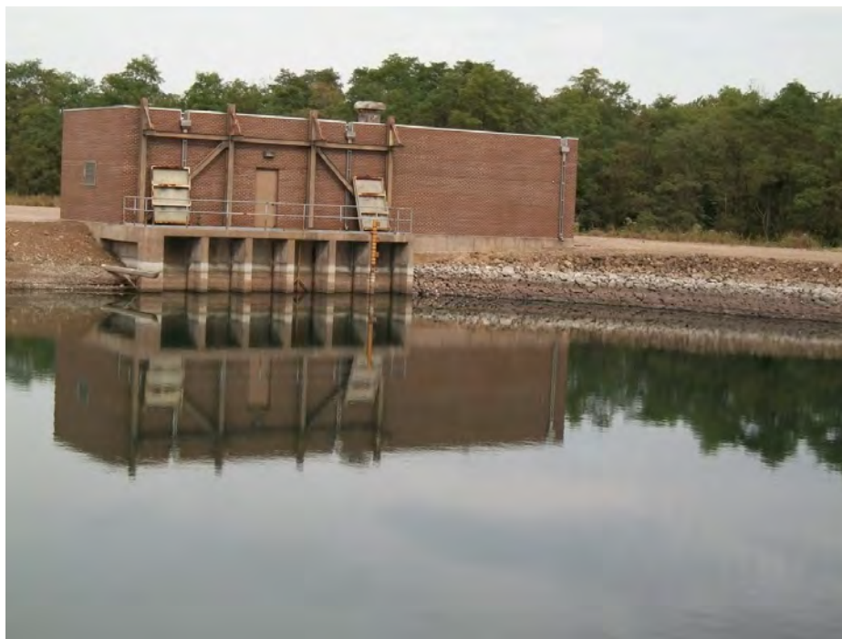
Figure 5.4.1: Pump-house serving Bottom Ash Pond.
