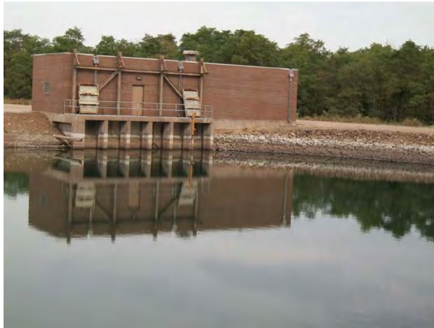
Figure 5.4.1: Pump-house serving Bottom Ash Pond.
