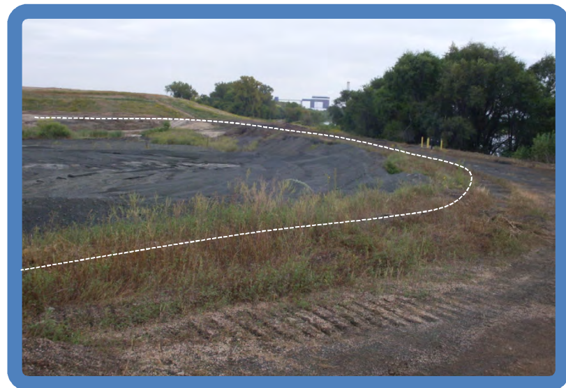
Photo 1.4 Pond 1 dike inside slope (SW side viewed SE) -mounded ash is in area of former erosion
