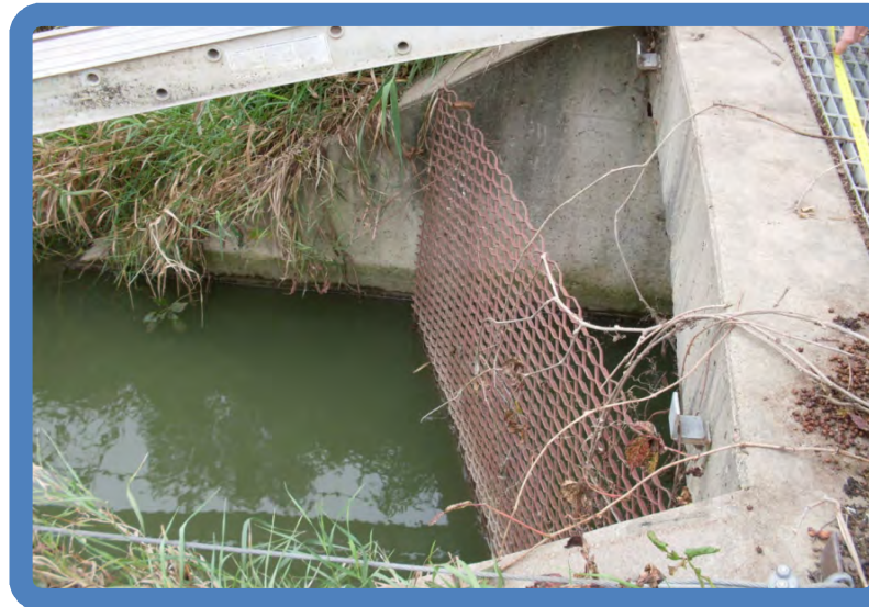
Photo 4.8 Inlet End of 48" RCP Culvert -screen to block animals and debris
