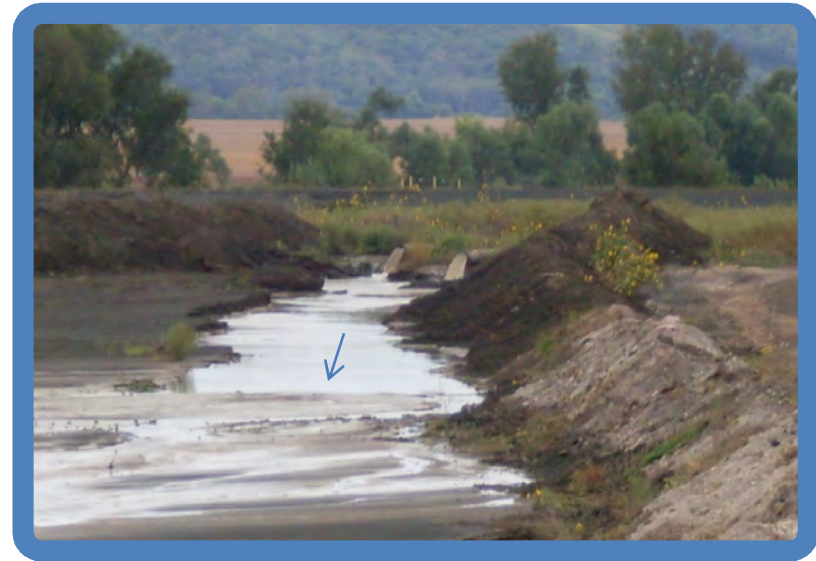
Photo 2.2 Pond 2 channel through ash from discharge lines
