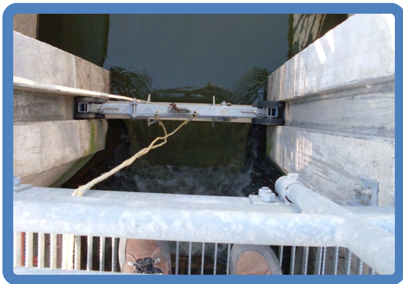
Photo 4.3 Pond 3B South Stop-log Structure adjustable weir
