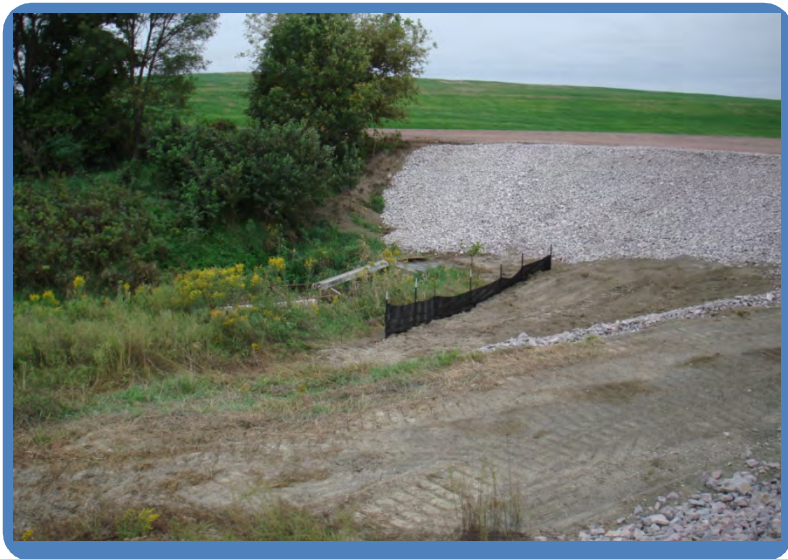
Photo 4.5 Outlet Pipe connects underground to 48" RCP, next to landfill
