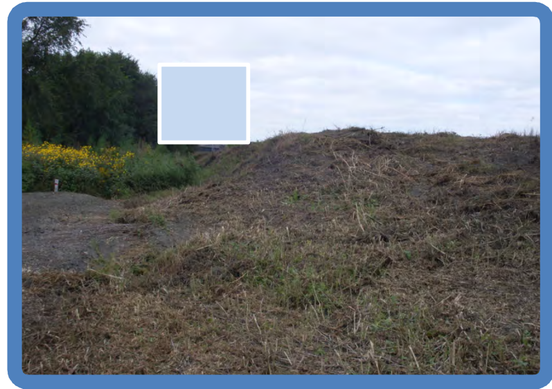
Photo 1.10 Pond 1 dike outside slope (SW side viewed NE)-note berm
