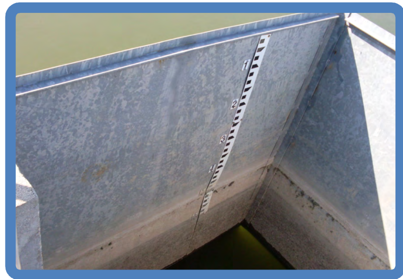
Photo 4.2 Pond 3B South Skimmer Box with staff gauge
