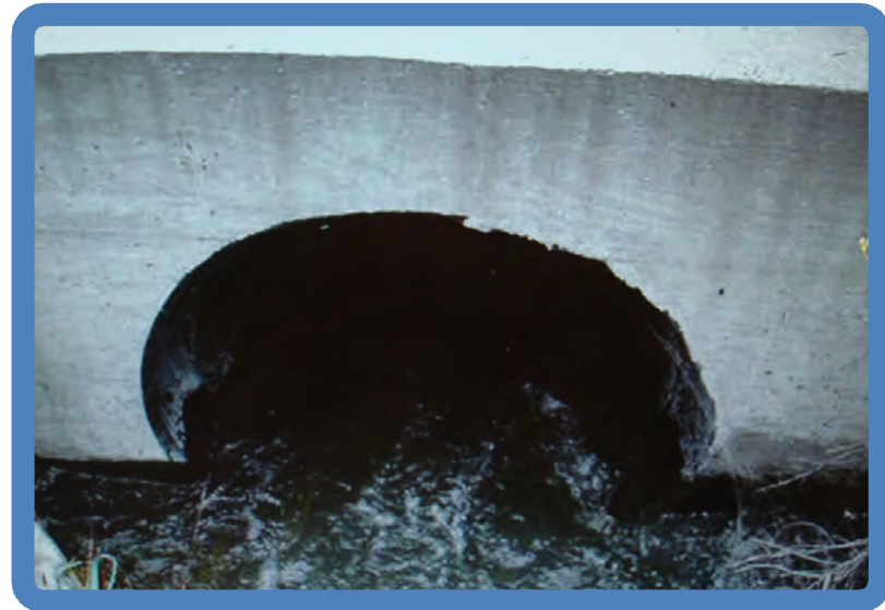
Photo 4.14 Final Outfall Structure 48" RCP to Missouri River
