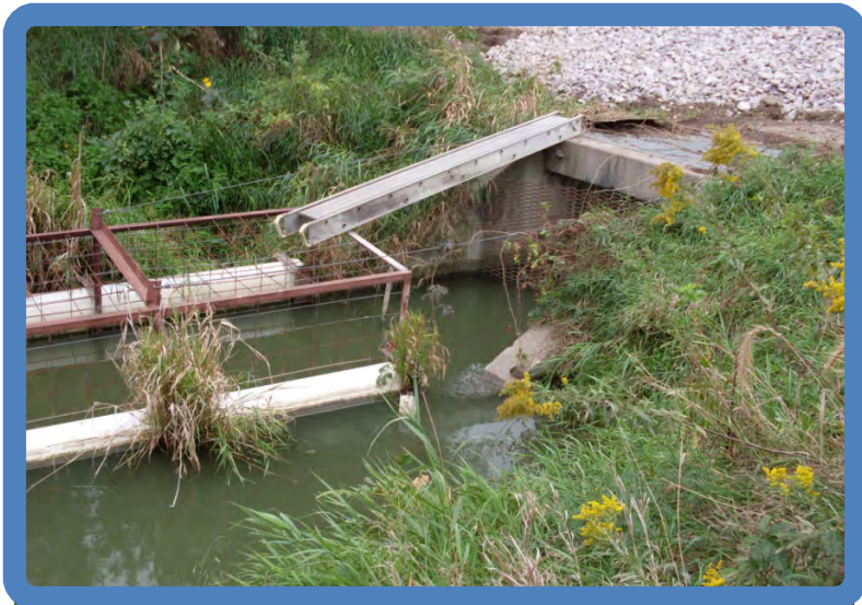
Photo 4.7 Inlet End of 48" RCP Culvert -cage to stop beaver activity
