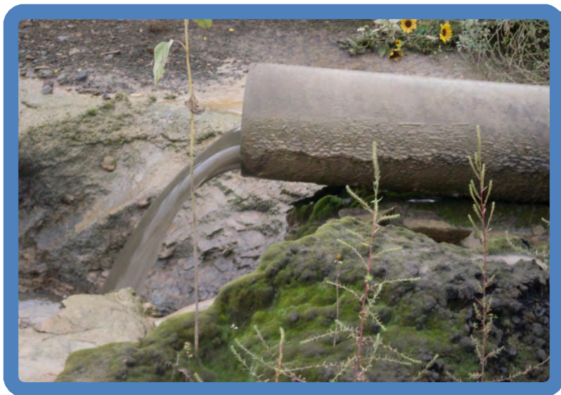
Photo 2.15 Pond 2 ash sluice discharge pipe
