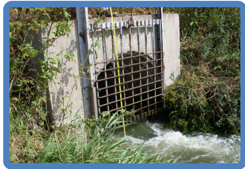
Photo 4.10 Close up of Outlet End of 48" RCP Culvert
