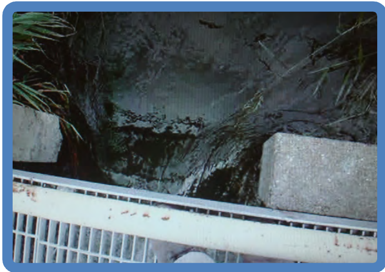
Photo 4.13 Final Outfall Structure Rectangular Weir 3'x3' opening
