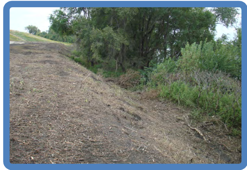
Photo 1.6 Pond 1 dike outside slope (SW side viewed SE)-note berm
