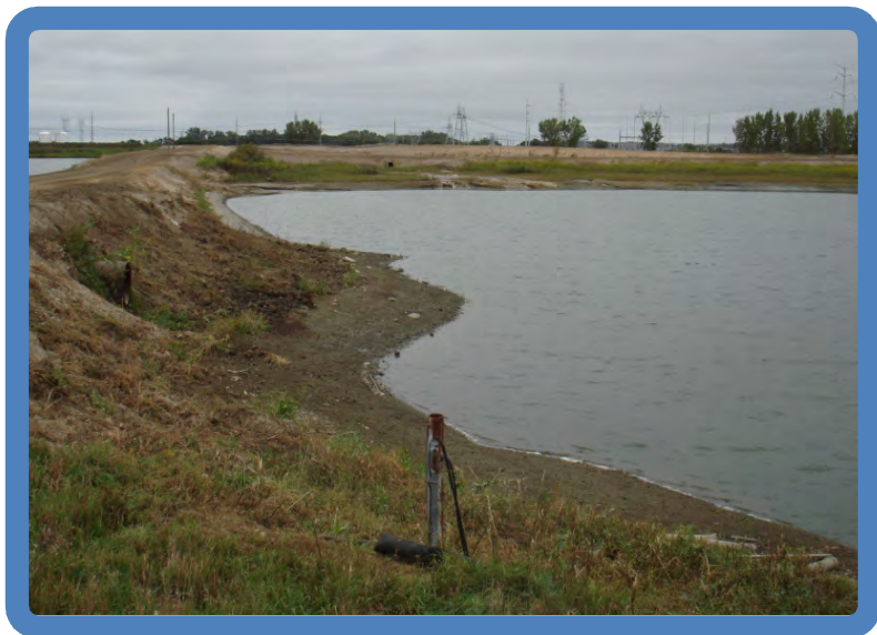
Photo 4.15 Pond 3B South cross dike inside slope with emergency high overflow pipe (SW side viewed NW)
