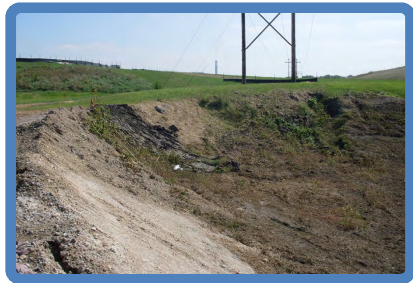
Photo 2.12 Pond 3A dike outside slope (SW segment viewed SE) -note erosion repair area
