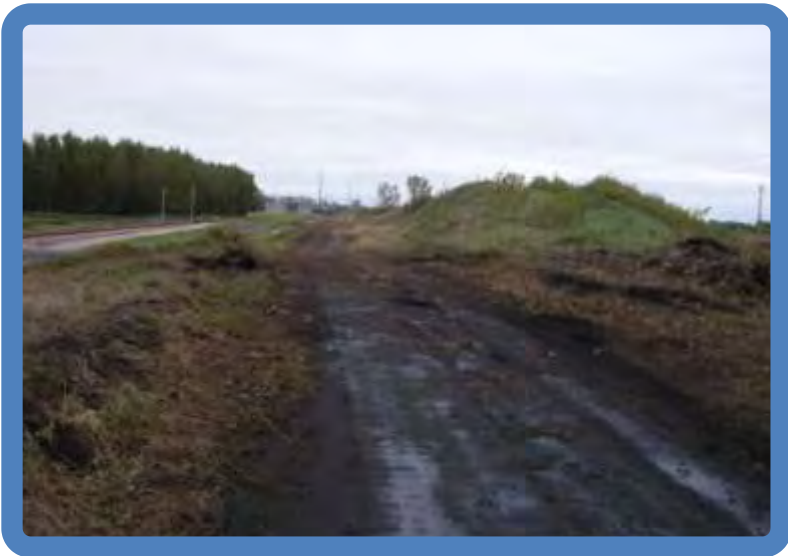
Photo 2.3 Pond 2 dike crest (NW side viewed NE)
