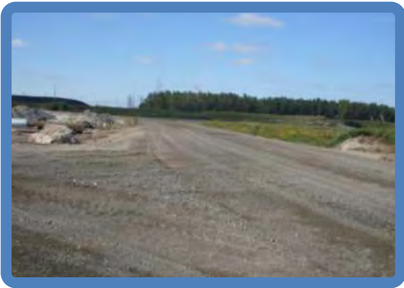
Photo 3.29 Pond 2 cross dike crest (NE side viewed NW)
