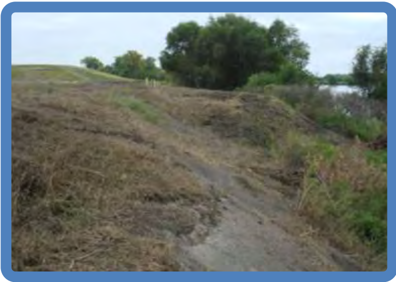
Photo 1.5 Pond 1 dike outside slope (SW side viewed SE)-note berm
