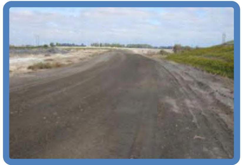
Photo 2.6 Pond 2 dike crest (SE side viewed NE)
