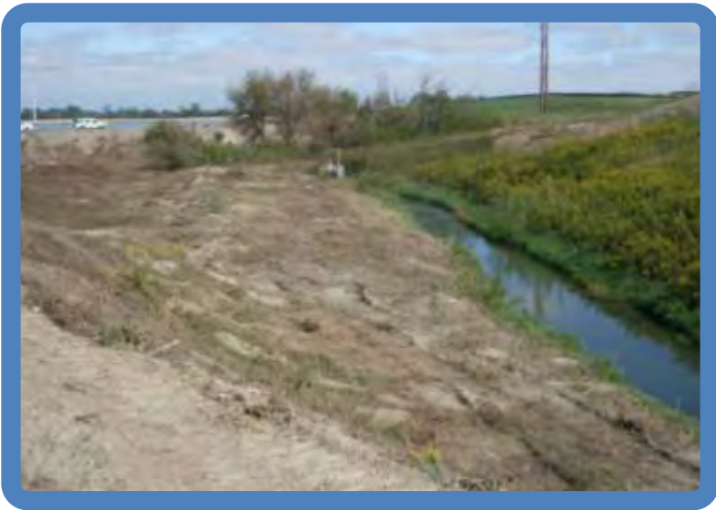
Photo 2.9 Pond 2 dike outside toe area (SE side viewed NE)
