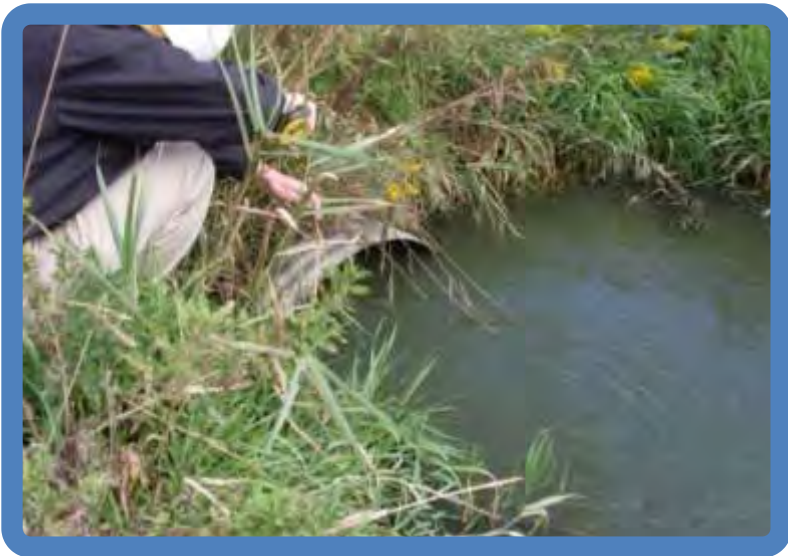
Photo 4.11 Outlet End of 48" Aluminum CMP Culvert in Discharge Channel
