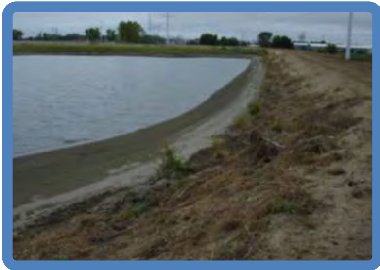
Photo 3.7 Pond 3B South dike inside slope (NE side viewed N)
