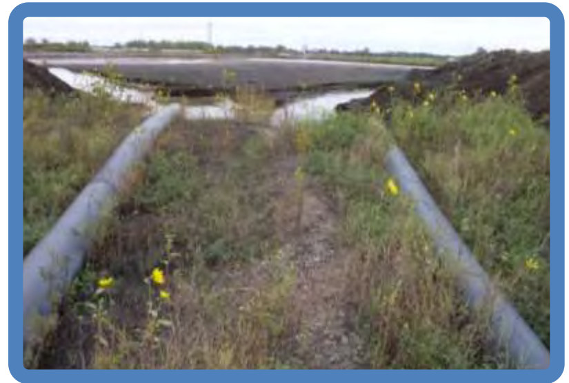
Photo 2.4 Pond 2 ash sluice and drainage discharge pipes to pond
