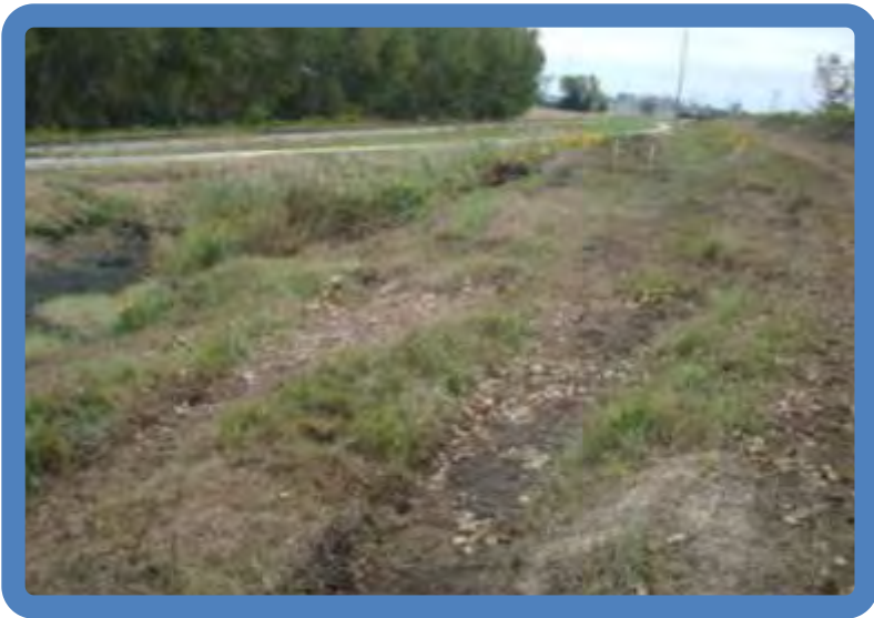
Photo 3.23 Pond 3A outside toe area (NW side viewed NE)
