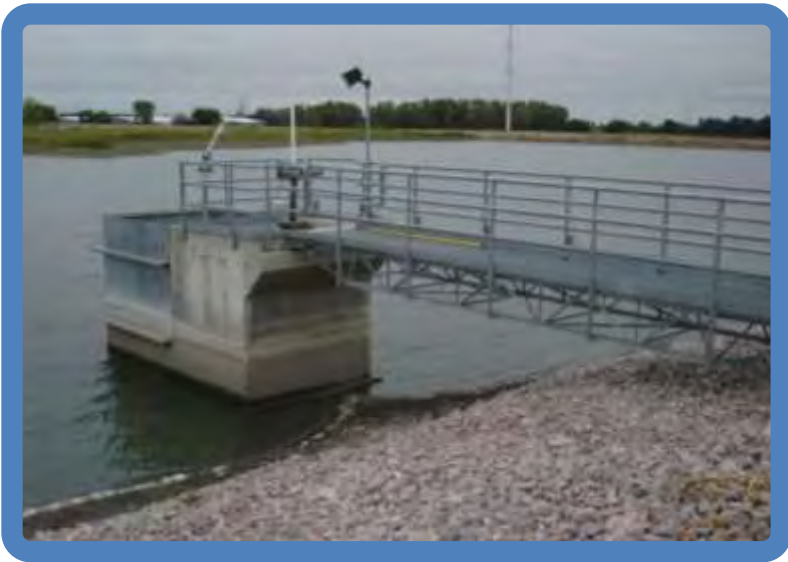
Photo 4.1 Pond 3B South Stop-log Structure
