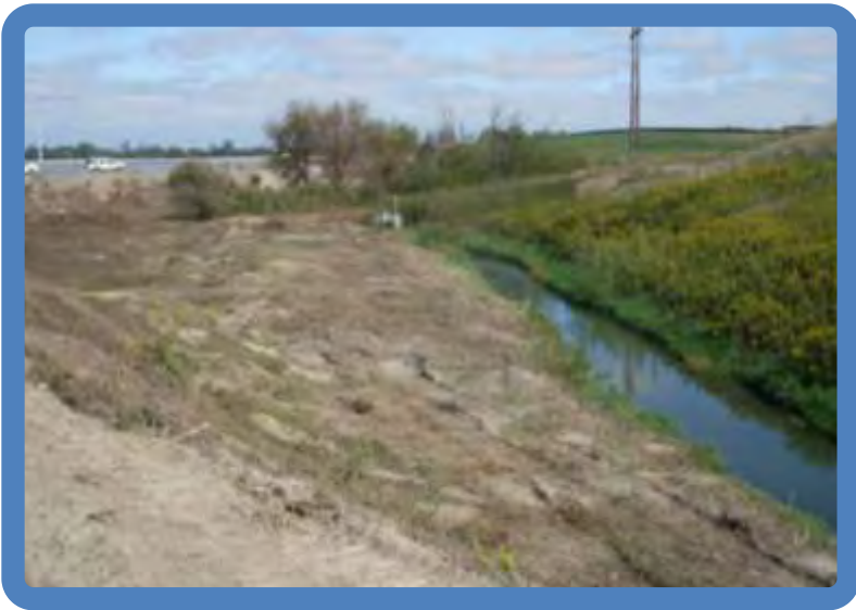
Photo 4.9 Outlet End of 48" RCP Culvert adjacent to landfill
