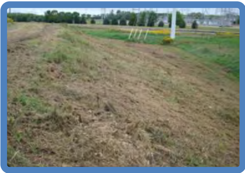
Photo 3.15 Pond 3B North dike outside slope (NE side viewed NW)
