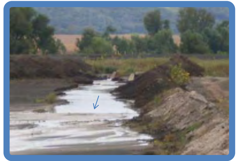
Photo 2.2 Pond 2 channel through ash from discharge lines
