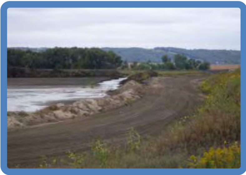
Photo 2.1 Pond 2 NW inside access road to NE cross dike (viewed SW)
