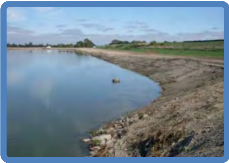
Photo 3.25 Pond 3A dike inside slope (S side viewed E)
