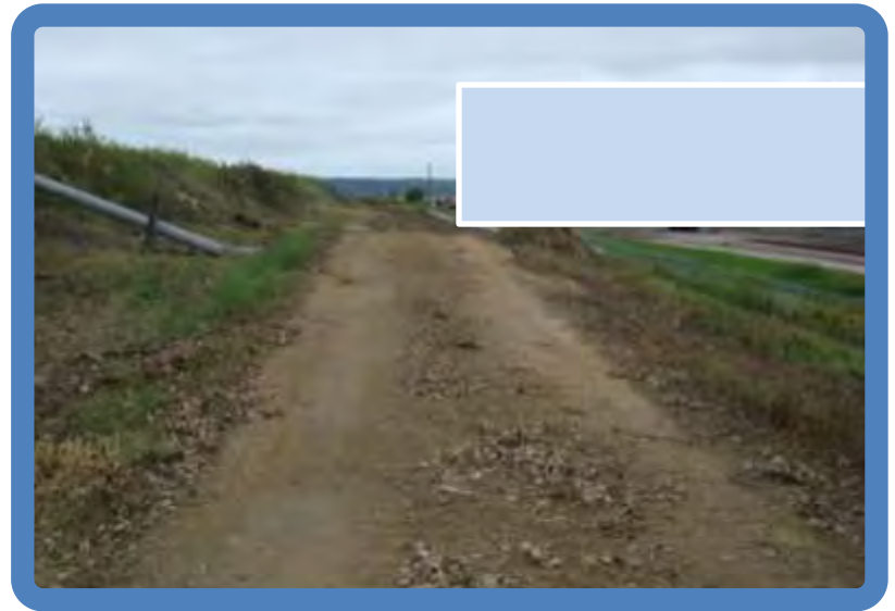
Photo 3.22 Pond 3A dike crest (NW side viewed SW)
