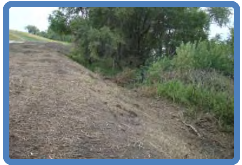
Photo 1.6 Pond 1 dike outside slope (SW side viewed SE)-note berm
