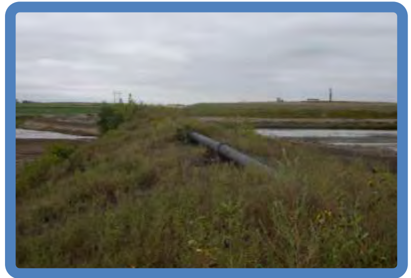
Photo 3.32 Pond 3A ash sluice discharge pipe infrequently used
