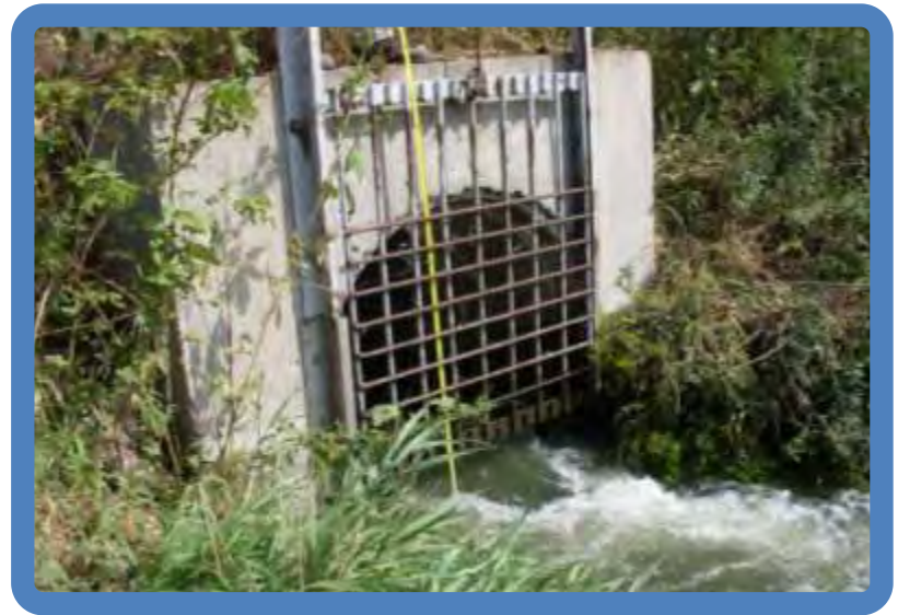
Photo 4.10 Close up of Outlet End of 48" RCP Culvert
