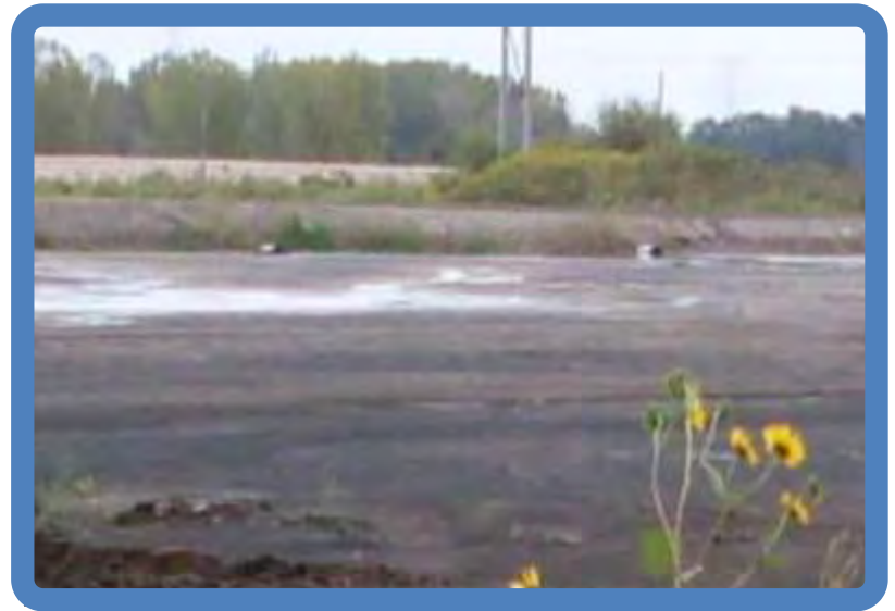
Photo 2.14 Pond 2 cross dike inside slope (NE side viewed NE)-culverts
