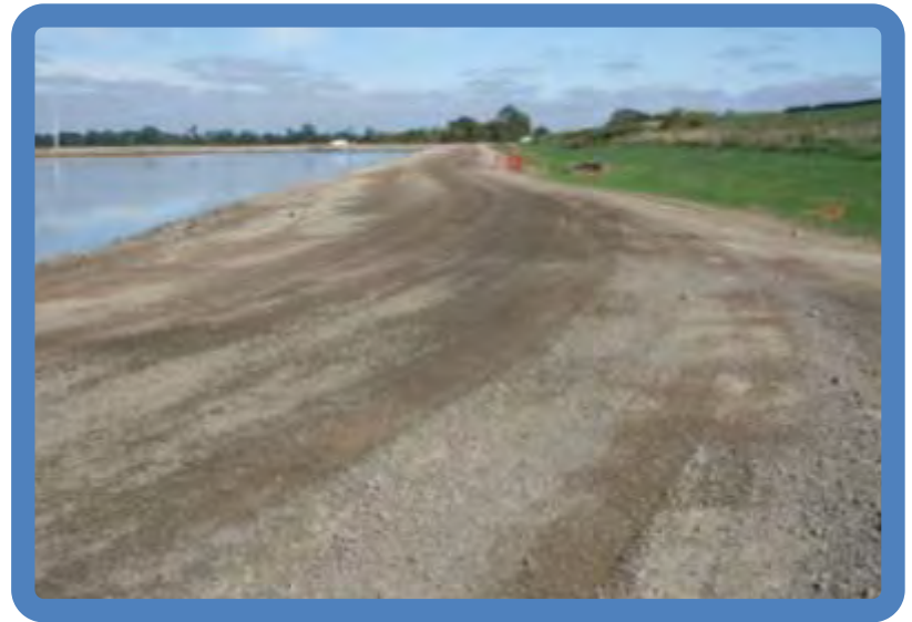
Photo 3.26 Pond 3A dike crest (S side viewed E)
