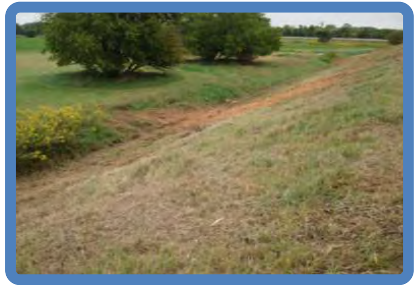
Photo 3.14 Pond 3B North dike outside slope (NE side viewed SE)
