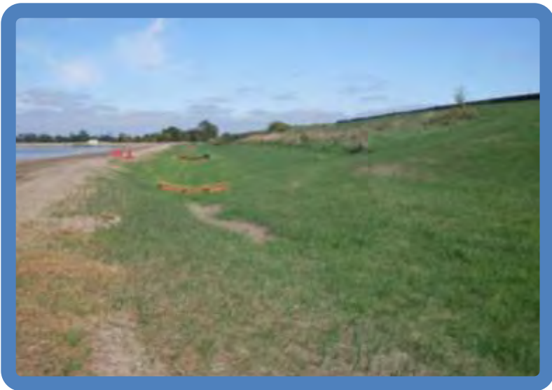
Photo 3.27 Pond 3A dike outside swale (S side viewed E)
