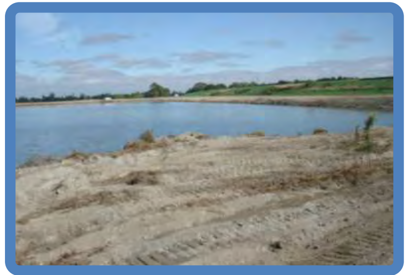
Photo 3.28 Pond 3A dike inside slope (S side viewed SE)
