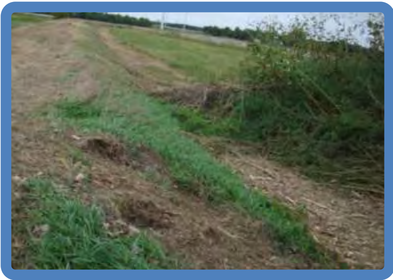
Photo 3.13 Pond 3B North dike inside slope (NE side viewed SE)
