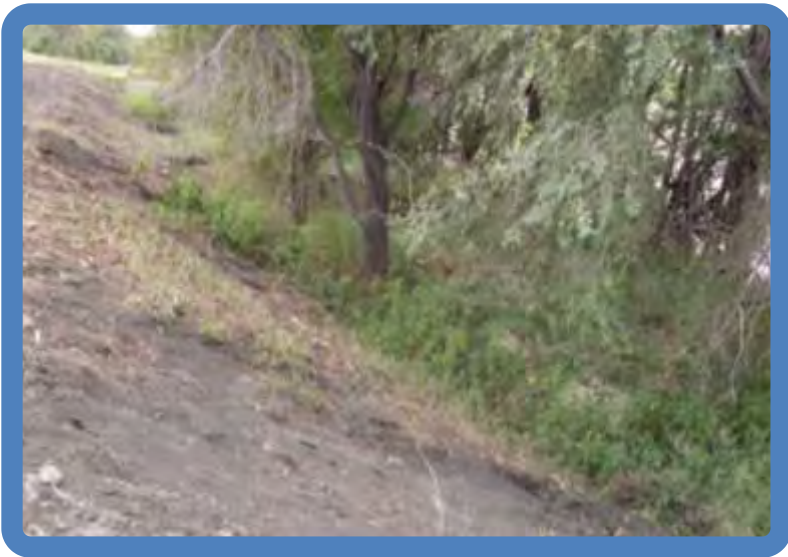
Photo 1.7 Pond 1 dike outside slope (SW side viewed SE)
