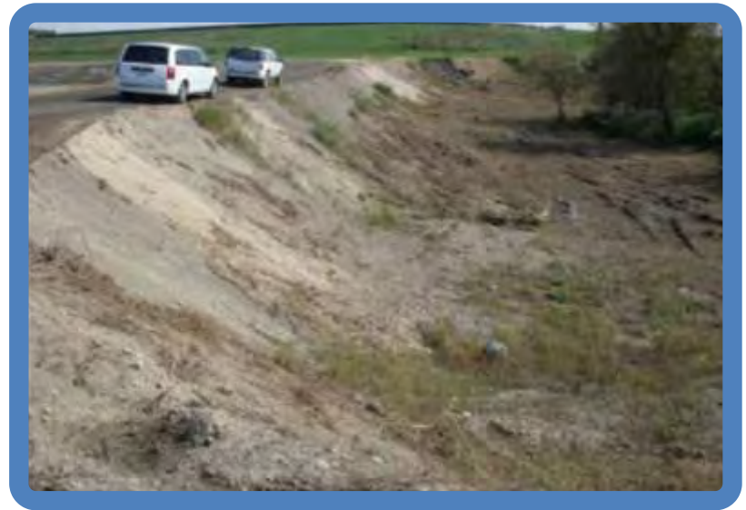
Photo 2.10 Pond 3A dike outside slope (SW segment viewed SE)
