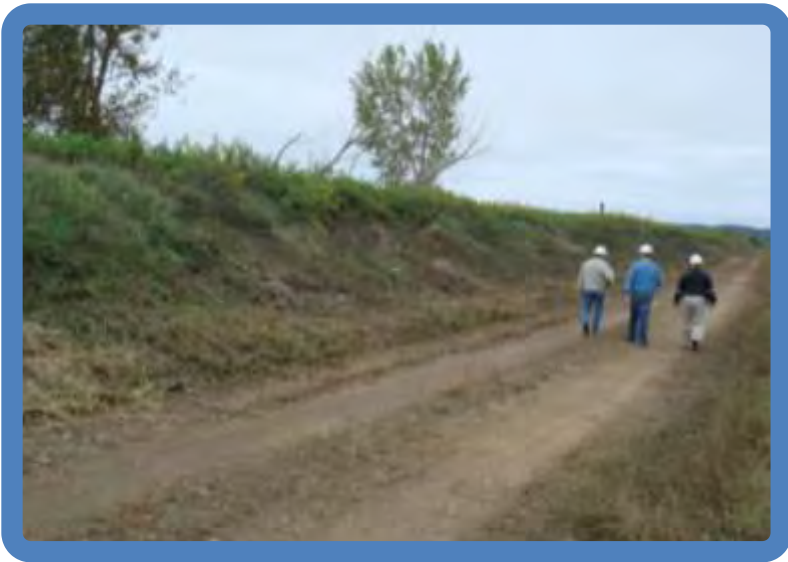
Photo 3.21 Pond 3A dike crest (NW side viewed SW)
