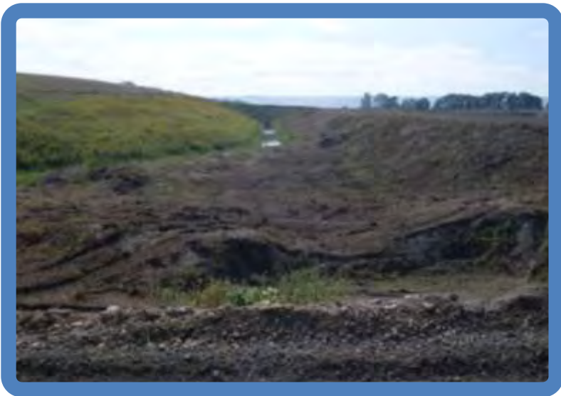
Photo 2.11 Pond 2 dike outside slope (SE side viewed SW)
