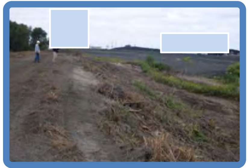
Photo 1.8 Pond 1 dike inside slope (SW side viewed NW)
