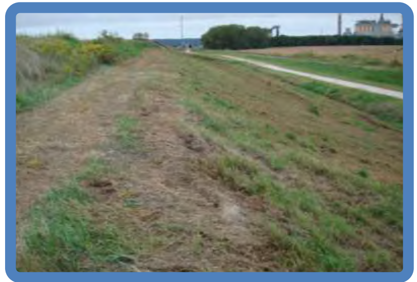
Photo 3.16 Pond 3B North dike outside slope (NW side viewed SW)
