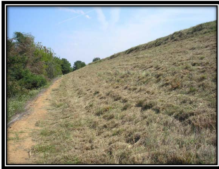
Figure 5.2.3-2 Ash Disposal Pond Emergency Sludge cell north exterior slope.
