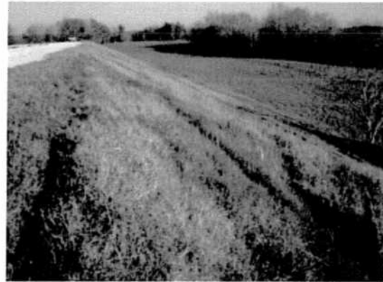
Figure 4: Downstream Slope of Berm
