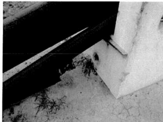
Figure 70: Return Line Southwest Structure
