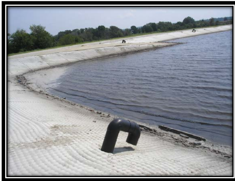
Figure 5.2.2-2 East cell interior slope.
