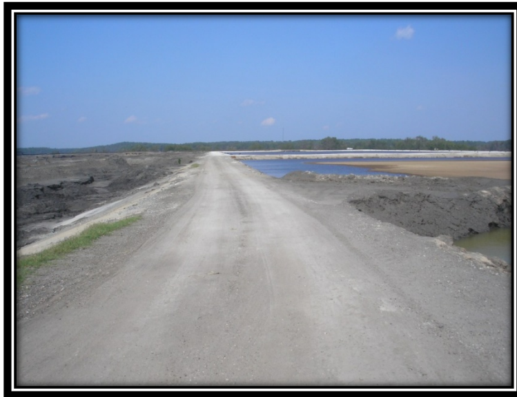
Figure 5.2.1-3 West-East Ash Disposal Pond interior dike.
