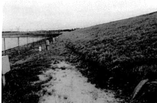
Figure 86: Downstream Toe of PDP #3 Berm
