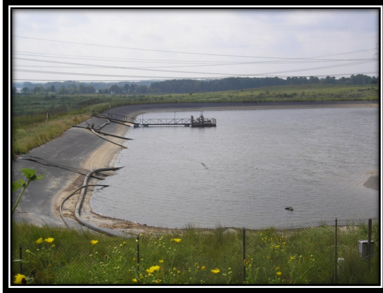
Figure 5.2.2-1 PDP-4 east interior slope.
