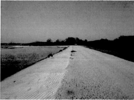
Figure 3: Upstream Slope of Berm and Crest
