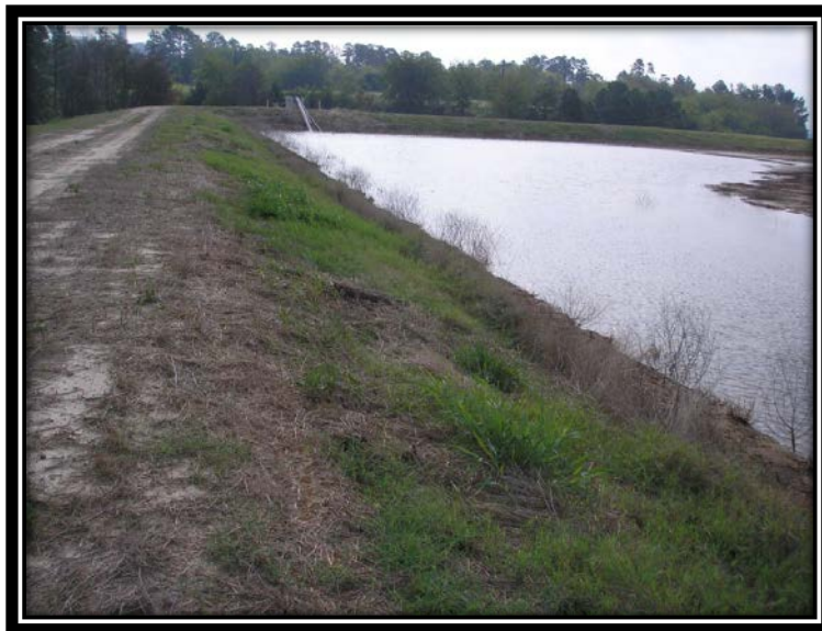
Figure 5.2.2-3 PDP-5 north interior slope.
