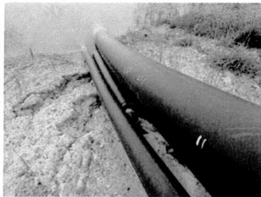
Figure 71: Return Line Northeast Structure
