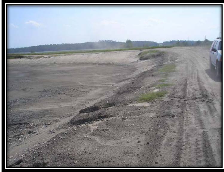
Figure 5.2.2-1 West cell interior slope.
