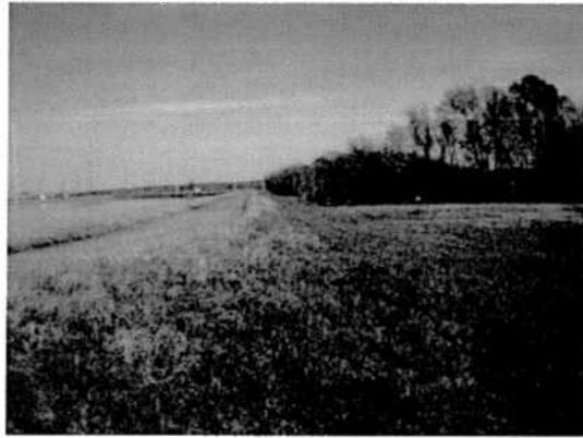
Figure 54: Downstream Embankment West LARP
