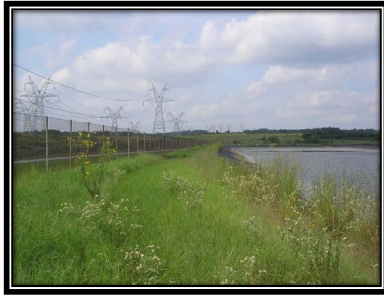
Figure 5.2.1-2 PDP-4 south crest.
