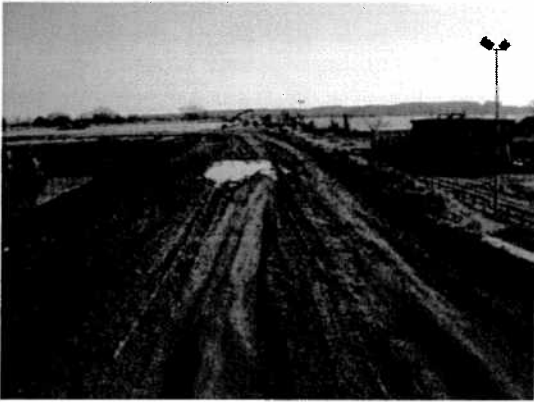
Figure 13: Rutting in Crest from Vehicular Traffic
