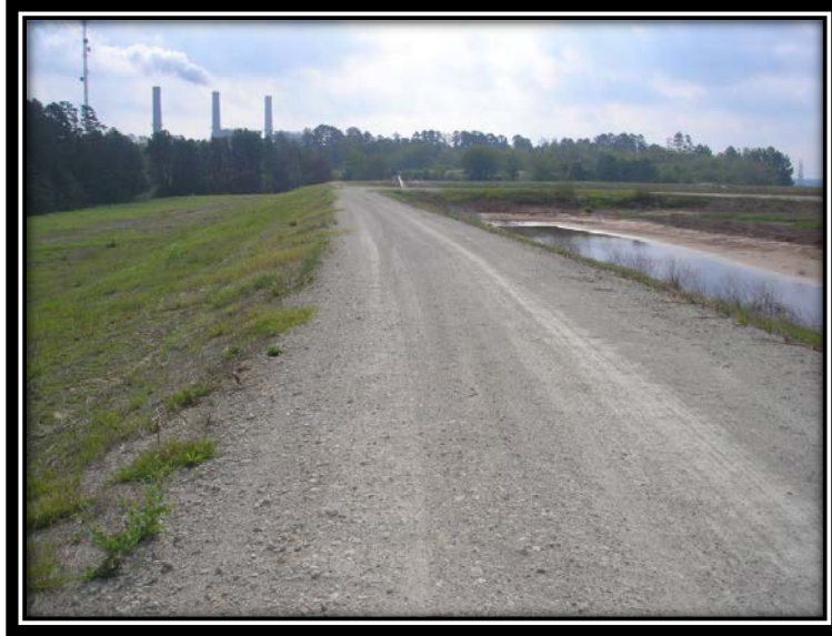
Figure 5.3.1-1 Typical crest around PDP-5 Pond.
