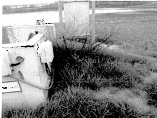
Figure 81: Bush near Southeast Dewatering Access Structure
