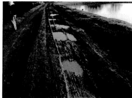
Figure 6: Crest Rutting North Side
