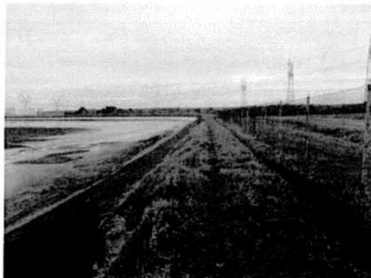
Figure 57: Typical Condition of Crest
