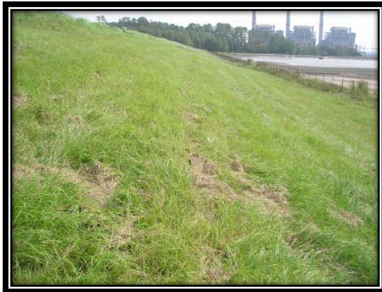
Figure 5.3.3-1 Typical exterior slope at PDP-4
