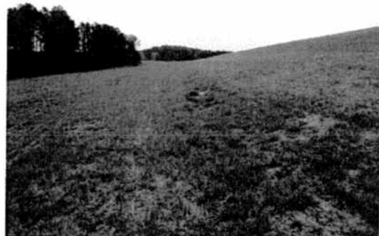
Figure 74: Downstream Side of Impoundment
