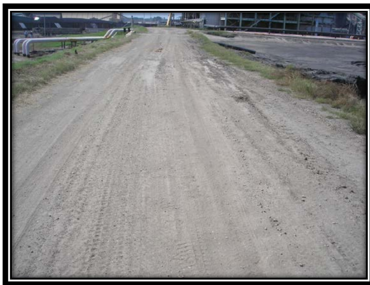
Figure 5.2.1-1 Ash Pond West Cell south Dike crest.
