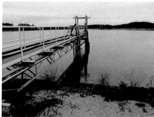
Figure 68: Submersible Pump at Decant Structure
