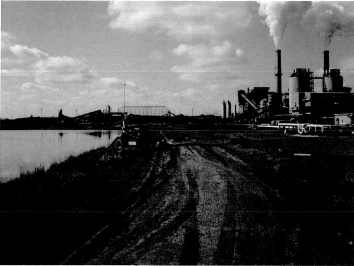
Figure 22: Portable Pump Removing Water from Storm Water Pond
