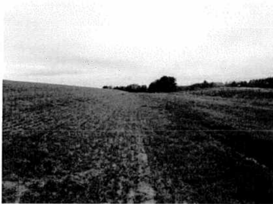
Figure 73: Downstream Side of Impoundment
