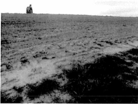
Figure 75: Minor Erosion Rills
