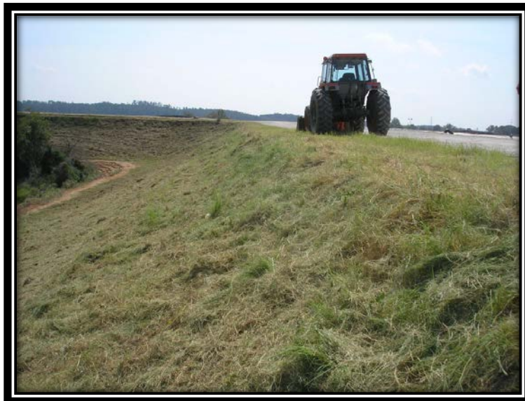
Figure 5.2.4-1 Typical exterior groin in the Ash Disposal Pond.
