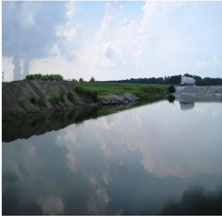
Figure 5.2.2-1. Photo Showing Upstream/Inside Slope at Fly Ash Cell
