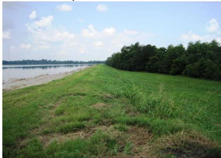
Figure 5.2.3-1. Photograph Showing Typical Downstream Slope Conditions
