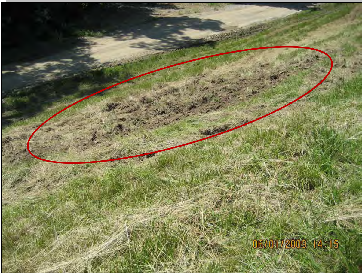
Photo 9 – Typical rutting and slope sloughing due to heavy mowing tractor, western downstream slope
