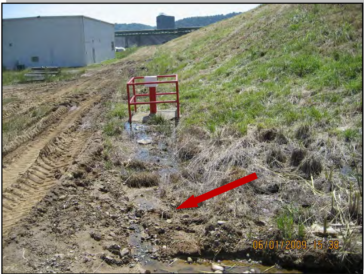
Photo 15 – Wet Area or minor seepage at toe of south embankment possibly due to discharge from gravel toe drain (View looking west)
