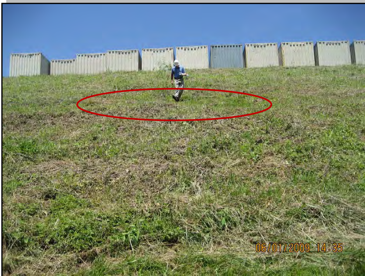
Photo 10 – Old slough on western downstream slope
