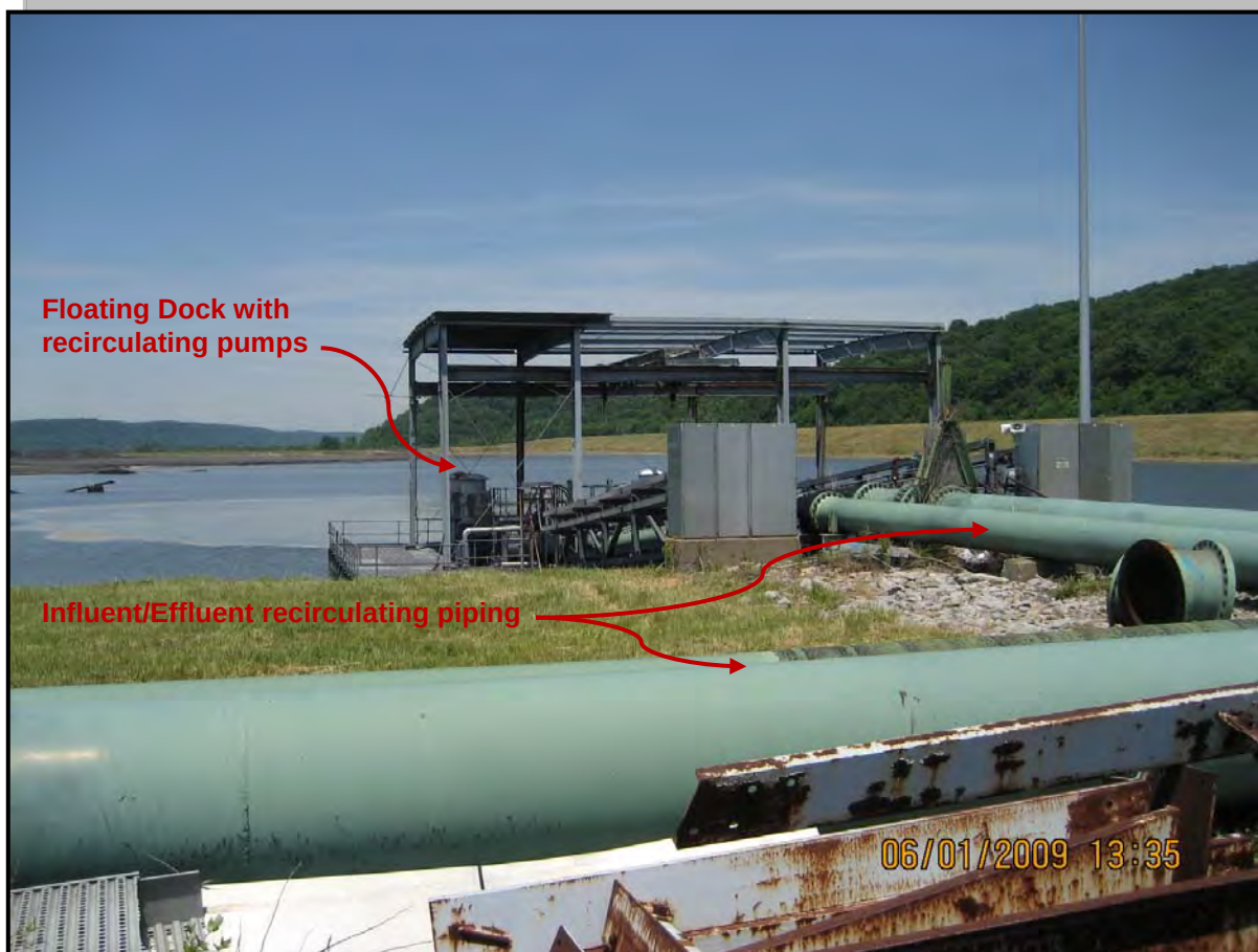
Photo 1 - View of Floating Dock with recirculating pumps and piping along South Dike
