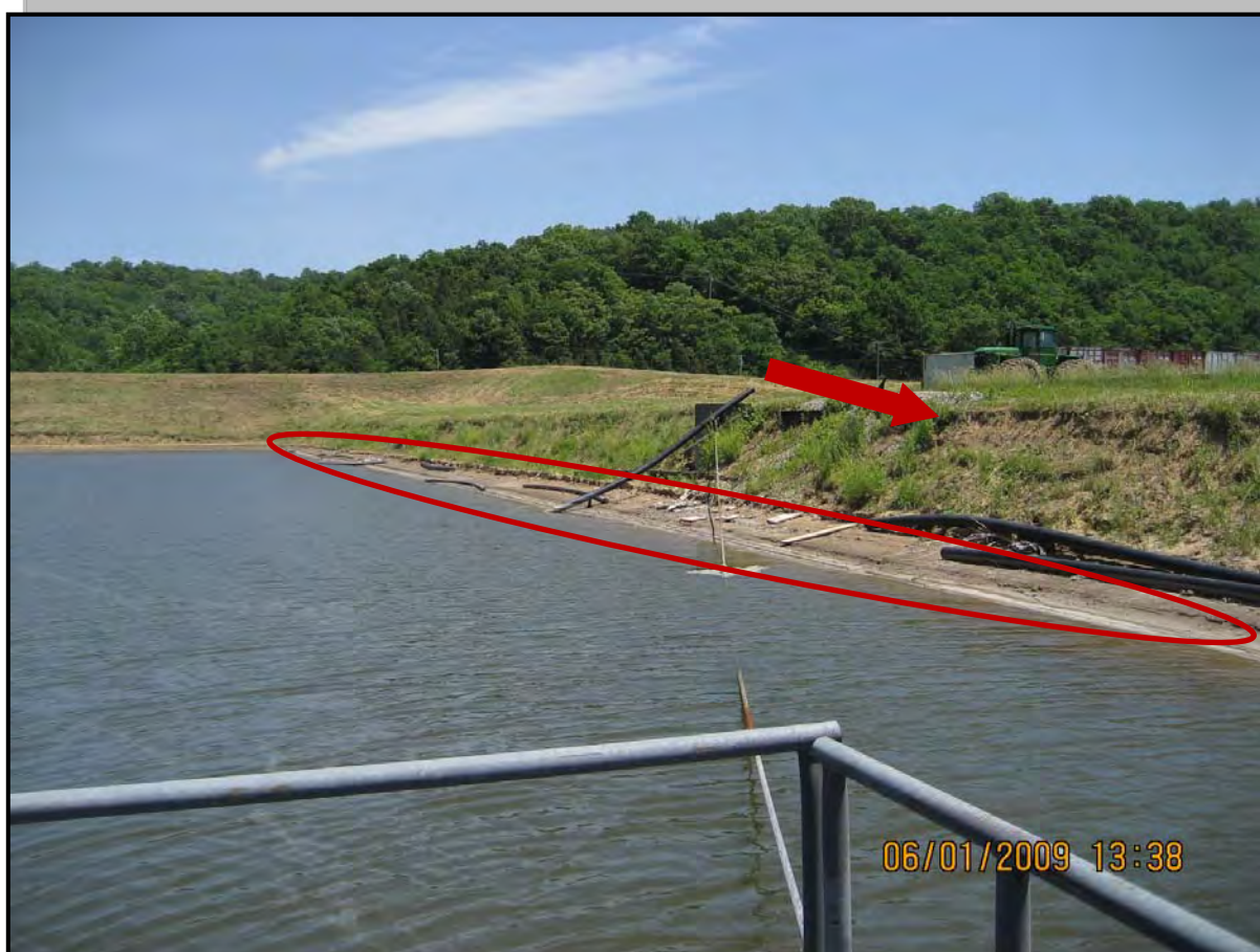
Photo 2 – View of South Dike with erosion and sloughing of upstream slope freeboard caused by wave action
