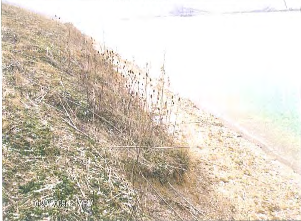
Photo #5: Wave erosion, steep drop near water surface, East embankment, upstream slope, directly across from bottom ash reclaim, looking South
