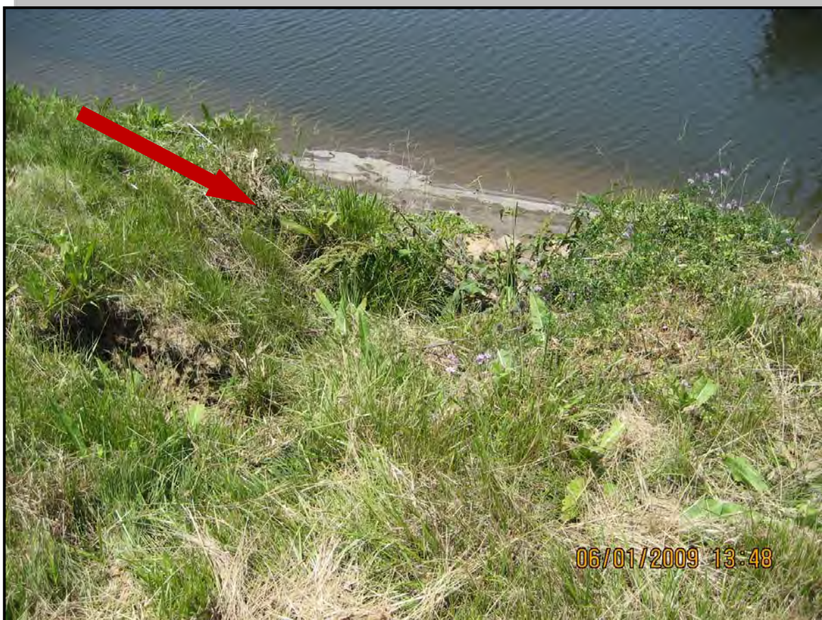
Photo 4 – View of typical erosion gullies in freeboard area along upstream slope near Floating Dock
