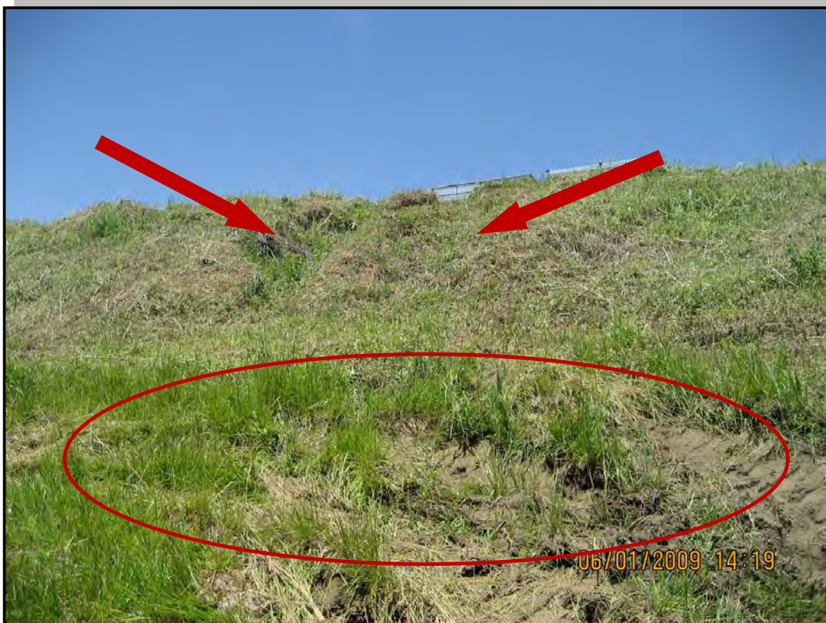
Photo 8 – Typical erosion gullies along western downstream slope near inside curved slope of embankment
