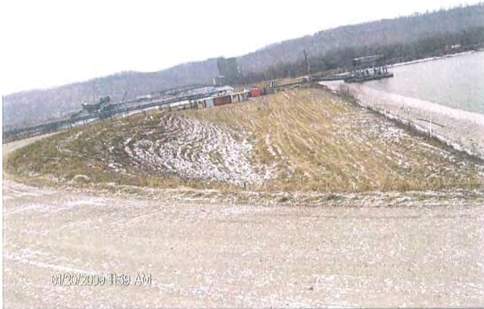
Photo #3: South embankment, upstream slope, looking West
