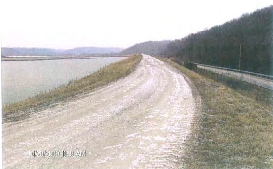
Photo #2: East embankment, crest, looking North
