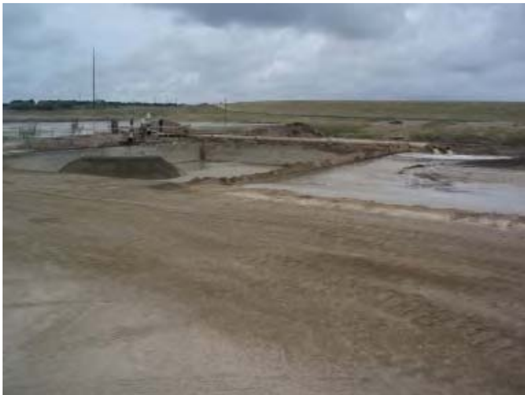
Photo No. 95: CADD – Overview of two primary settling basins where CCW is sluiced into the impoundment. Settling basins are alternated and cleaned out when full.
