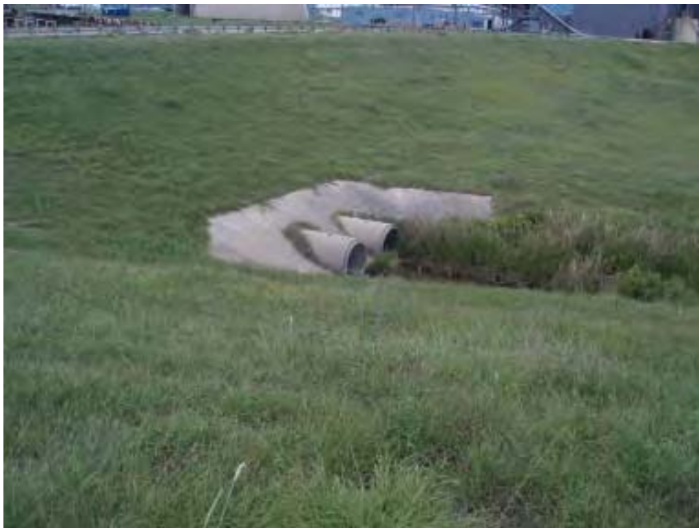
Photo No. 37: Reclaim Pond - North embankment exterior slope, looking north at two 8-foot-diameter drainage pipes at toe of slope.
