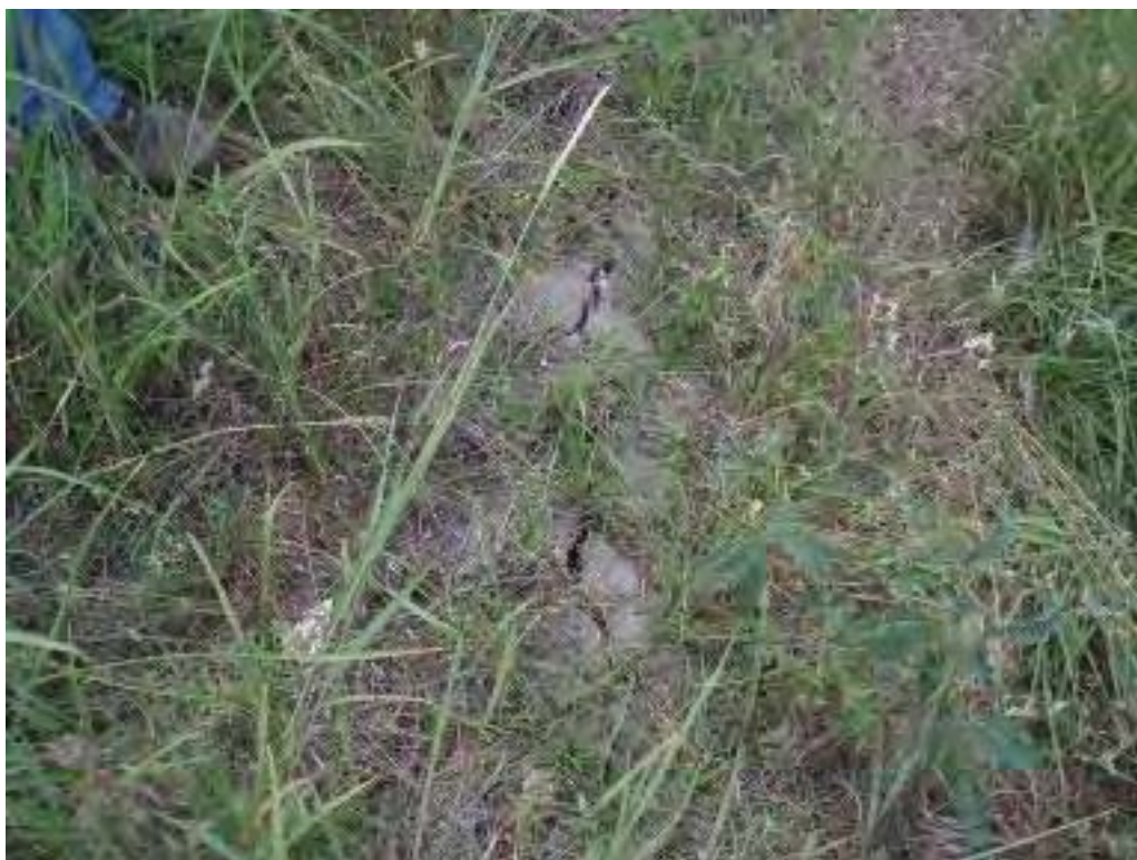
Photo No. 32: Reclaim Pond - North embankment exterior slope, looking at typical desiccation cracks.
