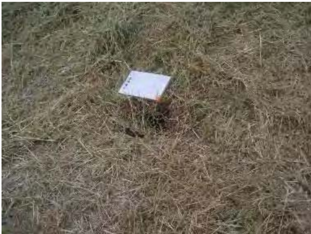
Photo No. 65: CADP - East embankment exterior slope, looking at an 8-inch-diameter rodent hole.
