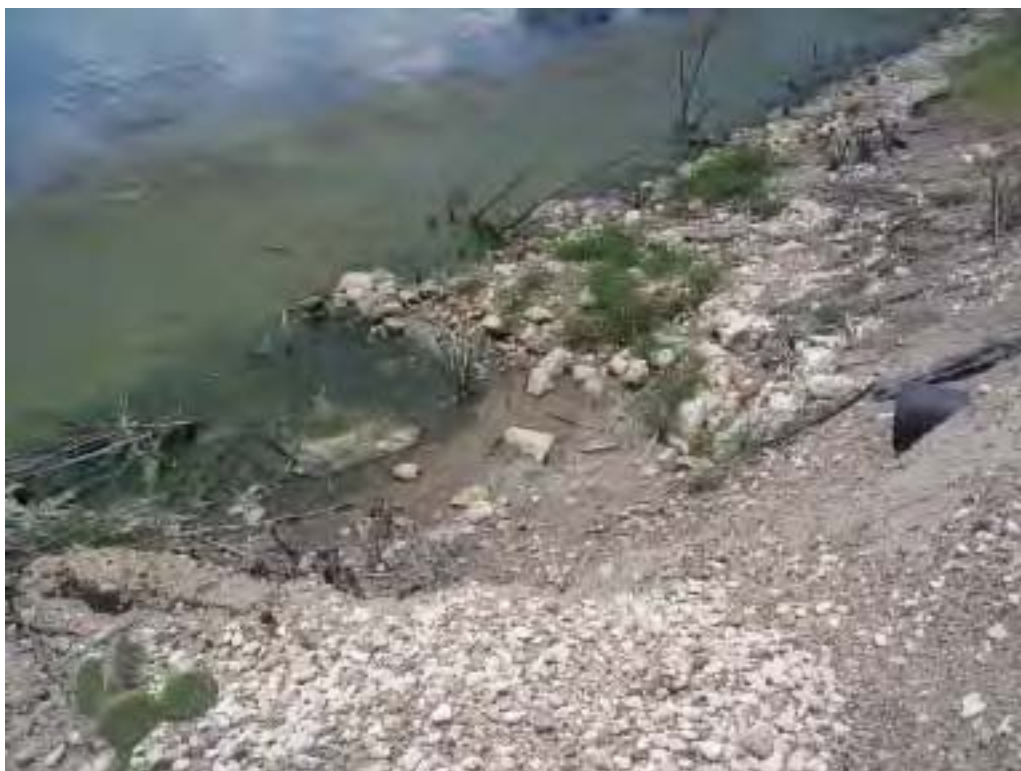
Photo No. 21: Reclaim Pond - East embankment interior slope, looking at abandoned 12-inch-diameter HDPE discharge pipe from the CADP. Note the embankment has been eroded at the discharge pipe.
