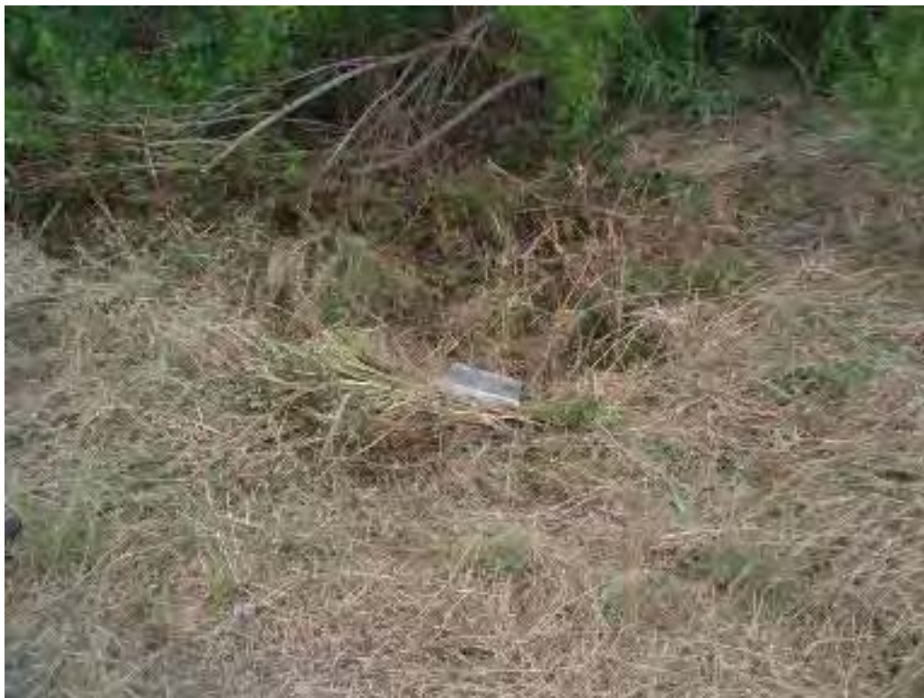
Photo No. 79: CADP - South embankment exterior slope, looking at 3'Wx4'Lx2'D depression at toe of slope. Possible collapsed rodent burrow
