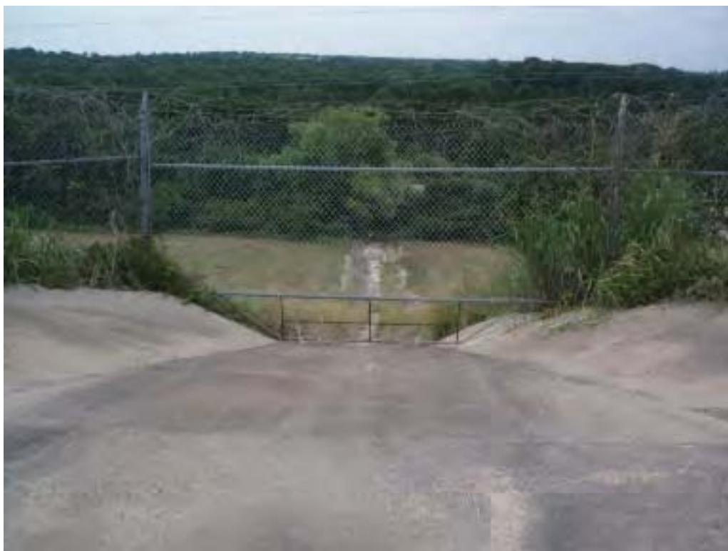
Photo No. 74: CADP - East embankment, looking south at stormwater control section outlet from capped portion of the impoundment.
