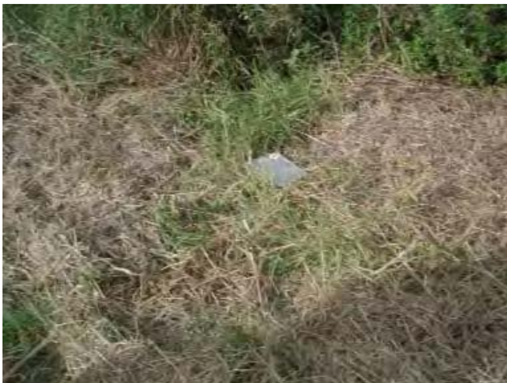
Photo No. 84: CADP - South embankment exterior slope, looking at 2'Wx4'Lx1'D depression at toe of slope. Possible collapsed rodent burrow.
