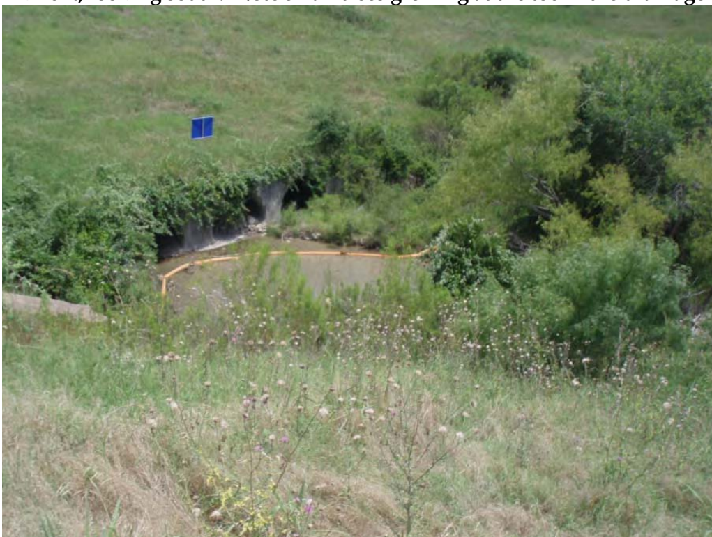
Photo No. 42: Reclaim Pond - Overview of triple arch culverts under railroad embankment. Note small trees and vegetation in the drainage ditch and debris in the arch culverts.
