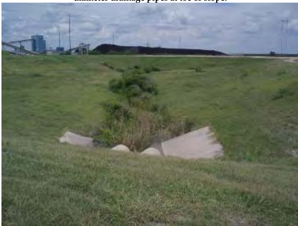
Photo No. 38: Reclaim Pond - Overview of north embankment exterior slope and downstream area, looking east. Note small trees and brush at the bottom of the slope growing in the drainage ditch.
