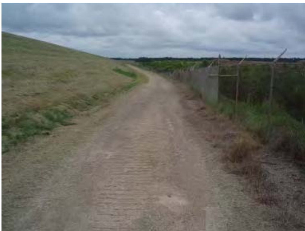
Photo No. 100: CADP - North embankment crest, looking east. Note trees growing inside the fence limits. Trees are in the area of the toe of the Cedar Creek Dam.
