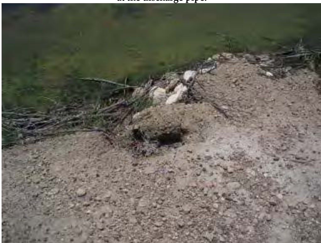
Photo No. 22: Reclaim Pond - East embankment interior slope, looking at 2.5'W erosion rill.
