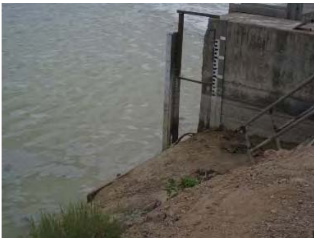
Photo No. 92: CADP - West embankment interior slope, looking at staff gage on intake structure.
