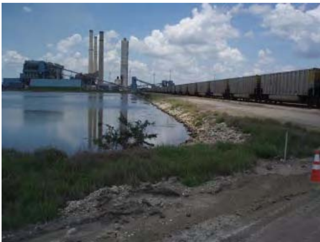
Photo No. 18: Reclaim Pond – East embankment interior slope, looking north. Small woody growth and minor surface erosion noted.
