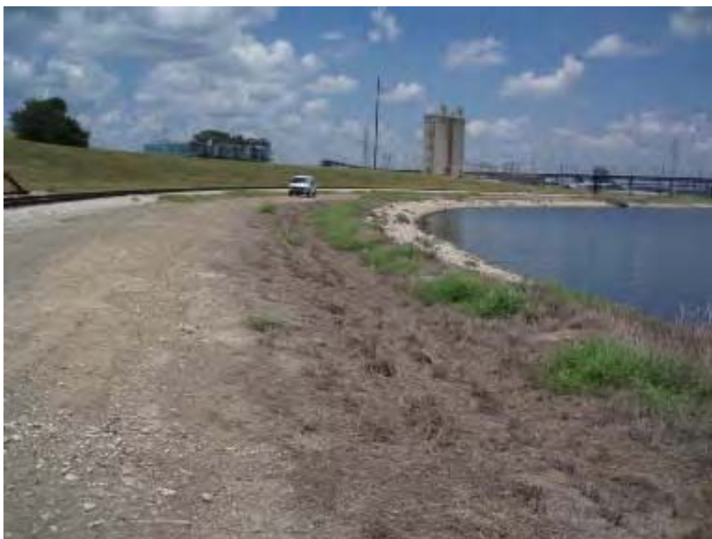
Photo No. 16: Reclaim Pond - South embankment, looking northwest at a low area on the crest
