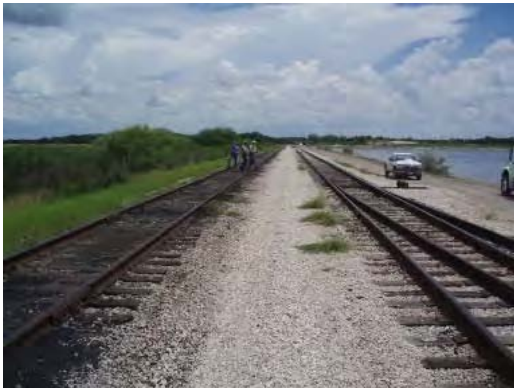
Photo No. 45: Reclaim Pond - East embankment crest, looking south. Note crest has two railroad spurs and an access road.
