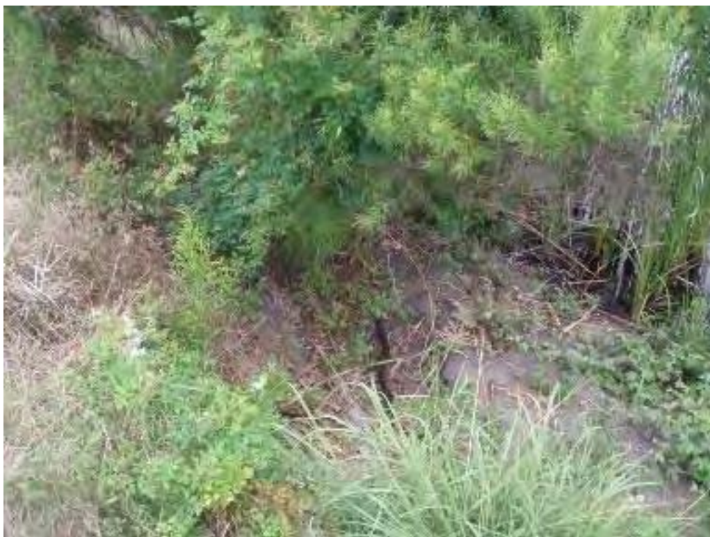
Photo No. 80: CADP - South embankment exterior slope, looking at 4'Wx5'Lx2'D depression at toe of slope. Possible collapsed rodent burrow.
