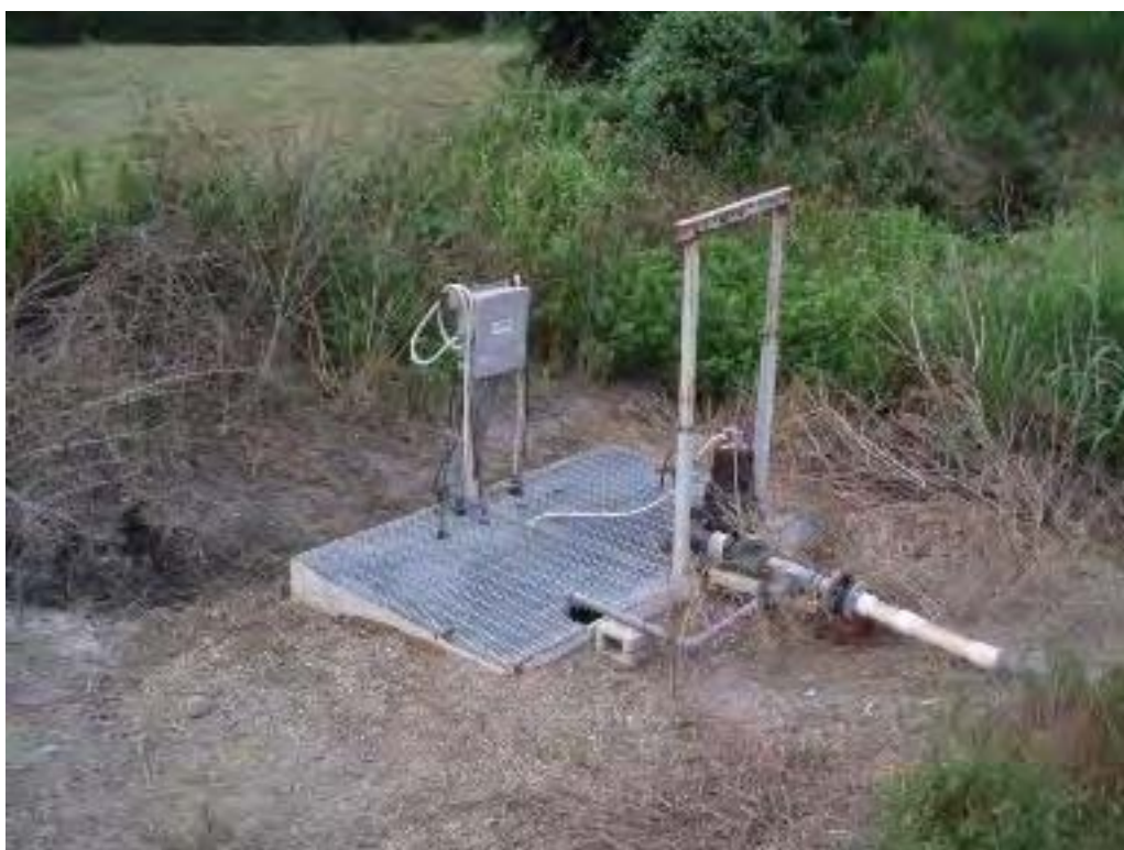
Photo No. 66: CADP - East embankment exterior slope, looking at toe drain seepage collection sump pit. Seepage water from the toe drain is pumped back to the impoundment.
