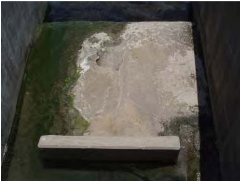
Photo No. 9: Reclaim Pond – Overview of stormwater outlet structure on west embankment interior slope. Stormwater is from FGD residue silos and truck wash area.
