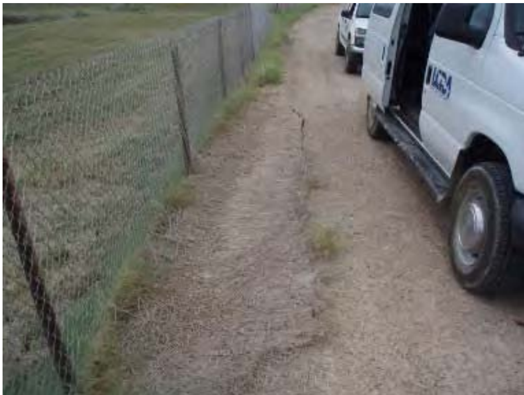
Photo No. 99: CADP - North embankment crest, looking at tension crack in road base fill.
