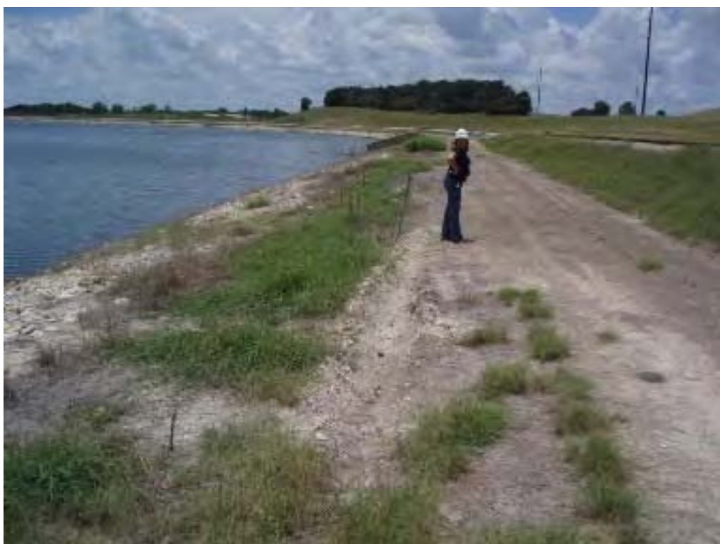
Photo No. 8: Reclaim Pond - West embankment, looking south at typical bare spots and tractor ruts on crest and interior slope.
