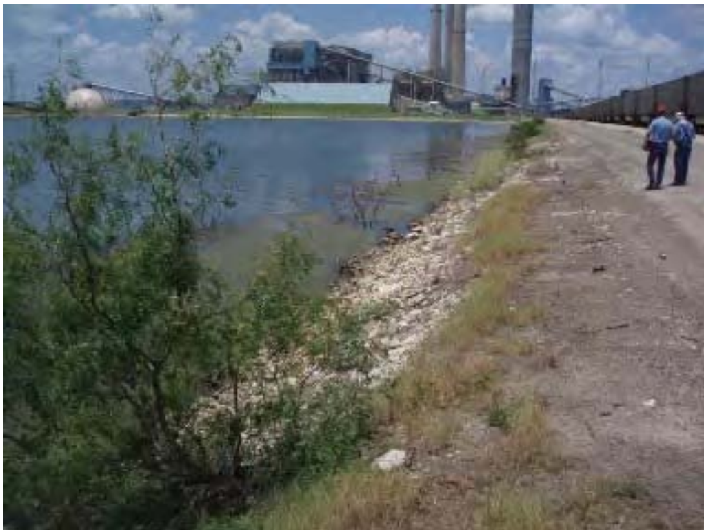
Photo No. 19: Reclaim Pond - East embankment interior slope, looking at a 4-inch-diameter mesquite tree and brush. Note some minor surface erosion near crest.
