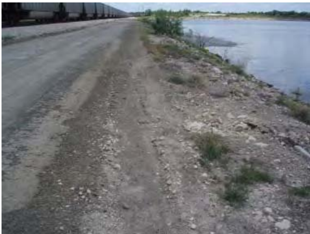
Photo No. 20: Reclaim Pond - East embankment interior slope, looking south at rutting and surface erosion. Note some riprap is missing and displaced.
