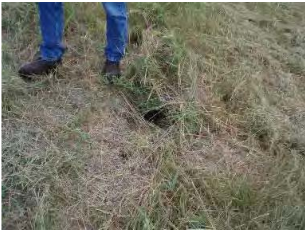
Photo No. 63: CADP - East embankment exterior slope, looking at a 6-inch-diameter rodent hole.
