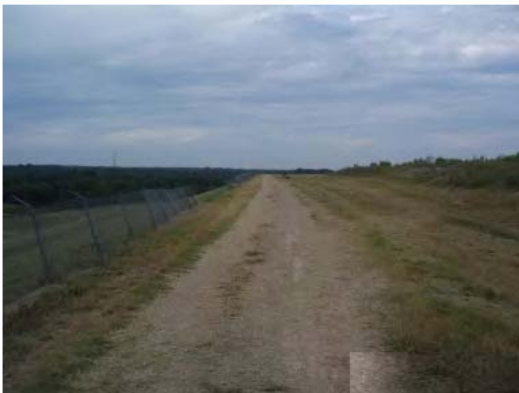
Photo No. 56: CADP - East embankment crest, looking south. Note the fence has been pushed over from raising the crest 2 feet.
