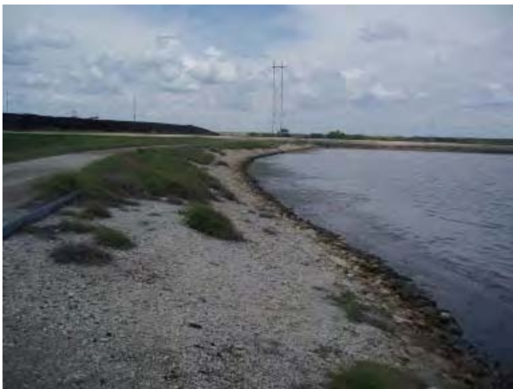
Photo No. 36: Reclaim Pond - North embankment interior Slope, looking east. Note 6-inch-diameter HDPE pipe from the CADP on left side of photo.
