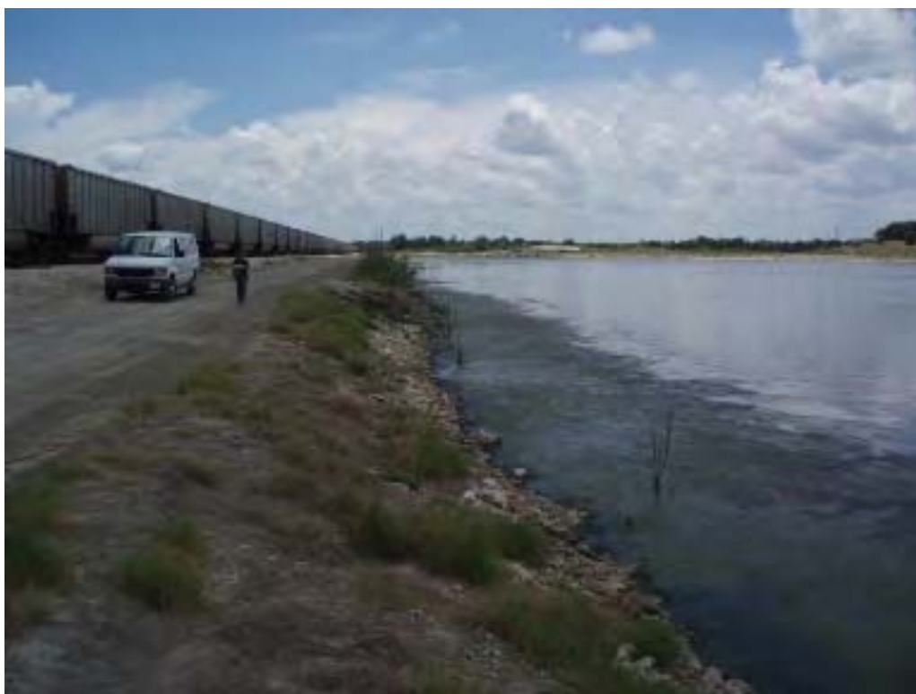
Photo No. 24: Reclaim Pond - East embankment interior slope, looking south. Note occasional mesquite trees growing on interior slope.
