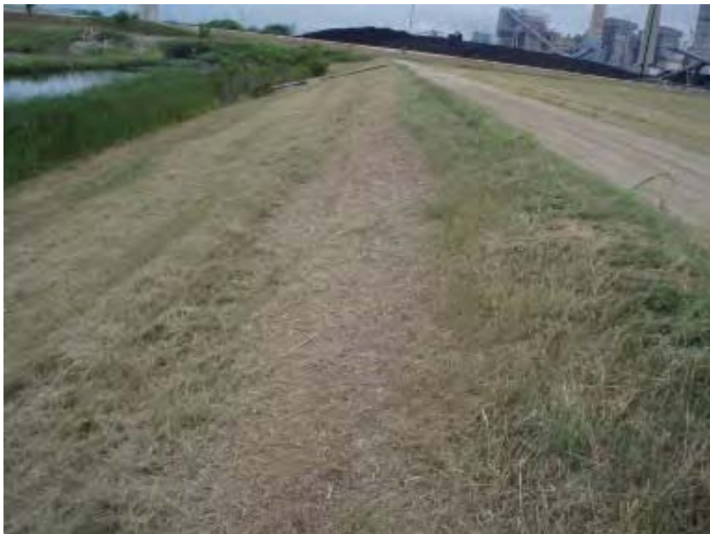
Photo No. 81: CADP - South embankment exterior slope, looking west. Note sparse vegetation near crest.
