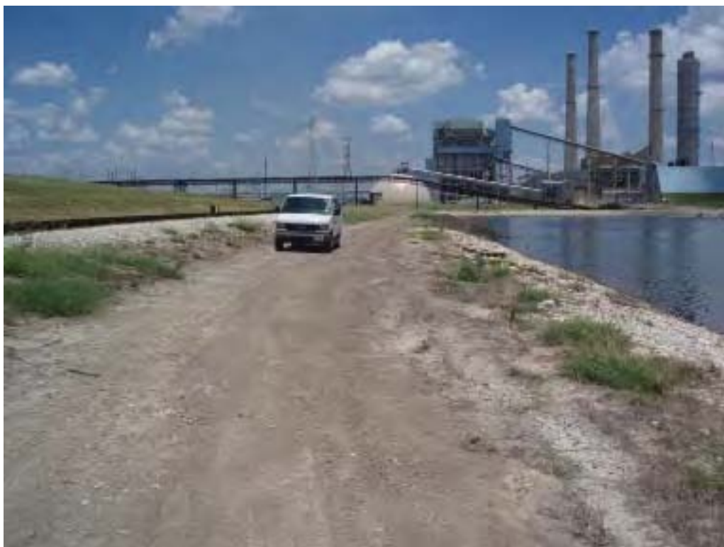
Photo No. 10: Reclaim Pond – West embankment crest, looking north at typical surface erosion and rutting.
