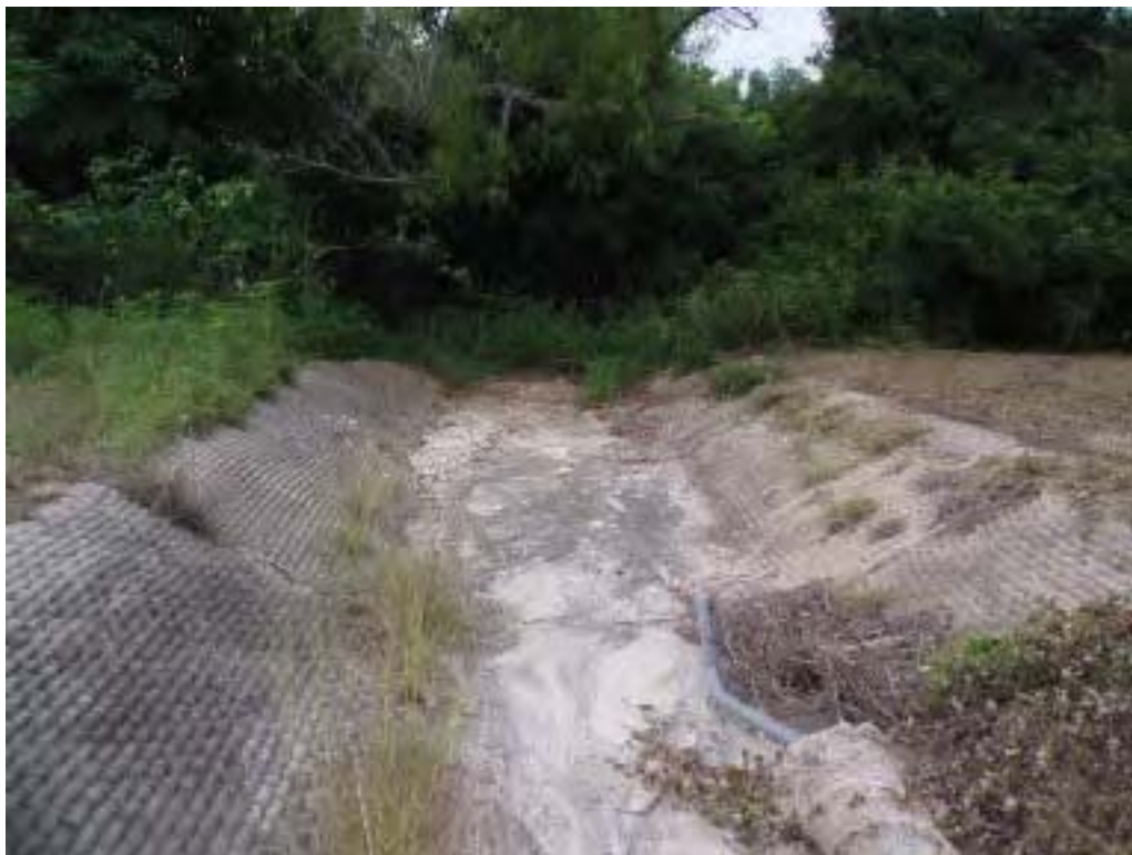
Photo No. 69: CADP - East embankment exterior slope, looking south at stormwater discharge channel from capped portion of the impoundment.
