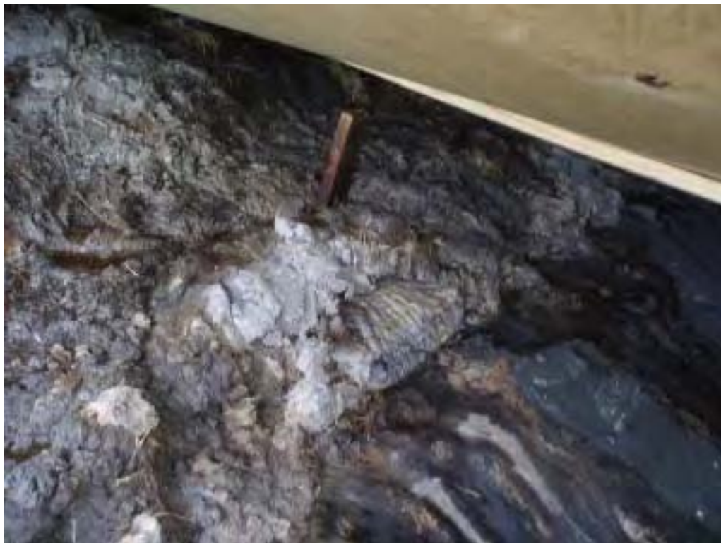
Photo No. 83: CADP - South embankment exterior slope, looking at seep. Note liner down slope of seep to collect water. Flow ~8 gallons per day.
