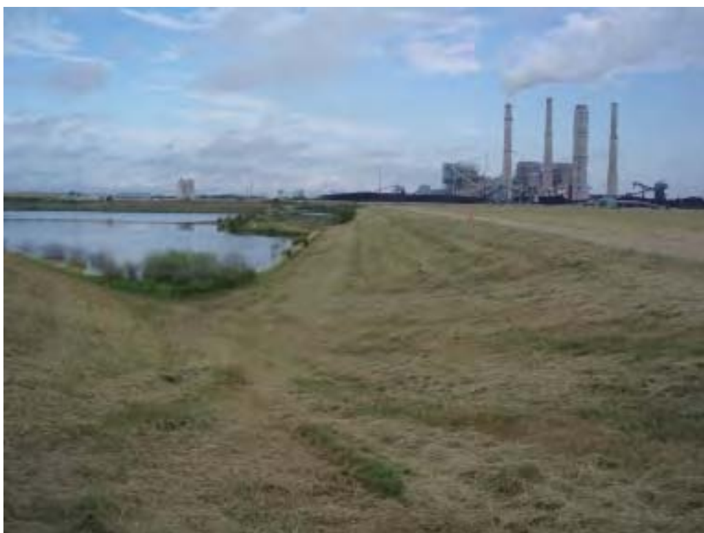
Photo No. 76: CADP - Groin of south embankment exterior slope and Coal Pile Run-off Pond interior slope, looking west. Note water, brush and small trees at toe of slope.
