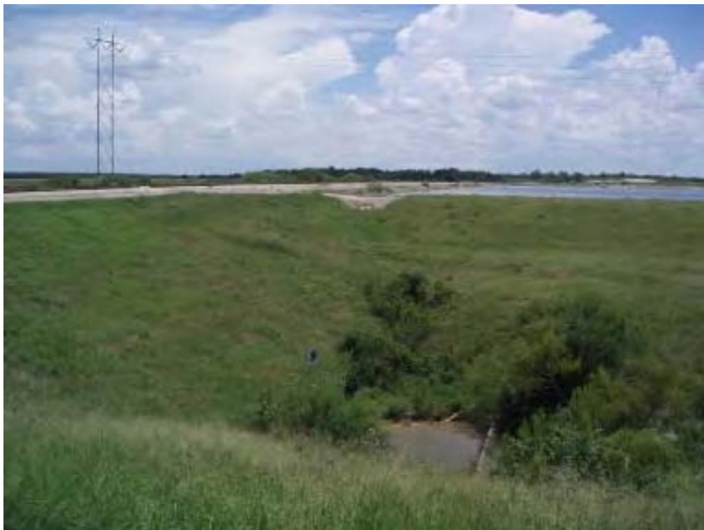
Photo No. 41: Reclaim Pond - Overview of north embankment spillway and railroad embankment, looking south. Note small trees growing at the toe in the drainage ditch.
