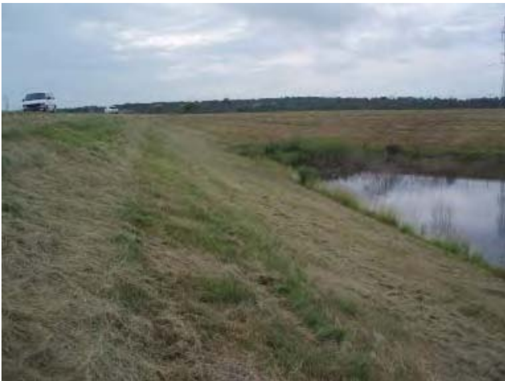
Photo No. 77: CADP - South embankment exterior slope, looking east at groin with Coal Pile Run-off Pond. Note water, brush and small trees at toe of slope.
