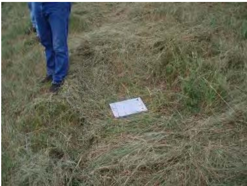
Photo No. 62: CADP - East embankment exterior slope, looking at 3'Wx3'Lx1'D depression. Possible collapsed rodent burrow.
