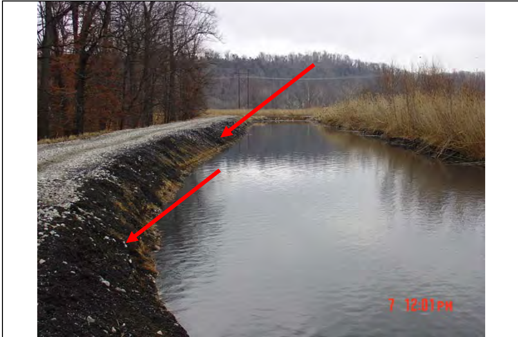
Photo #7: Interior slope west embankment, area needs erosion protection, looking north
