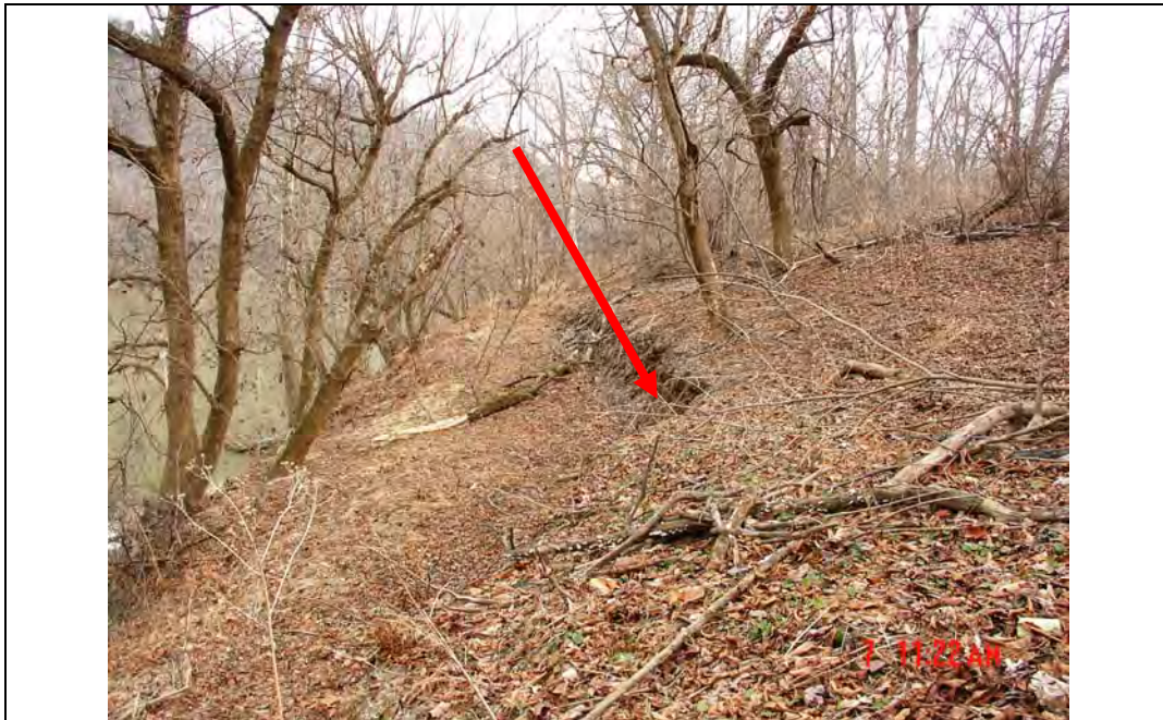
Photo #8: Slope scarp above cooling water canal, below toe of pond embankment, looking north
