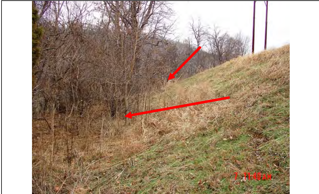
Photo #9: Woody vegetation at toe of embankment slope, west exterior slope, looking north
