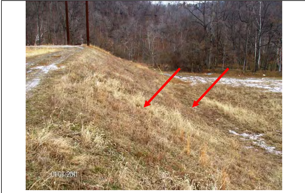
Photo #3: North Exterior slope, looking west Note: erosion gullies and steep slope at toe
