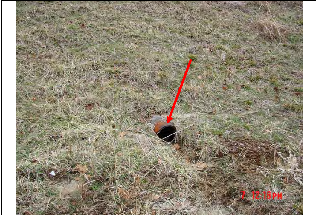
Photo #13: Steel pipe penetrating north embankment slope at toe of east side of pond, looking south
