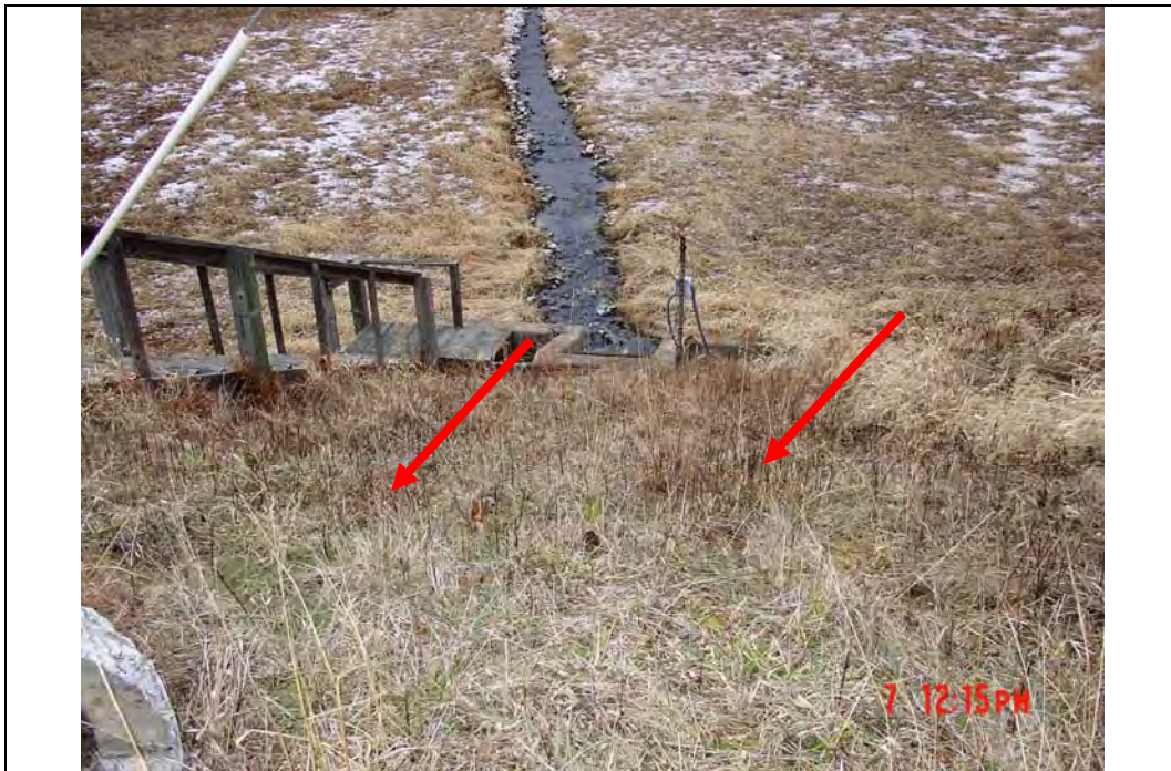
Photo #4: Erosion gullies north exterior slope at spillway, looking north
