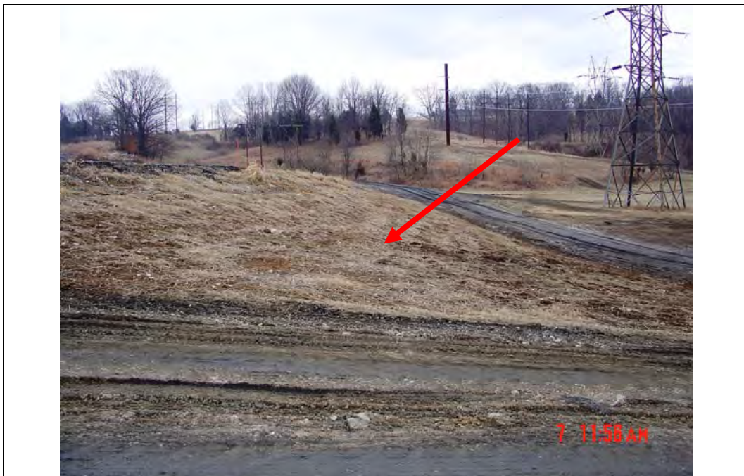
Photo #6: South exterior slope at recent repair, area needs vegetation established, looking east
