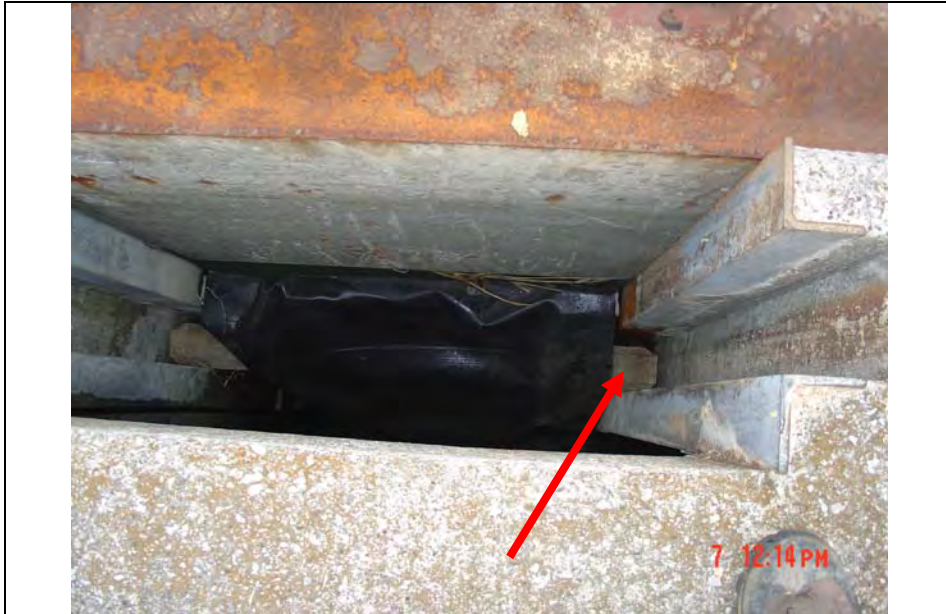
Photo #1: Stop logs in main spillway, no maximum placement elevation noted on spillway inlet
