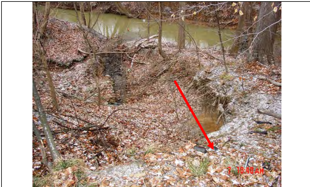
Photo #12: Ravine below south end of pond above cooling canal. Note: Erosion and water seepage, looking west
