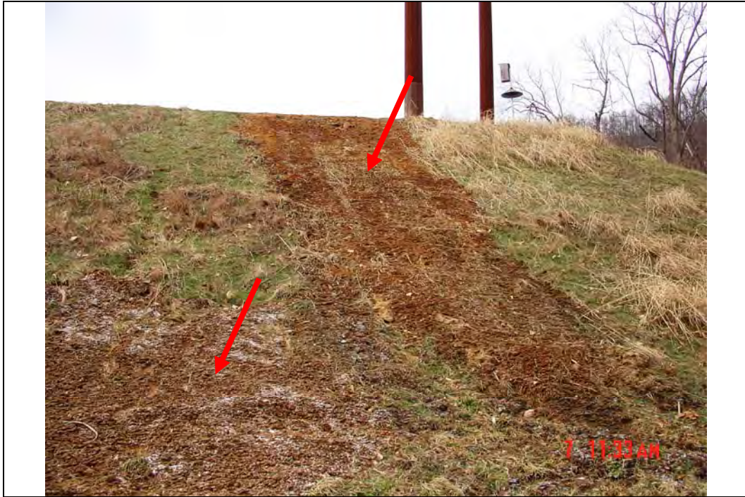
Photo #5: Exterior slope area needing revegetation looking southwest
