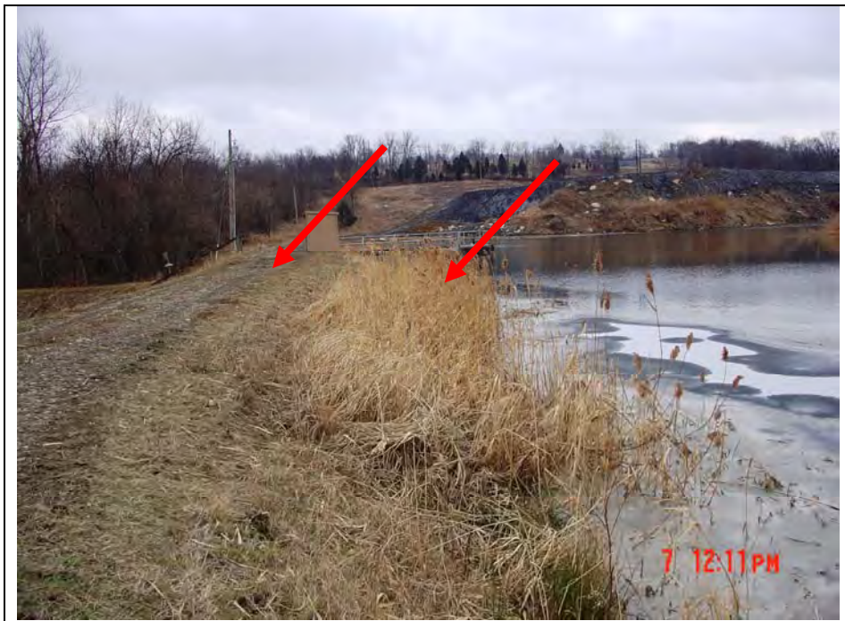
Photo #2: Vegetation on north embankment upstream slope, low elevation areas on dam crest, looking south
