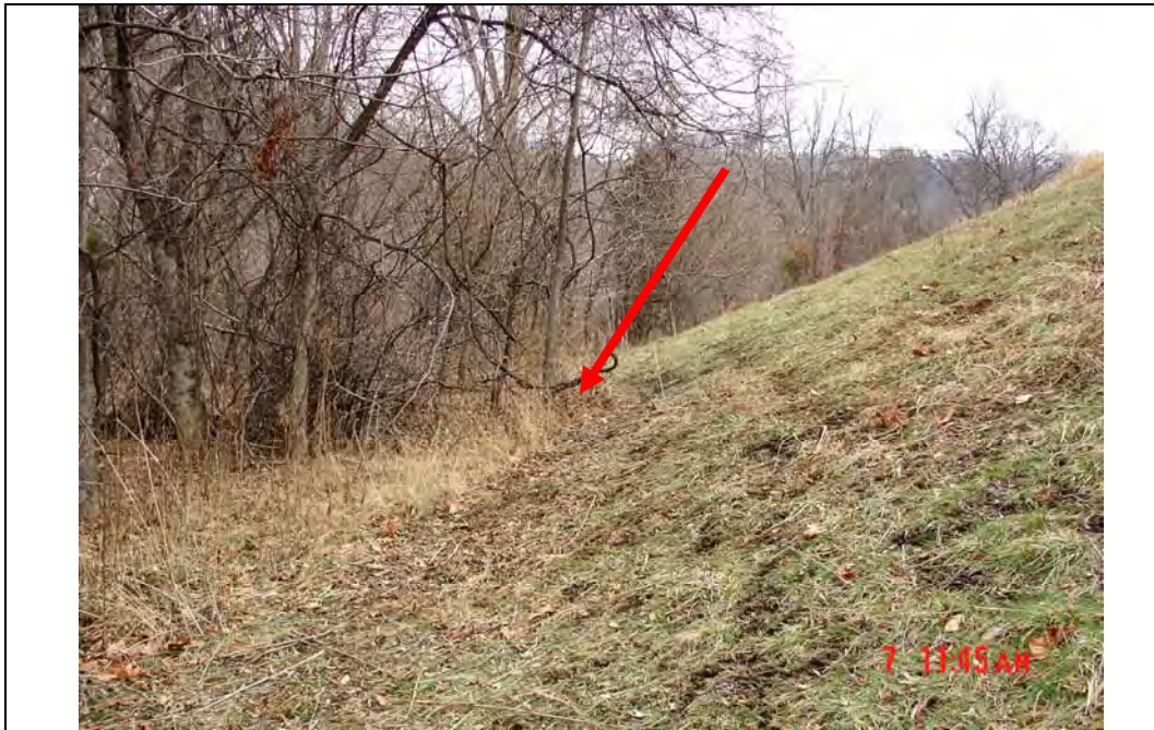
Photo #10: Woody vegetation at toe of embankment slope, west exterior slope, looking north
