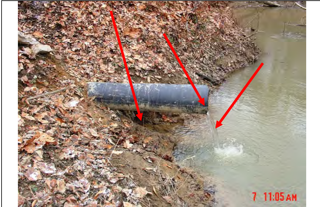
Photo #11: New pipe installed at cooling water canal Note: Seepage and erosion below pipe, looking south
