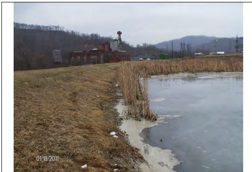
Photo #4: Interior slope, west embankment, looking north
