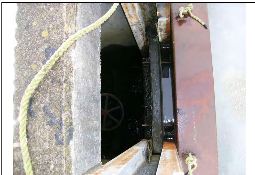
Photo #3: Principal Spillway inlet
