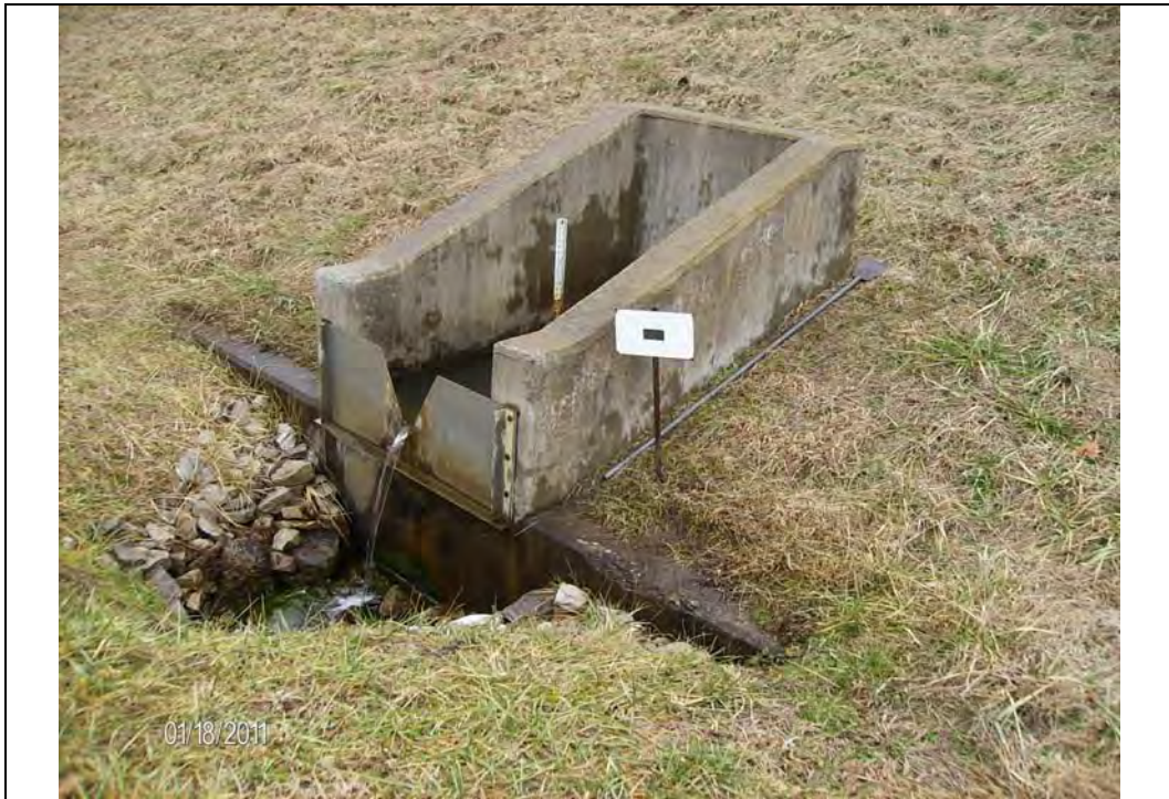
Photo #7: Principal spillway outlet, looking northwest
