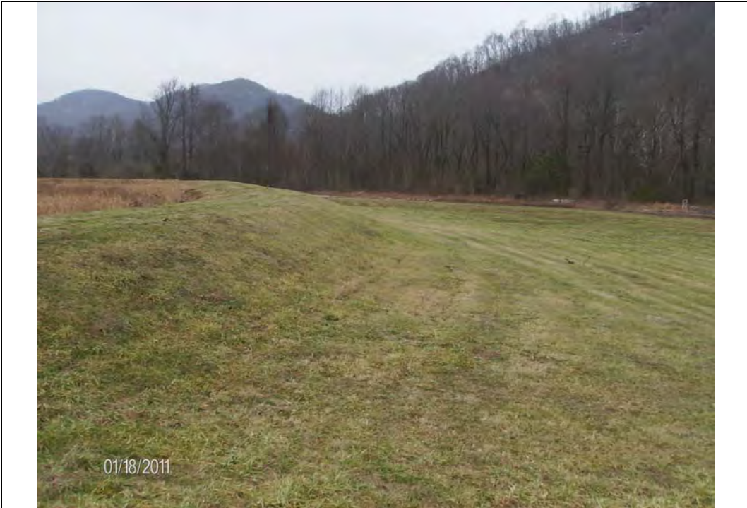
Photo #10: Exterior slope and toe of west embankment, looking south
