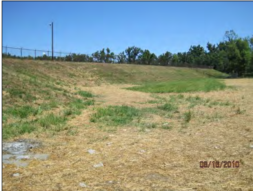
LOOKING E AT DOWNSTREAM SLOPE OF SOUTH DIKE, WET AREA BELOW TOE, STEEP SLOPE, SPARSE GRASS
