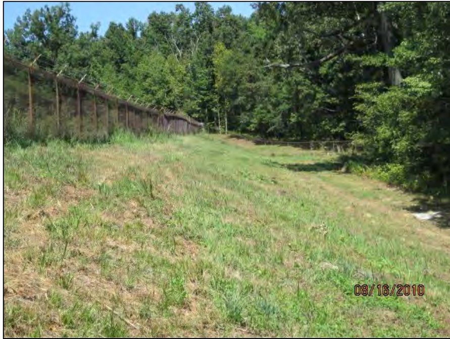
LOOKING N AT DOWNSTREAM SLOPE EAST DIKE, STEEP SLOPE, AREAS OF SPARSE GRASS, TIE INTO ORIGINAL IN BACKGROUND
