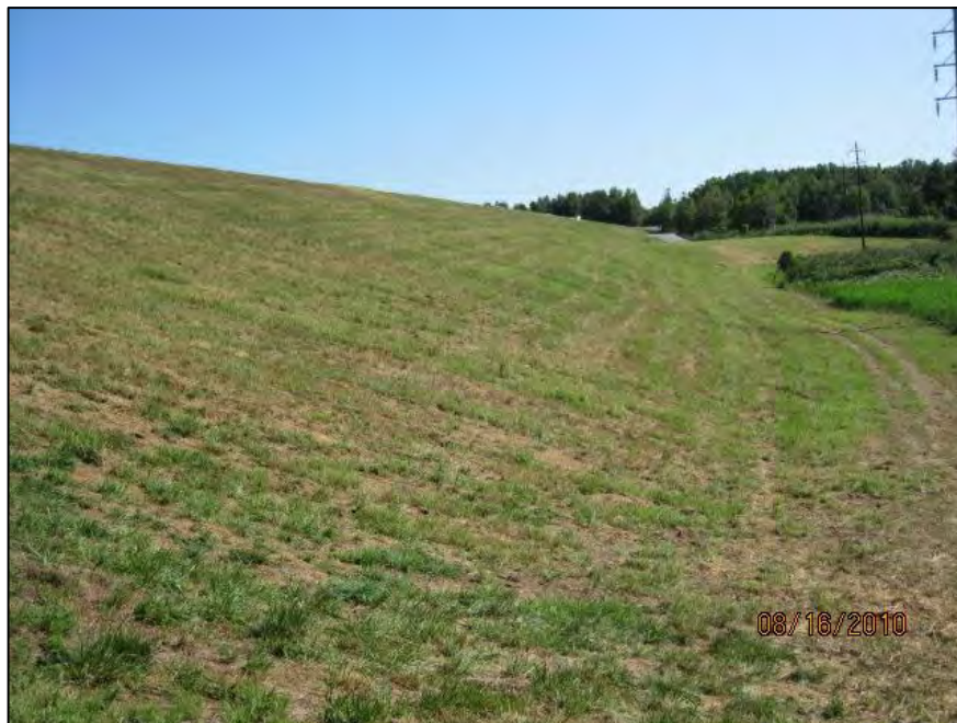
LOOKING EAST ON SOUTH DIKE, UNEVEN SLOPES AND SPARSE GRASS ON DOWNSTREAM SLOPE FROM WEST BUTTRESS TO ABOUT 300 FEET EAST
