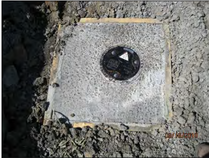
2-5 NEW PZ ON ROAD, SOUTH DIKE
