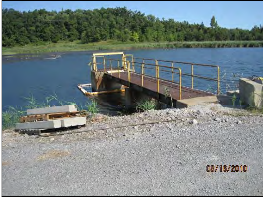
LOOKING NE AT OUTLET STRUCTURE, PERIMETER SKIMMER AND POND INTERIOR TO NATURAL HILLSIDE IN BACKGROUND, STACK OF CONCRETE STOP LOGS IN FOREGROUND
