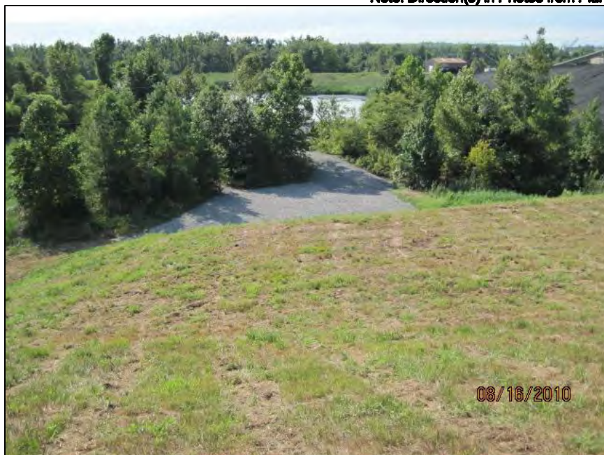
LOOKING S FROM SOUTH DIKE - AREAS WITH SPARSE GRASS ON DOWNSTREAM CREST, WEST BUTTRESS, AND COAL RUNOFF POND IN BACKGROUND
