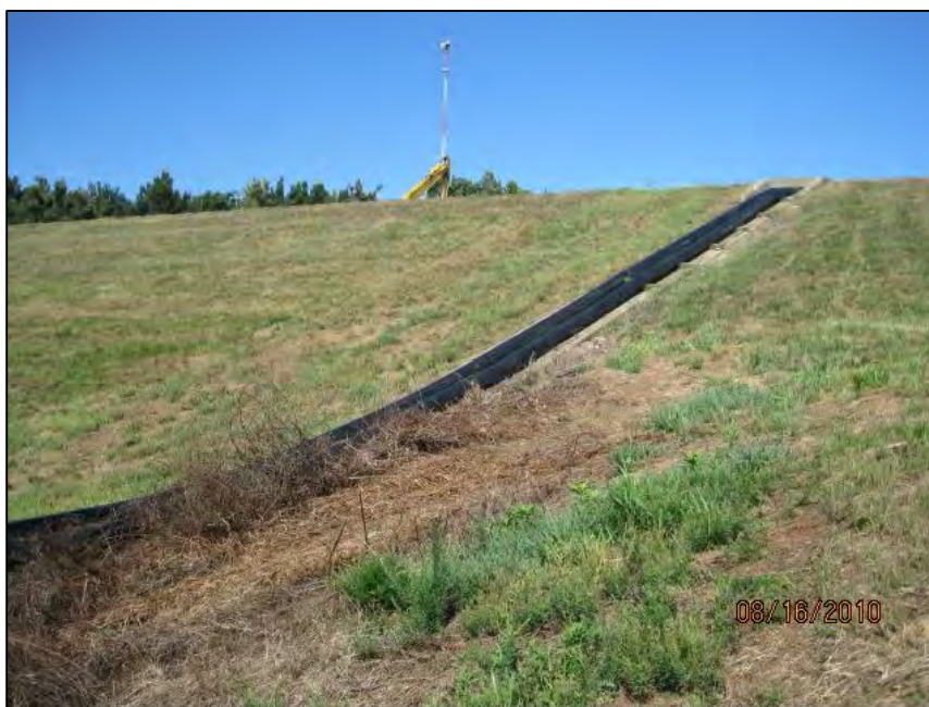
M-25 LOOKING NW AT SLUICE PIPES ON SOUTH DIKE
