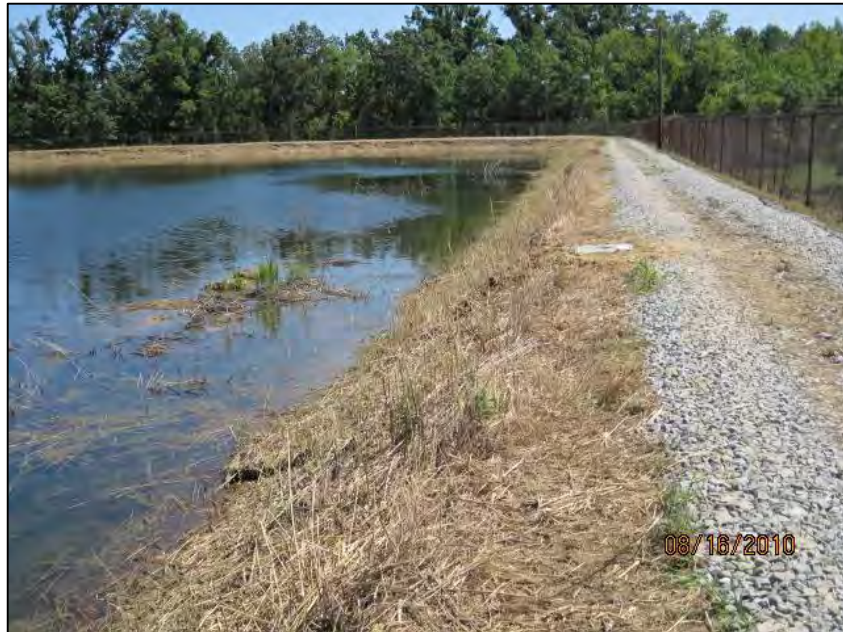
LOOKING E AT CREST AND UPSTREAM SLOPE OF SOUTH DIKE, NEW PZ IN CREST, AREAS WITH UNEVEN TO NEAR VERTICAL SLOPES ON UPSTREAM SLOPE ON SOUTH AND EAST DIKE
