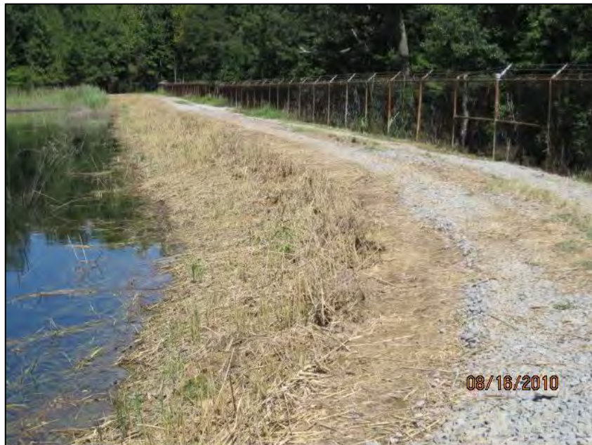
LOOKING N FROM SOUTHEAST CORNER AT CREST AND UPSTREAM SLOPE OF EAST DIKE, AREAS WITH UNEVEN TO NEAR VERTICAL SLOPES ON UPSTREAM SLOPE
