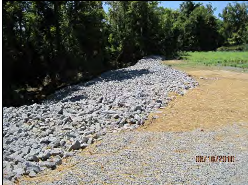
REGRADED AND RIP-RAP ARMORED SOUTH AND ONLY DIKE OF ASH POND 3
