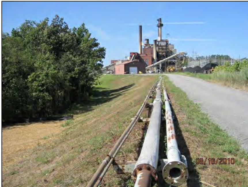
LOOKING W AT SOUTH DIKE (ROAD), EROSION, SPARSE GRASS, STEEP SLOPE
