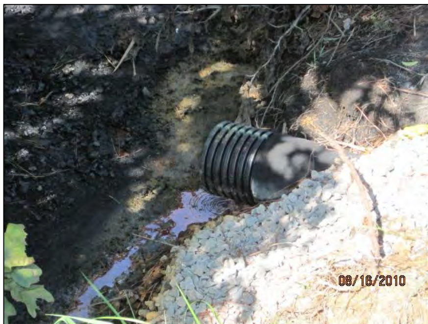
TOE DRAIN OUTLET FOR WEST BUTTRESS ON SOUTH DIKE
