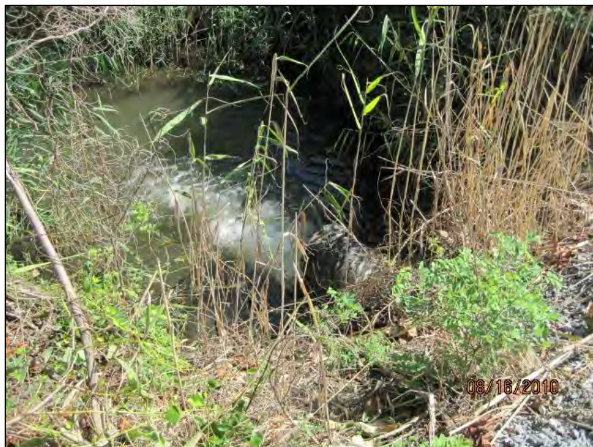
CR-8 CMP PIPE OUTLET TO ASH POND 2
