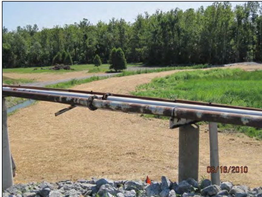
2-6 LOOKING SE FROM SOUTHEAST CORNER OF POND, ELEVATED PIPE LINES TO SCRUBBER POND, SITE DISCHARGE DITCH ON LEFT, PORTION OF FORMER ASH POND 3 ON RIGHT
