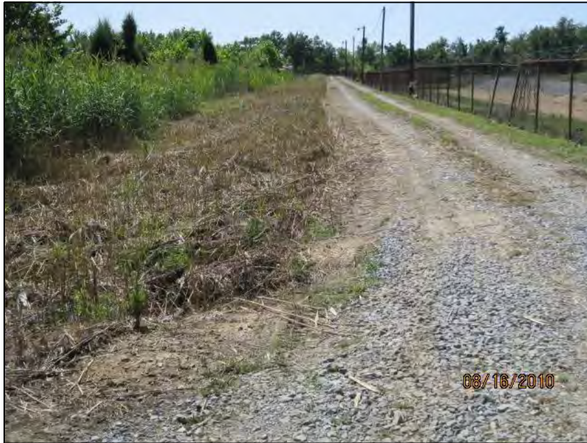
LOOKING S AT CREST AND UPSTREAM SLOPE OF WEST DIKE, HEIGHT OF INTERIOR AREAS OF ASH UP TO WITHIN 1-FOOT OF CREST
