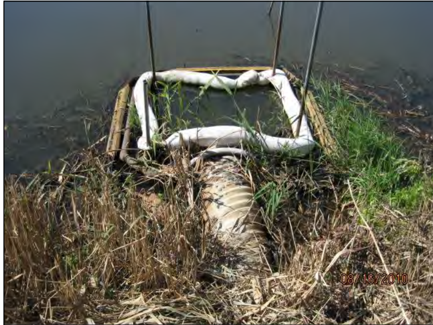
CR-7 METAL AND BOOM SKIMMER AND CMP PIPE INLET AT NORTH END OF EAST DIKE
