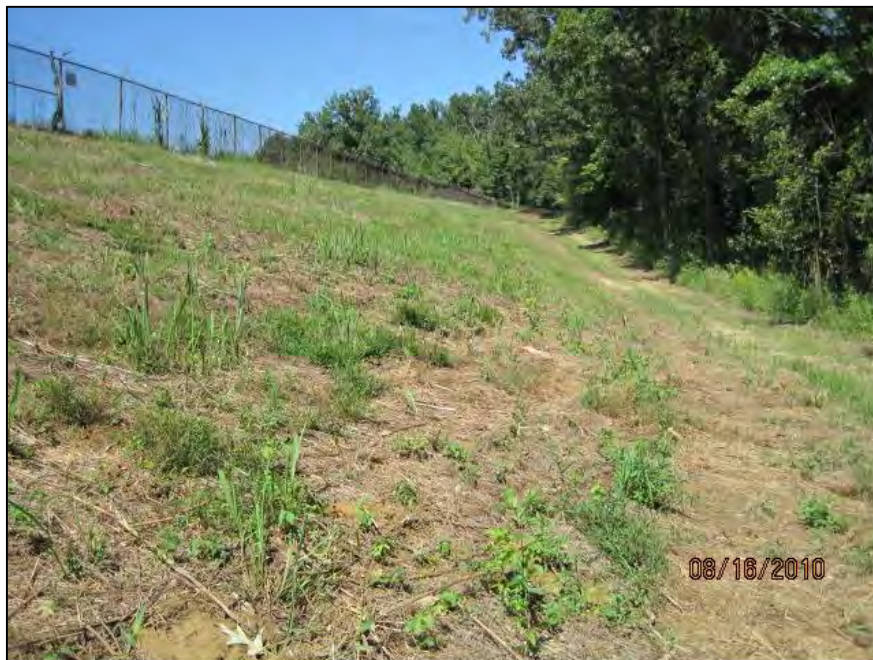
LOOKING NE AT DOWNSTREAM SLOPE OF SOUTH DIKE, STEEP SLOPE, SPARSE GRASS
