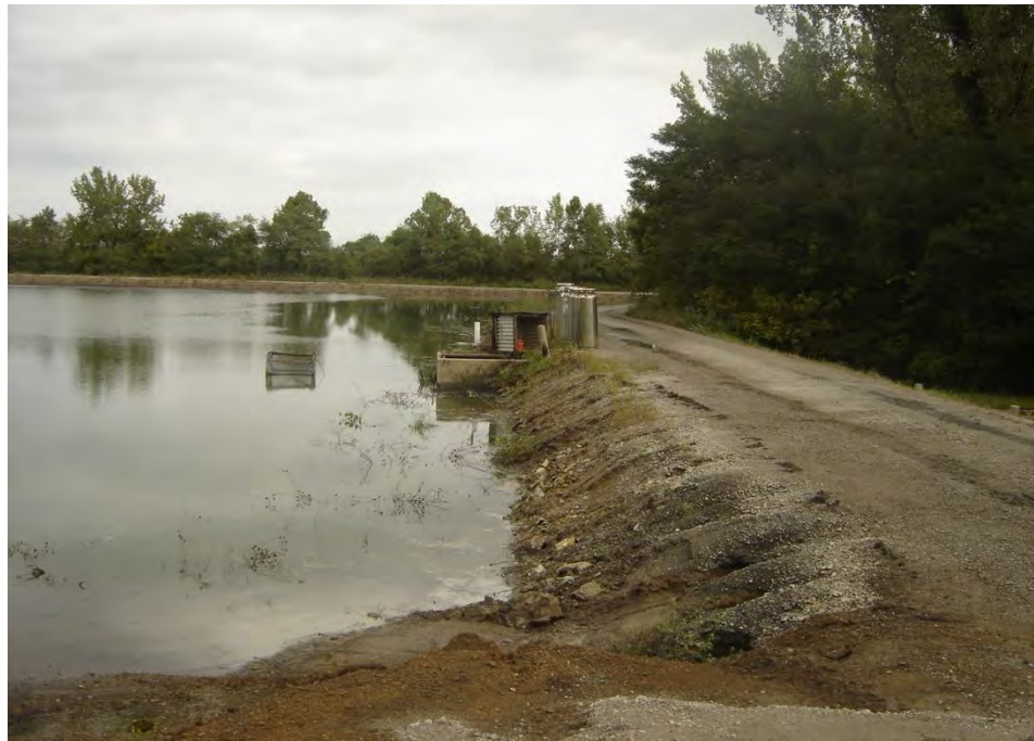
Figure 5.6.1-1. Main Outlet Structure.
