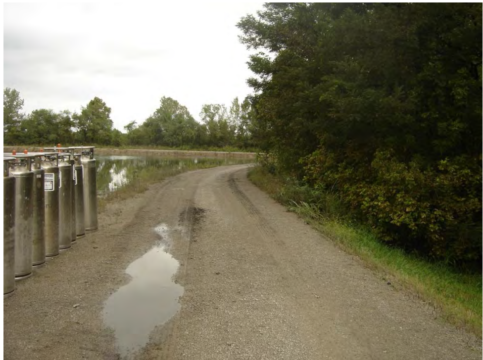
Figure 5.3.1-1. East Dike Crest
