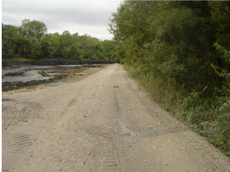
Figure 5.4.1-1. Crest of North Dike
