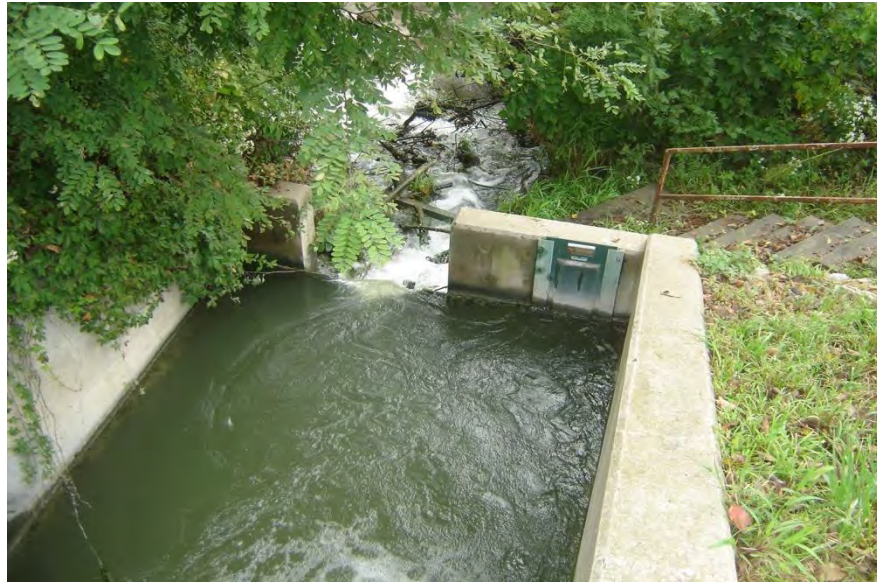
Figure 5.6.2-1. Main Spillway Outfall.
