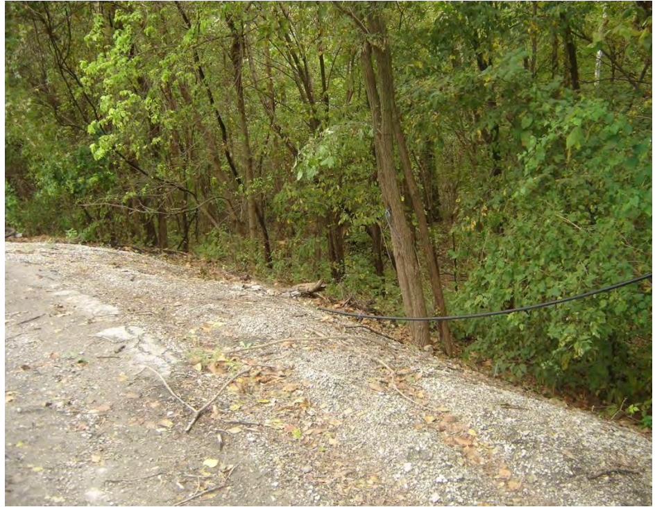
Figure 5.5.1-1. Crest of West Dike
