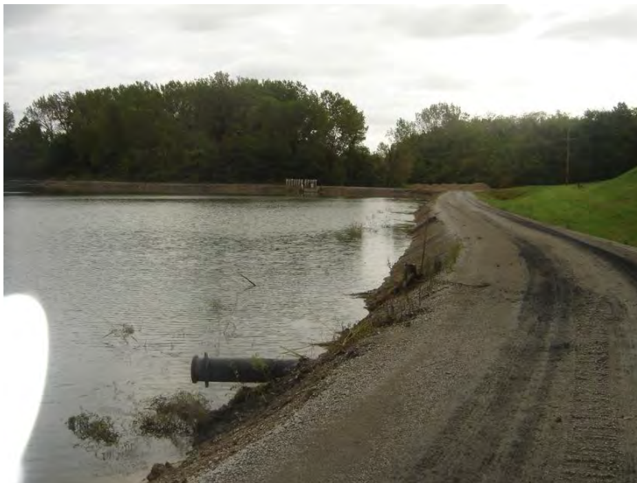
Figure 5.2.1-1. Photo Showing Crest/ inside slope of South Dike.
