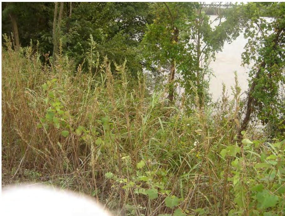
Figure 5.4.3-1. Outside Slope of North Dike.
