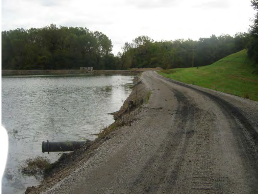
9. South Dike Inlet
