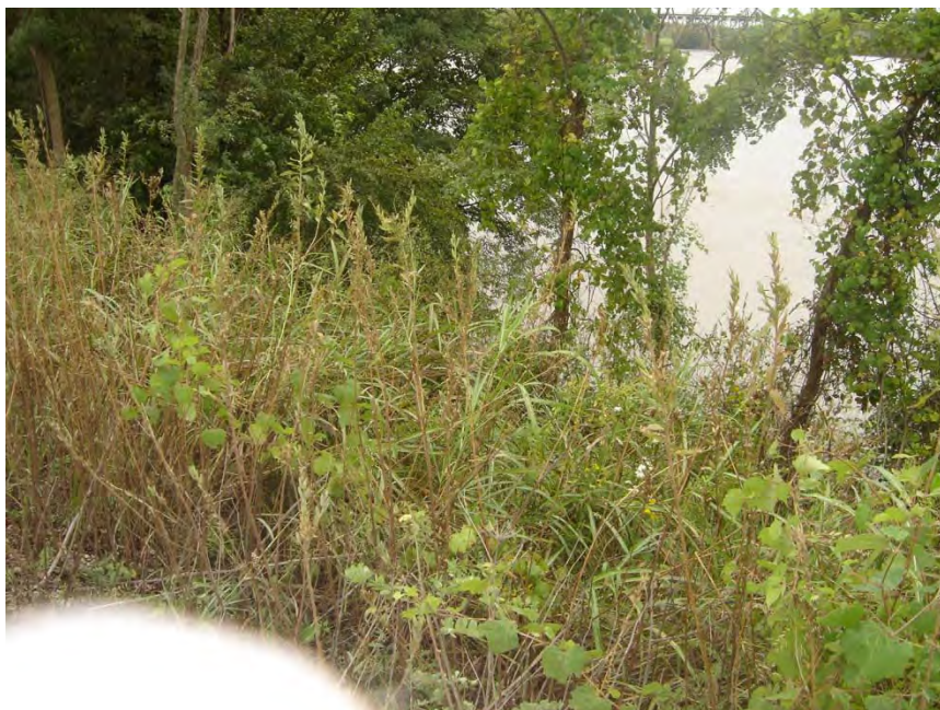
17. North Dike Outside Toe
