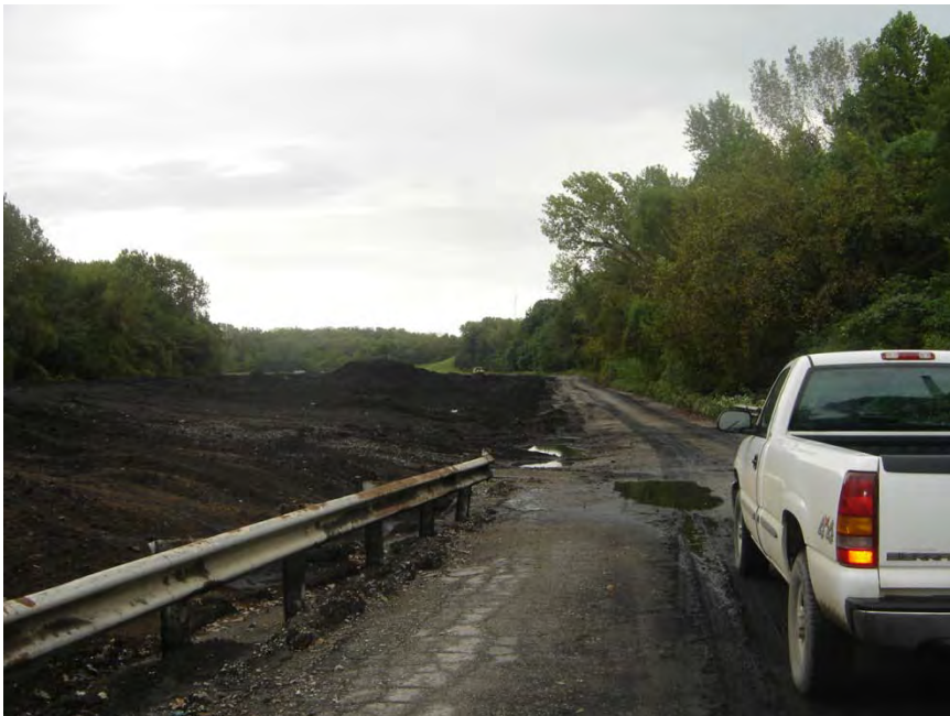
2. South Dike Crest
