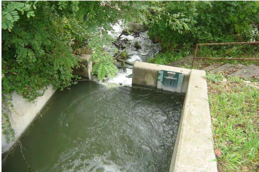
Figure 5.6.2-1. Main Spillway Outfall.
