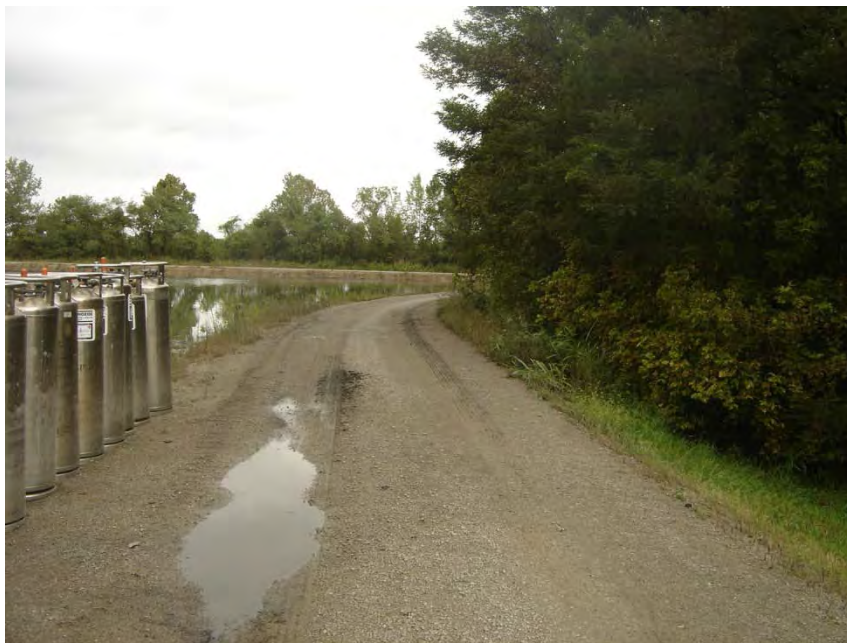
14. East Dike Crest
