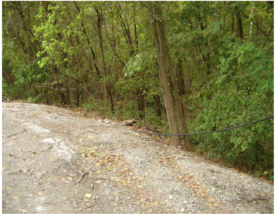
Figure 5.5.1-1. Crest of West Dike
