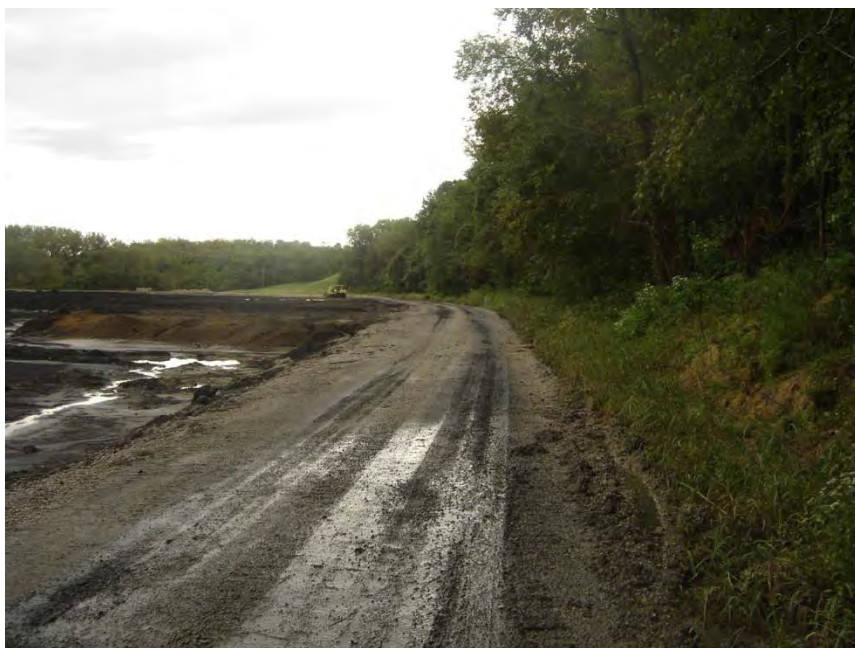
6. South Dike Looking Downstream
