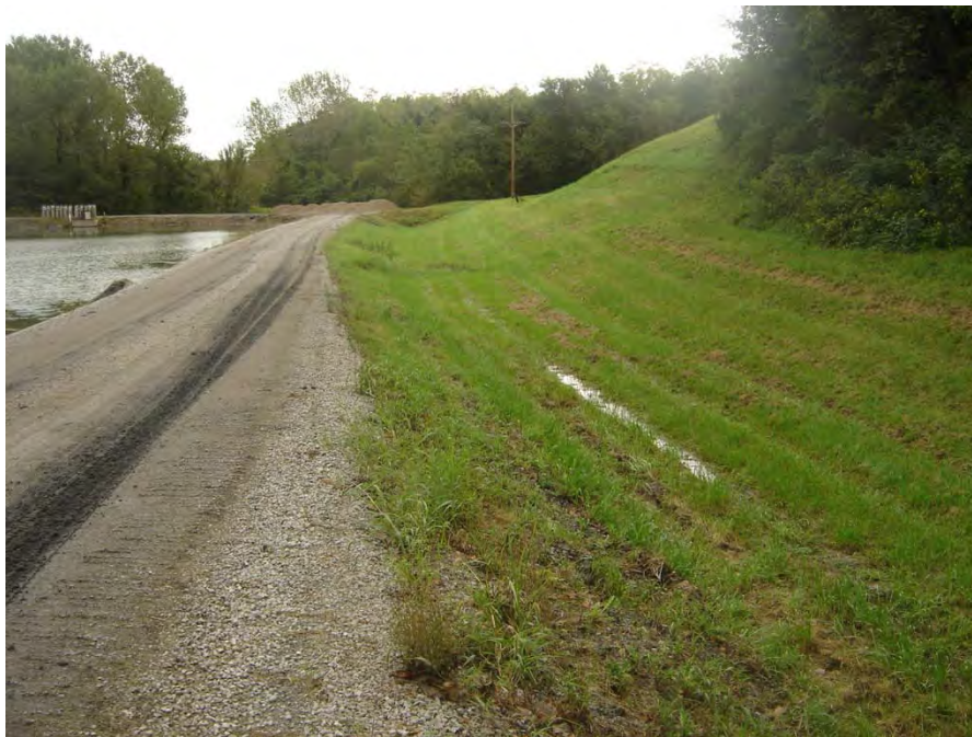
10. South Dike Outside Toe
