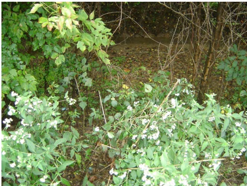
3. South Dike Outside Toe
