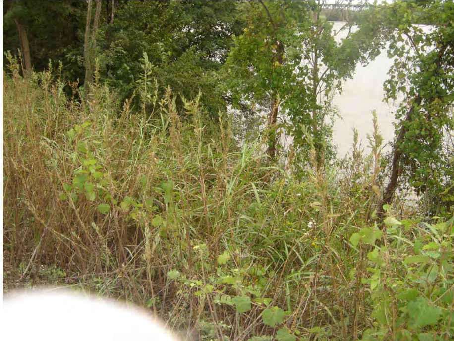
Figure 5.4.3-1. Outside Slope of North Dike.
