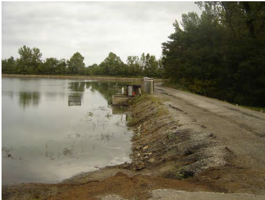
11. East Dike Outfall
