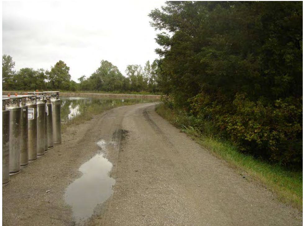
Figure 5.3.1-1. East Dike Crest
