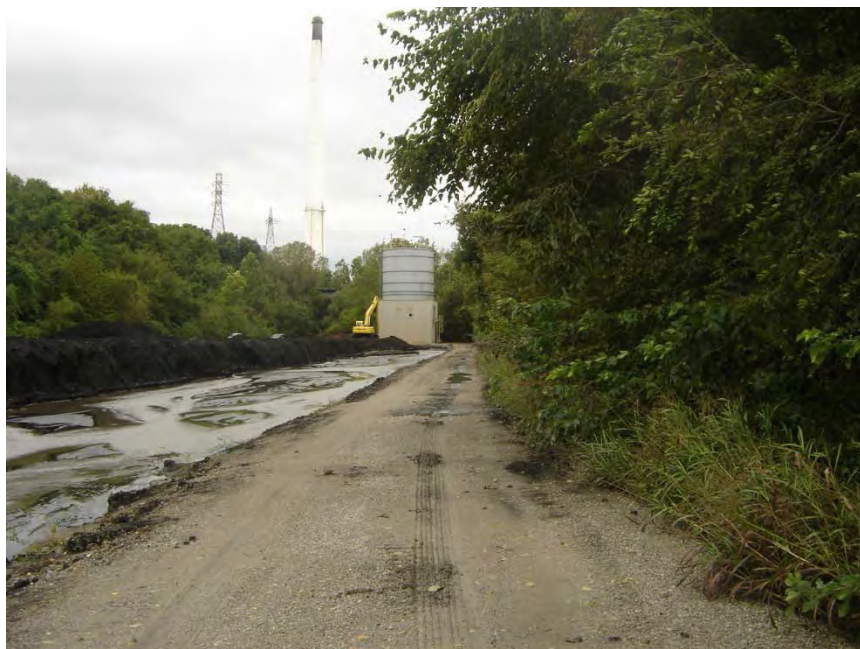
19. North Dike Crest
