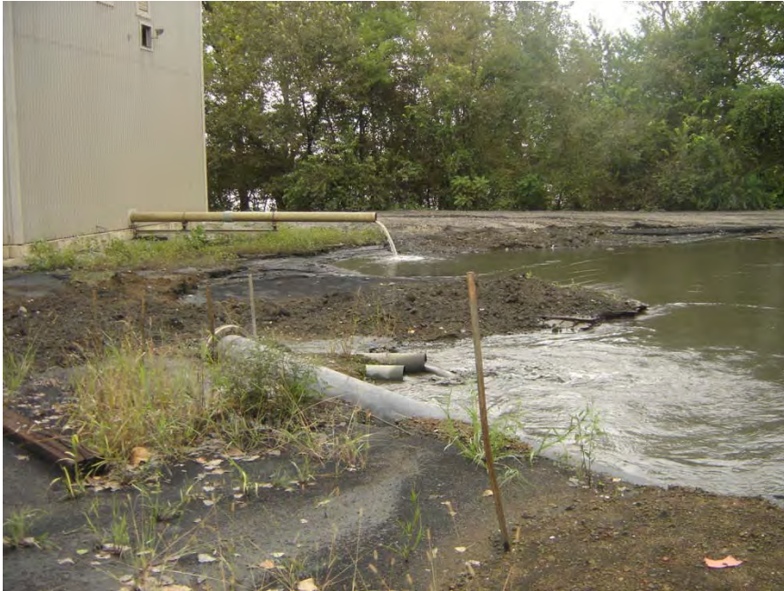
1. Fly Ash Outfall
