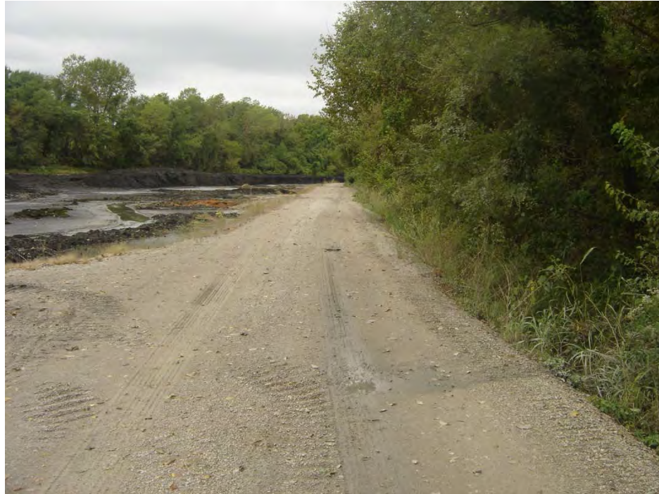
Figure 5.4.1-1. Crest of North Dike
