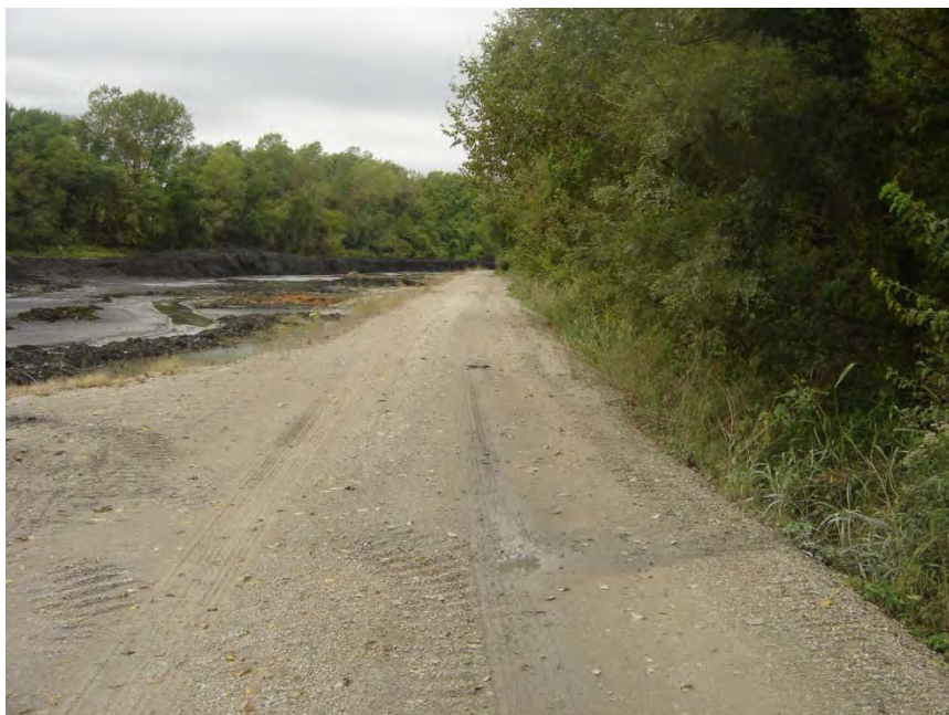
18. North Dike Crest
