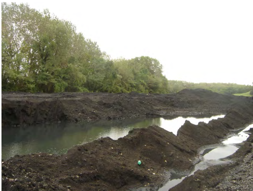
4. South Dike Inside Toe
