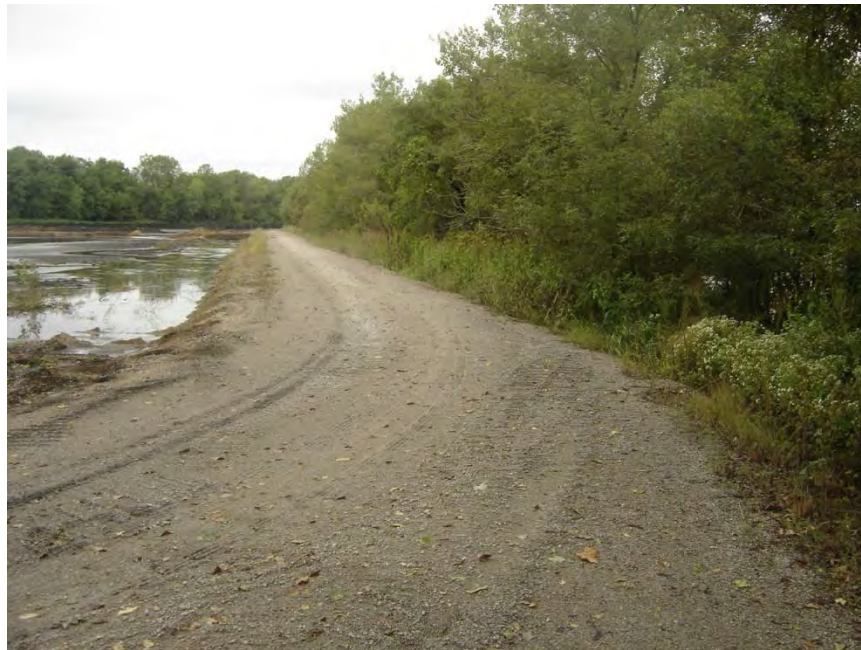
Figure 5.3.3-1. Photo Showing Typical Condition of Outside Slope of East Dike
