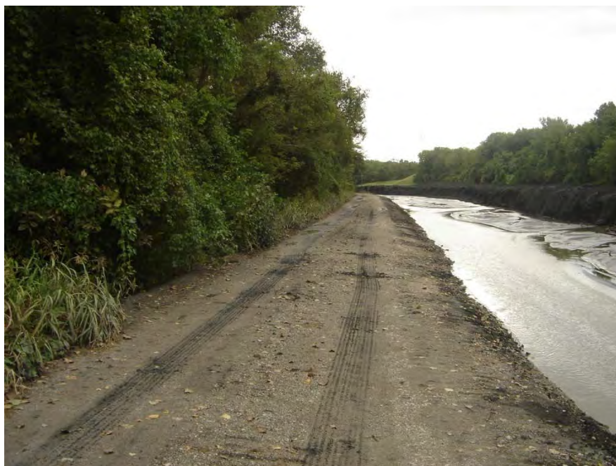
21. North Dike Crest Looking Upstream
