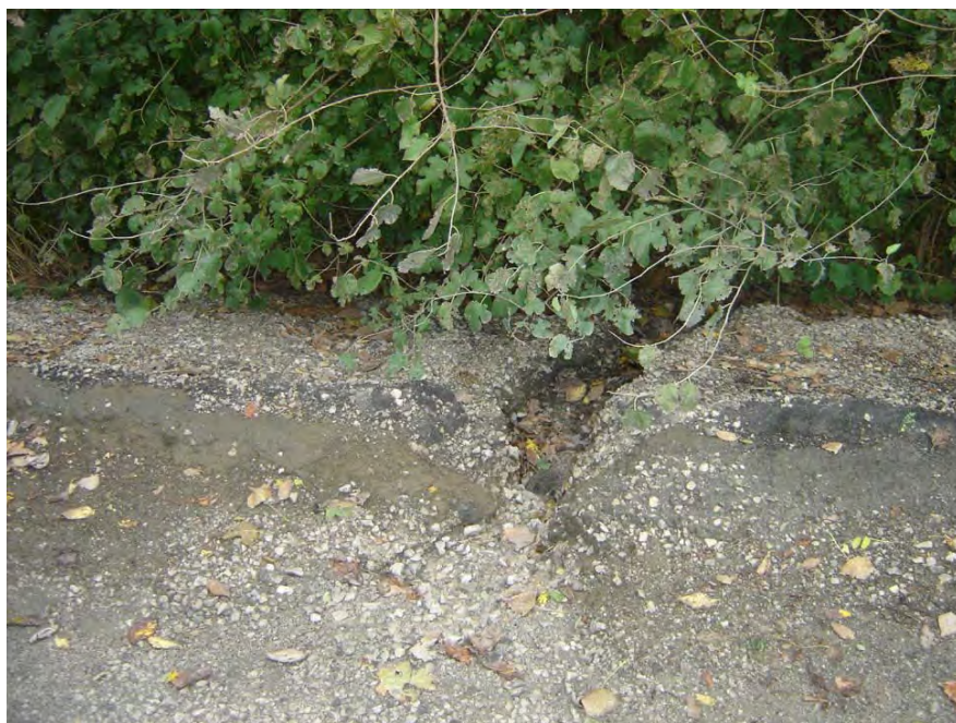
22. North Dike Outside Toe
