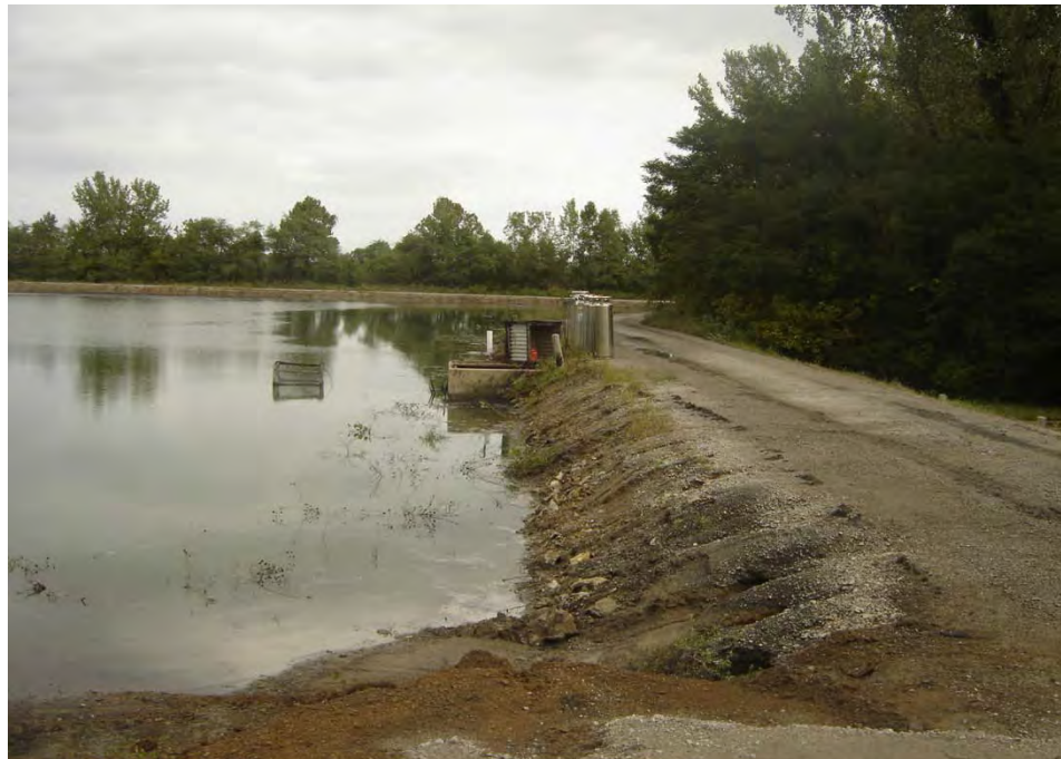
Figure 5.6.1-1. Main Outlet Structure.
