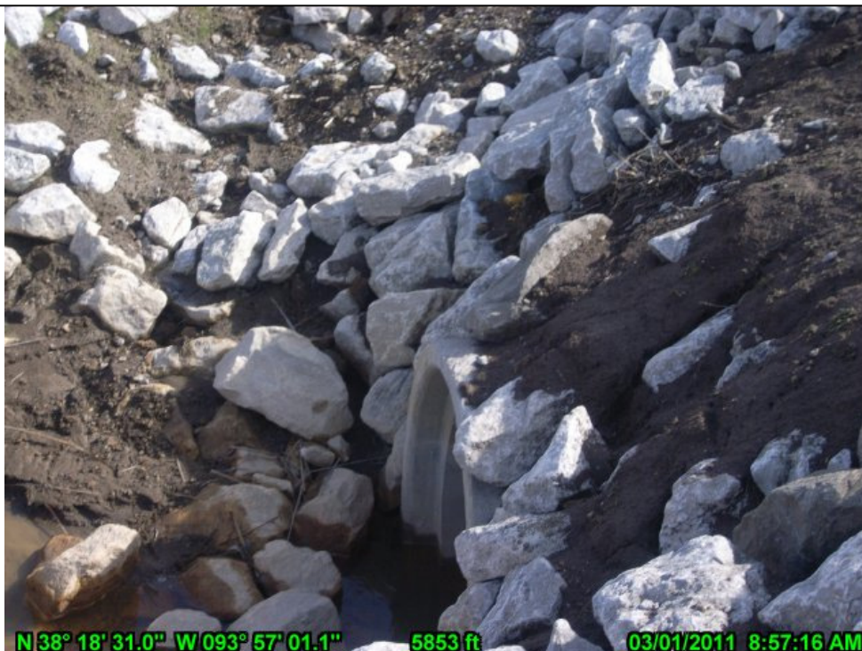
41-First Drainage Ditch Culvert Inlet (Replaced in 2010)
