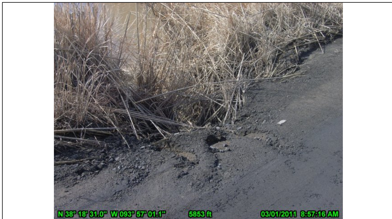
18-Erosion on Land Side of Embankment near Discharge Canal
