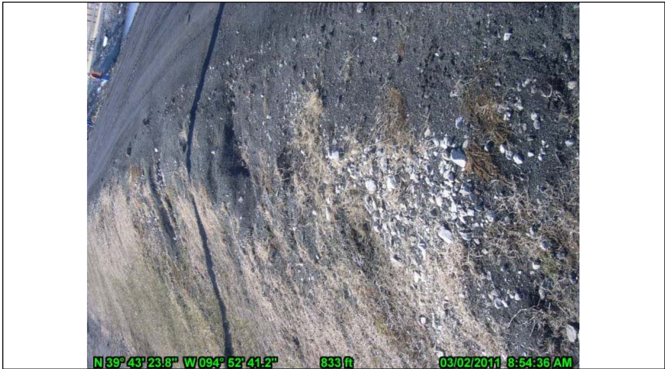
11-Crown and Landside of Slag Pool East Embankment Looking South
