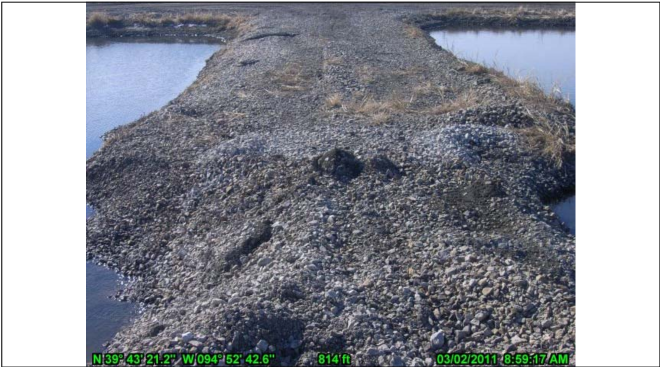
13-Stone Filter between Interim Settling Basin and Final Settling Basin Looking South
