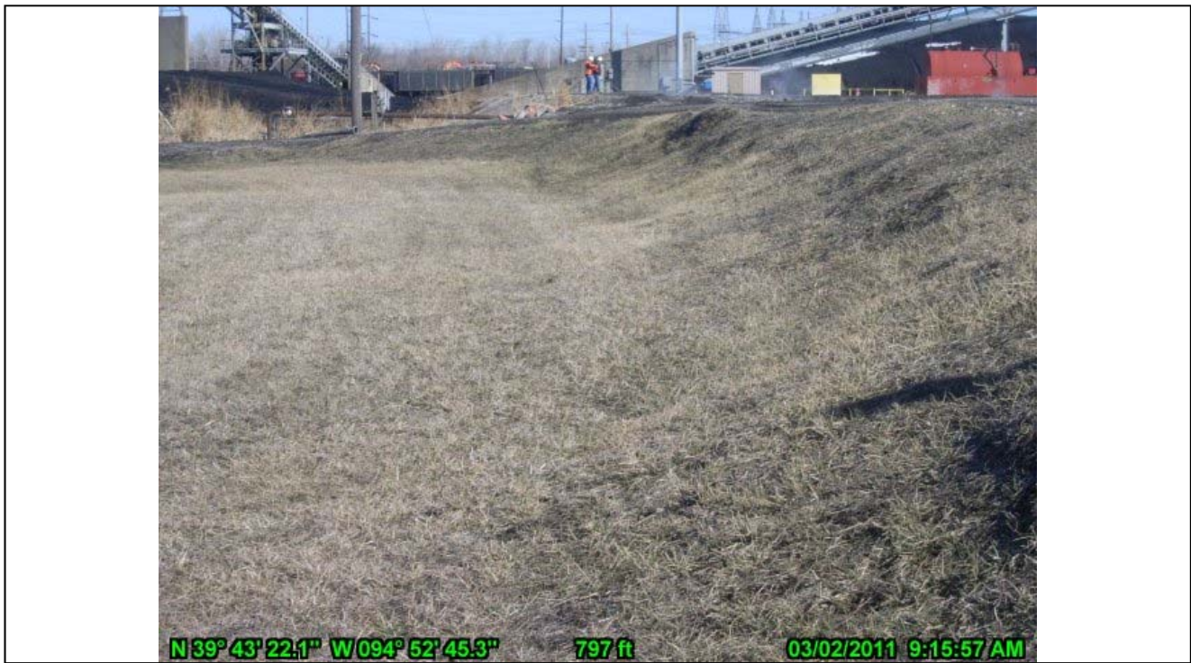
25-Landside Embankment of Coal Pile Run-off Pool Looking North
