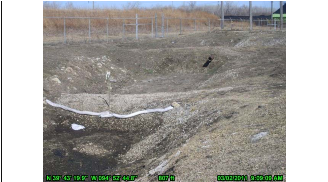
20-Stormwater Erosion Control Channel West of West Embankment Toe
