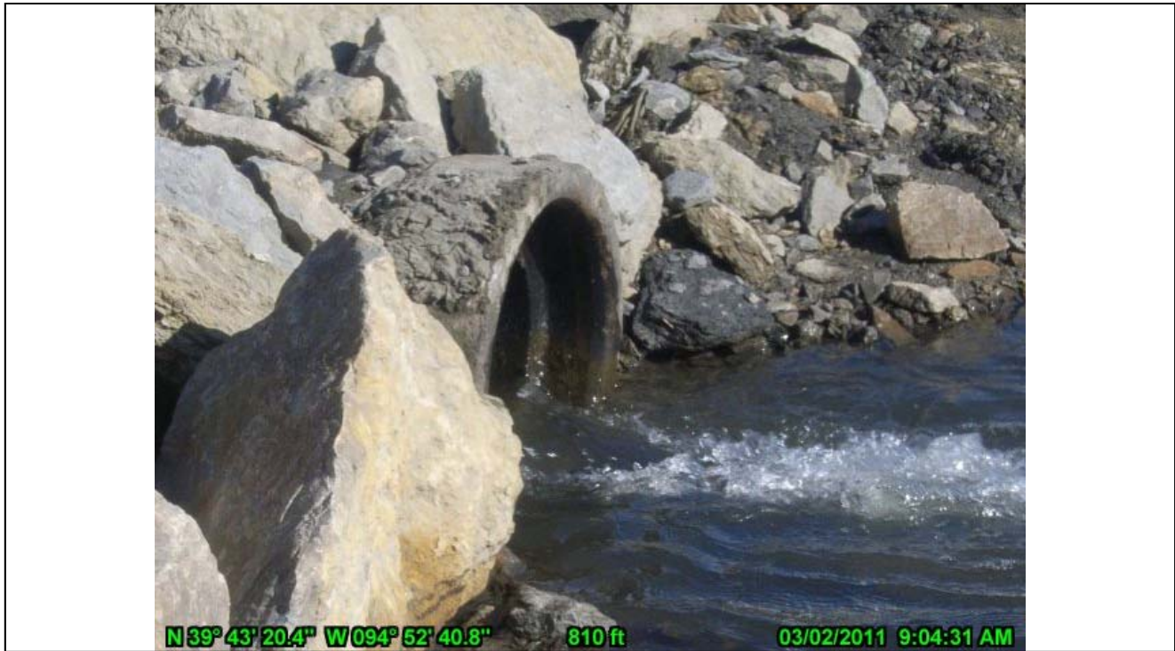
16-Decanter 12" Outlet Pipe
