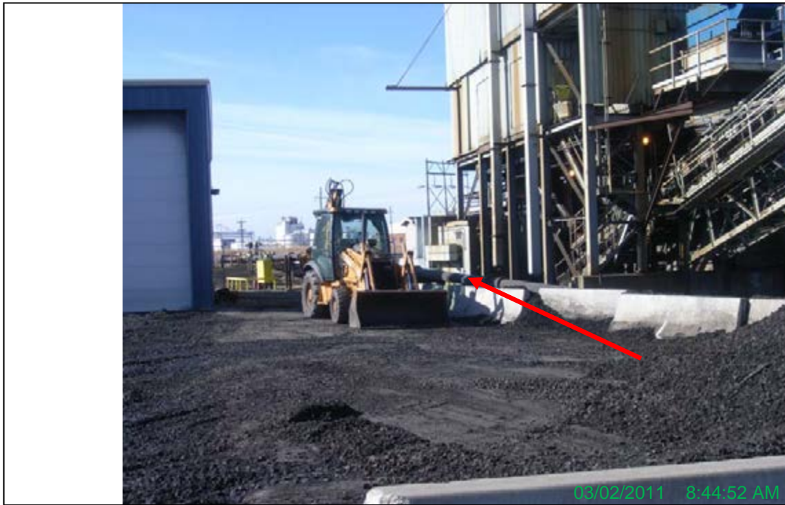
5-Slag Sluice Pipe to Pond Looking West
