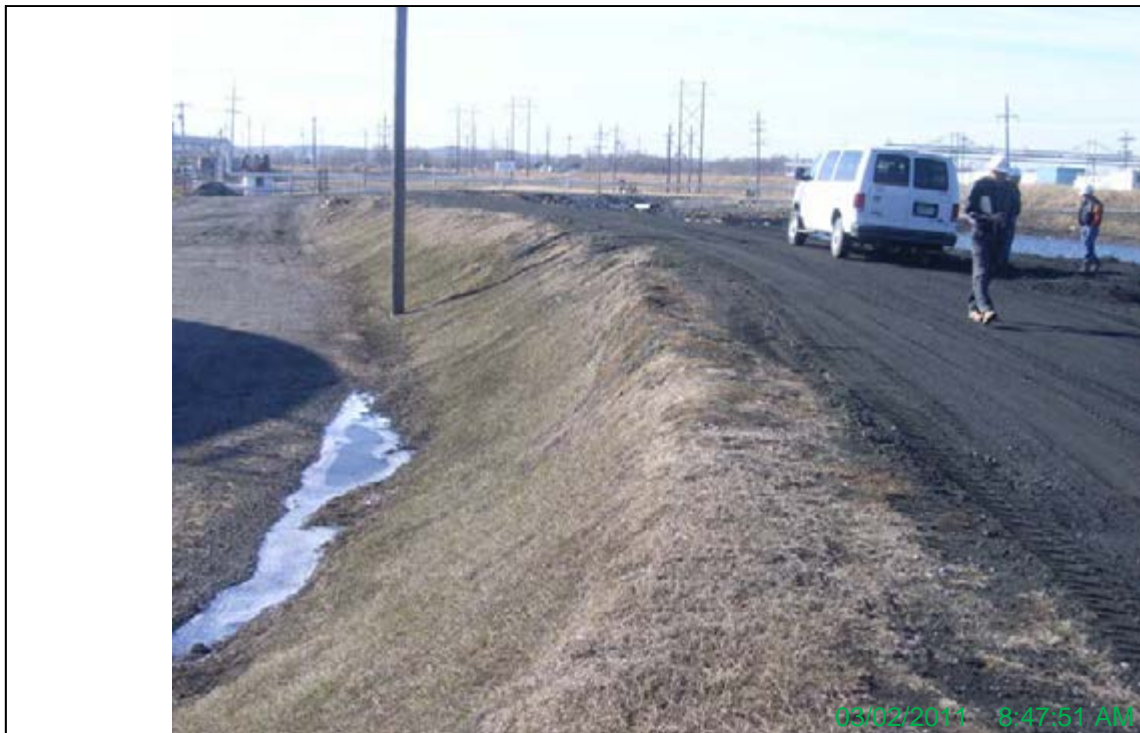
6-Landside East Embankment of Slag Pool (East Pool) Looking South
