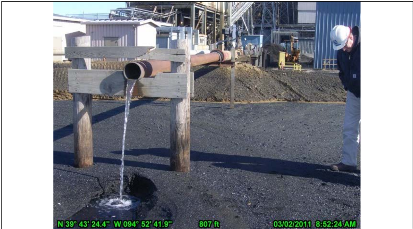
7-Slag Inlet Sluice Pipe looking Northeast
