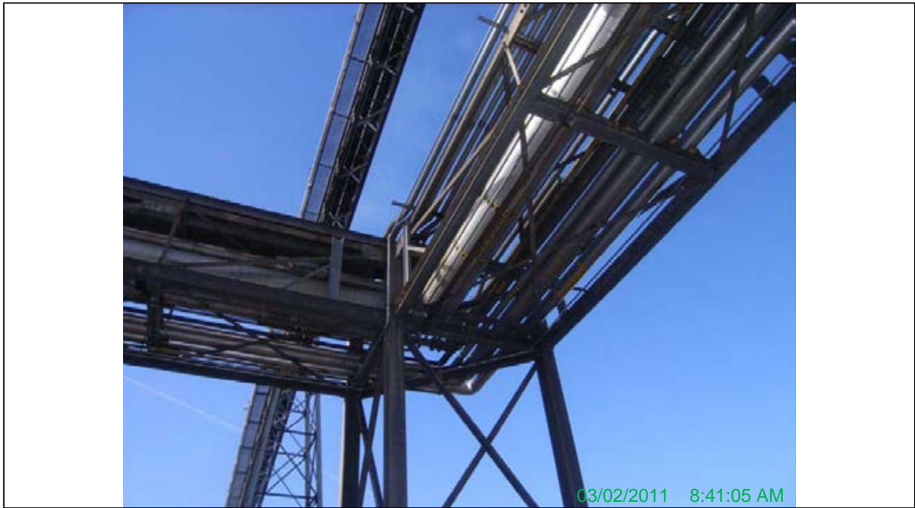
3-Fly Ash Pneumatic Pipe
