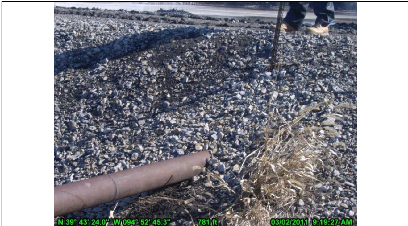
28-Coal Pile Run-off Pipe Landside Penetration
