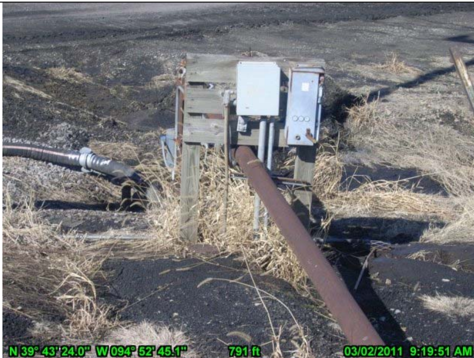
29-Coal Pipe Run-off Pipe and Electric Boxes at Landside Toe
