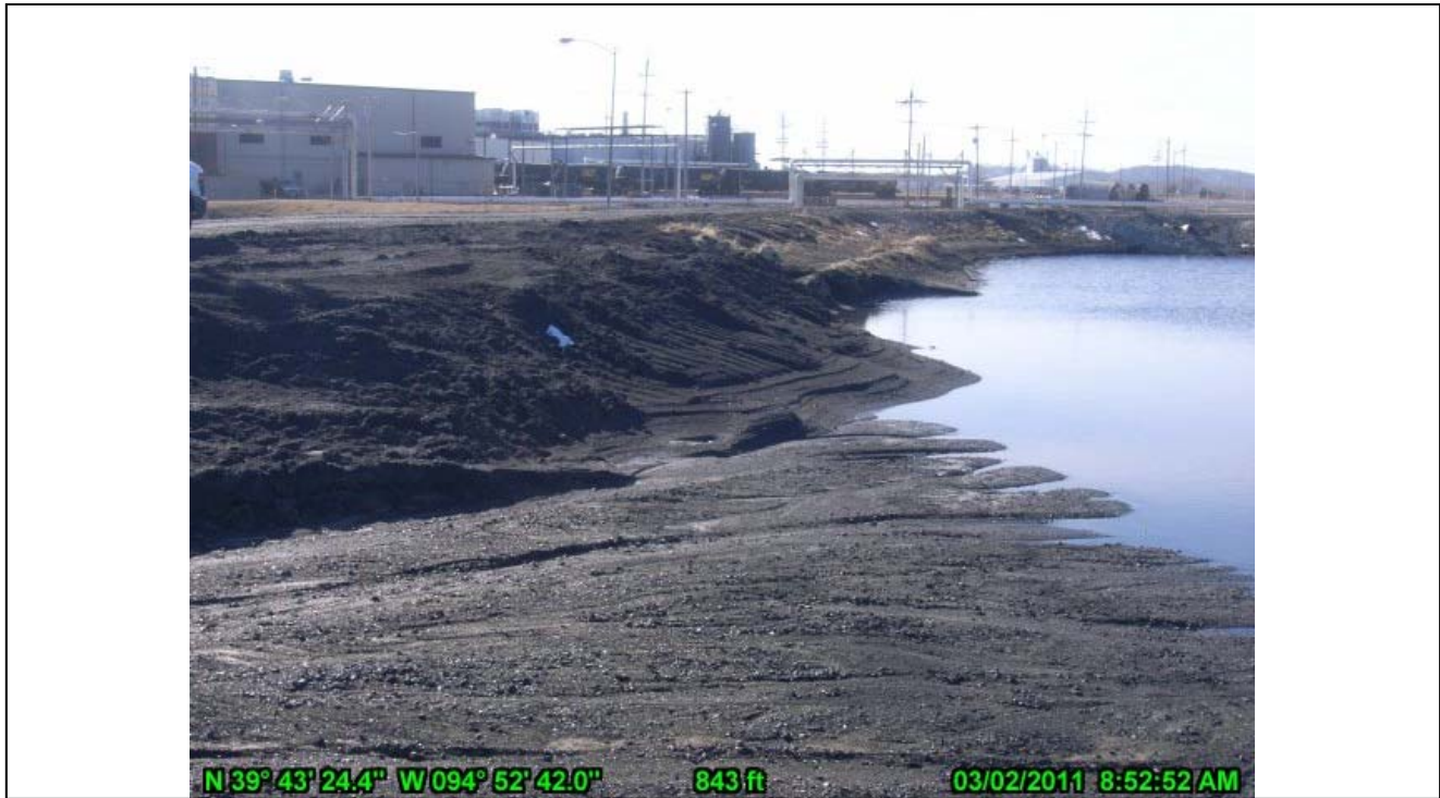
8-Waterside East Embankment of Slag Pool (East Pool) Looking South
