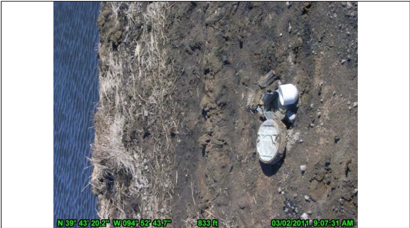
18-Piezometer on South Embankment of Interim Settling Basin
