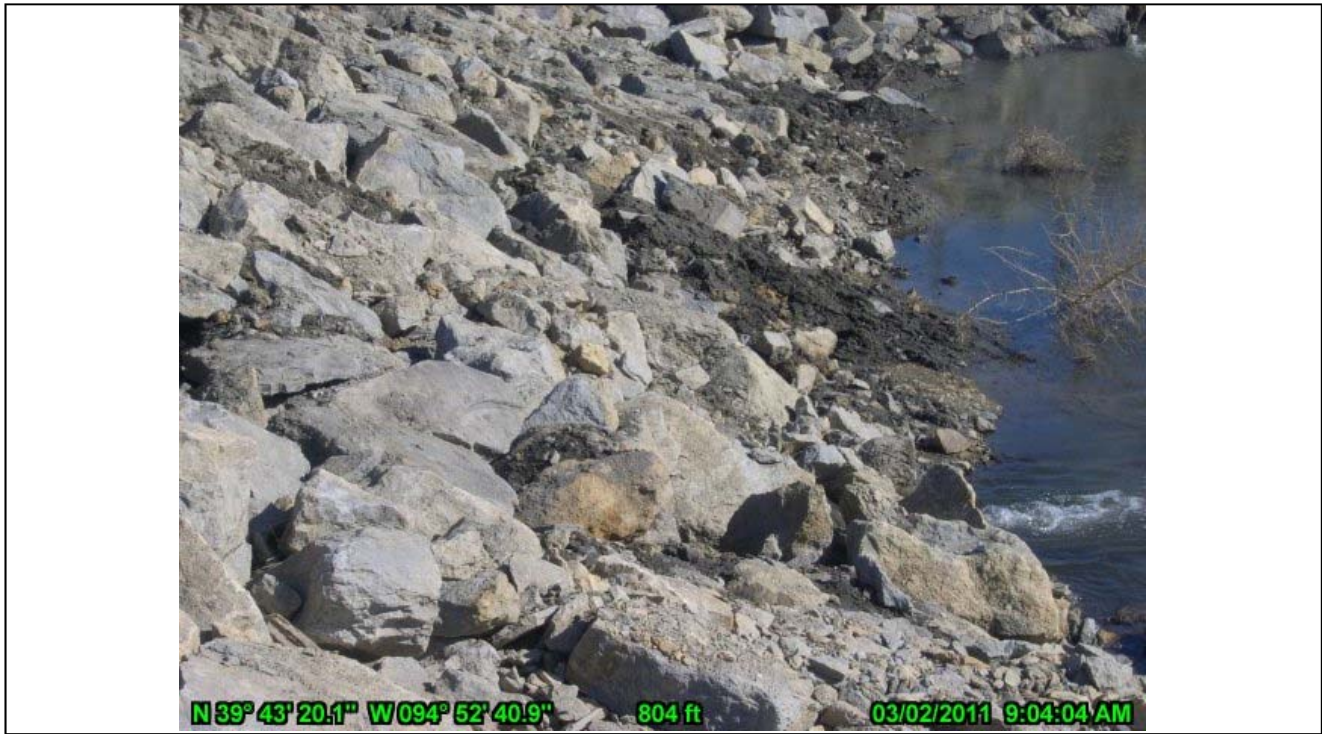
15-Landside of South Embankment/Drainage Canal and Outlet Pipe
