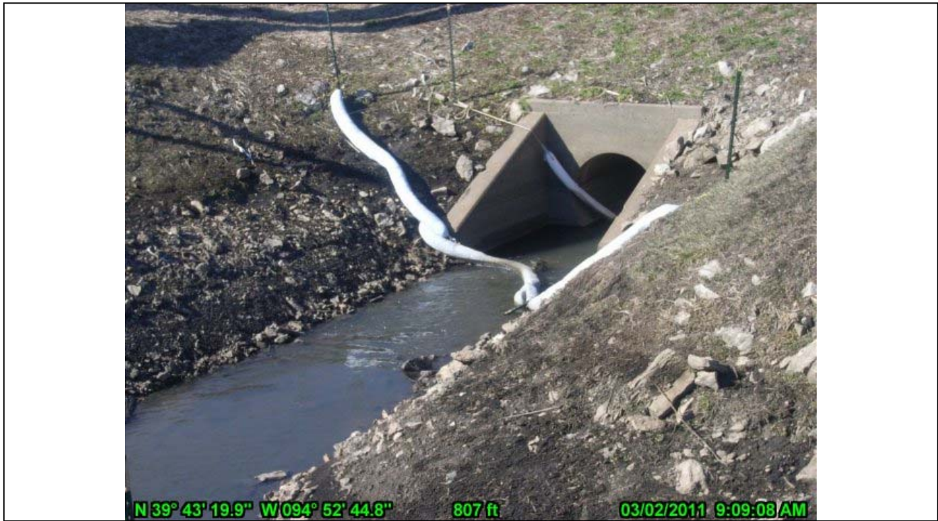
19-Discharge Canal to Brown's Branch Culvert Inlet
