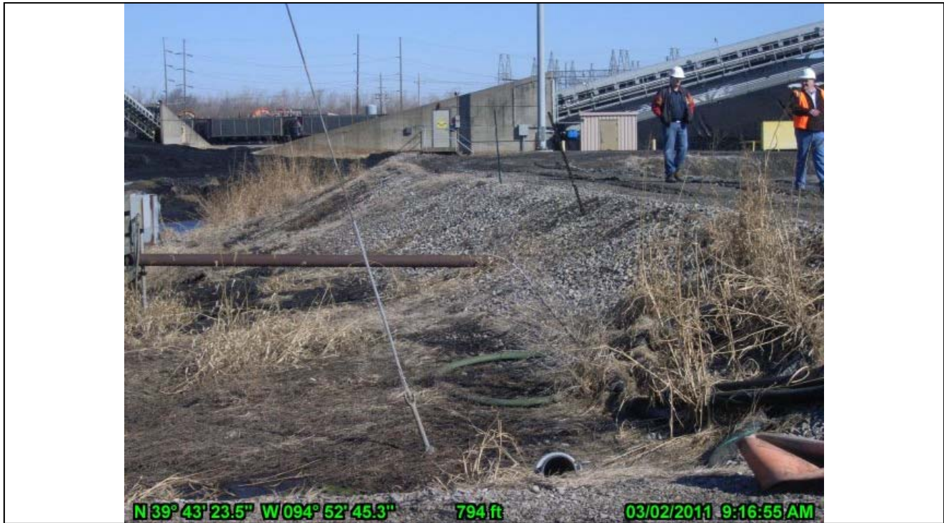
26-Landside Embankment of Coal Pile Run-off Pool Looking North
