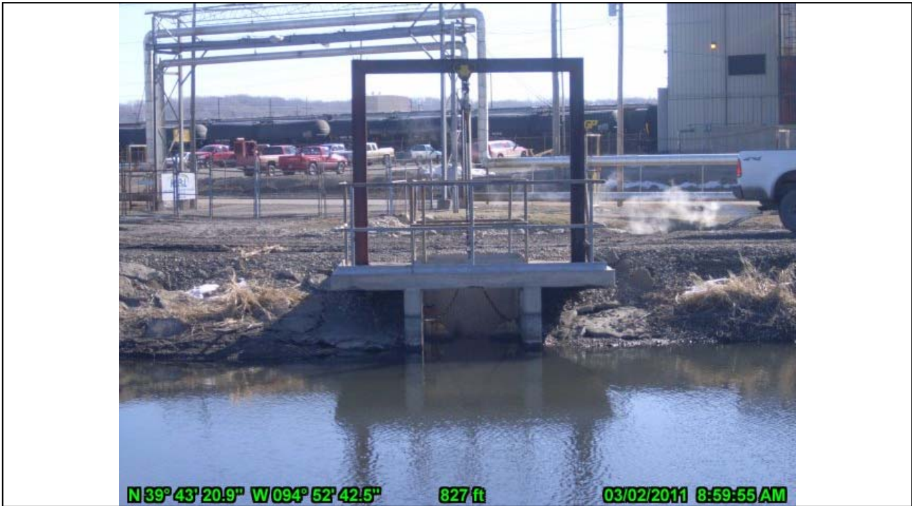
14-Final Settling Basin Decant Outlet Works Intake
