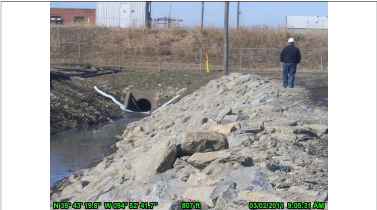
17-Landside South Embankment/Drainage Canal and Inlet Culvert to Brown's Branch
