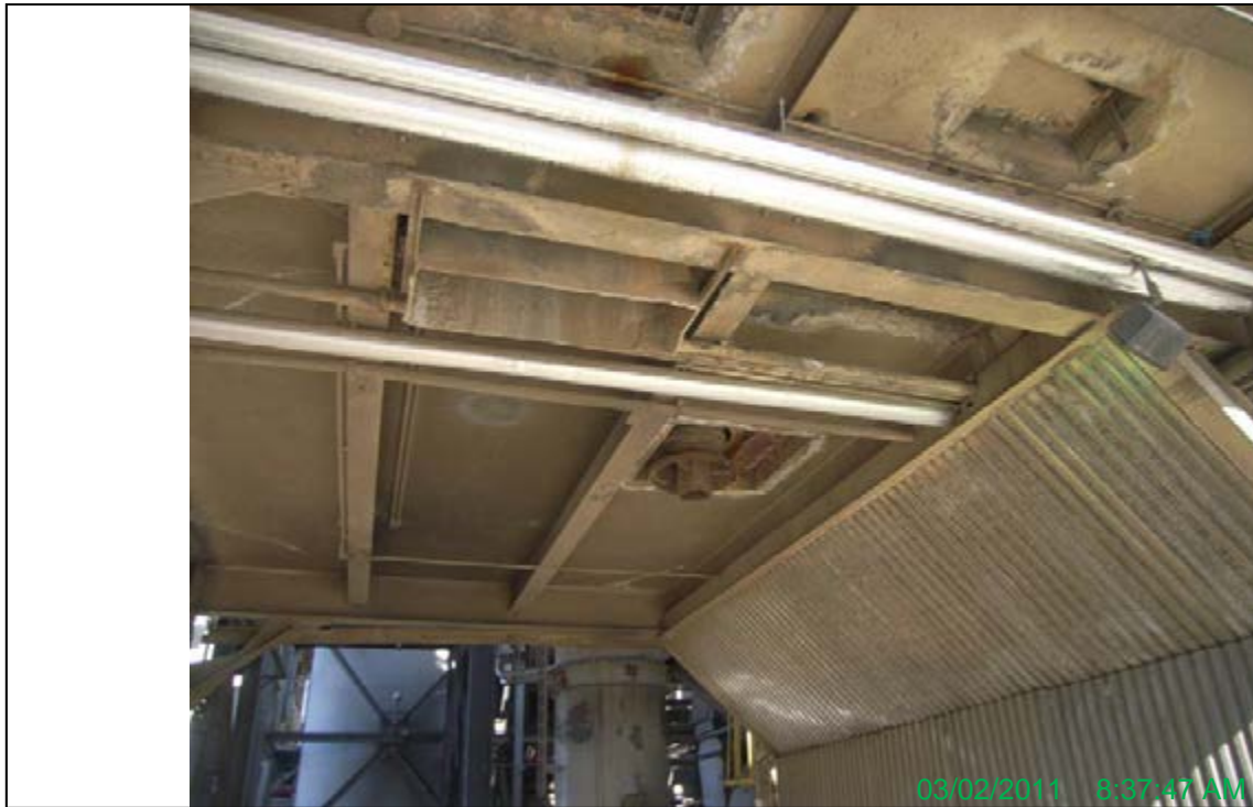
2-Bottom Ash Silo Outlet
