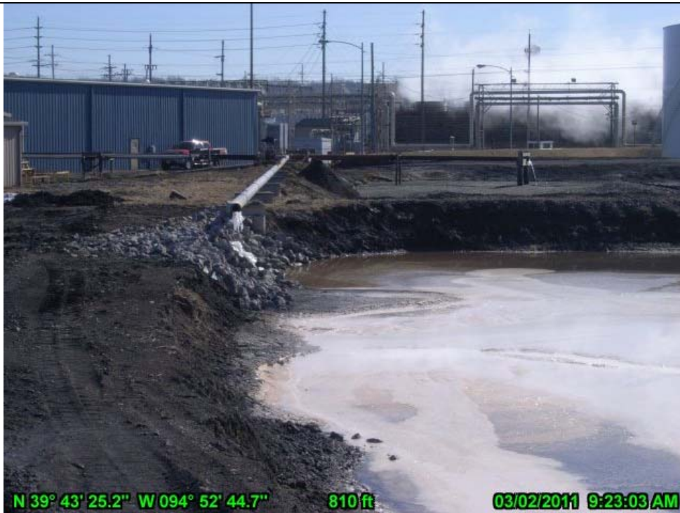
30-Fly Ash Inlet and North Embankment of Coal Pile Run-off Pool Looking East
