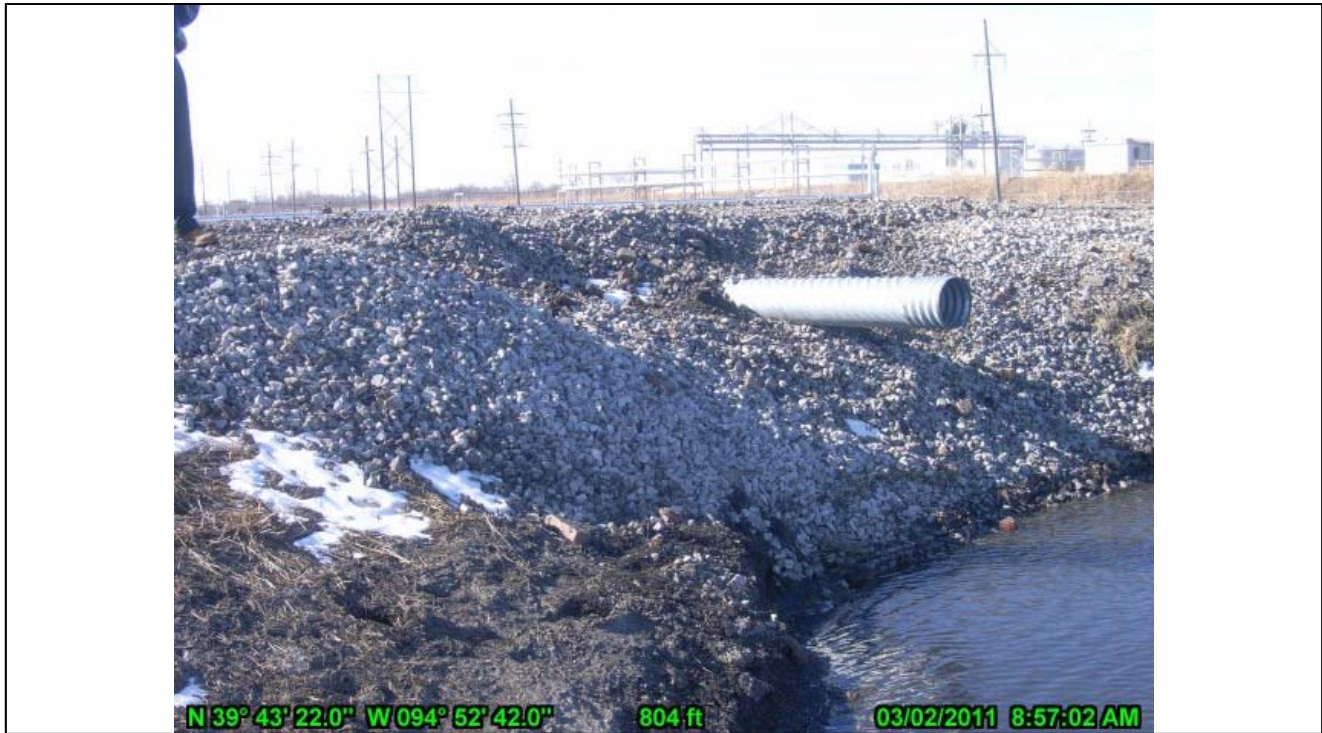
12-Stone Filter Outlet and Overflow Pipe at South End of Slag Pool
