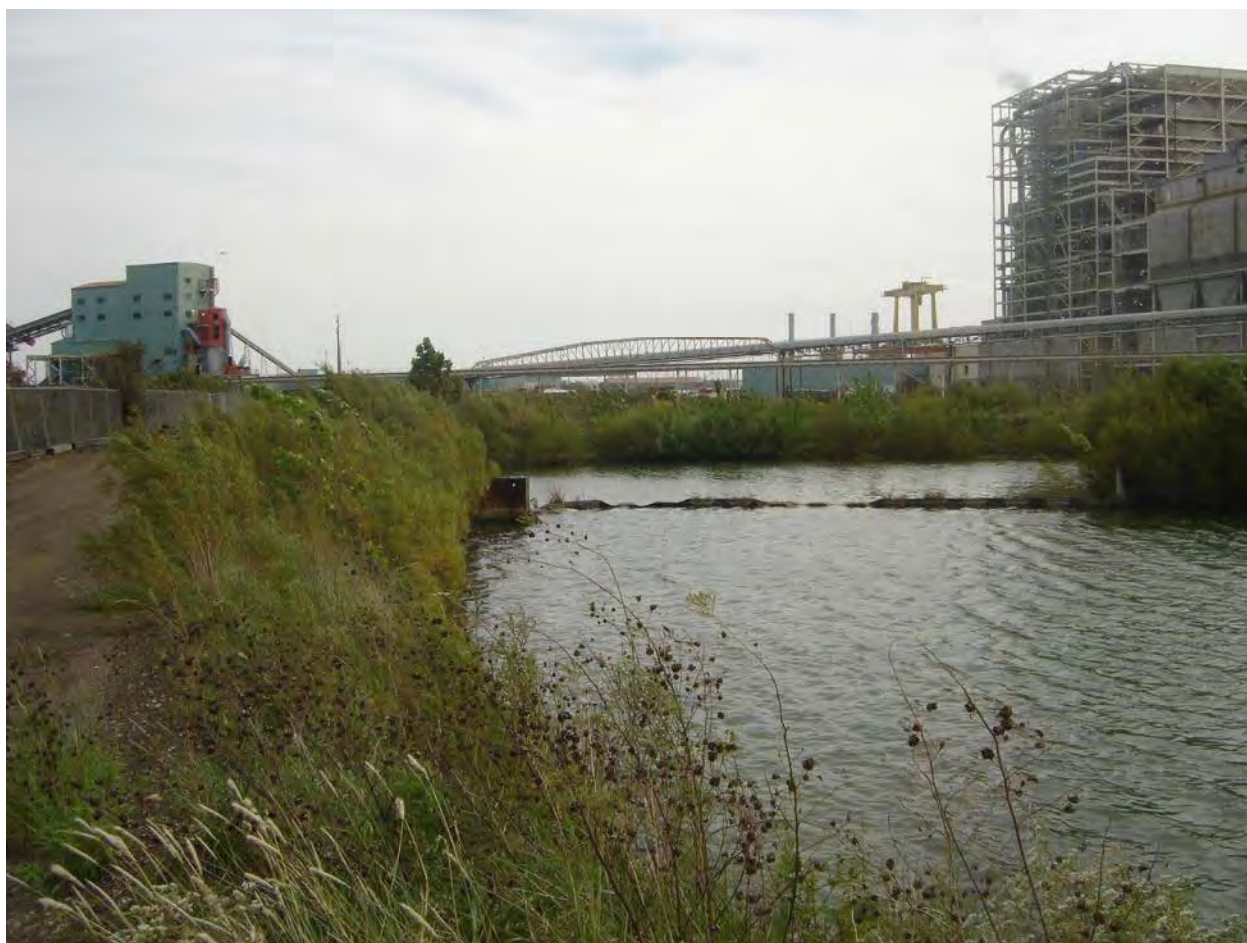
B- 3: Bottom Ash Pond looking north
