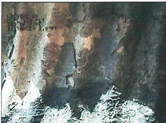
Photo: 1, Tape/Media No.: 082310 KCPL, 00:00:45 1.9FT, Manhole
