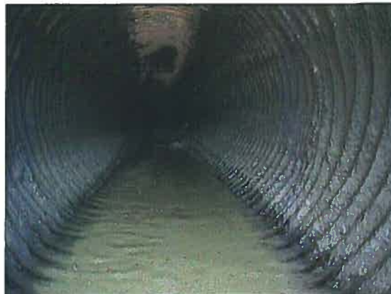
Photo: 2, Tape/Media No.: 082310 KCPL, 00:00:45 1.9FT, Manhole
