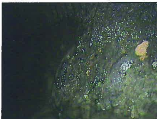
Photo: 4, Tape/Media No.: 082310 KCPL, 00:02:28 13.2FT, Deposits Attached Encrustation, 2 % of cross sectional area, from 04 to 07 o'clock, within 8 inch: YES
