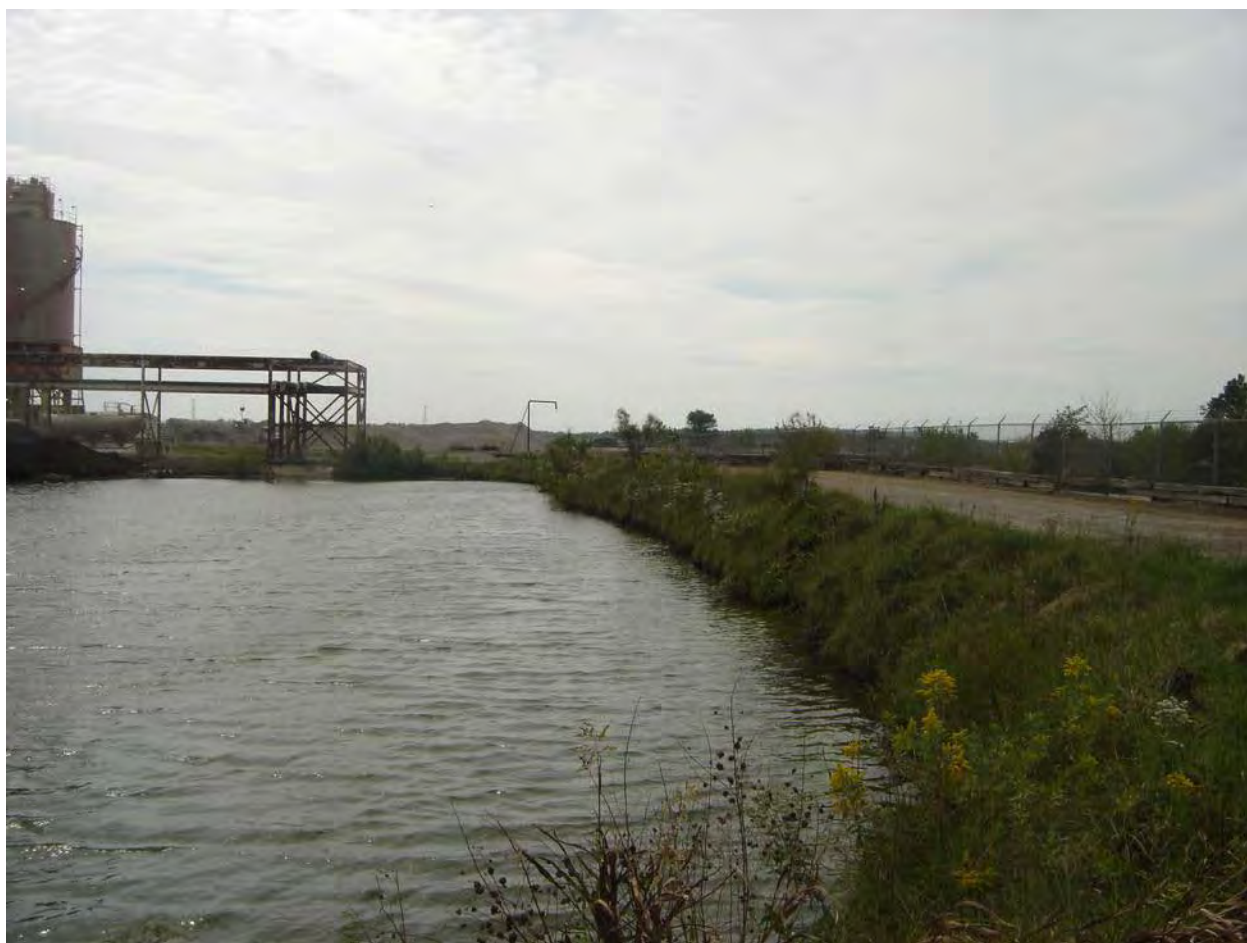
B- 2: Bottom Ash Pond looking east
