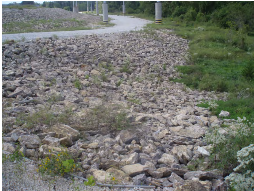
Figure 5.2.4-2: Photo of Exterior Groin at Northwest Corner of Impoundment. Note that the dike in upper left hand corner also serves as the flood prevention dike for the plant.
