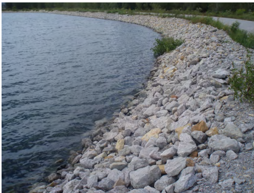
2. Interior of dike – Taken from east end of pond, looking northwest
