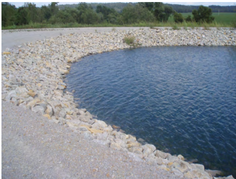
35. Tie-in of interior separation dike at east end – clearwater pond side.
