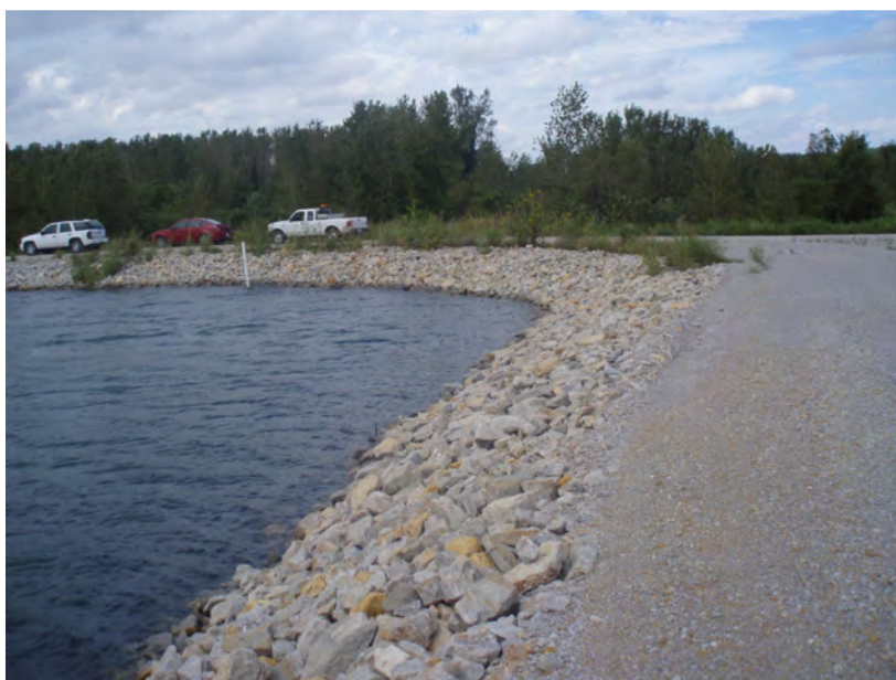
36. Tie-in of interior separation dike at east end – ash pond side.
