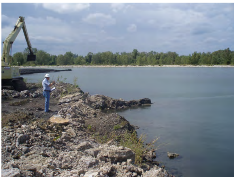
34. Interior of separation dike – Ash pond side, taken from separation dike looking north across pond.
