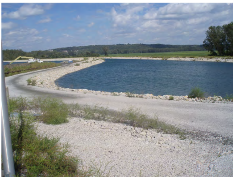
28. Stillwater pond and interior dike, from west end looking east.
