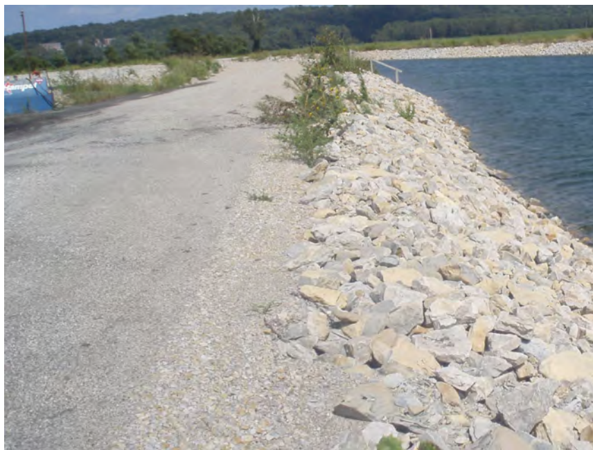
Figure 5.2.1-1: Photograph of Impoundment Dike Crest View
