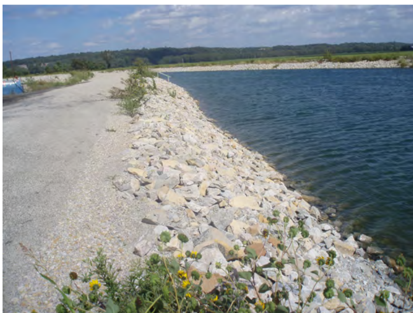
30. Interior separation dike – Clearwater side, taken from separation dike looking east.
