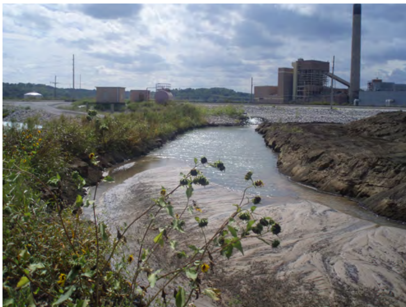
32. Interior of separation dike – Ash pond side, taken from separation dike looking west.
