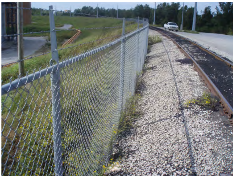
23. Exterior of dike (plant ring berm) – Taken from west side of pond looking north.
