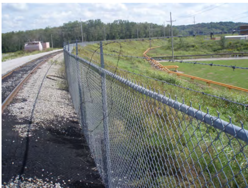
24. Exterior of dike (plant ring berm) – Taken from west side of pond looking south.
