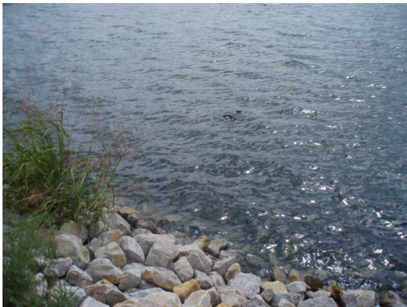
1. Outfall Gate – East Side of Pond
