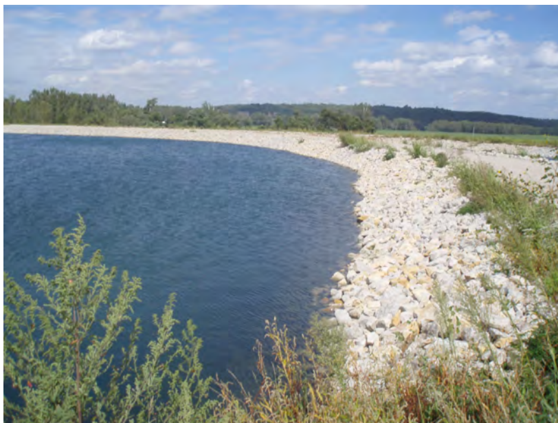
33. Interior of separation dike – Ash pond side, taken from separation dike looking east.
