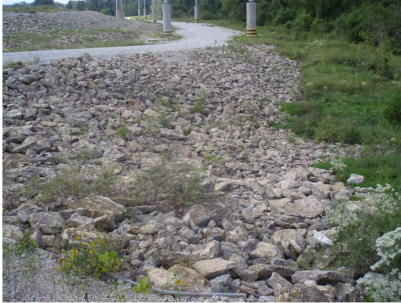
21. Exterior of dike, groin at northwest corner.
