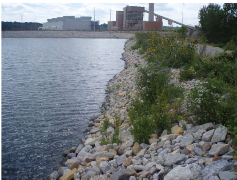
18. Interior of dike – Taken from north side of pond looking west.
