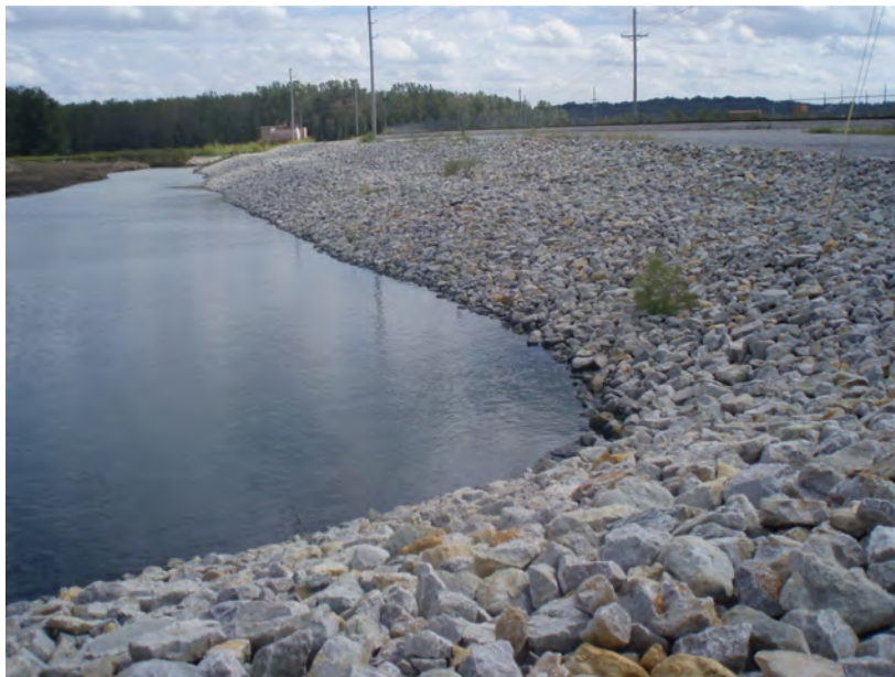
22. Interior of dike, groin at northwest corner.
