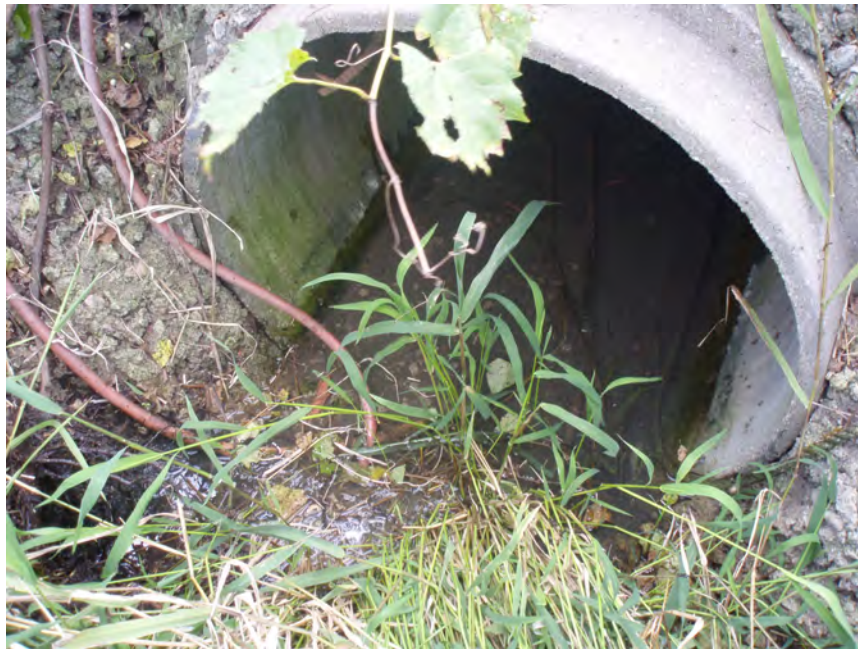
Figure 5.3.2-2: Photo of Drainage at Exterior End of 30" Discharge Pipe
