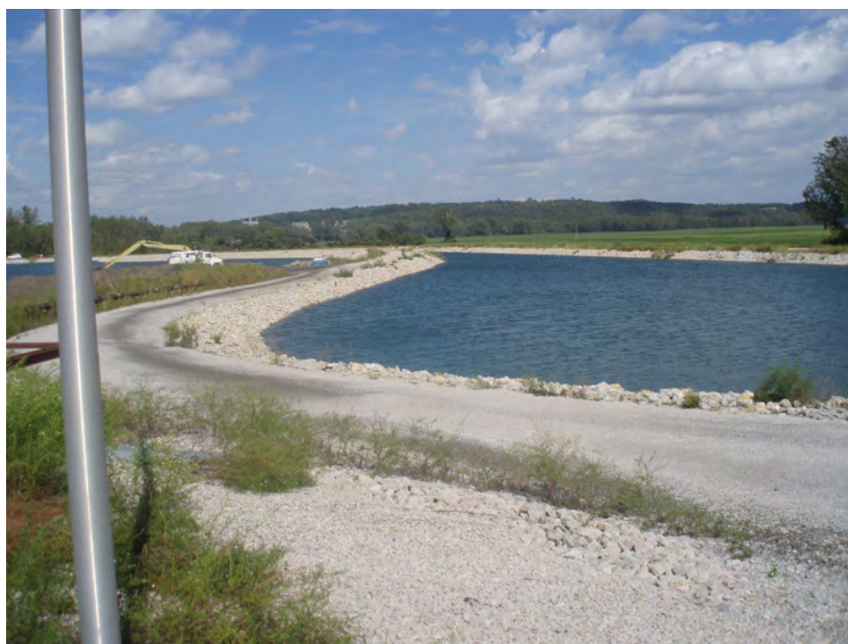
Figure 8.1-1: Photo of dike dividing ash pond from clear water pond.
