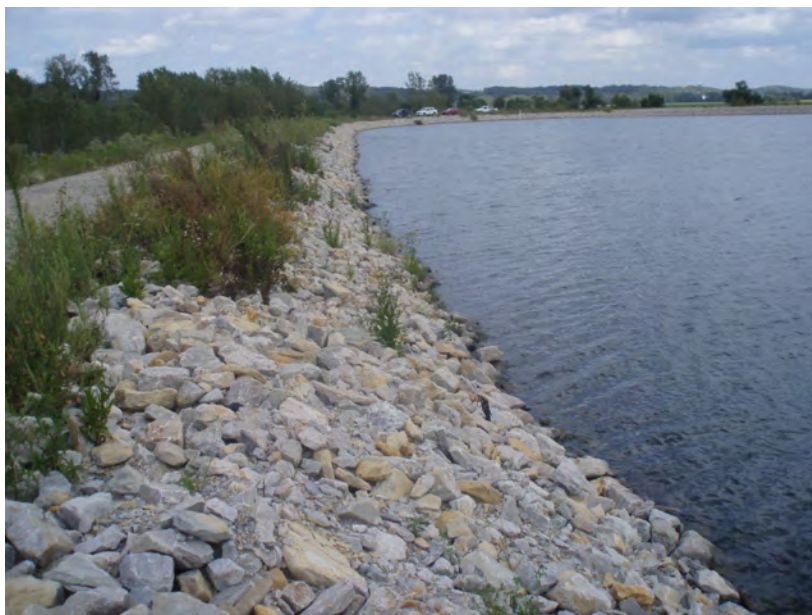
17. Interior of dike – Taken from north side of pond looking east.
