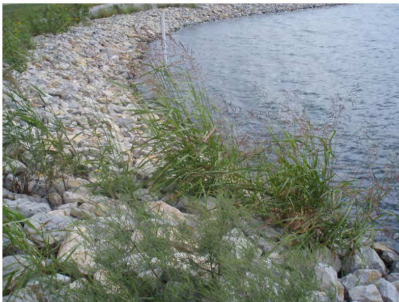
3. Interior of dike – Taken from east end of pond, looking south
