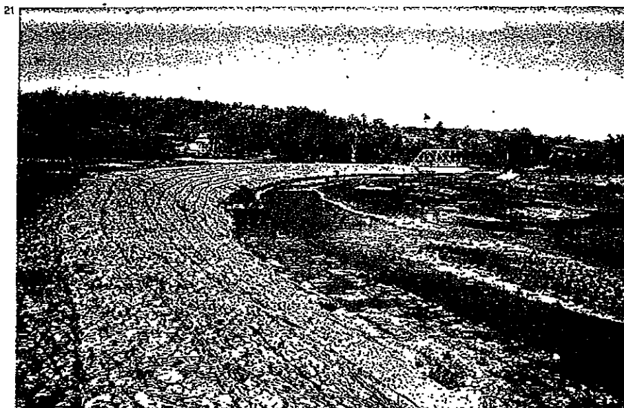
Fig. 21 - U.S.A. - New York Gabion bank protection near Buffalo.
