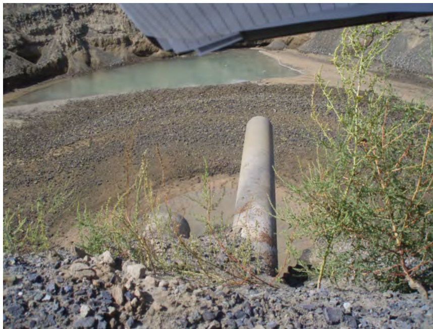
Figure 5.3.2-1: Photo of Bottom Ash Discharging into Ash Pond.
