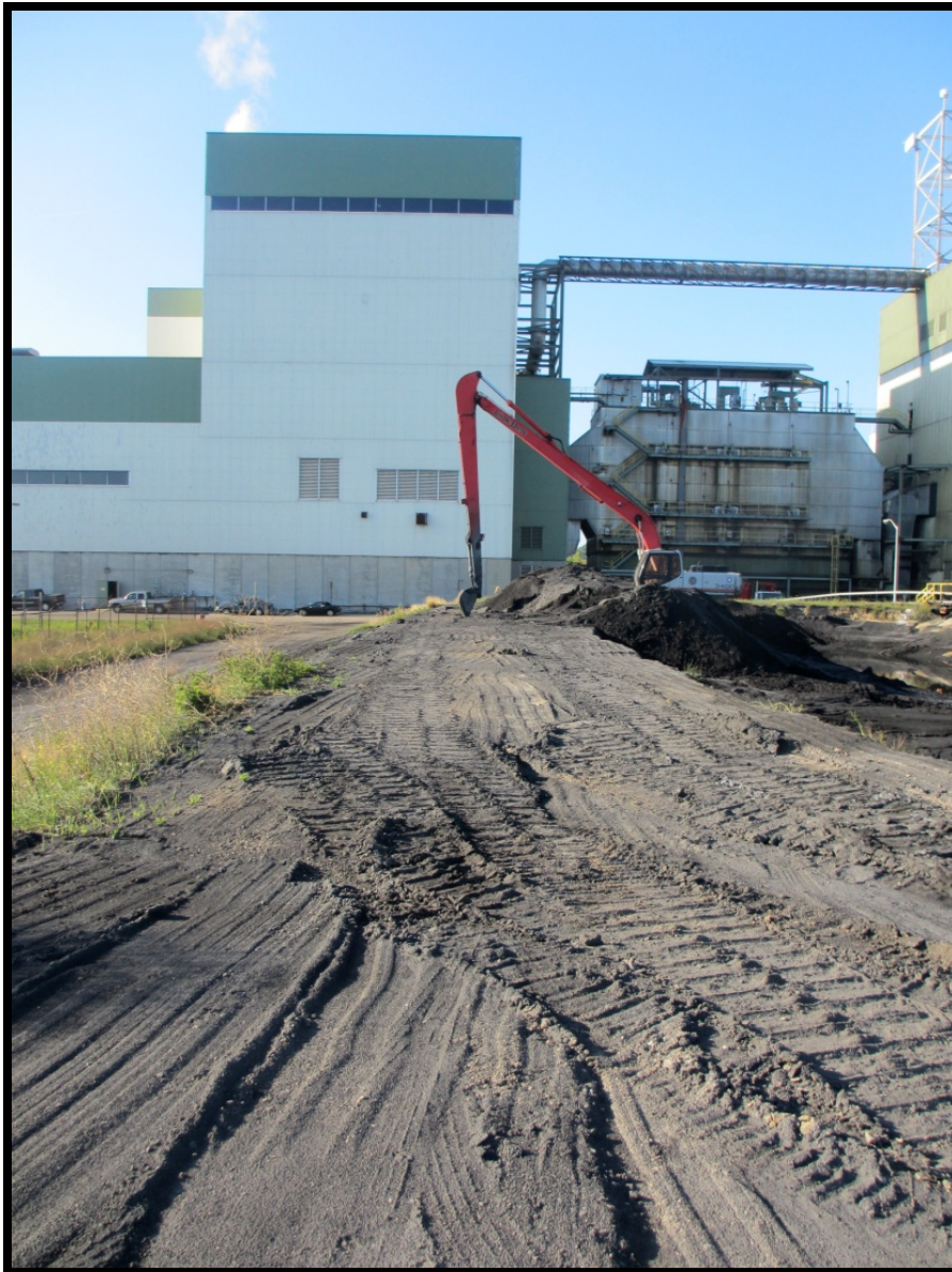
Photo 5.2.1: Looking south at East Pond's east berm
