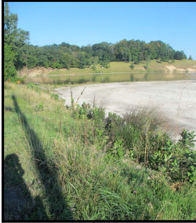
Photo 5.3.3b: Looking down at West Pond's north toe along adjacent property
