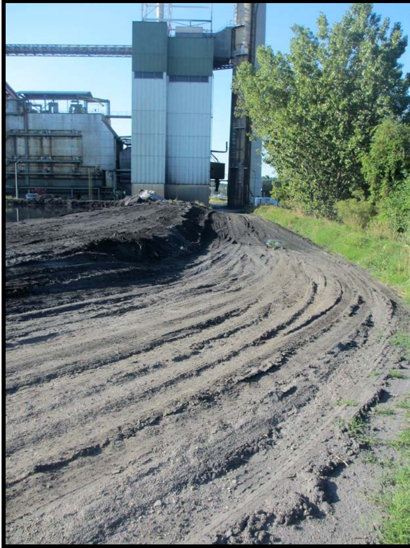
Photo 5.3.1b: Looking south along west embankment/toe of West Pond (note the water midway south along the toe of the embankment)
