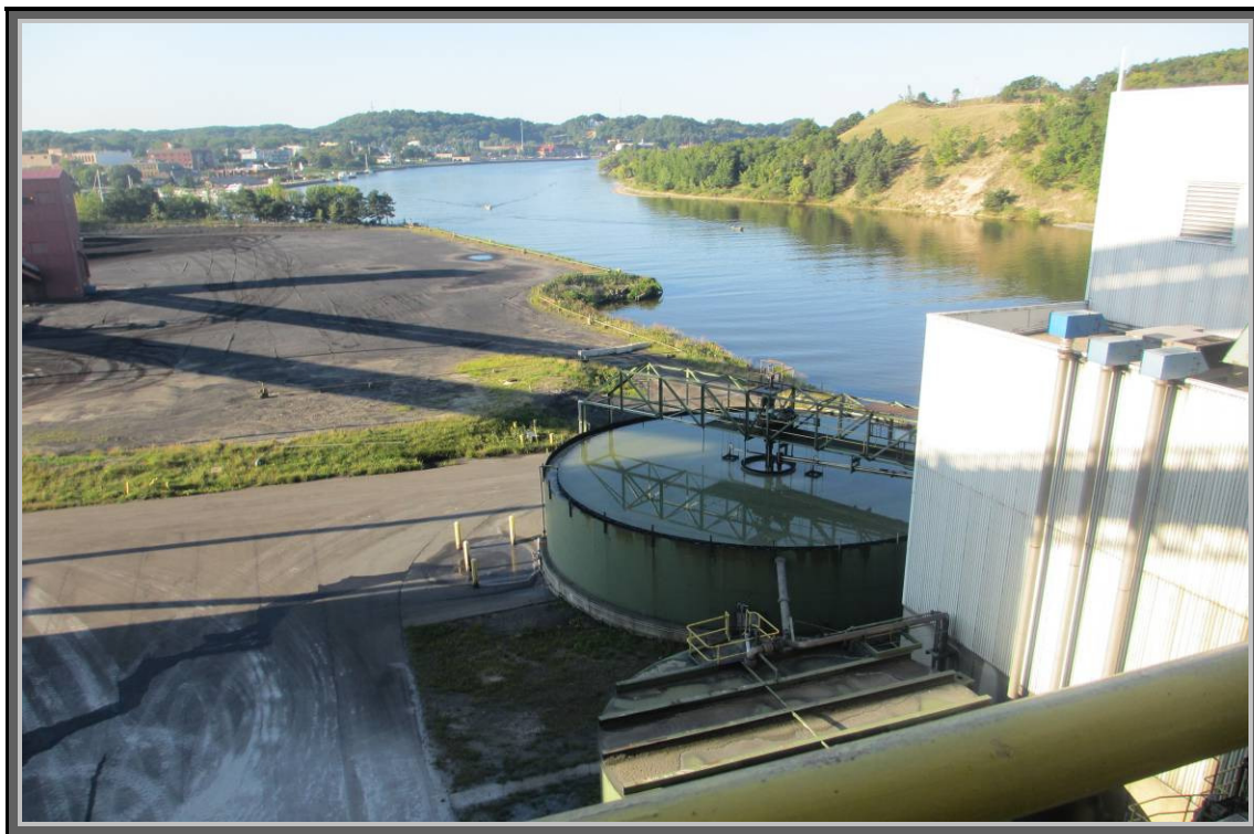
Photo 10. Looking S from Plant at Grand River _JB Sims Power Plant_082212
