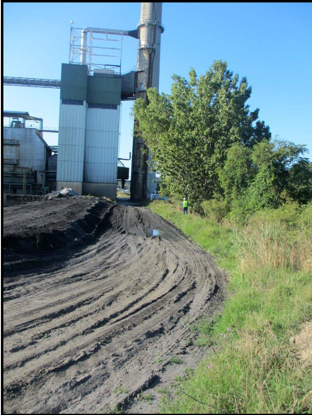
Photo 5.3.3f: Looking south down west toe of West Pond (treeline is along a natural river embankment (not part of the bottom ash pond systems))
