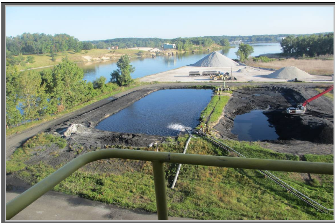
Photo 4. Looking NW at primarily W Pond _JB Sims Power Plant_082212
