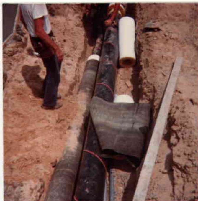
78. Heat tracing and insulating the piping through the center dike at the location of the overflow wier.
