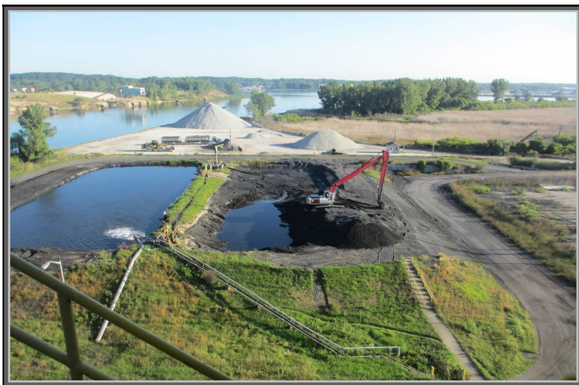
Photo 3. Looking NE at primarily E Pond _JB Sims Power Plant_082212
