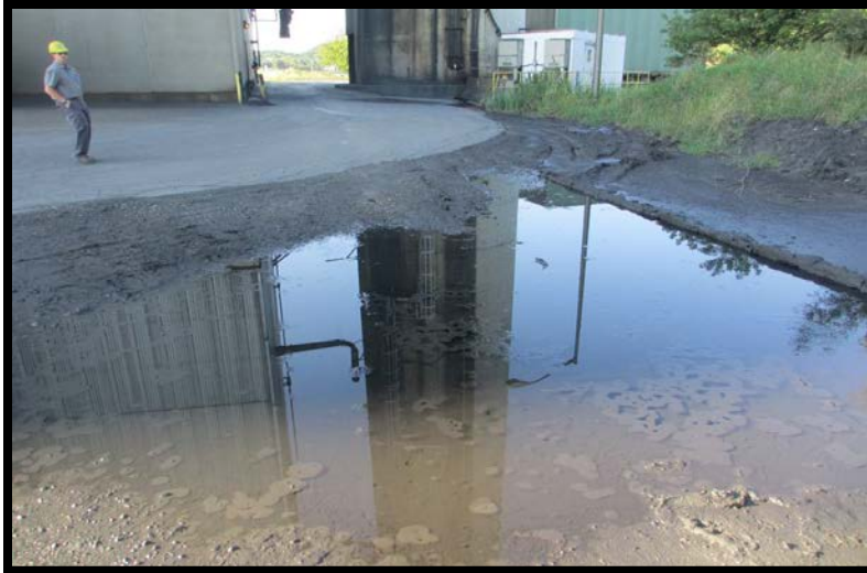
Photo 5.3.3i: Looking south from West Pond's southwest embankment (note ponded water)
