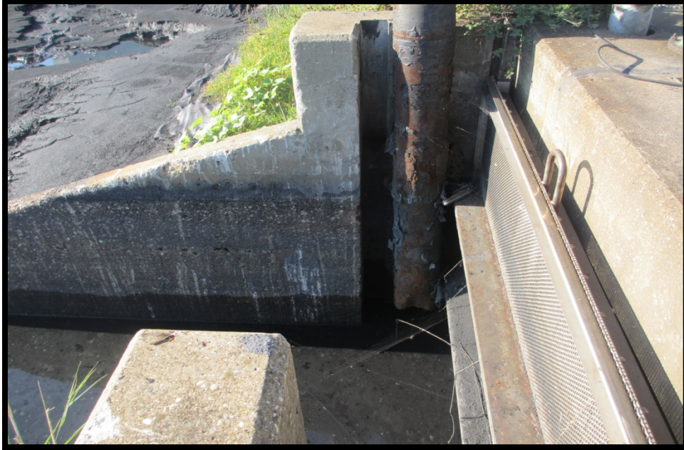
Photo 5.4.2a: Valve pit/ low level sluice gate conduit (eastern side)
