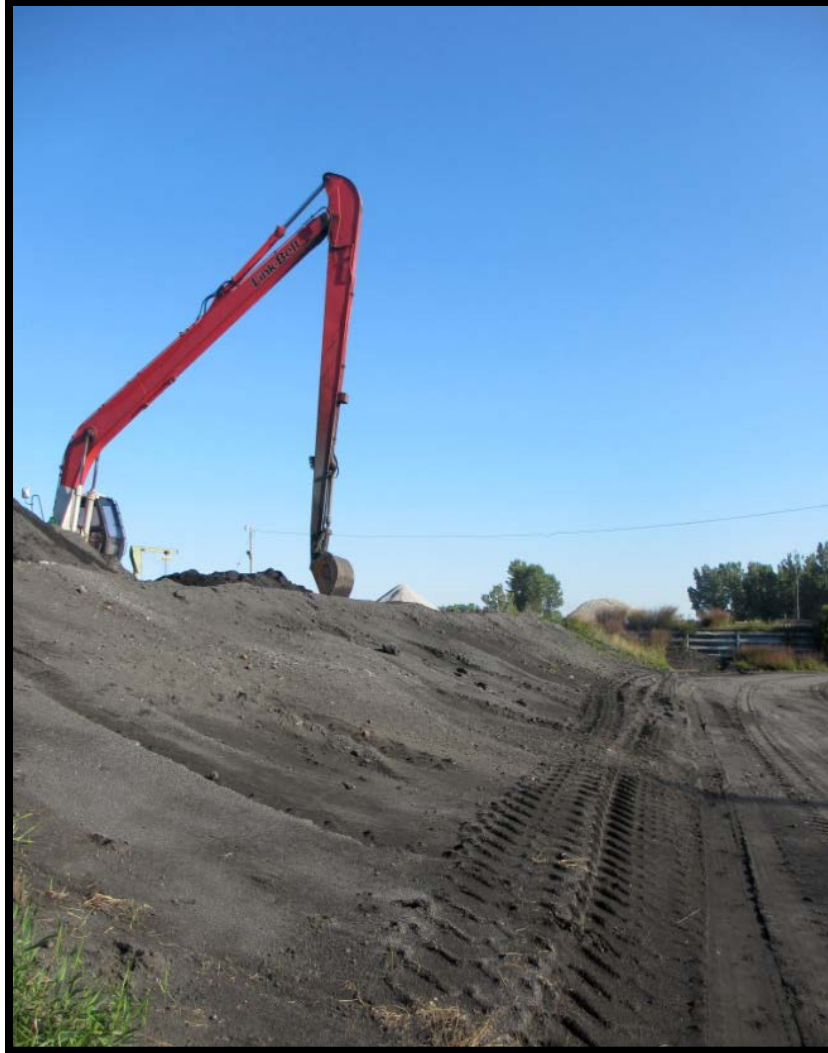
Photo 5.2.3c: Looking northwest along eastern embankment and toe of East Pond; note presence of bottom ash (black material covering ground) on the outside slope.
