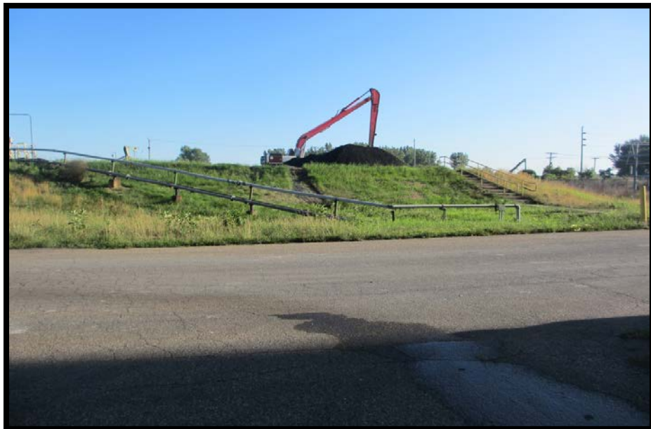
Photo 5.2.3a: Looking north from plant at East Pond's south embankment
