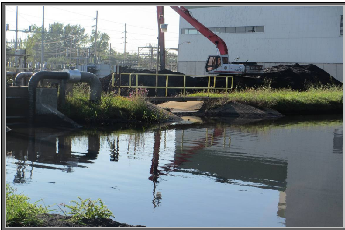
Photo 8. Looking SE at spillover from E to W Pond and vice versa _JB Sims Power Plant_082212
