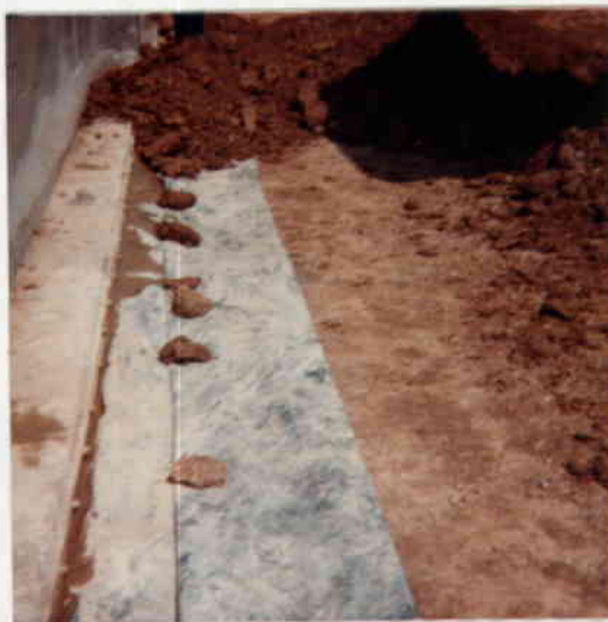
34. Hypalon membrane lapped and ready for burial.
