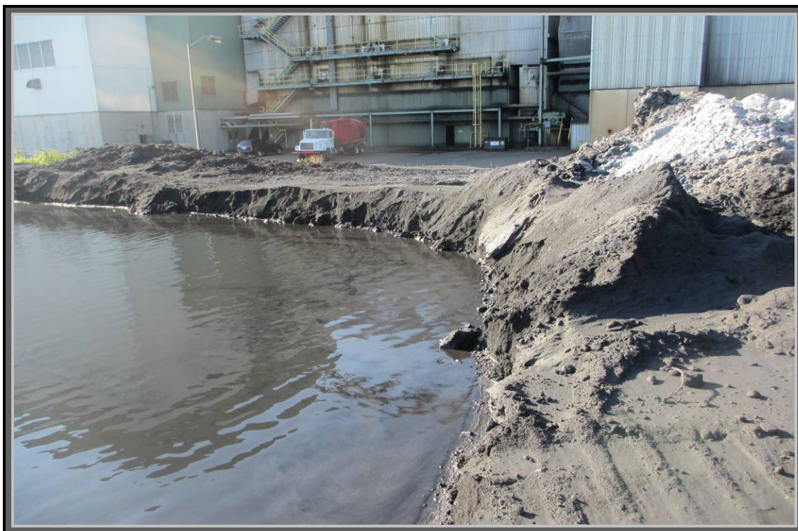
Photo 6. W Pond's SW corner (gypsum seen misplaced in storage pile in top right corner; not typically stored here) _JB Sims Power Plant _082212
