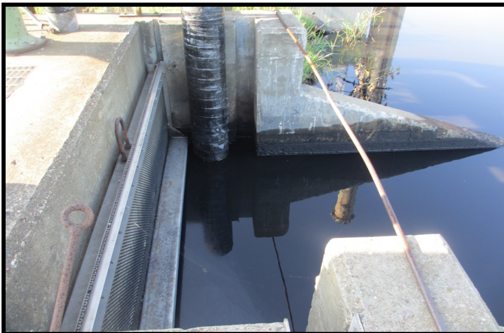
Photo 5.4.2b: Valve pit/ low level sluice gate conduit (western side)
