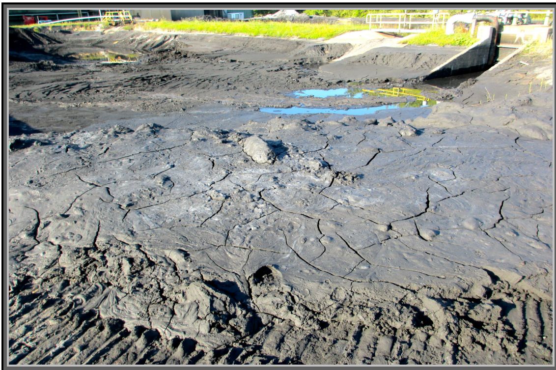
Photo 9. Wet bottom ash on NE corner of E Pond (note indentation of my footprint) _JB Sims Power Plant_082212
