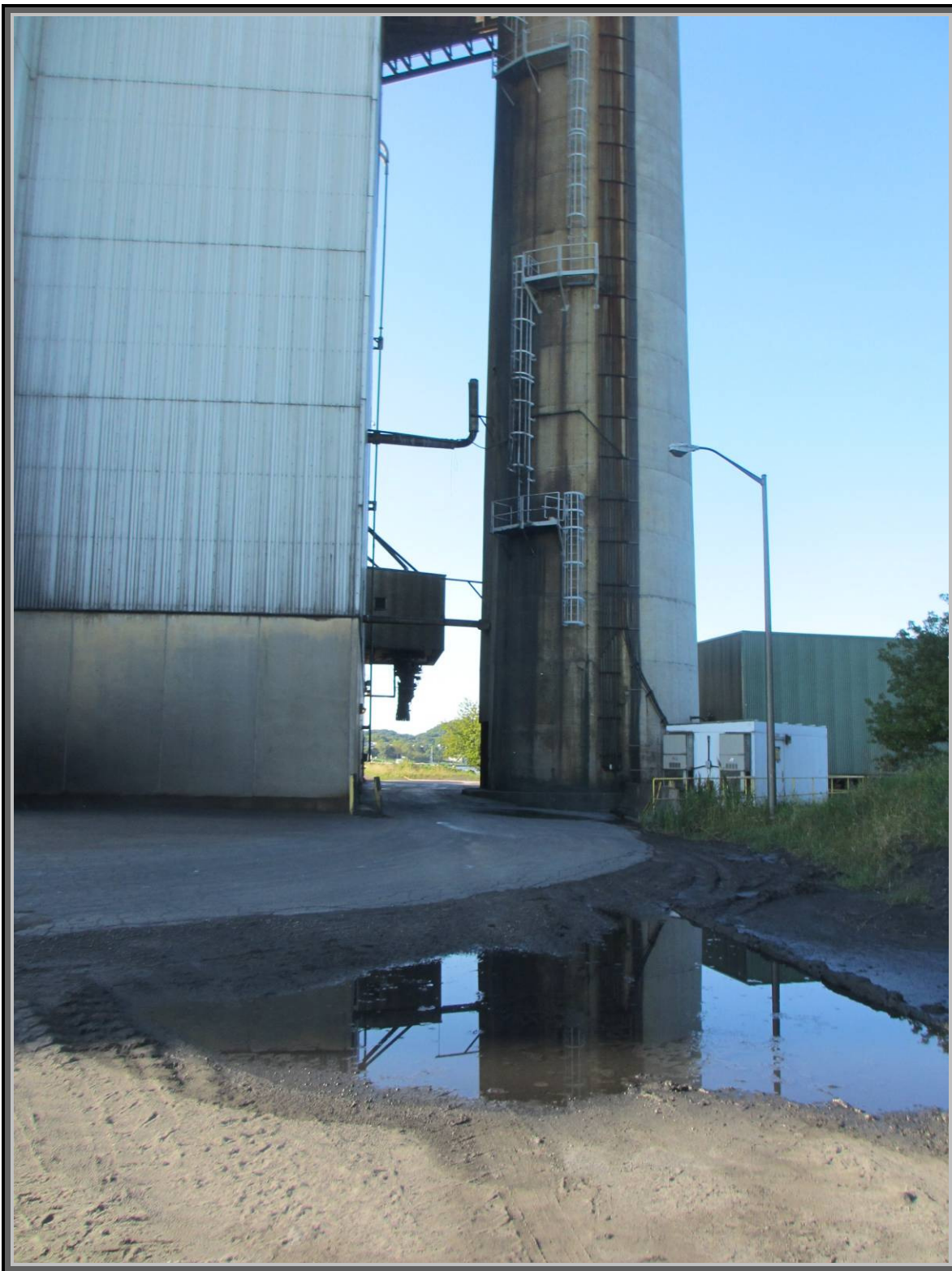
Photo 1. Looking S from W Pond's SW embankment at fly ash loader _JB Sims Power Plant _082212
