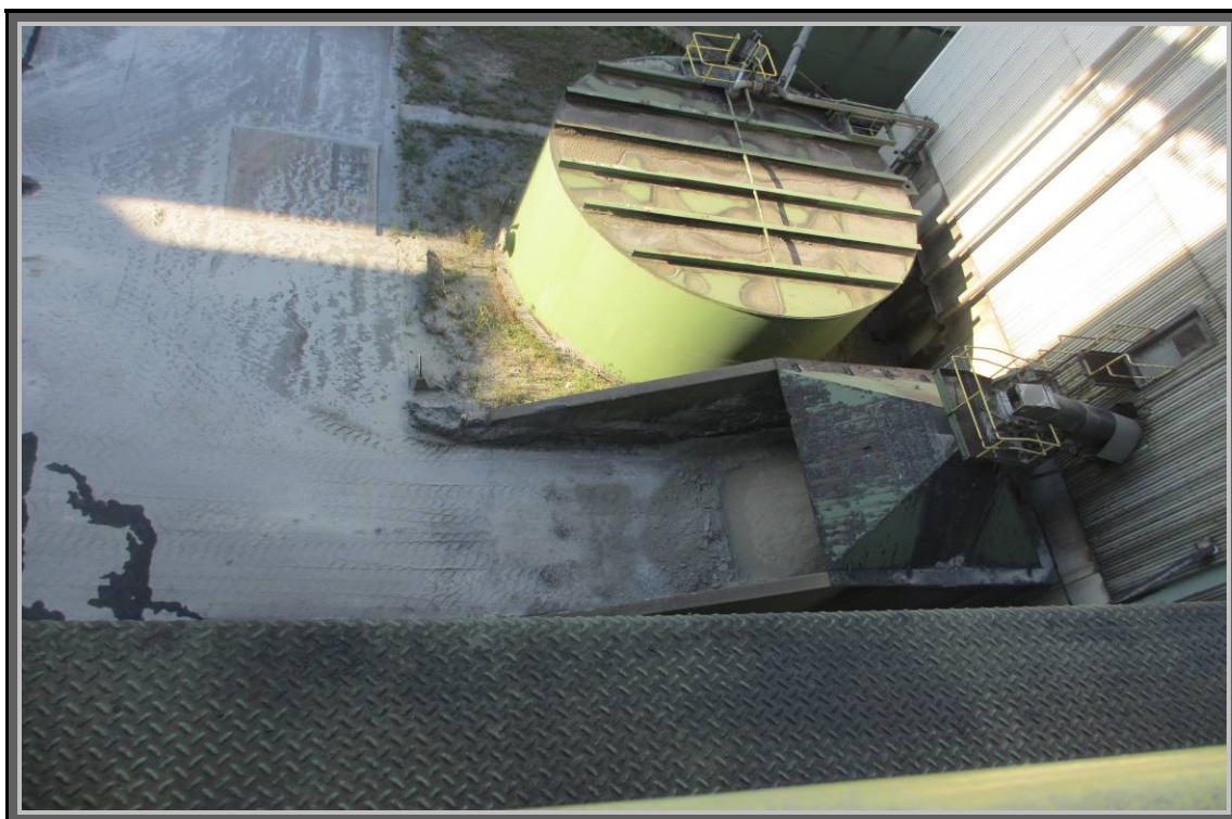
Photo 5. Looking down from Power Plant (SW) at Gypsum Bunker _JB Sims Power Plant_082212
