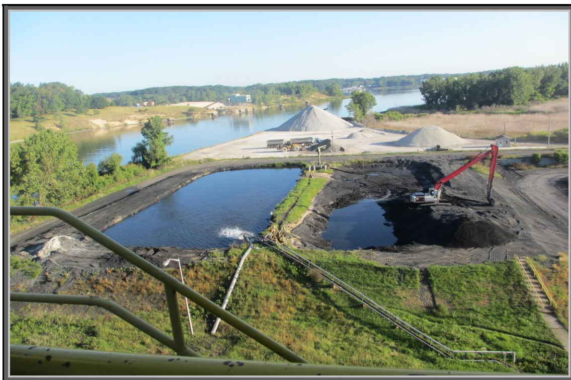
Photo 2. Looking N at E and W Ponds _JB Sims Power Plant_082212
