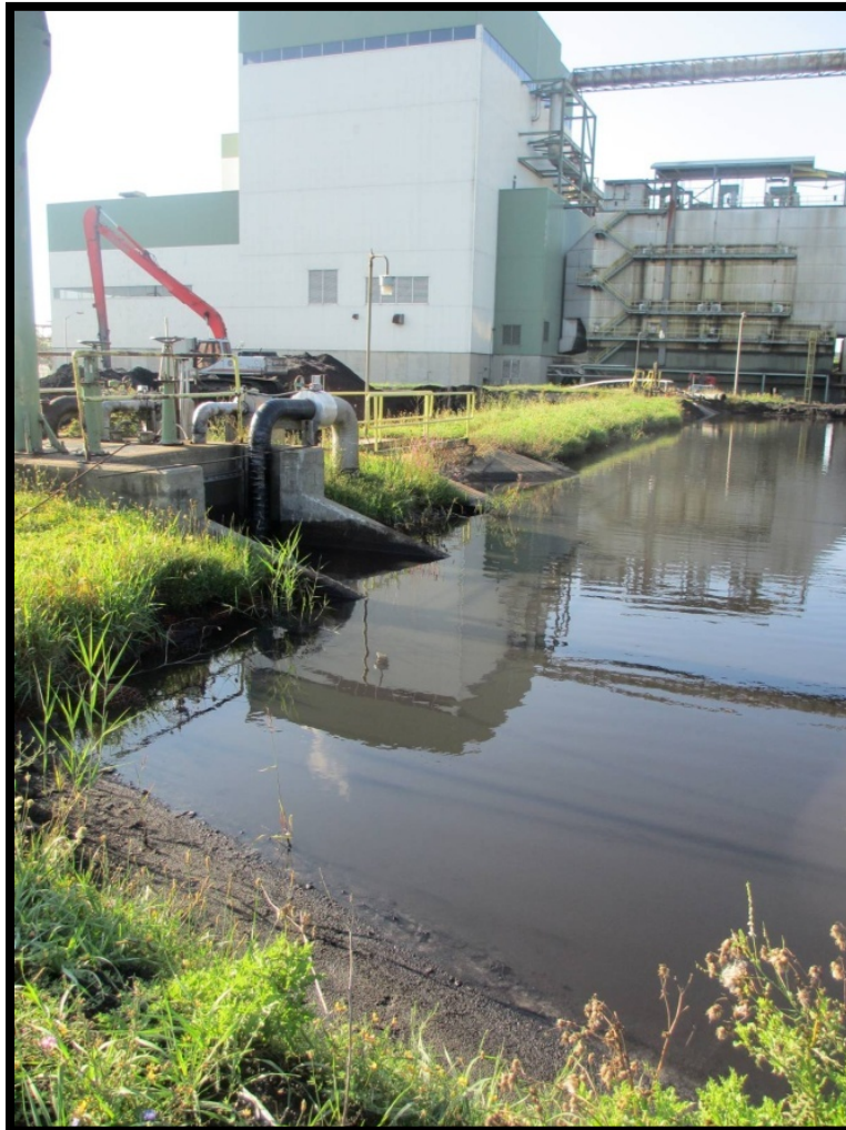
Photo 5.3.2: East embankment of West Pond (divider dike)
