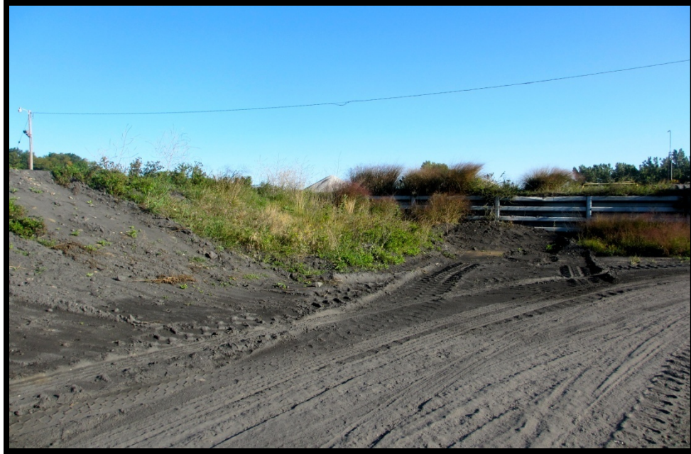
Photo 5.2.3d: Northeast toe corner of East Pond
