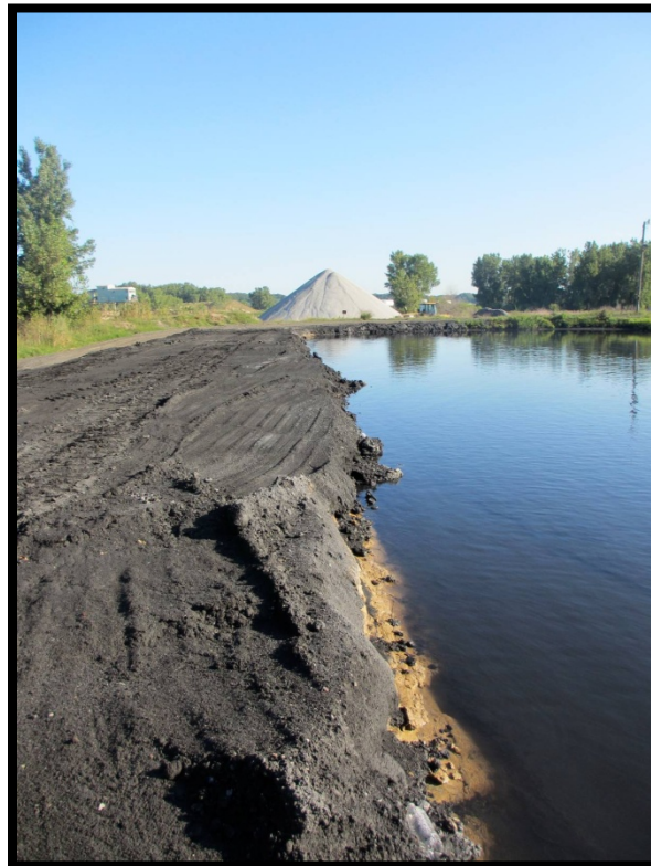
Photo 5.3.1d: Looking north along West Pond's west embankment (note visibility of clay liner)
