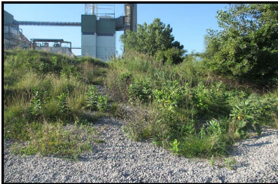
Photo 5.3.3c: Northwest toe at northwest corner of West Pond
