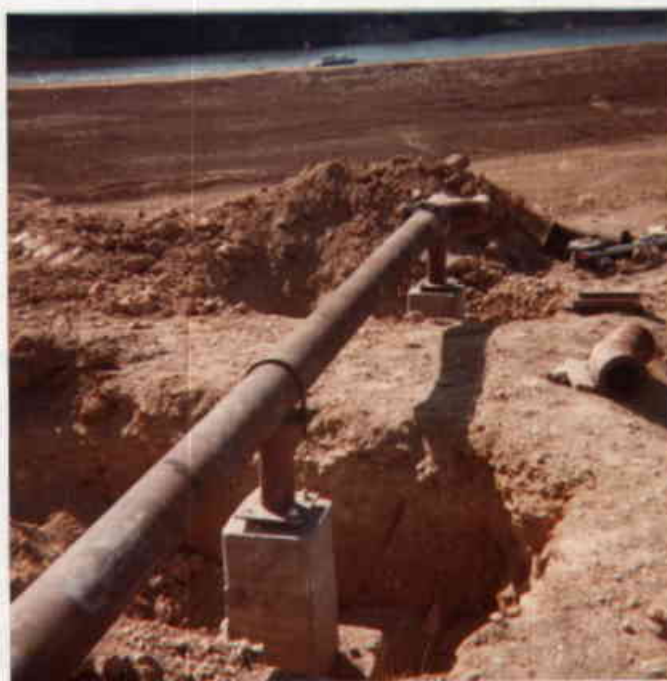
70. Bottom ash line installation at the south end of the center dike.
