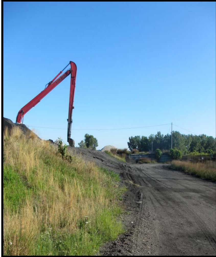
Photo 5.2.3b: Looking north along eastern embankment and toe of East Pond
