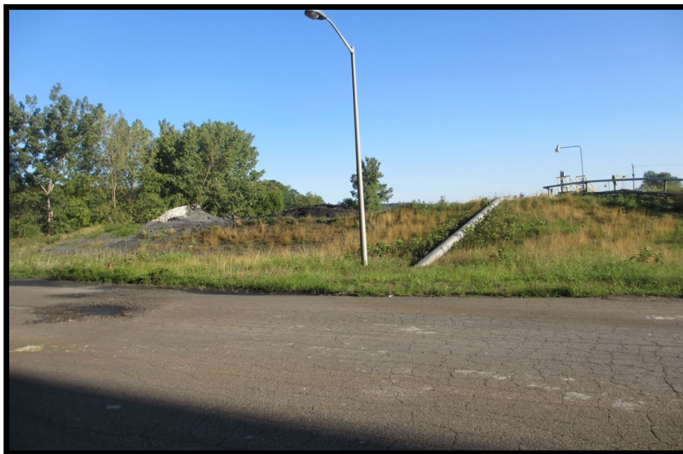
Photo 5.3.3a: Looking north from plant at West Pond's southern embankment (observed height approximately 8-10 ft)
