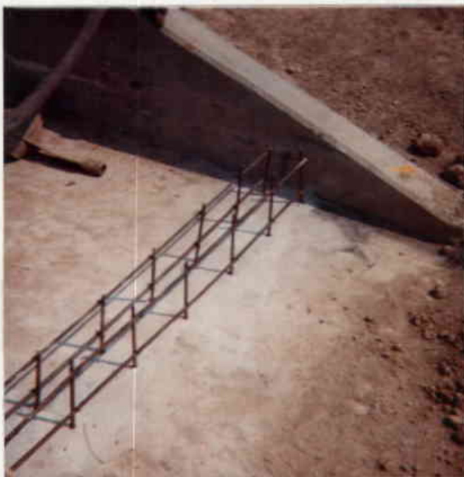
54. Re-steel set in place for the stop log wall at the west end of the structure.
