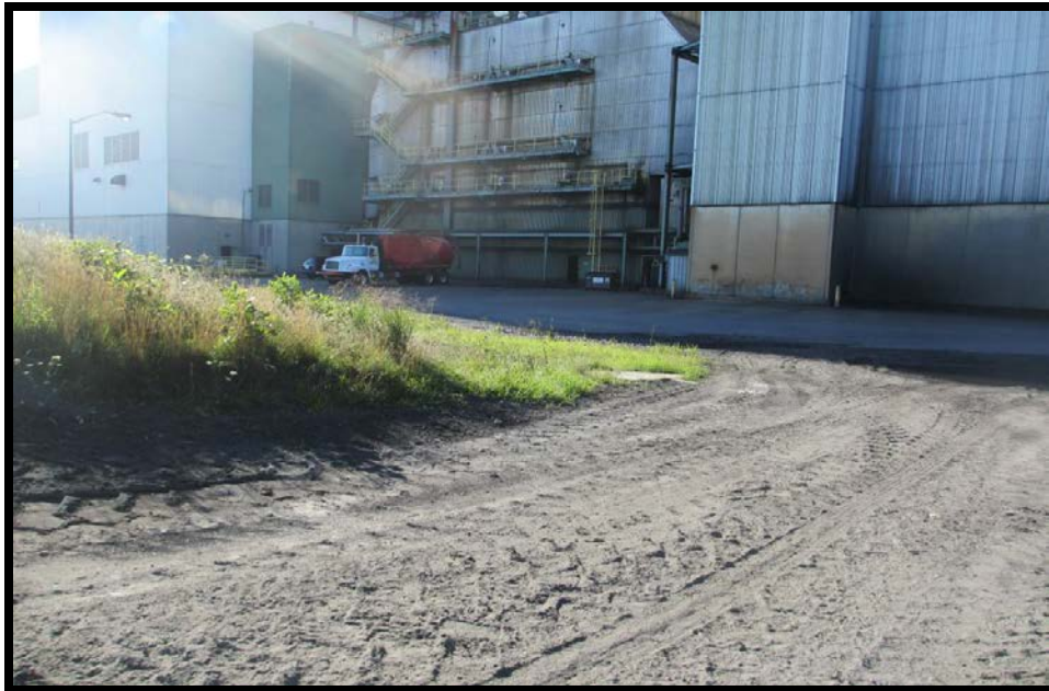
Photo 5.3.3d: West Pond's southwest corner/toe
