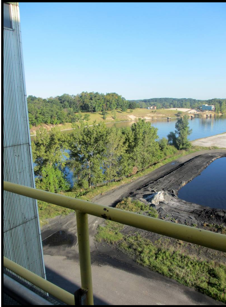
Photo 5.3.3e: Looking northwest from plant; water course is the Grand River. Note two wet areas along toe of West Pond at west and southwest locations; plant personnel said this is from rain and a surface that is not very permeable.
