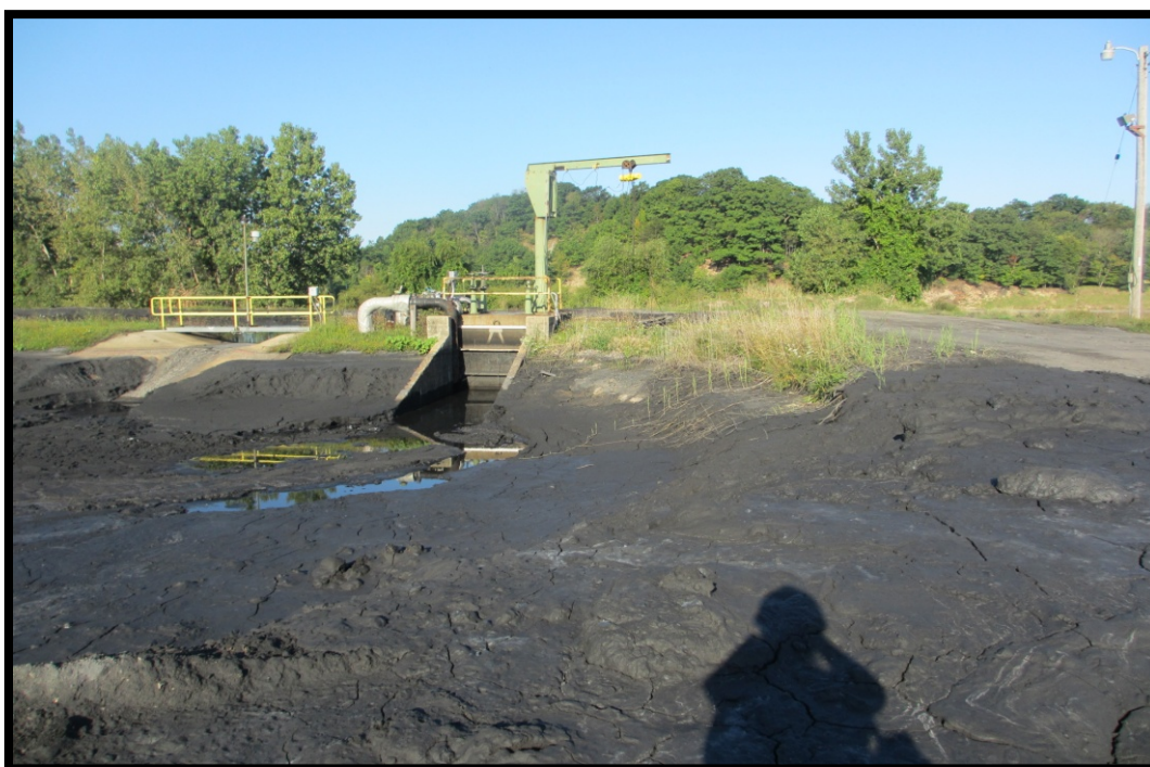
Photo 5.4.1a: Northwest corner of East Pond
