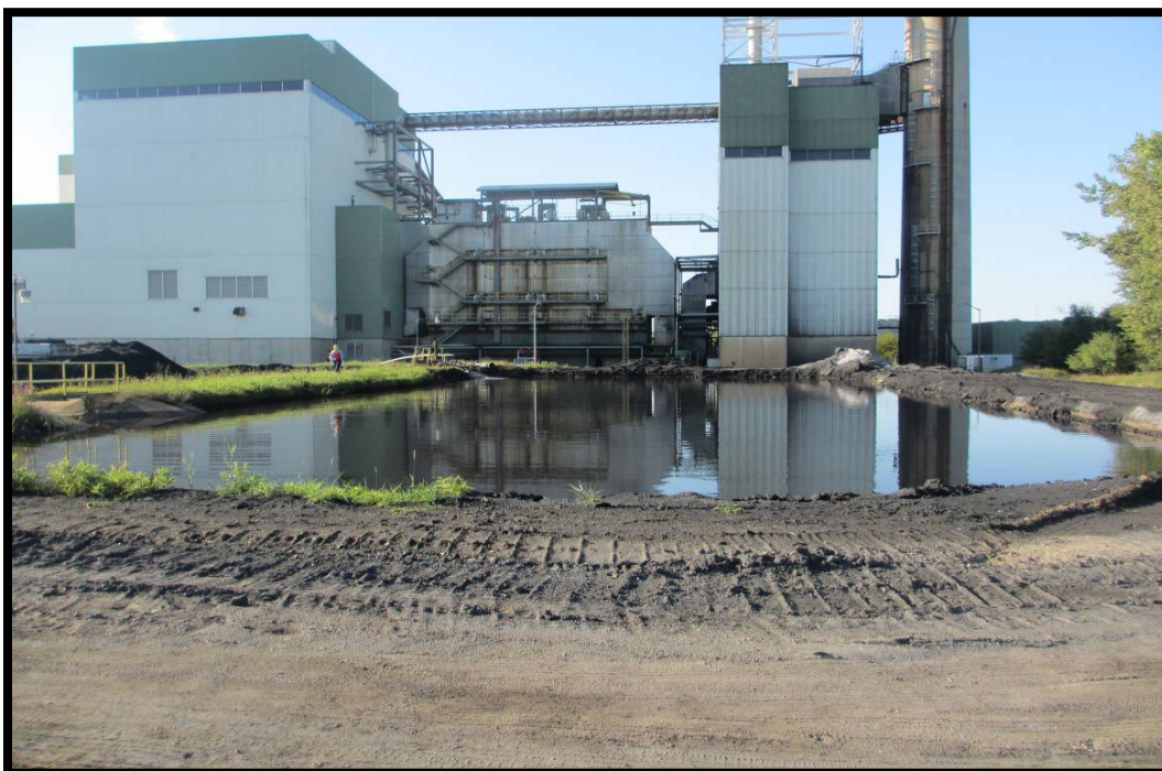
Photo 5.3.1a: Looking southeast at West Pond
