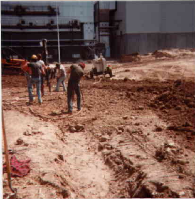
37. Hand compaction of clay along the ASA-A pipe trench.
