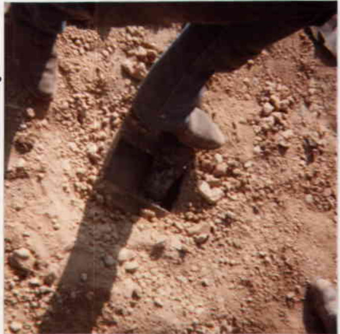
59. Pumping bentonite slurry into the backfilled culverts.
