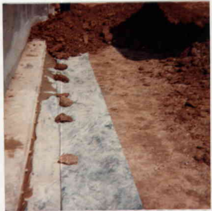
34. Hypalon membrane lapped and ready for burial.
