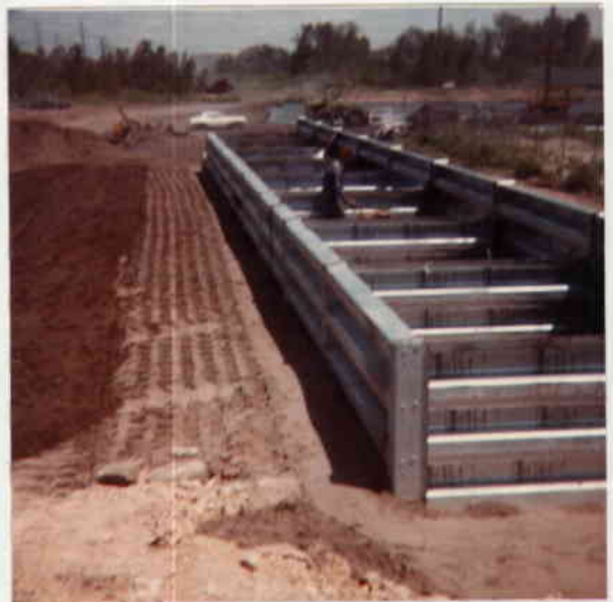
66. Hand compaction of granular backfill in the bin retaining wall
