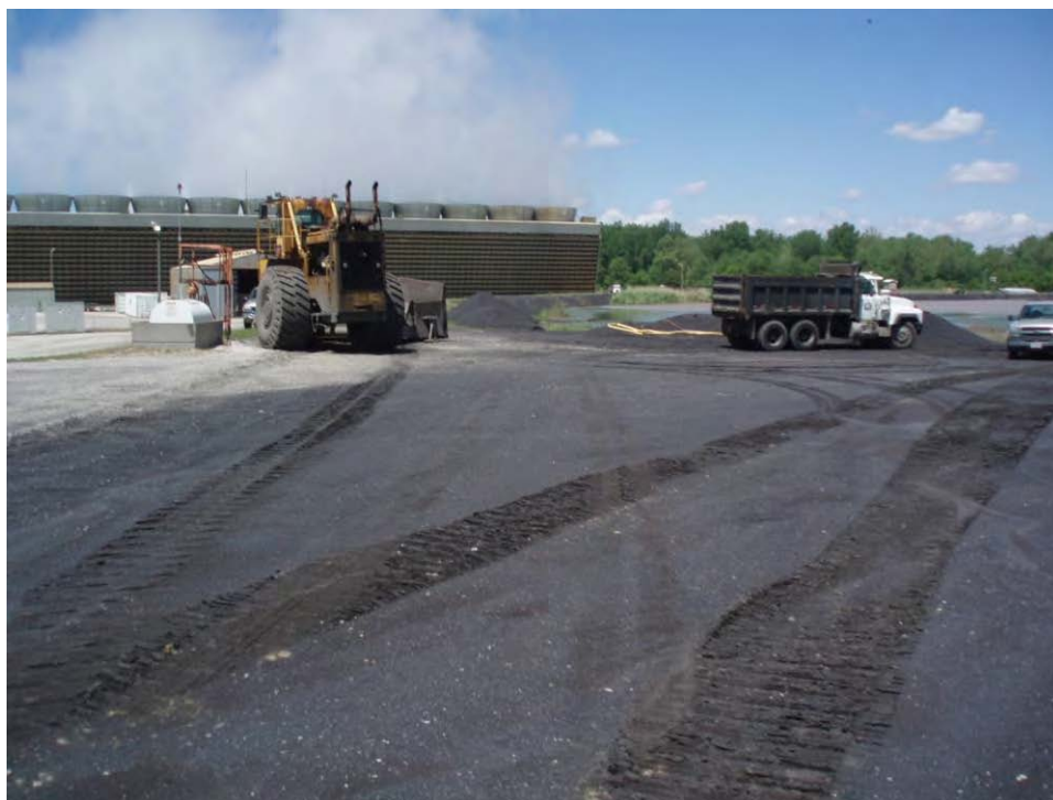
14. Pond A - South embankment crest, looking northwest.
