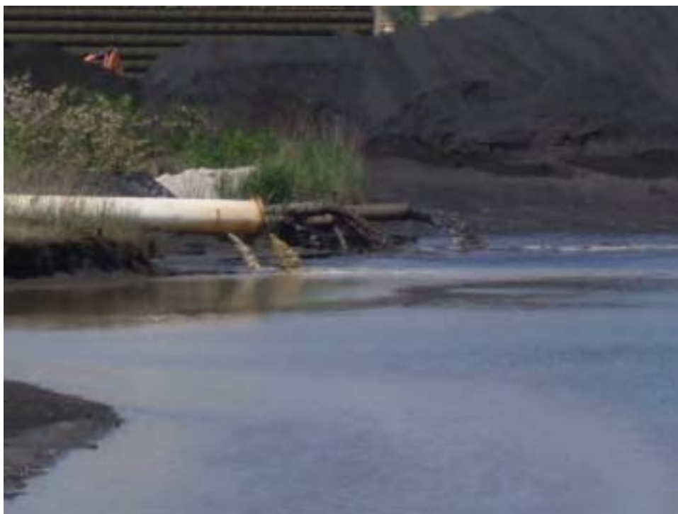
8. Close up of two (2) 36-inch-diameter and five (5) 10-inch-diameter DI sluice pipes.
