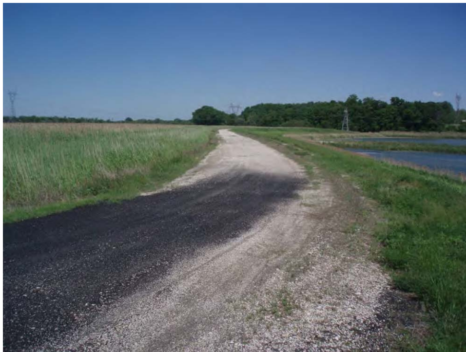
67. Pond B - South embankment crest, looking northeast.
