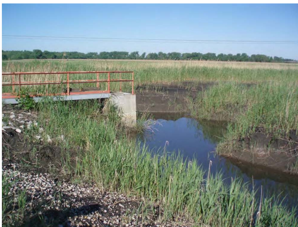
132. Pond C - Outlet structure with stoplogs, looking southwest. Note water level 6.6' below crest at outlet.
