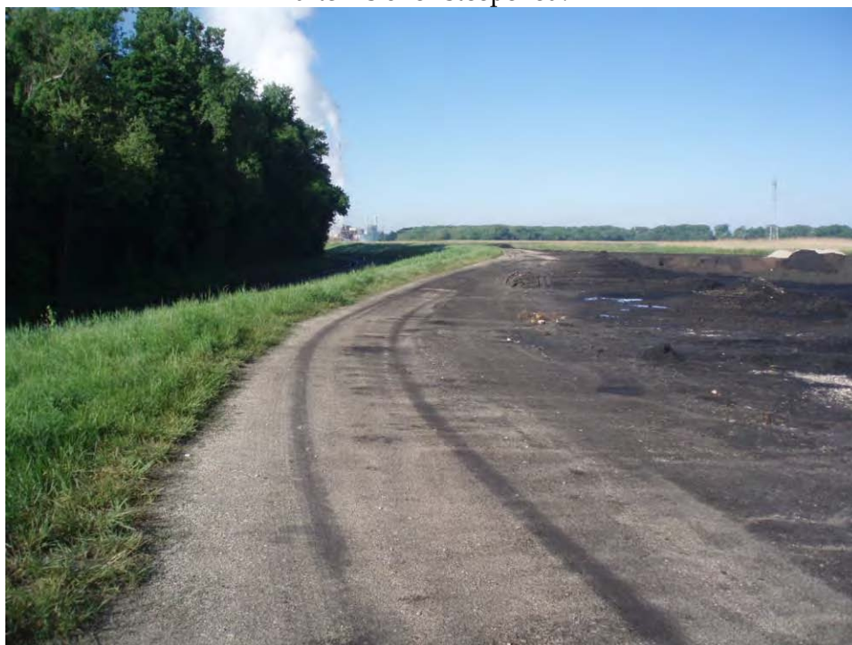
128. Pond C -East embankment crest, looking southwest. Note tire rutting was observed in very soft stabilized FGD near the crest.
