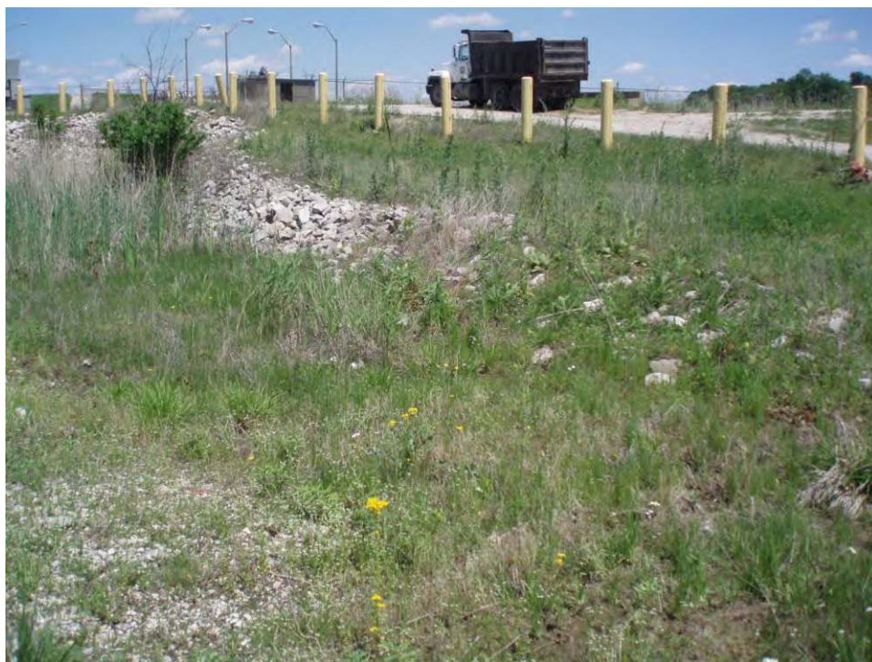
34. Pond A - Former location of Lick Creek at west embankment exterior toe.
