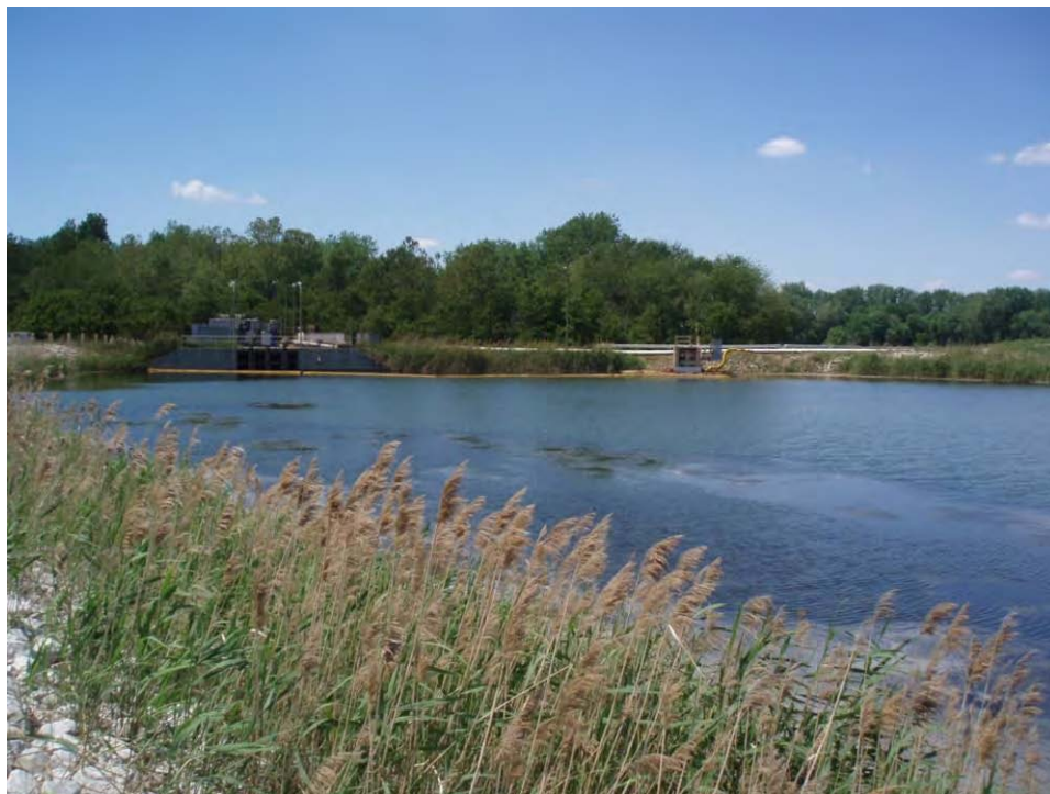
41. Overview of Pond A - Discharge recycle pump station and outlet structure, looking west
