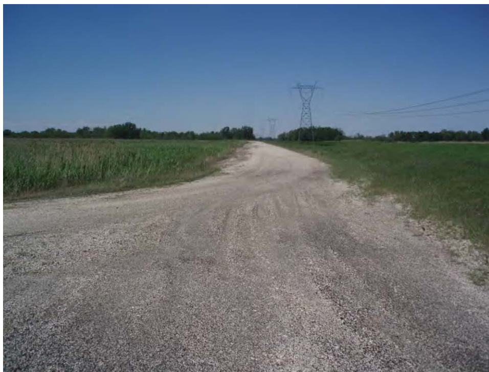
54. Pond B - East embankment crest, looking north.
