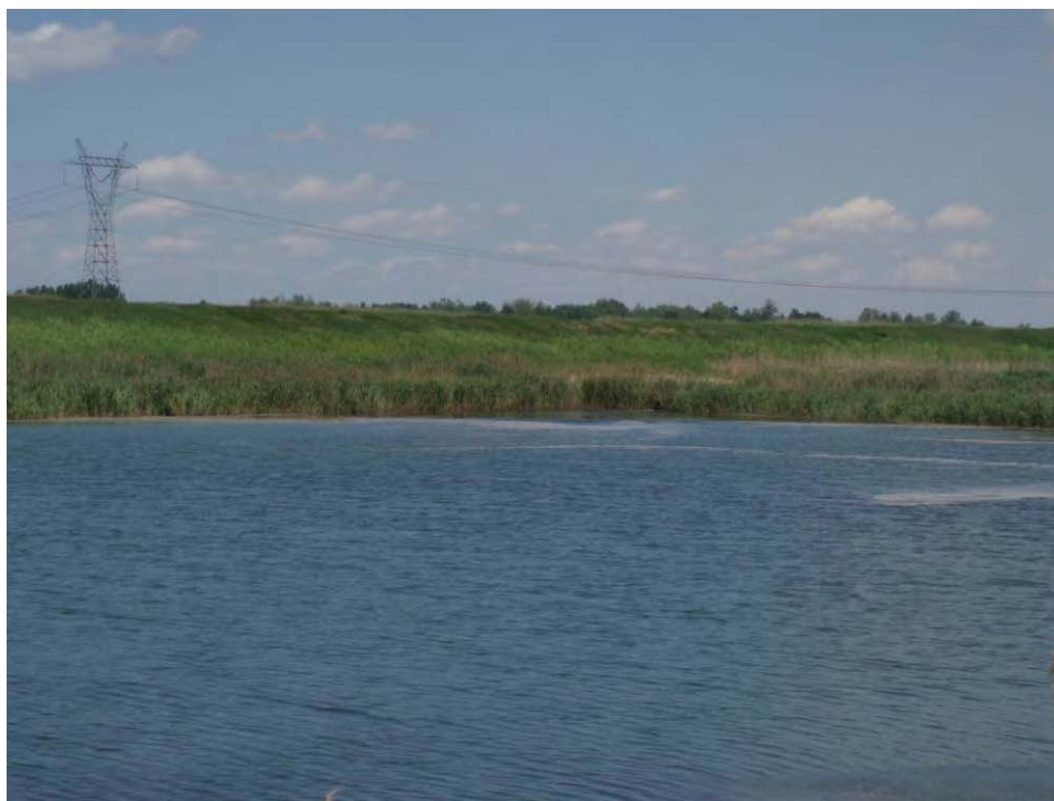
42. Overview of Pond A - Discharge, looking northeast at inlet pipes from Pond A.
