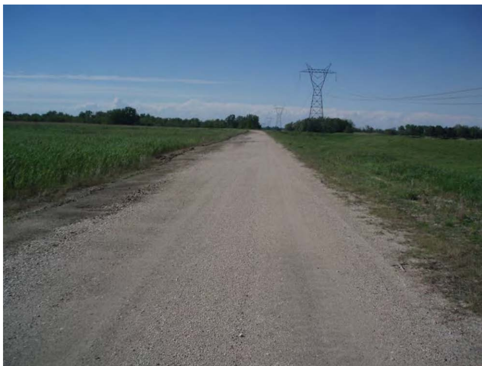
98. Pond B - North embankment crest, looking northwest.
