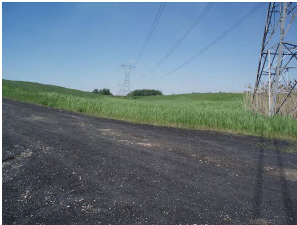
50. Pond B - North embankment exterior slope, looking northwest between Pond B and Pond C.
