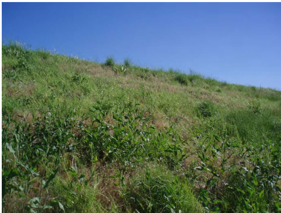
88. Pond B - West embankment lower exterior slope, looking southwest.
