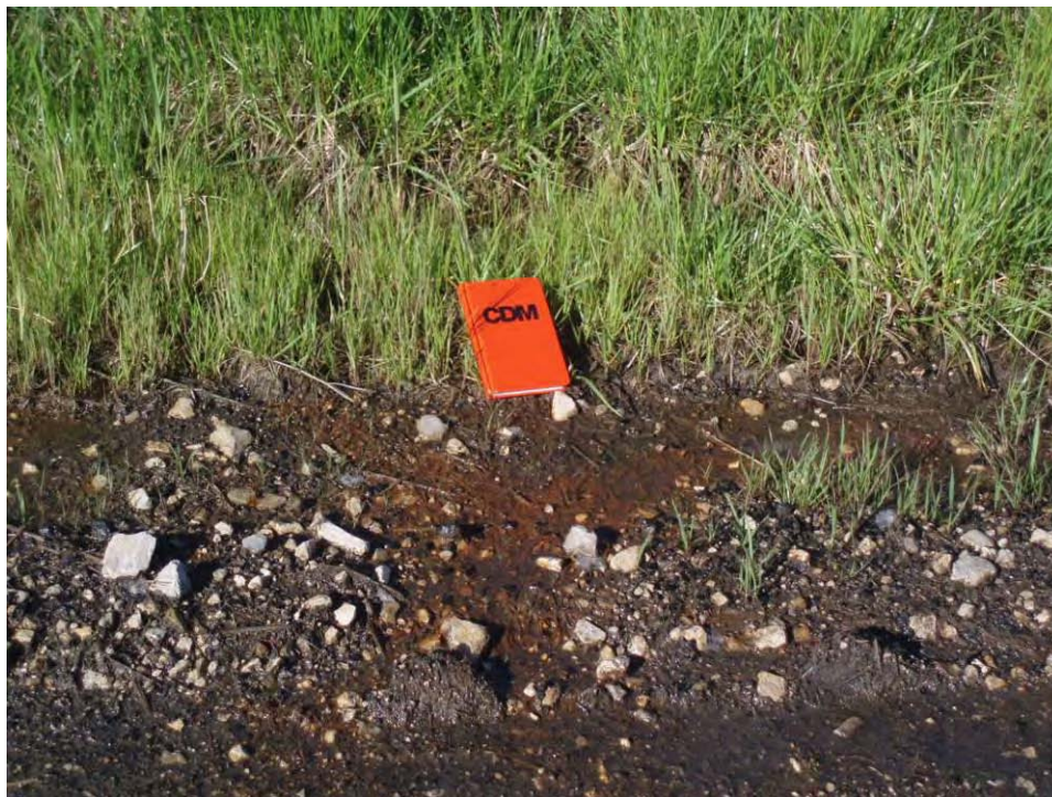
125. Pond C - North embankment bench, looking at active seepage located at toe of upper exterior slope. Note the iron staining in the water
