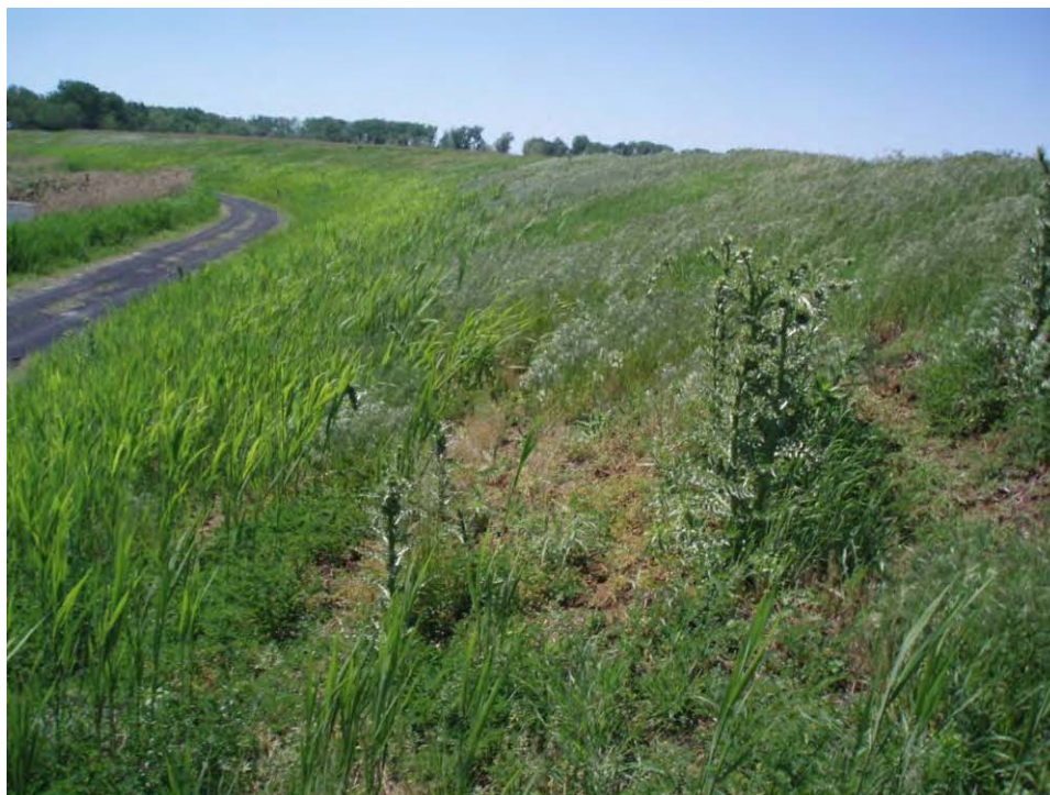
58. Pond B - South embankment exterior slope, looking west at tractor rutting and minor surficial erosion. Note change in vegetation at mid slope and stabilized FGD material very soft.
