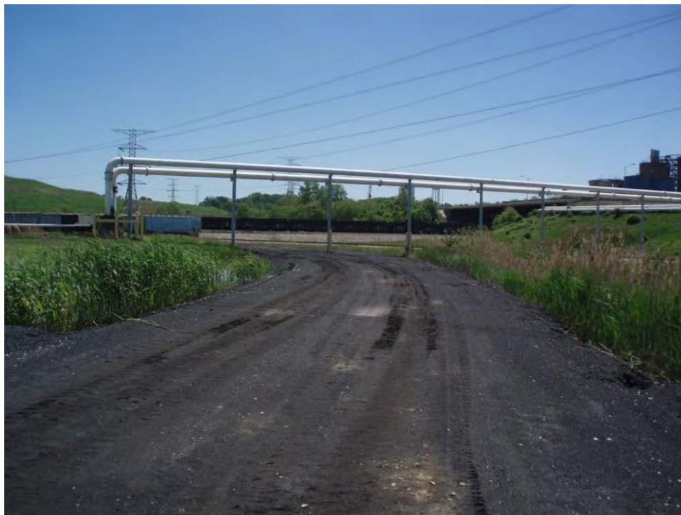
11. Pond A - South embankment looking southeast.
