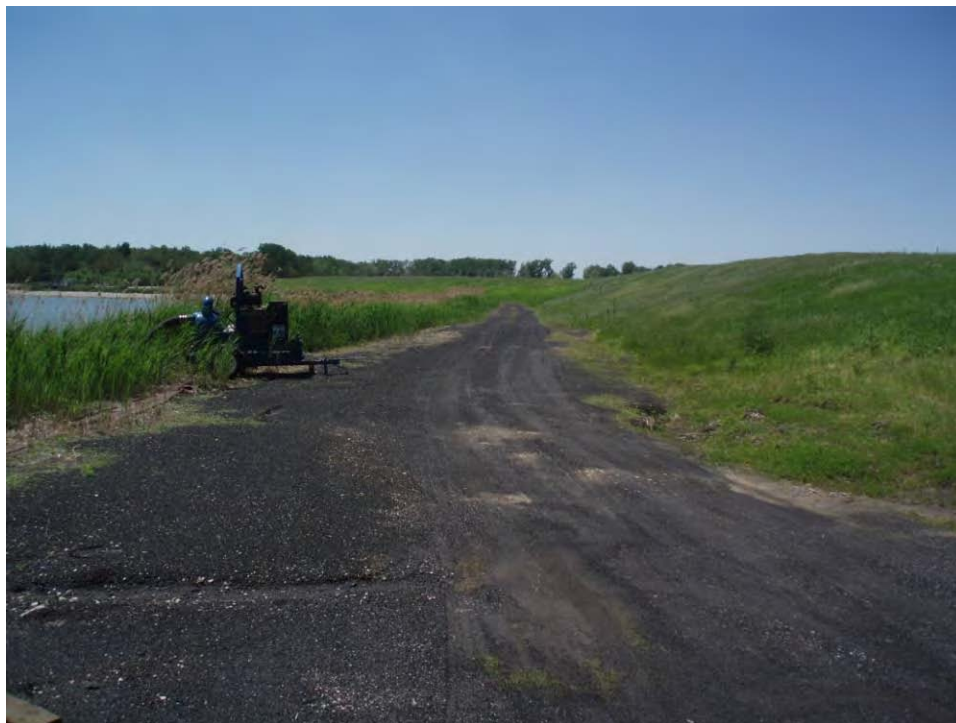
49. Pond A - North embankment crest and Pond B - South embankment exterior slope, looking west.
