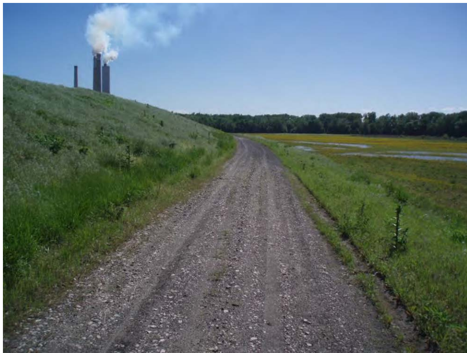
89. Pond B - West embankment bench, looking southwest.
