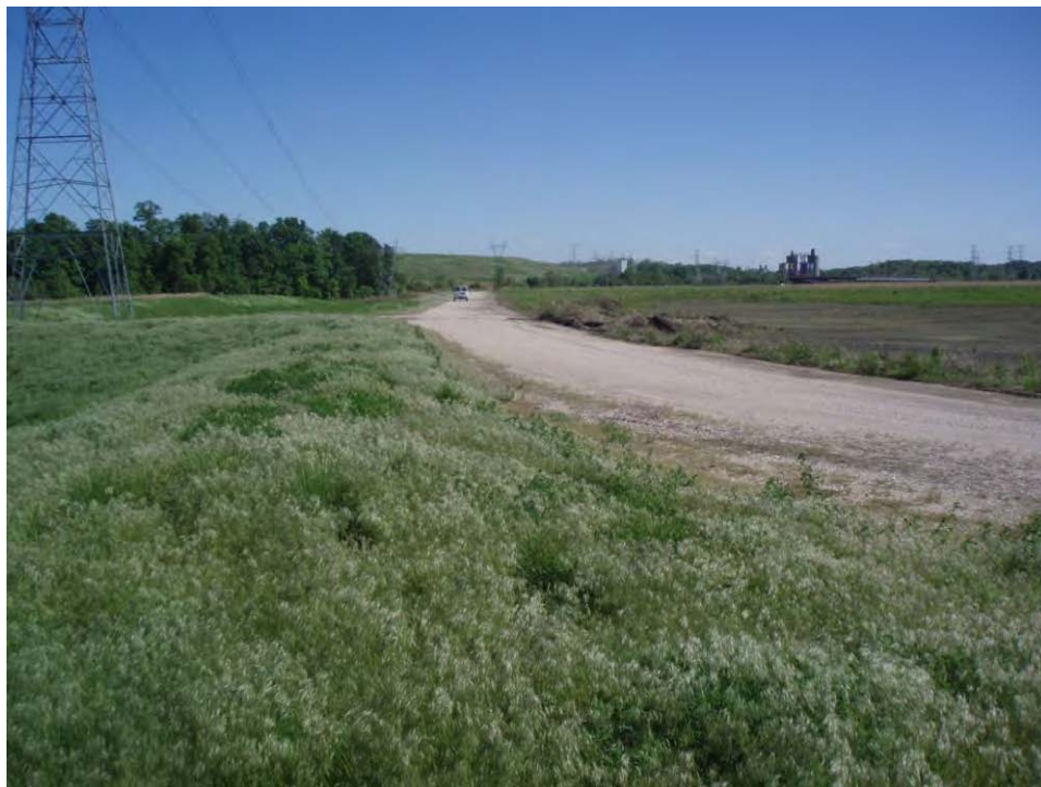
93. Pond B - North embankment crest, looking southeast.
