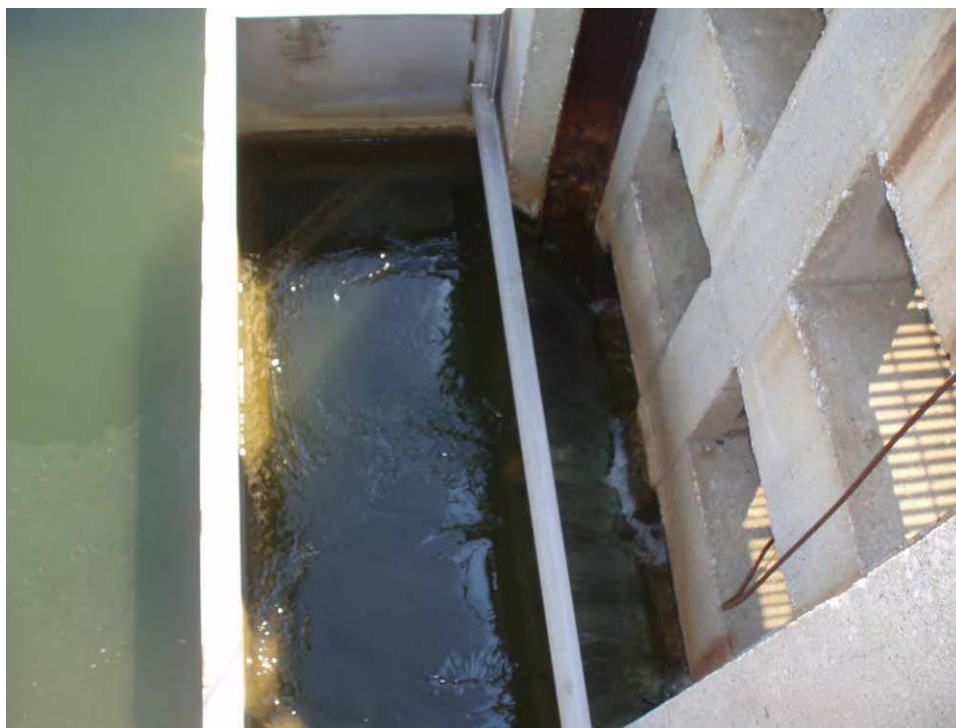
72. Pond A - Discharge, looking south at inlet to outlet control structure.
