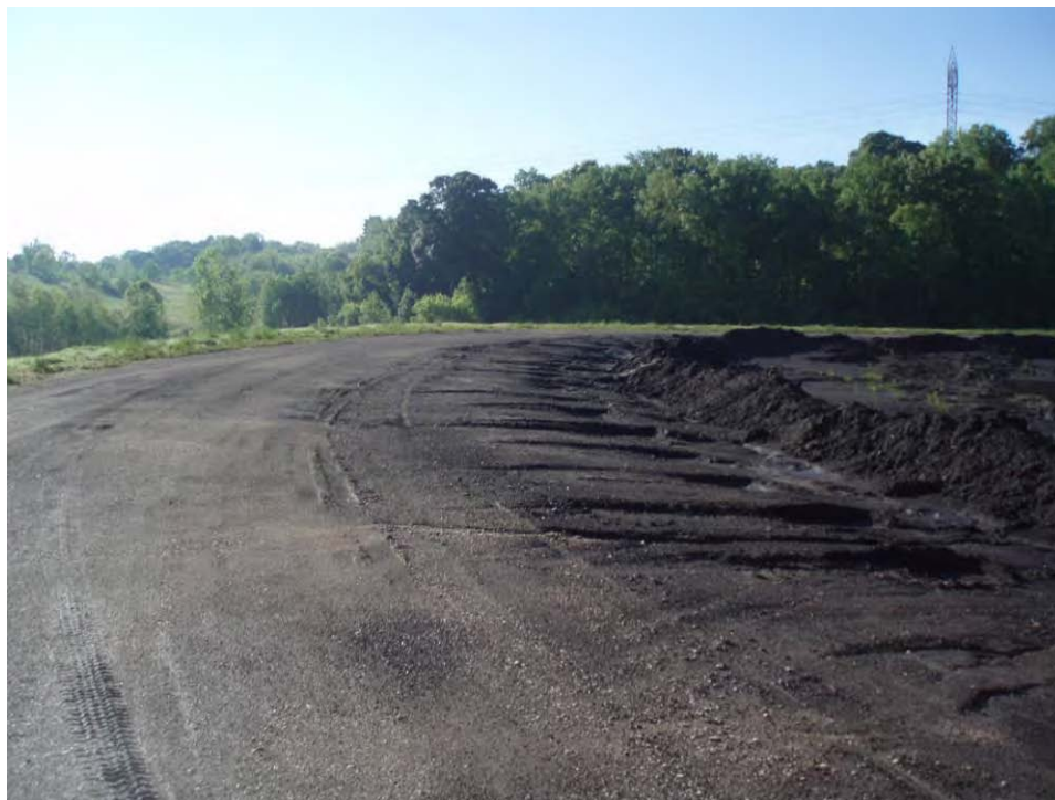
121. Pond C - North embankment crest, looking southeast.
