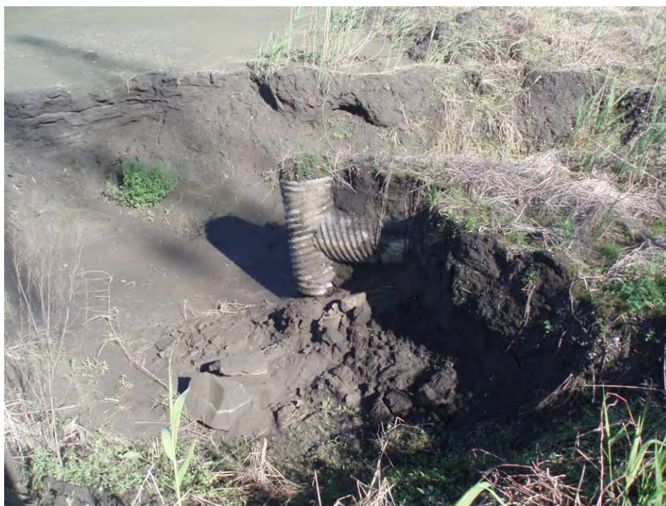
146. 24-inch-diameter CM equalizer pipe from Pond B to Pond C. Note inlet has a T connection on the end of the pipe and is filled with ash.
