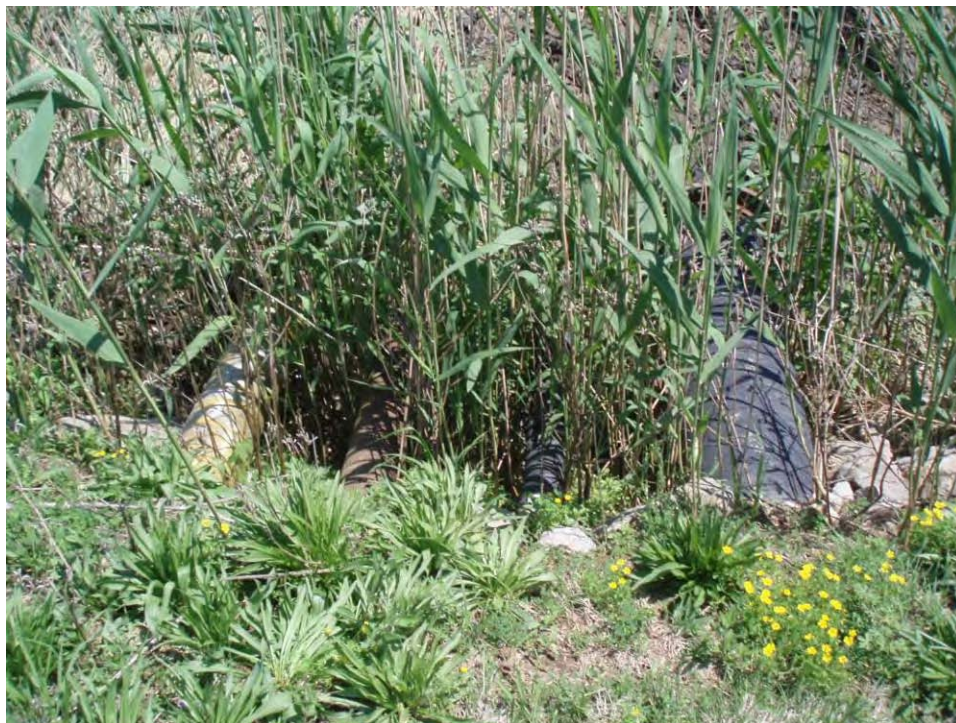
35. Pond A - Looking east at inactive 4-, 6-, 8-, and 15-inch-diameter sluice pipes from unknown origin. Use unknown.
