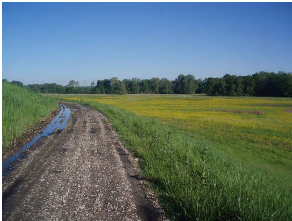
123. Pond C - North embankment bench, looking northwest.
