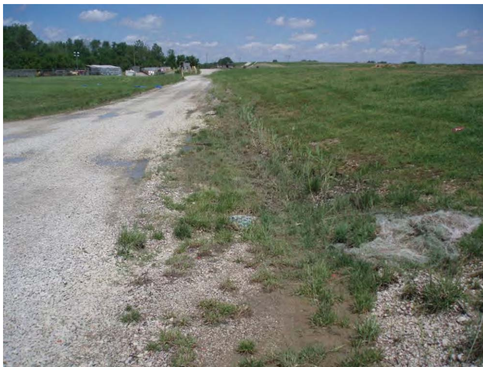
24. Drainage ditch at toe of Pond A west embankment. Note ditch has sparse vegetation.
