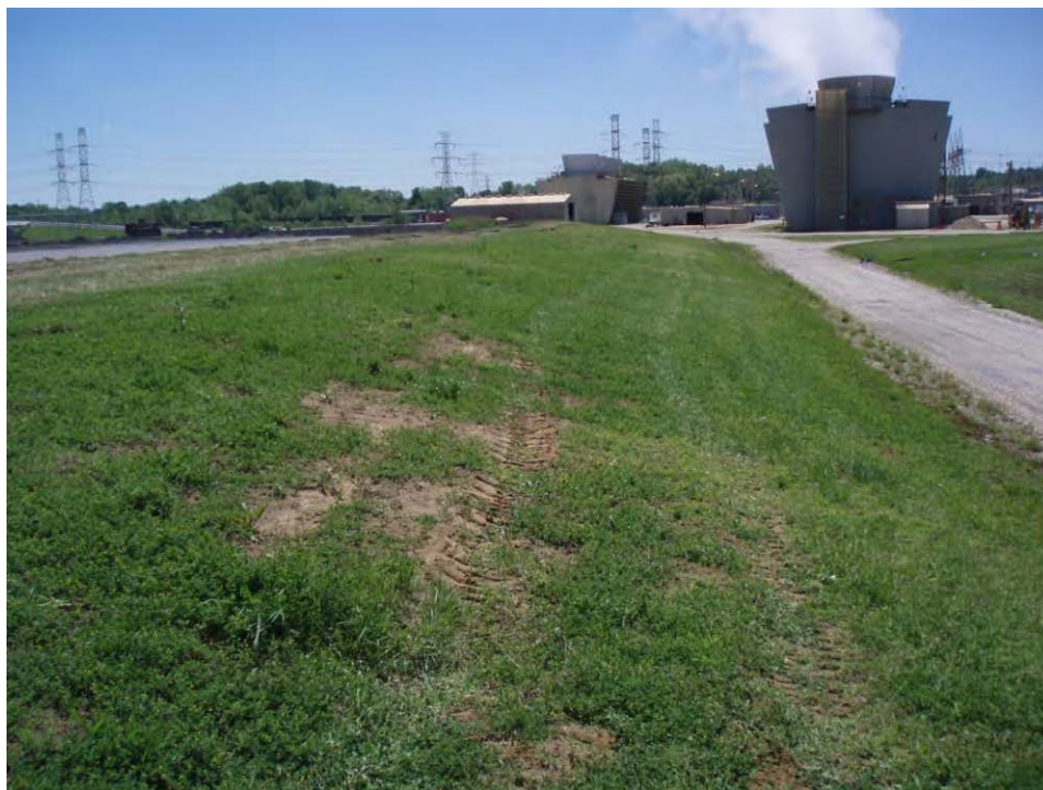
28. Pond A - West embankment exterior slope, looking south.
