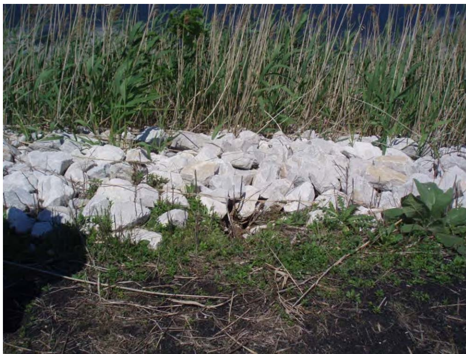
40. Surficial erosion under riprap on north slope of divider embankment between Pond A and Pond A - Discharge.
