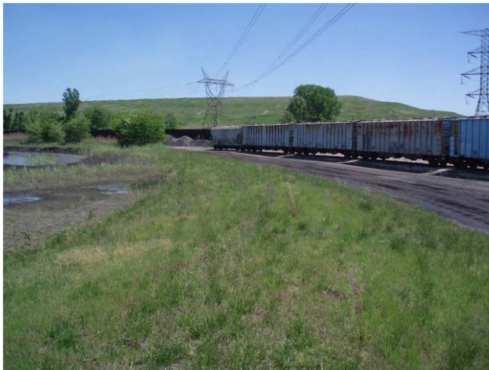
9. Pond A - South embankment crest, looking east.
