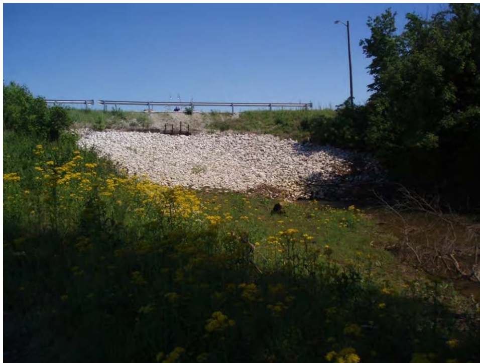
71. Pond A - Discharge, overview of downstream area from outfall.
