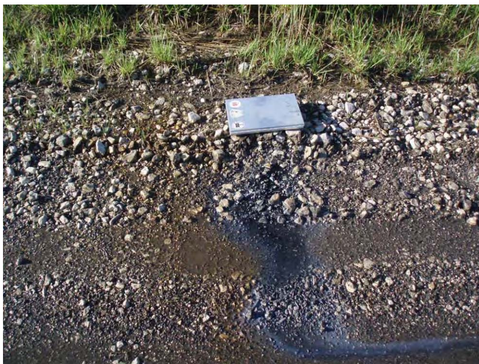
116. Pond C - West embankment bench, looking at active seepage located at toe of upper exterior slope. Note the white and black sheen in the water.
