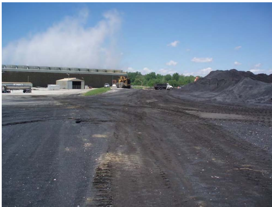
12. Pond A - South embankment crest, looking northwest.
