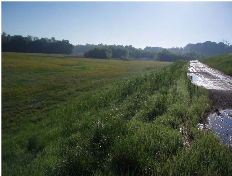
113. Pond C - West embankment bench, looking east.
