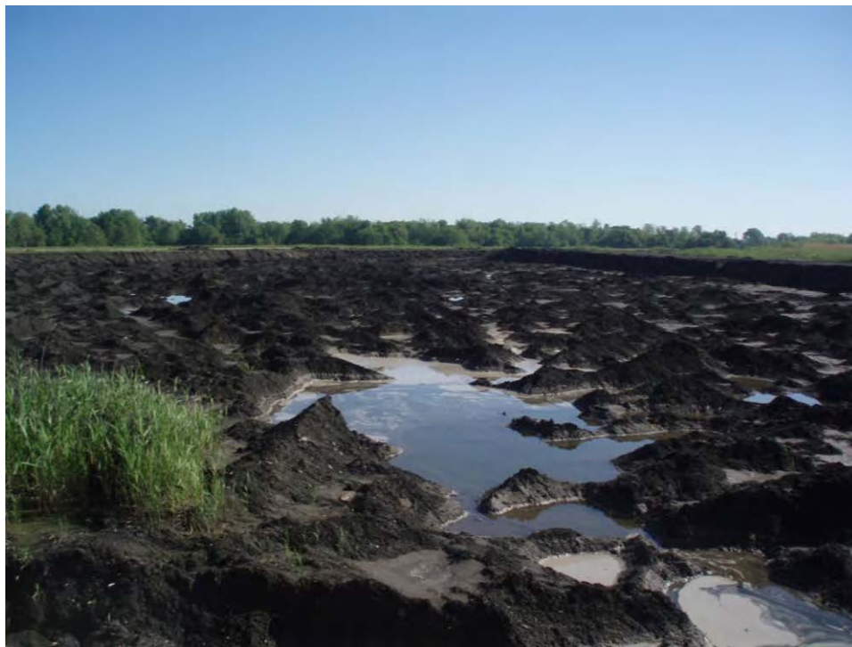
143. Overview of Pond C, looking northeast.
