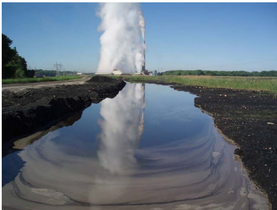
134. Pond C - East embankment interior slope, looking southwest at rim ditch to outlet structure. Note water level 3' below crest.
