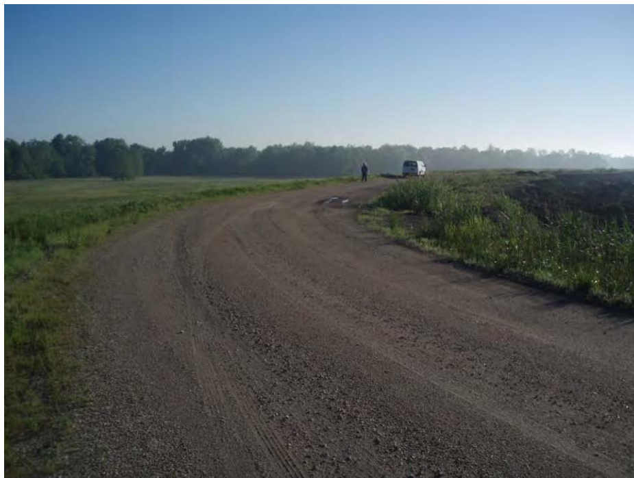
99. Pond C - West embankment crest, looking northeast.
