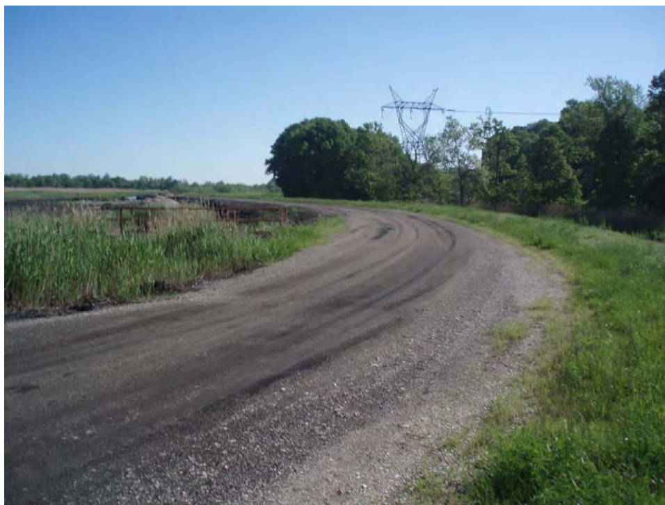
136. Pond C - East embankment crest, looking northeast.
