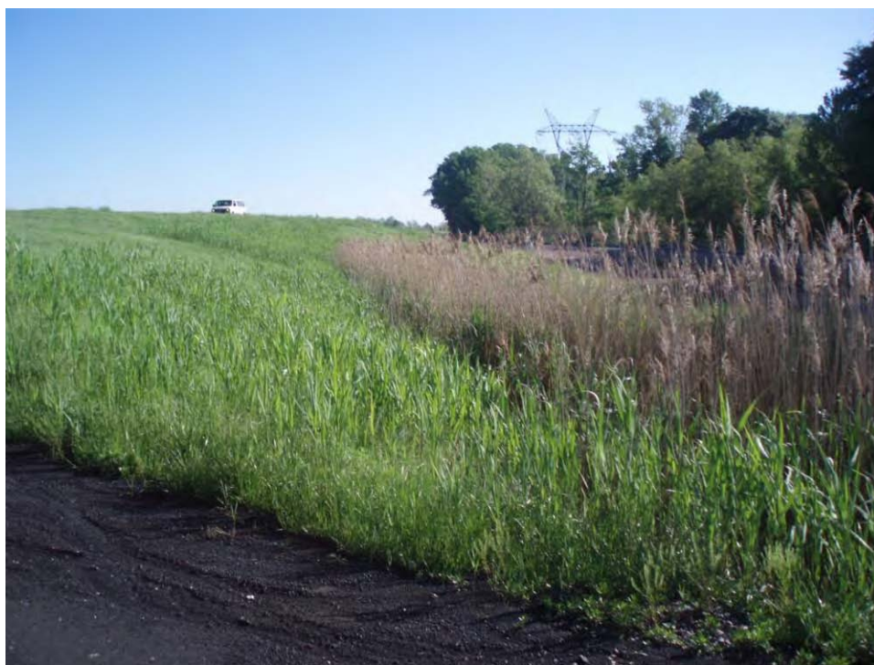
130. Pond C - East embankment exterior slope and drainage ditch, looking northeast.
