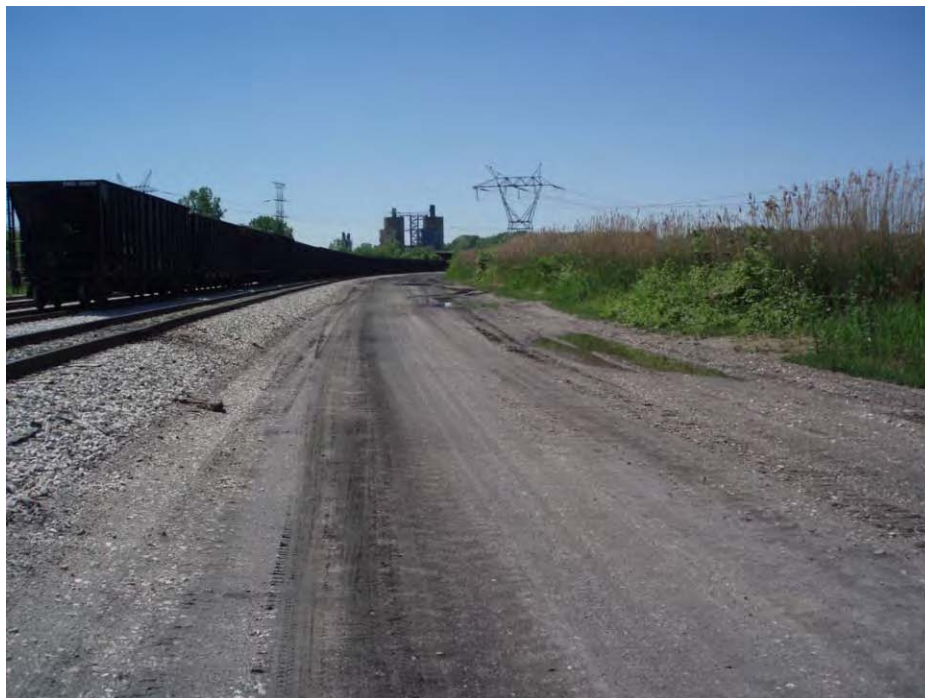
3. Pond A – East embankment crest, looking south.
