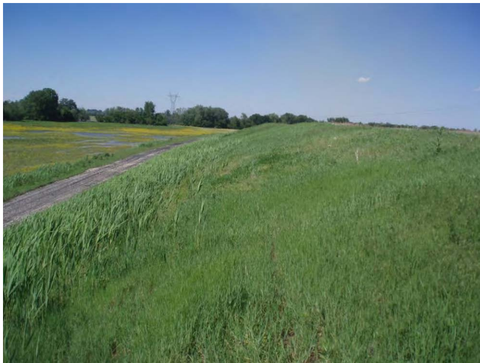
83. Pond B - West embankment upper exterior slope, looking north.
