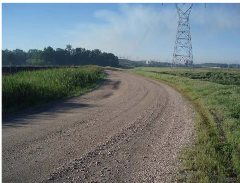
100. Pond C - South embankment crest, looking southeast.
