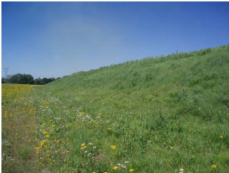
81. Pond B - West embankment lower exterior slope, looking north.
