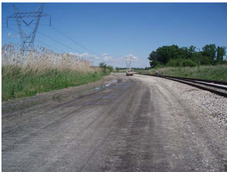
4. Pond A – East embankment crest, looking north
