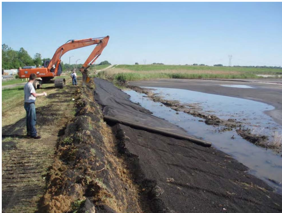
31. Pond A - West embankment interior slope, looking north at rough embankment grading. Note Mirafi geofabric does not extend to the toe of the slope.
