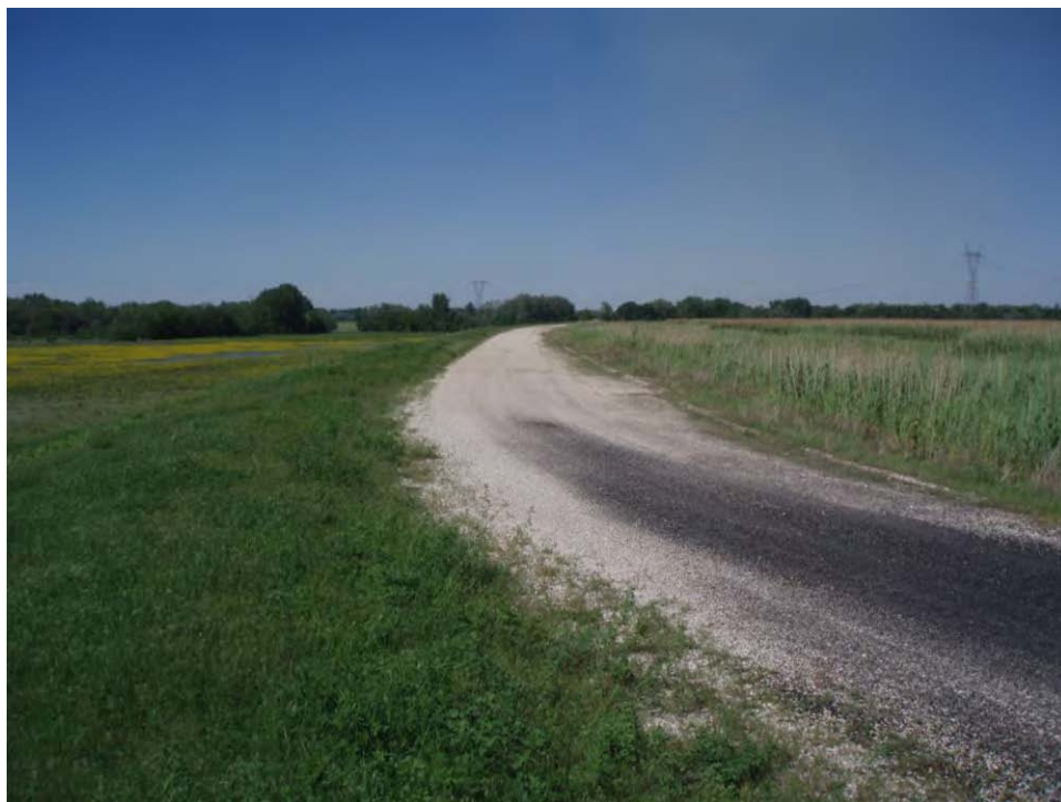
76. Pond B - West embankment crest, looking north.
