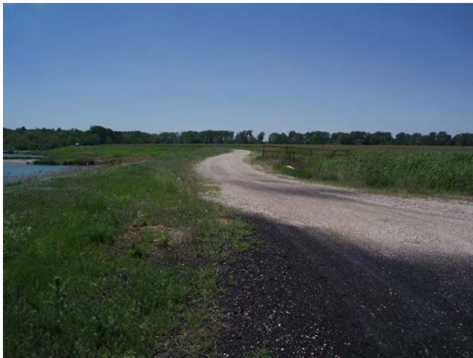
53. Pond B - South embankment crest, looking west.
