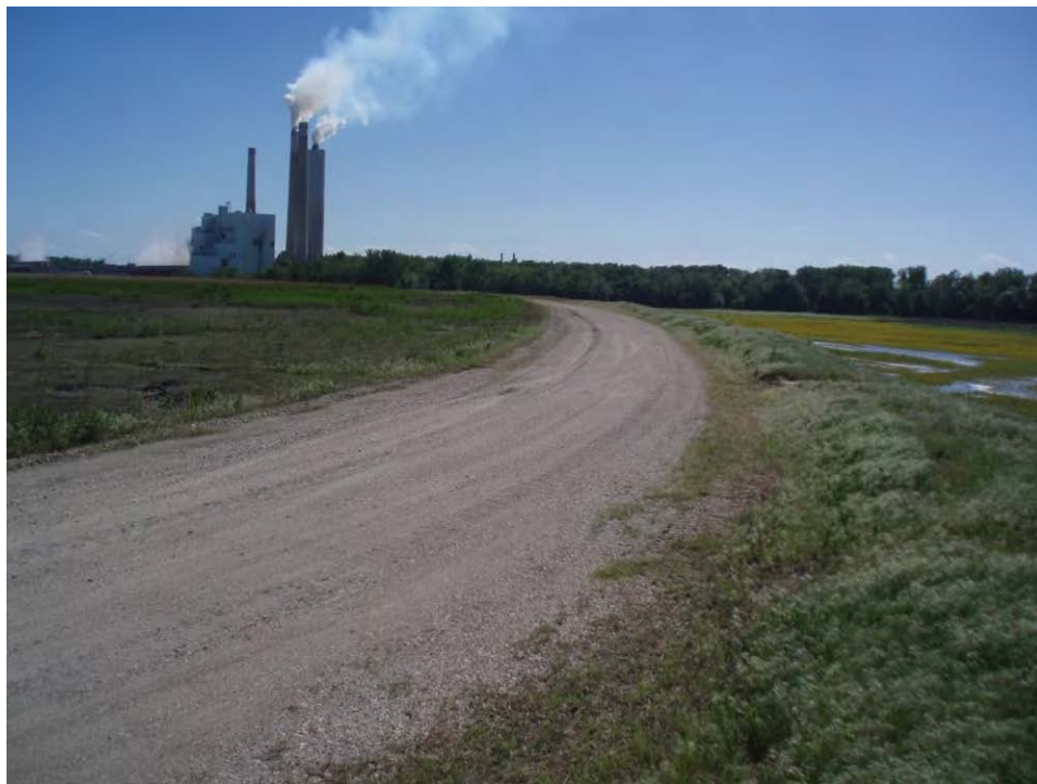
91. Pond B - West embankment crest, looking southwest.
