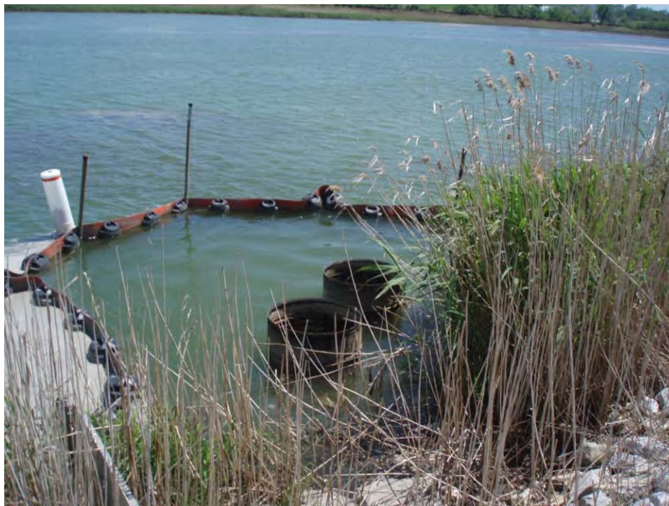
45. Inlet of two (2) 36-inch-diameter CM pipes from Pond A to Pond A - Discharge. Note pipes have T's at inlets and the floating boom to reduce the potential for surface debris from clogging pipes.
