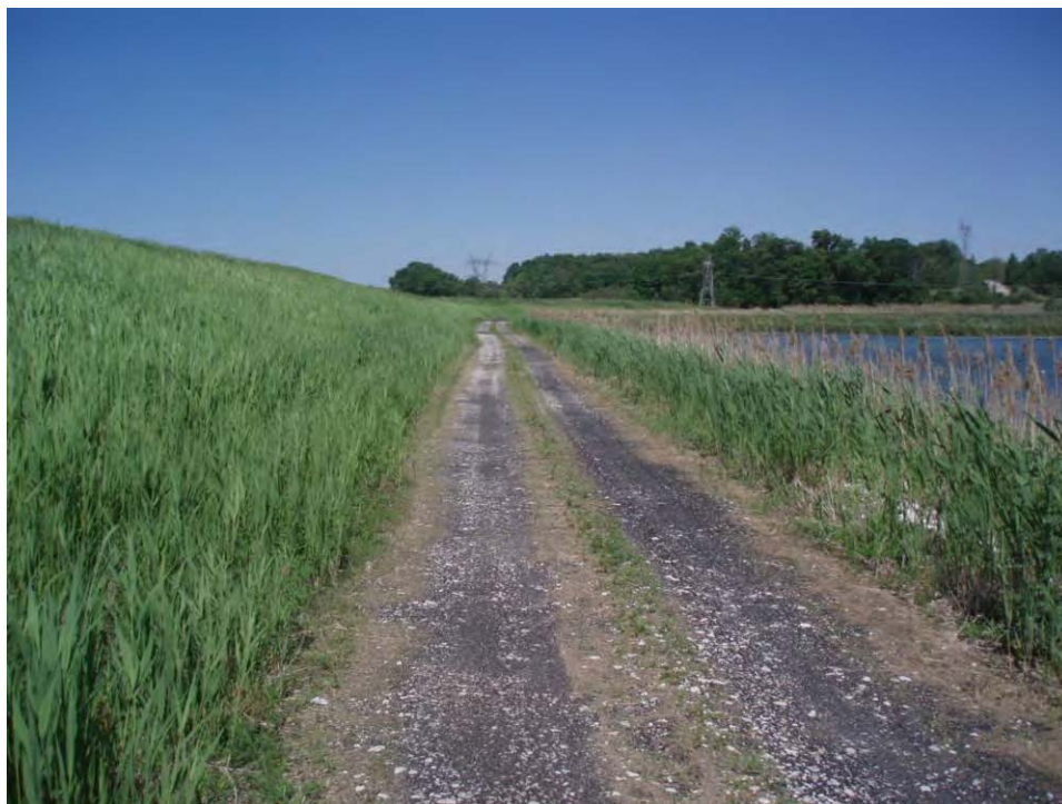
64. Pond A - Discharge north embankment crest and Pond B south embankment toe, looking northeast.
