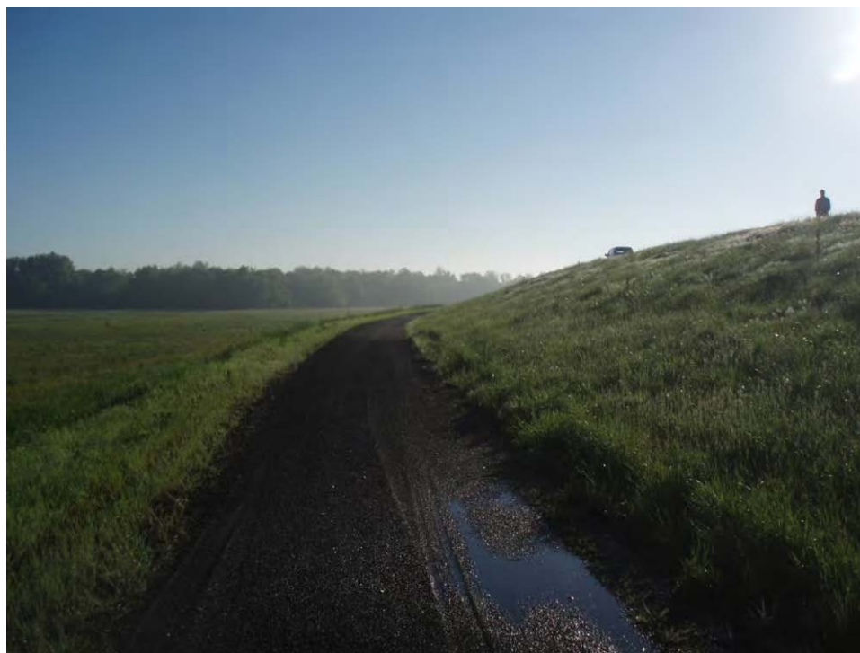
102. Pond C - West embankment bench, looking northeast.
