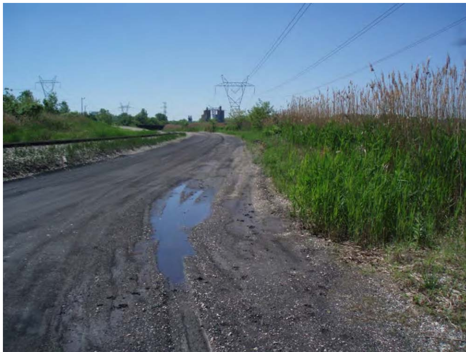
1. Pond A - East embankment crest, looking south.
