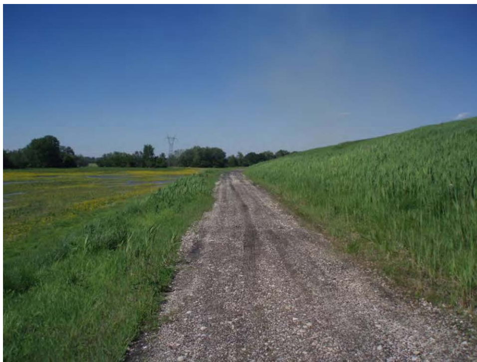
82. Pond B - West embankment bench, looking north.
