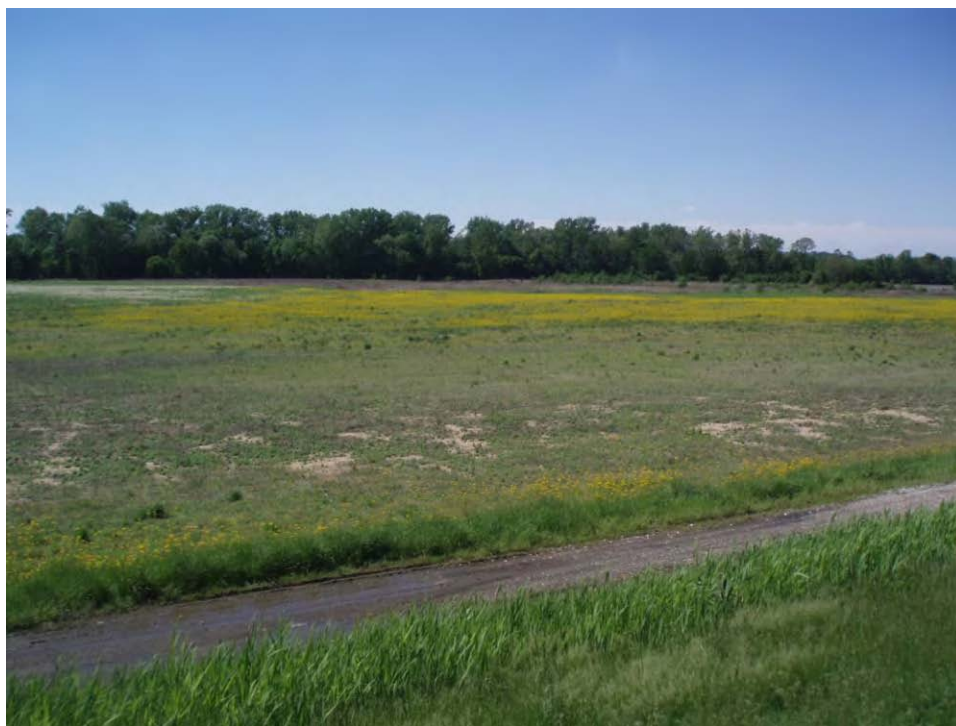
78. Overview of Pond B - West embankment, downstream area, looking west.
