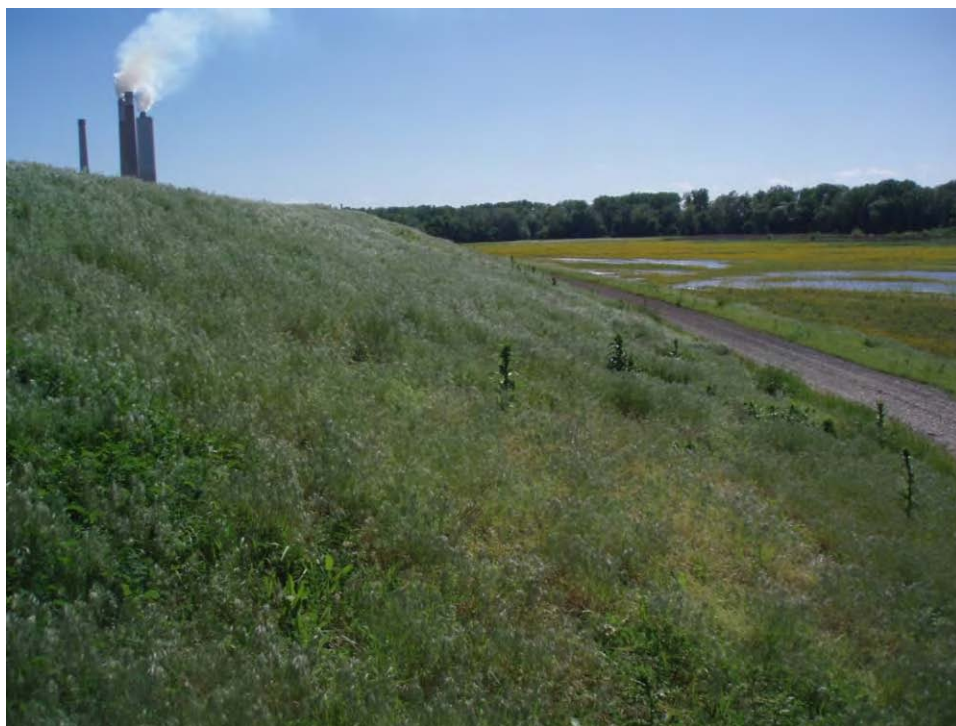
90. Pond B - West embankment upper exterior slope, looking southwest.
