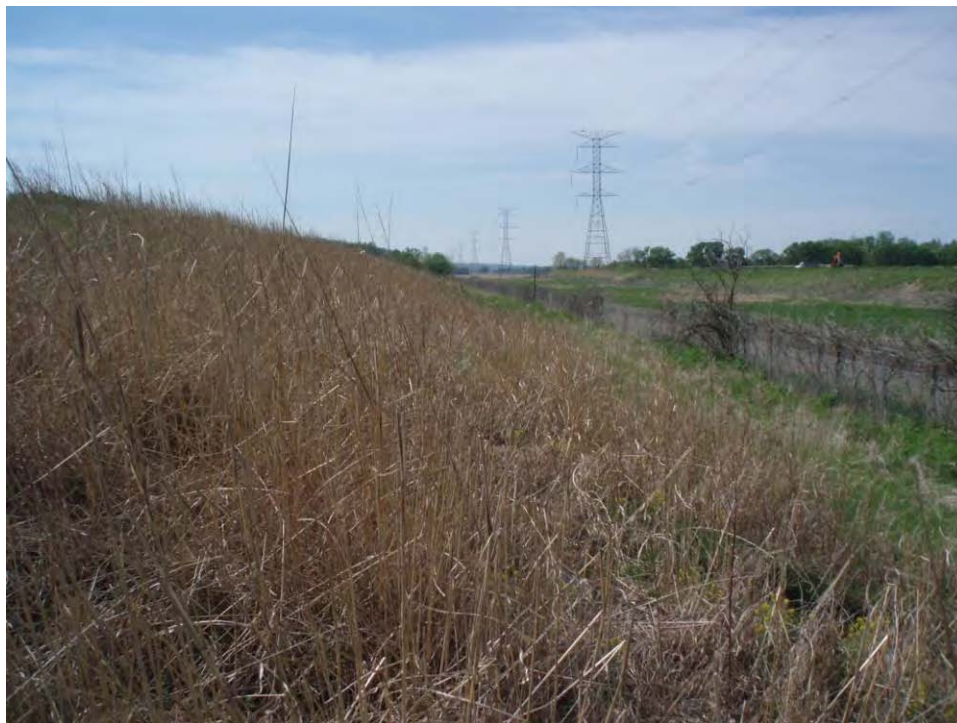
111. Pond E - West embankment exterior slope, looking south.
