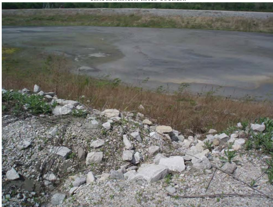
126. Pond D - Erosion rill on west slope of divider embankment, looking southwest.
