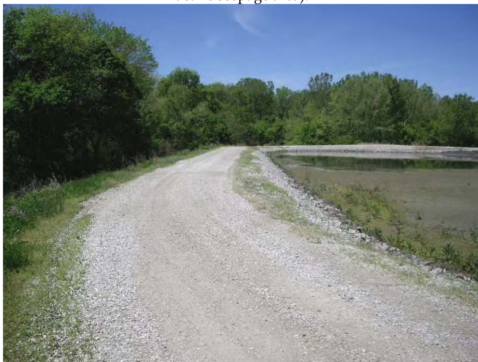
22. Pond A - South embankment crest, looking west.
