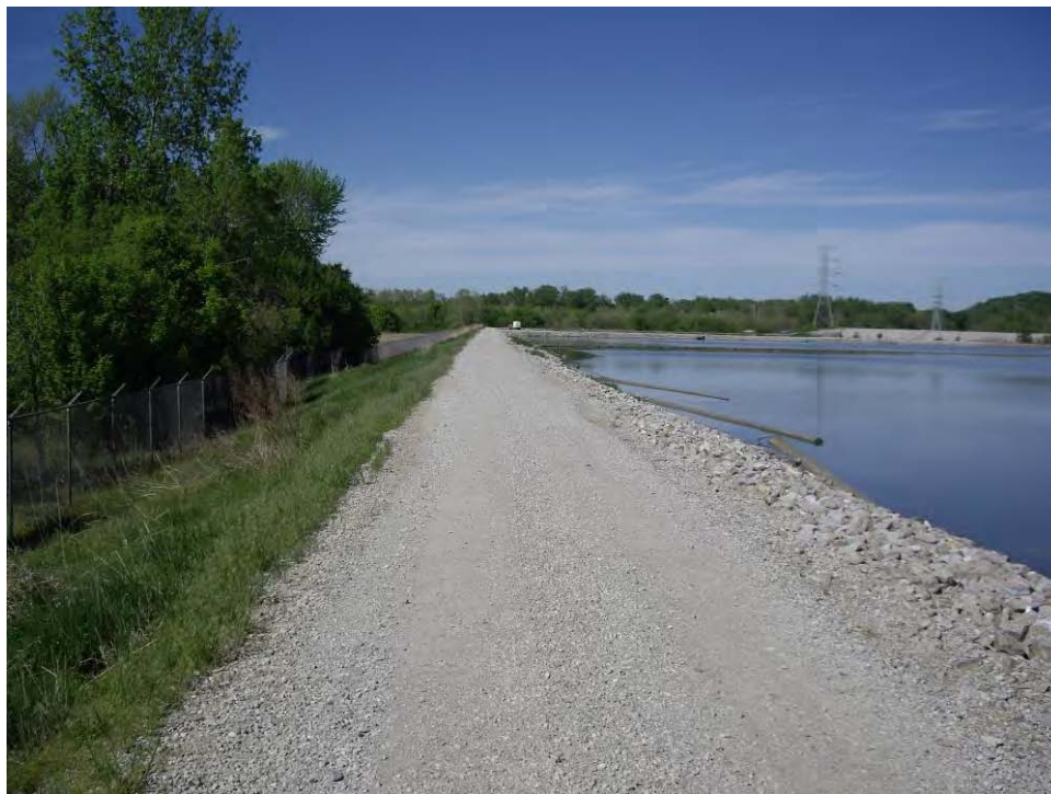
63. Pond B – west embankment crest, looking north
