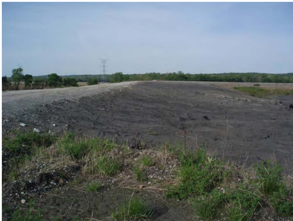
79. Pond D - Southeast embankment interior area, looking southwest
