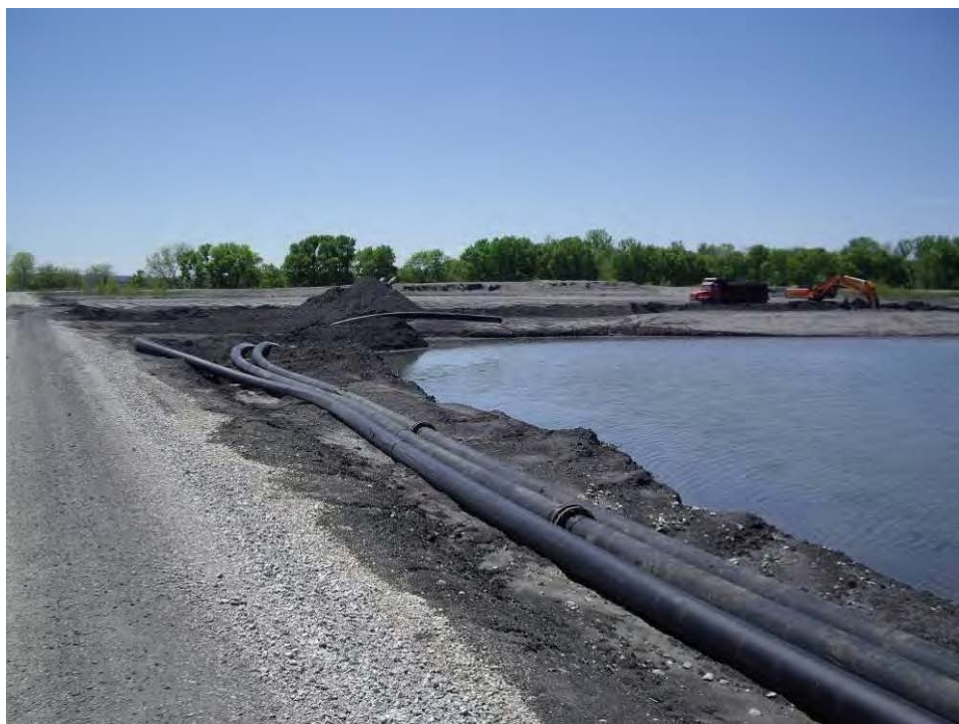
8. Overview of three 10-inch-diameter HDPE discharge pipes into Pond A, looking southwest. Note two right-most pipes are disconnected.
