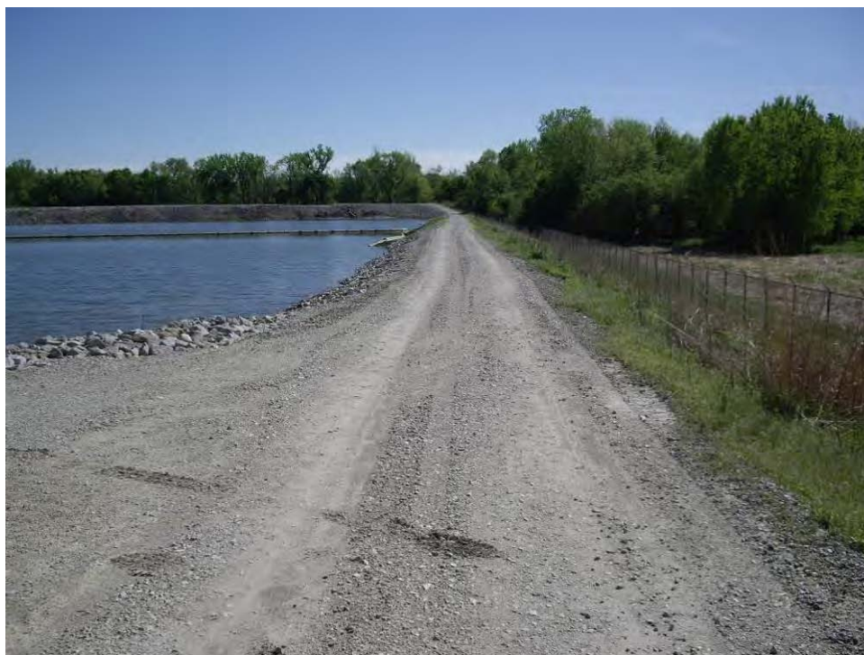
60. Pond B - west embankment crest, looking south.
