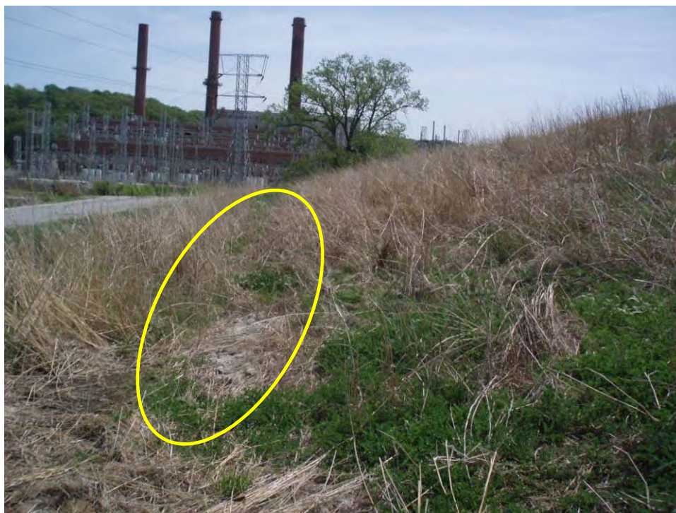
134. Pond D - Toe of north embankment, looking east. Note drainage ditch with seepage collector pipe.
