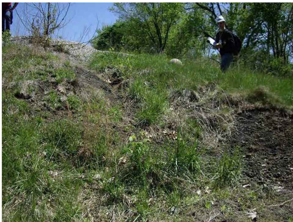
26. Pond A – Erosion rill on west embankment exterior slope, looking east.
