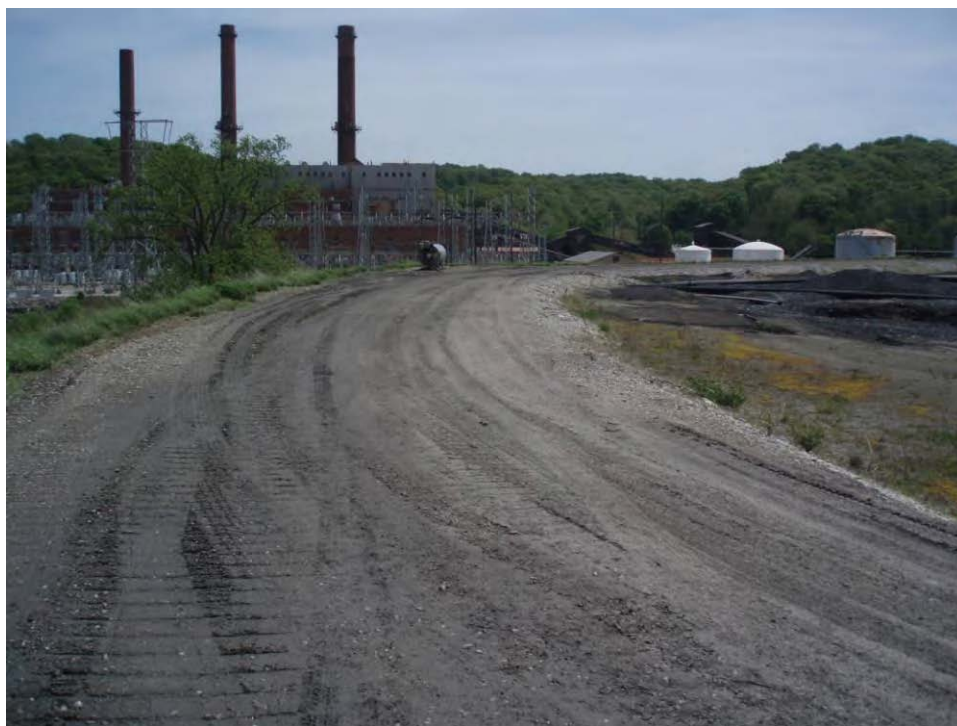
132. Pond D - North embankment crest, looking east.
