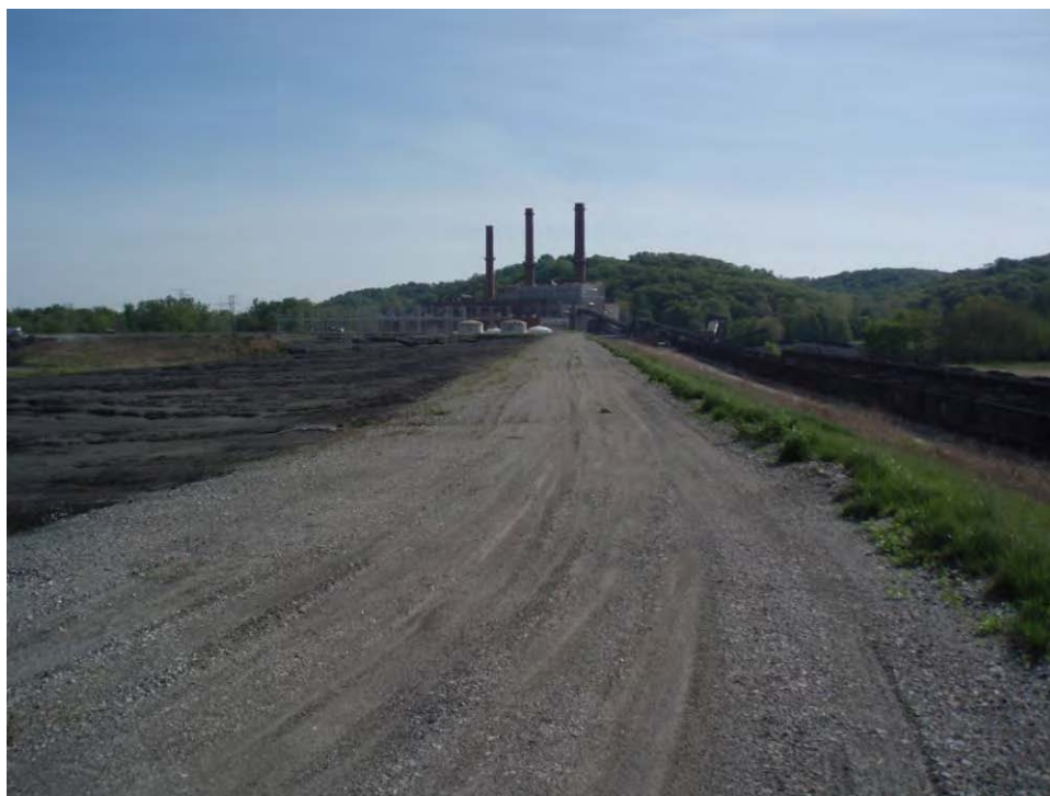
84. Pond D - Southeast embankment crest, looking northeast.
