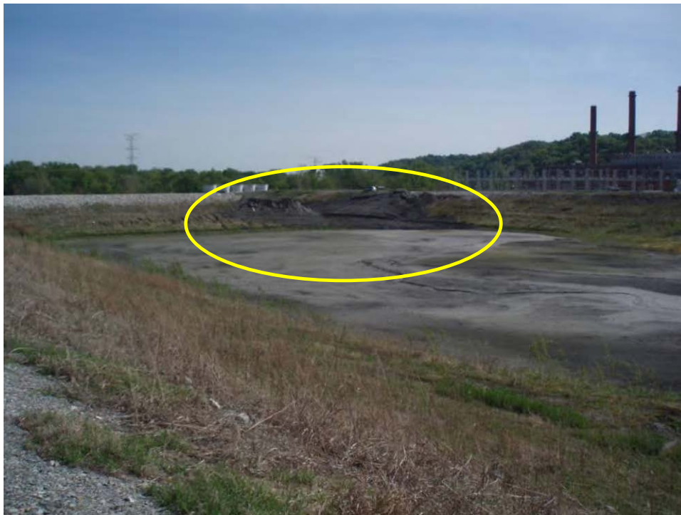
94. Overview of Pond D, south slope of divider embankment D/E, and west slope of Pond D divider embankment. Note breach (circled) in divider embankment D/E.
