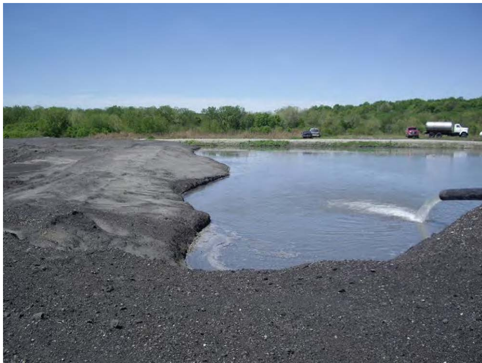
10. Overview of 10-inch-diameter HDPE discharge pipe into Pond A, looking west.
