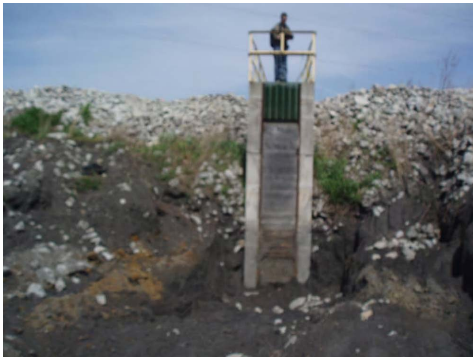
115. Pond E - Overview of outlet control structure with stoplogs and butterfly valve, looking northwest.
