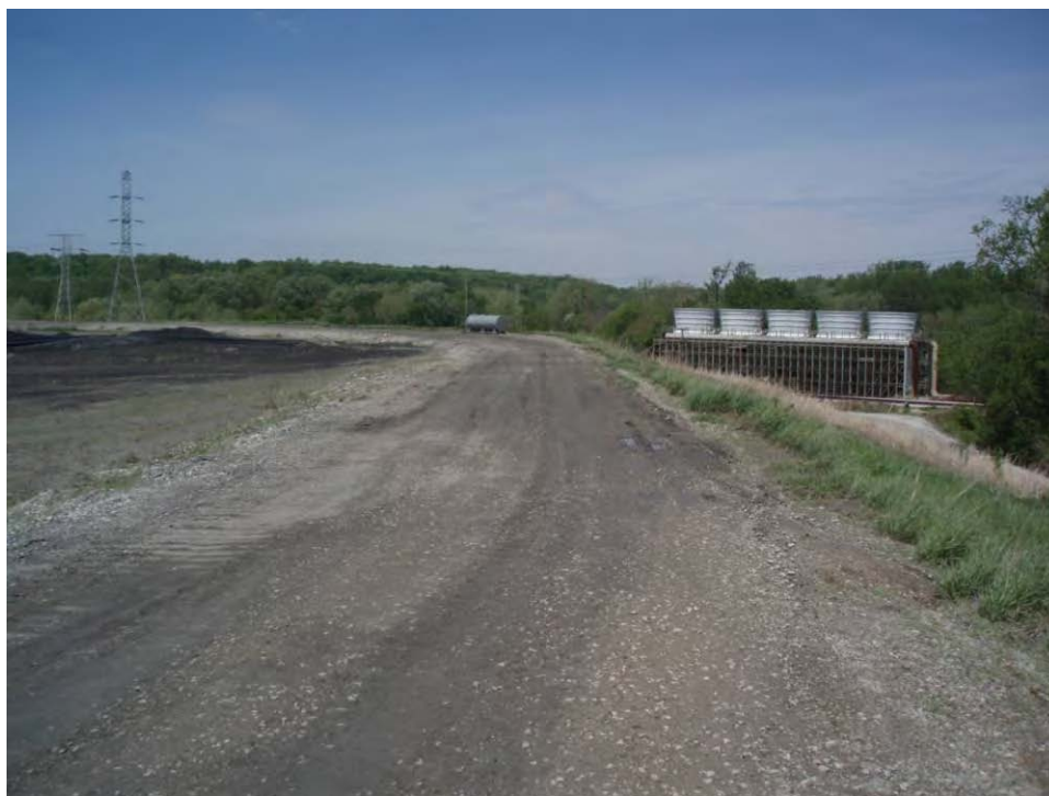
142. Pond D - Northeast embankment crest, looking northwest.
