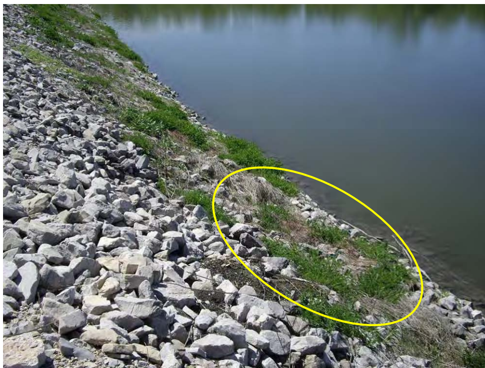
32. Depression in north slope of Pond A/B divider embankment.
