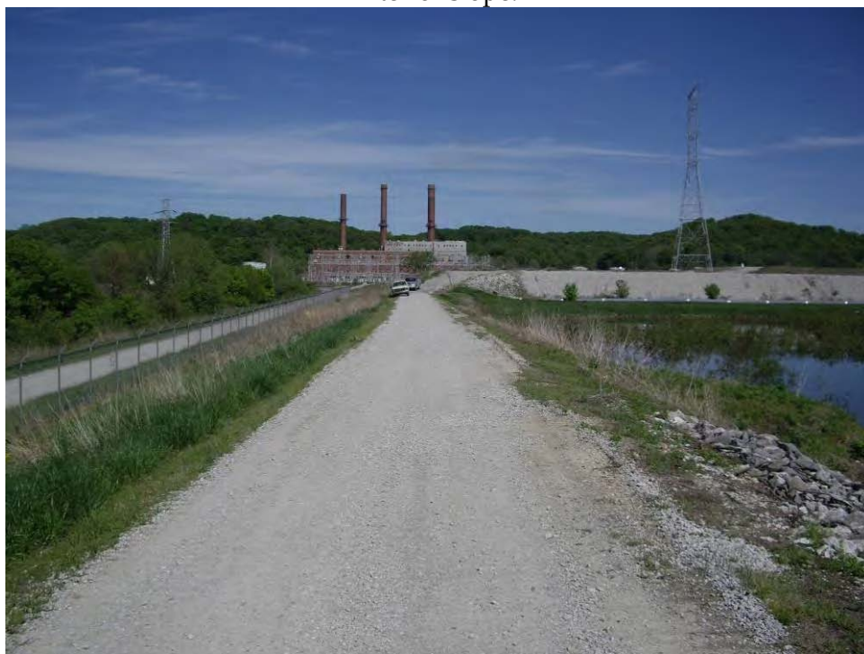
48. Pond C – North embankment crest, looking east.
