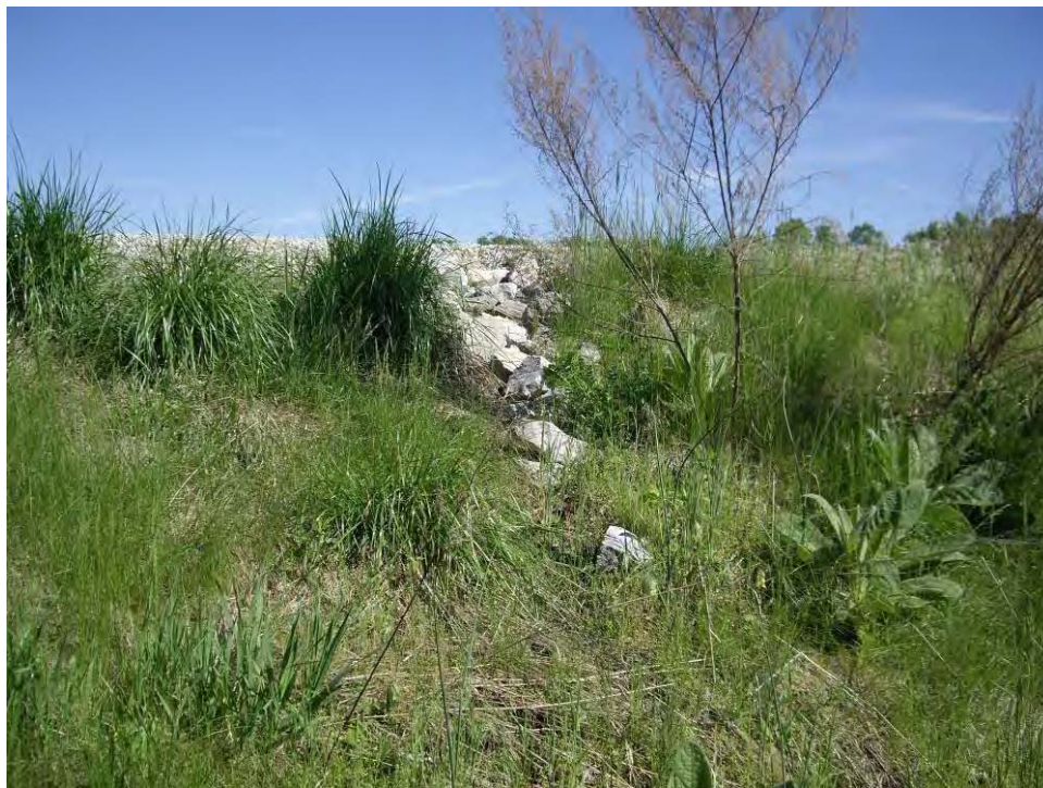
65. Pond B - erosion rill on exterior slope recently filled in with riprap, looking east.
