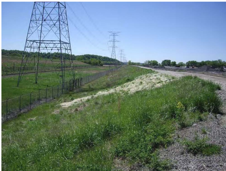
1. Pond A - East embankment exterior slope looking south.
