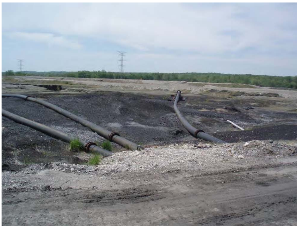
140. Overview of three 10-inch-diameter HDPE discharge pipes into Pond D, looking southwest.
