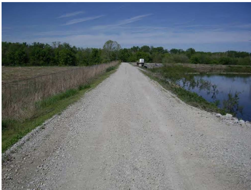
56. Pond C - West embankment crest, looking north
