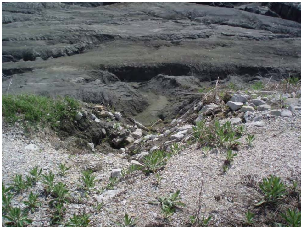
127. Pond D - Erosion feature on east slope of divider embankment, looking east.
