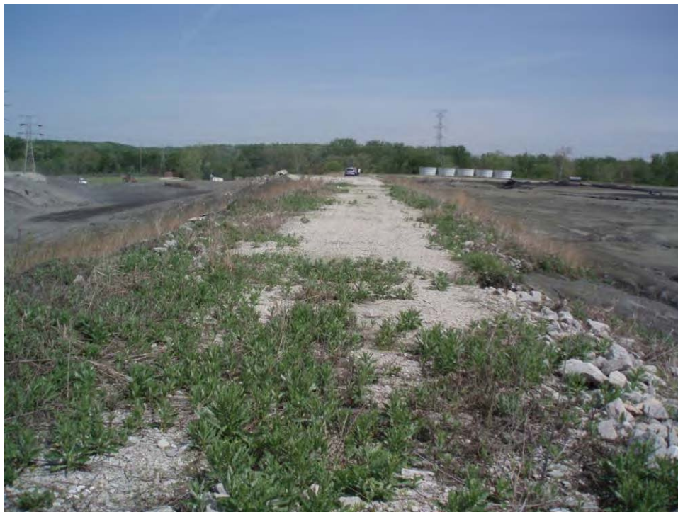
129. Pond D - Crest of divider embankment, looking north.
