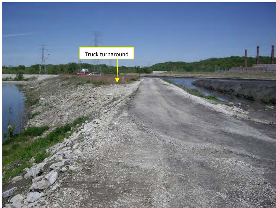
34. Crest of divider embankment A/B, looking northeast.
