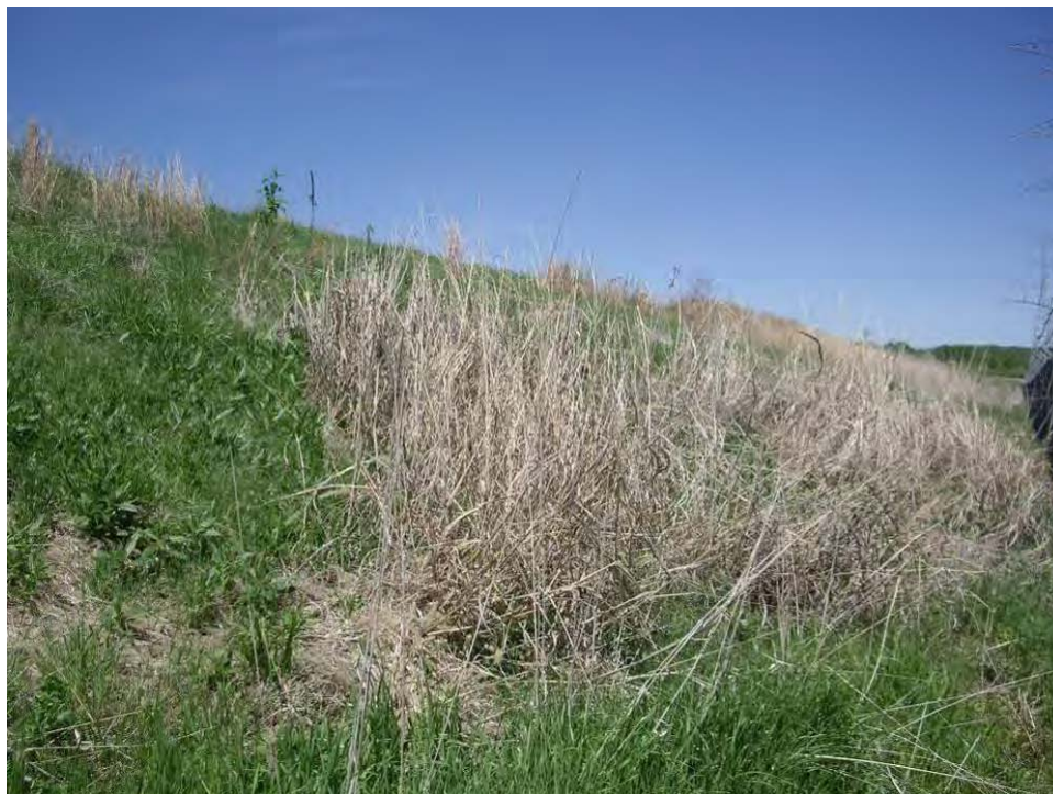
12. Pond A looking north - Possible former seep location at toe of east embankment.,.
