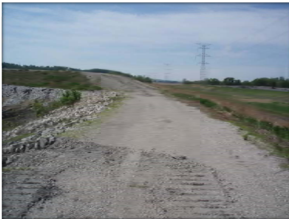
110. Pond E - West embankment crest, looking south.
