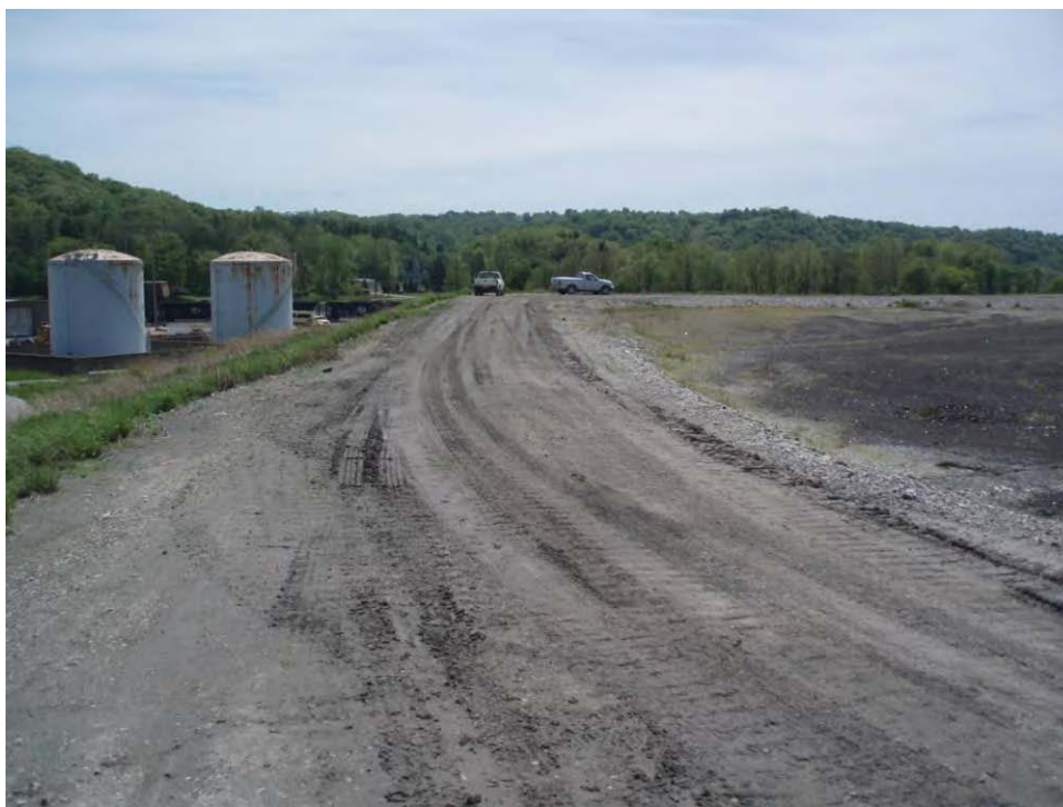
138. Pond D - Northeast embankment crest, looking southeast.
