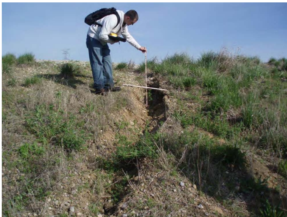
82. Pond D - Erosion rill on southeast embankment exterior slope, looking northwest.
