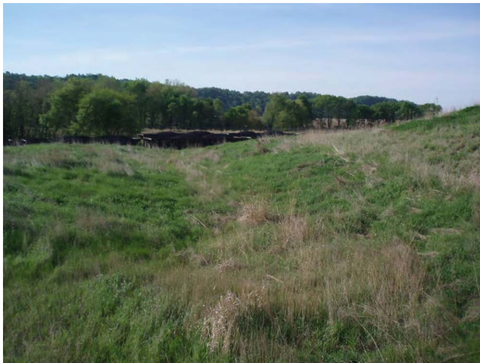
75. Pond D - Crest of east embankment buttress berm, looking south
