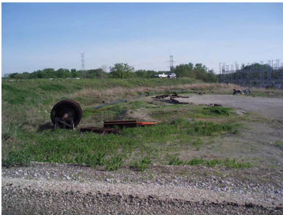
74. Pond D - Crest of east embankment buttress berm, looking north
