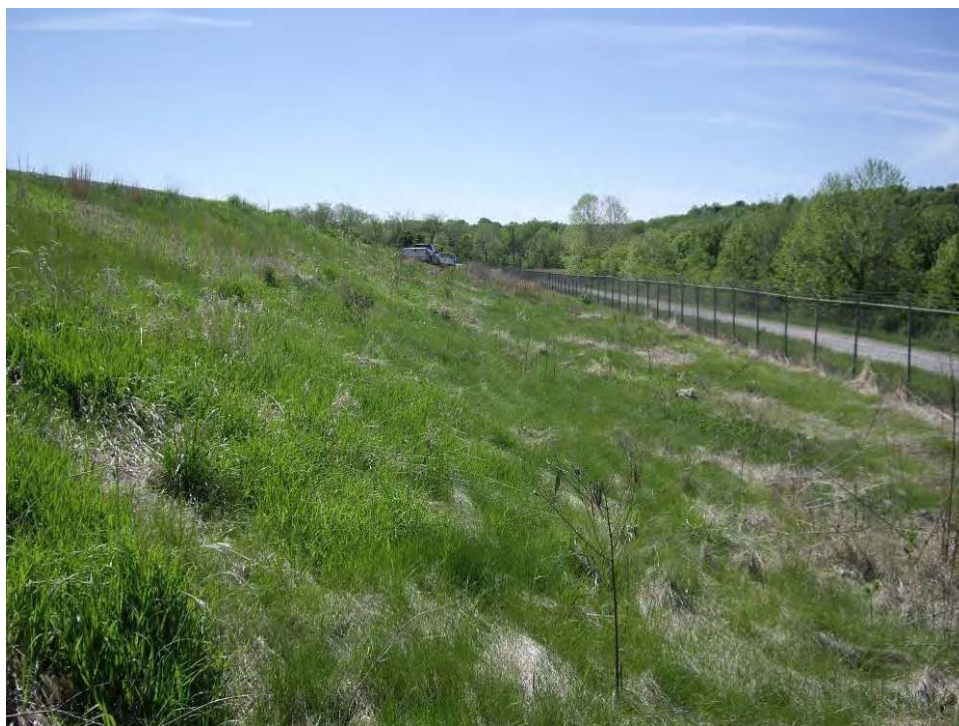
46. Pond C - North embankment exterior slope, looking west.
