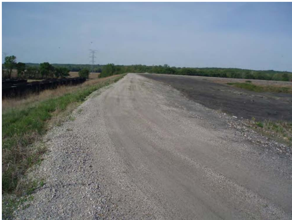
77. Pond D - Southeast embankment crest, looking southwest.
