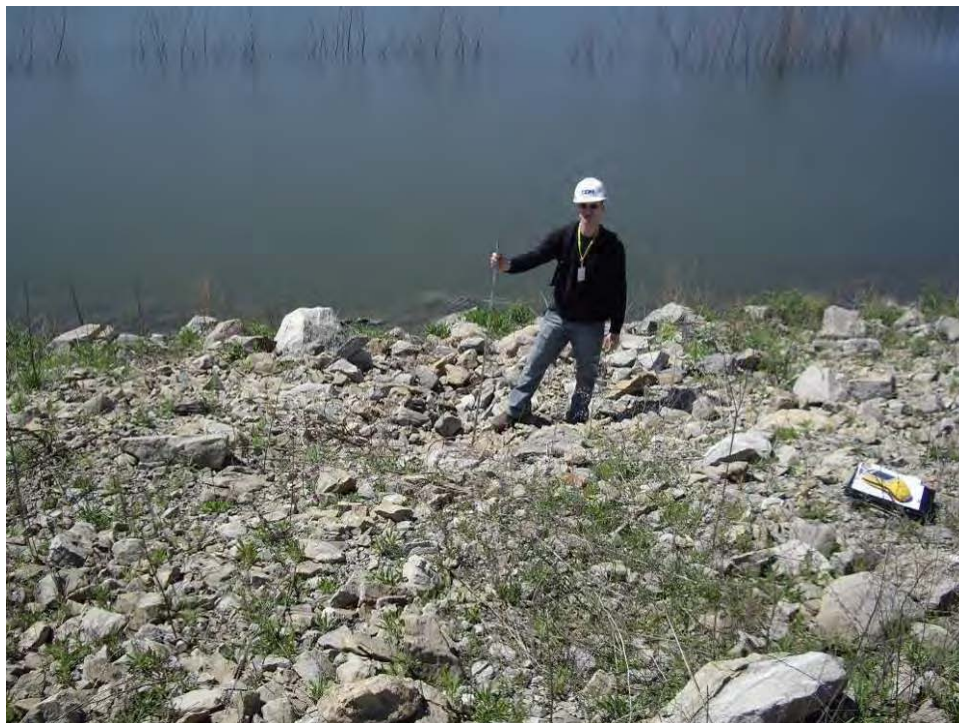
36. Depression in north slope of divider embankment A/B.
