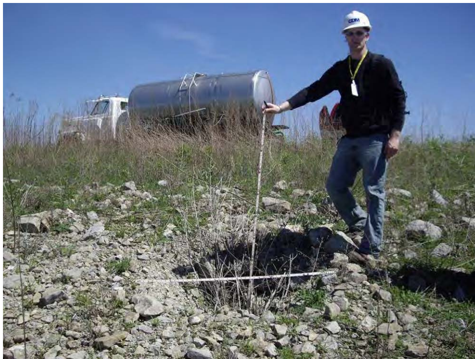
37. Depression in northwest slope of divider embankment A/B.
