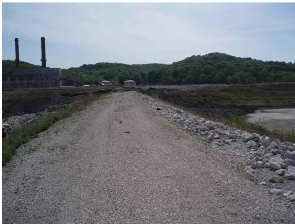
100. Crest of divider embankment D/E, looking east.
