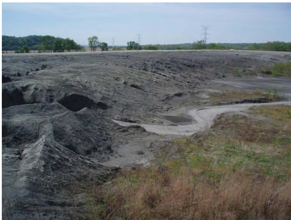
128. Pond D - Limit of ash at end of divider embankment prior to failure, looking southwest.
