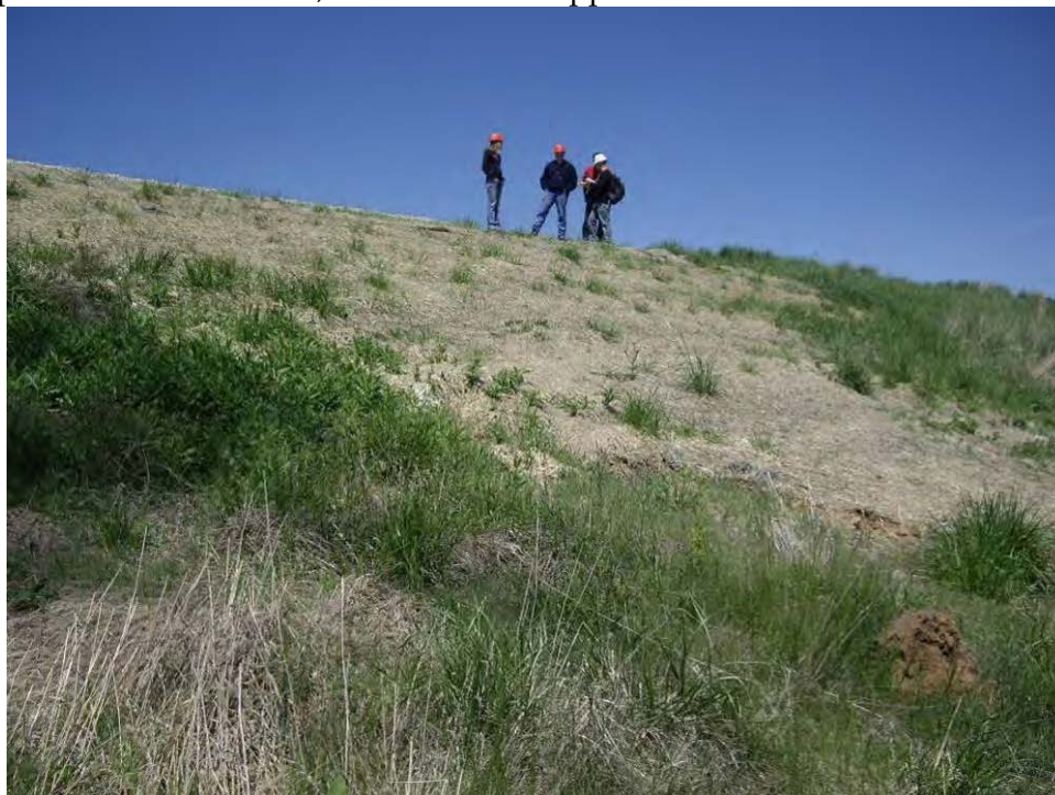
4. Pond A - East embankment exterior slope. Erosion control blanket installed near northeast corner looking northwest.
