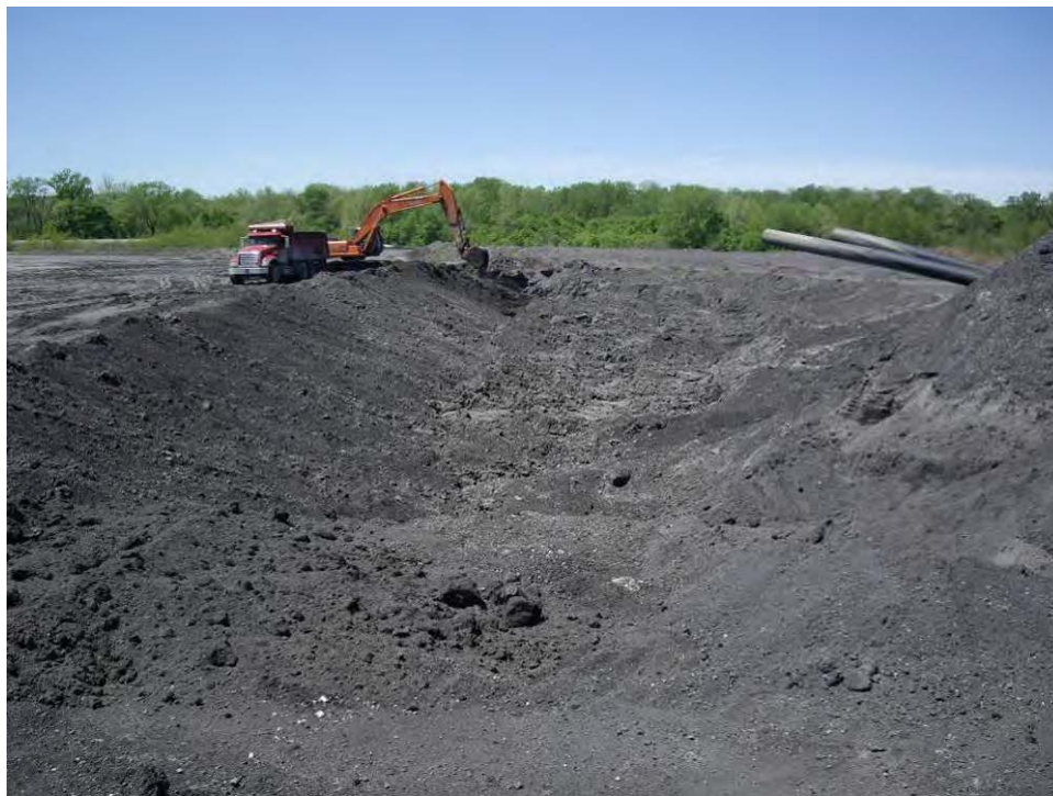
11. Overview of ash excavation in Pond A looking west. Ash being used as fill to repair Ponds D and E..
