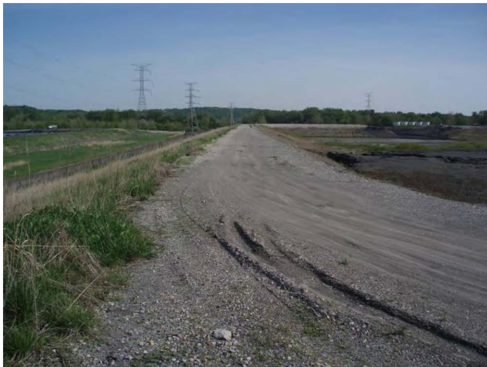
87. Pond D - West embankment crest, looking north
