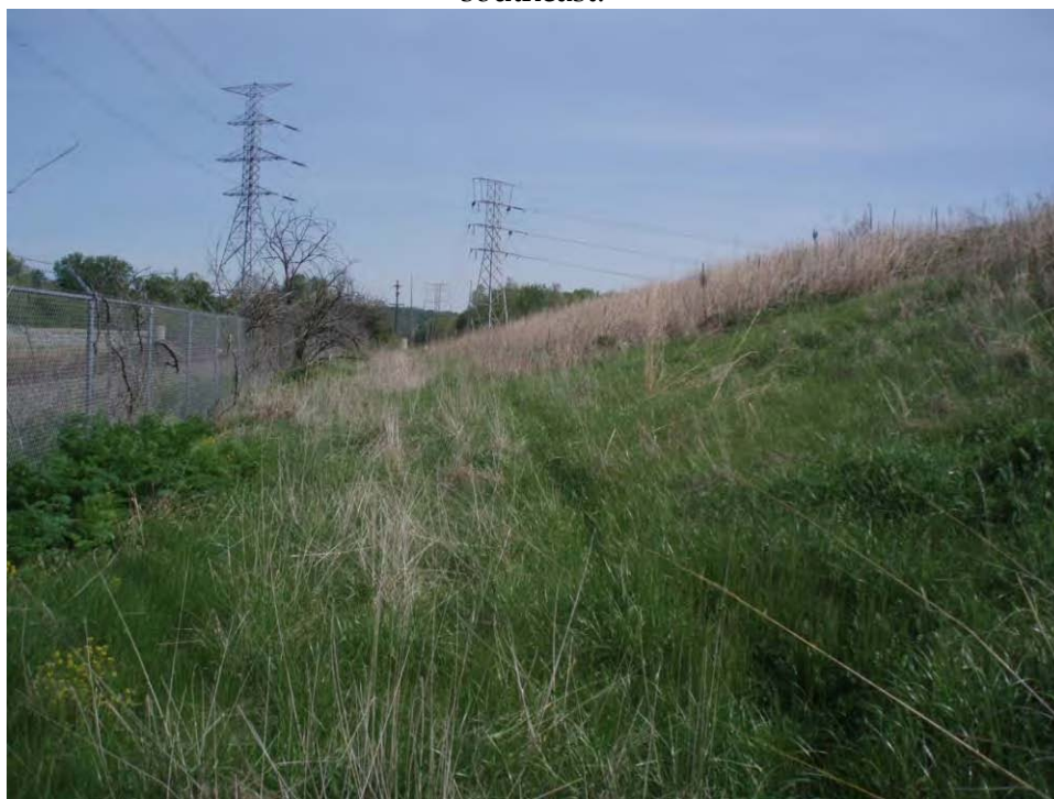
98. Pond D - West embankment exterior slope at toe, looking north.
