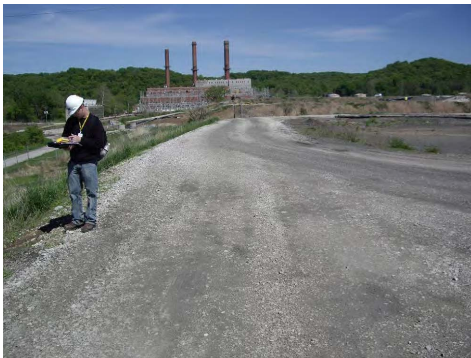
44. Pond A - North embankment crest, looking east.
