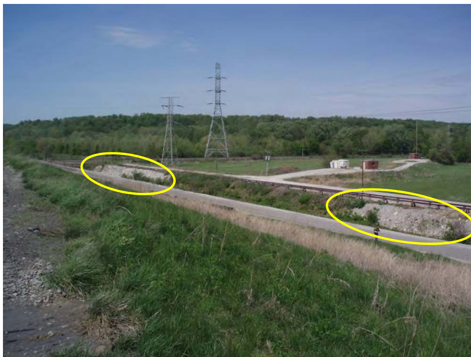
136. Overview of downstream area north of Pond D and Pond E. Note repair of erosion areas which resulted from breach.
