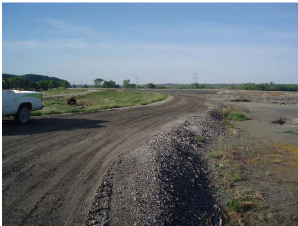
68. Pond D - east embankment crest, looking southwest.
