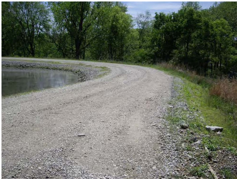
27. Pond A – West embankment crest, looking south.
