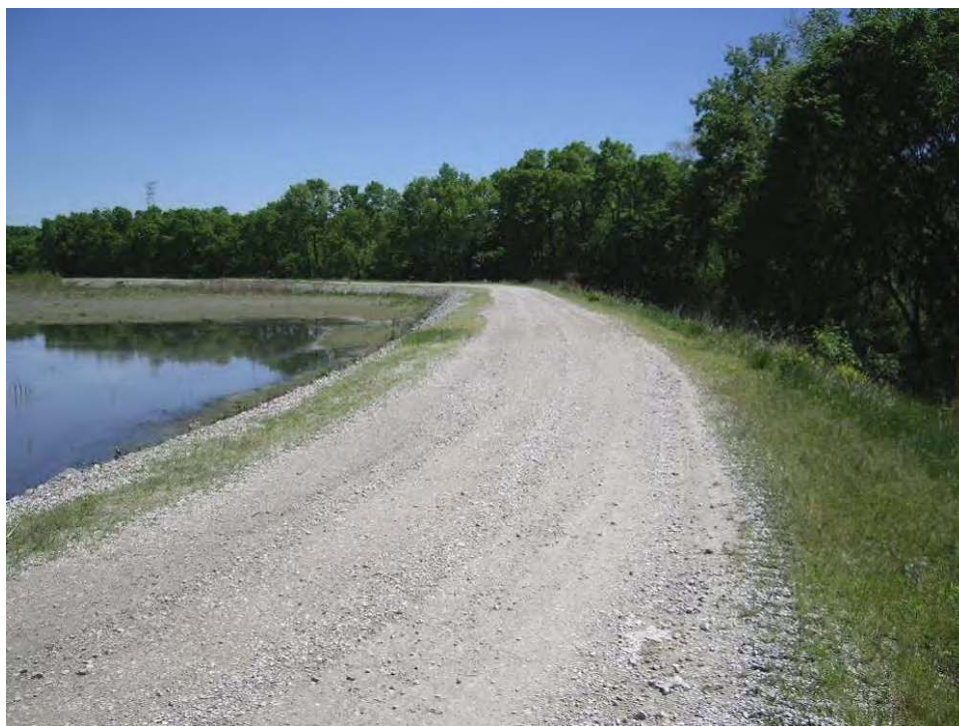
24. Pond A – South embankment crest, looking southeast.
