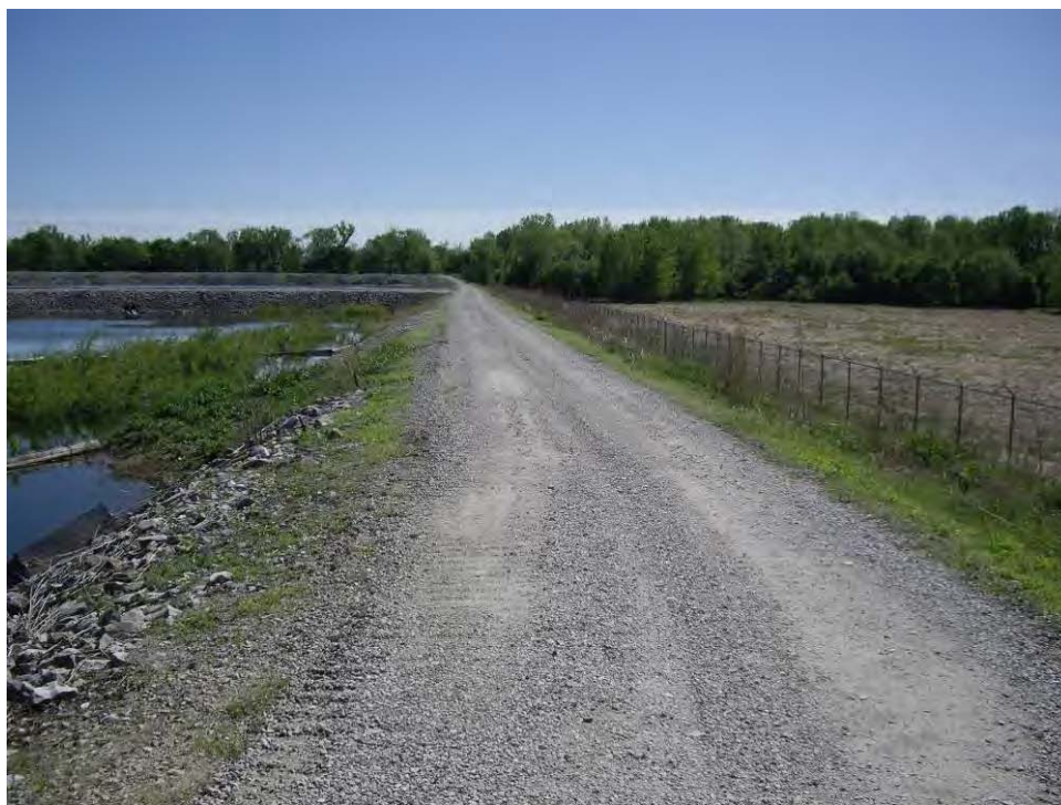
52. Pond C - West embankment crest, looking south.
