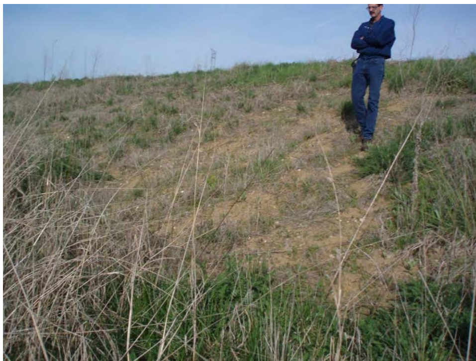
80. Pond D - Large bare spot on upper third of southeast embankment exterior slope, looking northwest.
