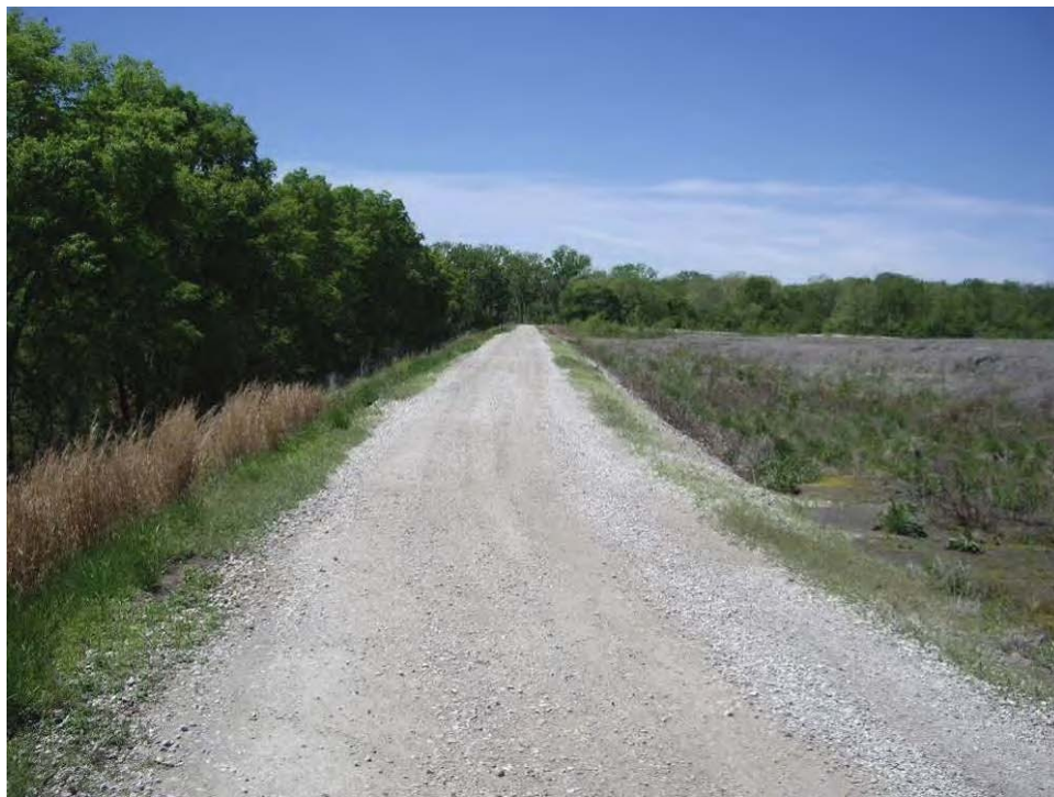
19. Pond A – South embankment crest looking west.
