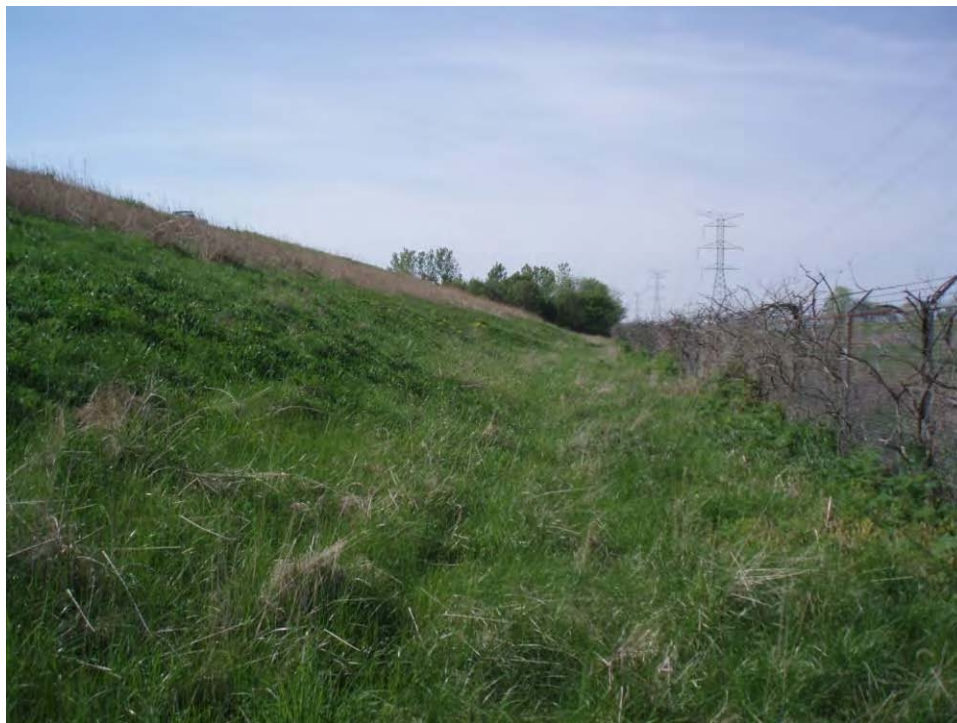
91. Pond D - West embankment exterior slope, looking south.
