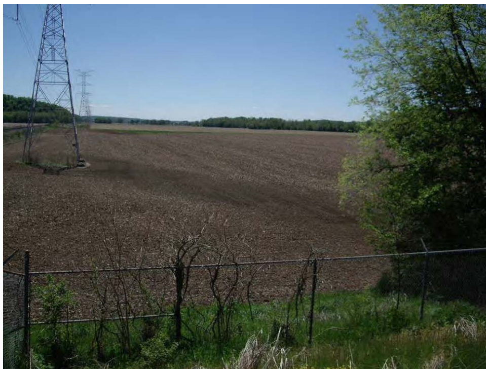
18. Pond A - Downstream area of east embankment at southeast corner of embankment looking south.
