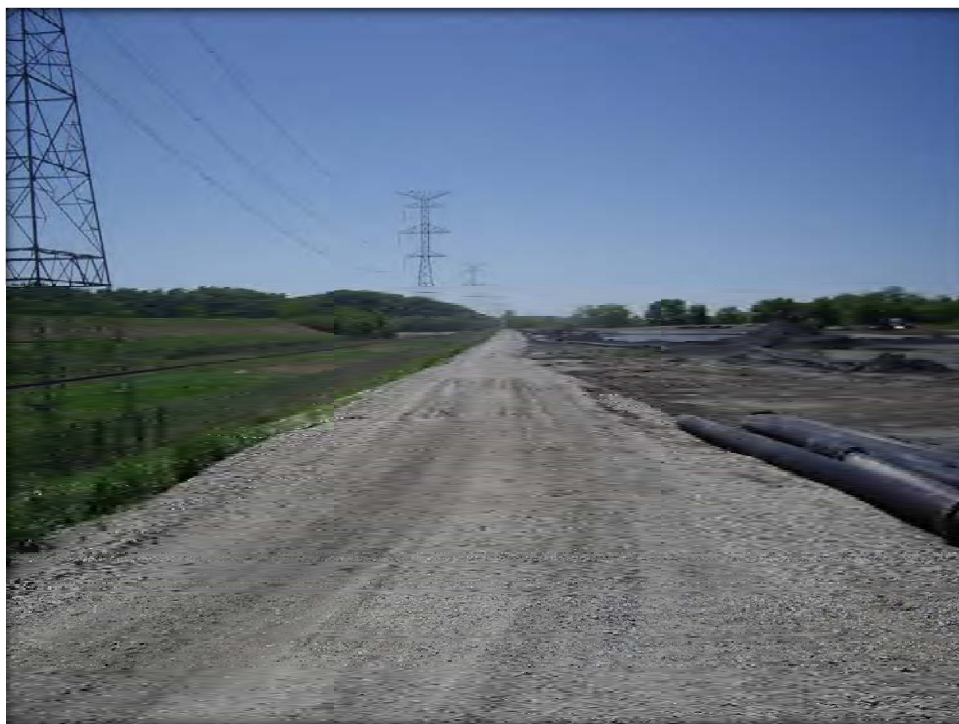
2. Pond A - East embankment crest looking south.
