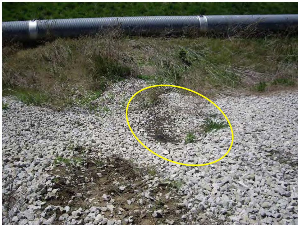
41. Minor sloughing and erosion feature on west slope of divider embankment A/C.
