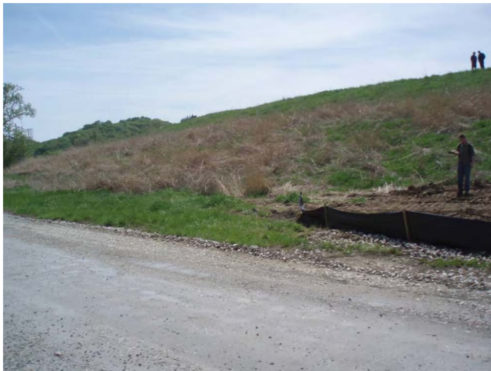
135. Pond D - North embankment exterior slope, looking southeast.
