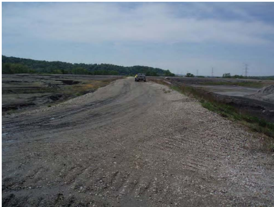
121. Crest of divider embankment D/E, looking south.
