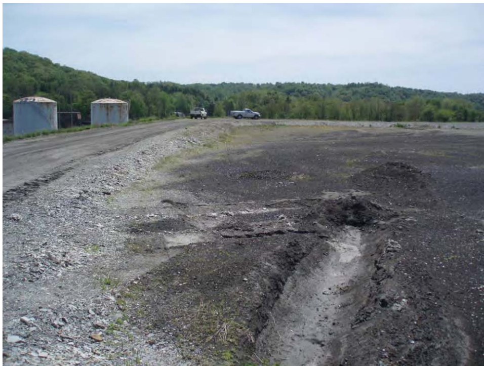
139. Pond D - Northeast embankment interior slope, looking southeast.
