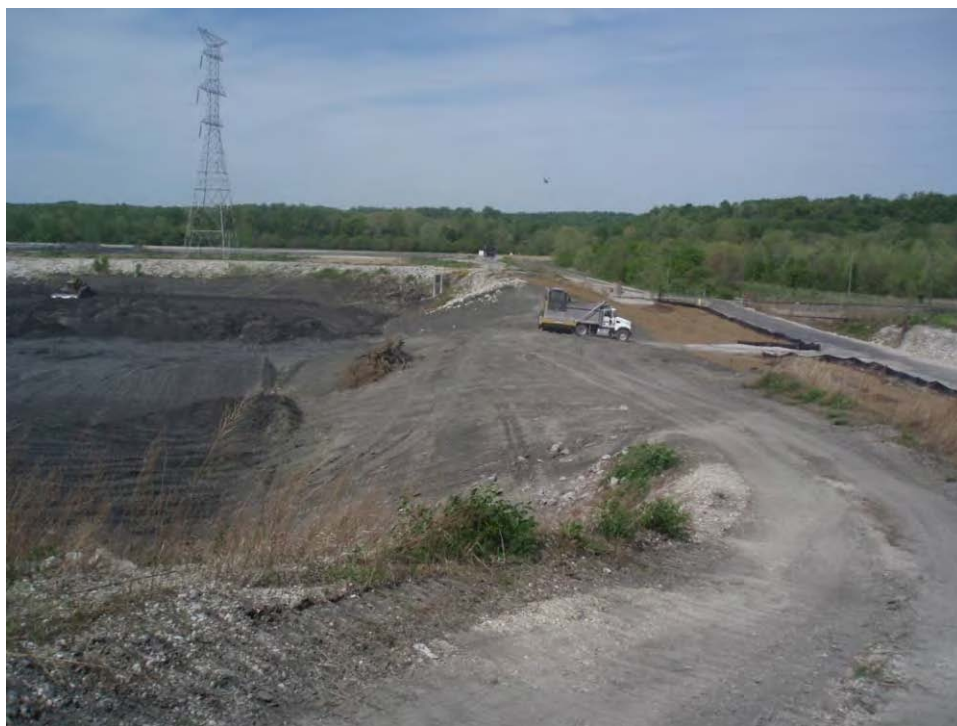
120. Pond E - Overview of north embankment reconstruction, looking west.
