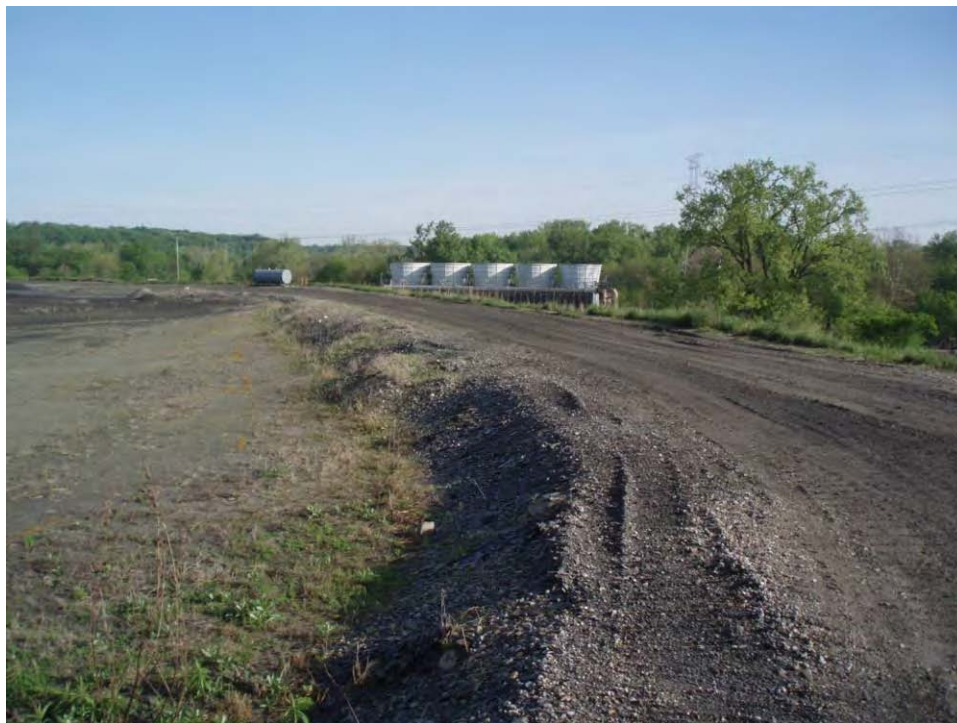
69. Pond D - north embankment crest, looking northwest.
