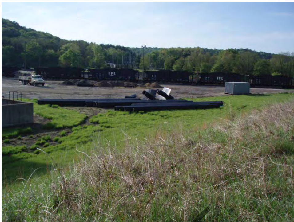
71. Pond D - East embankment downstream area looking southeast. Note new piping for Ponds D & E.
