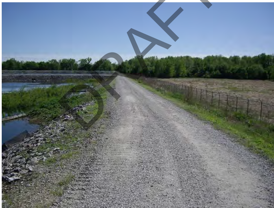
52. Pond C - West embankment crest, looking south.
