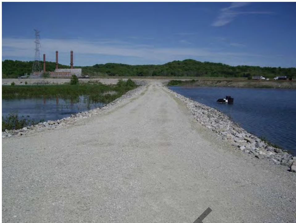
57. Crest of divider embankment B/C, looking east.
