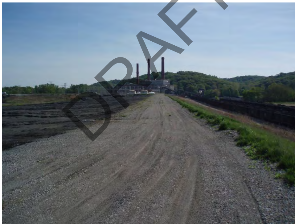
84. Pond D - Southeast embankment crest, looking northeast.
