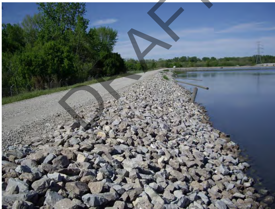
62. Pond B - west embankment interior slope, looking north
