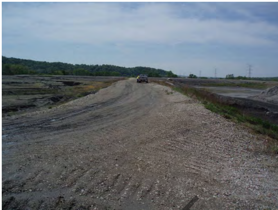
121. Crest of divider embankment D/E, looking south.
