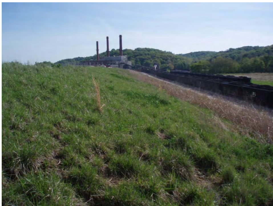
83. Pond D - Southeast embankment exterior slope, looking northeast.
