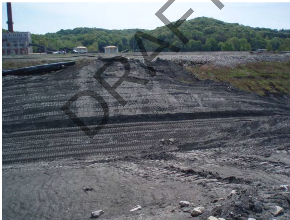
102. Overview of cut in divider embankment D/E for repair work.
