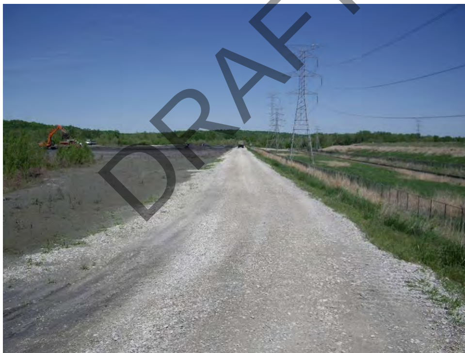
16. Pond A - East crest looking north.
