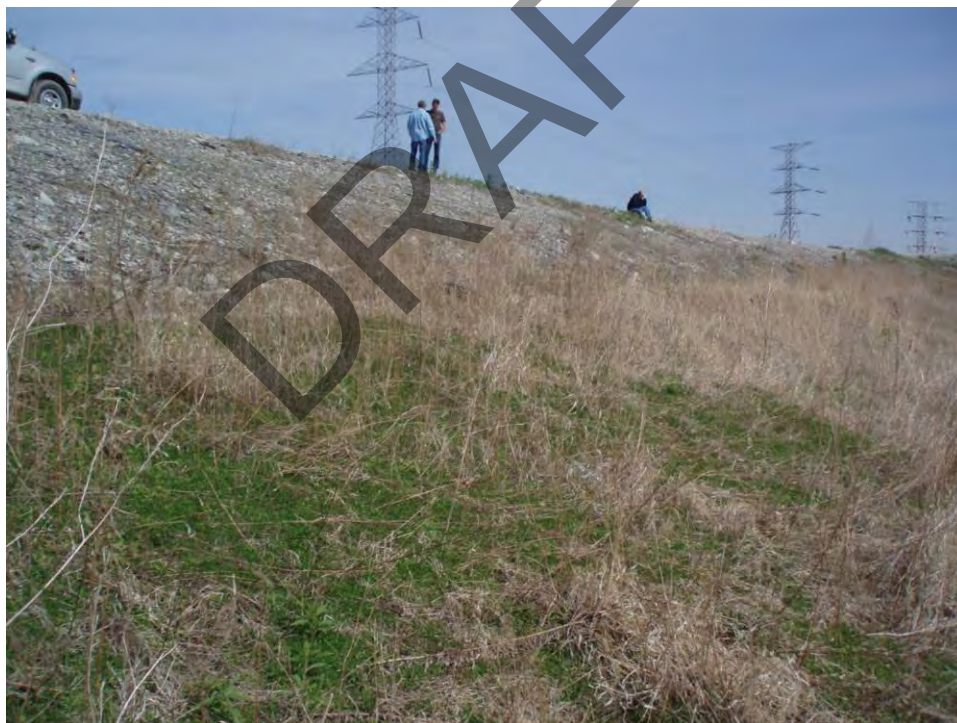
96. Pond D - West embankment typical interior slope with shale armor near crest.
