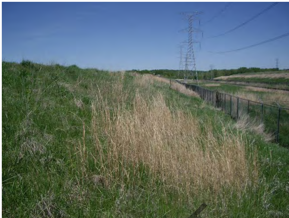
15. Pond A - East embankment exterior slope looking north.
