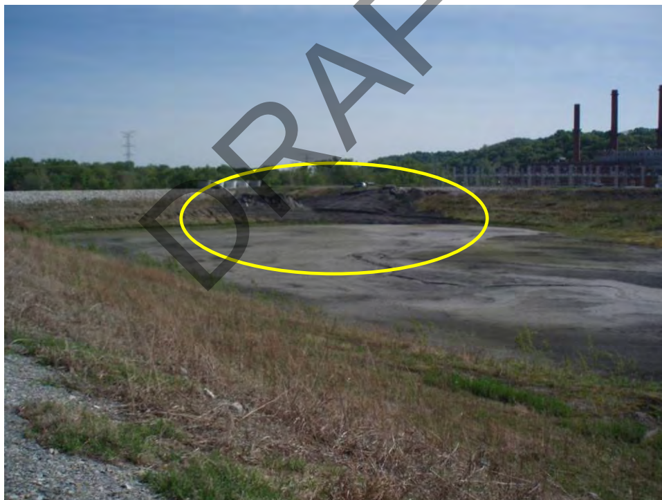
94. Overview of Pond D, south slope of divider embankment D/E, and west slope of Pond D diversion embankment. Note breach (circled) in divider embankment D/E.
