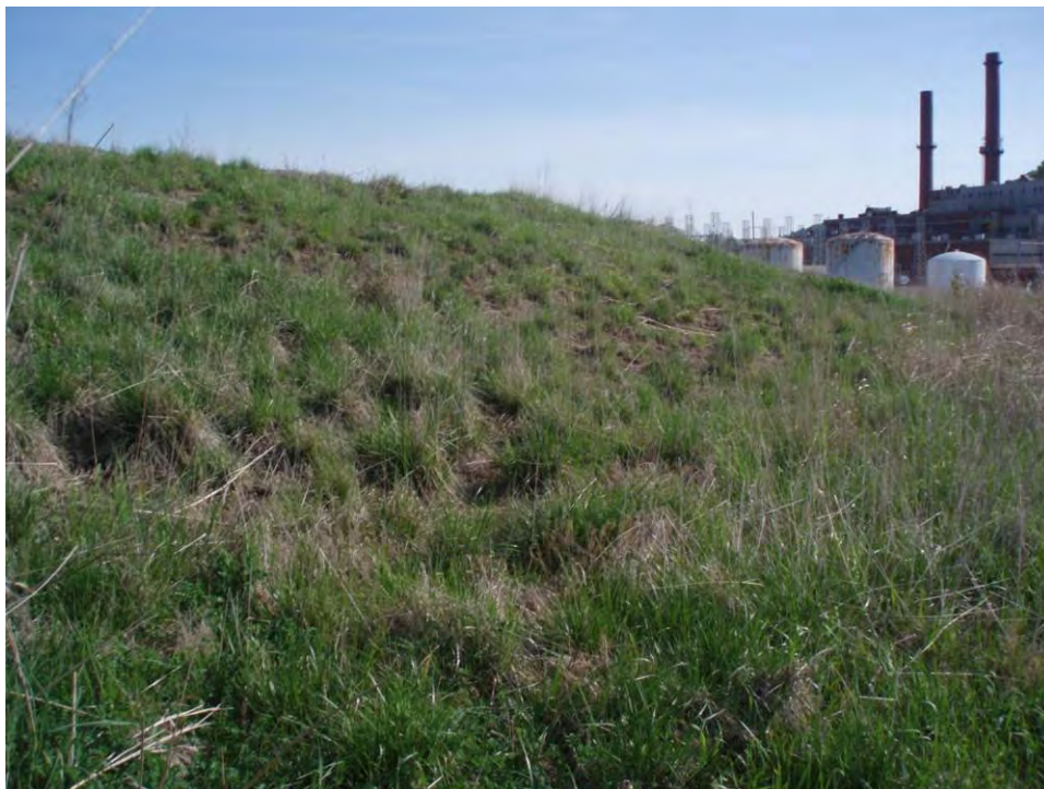
81. Typical bare spots on upper third of Pond D exterior embankment (last expansion).
