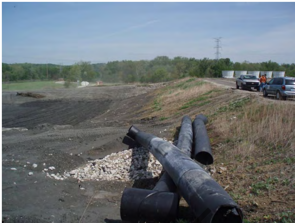
125. West slope of divider embankment D/E, looking north. Note pipes removed from embankment after breach.
