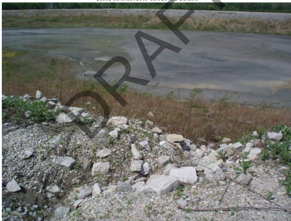
126. Pond D - Erosion rill on west slope of diversion embankment, looking southwest.
