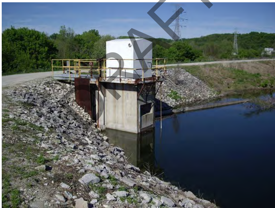
54. Pond C – Outlet structure gatehouse. Note stoplogs and butterfly valve in catwalk.
