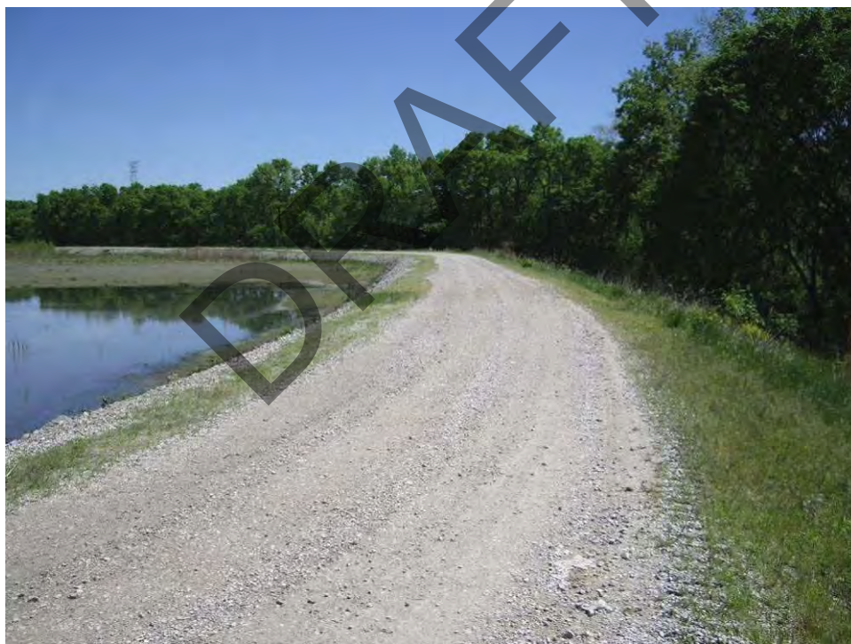
24. Pond A – South embankment crest, looking southeast.
