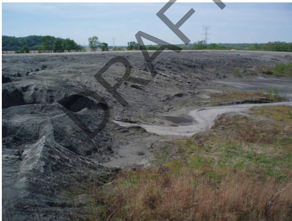
128. Pond D - Limit of ash at end of diversion embankment prior to failure, looking southwest.
