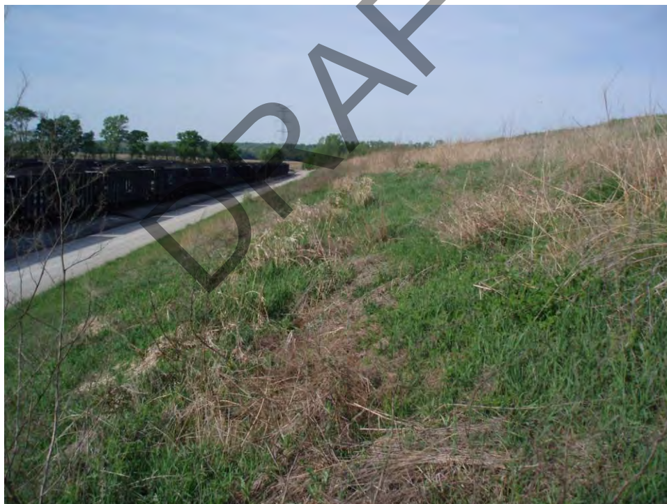
76. Pond D - Southeast embankment exterior slope, looking southwest.
