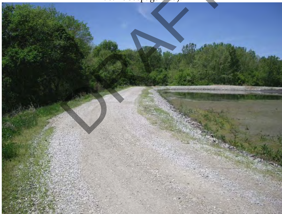
22. Pond A - South embankment crest, looking west.
