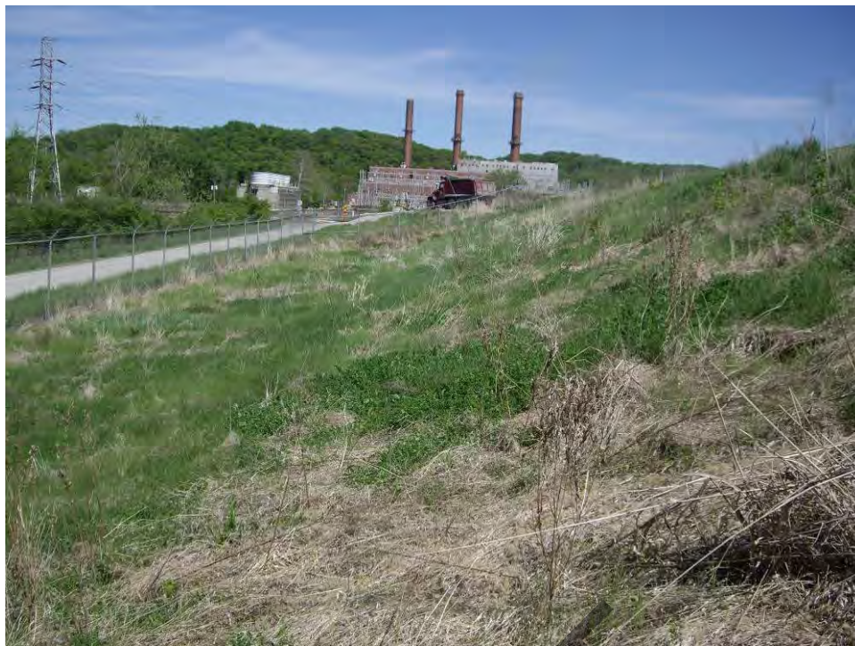
45. Pond A - North embankment exterior slope, looking east.
