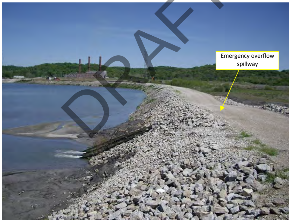
28. Pond A/B - north slope of divider embankment, looking east.
