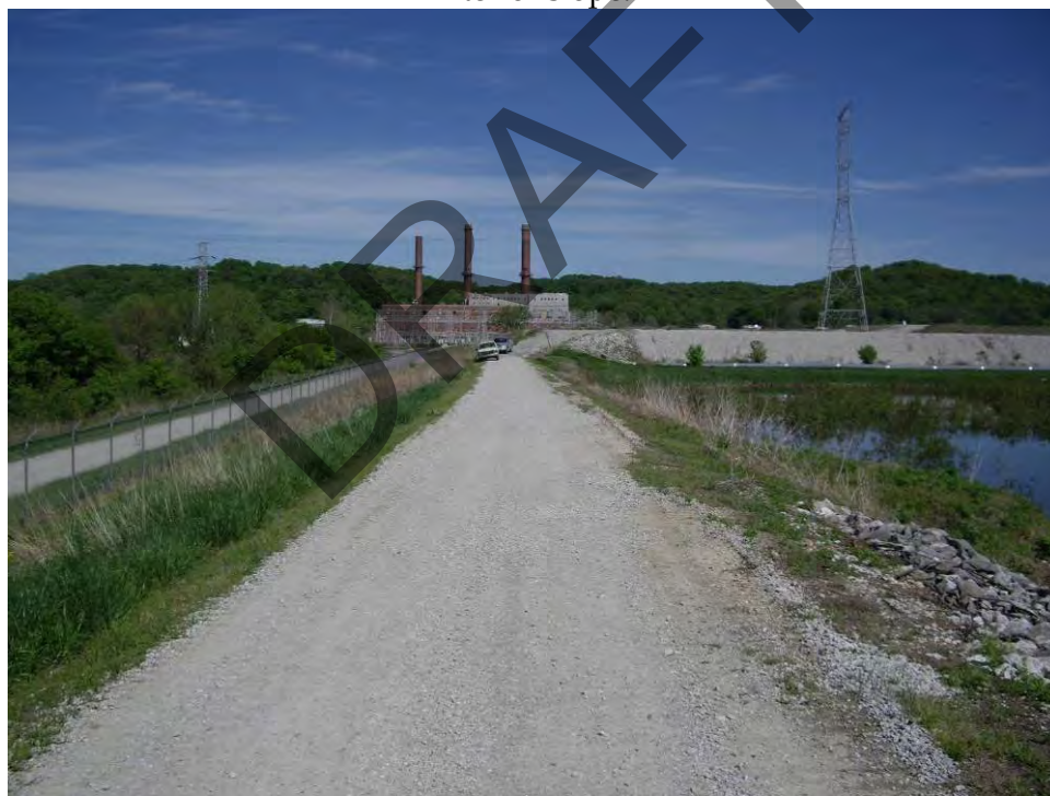
48. Pond C – North embankment crest, looking east.
