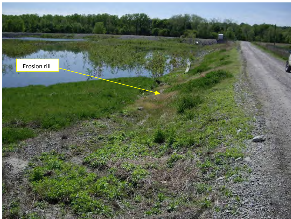
47. Pond C – North embankment interior slope and crest, looking west. Note erosion rill on interior slope.
