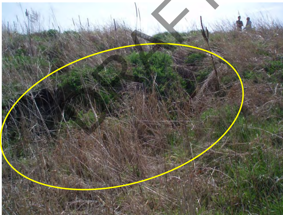
106. Pond E - 16'Wx4'Dx17'L erosion gulley at toe of west embankment exterior slope from previous failure event. Note erosion is scheduled to be repaired.
