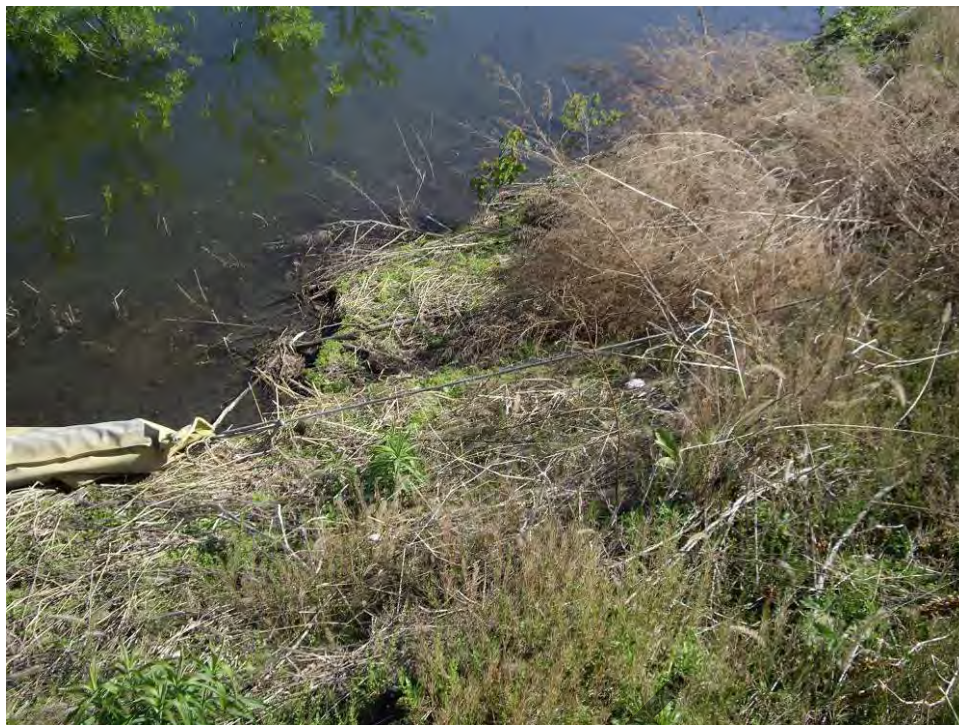
55. Pond C - Erosion feature from diversion boom tie line.
