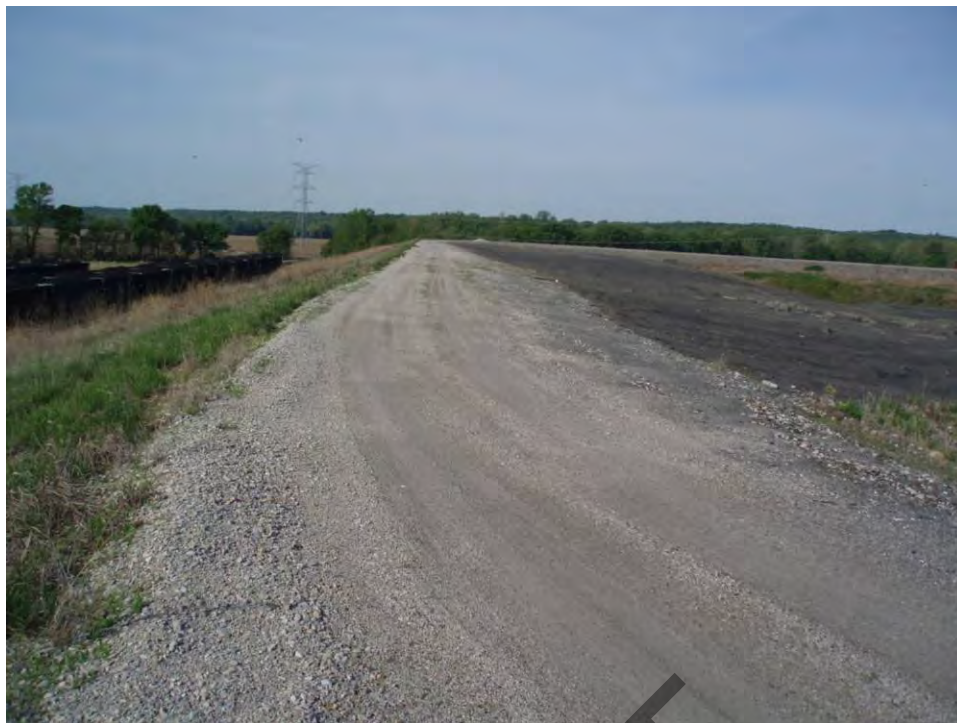
77. Pond D - Southeast embankment crest, looking southwest.
