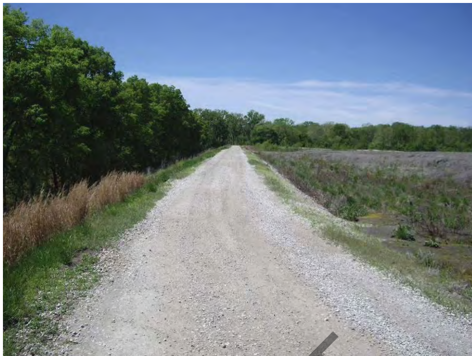
19. Pond A – South embankment crest looking west.
