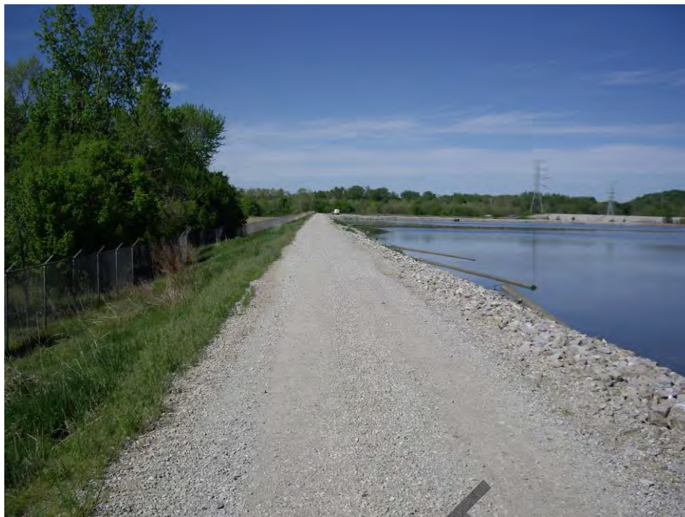
63. Pond B – west embankment crest, looking north
