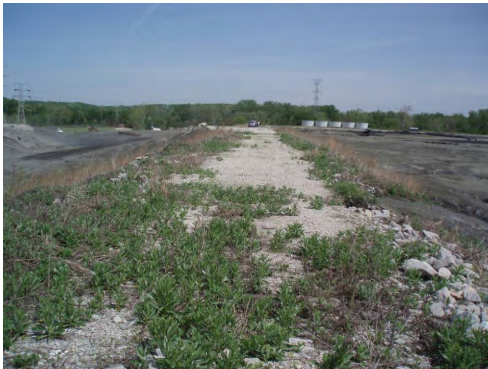
129. Pond D - Crest of diversion embankment, looking north.
