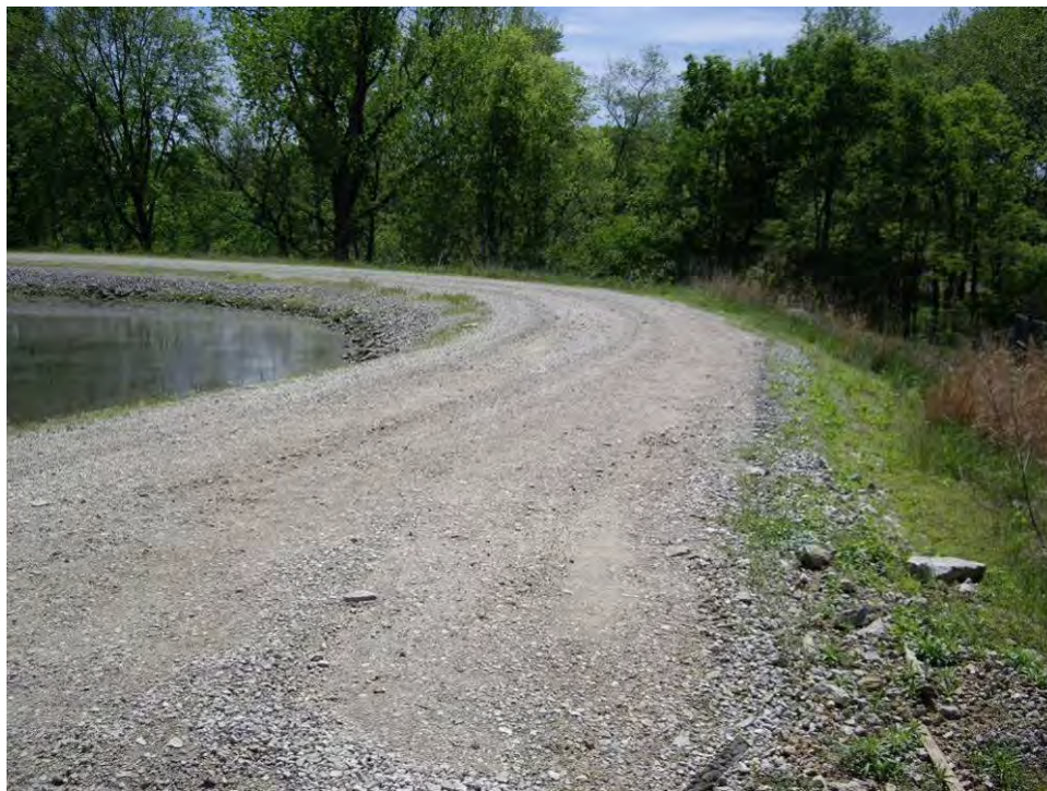
27. Pond A - West embankment crest, looking south.
