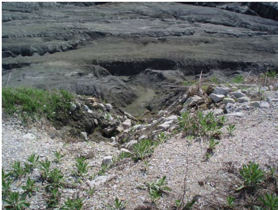
127. Pond D - Erosion feature on east slope of diversion embankment, looking east.
