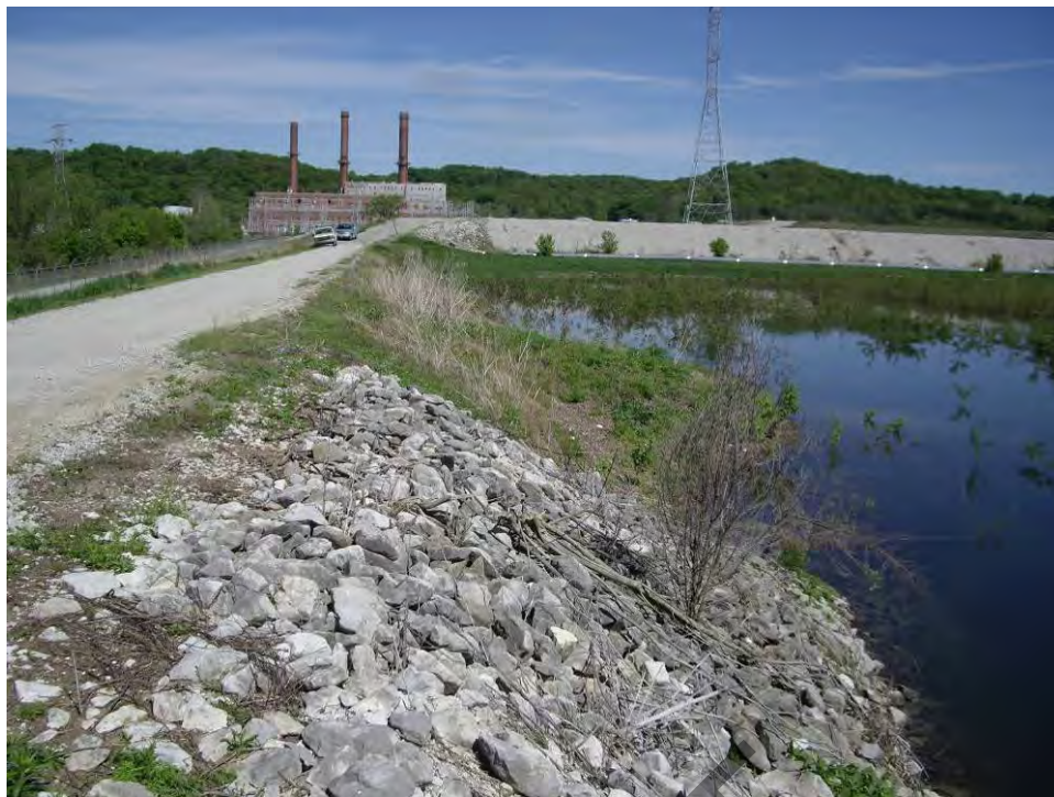
49. Pond C - North embankment interior slope, looking east. Note brush and limited riprap on slope.
