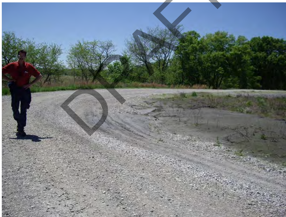
14. Pond A - Depression in crest from truck traffic, looking south.
