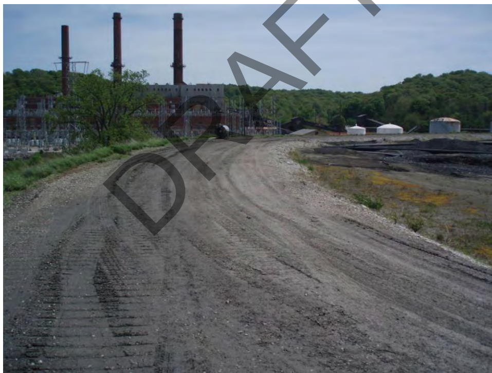
132. Pond D - North embankment crest, looking east.
