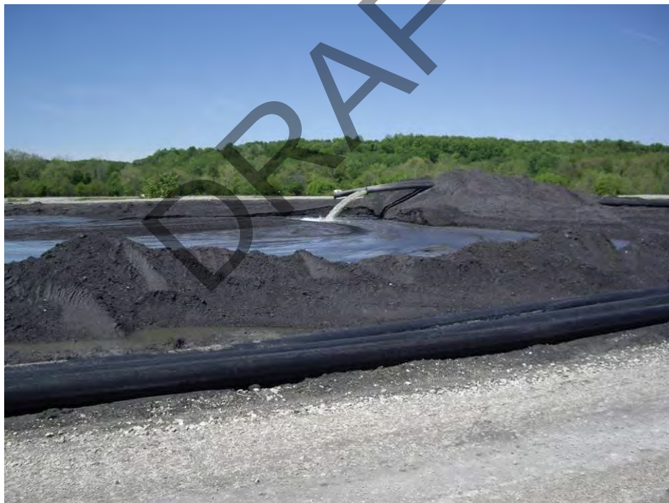
6. Overview of two 10-inch-diameter HDPE discharge pipes into Pond A, looking northwest.
