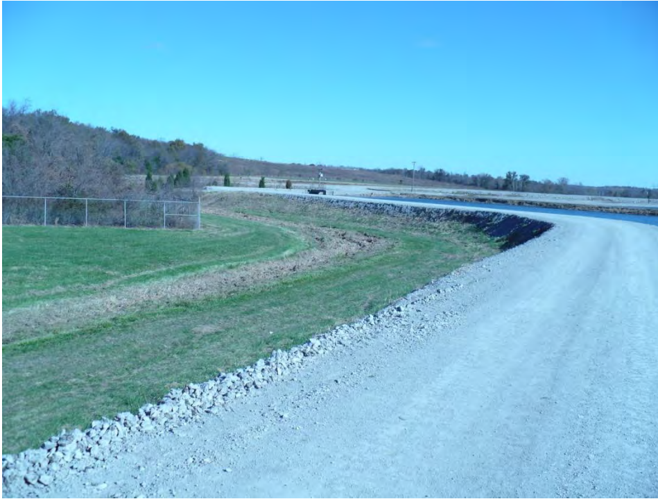
Photo 15: Looking north at the west dike of the Bottom Ash Pond.
