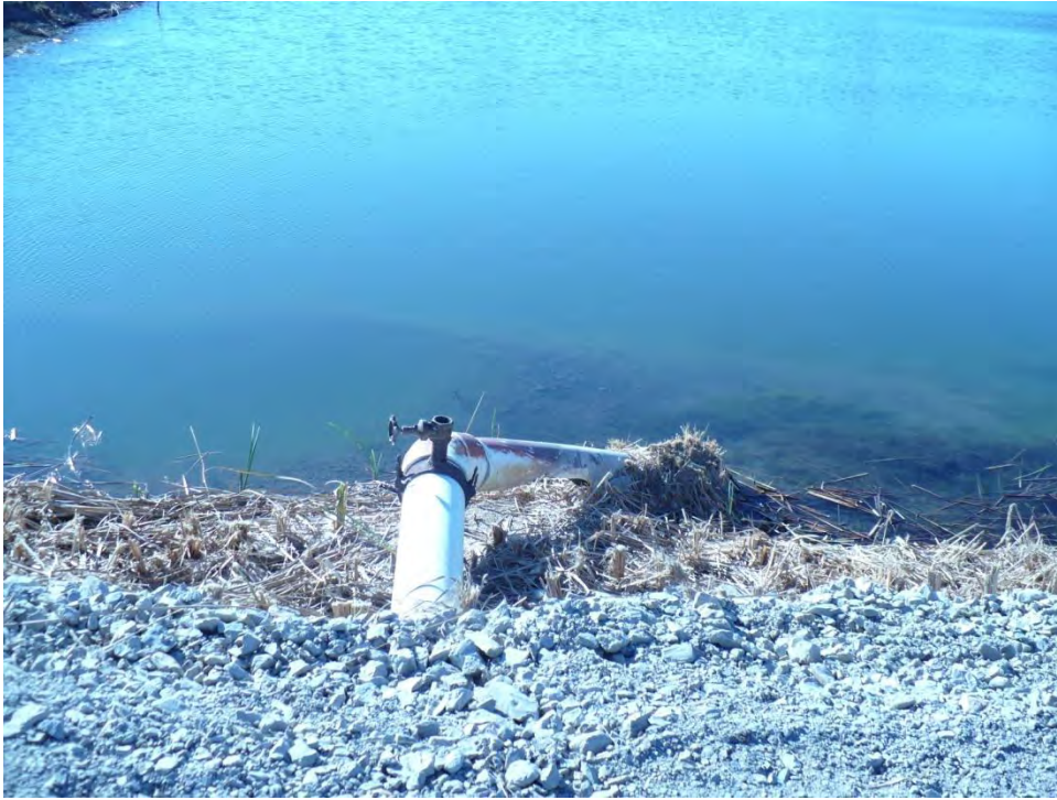
Photo 7: The overflow outlet from the North Flyash Pond into the Bottom Ash Pond.
