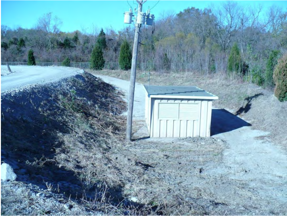
Photo 5: Return water pump house at north end of the Bottom Ash Pond.
