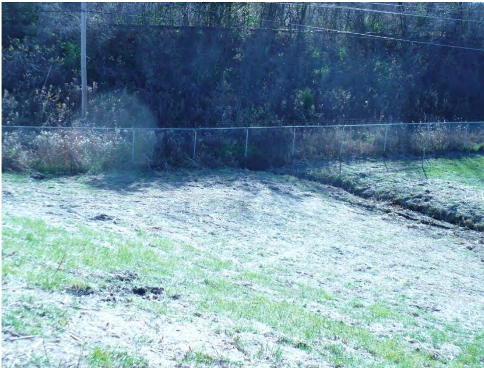
Photo 4: Looking east from the North Ash Pond dike at the abandoned railroad embankment. Site storm water is discharged to a 48 inch diameter culvert.
