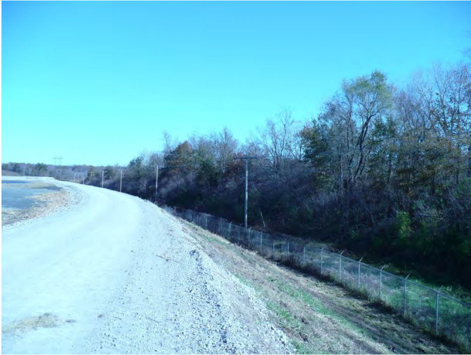
Photo 11: Looking north at the east dike of the South Fly Ash Pond.
