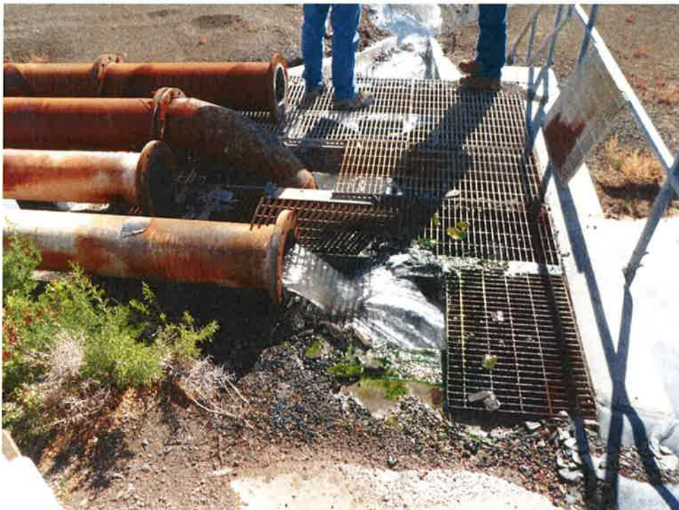
Photo 30: Bottom Ash Basin #3, looking at inlet pipeline discharging into rundown structure.
