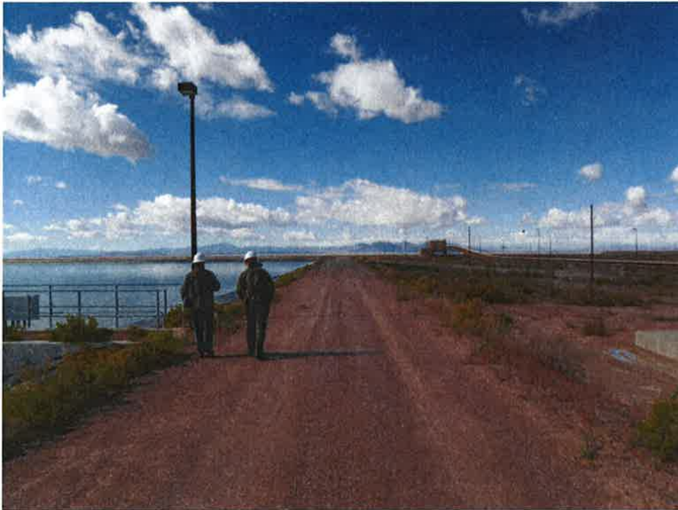
Photo 3: Wastewater Holding Pond, looking west at north dike crest and downstream slope.
