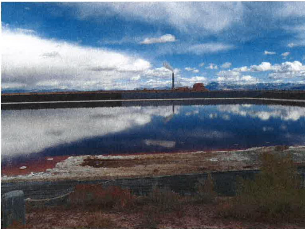
Photo 44: Evaporation Pond #2, looking east at reservoir area and upstream liner, note considerable salt accumulation.
