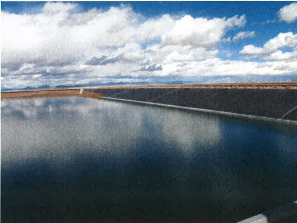
Photo 26: Bottom Ash Basin #3, looking northeast at BA#2/#3 inner dike and liner.
