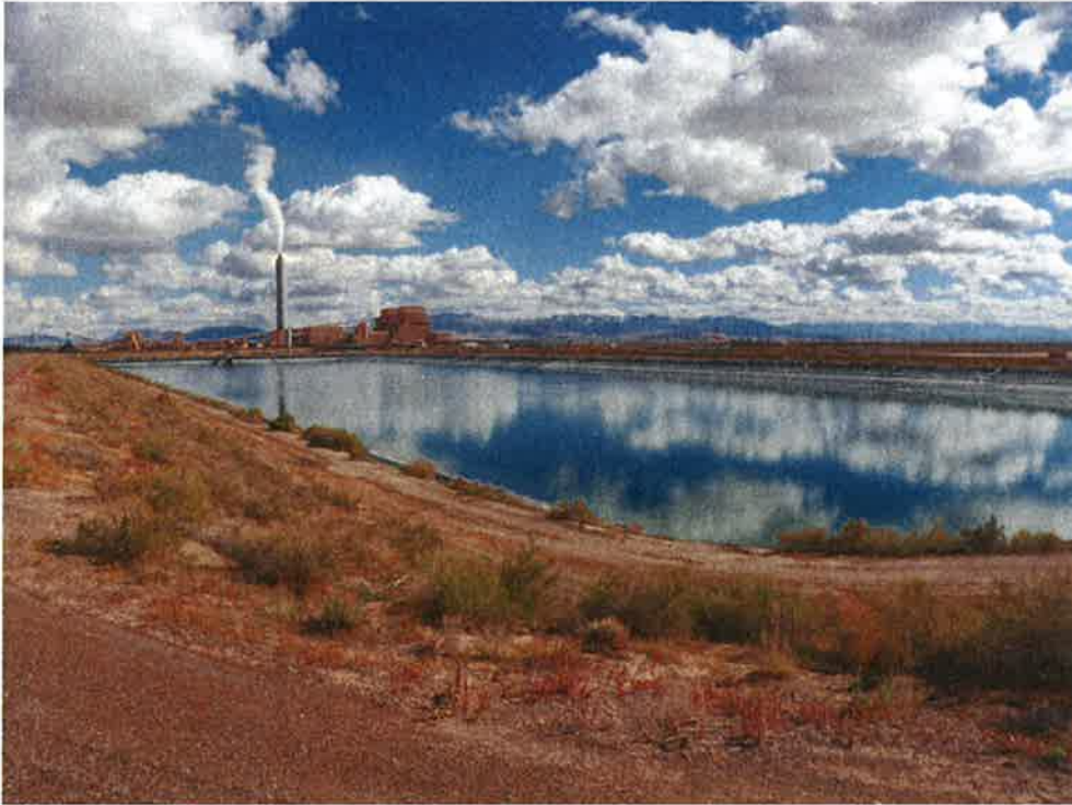
Photo 23: Settling Basin, looking east from BA#3 south dike at settling basin reservoir area.
