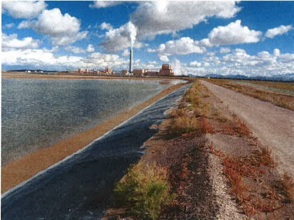
Photo 18: Wastewater Holding Pond, looking east at south dike upstream slope and liner.
