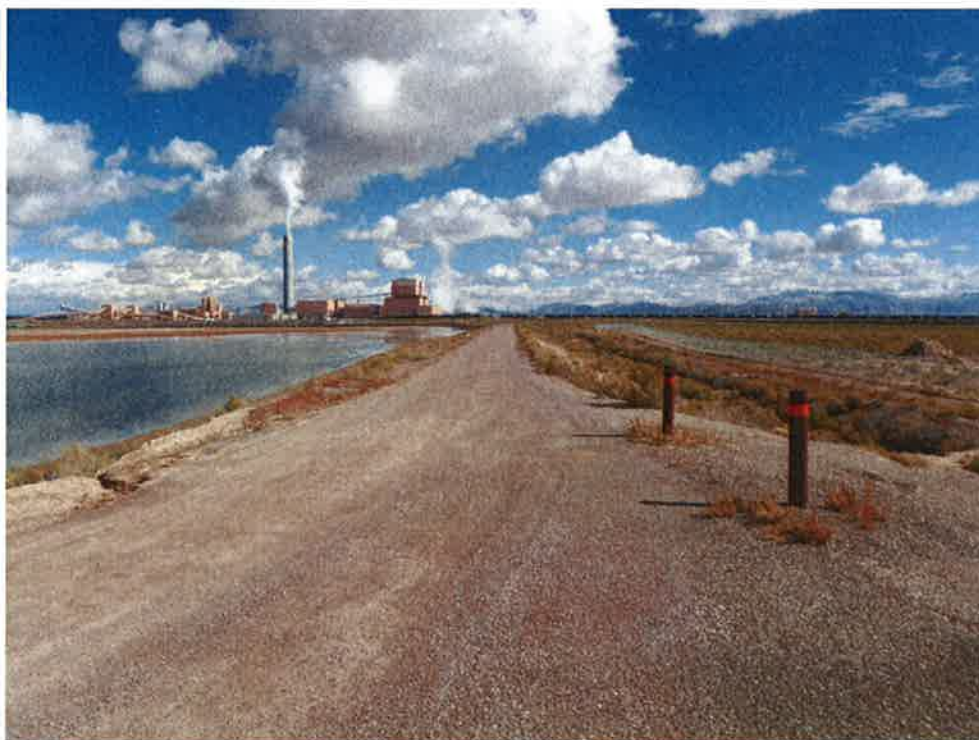
Photo 17: Wastewater Holding Pond, looking east at south dike crest.
