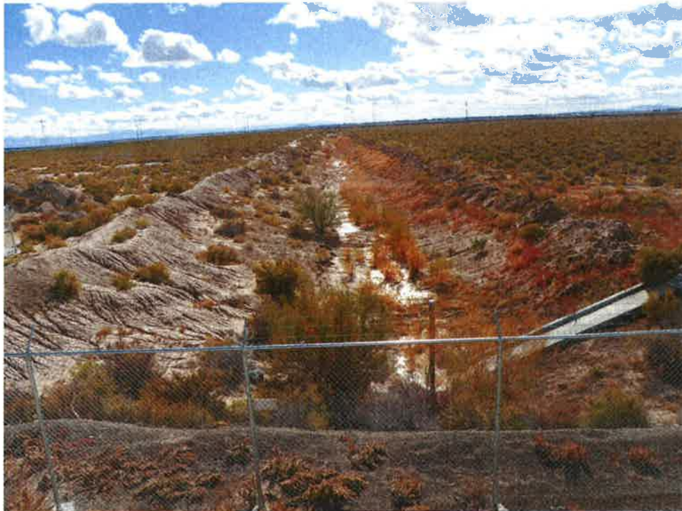
Photo 16: Wastewater Holding Pond, looking south from south dike at stormwater channel.
