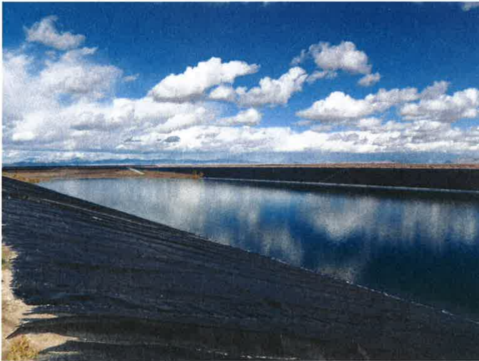
Photo 21: Bottom Ash Basin #3, looking northeast from west dike at reservoir area and east inner dike.
