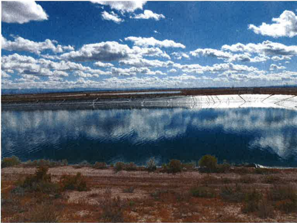
Photo 27: Bottom Ash Basin #2, looking south from south dike at Settling basin slopes and reservoir area.
