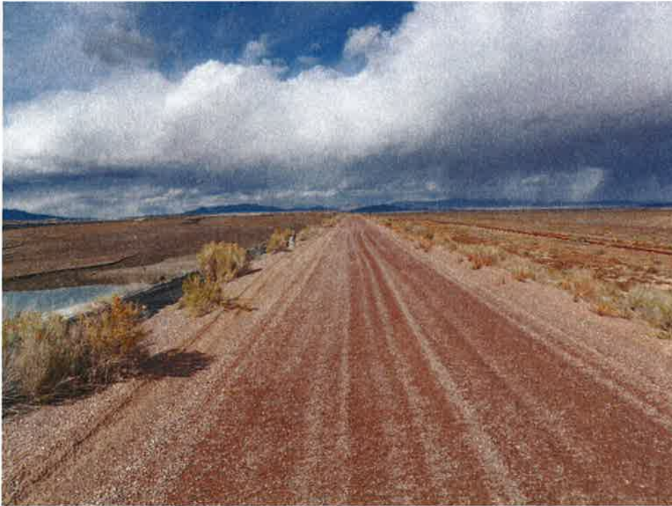
Photo 39: Bottom Ash Basin #1, looking north at east dike crest.
