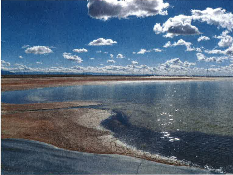
Photo 1: Wastewater Holding Pond, looking south from north dike.
