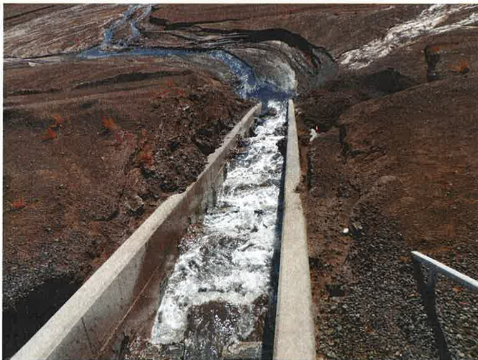
Photo 31: Bottom Ash Basin #3, looking at discharge through rundown structure.
