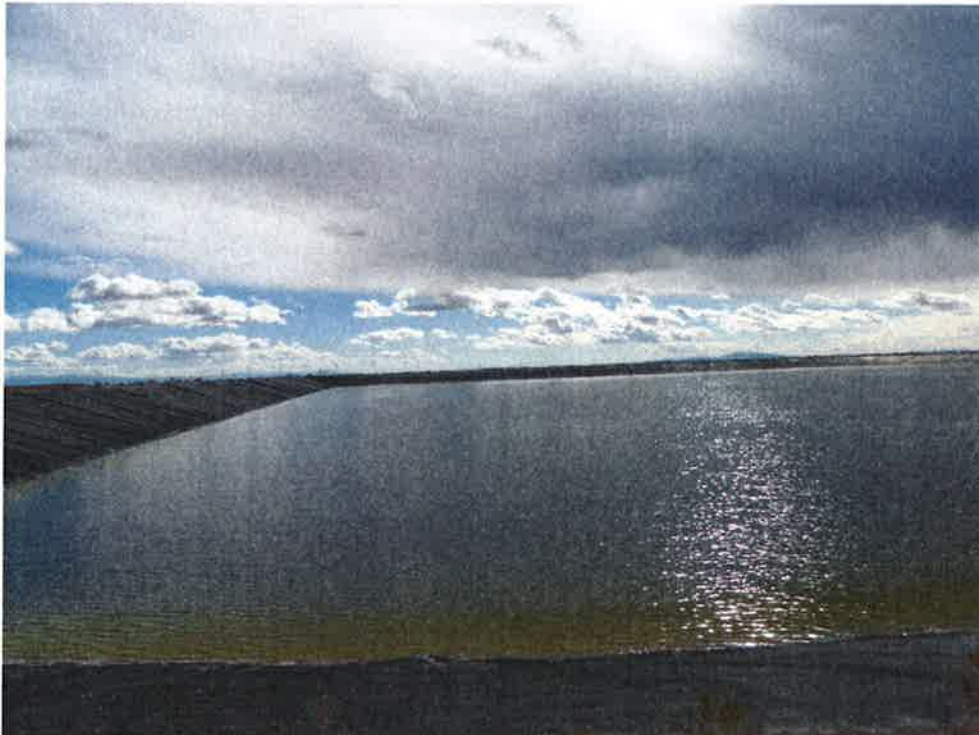
Photo 42: Evaporation Pond #6, looking south at reservoir area and upstream liner.
