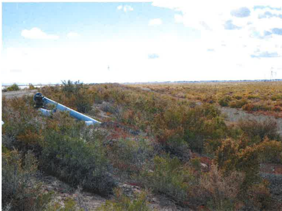
Photo 12: Wastewater Holding Pond, looking south at west dike downstream slope.
