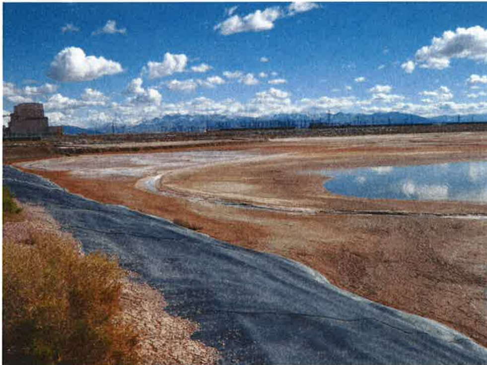
Photo 10: Wastewater Holding Pond, looking east at east dike and liner.
