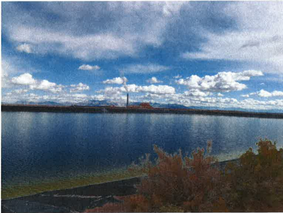
Photo 43: Evaporation Pond #6, looking southeast at reservoir area and inner dikes.
