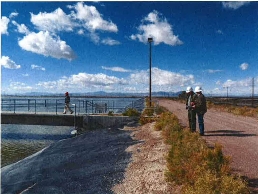
Photo 2: Wastewater Holding Pond, looking west at north dike upstream slope.
