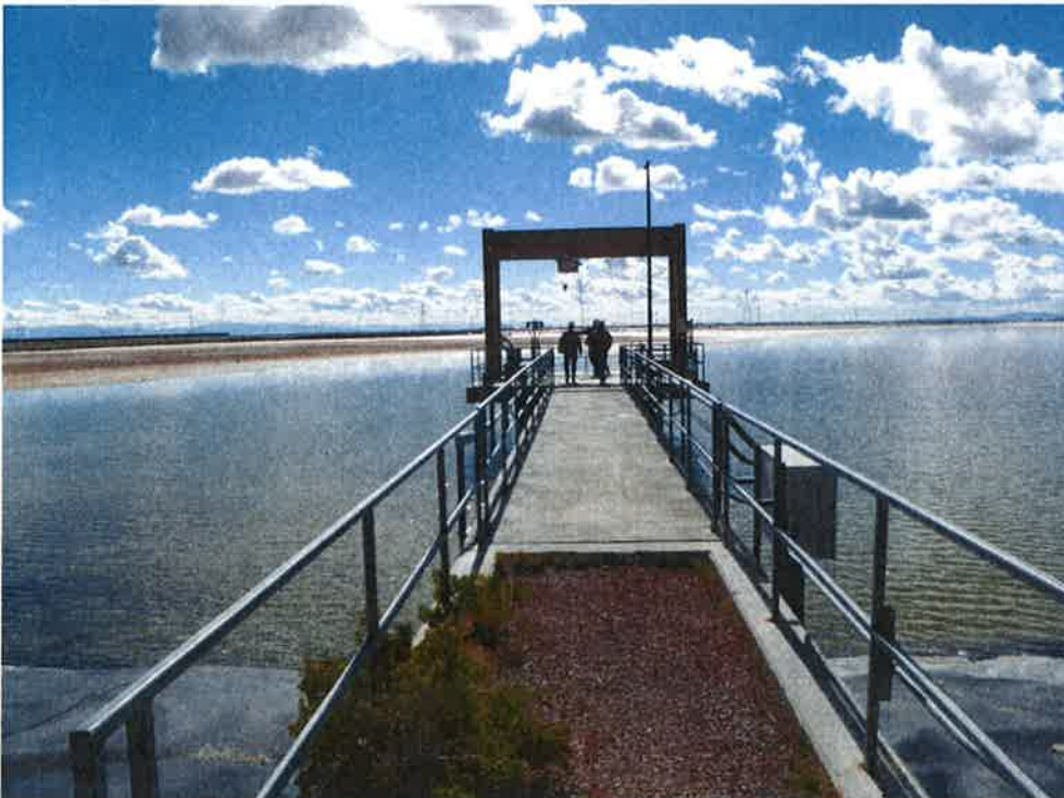
Photo 4: Wastewater Holding Pond, looking south at intake structure from north dike.
