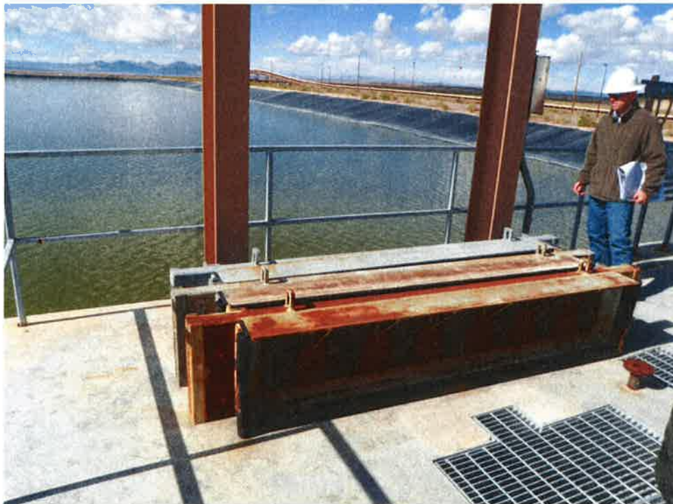
Photo 6: Wastewater Holding Pond, intake structure steel stop logs.
