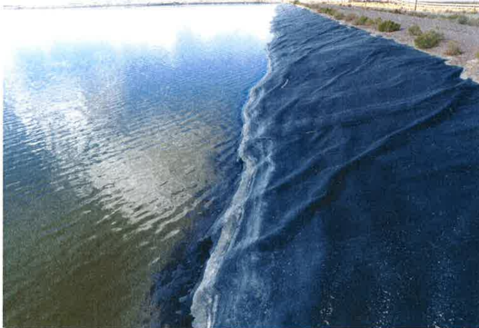
Photo 9: Wastewater Holding Pond, looking west at north dike liner.
