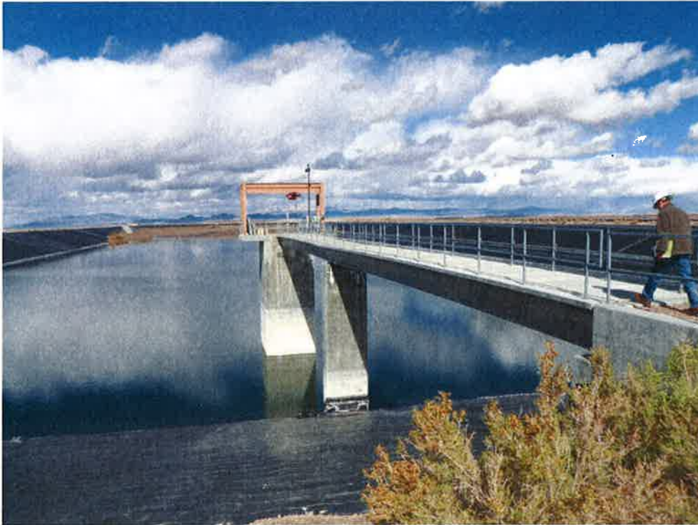
Photo 25: Bottom Ash Basin #3, looking north at intake structure.
