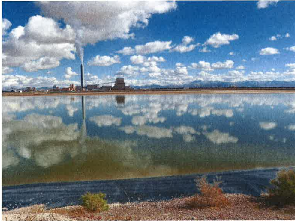
Photo 15: Wastewater Holding Pond, looking east at reservoir area and east dike from west dike.
