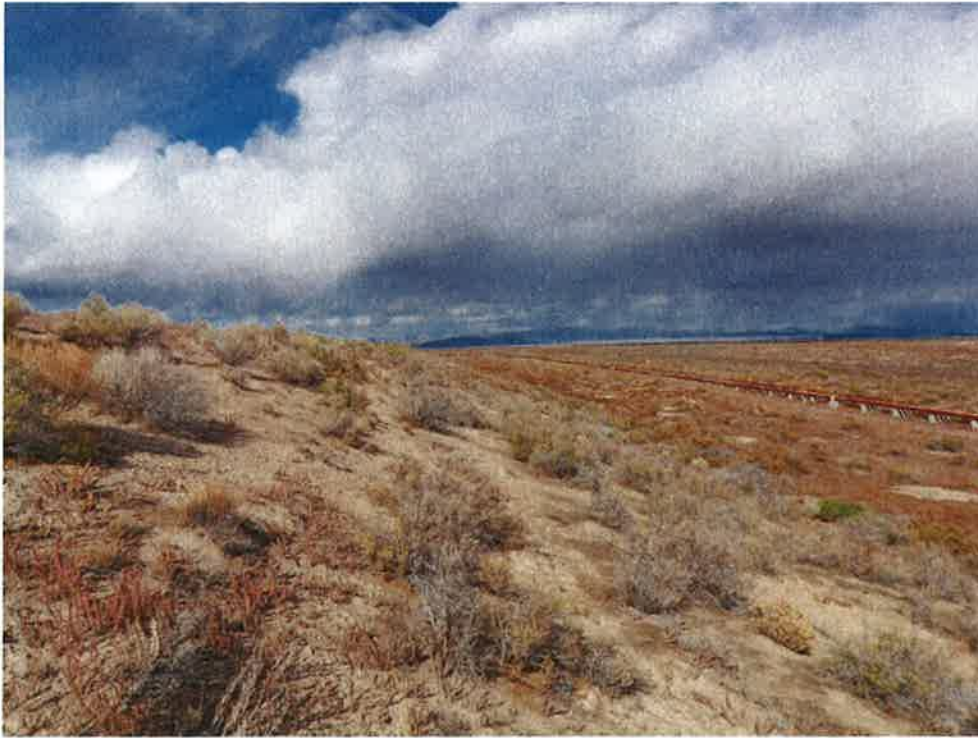
Photo 37: Bottom Ash Basin #1, looking north at east dike downstream slope.
