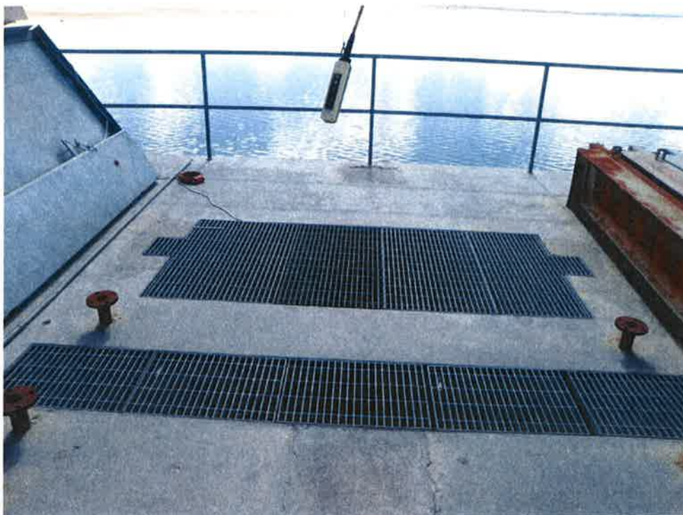
Photo 8: Wastewater Holding Pond, Intake structure platform and removable grate.
