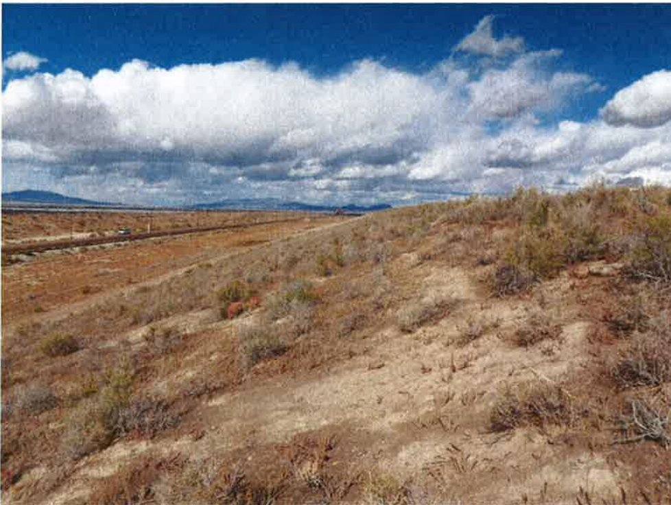
Photo 22: Bottom Ash Basin #3, looking north at west dike downstream slope.
