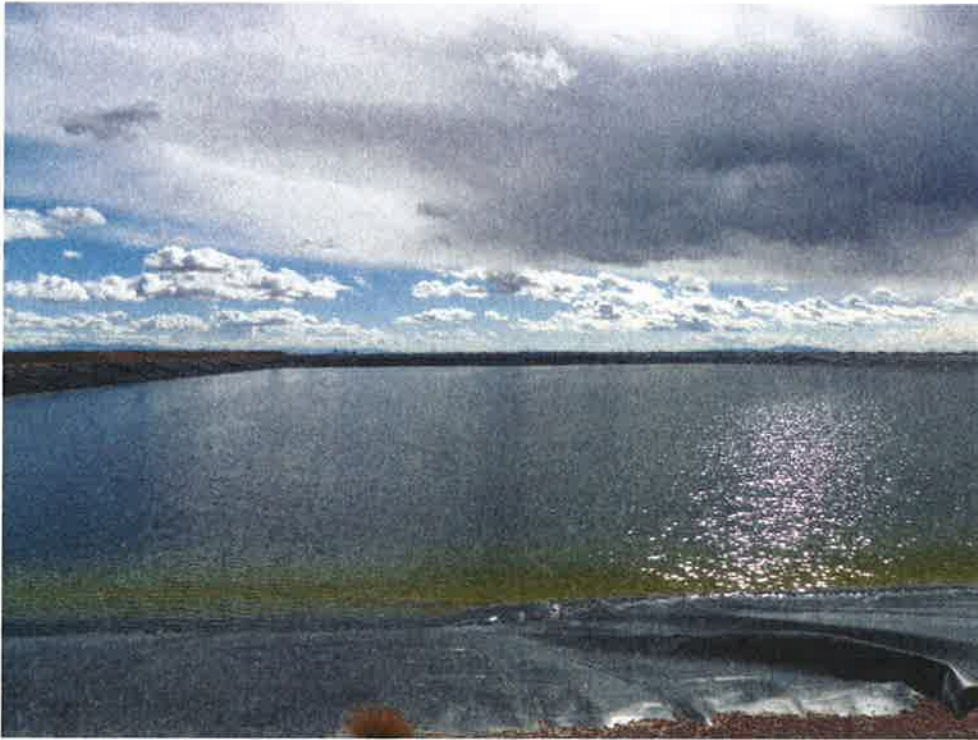
Photo 41: Evaporation Pond #5, looking south at reservoir area and upstream liner.
