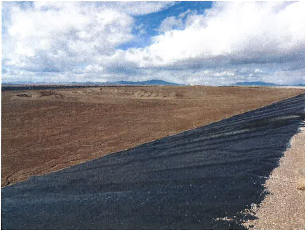
Photo 35: Bottom Ash Basin #2, looking northwest from inner dike at inlet and reservoir area.
