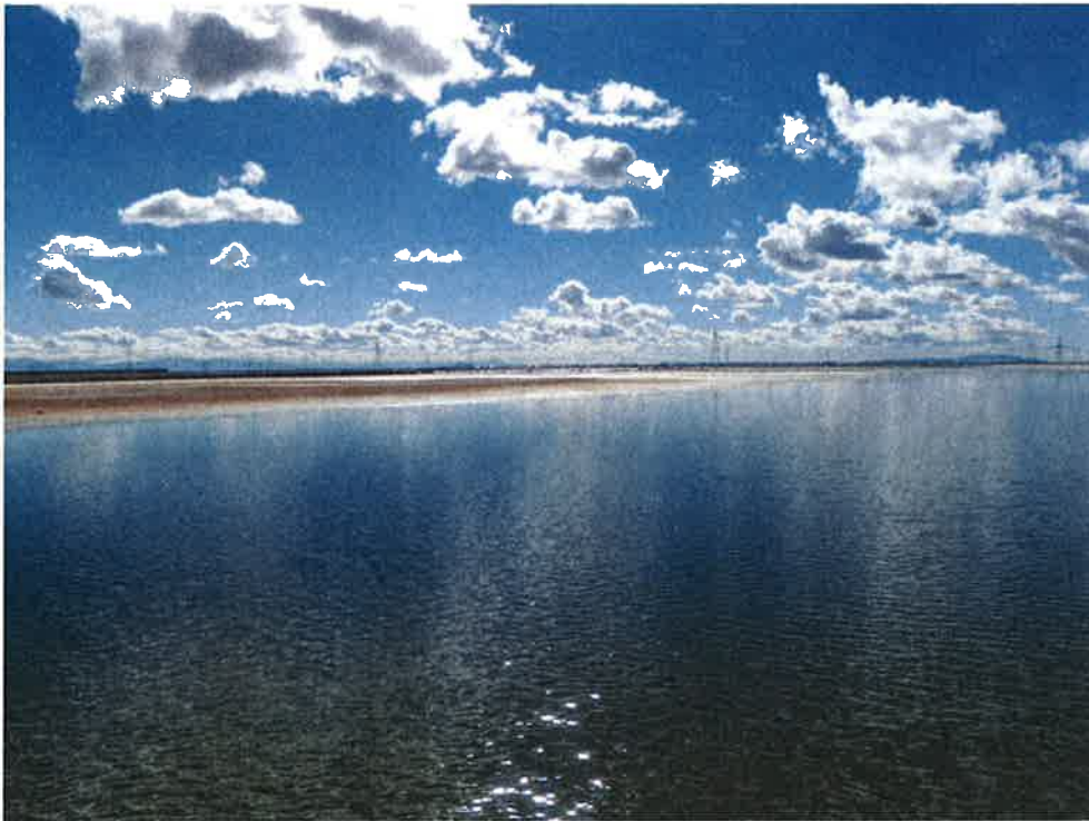
Photo 5: Wastewater Holding Pond, looking south at reservoir area from intake structure.
