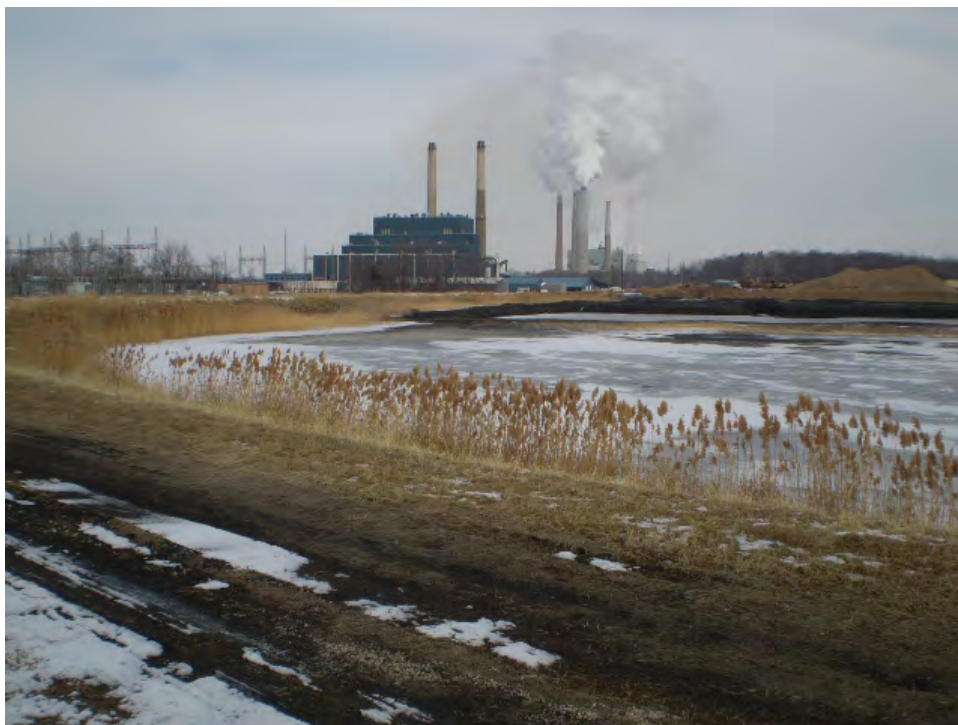
Photo 16: Northeast Corner of Pond 4
