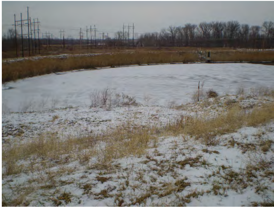
Photo 19: Settling Basin at North End of Pond 4
