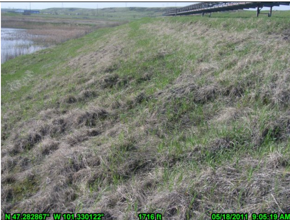
6-Surface Erosion on Original Landside East Embankment (looking south)
