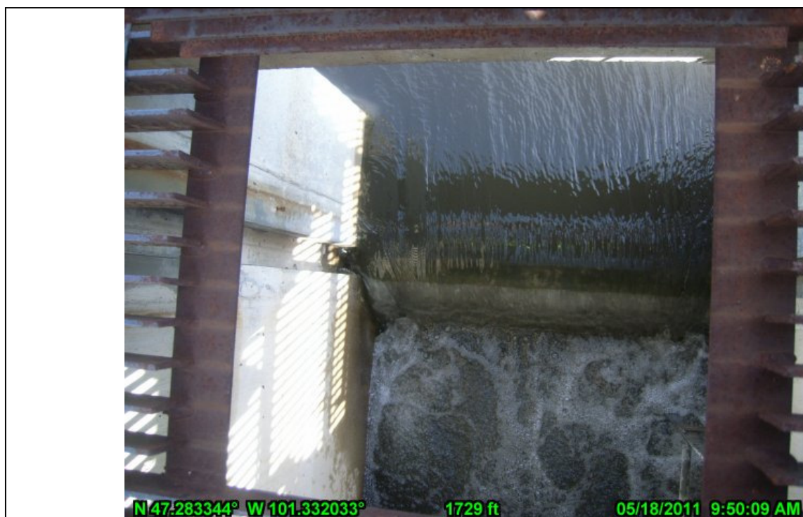
26-North Pond Decant Intake with Stop Logs
