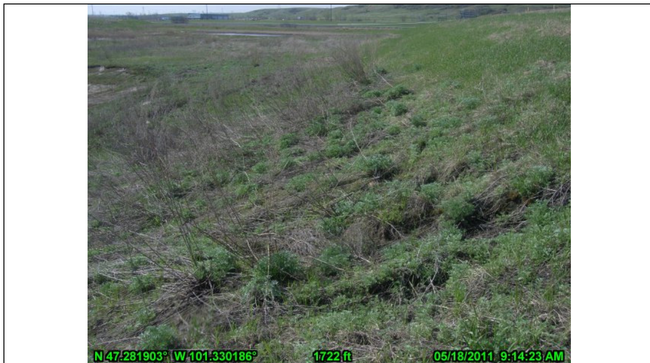
10-Erosion and Vegetation on Slope of Original Landside East Embankment (looking south)
