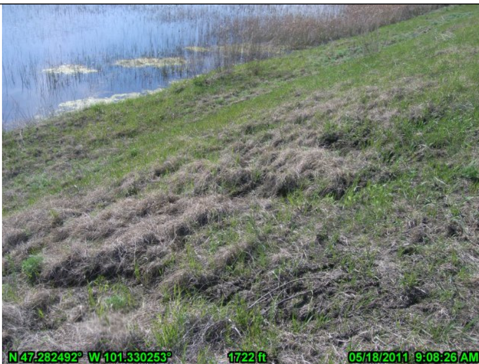
8-Erosion Rills on Original Landside East Embankment (looking southeast)
