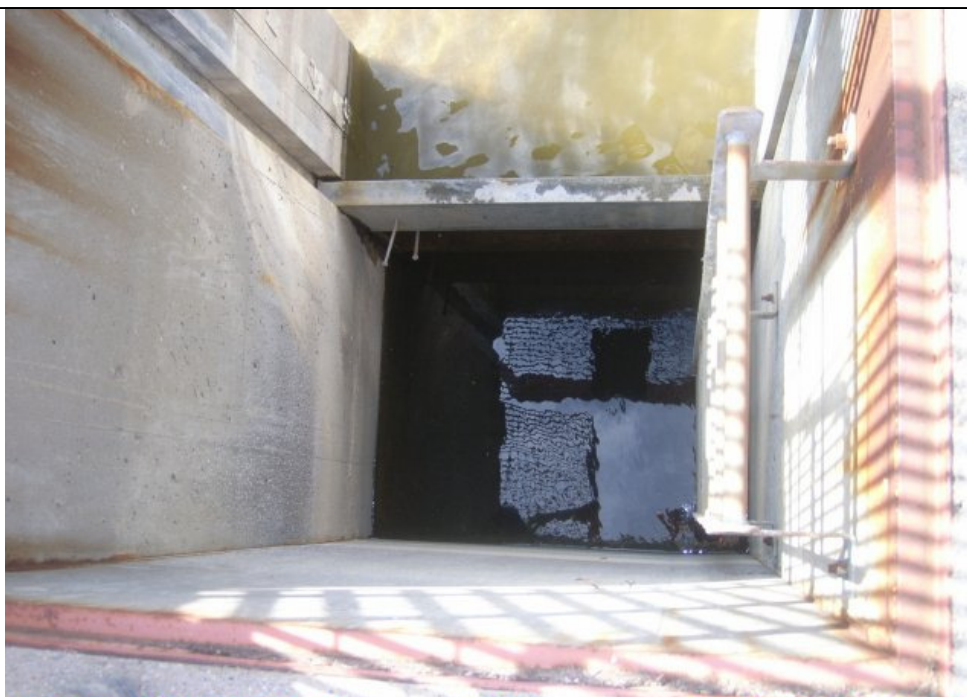
18-South Pond Decant Inlet Structure, Not in Use
