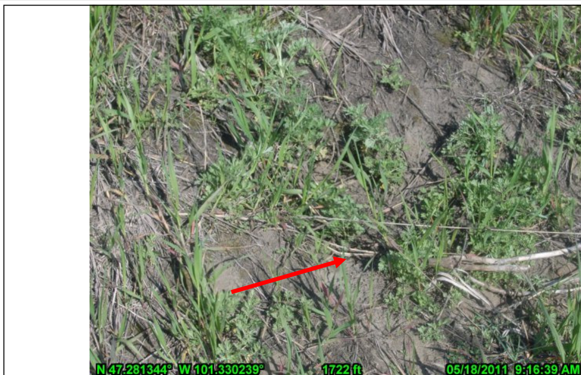
11-Animal Burrow on Landside East Embankment
