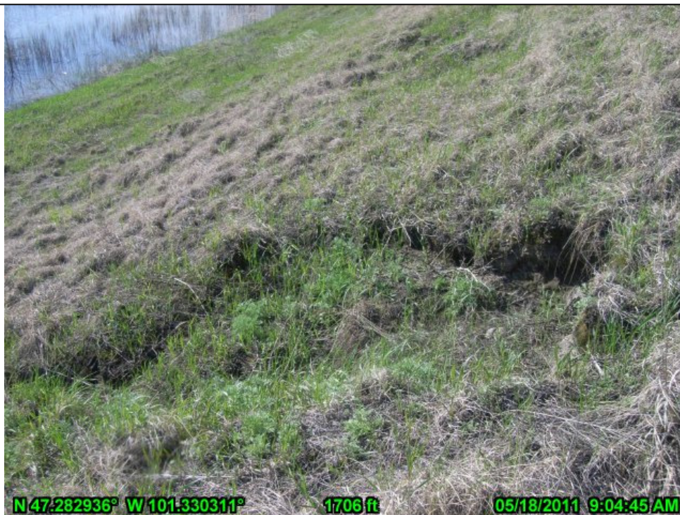
5-Scarp on Original Landside East Embankment (looking southwest)
