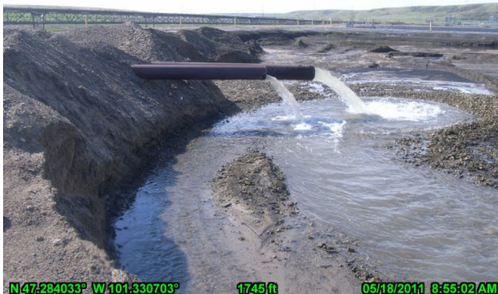
1-North Ash Pond 12" and 16" Steel Pipe Inlets (looking south)
