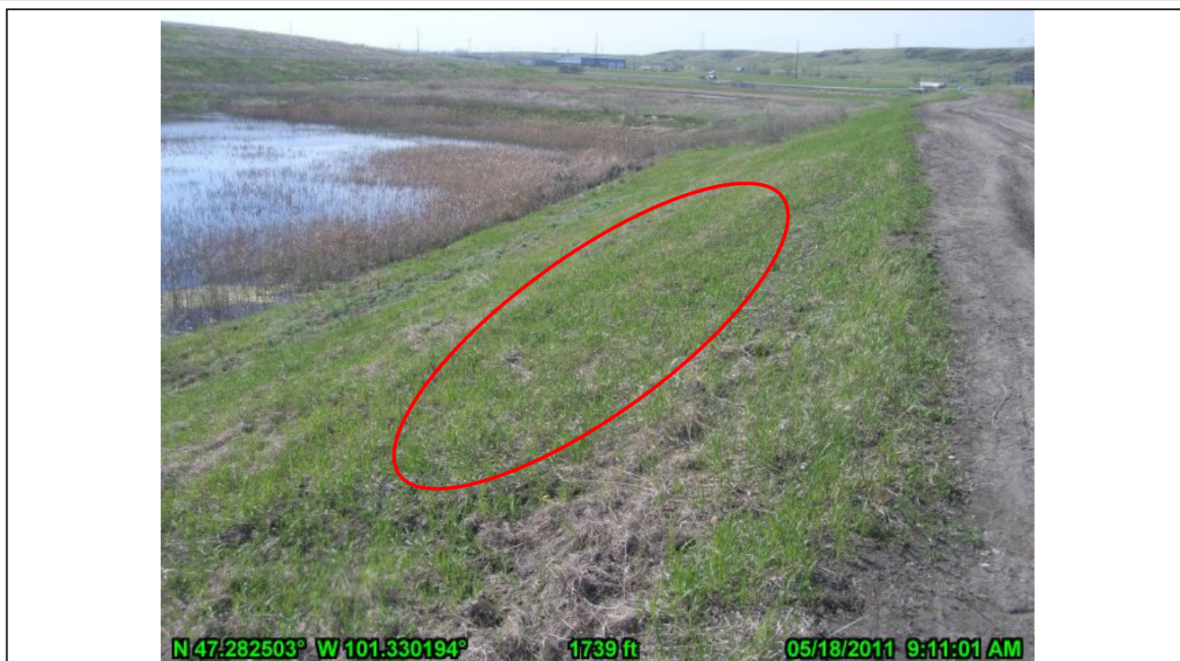
9-Bulging of Original Landside East Embankment (looking south)
