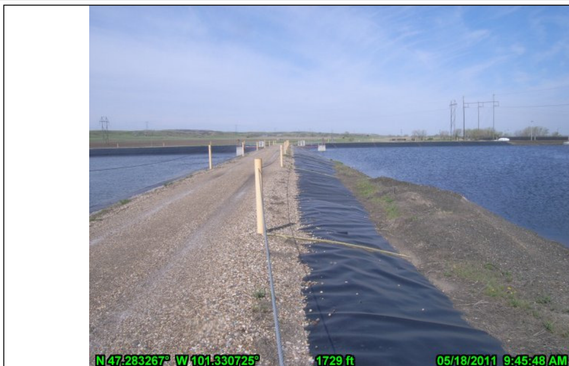
25-Divider Dike Liner on South Side of North Pond (looking west)
