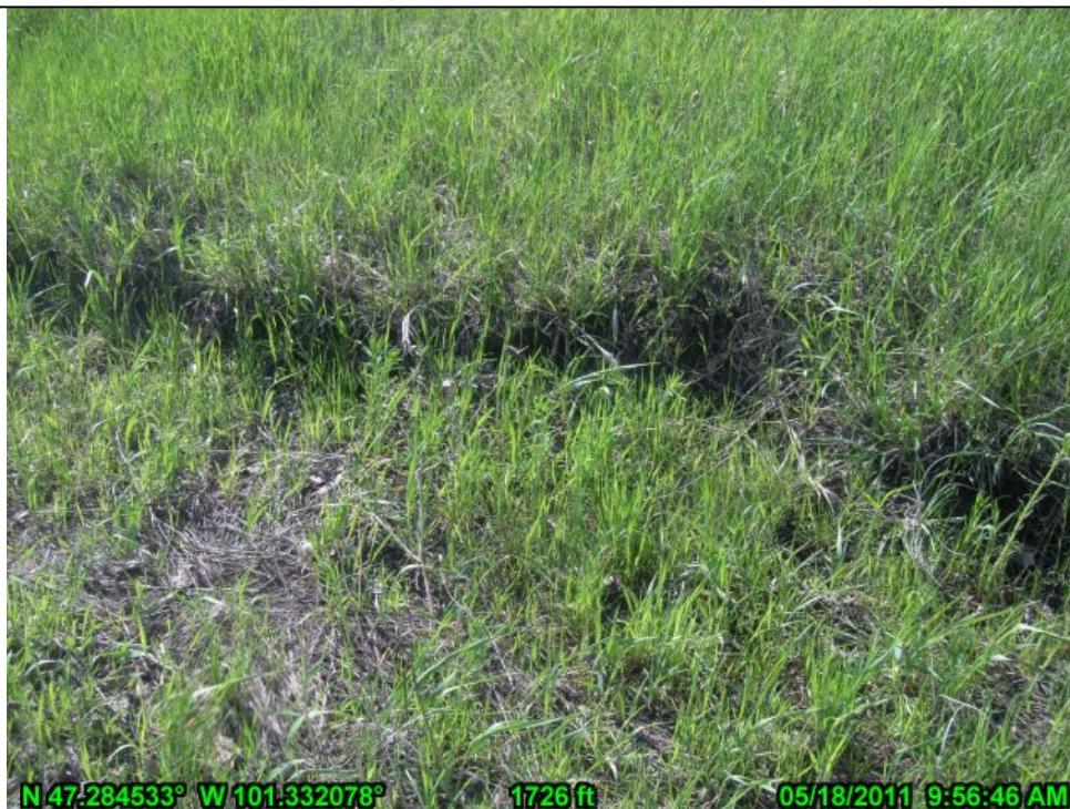
33-Scarp at Toe of North Embankment Approximately 8" Deep
