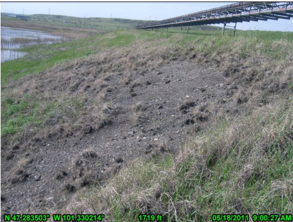
4-Landside Erosion on Original East Embankment from Sluice Pipe Leak (looking south)
