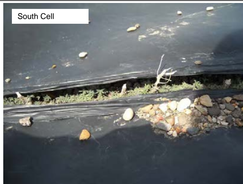
Open Geomembrane Seam on West Upstream Slope (082)
