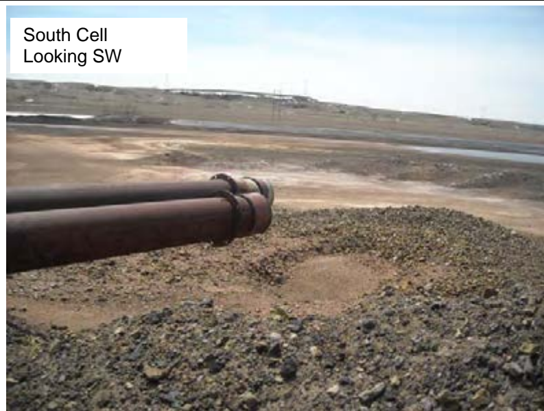
Bottom Ash Inlet Pipes (091)
