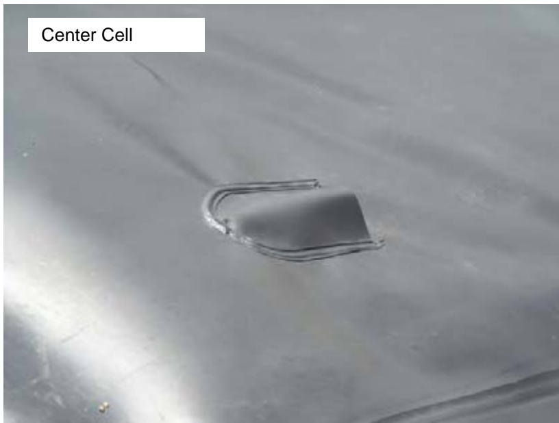
Vent in Geomembrane Liner (057)
