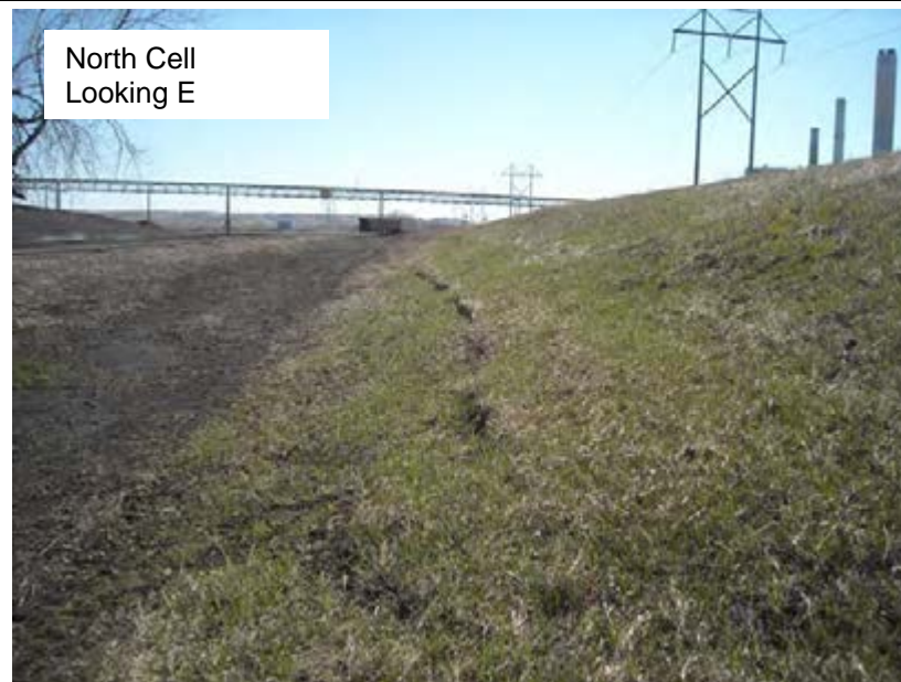
Steepened Toe of North Downstream Slope (023)
