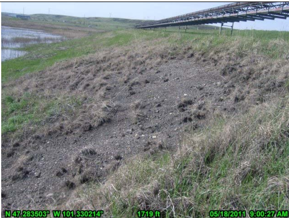
4-Landside Erosion on Original East Embankment from Sluice Pipe Blow-out (looking south)
