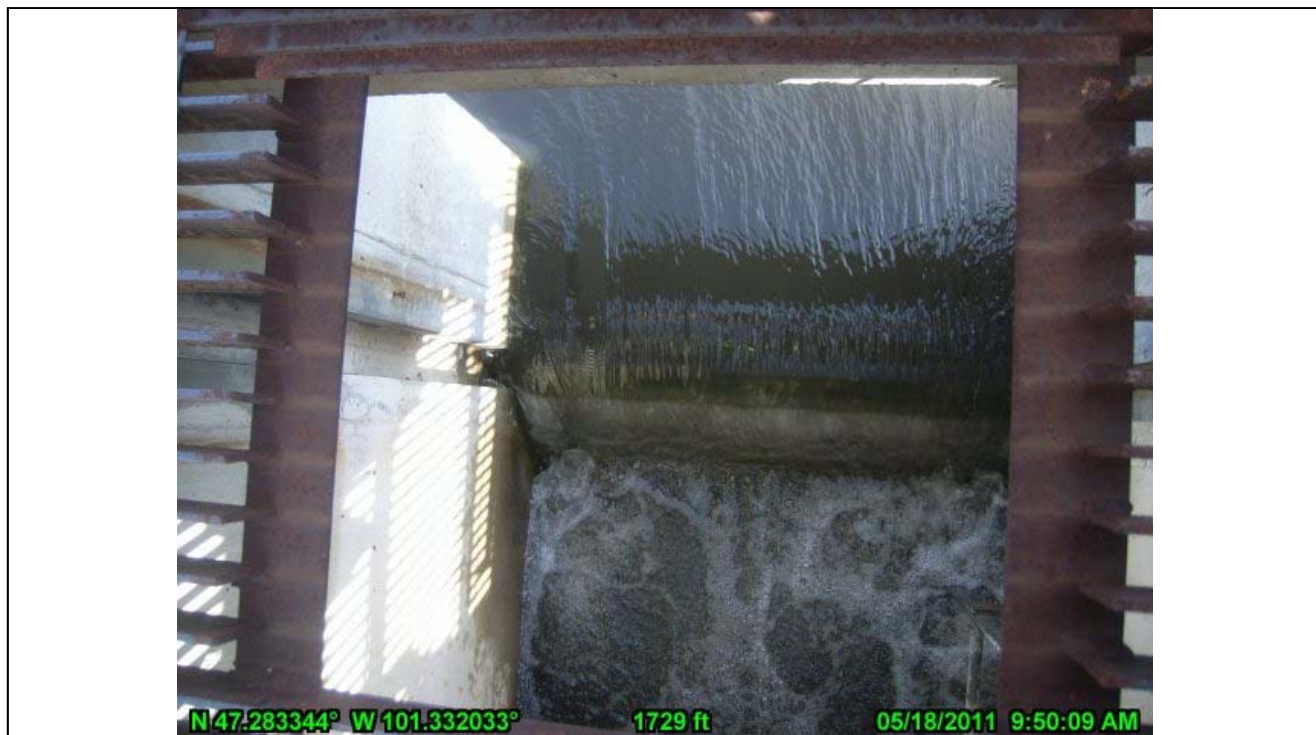
26-North Pond Decant Intake with Stop Logs
