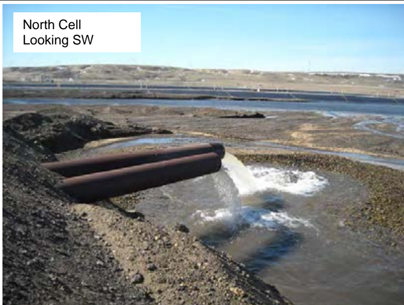
Bottom Ash Inlet Pipes (001)
