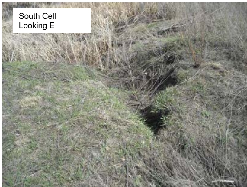
Erosion Rill/Slough/Scarp on East Downstream Slope (103)
