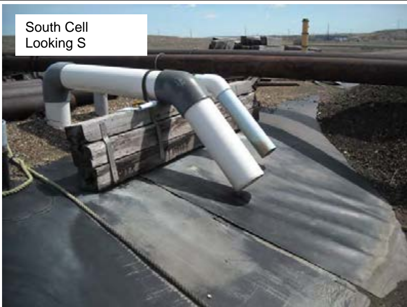
Coal Pit and Retention Ponds Inlets (090) Trapped Water Between Geomembrane and Clay Liners
