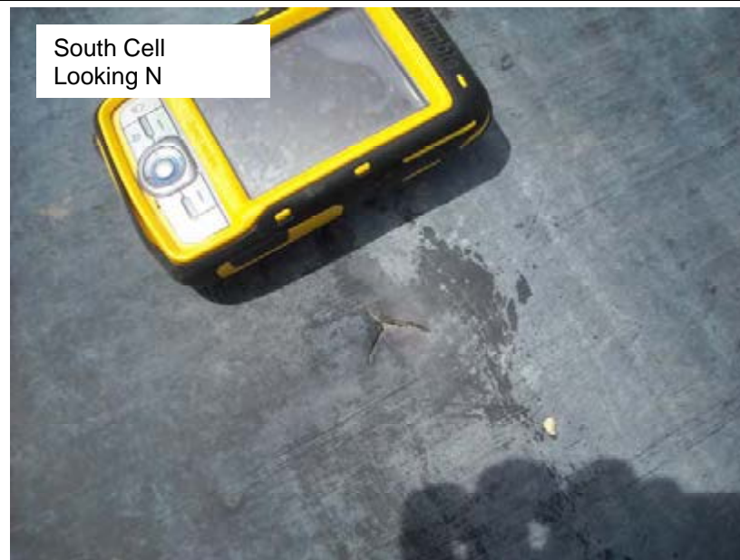
Puncture of Geomembrane Liner on North Upstream Slope (089)
