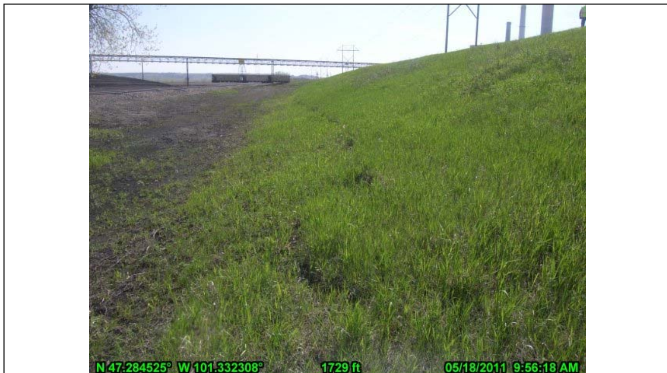
32-Approximately 100' Long Scarp Along Toe of North Embankment (looking east)
