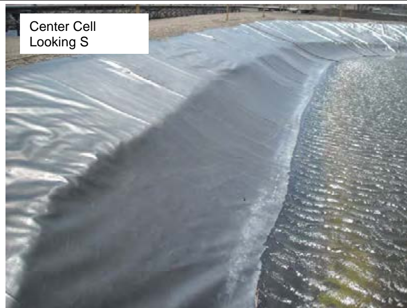
Displacement of Lower Upstream Slope, East Berm (056)
