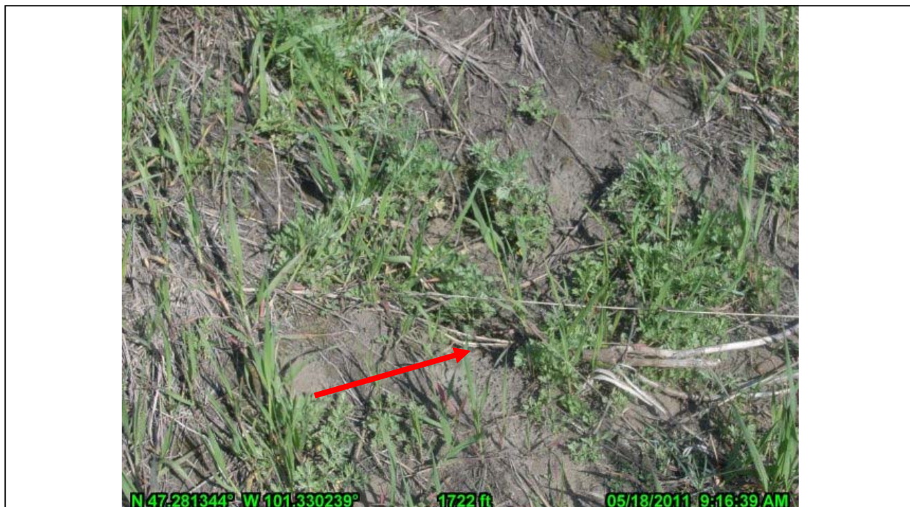
11-Animal Burrow on Landside East Embankment
