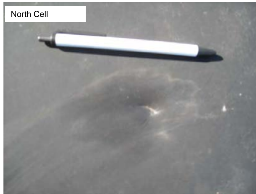
Small Puncture in Geomembrane Liner (006)
