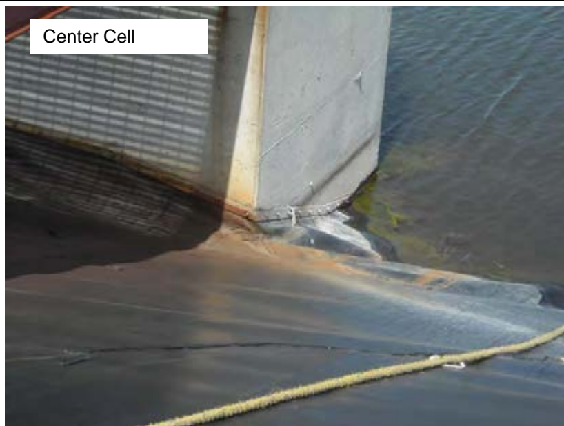
Geomembrane Attachment to Inlet Structure (052)
