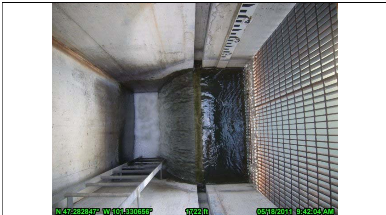
23-Center Pond Outfall Structure and Trashrack
