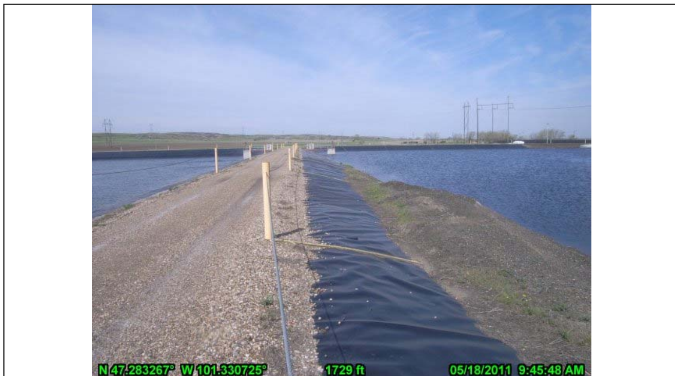
25-Divider Dike Liner on South Side of North Pond (looking west)
