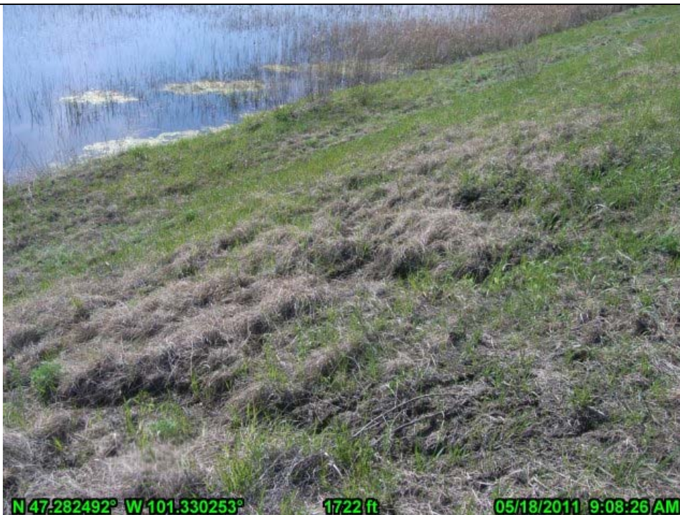
8-Erosion Rills on Original Landside East Embankment (looking southeast)
