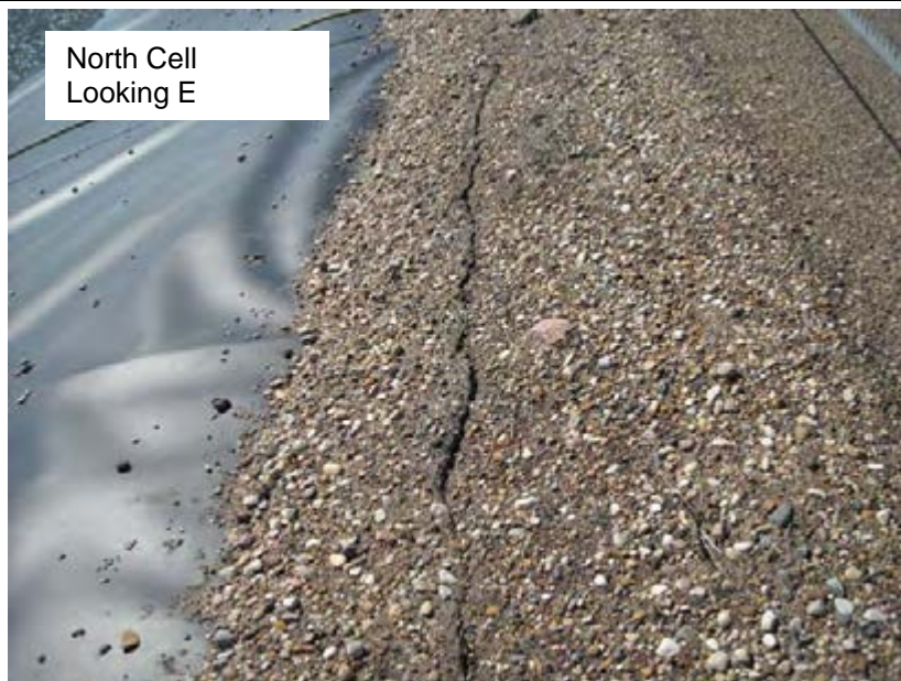
Crack in Shallow Cover over Anchor Trench (021)
