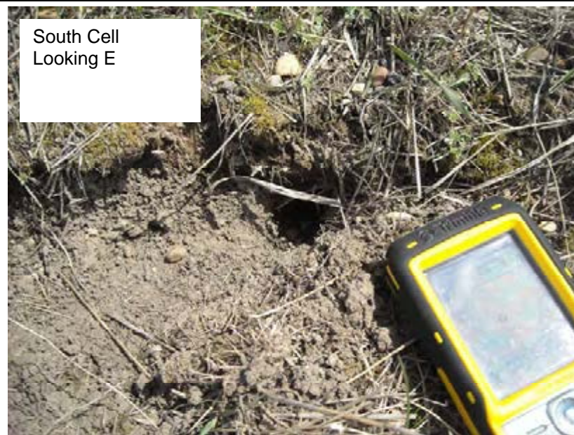
Small Animal Burrow in East Downstream Slope (079)
