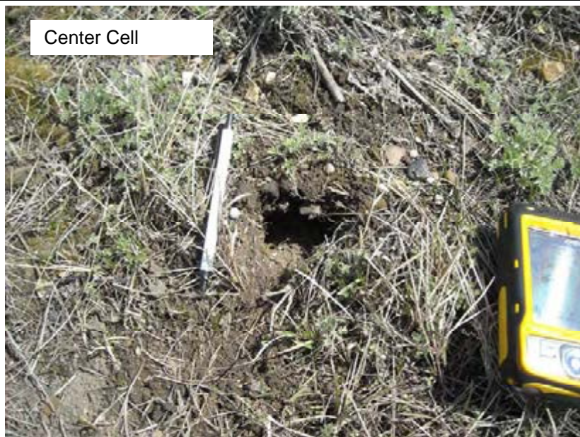
Small Animal Burrow on West Downstream Slope (048)
