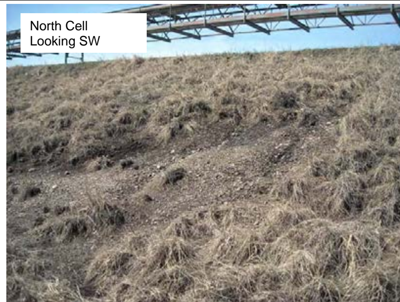
Erosion and Bottom Ash on East Downstream Slope (027)
