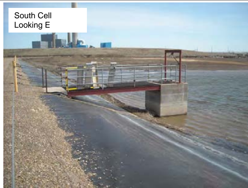
Outlet Structure on North Berm (087)
