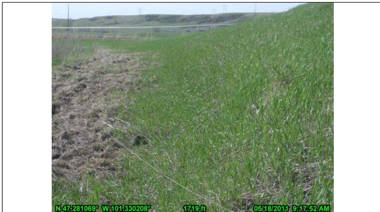
12-Toe of Original East Embankment Over Steepened (looking south)
