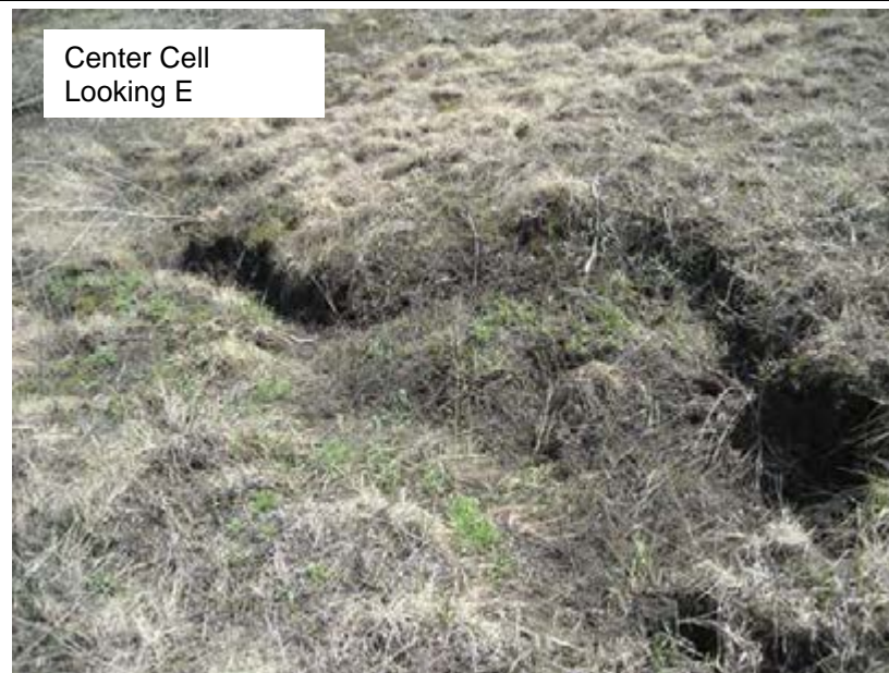
Erosion Rill/Slough/Scarp on East Downstream Slope (064)
