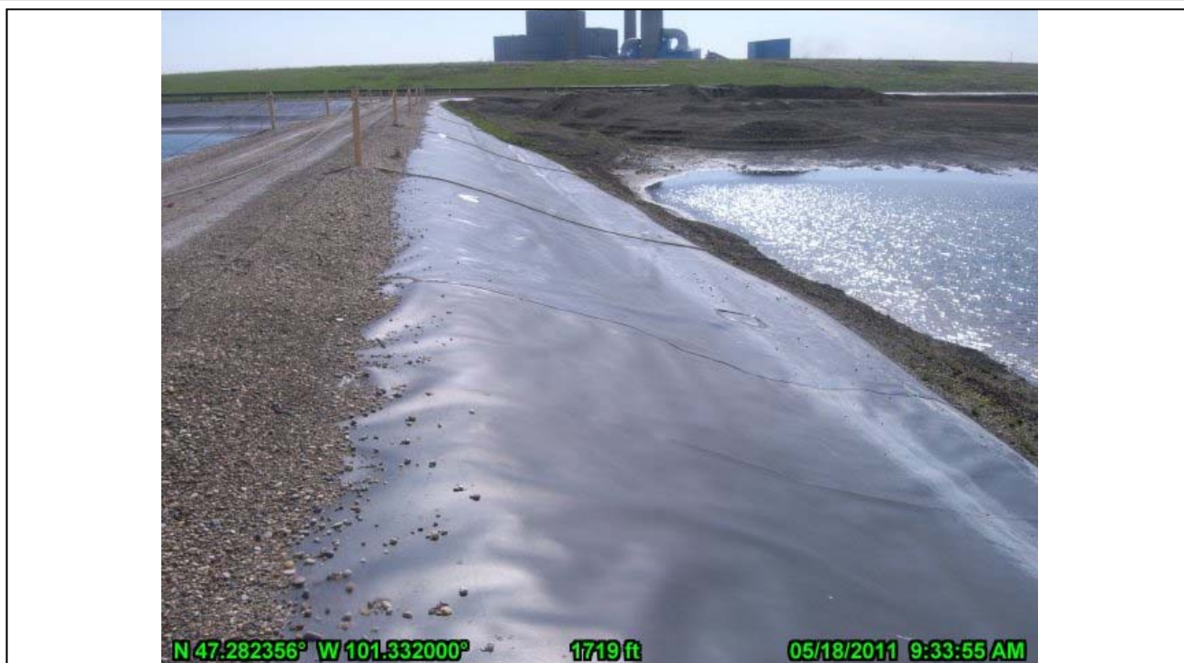
19-Divider Dike Liner on North Side of South Pond (looking east)
