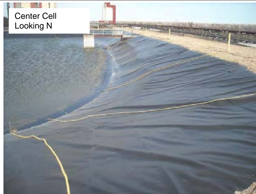
Displacement of Lower Upstream Slope, East Berm (054)
