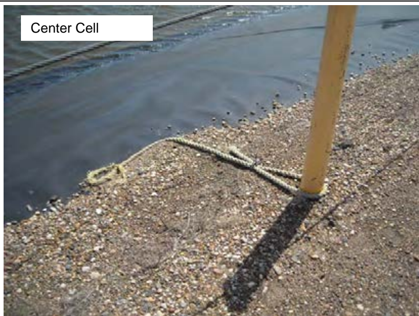
Damaged/Broken Egress Safety Rope (045)
