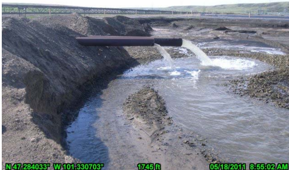
1-North Ash Pond 12" and 16" Steel Pipe Inlets (looking south)
