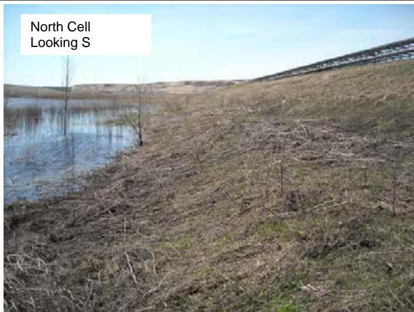
Ponded Water at Toe of East Downstream Slope (028)
