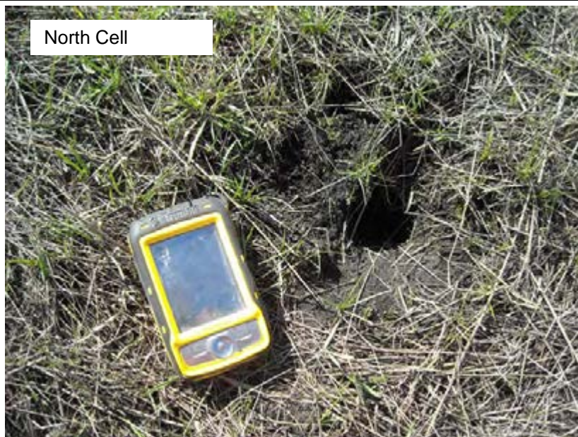
Small Animal Burrow on North Downstream Slope (024)
