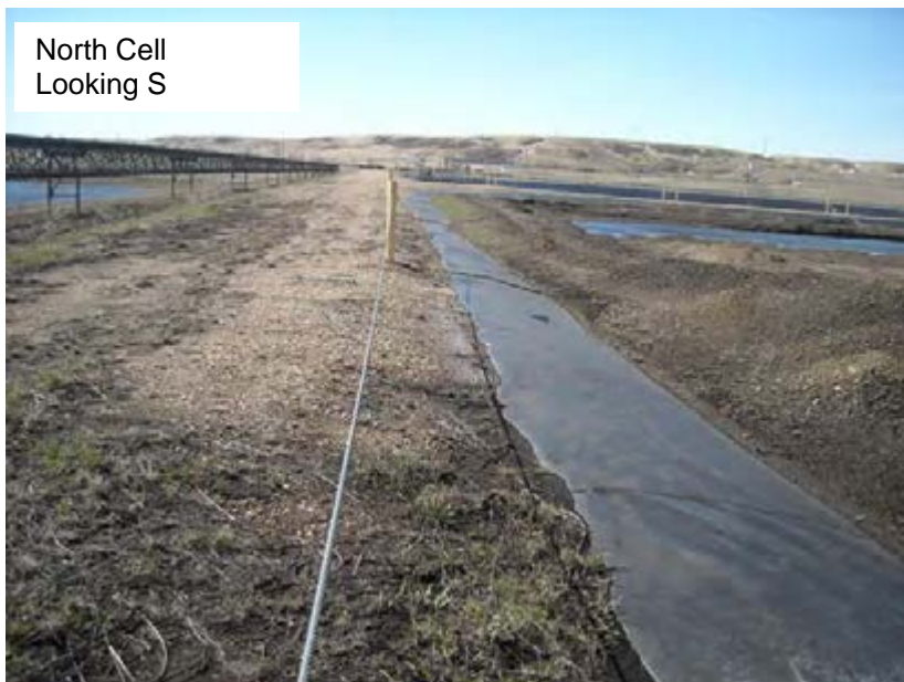
Exposed Geomembrane on East Upstream Slope (004)
