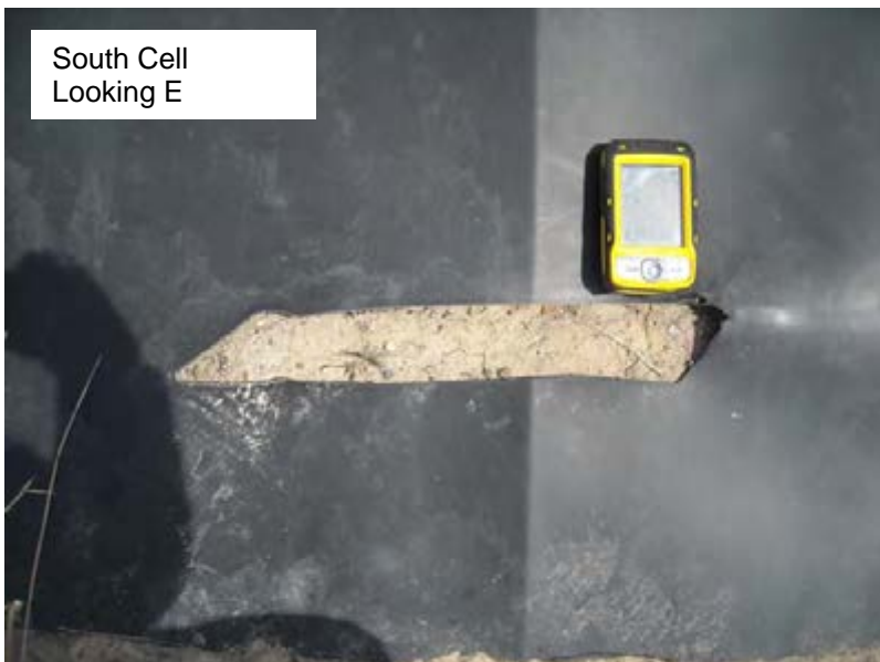
Torn Geomembrane Liner on East Upstream Slope (095)
