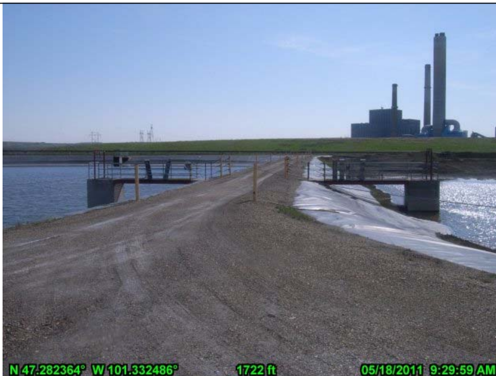
17-Divider Dike between South and Center Ponds with Decant Structure (looking east)
