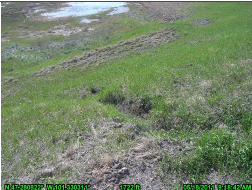
13-Erosion Channel on Original Landside East Embankment (looking east)
