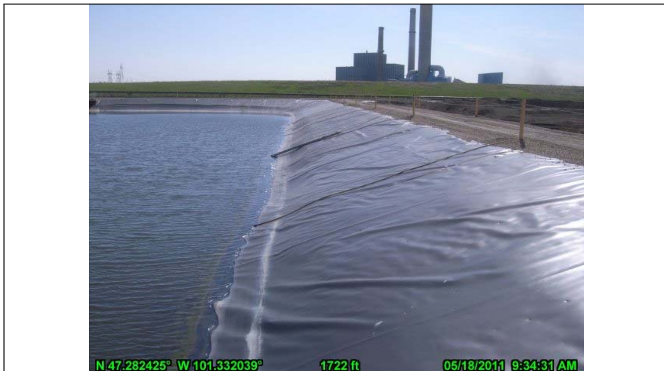
20-Divider Dike Liner on South Side of Center Pond (looking east)
