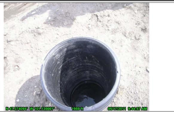
9-Ash Pond 92 Vertical Pipe with Cap, Water 4 Feet Down
