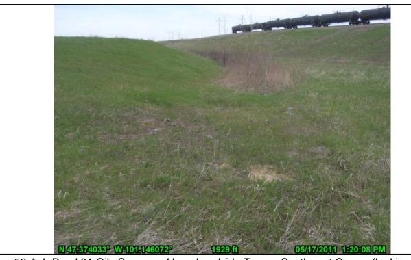
52-Ash Pond 91 Oily Seepage Along Landside Toe on Southwest Corner (looking SE). Source Unknown
