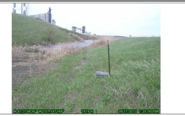
53-Ash Pond 91 Gas Vent Pipe and Slough Along West Embankment (looking north)
