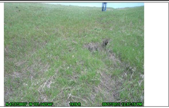
43-Ash Pond 91 Landside Erosion near Ramp Groin (looking northeast)
