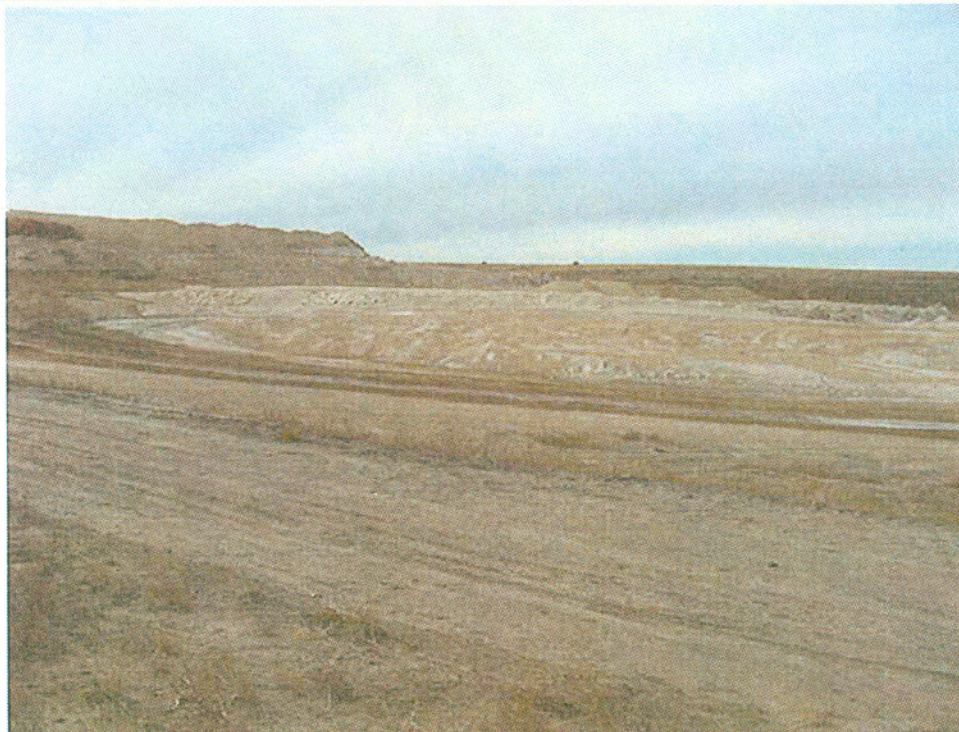
Subject GRE (0085) Description Fly and coal ash disposal site Date 11/19/2009 Location Great River Energy - Stanton (Glenh Witness Derek Laning Time Photographer Kirk Johnson
