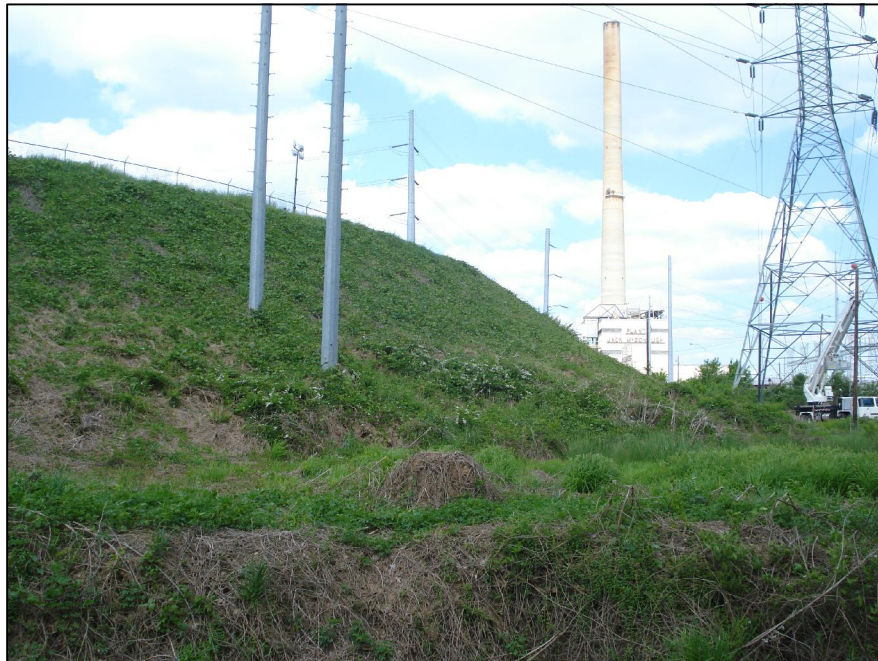
1-6 GENERAL SITE PHOTO
