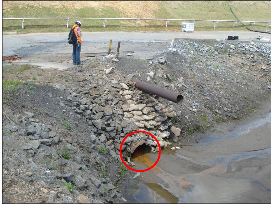
2-5 EMERGENCY OVERFLOW OUTLET
