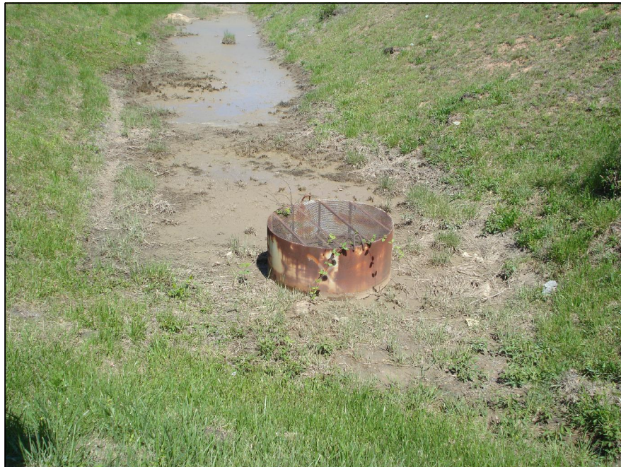
4-6 INLET TO EMERGENCY OVERFLOW DROP STRUCTURE
