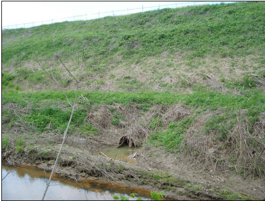
1-3 PRIMARY SPILLWAY OUTLET
