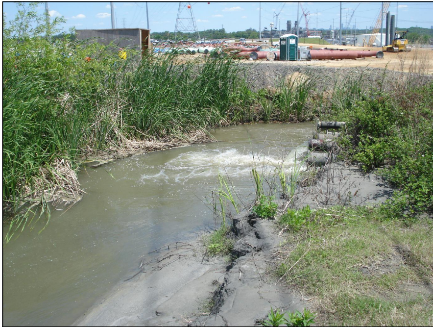
SLUICE LINE DISCHARGE FROM PLANT
