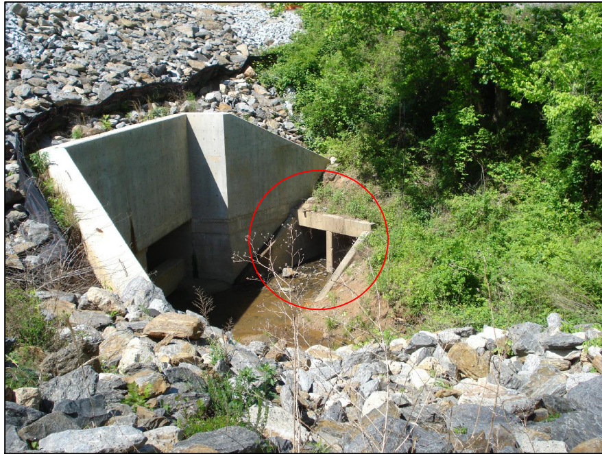
4-5 OUTLET FOR DIVERSION PIPE
