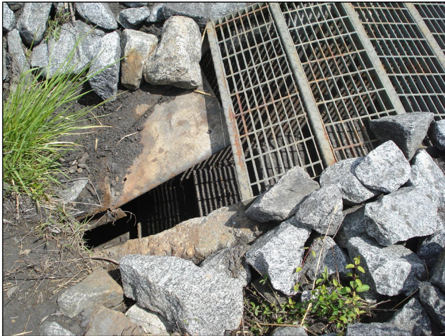
2-4 INLET AT EMERGENCY OUTLET PIPE
