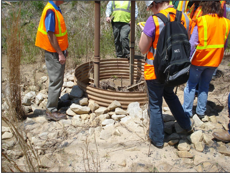
SECONDARY OULET (FORMERLY PRIMARY DISCHARGE STRUCTURE)
