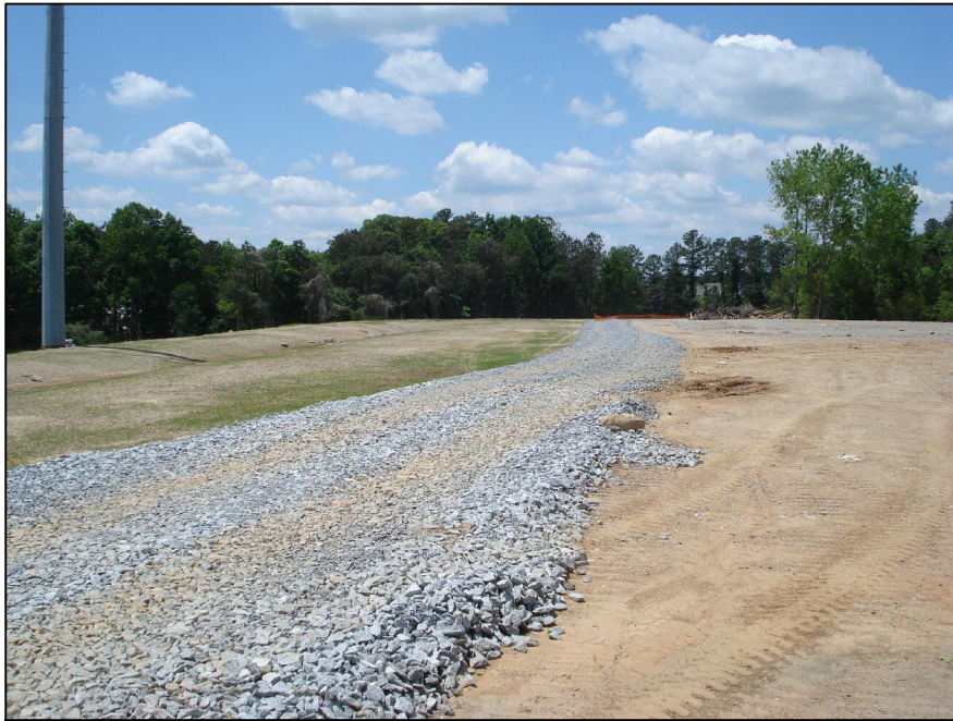
3-3 GRASSY AREAS RESEEDED ON DIKE
