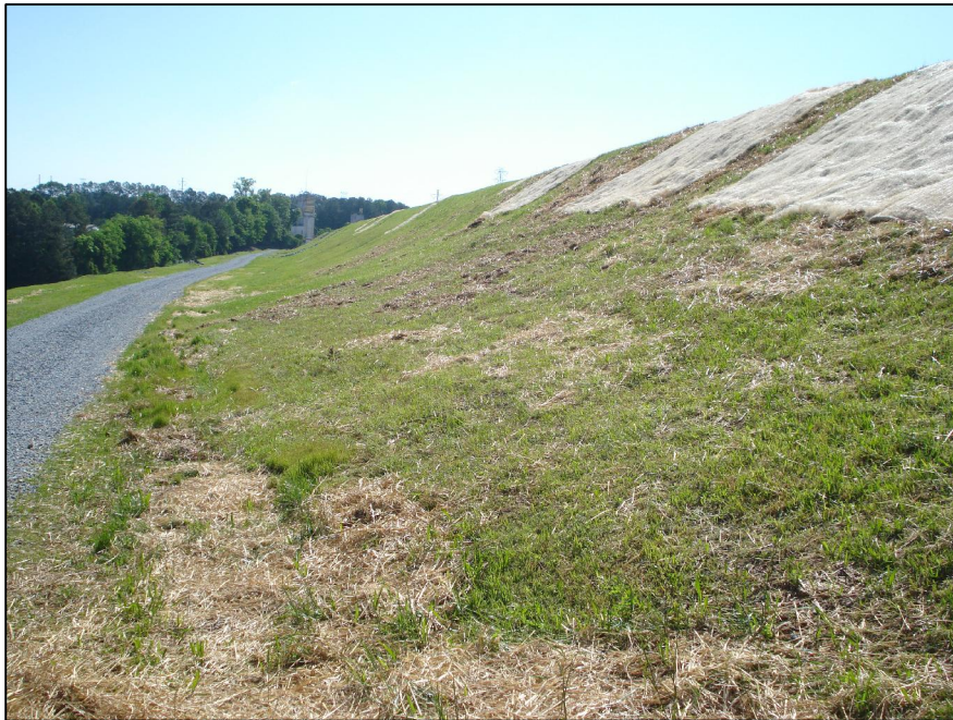
RESEEDED AREA ALONG WESTERN DOWNSTREAM TOE
