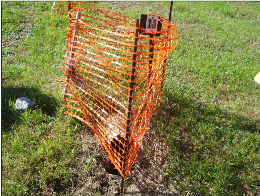
4-2 DRAIN NUMBER 15 (FLOWING) ALONG WESTERN DOWNSTREAM TOE
