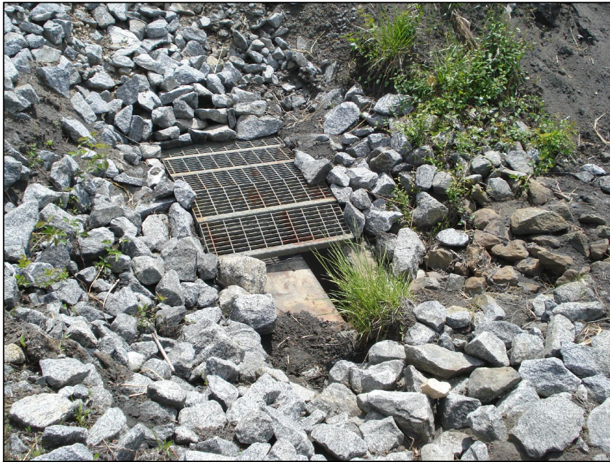
2-3 INLET AT EMERGENCY OUTLET PIPE
