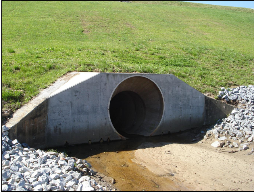
4-1 ENTRANCE TO DIVERSION PIPE
