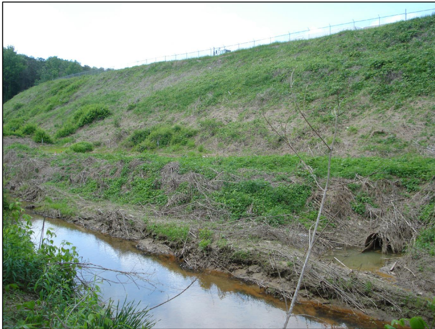
1-4 PRIMARY SPILLWAY OUTLET
