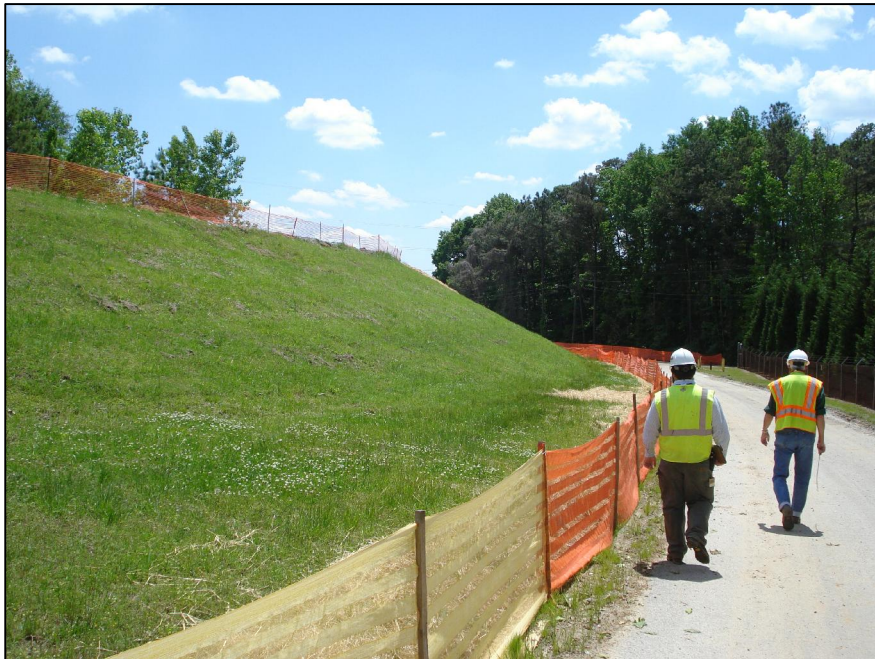
3-4 GENERAL SITE PHOTO
