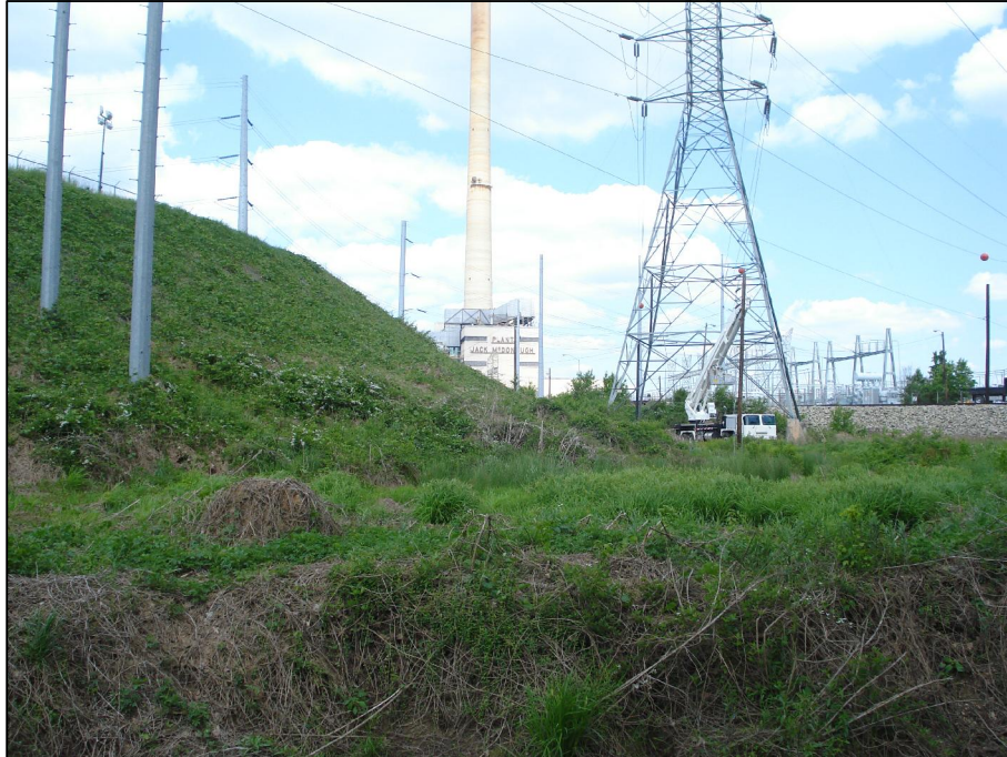
1-7 GENERAL SITE PHOTO
