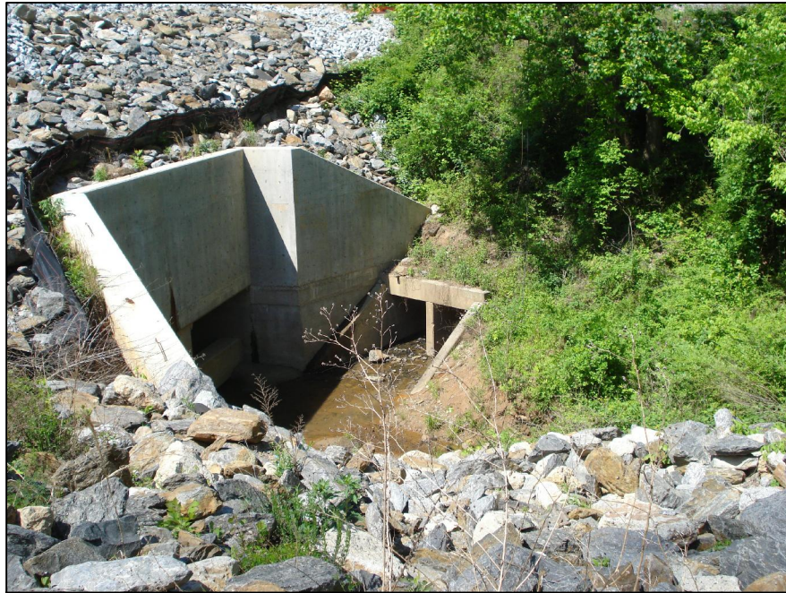
4-5 OUTLET FOR DIVERSION PIPE
