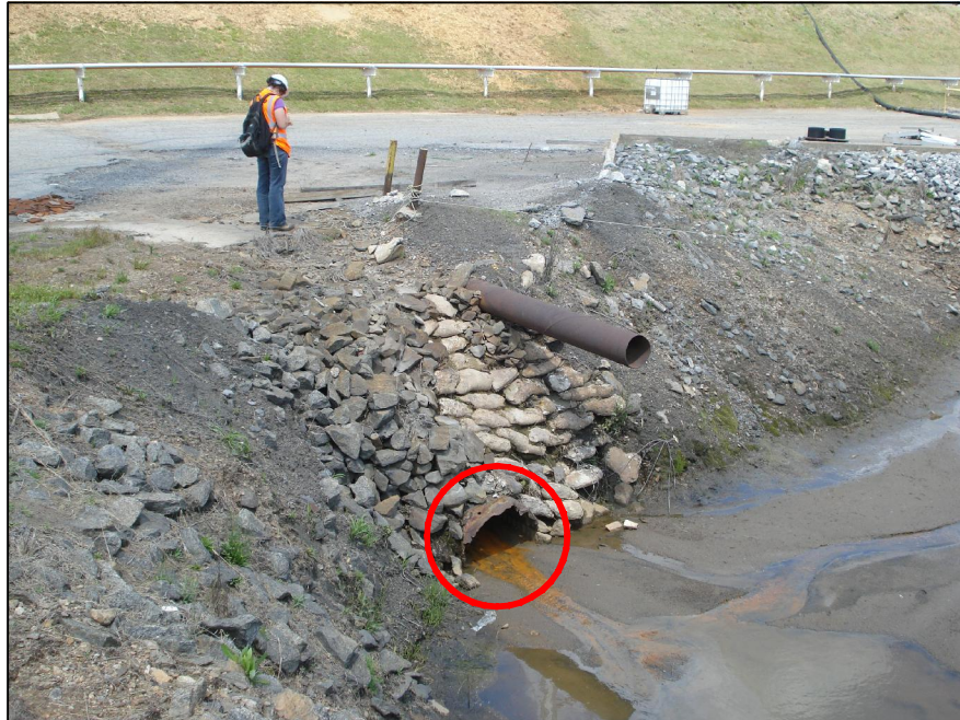
2-5 EMERGENCY OVERFLOW OUTLET
