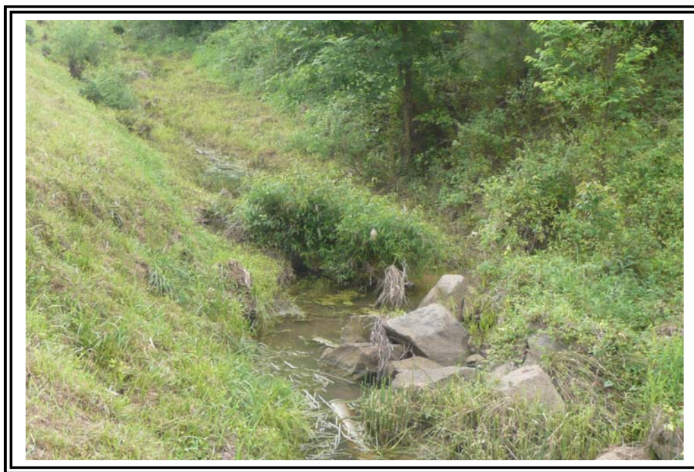
Perimeter ditch at south end of main dike, looking east. Another area of slough in natural cut slope has choked the channel and has reportedly remained unchanged in 6 to 10 years per Georgia Power Engineer responsible for inspections.
