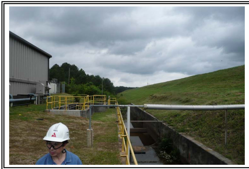
South end of main dike at NPDES Sampling flume, looking west. The majority of the slope shown is a natural cut slope, 5 to 10 foot high embankment constructed to blend into slope in this area.
