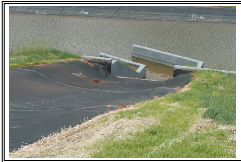
Emergency overflow and outlet sluice (via buried outlet pipe) from the gypsum pond into the drainage swale running to the reclaim pond.
