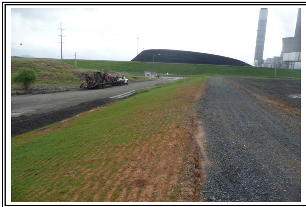
North embankment of wet ash ponds, looking east.
