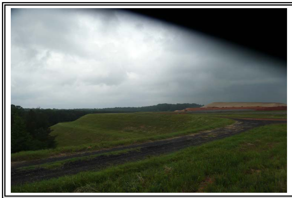
Embankment at the "Horseshoe" looking north. Note original embankment crest width was 15 feet. Dry stacked ash placed uniform to dam crest.
