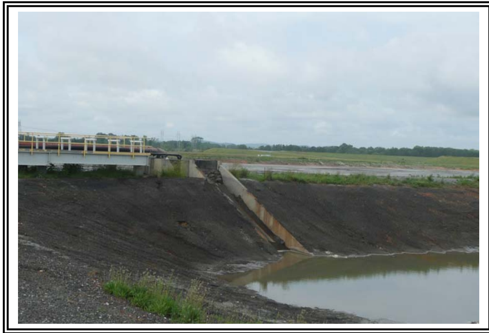
Sluiceway into the north wet ash pond.
