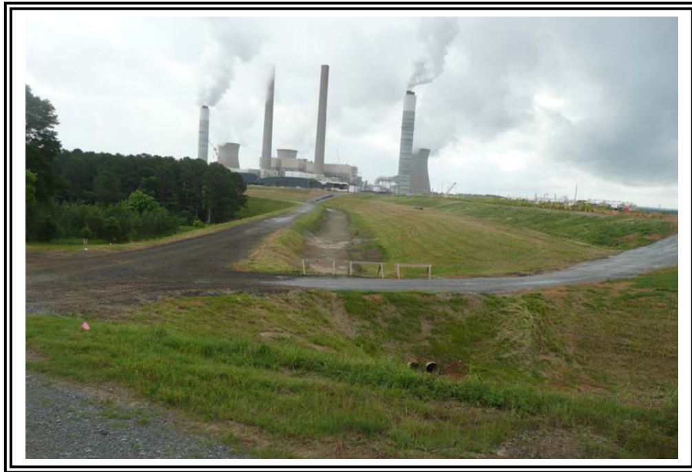
Overview of north dike, looking east.
