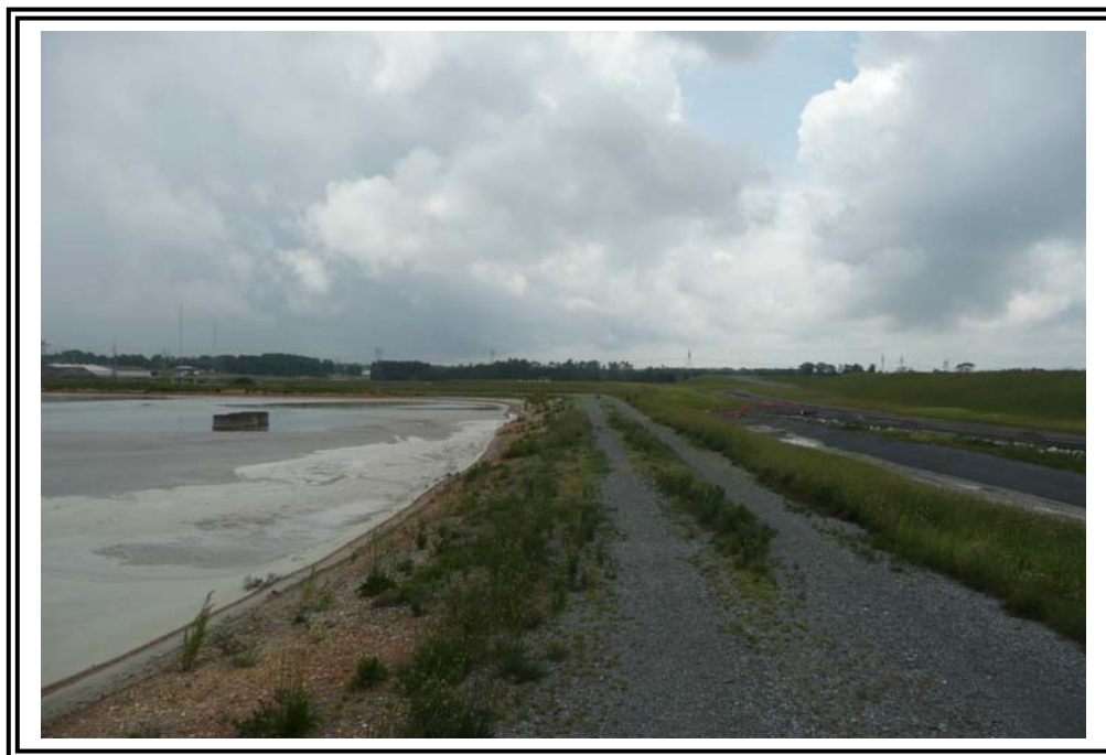
West embankment of south wet ash pond, looking south.
