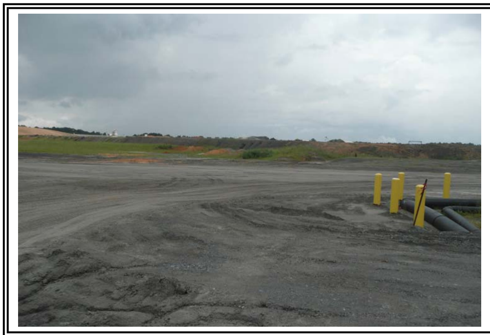
Within the main impoundment looking north toward the dry stack area.
