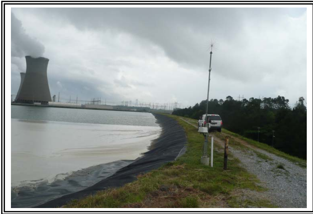
Reclaim Pond and south end of the embankment crest looking east. Note the Reclaim Pond is lined with and HDPE liner.
