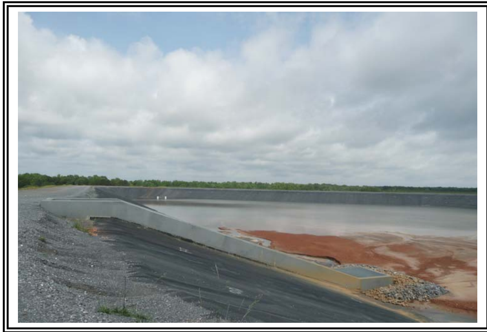
Lined gypsum pond.
