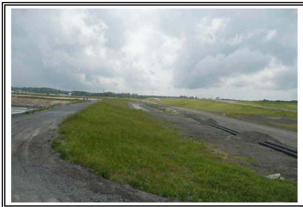
The west embankment of the wet ash ponds. Note short height and 3H:1V slope.
