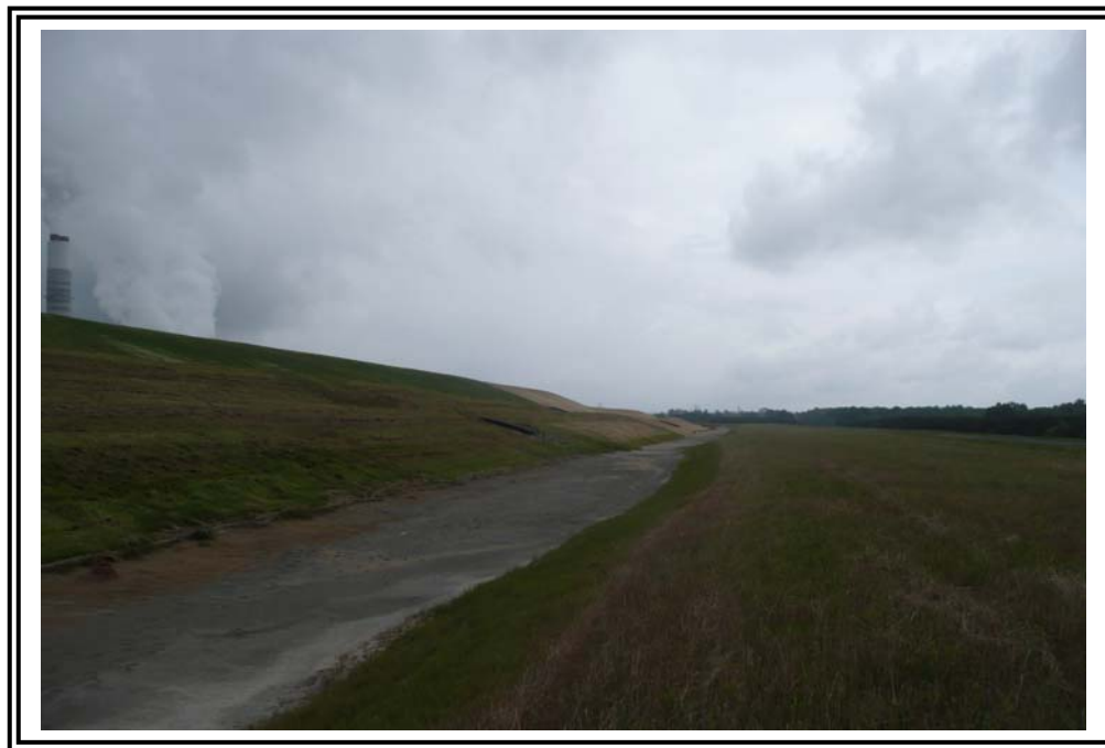
Main Embankment Crest looking south. Note dry ash stack area in the left of the photo, original embankment crest width 15 feet. Drainage swale is located between the dam and the dry stacked ash pile.
