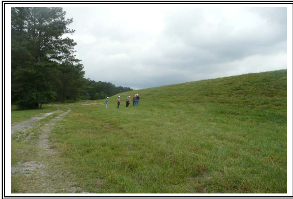
South end of the west portion of the Dike.
