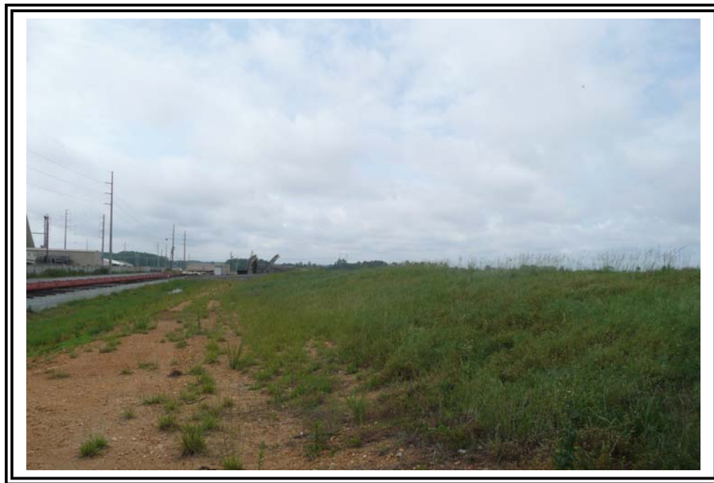
East slope of wet ash ponds looking south.
