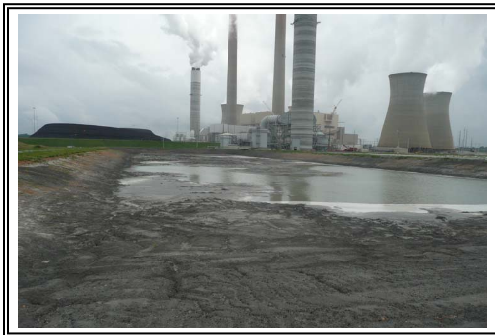
North wet ash pond looking east.
