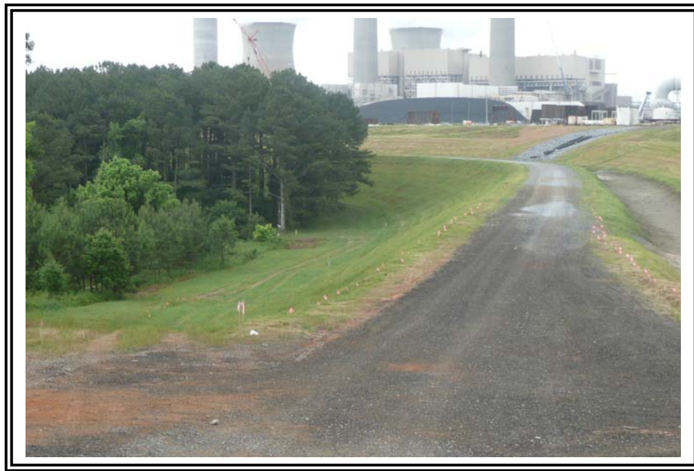
West end of north dike, looking east.
