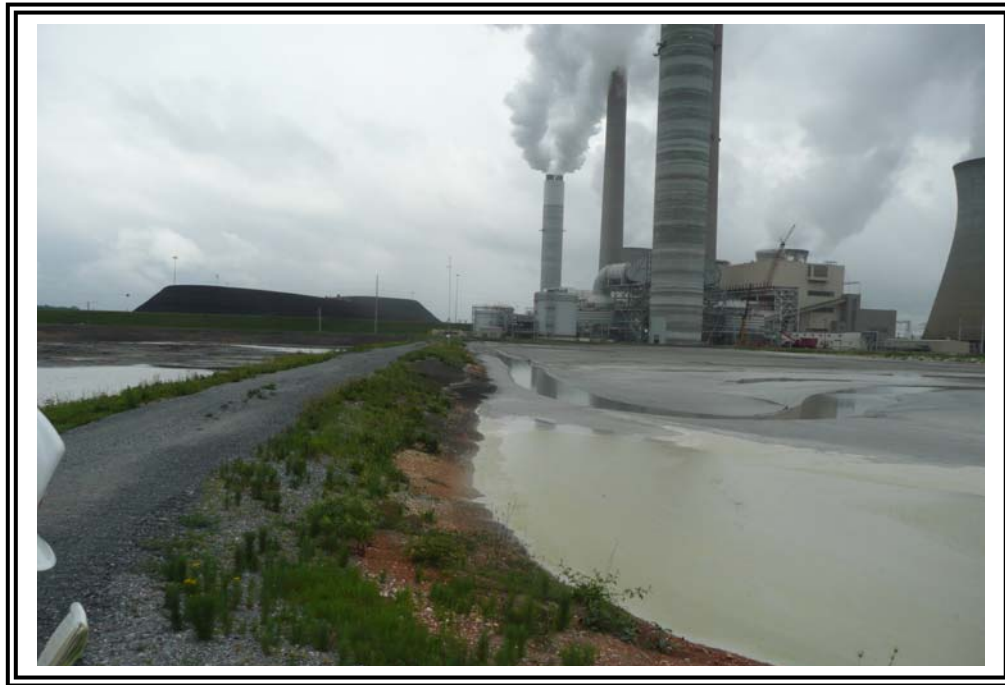
Separator dike between two wet ash ponds.
