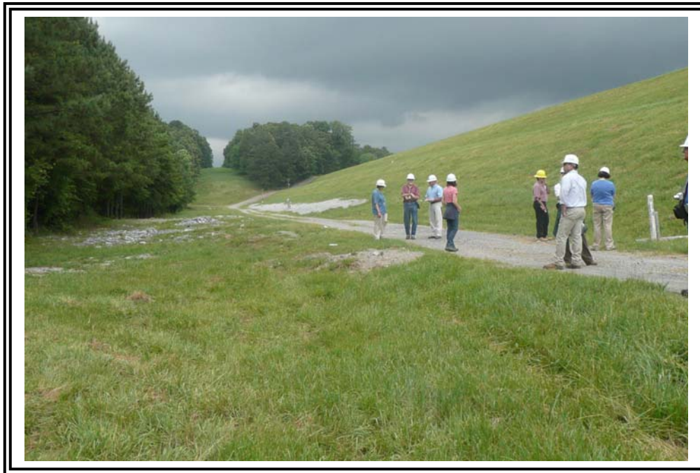
Embankment at the “Horseshoe” (looking south). Note the gravel at the toe which was placed during the grouting program to seal karst features below the embankment.
