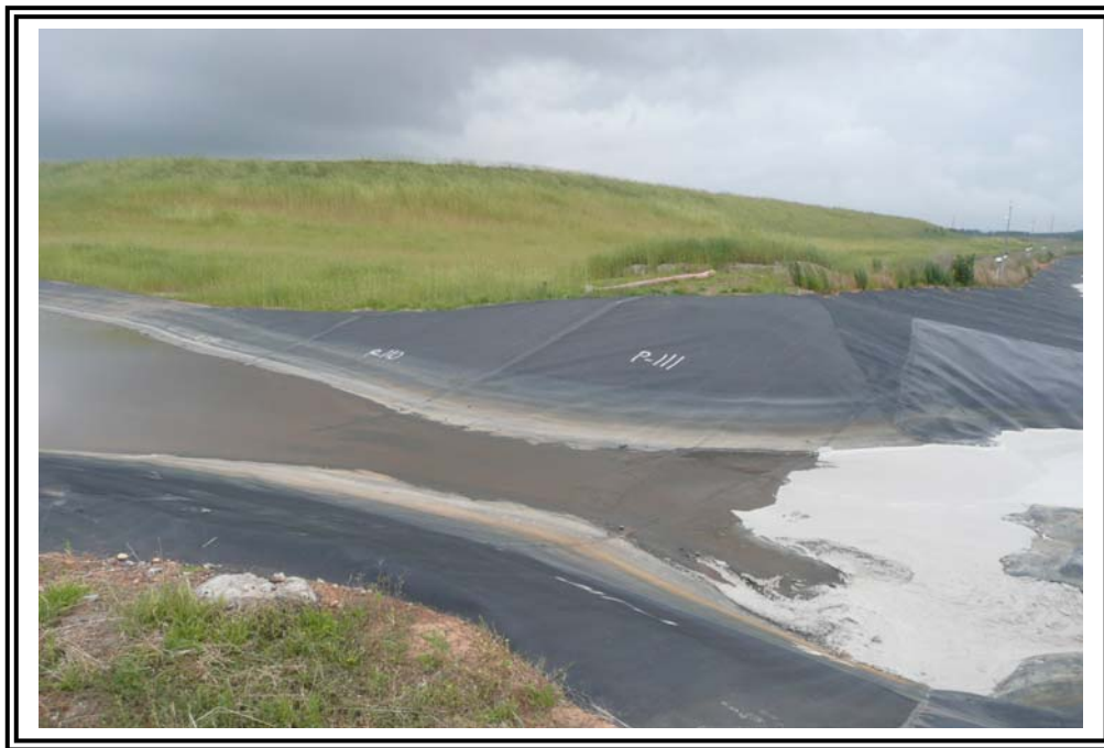
Drainage Swale noted in Photos 15, 16, and 17 discharges into the Reclaim Pond. Note the drainage swale is also HDPE lined. Behind the swale in this photo is one of two gypsum ponds.
