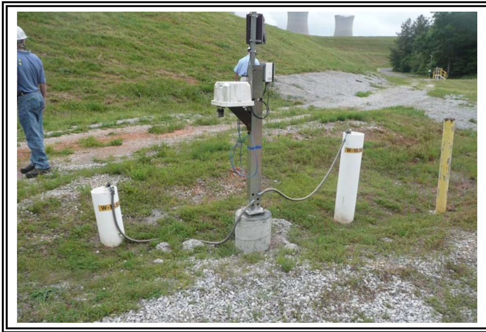
Embankment at the “Horseshoe” (looking south). Note the gravel at the toe which was placed during the grouting program to seal karst features below the embankment.
