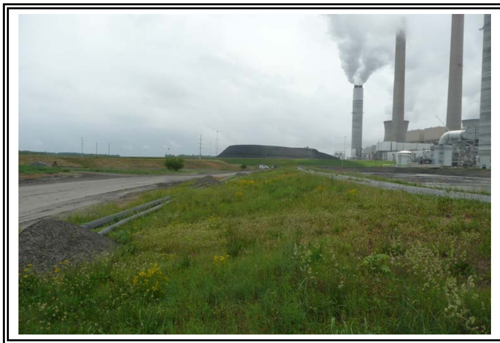
North embankment of wet ash ponds.
