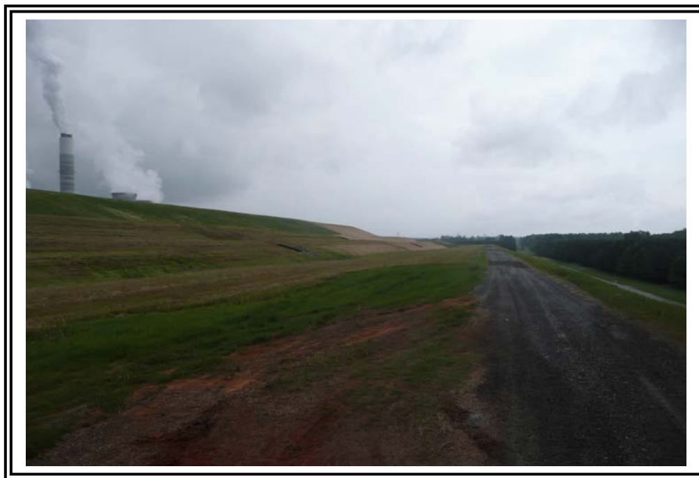
Main Embankment Crest looking south. Note dry ash stack area in the left of the photo, original embankment crest width 15 feet. Drainage swale is located between the dam and the dry stacked ash pile.
