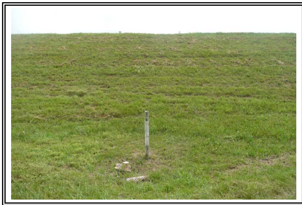
South end of the west portion of the Dike. Toe drain outlets are marked with concrete posts. Toe drain outlets located about every 200 feet. No flow noticed, and Georgia Power indicates they have not seen water flowing in the toe drain.
