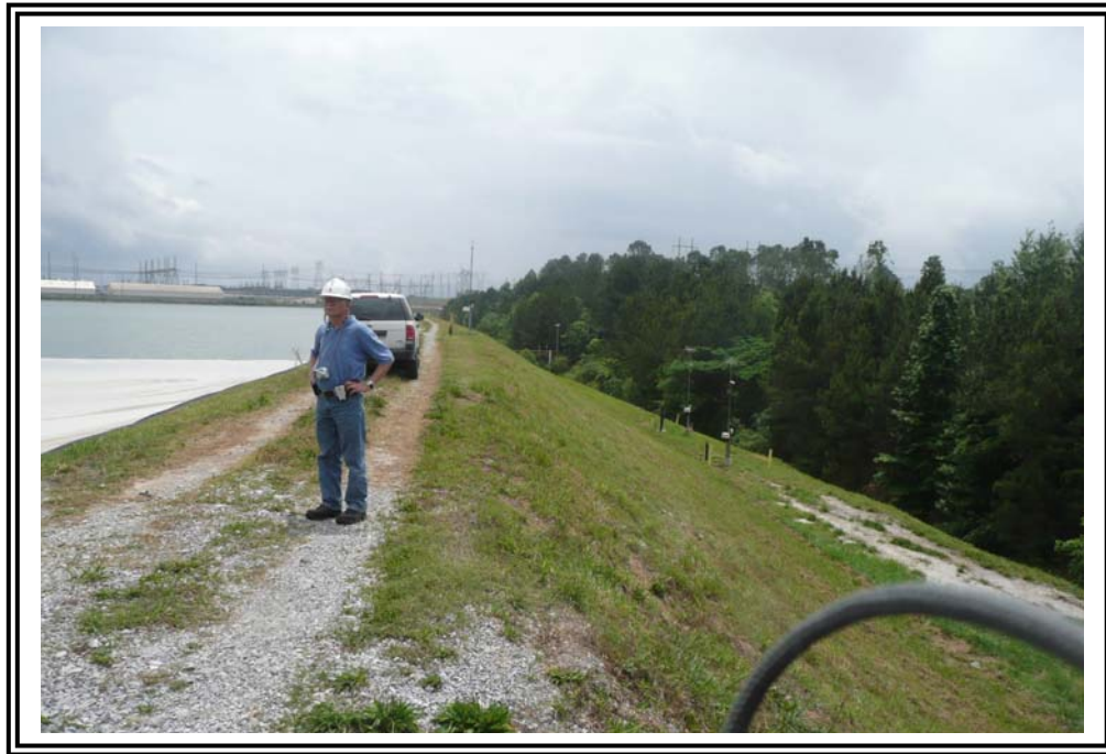
Crest of south end of main embankment looking east.
