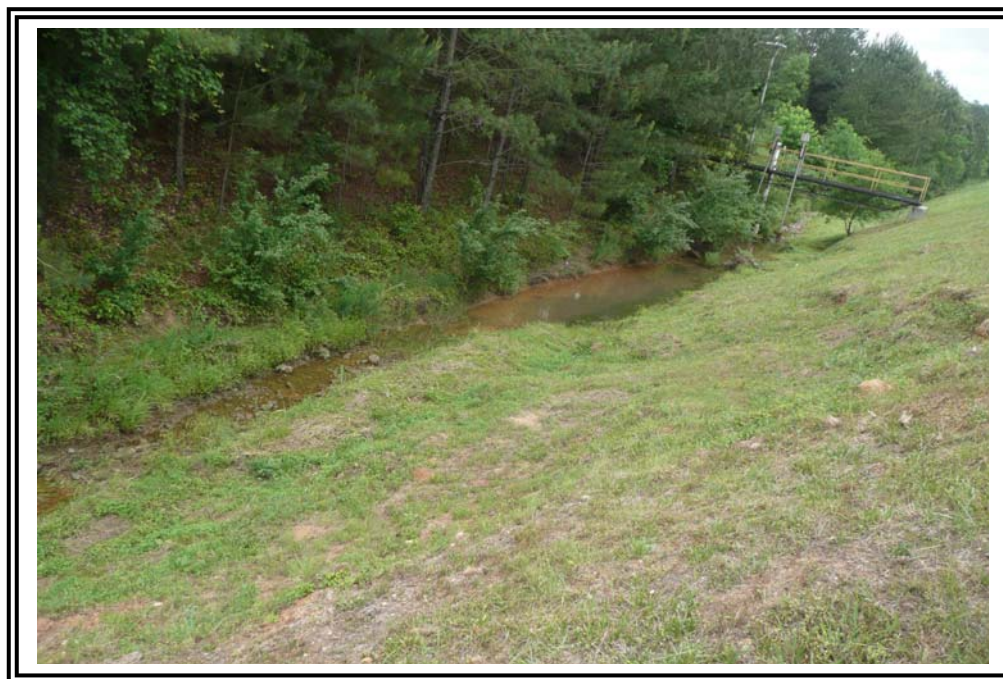
Continuing west on south end of main dike, another slough area in the natural cut slope, reportedly unchanged in 6 to 10 years per Georgia Power engineer responsible for inspections.
