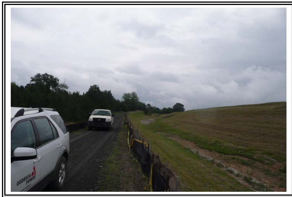
Upstream side of North Dike looking east. Dry Stack ash piles in the right of the photo. Drainage swale in this area is unlined, but lining is planned for the 2009 construction season.
