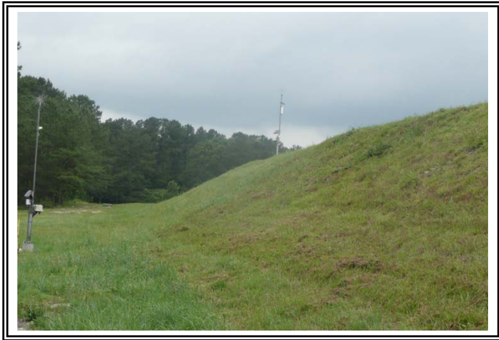
South portion of the embankment near the end of the reclaimed water portion of the impoundment (looking west). Reclaim Pond is lined. Note set up for remote monitoring of piezometers (not operational as of our visit).
