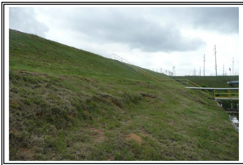
South end of main dike at NPDES sampling flume, looking east. Scarp in natural cut slope, reportedly unchanged in 6 to 10 years per Georgia Power Engineer responsible for inspections.
