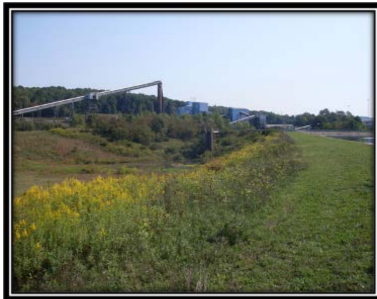
Figure 5.3.3-3 Outside slope of embankment dam on north side of Thermal Pond, which forms south inside slope of retired basin on the north side of the Thermal Pond– viewed east.
