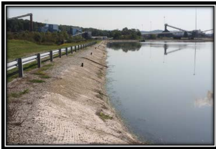
Figure 5.3.2-1 Typical upstream (inside) slope of Thermal Pond – north side viewed east.
