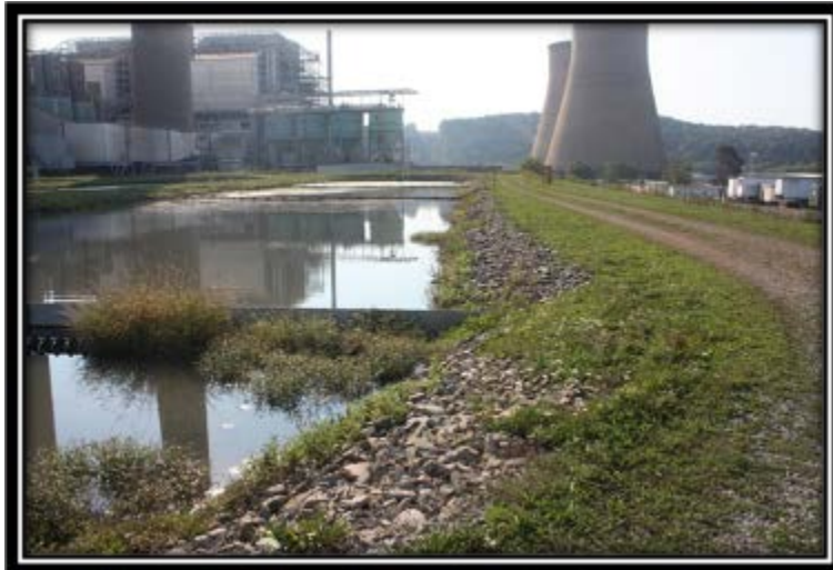
Figure 5.2.1-2 Crest and inside slope of Ash Filter Ponds – southwest side viewed southeast (highest embankment, next to Pond A).
