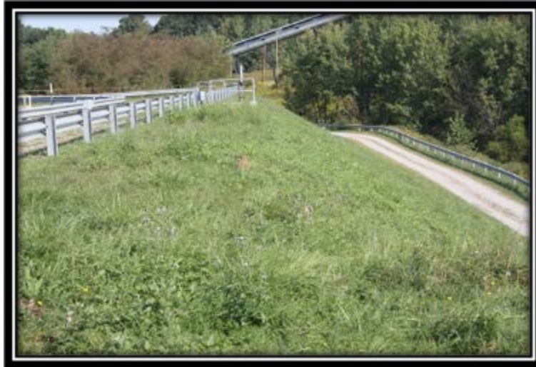
Figure 5.3.3-2 Outside slope above access road berm – viewed north.
