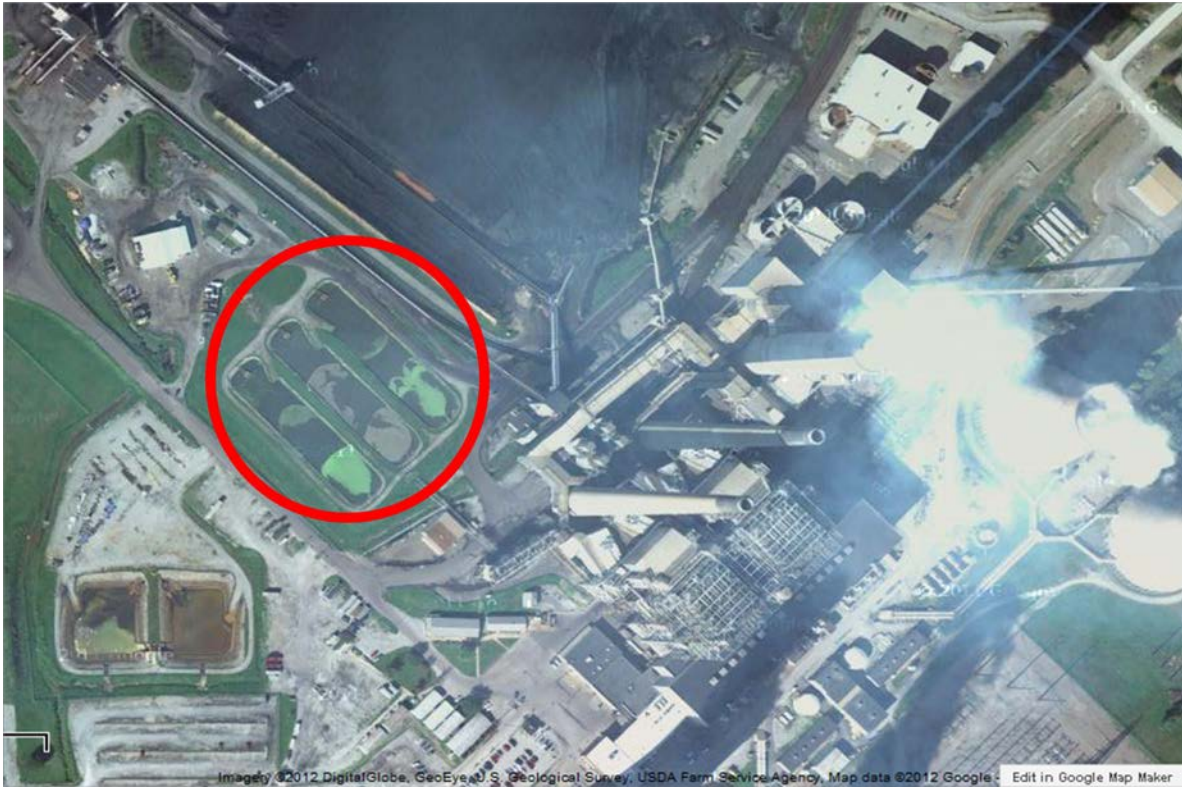
Figure 2.1-2: CCR Impoundment (Ash Filter Ponds) at Keystone Generating Plant
