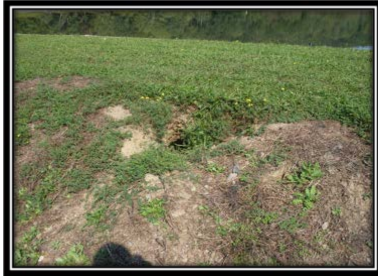
Figure 5.3.3-4 One of several animal holes observed at top of outside slope of low embankment on south side of Thermal Pond – viewed north.
