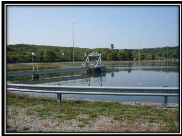
Figure 5.4.2-1 Thermal Pond outlet structure – viewed southwest from main embankment dam on east side of Thermal Pond.
