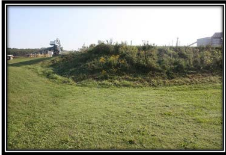
Figure 5.2.4-1 Groin area at the west corner of the Ash Filter Ponds
