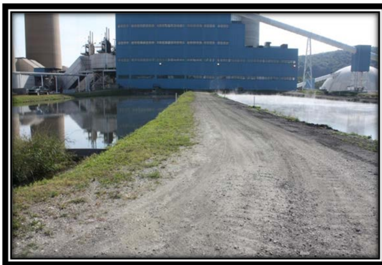
Figure 5.2.2-1 Inside slopes of the Ash Pond and interior dikes between the cells.
