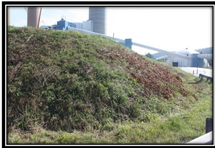
Figure 5.2.4-2 Groin area of the Ash Filter Ponds (southwest corner)
