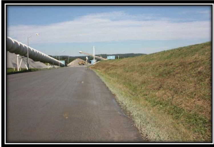
Figure 5.2.3-1 Toe of the downstream dike (south side of Pond).
