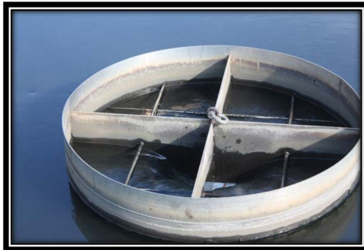
Figure 5.4.1-2 Outlet structure for Desilting Basin.
