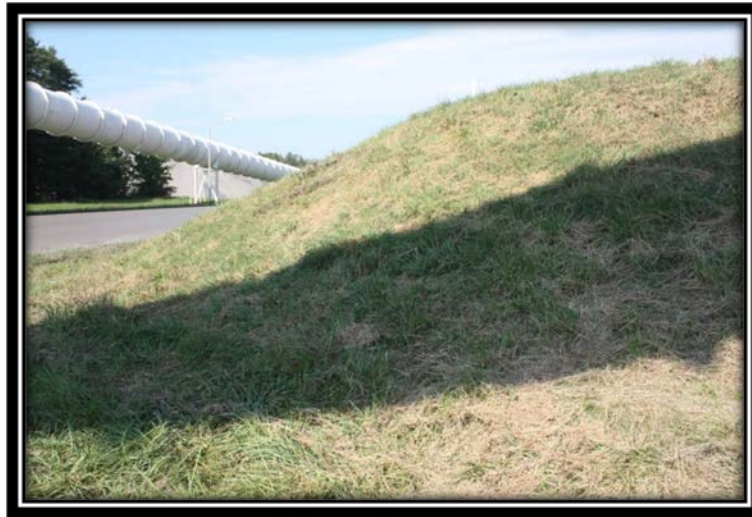
Figure 5.2.4-1 Groin area of the Ash Filter Ponds (southeast corner)
