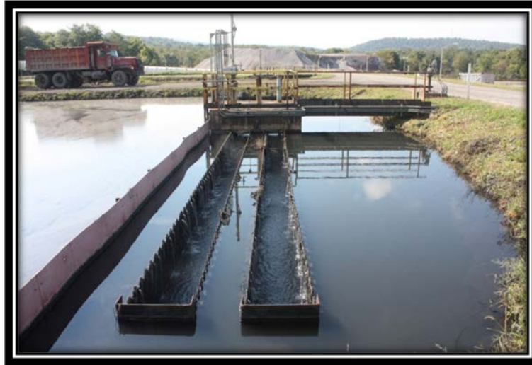
Figure 5.4.1-1 Typical outlet structure for Ash Filter Ponds.
