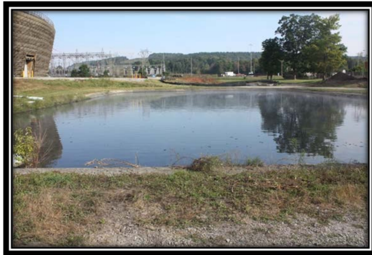
Figure 5.3.1-1 Crest and embankments of the Desilting Basin.
