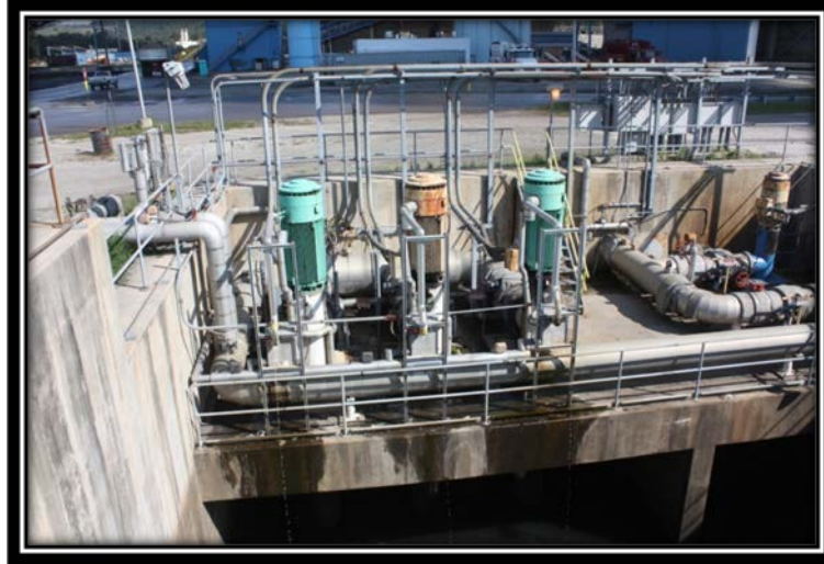
Figure 5.4.2-3 Recycling Pumps.
