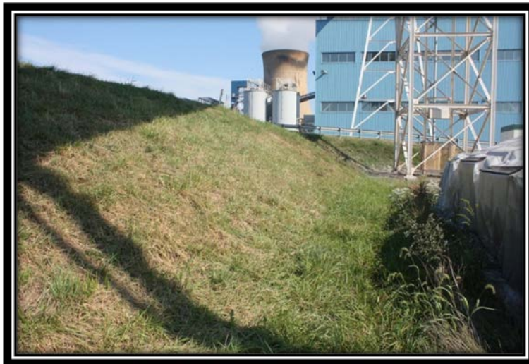
Figure 5.2.3-2 Toe of the east side dike of Ash Filter Ponds).
