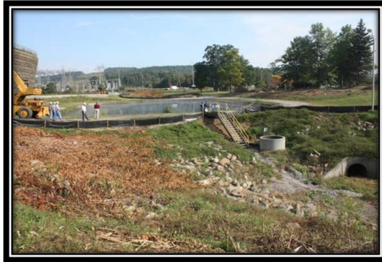
Figure 5.3.3-1 Desilting Basin Outside slope.
