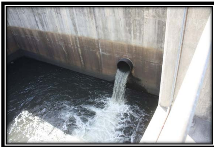
Figure 5.4.2-1 Outlet structure from the Ash Filter Ponds to the recycling structure.
