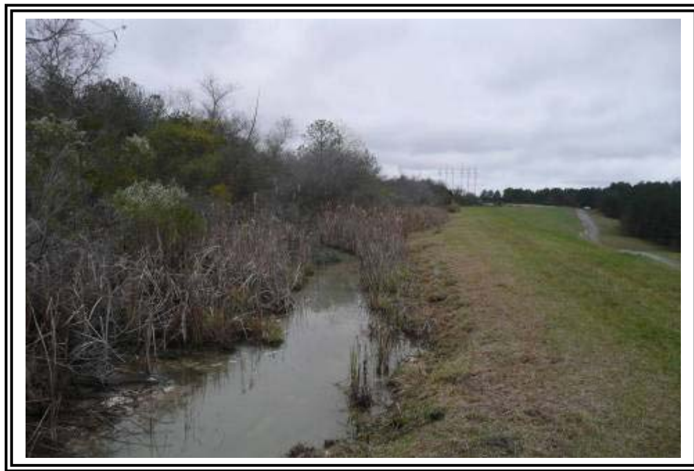
Ash Pond D, north edge of dike facing south east. Note widened crest of dike.
