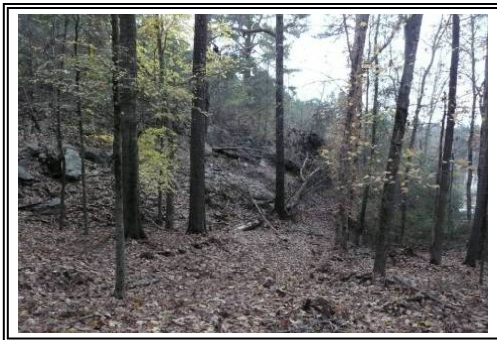
Ash Pond B, central portion of dike along the toe facing east. Heavy vegetative growth present and large boulders present throughout. Lake Sinclair shown frame right.
