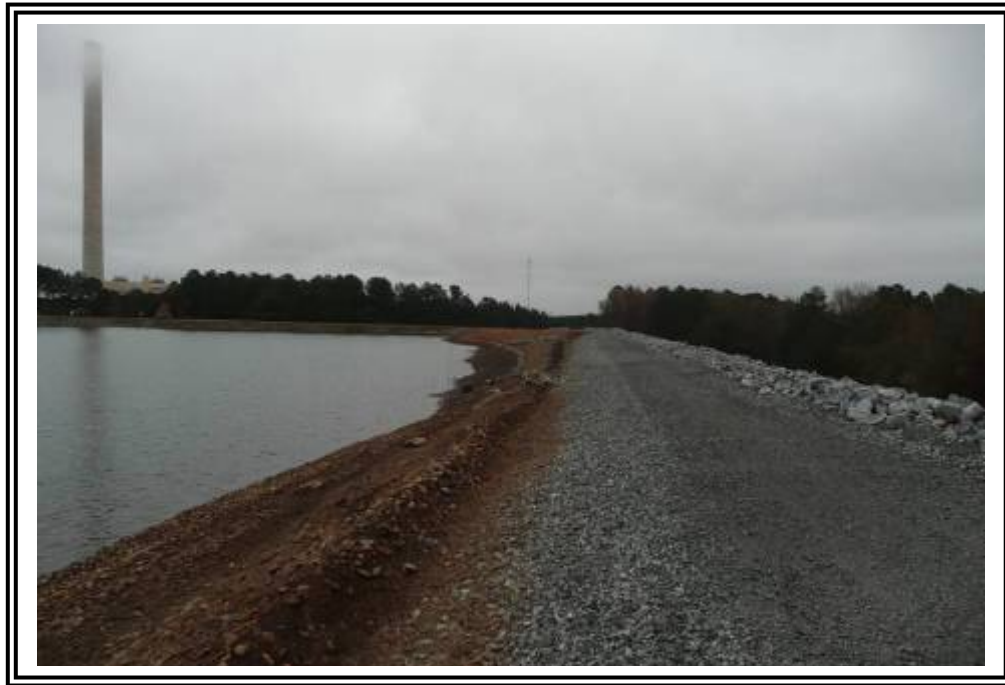
Ash Pond C, west end of south dike facing east.
