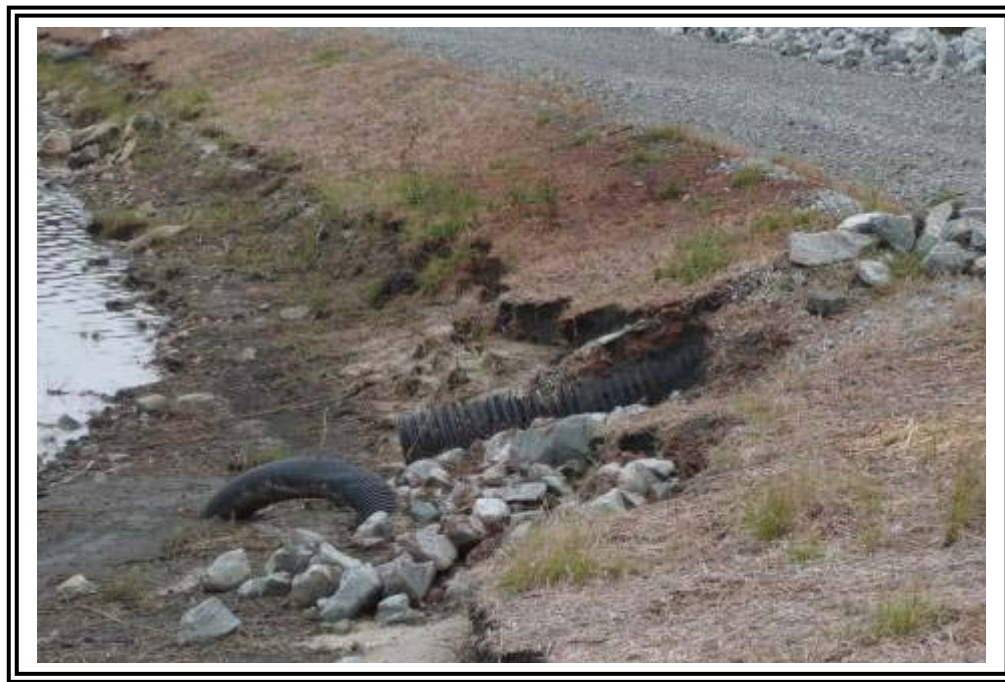
Upstream side of Ash Pond C west end of south dike facing east. Crest run-off drain shown.
