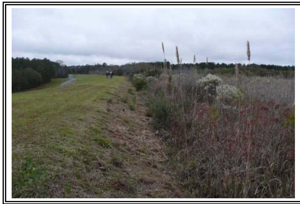
Ash Pond D, south end of dike facing north. Upstream slope and vegetation in the pond shown frame right.
