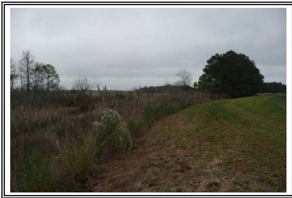
Ash Pond C, upstream dike edge shown at north portion of the west dike, facing south.
