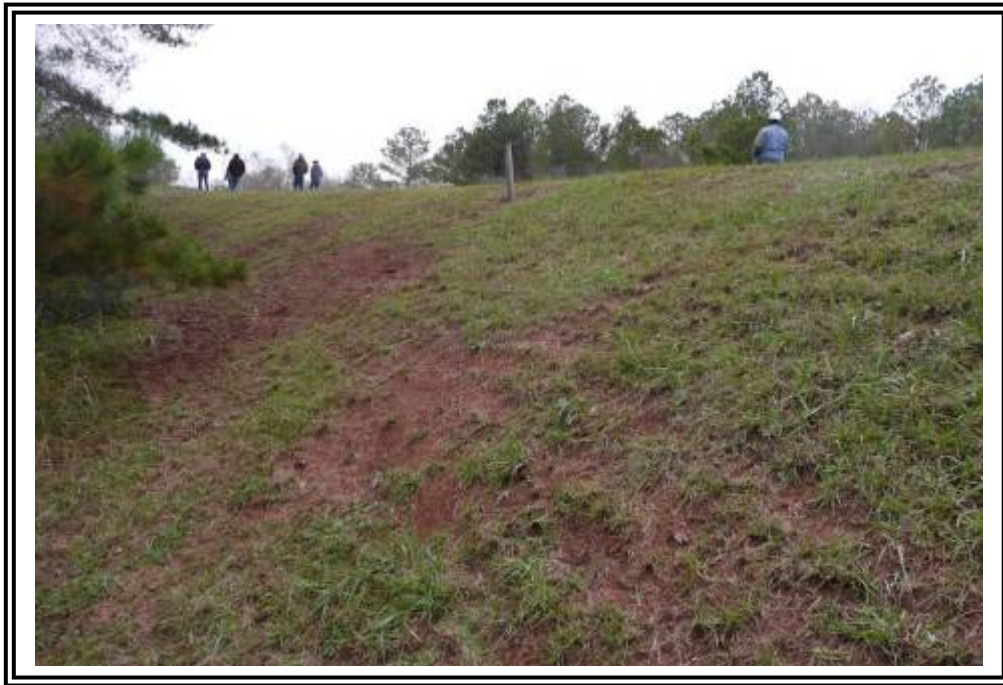
Sparse grass cover on north central portion of Ash Pond C west dike toe, facing north.
