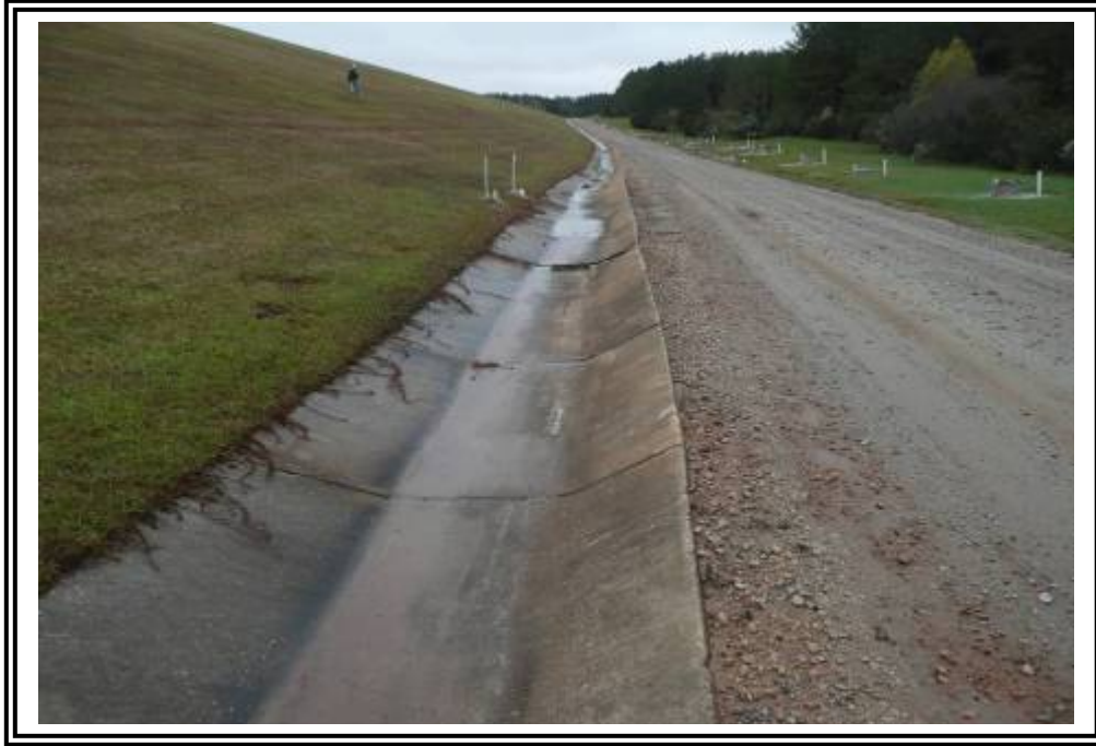
Ash Pond E, concrete lined channel drain at the base of the dike (upper channel).
