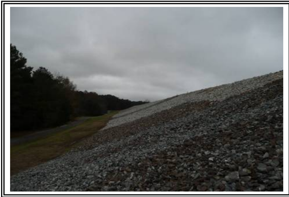
Ash Pond C, east end of south dike facing west. Downstream slope shown with rip-rap facing.
