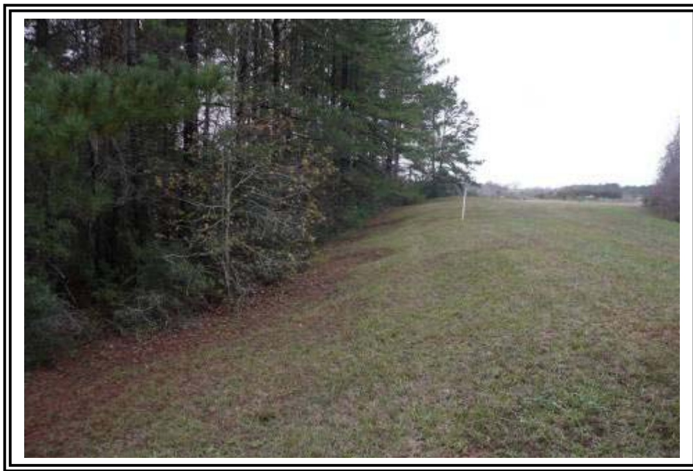
Ash Pond C, downstream edge of west dike at north end of dike, facing north.
