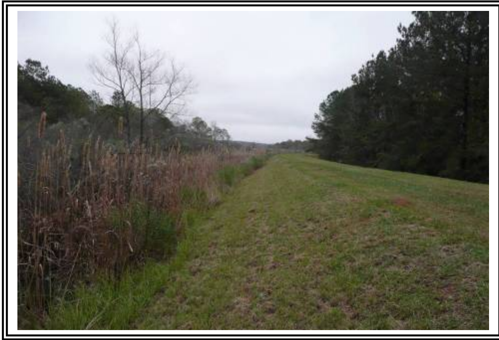
Ash Pond C, north end of west dike interior, facing south. Interior edge of dike shown frame left with vegetation present. Exterior edge of dike shown frame right with heavy vegetative cover present past dike toe.
