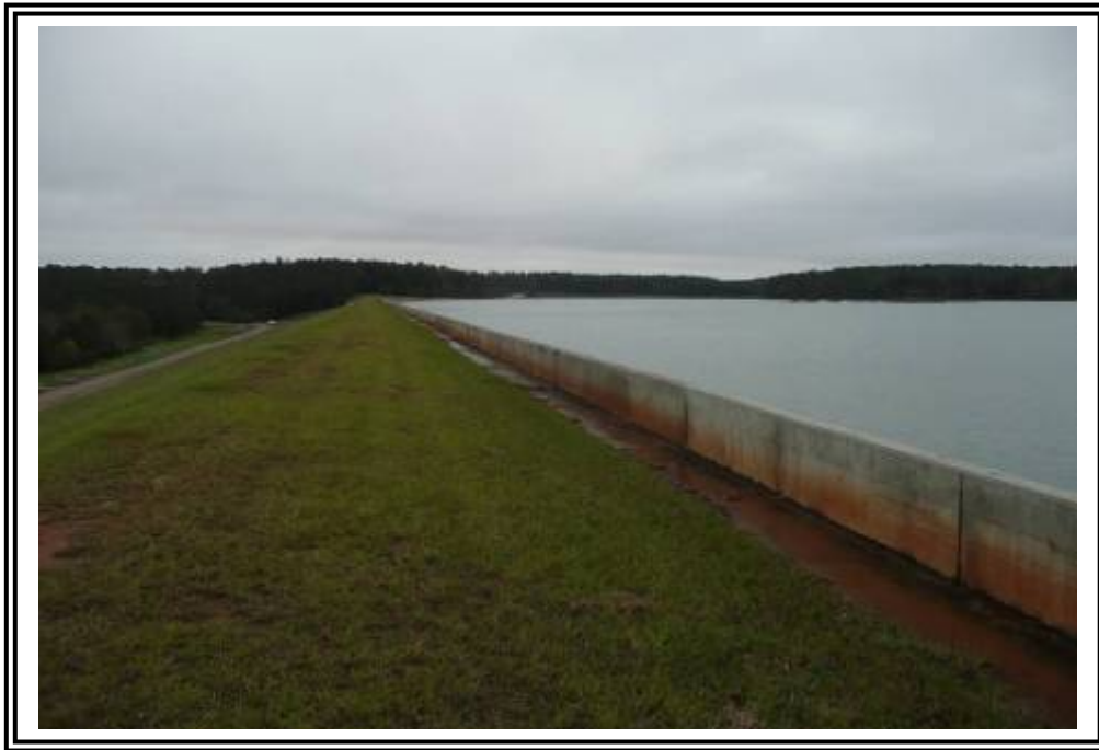
Northern end of Ash Pond E dike crest, facing south.
