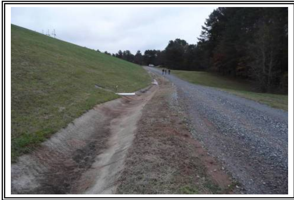
Ash Pond D, central portion of dike along toe facing south east. Concrete lined channel drain along toe and finger drains shown frame left.
