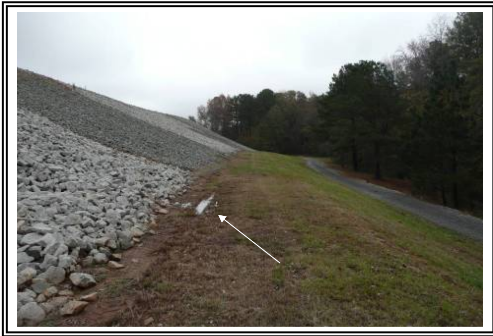
Ash Pond C, central portion of south dike along toe facing east. Water due to rainfall shown frame left.
