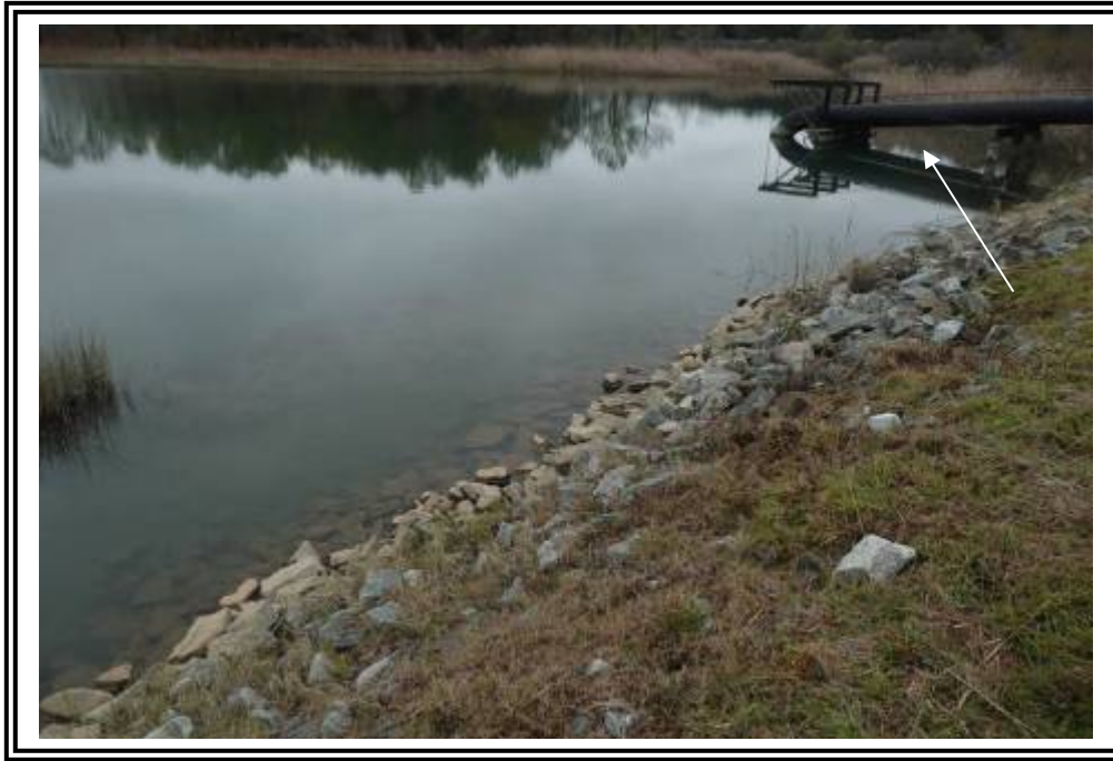
South central portion of Ash Pond C east dike, upstream slope shown with rip-rap. Re-cycle water system intake shown frame right.
