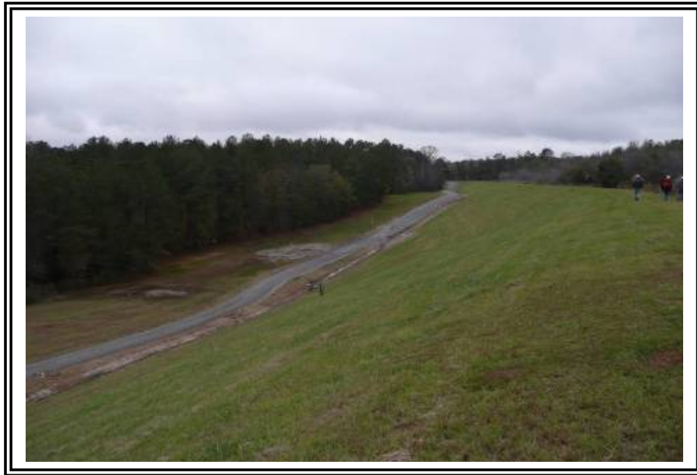
Ash Pond D, central portion facing north east.
