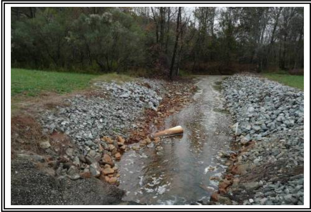
Ash Pond E, receiving stream for drainage from the blanket drain system.
