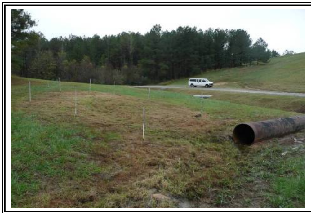
Ash Pond E, "soft spot" located south of emergency overflow drain (1 of 3 observed near Ash Pond E). This area has been monitored for 9 years by Georgia Power with no additional expansion observed. Perimeter stakes have been placed to aid in monitoring.
