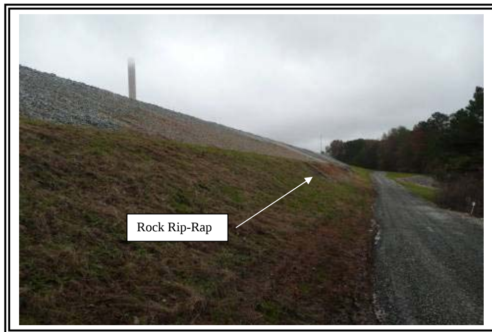
Ash Pond C, western central portion of south dike facing east. Toe re-faced utilizing rock rip-rap.
