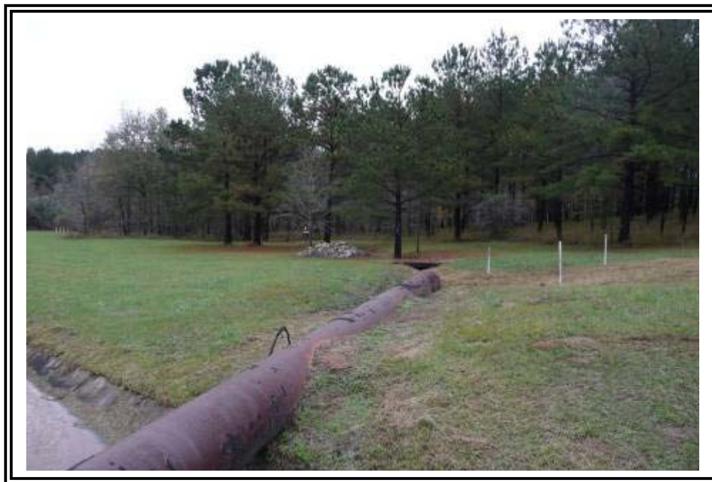
Ash Pond E abandoned overflow drain located along southern portion of the dike. The drain pipe is constructed of welded steel.
