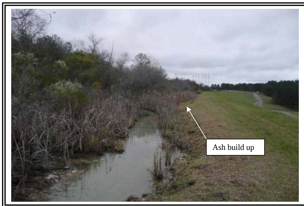
Ash Pond D, north edge of dike facing south east. Note widened crest of dike. Crest widening due to build up of ash per Georgia Power personnel.
