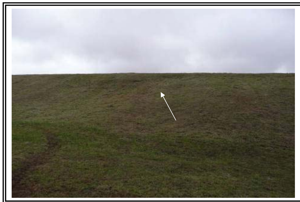
Downstream slope of Ash Pond C east dike near the south end showing variations in elevation.
