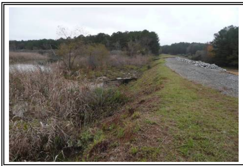
Central portion of Ash Pond C east dike facing north. Interior pond edge shown with thick and tall vegetative growth.
