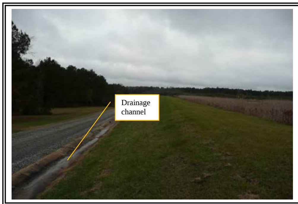
Ash Pond D, south edge of dike facing north. Concrete lined drainage channel shown frame left.
