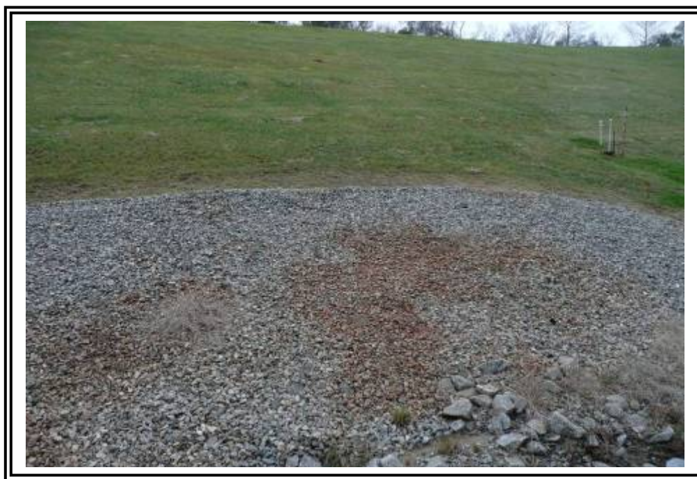
Ash Pond D, central portion of dike at edge of toe. Seepage remediation area shown.
