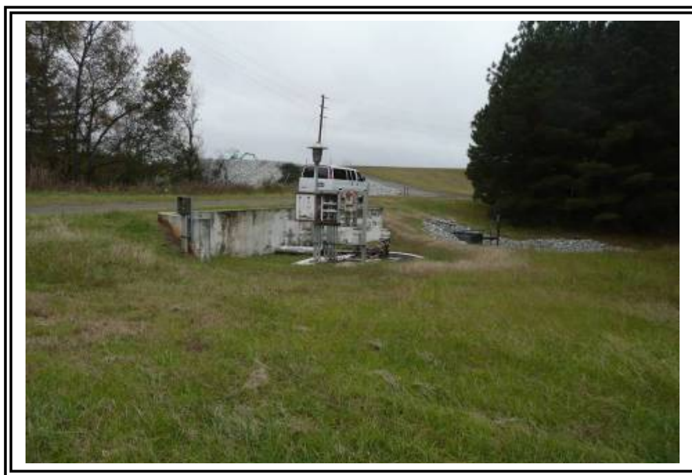
Ash Pond B, west end of dike. Emergency spillway (black pipe in background) and abandoned primary discharge facility shown.
