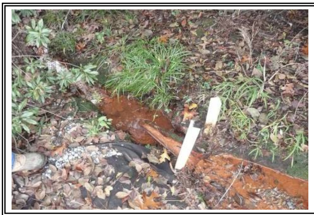
Ash Pond C, west end of south dike. Seepage weir shown.
