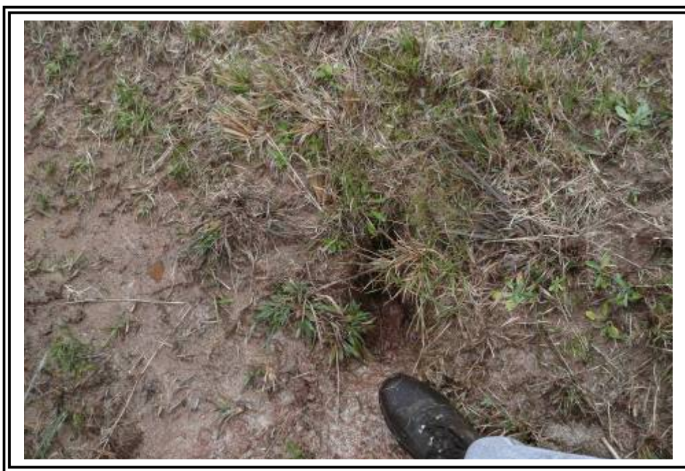
Ash Pond C, north portion of west dike, rodent burrow observed on upstream side of dike.
