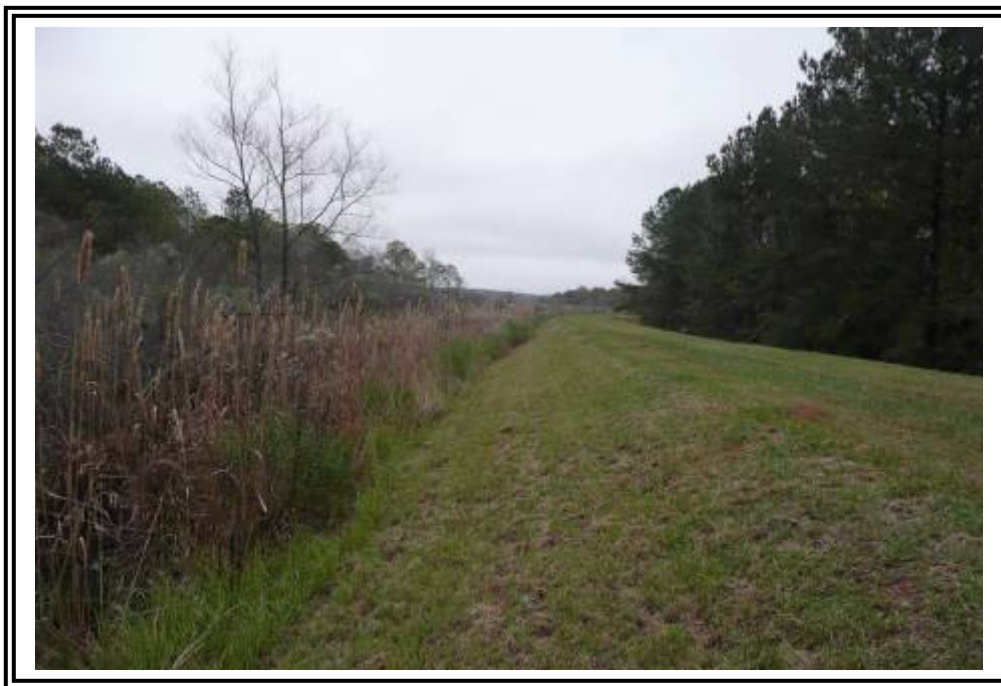
Ash Pond C, north end of west dike interior, facing south. Interior edge of dike shown frame left with vegetation present. Exterior edge of dike shown frame right with heavy vegetative cover present.
