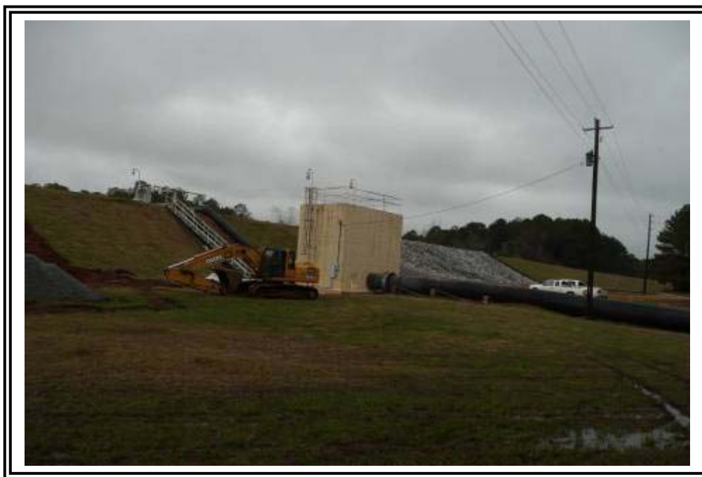
Ash Pond C, south central portion of east dike. Recycle water system shown. This system discharges recycle water to Ash Pond B.
