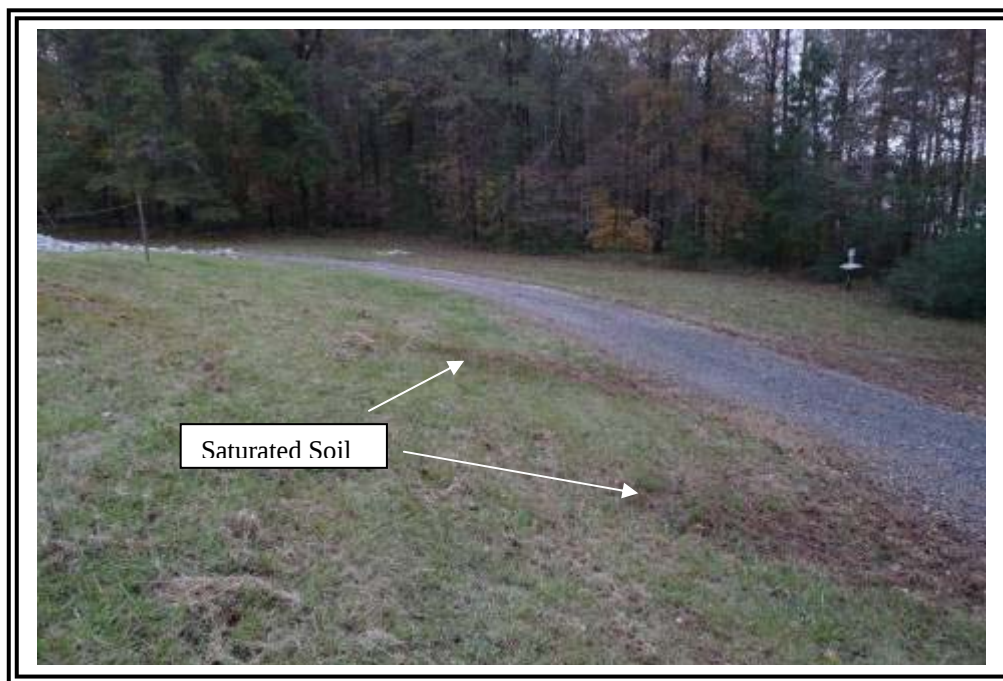
Ash Pond C, east end of south dike at the toe, facing east. Two saturated areas shown (several located in this area). Saturated areas possibly due to buried drains.
