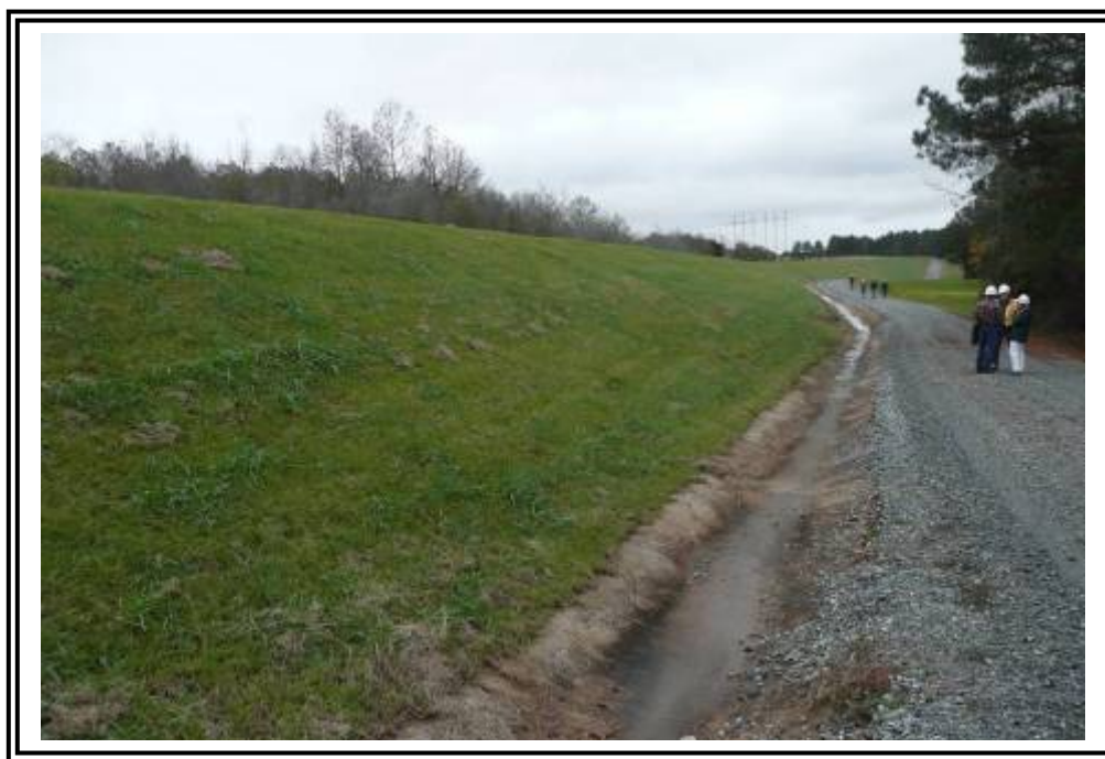
Ash Pond D, north end of dike at edge of toe facing southeast showing concrete lined drainage channel along toe of dike.
