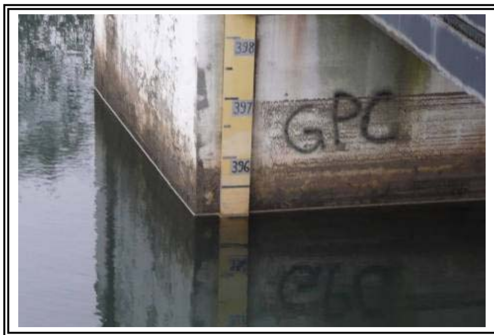
Ash Pond C water level indicated by the gauge at the historic discharge facility (395.0').
