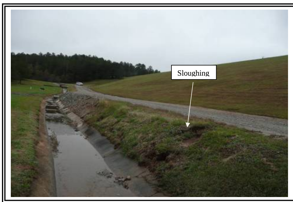
Ash Pond E, sloughing observed along west edge concrete line channel at the base of the toe, central portion of the dike.
