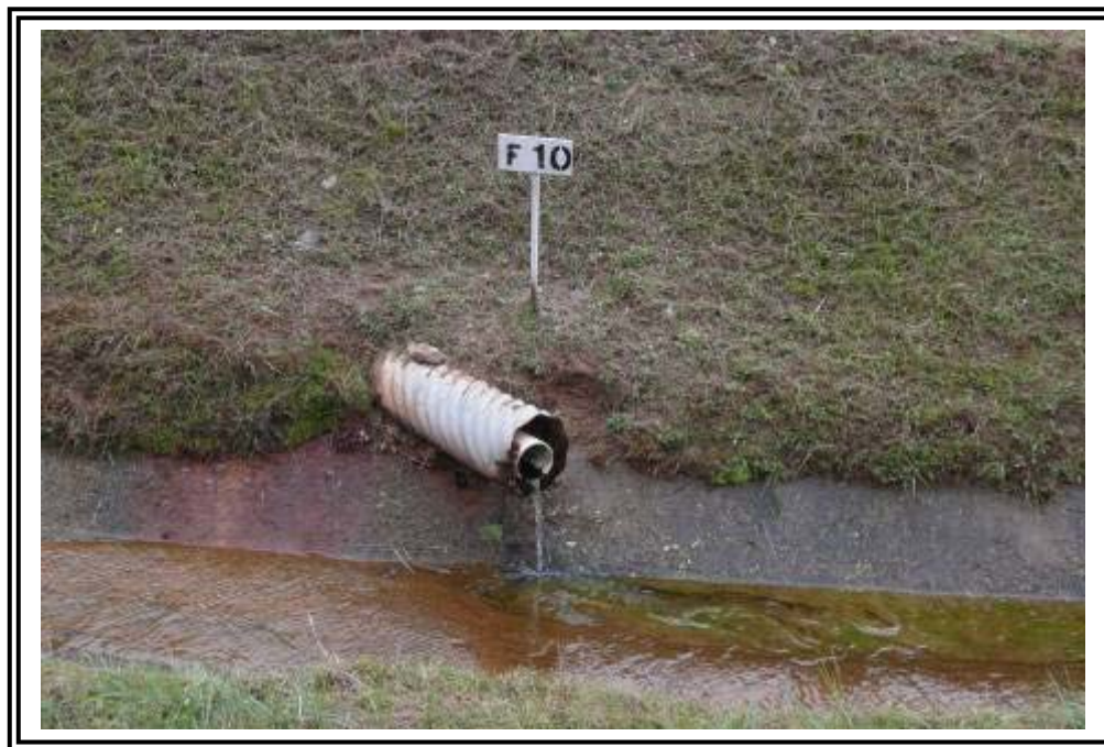
Ash Pond E, "soft spot" located south of emergency overflow drain (1 of 3 observed near Ash Pond E). This area has been monitored for 9 years by Georgia Power with no additional expansion observed. Perimeter stakes have been placed to aid in monitoring.
