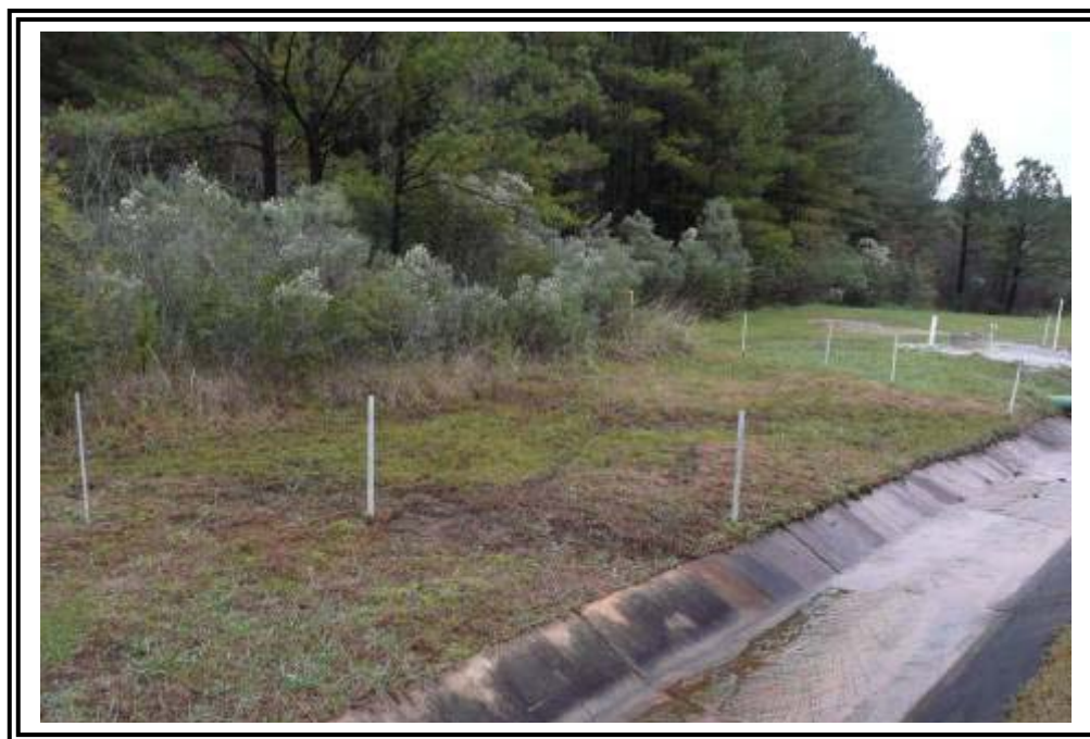
Ash Pond E, 3 rd observed "soft spot" located east of finger drain #5. Perimeter stakes installed for all soft spots in effort to monitor expansion. No observed expansion for any of the 3 soft spots in at least 9 years, as indicated by Georgia Power.
