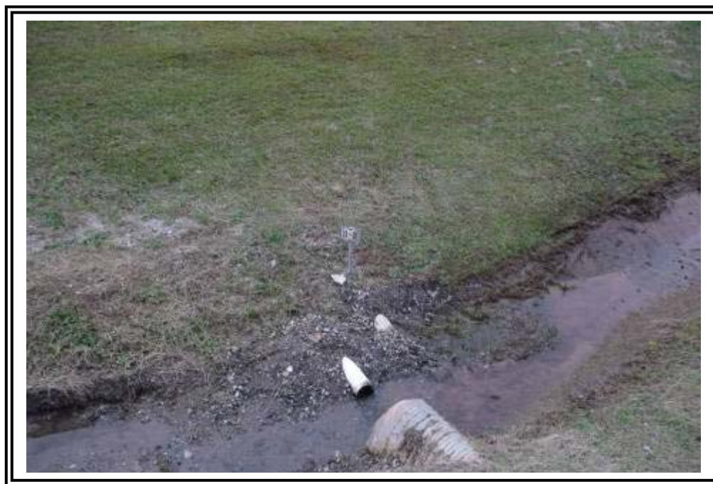
Ash Pond D finger drain D-3. Georgia Power personnel indicated that this area was previously remediated and the concrete lined channel was inadvertently razed during remediation.
