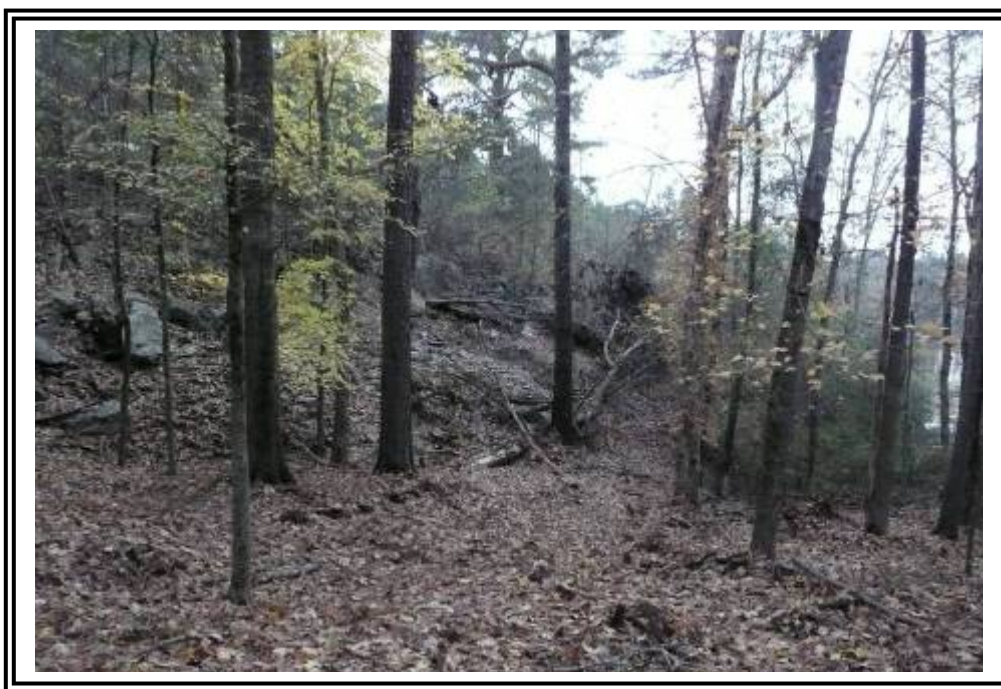
Ash Pond B, central portion of dike along the toe facing east. Heavy vegetative growth present and large boulders present throughout. Lake Sinclair shown frame right.
