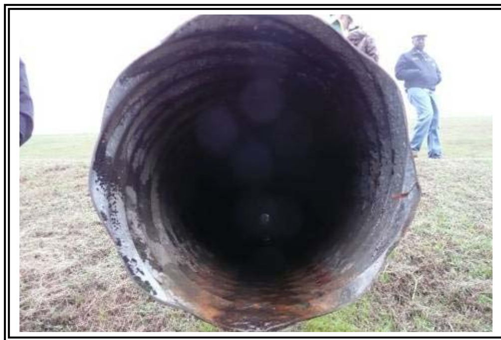
Corrugated metal drain pipe located north of Ash Pond E finger drain #11. Light can be seen at the western most end of the drain pipe, indicating a clear drainage channel from upper channel drain to lower channel drain.
