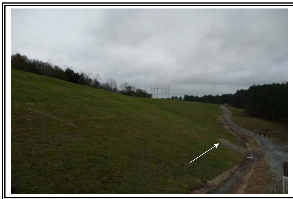
Ash Pond D, south central portion of dike facing south east at edge of toe. Dike seepage remediation shown by arrow
