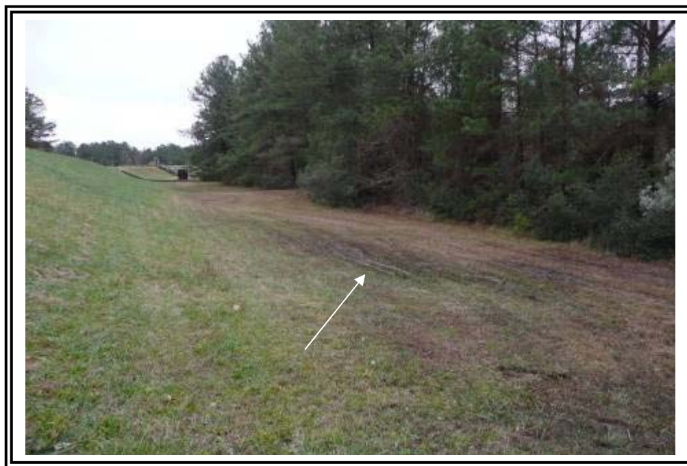
Central portion of Ash Pond C west dike toe facing south. One of two "soft spot" s indicated by arrow.
