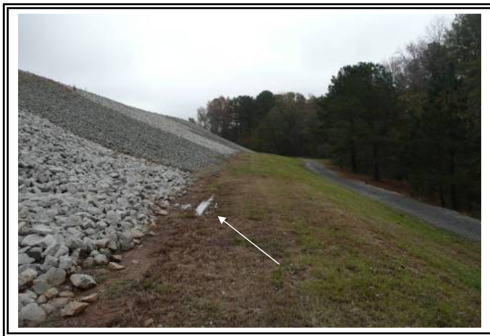
Ash Pond C, central portion of south dike along toe facing east. Pooled water shown frame left.
