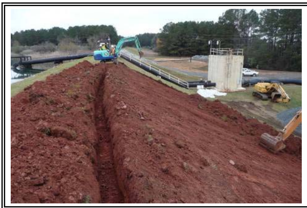
Ash Pond C, south end of east dike. Historic drain shown.
