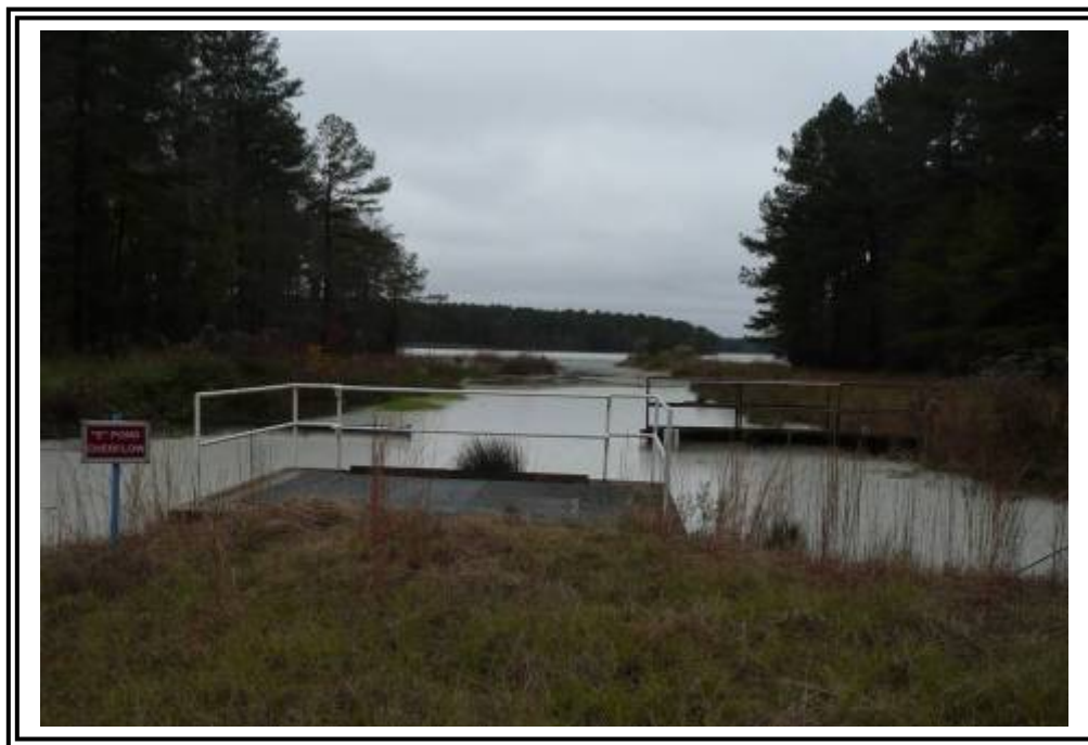
Ash Pond E decant spillway structure.
