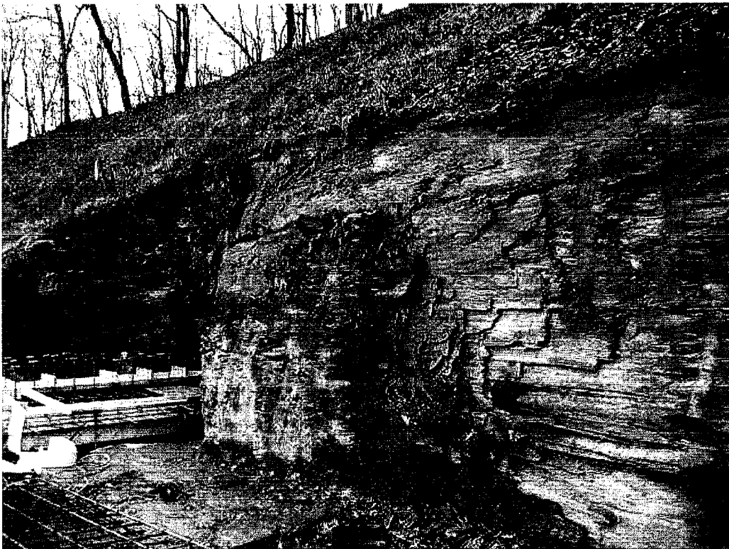
d04-049 11/20/06 left US wall notch
