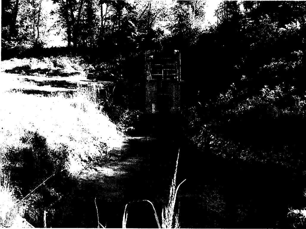
d04-049 9/21/06 right primary spillway intake
