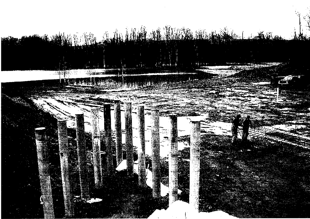
d04-049 11/20/06 spillway approach
