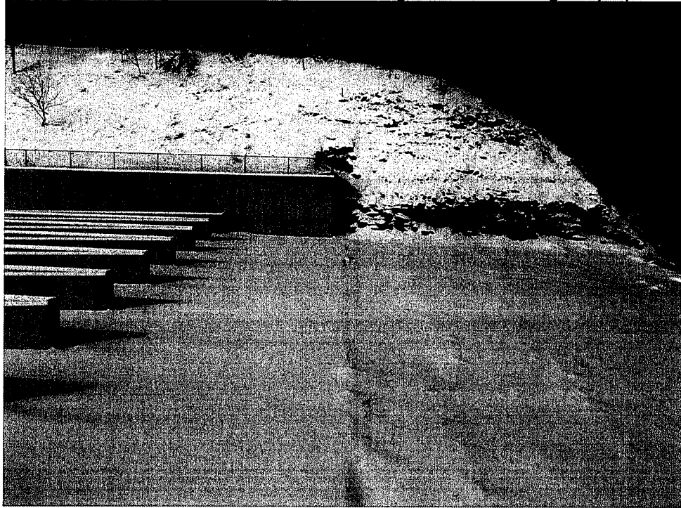
D04-049 01/21/09 Figure 11 View of discharge end of emergency spillway.
