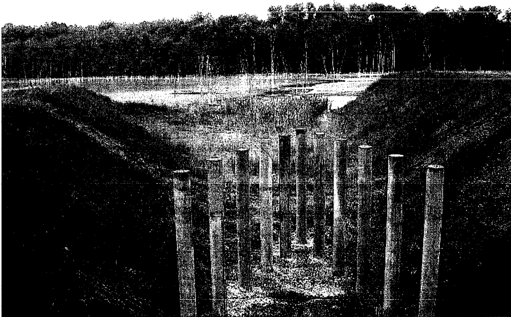
d04-049 8/29/05 looking from left primary spillway toward impoundment
