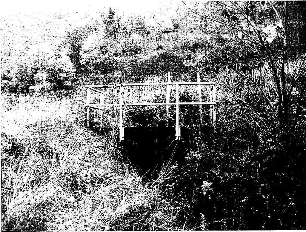
d04-049 10/23/07 discharge from left abutment
