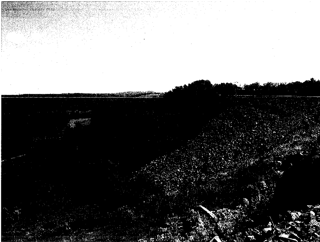
d04-049 9/21/06 DS slope from left
