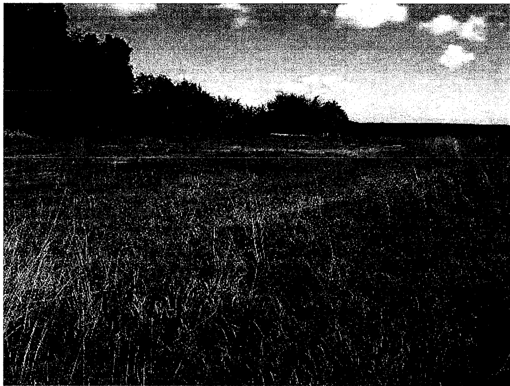
d04-049 9/21/06 area between left primary spillway and emergency spillway
