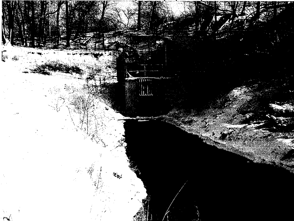
D04-049 01/21/09 Figure 4 View of primary spillway inlet and treatment system.
