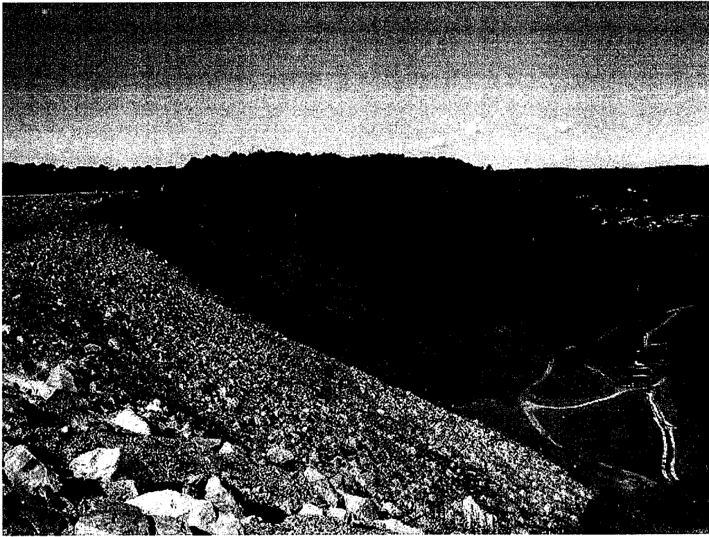
d04-049 9/21/06 DS & left abutment from right crest
