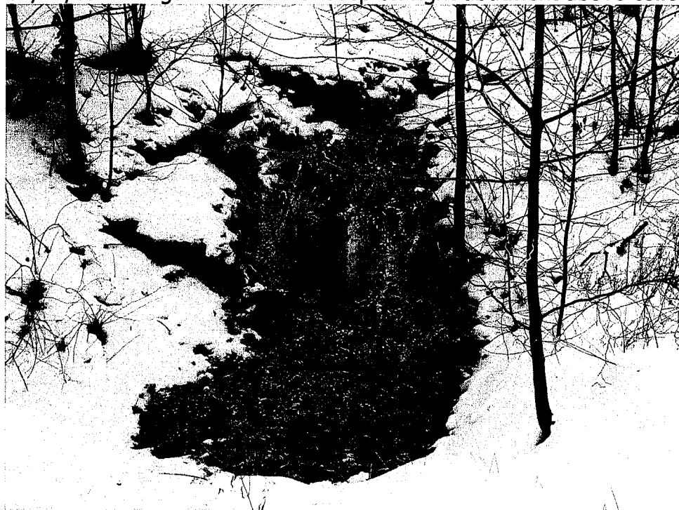
D04-049 01/21/09 Figure 19 View of seep on right abutment above collection system.
