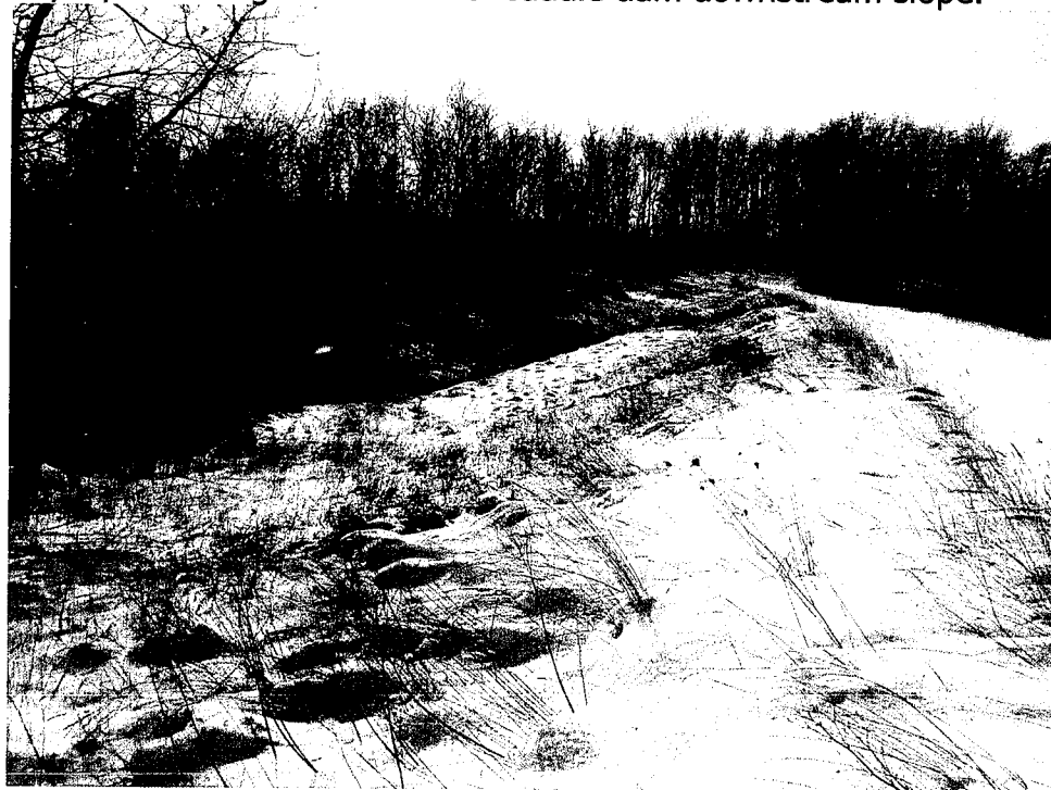
D04-049 01/21/09 Figure 16 View of saddle dam downstream slope.
