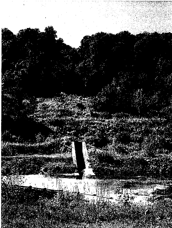
d04-049 9/21/06 outlet of left primary spillway
