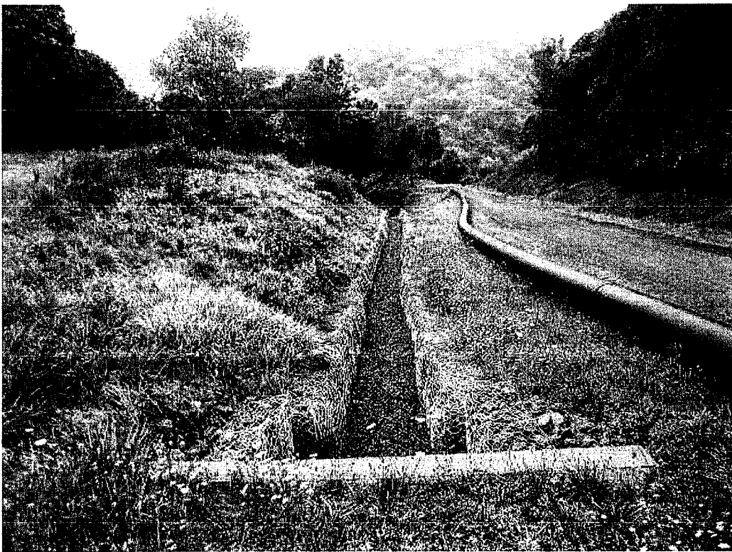
d04-049 8/29/05 gabion channel for right abutment seepage
