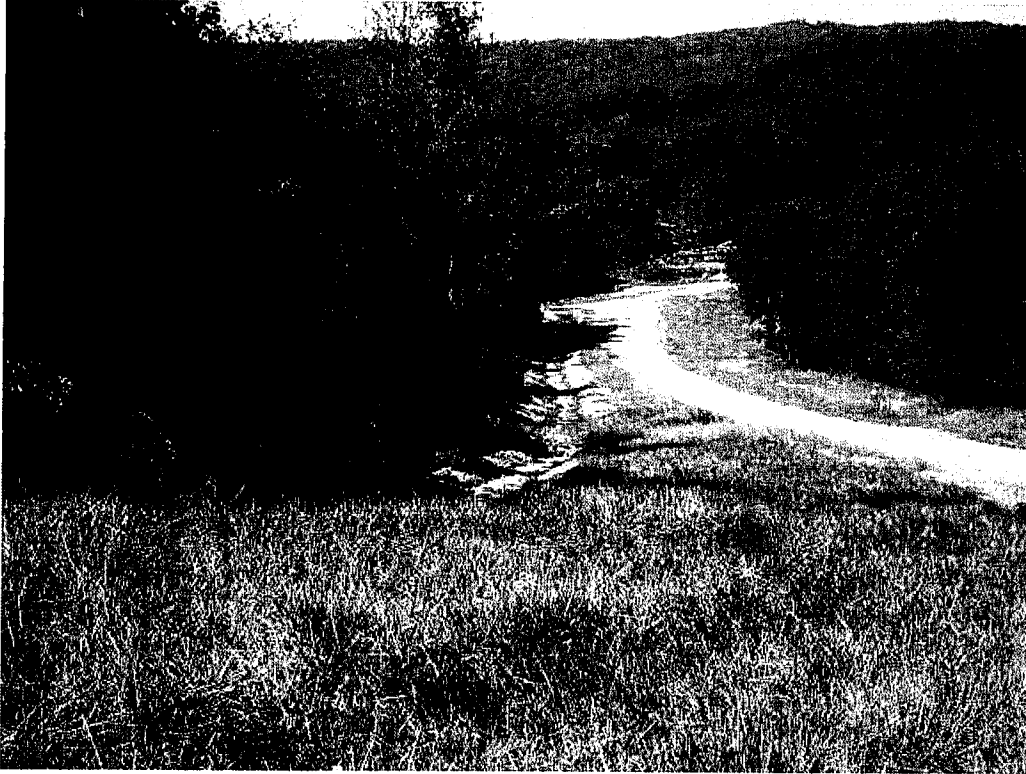
d04-049 9/21/06 right primary spillway wasteway
