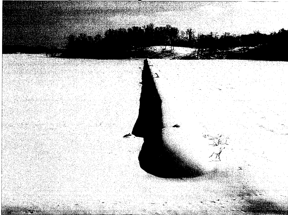
D04-049 01/21/09 Figure 21 View of geotube.
