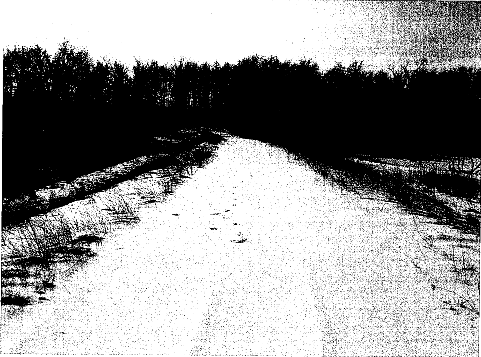
D04-049 01/21/09 Figure 17 View of saddle dam crest.
