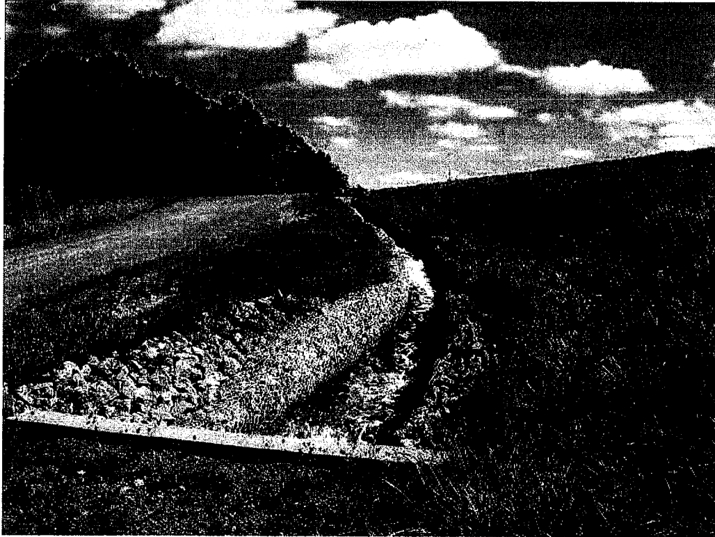
04-049 9/21/06 right primary spillway wasteway
