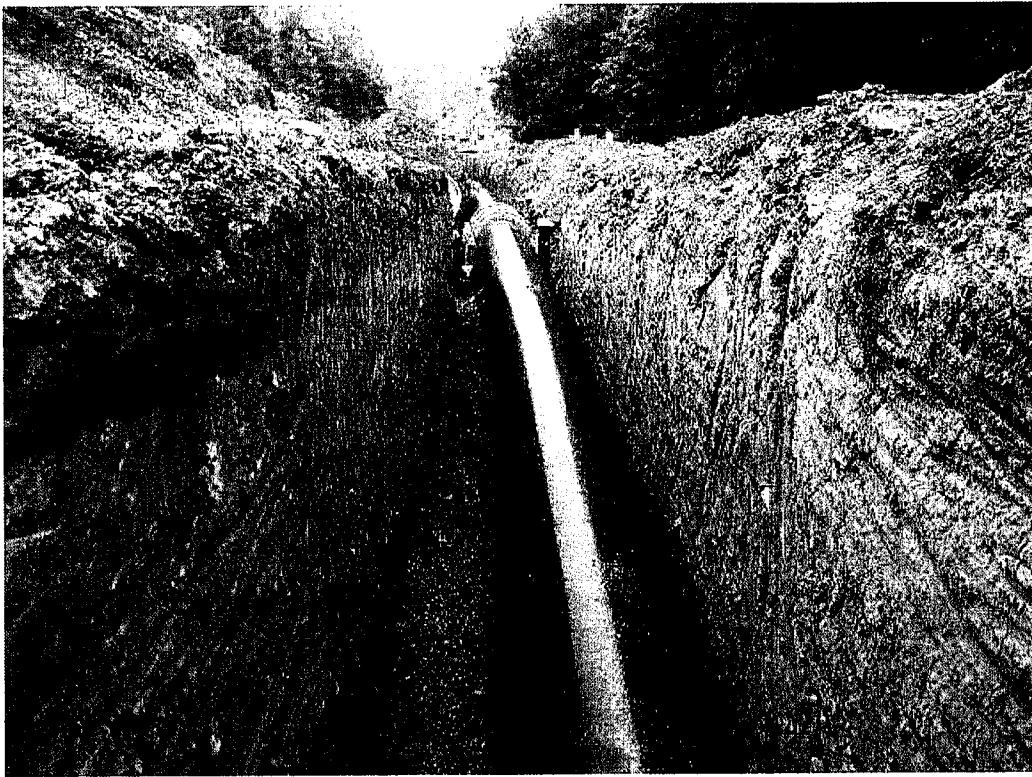
d04-049 8/29/05 soil cut on right side of abutment
