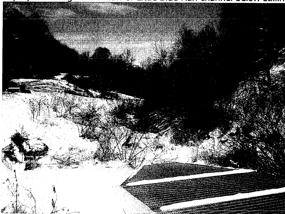
D04-049 01/21/09 Figure 14 View of Little Blue Run channel below stilling basin.
