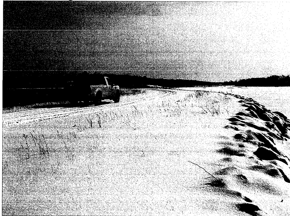
D04-049 01/21/09 Figure 2 View of crest.
