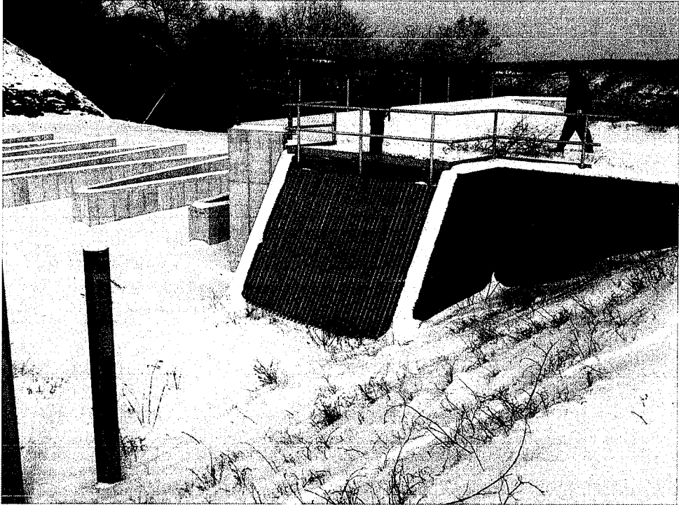
D04-049 01/21/09 Figure 8 View of secondary spillway inlet.
