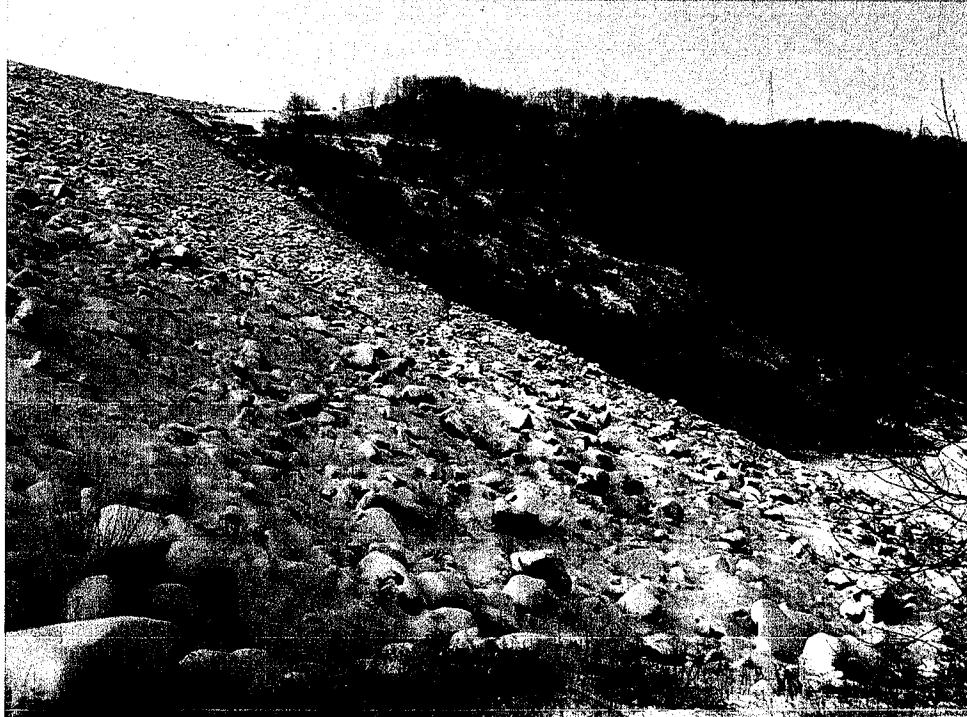
D04-049 01/21/09 Figure 12 View of left abutment and downstream face.
