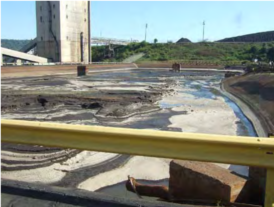
PHOTO 3: NORTH LDS POND DRAINED AND CLEANING
