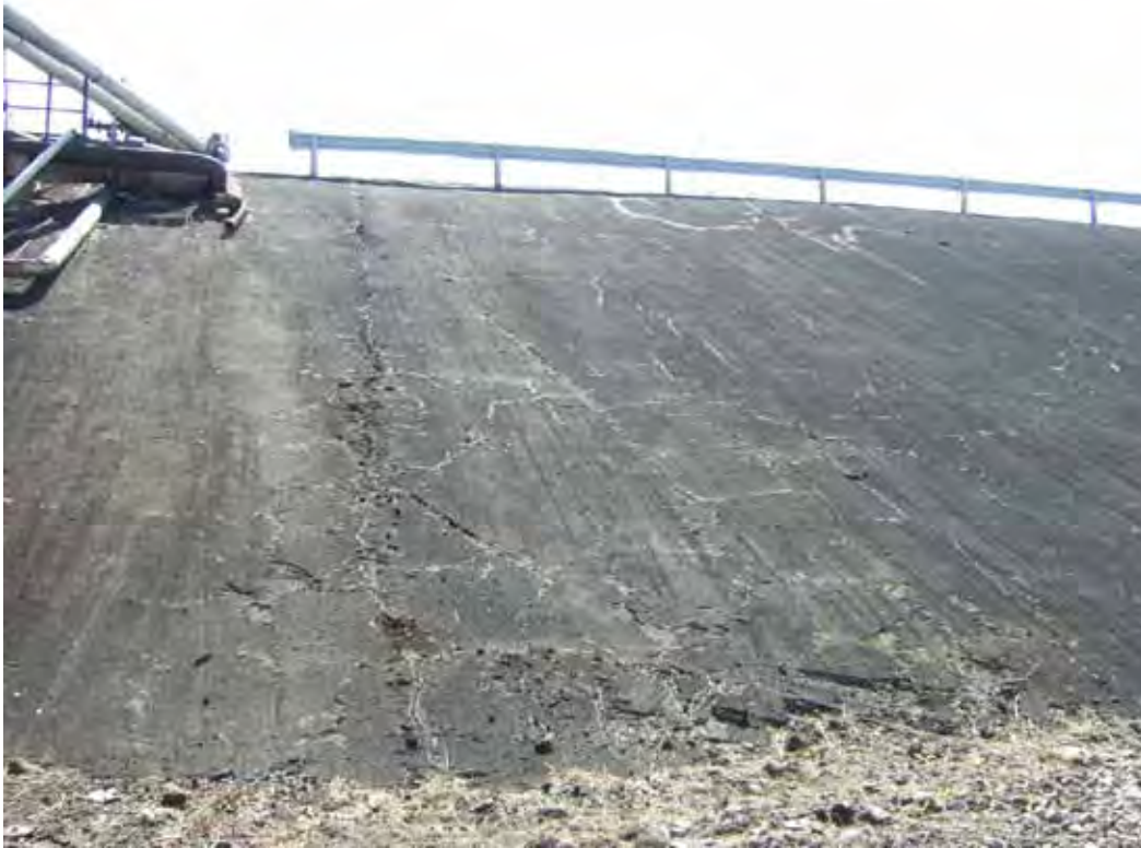
PHOTO 22: NORTH DOWNSTREAM SLOPE OF WEST HDS POND
