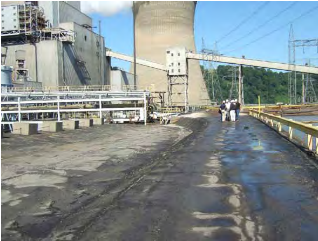
PHOTO 11: WEST EMBANKMENT CREST FOR SOUTH LDS POND
