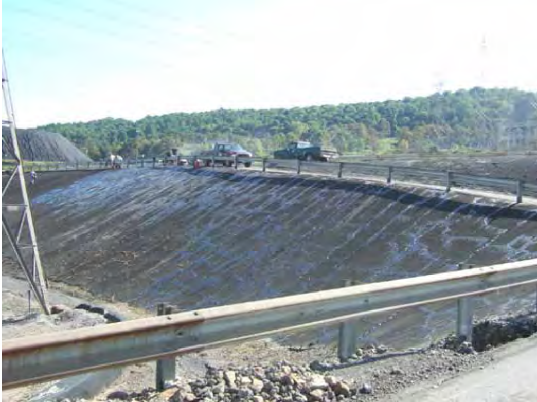
PHOTO 13: REPAIR OF ASPHALT ON WEST HDS POND NORTH SLOPE
