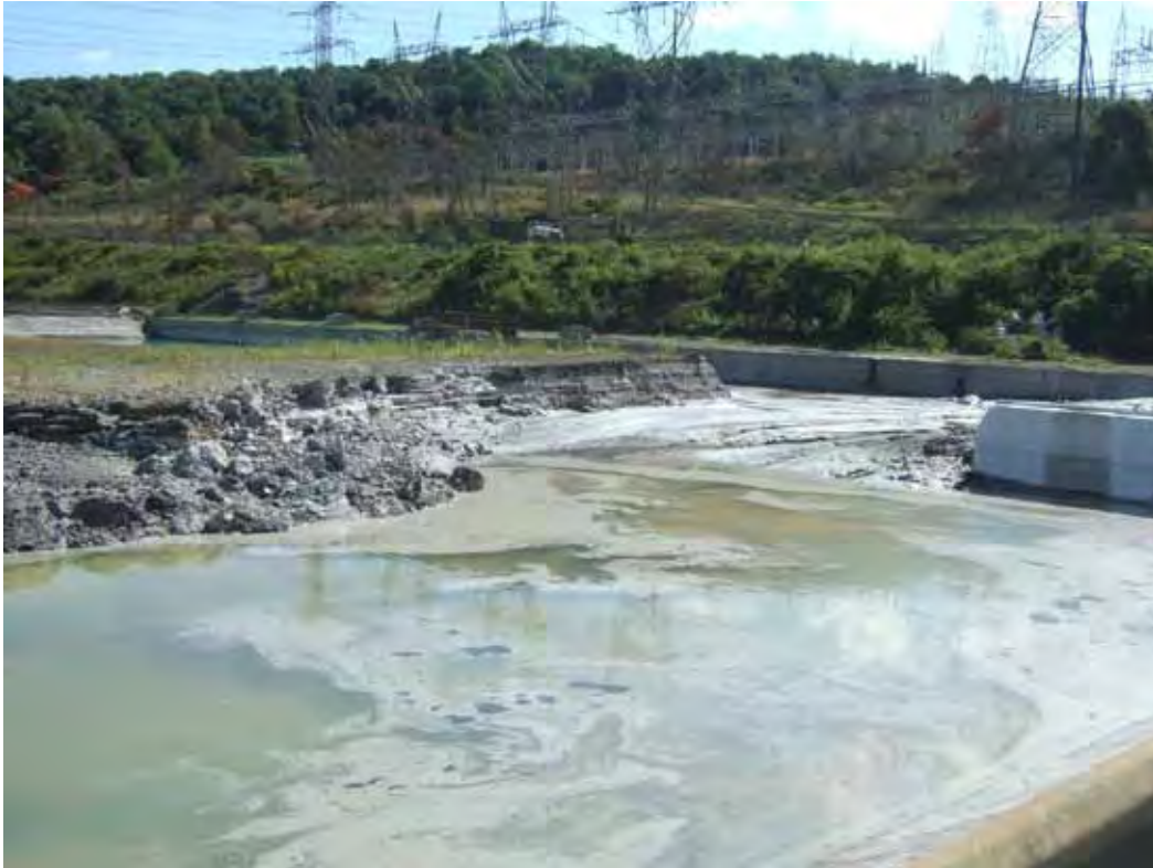
PHOTO 15: WASTE BUILDUP IN WEST HDS POND
