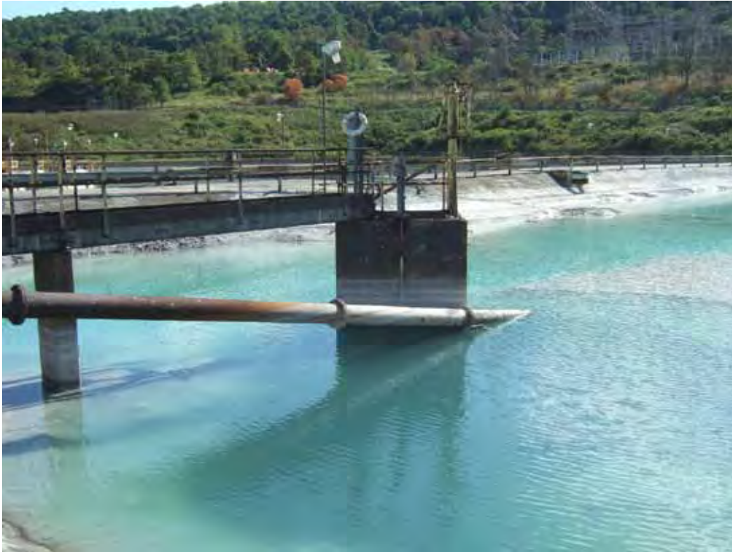
PHOTO 20: DECOMMISSIONED STRUCTURE IN WEST HDS POND
