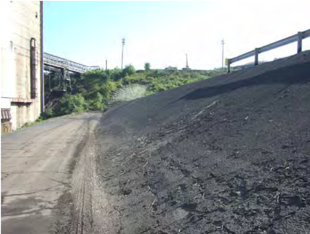
PHOTO 1: DOWNSTREAM NORTH SLOPE OF NORTH LDS POND
