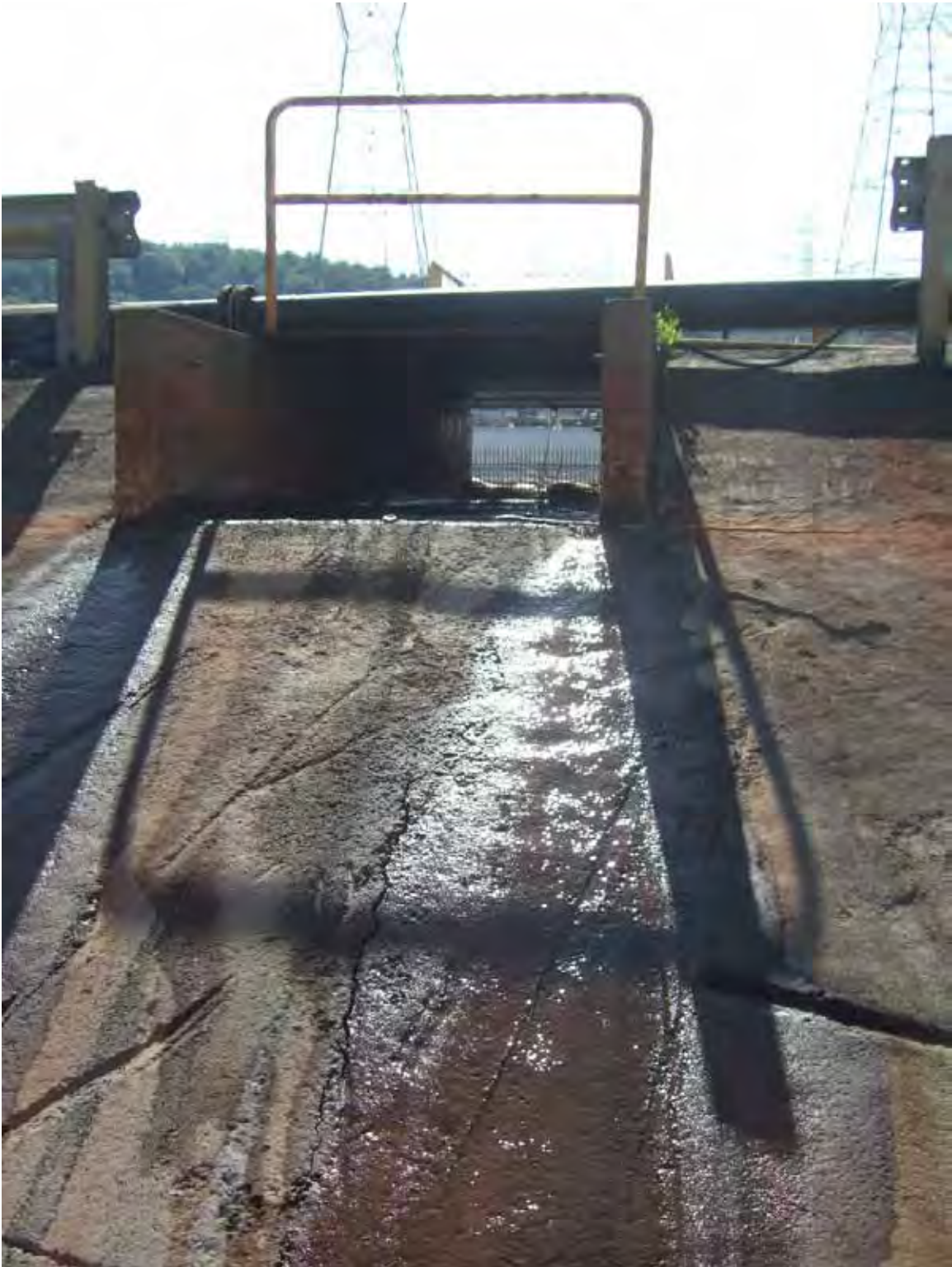
PHOTO 10: SPILLWAY BETWEEN NORTH AND SOUTH LDS PONDS
