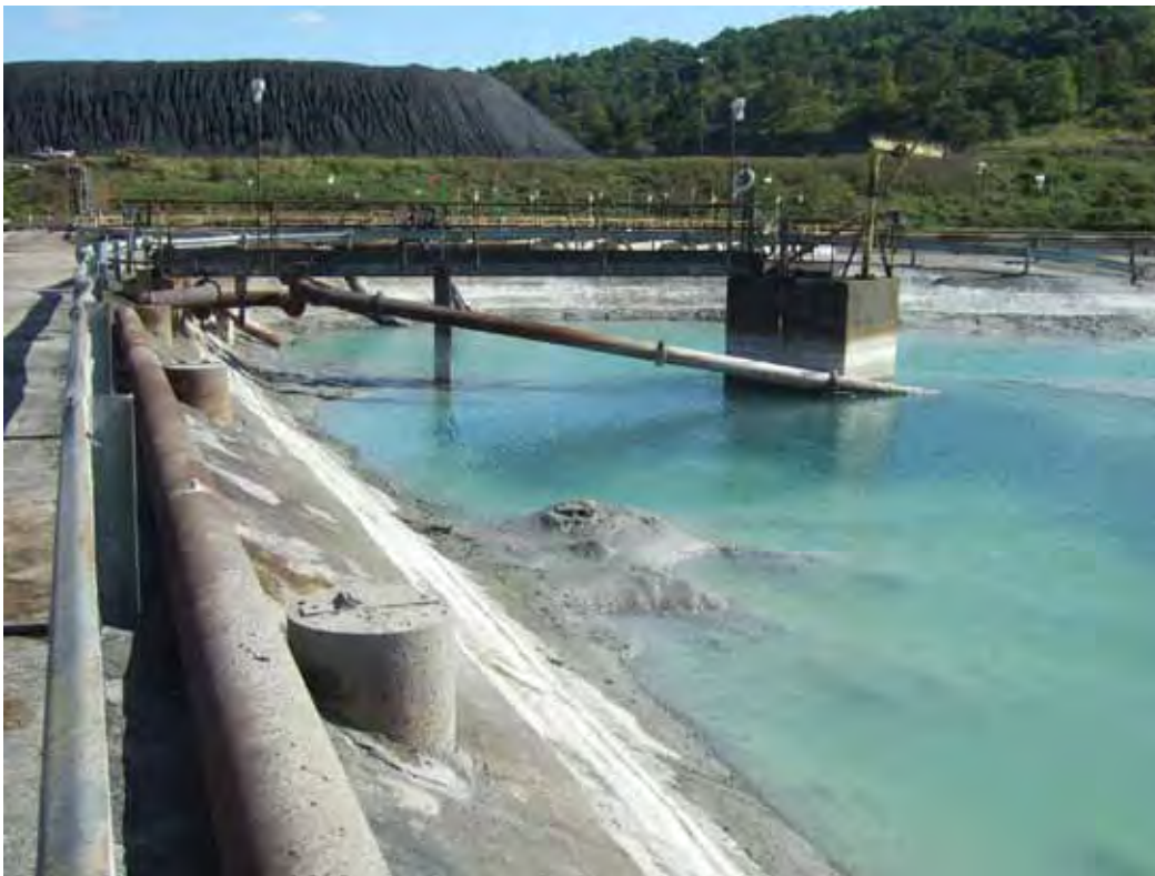
PHOTO 19: ALONG NORTH CREST OF WEST HDS POND
