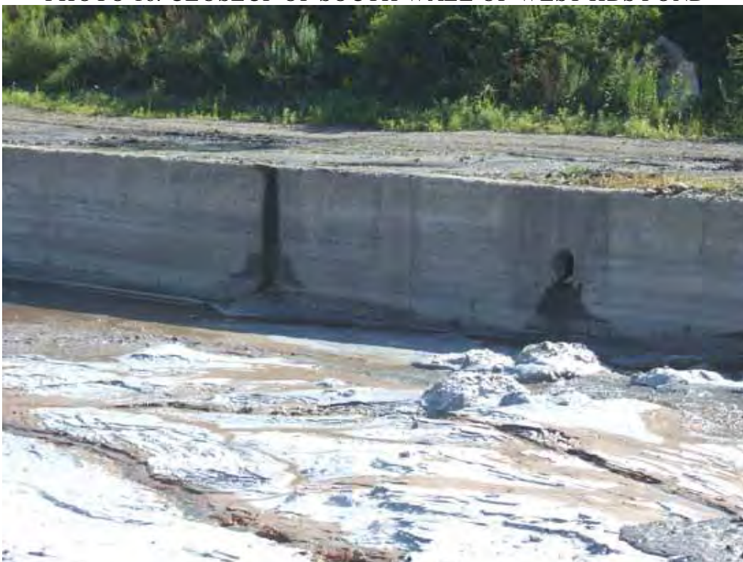
PHOTO 16: CLOSEUP OF SOUTH WALL OF WEST HDS POND
