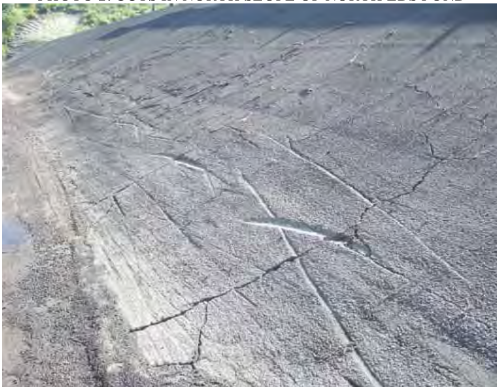
PHOTO 2: CUTS IN NORTH SLOPE OF NORTH LDS POND
