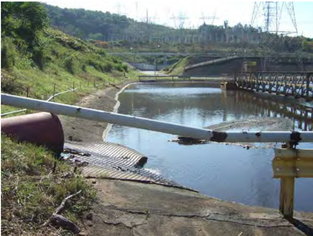
PHOTO 6: COAL AREA STORM DISCHARGE INTO SOUTH LDS POND
