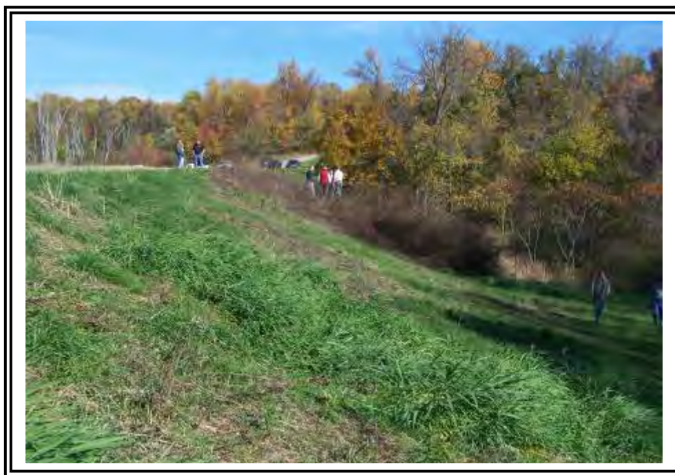
Downstream slope of Little Blue Run Saddle Dam, looking north. Vegetation near group of people on slope consists of material that the mower cannot traverse.
