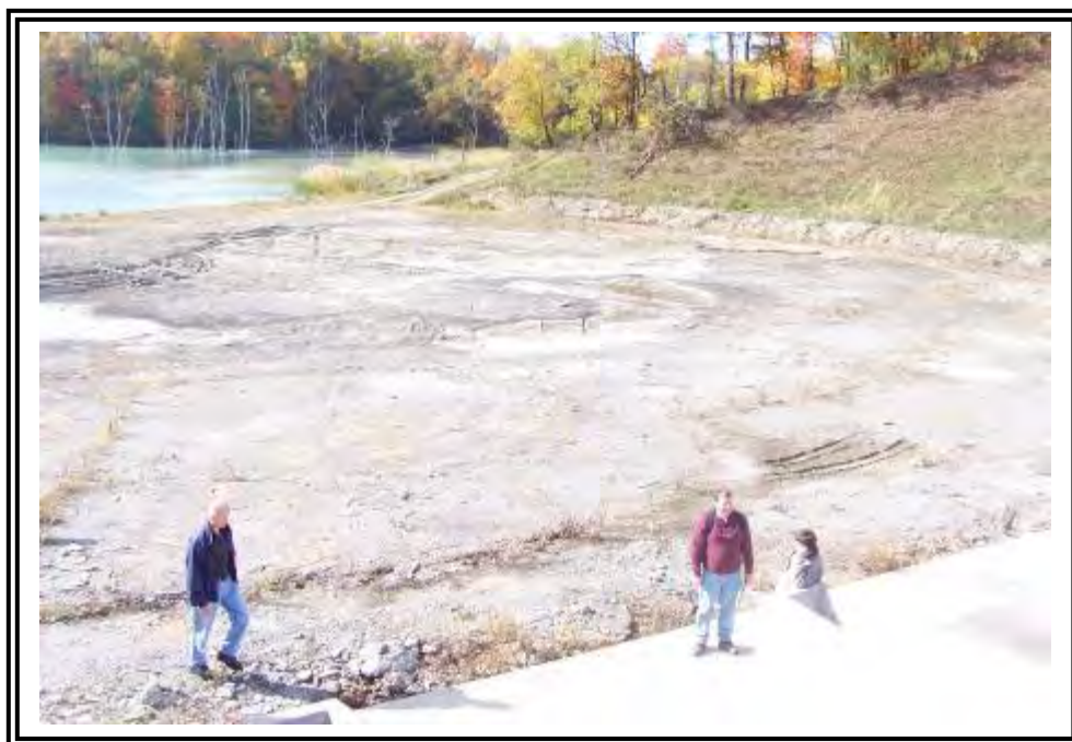
Approach to emergency spillway in bedrock.
