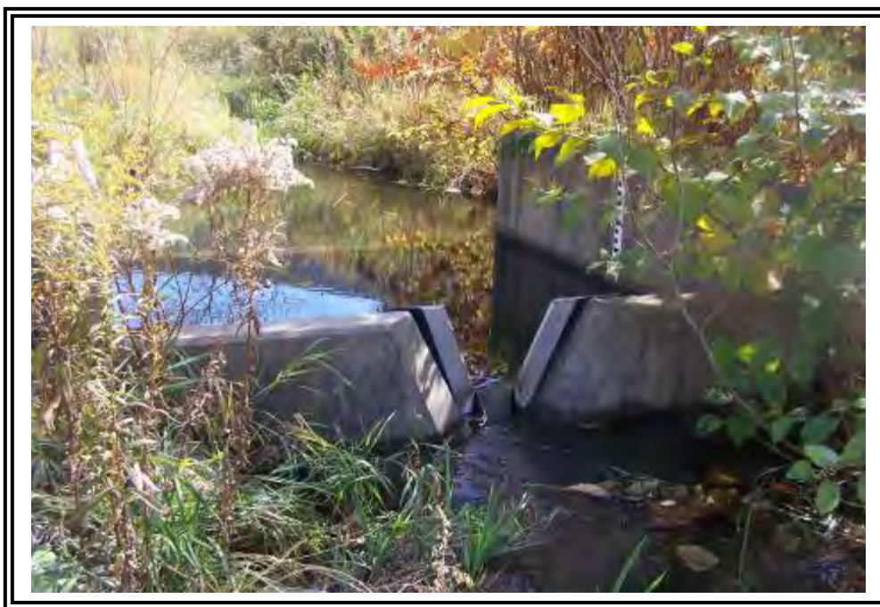
ULA v-notch monitoring weir for west abutment seepage monitoring. Clogged culvert was causing back flow during our site visit.
