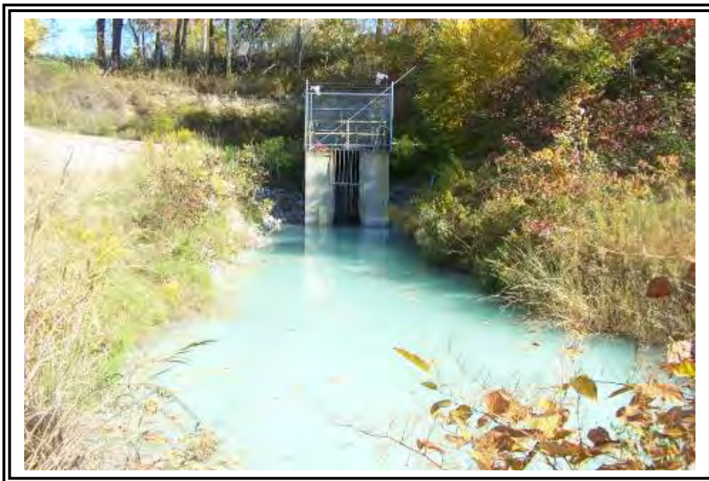
Secondary spillway approach channel and inlet.
