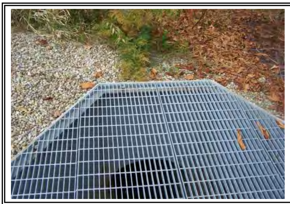
Outfall from stilling basin conveyed by buried HDPE pipe to the Ohio River.
