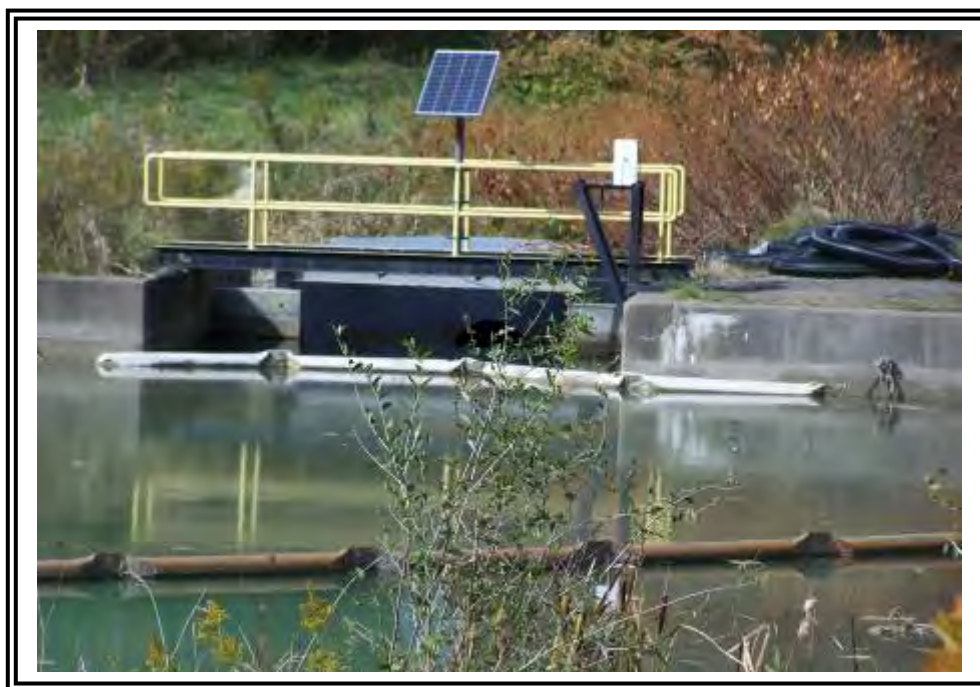
Stilling basin with floating debris barriers.
