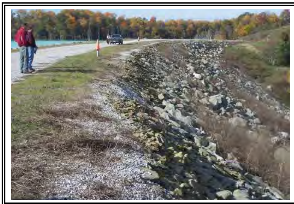
The crest elevation and 2-foot camber was made by adding 0 to 3.5 feet of rock fill to the top of the dam and rip rap slope protection to the upstream and downstream slope.
