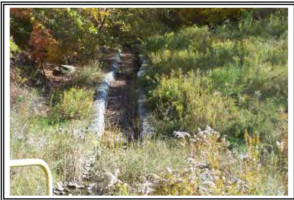
Gabion channel from secondary spillway.
