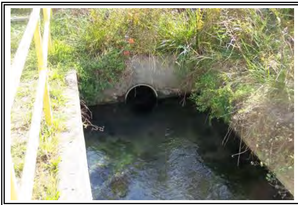
Toe drain (TD) collection pipe terminating in Parshall Flume.
