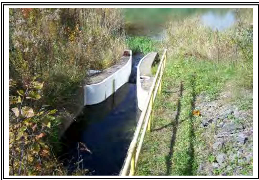
TD Parshall flume monitoring point for blanket drain seepage.
