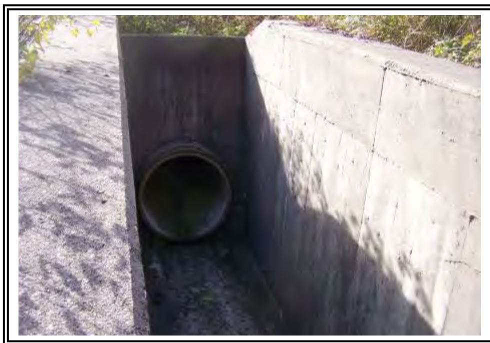
Terminus of service spillway at stilling basin.
