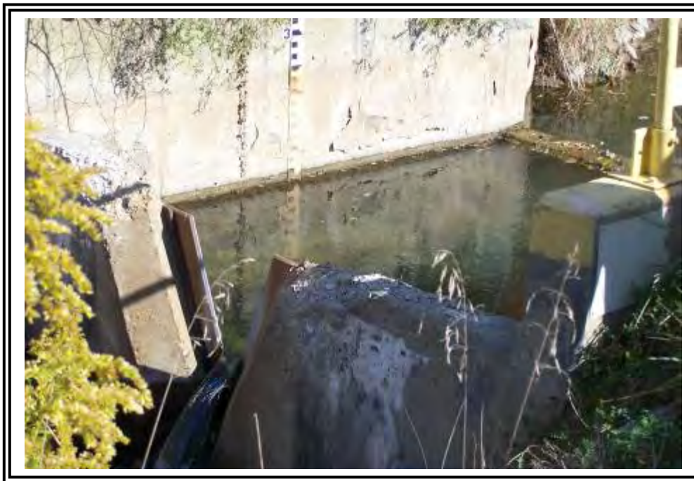
Right Abutment (RA) v-notch monitoring weir containing secondary spillway and east abutment seepage flow.
