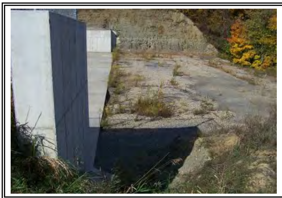
Downstream channel of emergency spillway.
