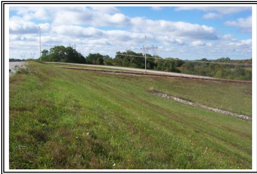
Downstream slope looking west toward access road.
