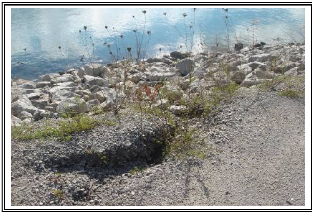
Erosion rill on upstream slope.
