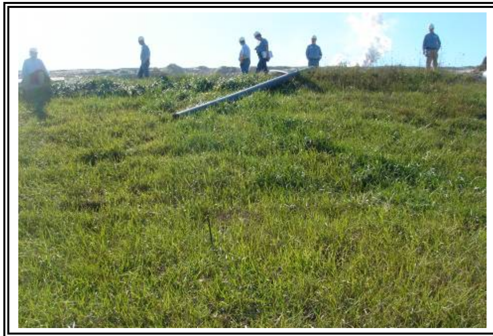
Area of seep near top of gypsum stacking facility east starter dike. Kentucky Utilities is working with Stantec (Engineer of Record) to resolve this issue. Seepage is at approximate elevation of current water surface in the pond.
