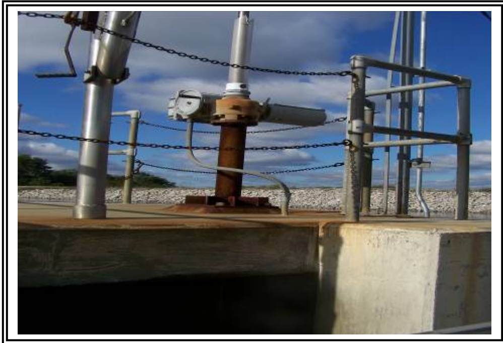
Outlet structure equipped with gates to close outlet flow from discharge pipe.
