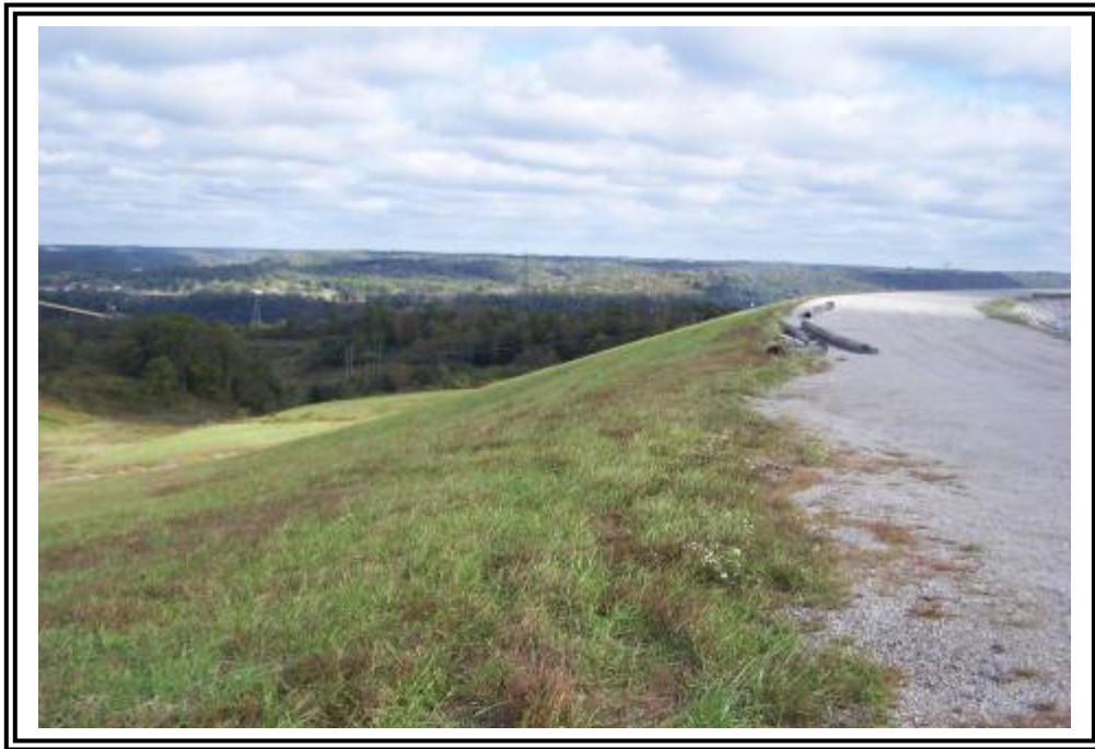
Downstream slope from access road looking northeast.
