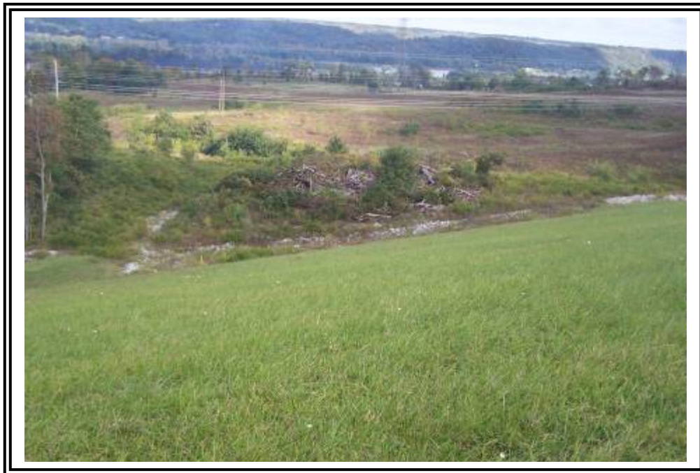
Downstream slope of ATB #2 at eastern knoll looking northeast.
