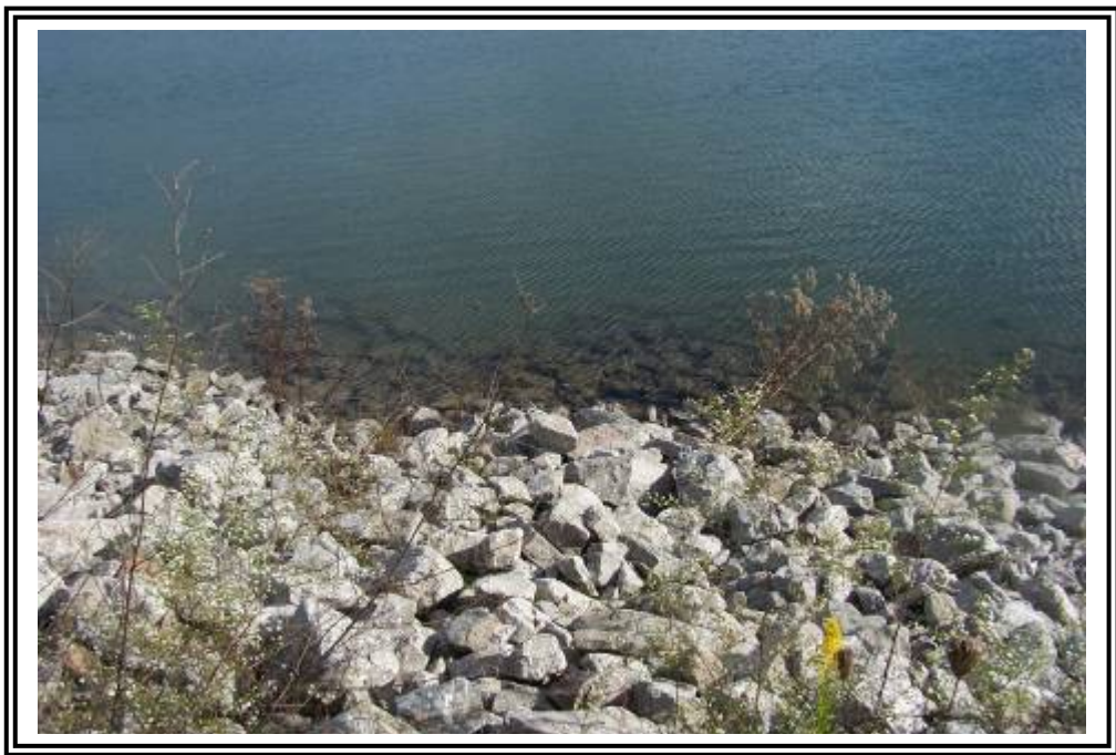
Rip rap protection on upstream slope of ATB #2 extends below the normal pool elevation.
