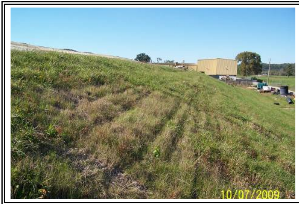
Area of repaired surficial slough on the east side of the gypsum stacking facility starter dike. Slough occurred and was repaired in Spring 2009.
