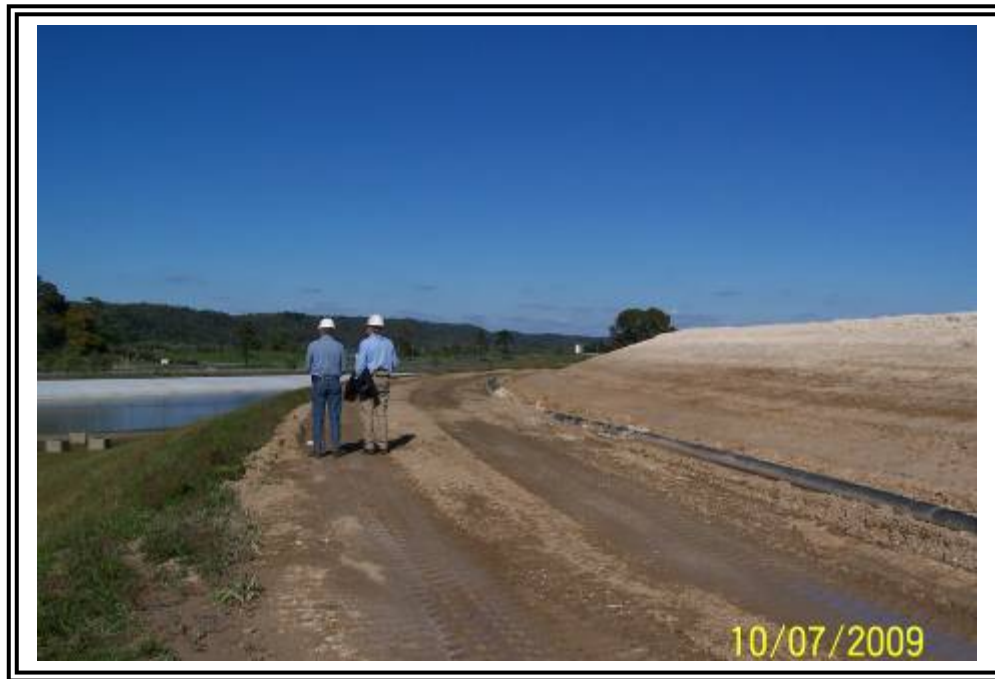
Crest of starter dike at northwest corner of gypsum stacking facility dike, looking northeast.
