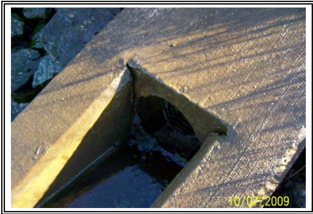
Toe drain at northeast corner of ATB #1. No apparent flow, concrete is wet from splash from outlet pipe.
