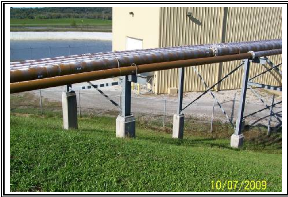
Pipe rack diverting gypsum to reuse facility on northeast corner of the gypsum stacking facility starter dike.
