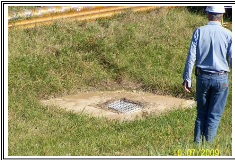
Surface drainage system on east side of gypsum stacking facility starter dike.
