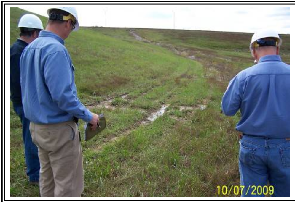
Standing water on west end of upper bench.
