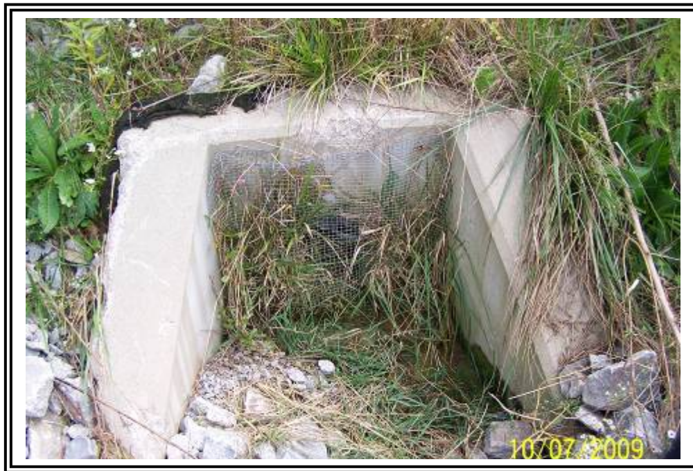
Toe drain at base of main fill.
