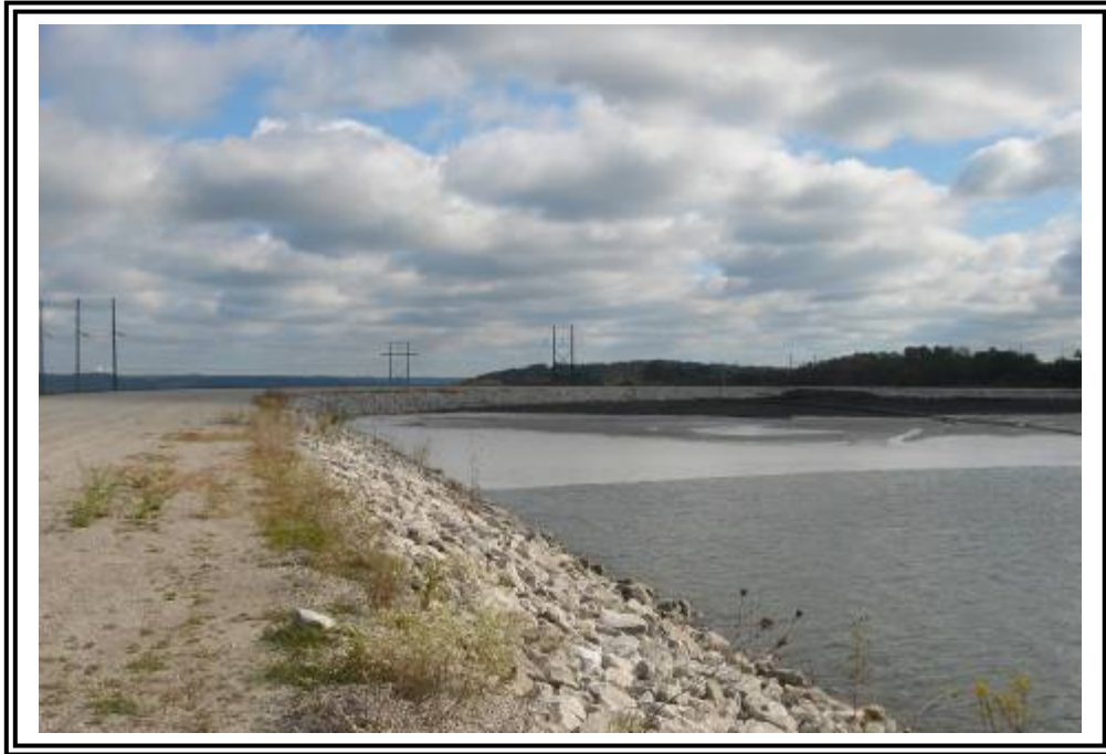
Upstream slope of ATB #2 looking east.
