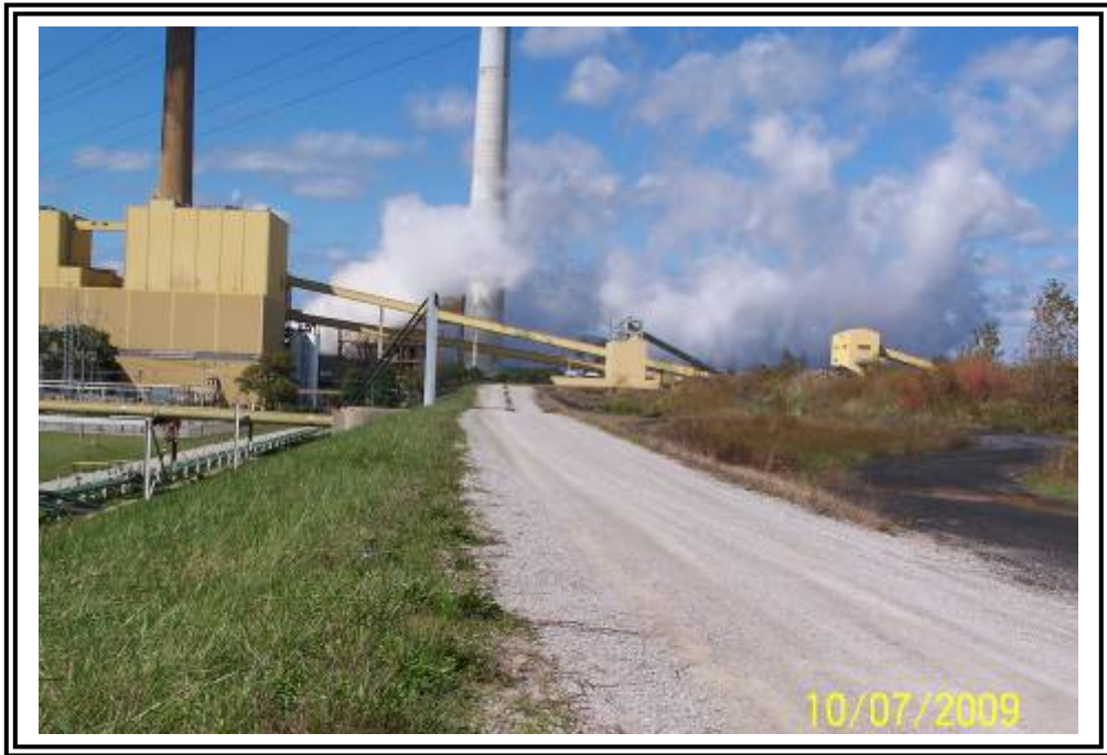
Crest of west dike ATB #1 looking north, "bumpiness" from buried sluice pipe crossing.
