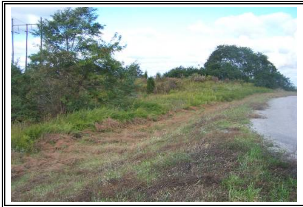
Downstream slope west end of dike looking north. Taller grass is on natural ground.
