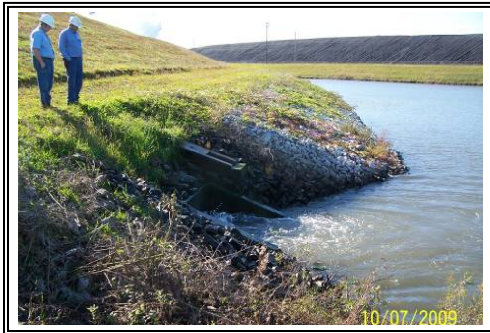
Outlet pipe discharge into secondary Ash treatment basin.
