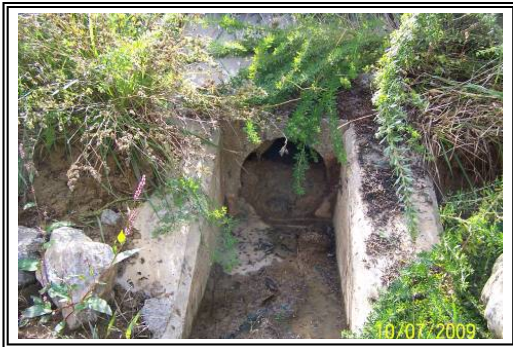
Toe drain on east side of secondary drainage fill about ¾ clogged at outlet. Signs of erosion on slopes around outlet so unclear if sediment is from pipe or other causes.
