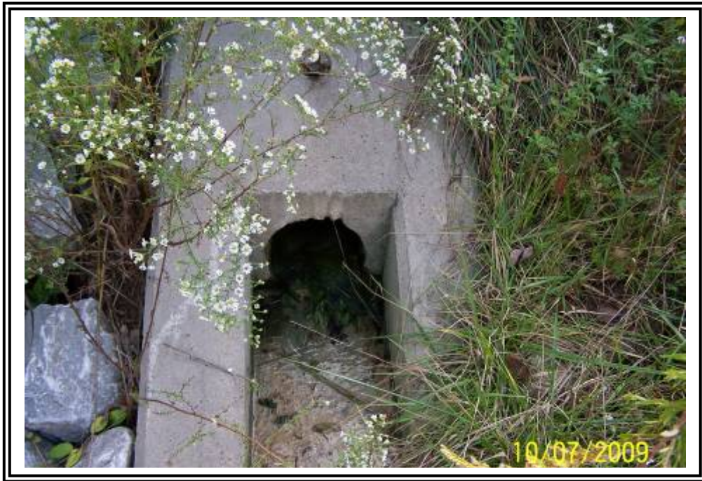
Toe drain on east side of main fill between upper bench and next lower bench.
