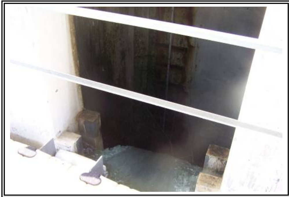
Decant over stop logs in outlet structure.
