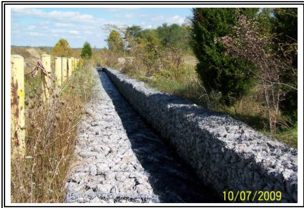
Sluiceway from ATB #2 discharge into ATB #1.
