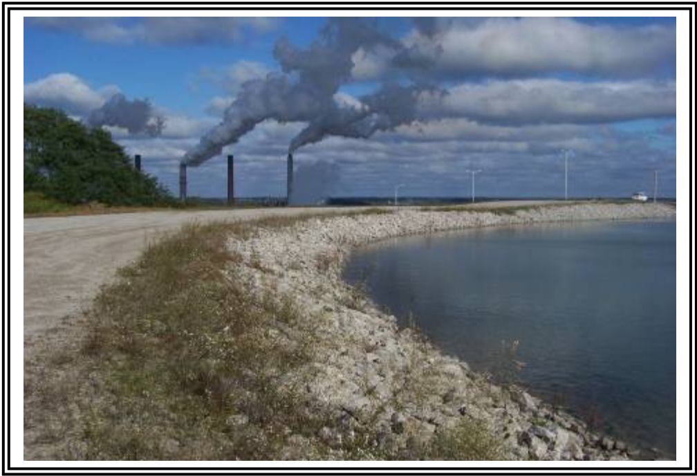
Upstream slope of ATB #2 looking north.
