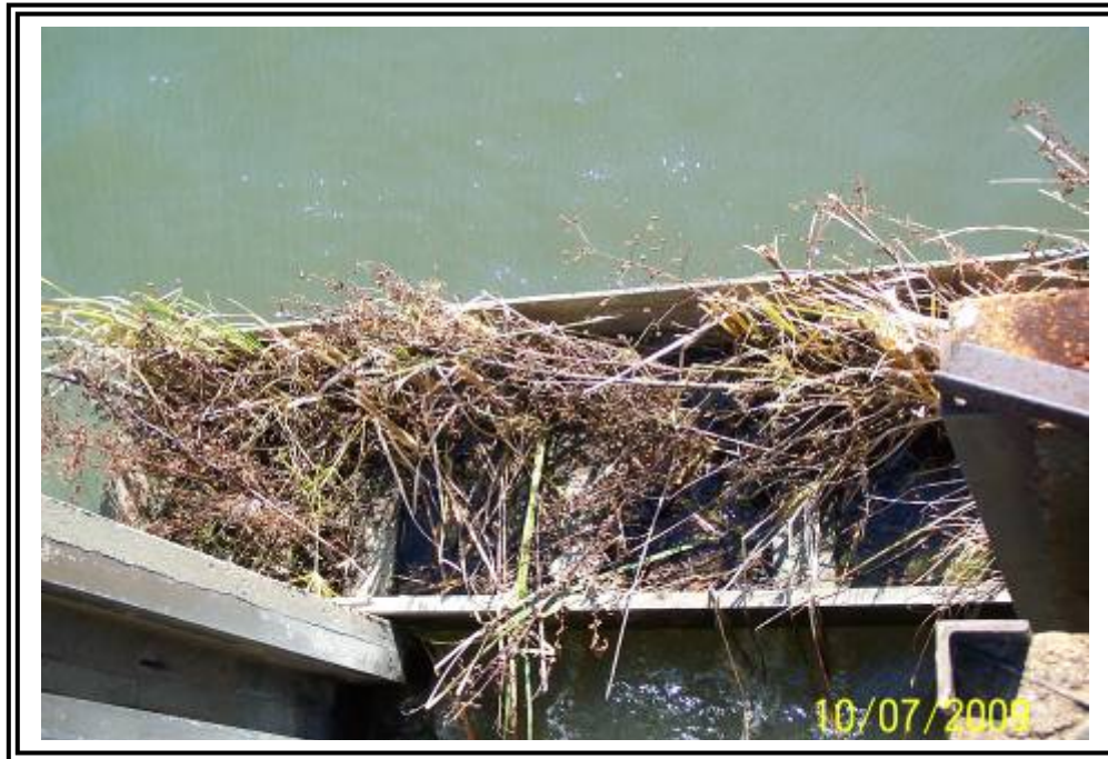
Decant structure in ATB #1.
