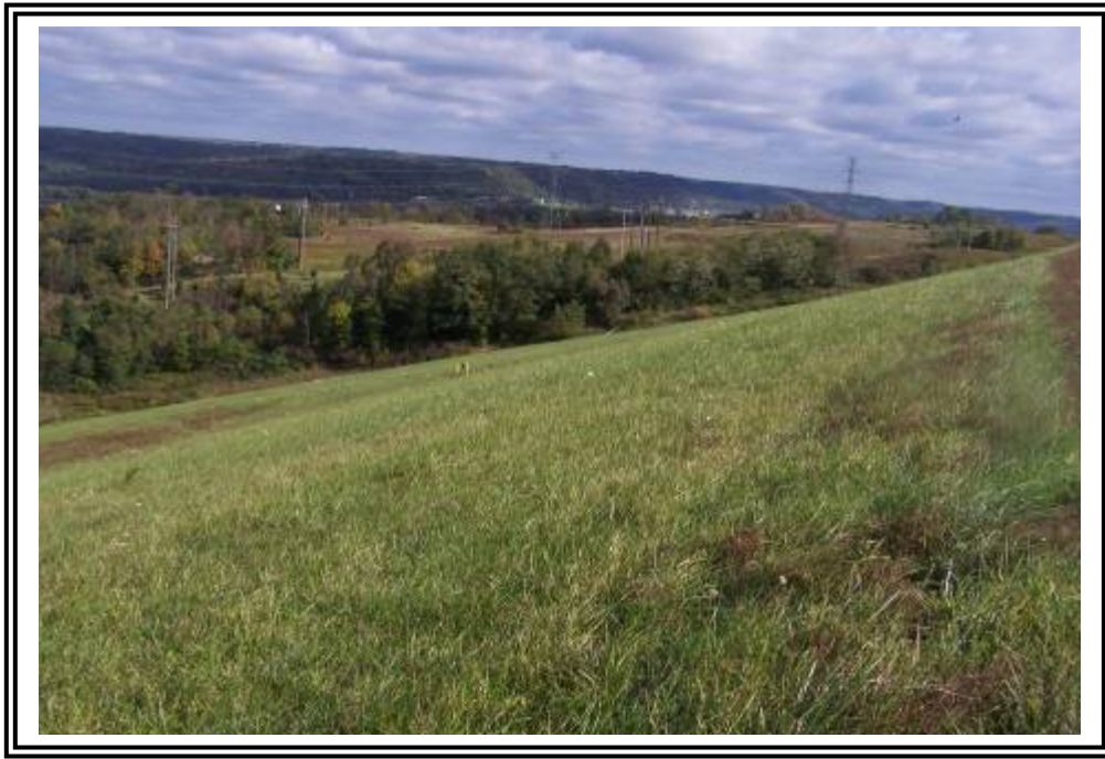
Upper portion of downstream slope of ATB #2 looking northeast. Instrumentation marked with yellow bollards, horizontal benched in main section of Dike at 50 vertical foot increments. .
