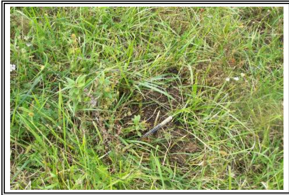
Small rodent hole on bench in secondary drainage fill section about 18 inches deep..
