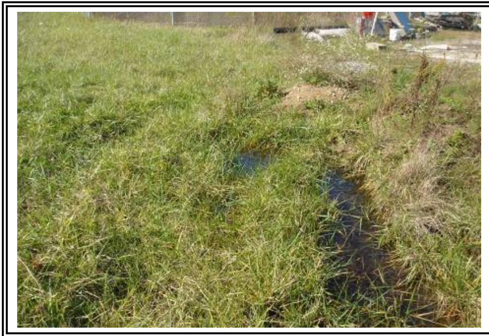
Standing water at the toe along the east side of the gypsum stacking facility starter dike. Ground is firm, appears to be surface water drainage.
