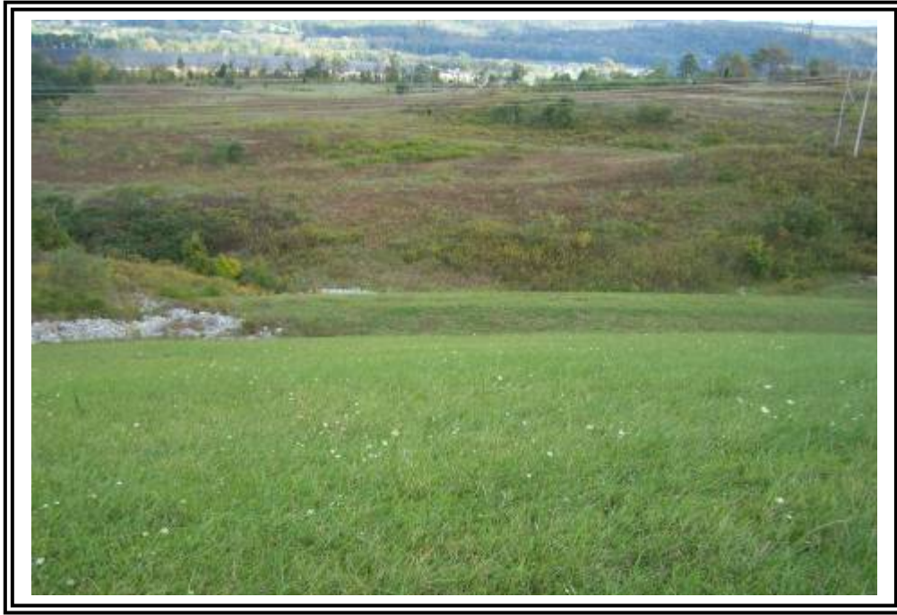
Downstream slope of ATB #1 just east of eastern knoll looking northeast.
