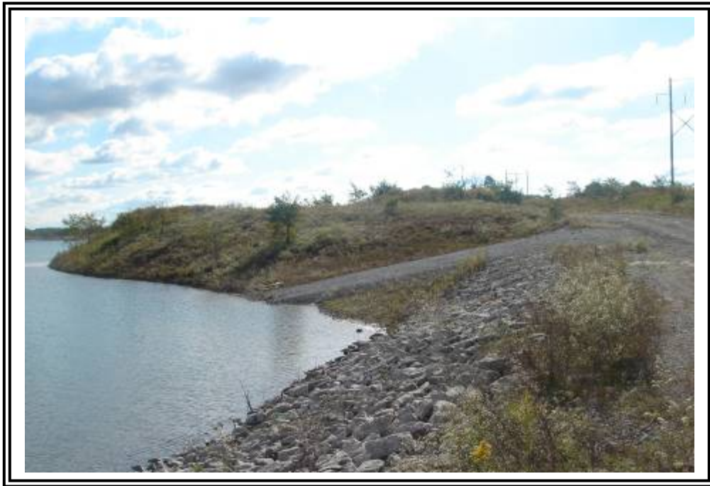
Upstream slope of ATB #2 looking south at west abutment and boat ramp.
