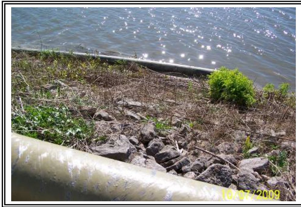
Upstream slope of ATB #1 east dike. Rip rap has been placed to fill areas of erosion.
