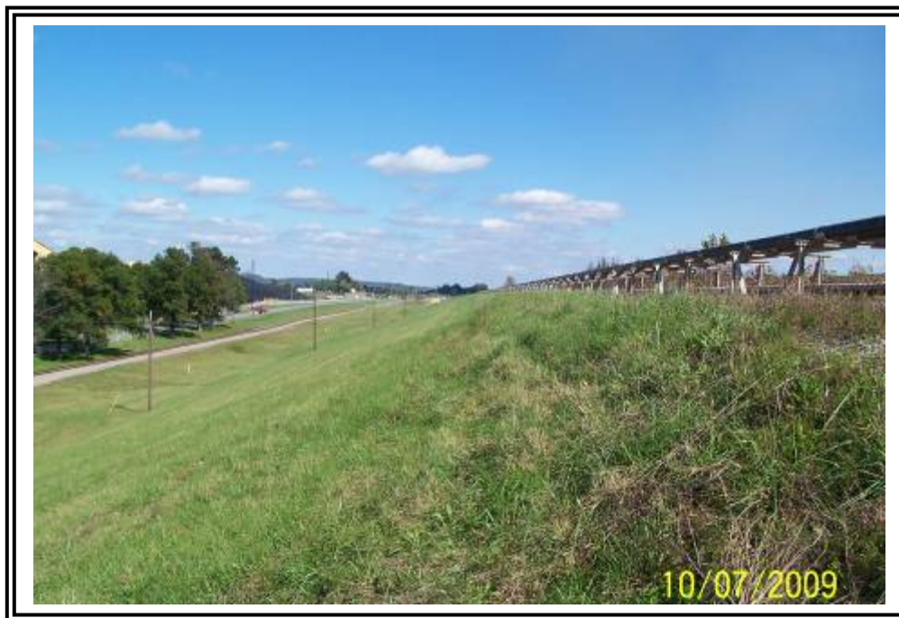
Downstream slope of ATB #1 north dike. Note over steepening adjacent to crest, looking east.
