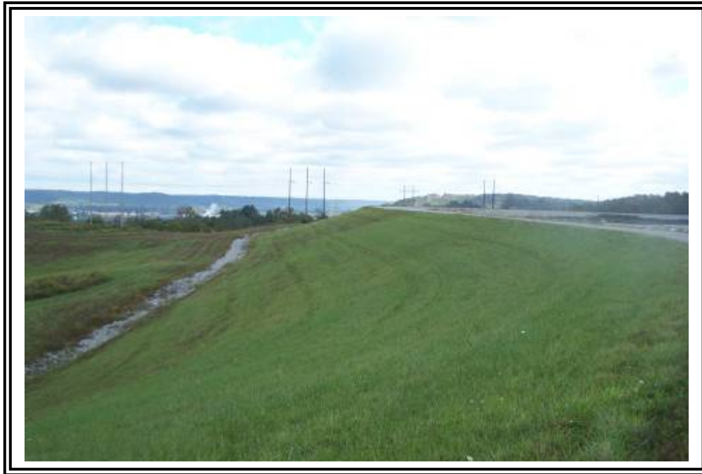
Downstream slope of ATB #1 looking east.
