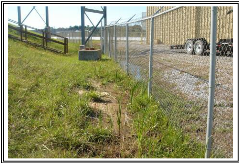
Standing water at toe at northeast corner of gypsum stacking facility starter dike. Appears to be surface drainage water.
