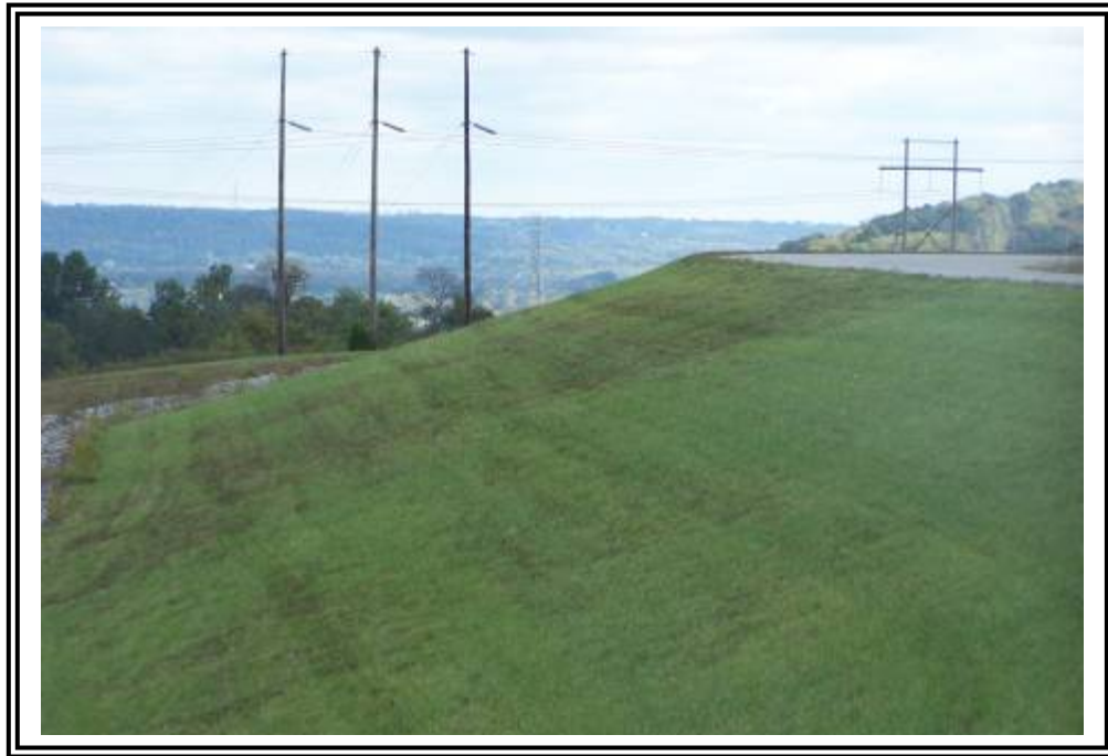
Downstream slope of east end of ATB #2 dike looking north from east abutment.
