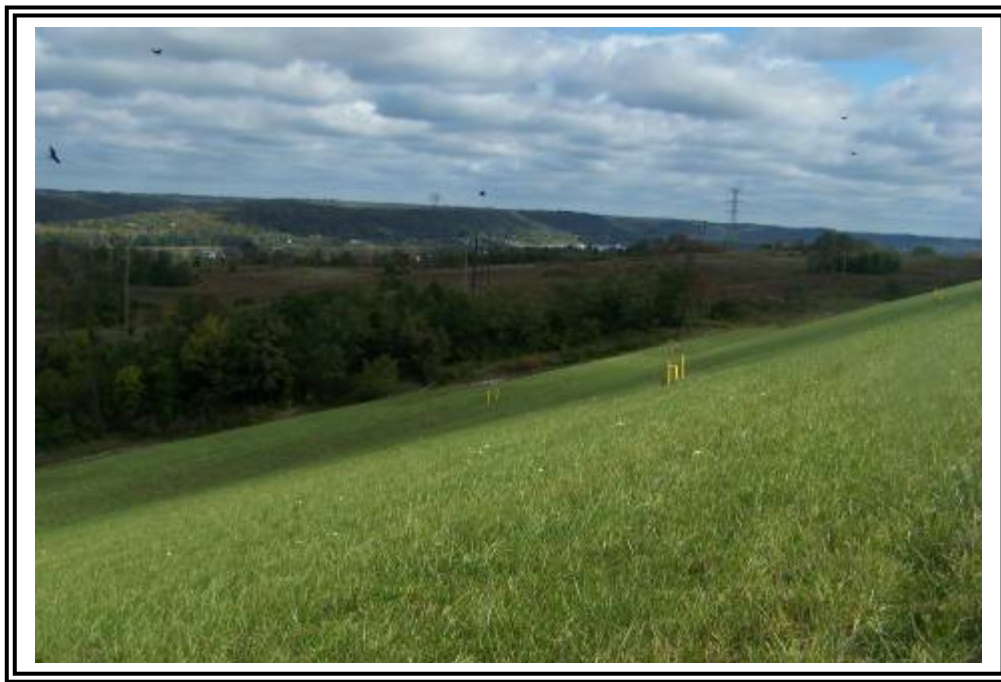
Upper portion of downstream slope of ATB #2 looking northeast. Instrumentation marked with yellow bollards, horizontal benched in main section of Dike at 50 vertical foot increments.
