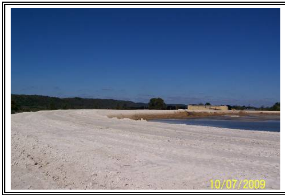
Crest of west end of gypsum stacking facility dike, looking northeast (under construction from dewatered gypsum).
