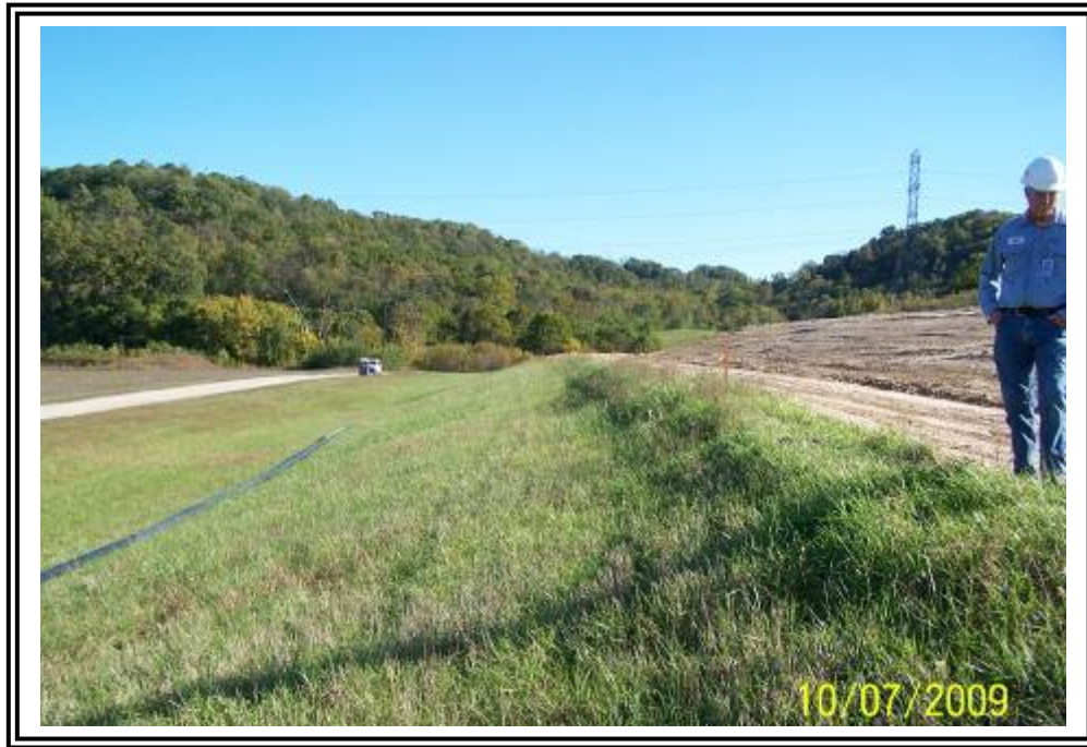
Over steepening at crest of east side of gypsum stacking facility starter dike, looking south.
