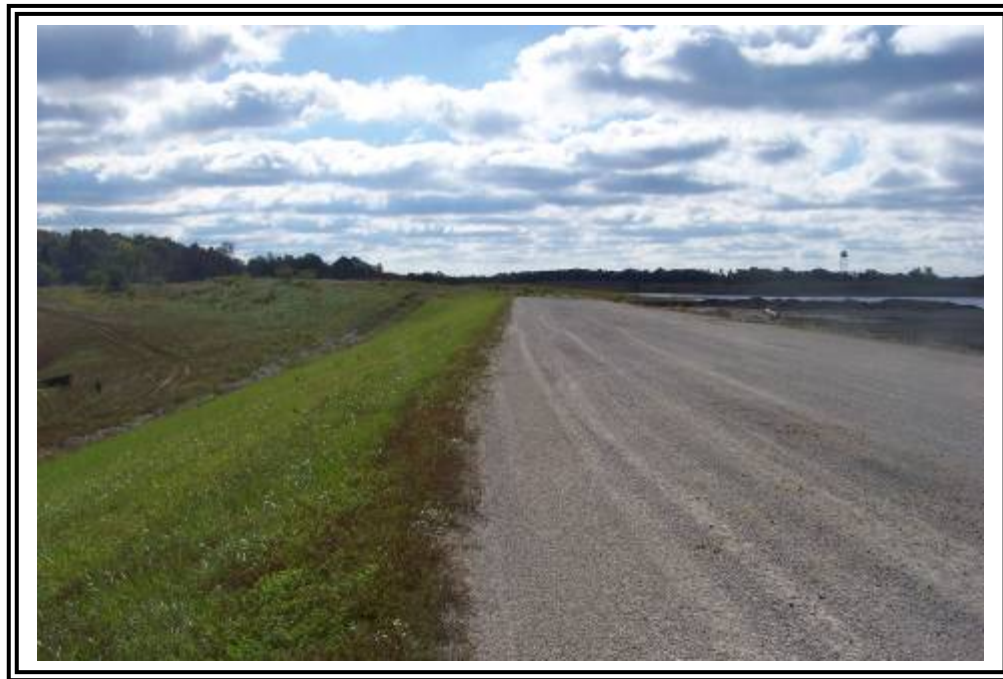
Crest of ATB #2 looking south toward east abutment.
