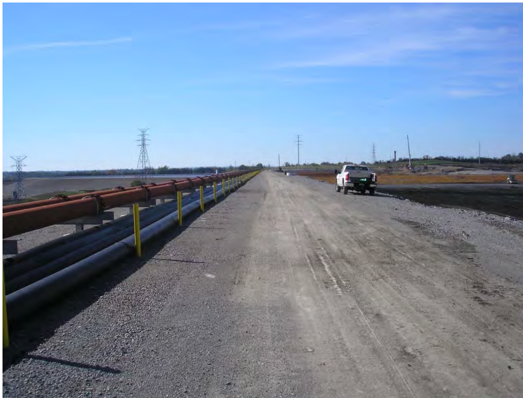
Figure 5.2.1-1 Crest of Main Fly Ash Pond Dam Looking Westward.
