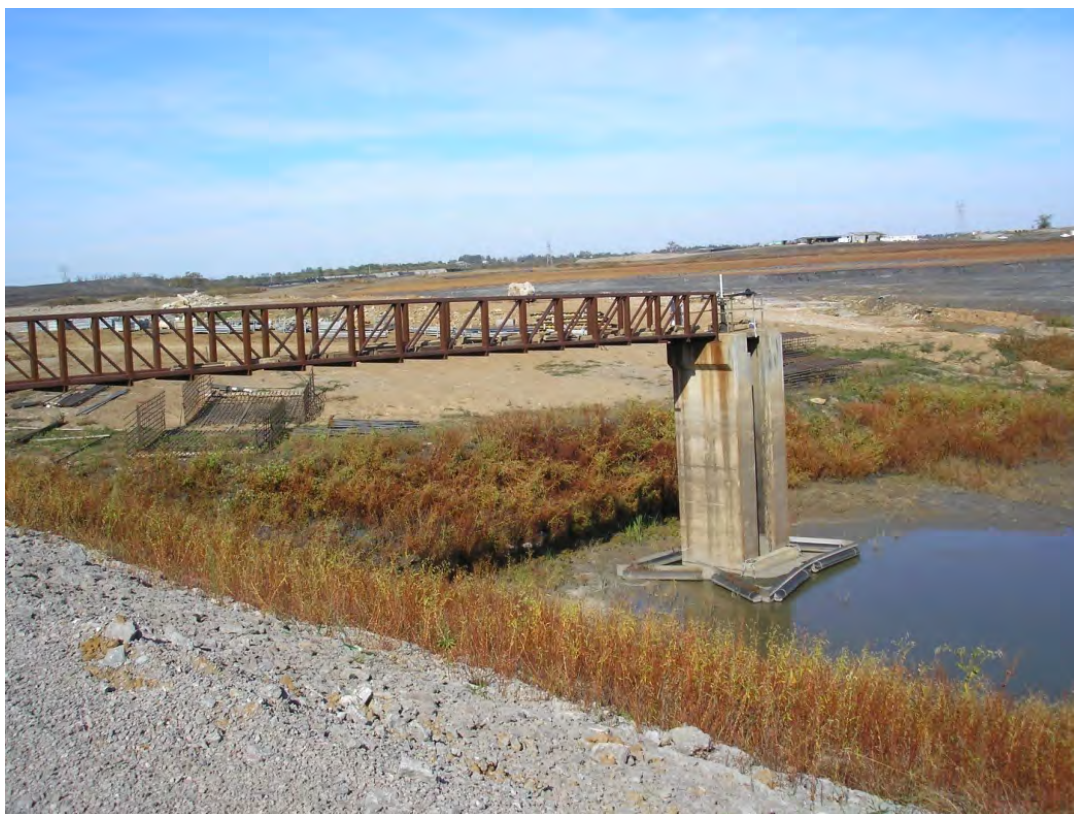
Figure 5.3.1-1. Existing Primary Spillway Structure.
