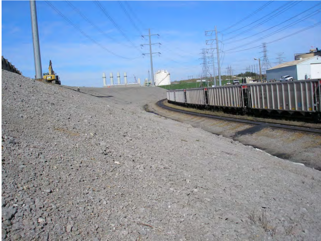
Figure 5.2.3-2. Downstream Slope at the Northeast Side of Impoundment
