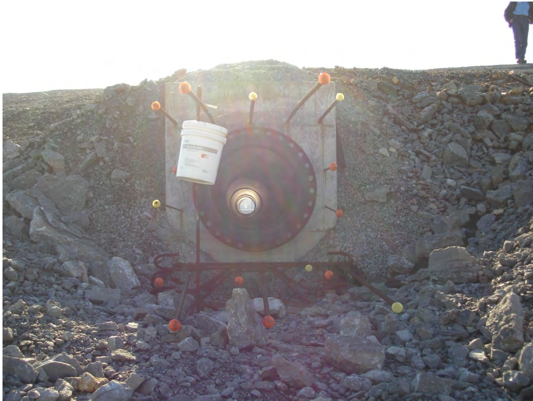
Figure 5.3.2-1. New Emergency Spillway from Reconfigured Main Fly Ash Pond to Auxiliary Fly Ash Pond (Discharge End Shown)
