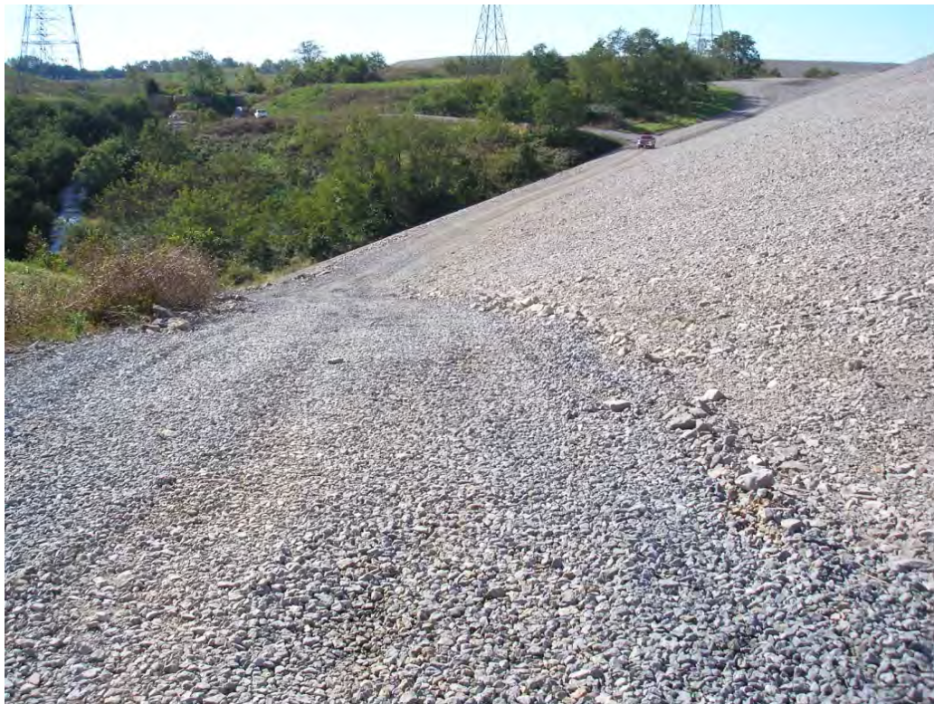
Figure 5.2.3-1. Downstream Slope at the Southeast Side of Impoundment
