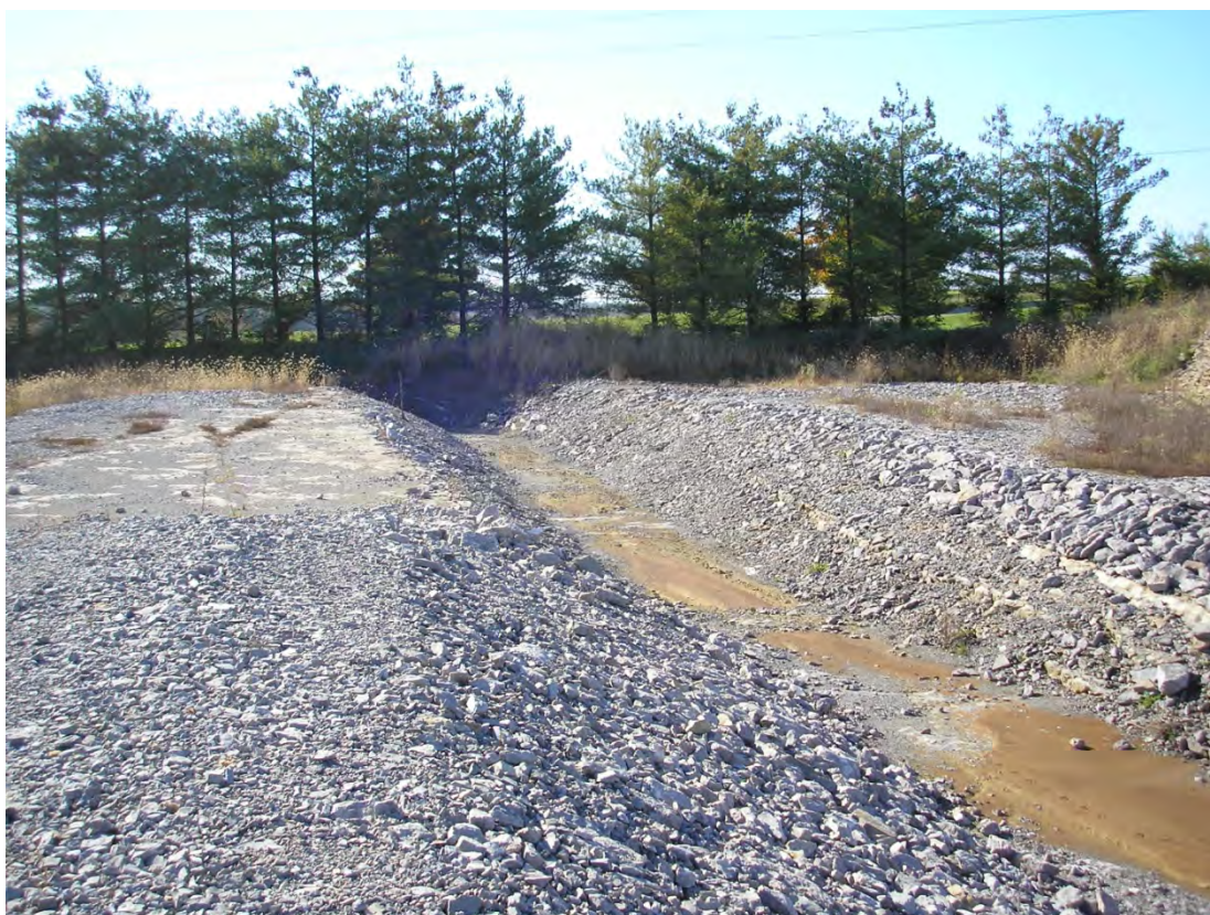
Figure 5.3.3-1. Emergency Spillway at the Southwest end of Dam.
