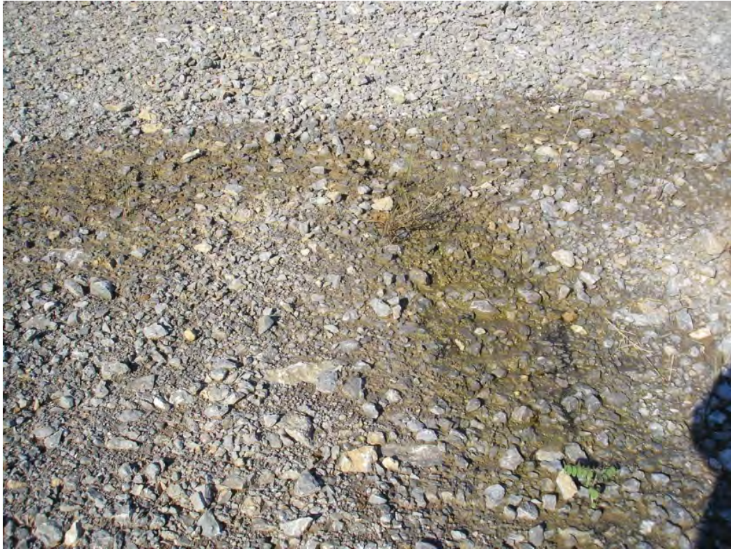
Figure 5.2.3-2. Small Seepage Area Southern Segment, Downstream Embankment.
