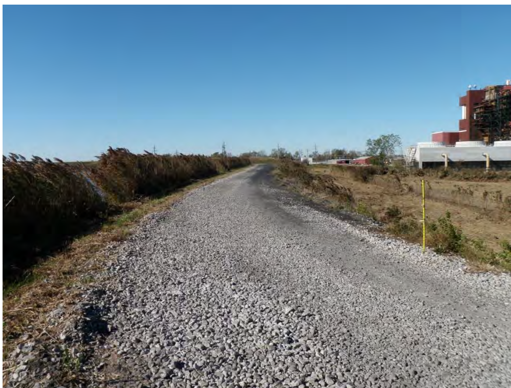
Photo 24: Upper Pond crest and downstream slope at inside corner looking west. Note heavy vegetation on upstream slope.
