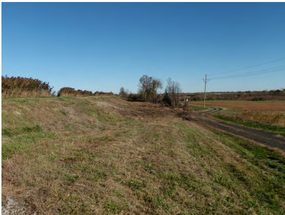
Photo 12: Upper Pond downstream slope and tree growth at southeast corner of pond looking north.
