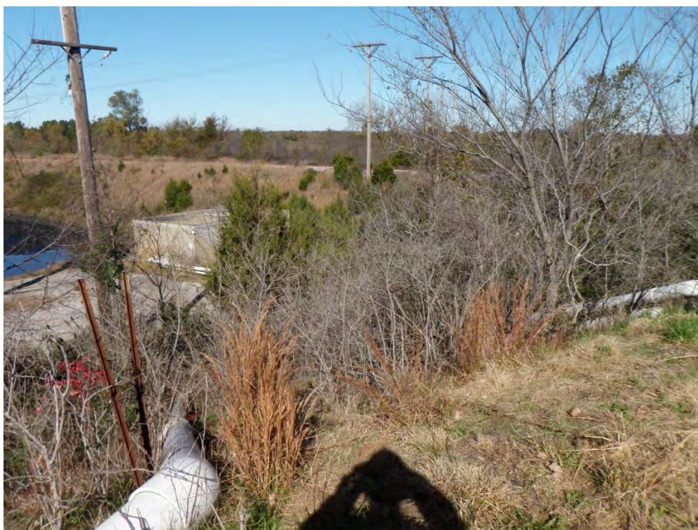
Photo 18: Upper Pond coal pile sump at northwest corner. Note sump discharge pipes aligned into Upper Pond.
