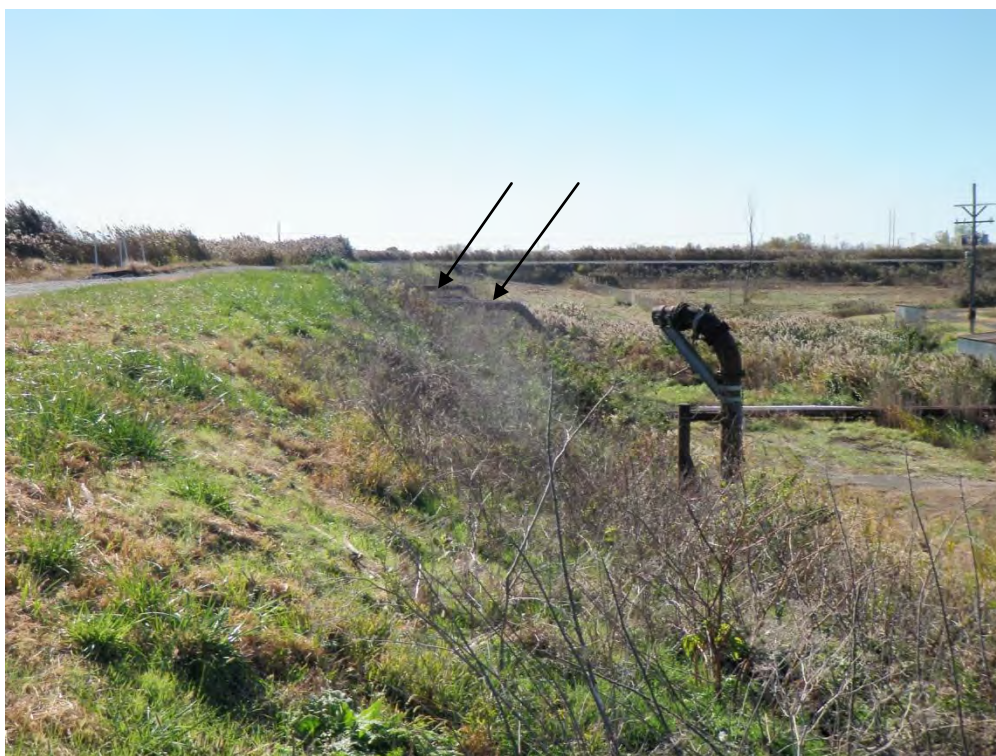
Photo 22: Upper Pond downstream slope where CCW discharge pipes (note arrows) cross through and continue to the Lower Pond.
