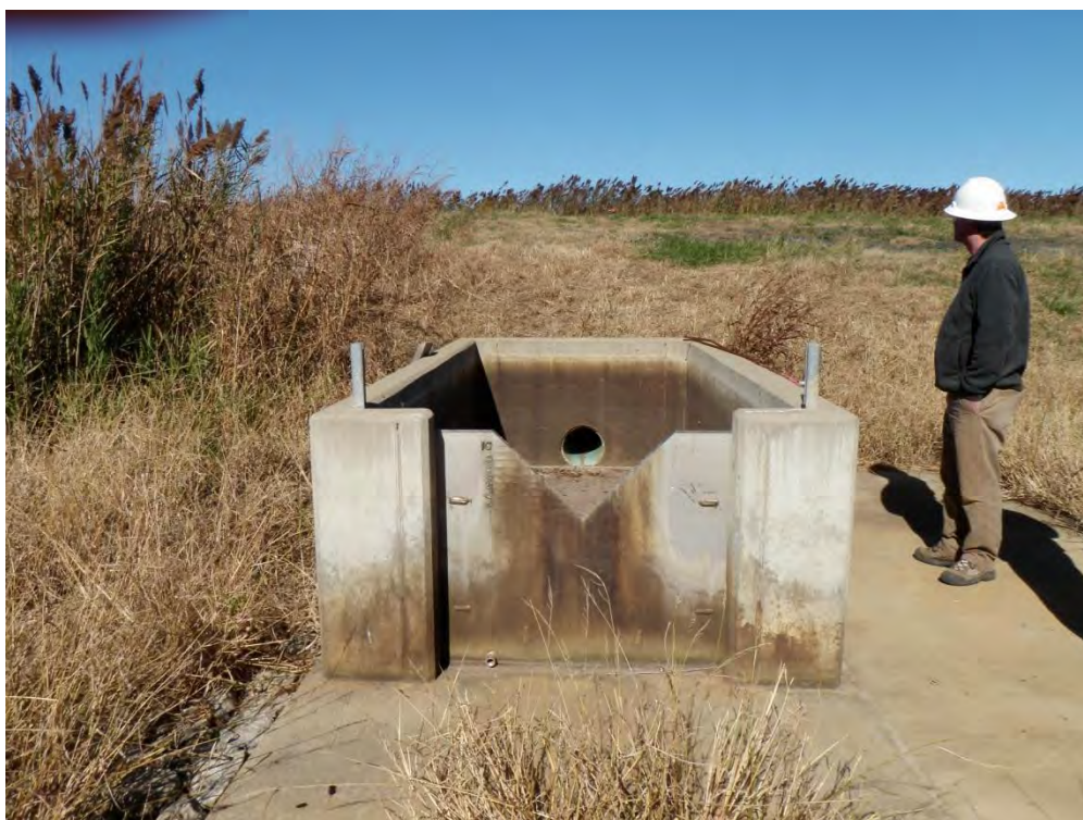
Photo 4: Lower Pond V-notch weir next to overflow spillway.
