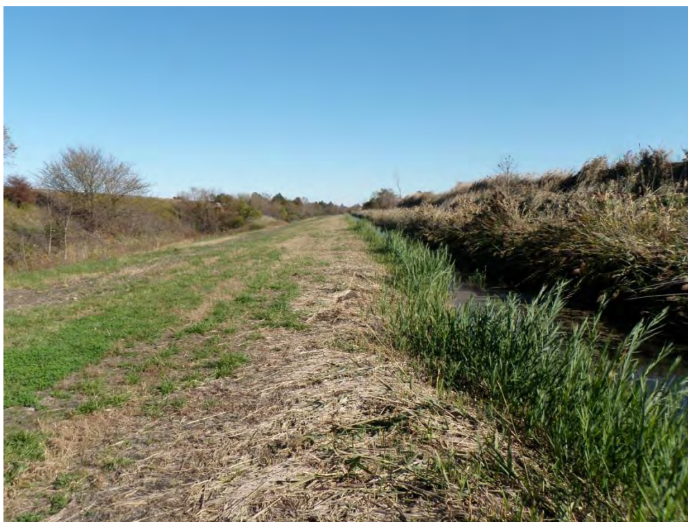
Photo 10: Lower Pond crest and interior perimeter ditch at northwest corner of pond looking east. Note ash pile built up to the right of the ditch.
