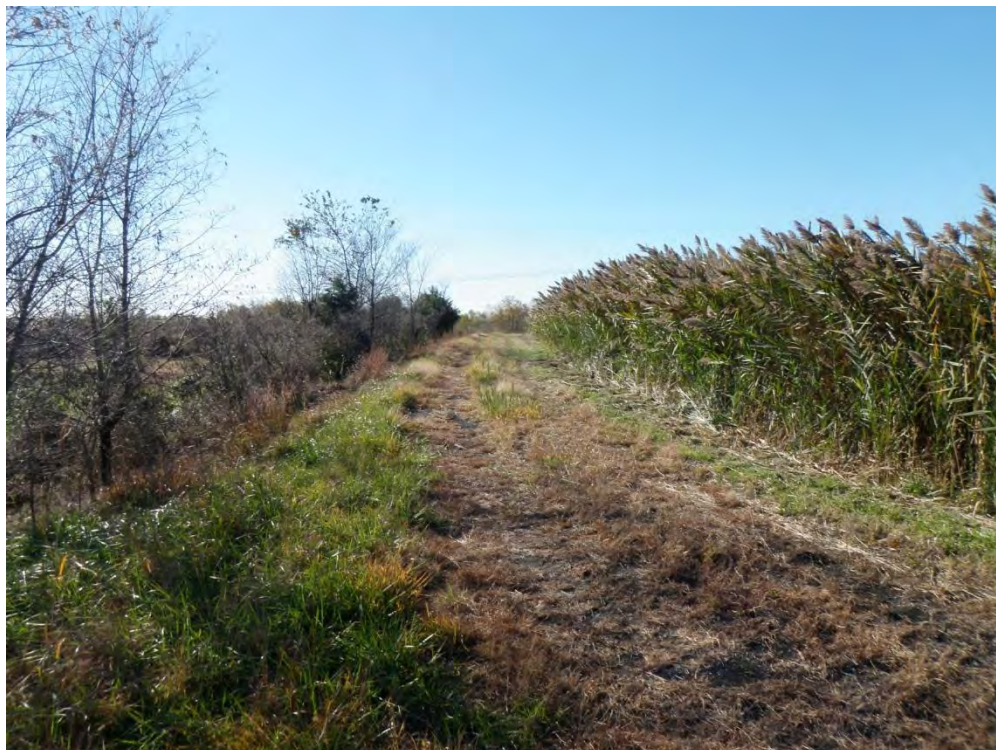
Photo 28: South Pond crest and downstream slope at northeast corner of pond looking south. Note heavy vegetation on upstream and downstream slopes.
