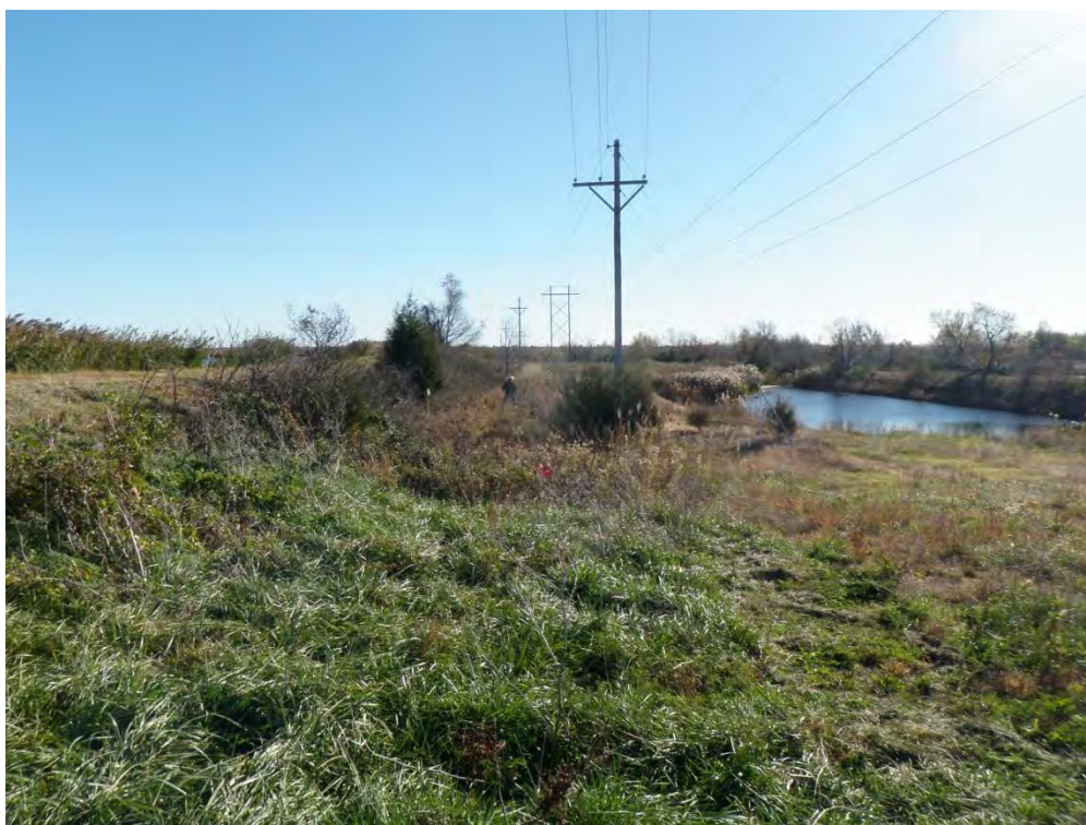
Photo 26: South Pond downstream slope at southwest corner looking east. Note heavy vegetation on downstream slope and standing water in excavated borrow area.
