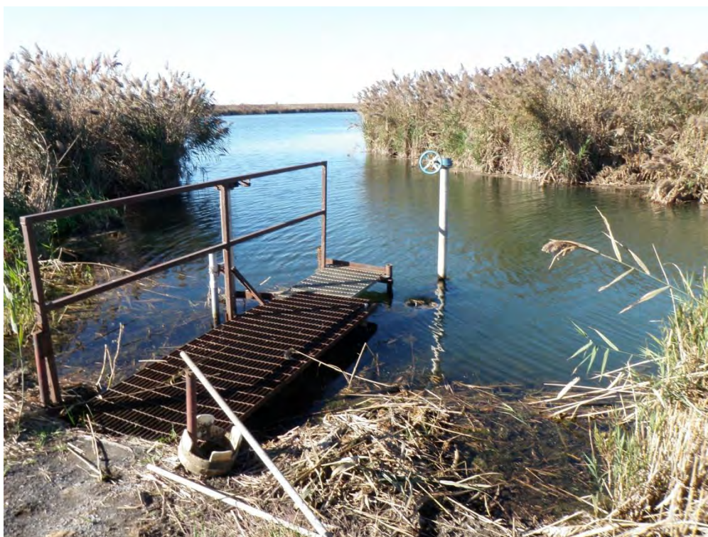
Photo 13: Upper Pond overflow drop inlet and outlet valve.
