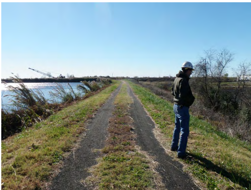
Photo 20: Upper Pond upstream and crest at northwest corner looking south. Note tree growth on downstream slope.
