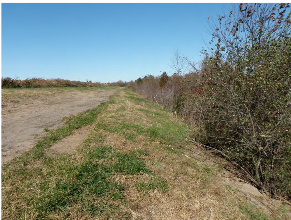
Photo 6: Lower Pond downstream slope at southeast corner of pond looking north. Note heavy tree growth at the downstream toe.
