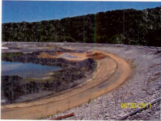
Recompaction of Interior Slopes to Repair Erosion on Ash Pond No. 4
