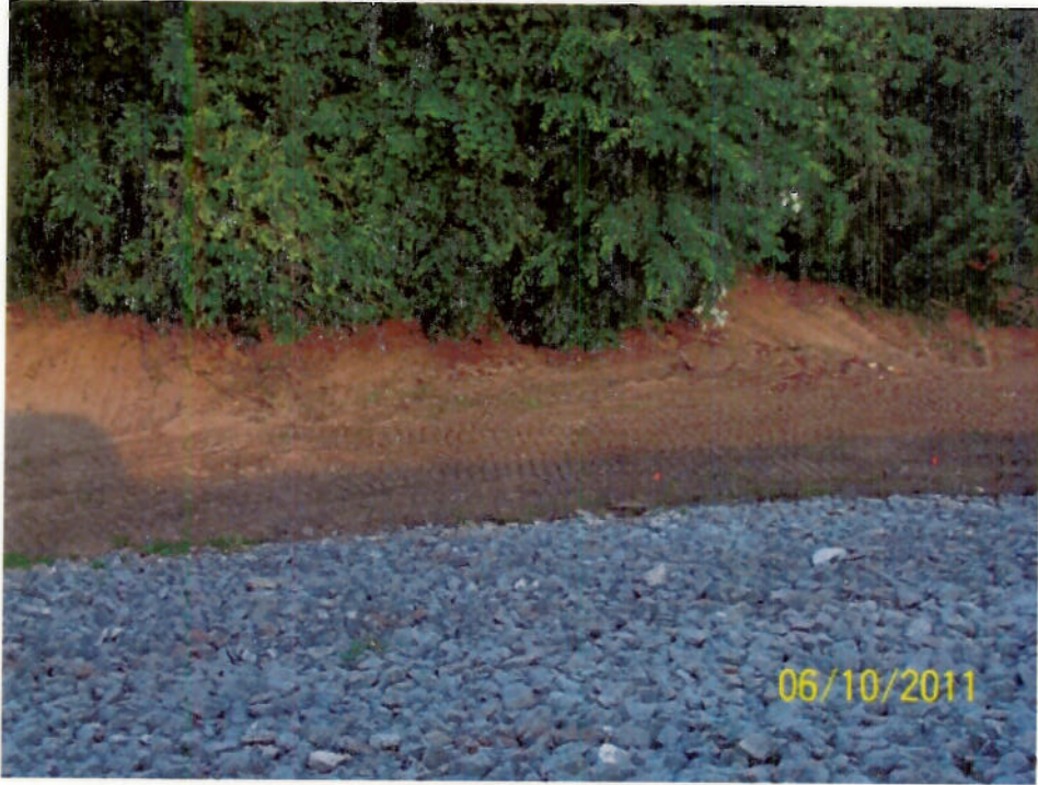
Re-grade to Achieve Positive Drainage Away from Pond No. 4 Dam
