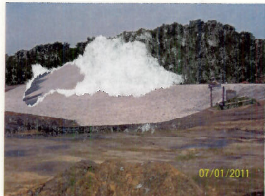
Finished Interior Slope at Ash Pond No. 4
