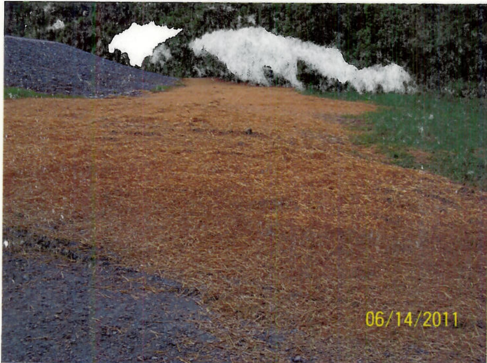
Re-grade to Achieve Positive Drainage Away from Pond No. 4 Dam
