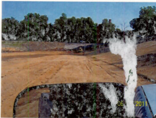
Preparing Subgrade for Liner at Ash Pond No. 4
