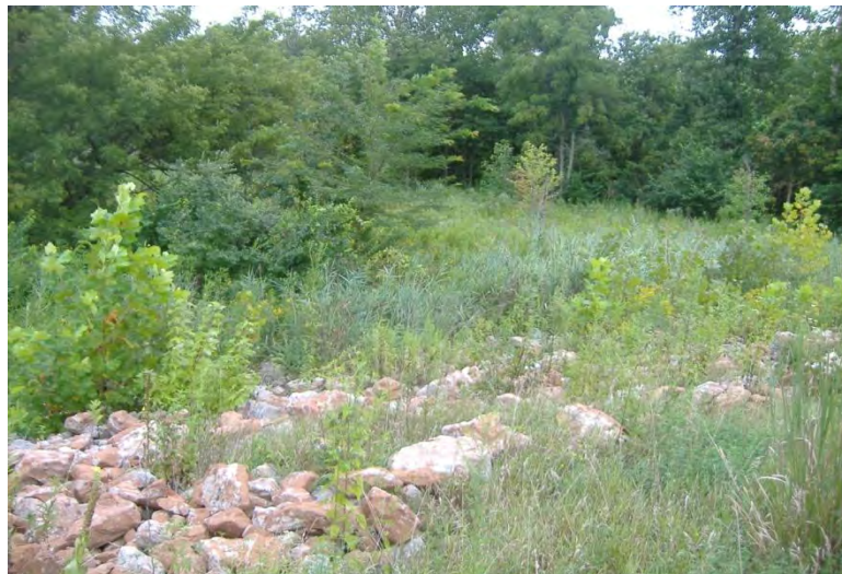
Figure 5.3.3-2: Photograph of Riprap and Vegetation at the Toe of the East Ash Pond System Embankment.
