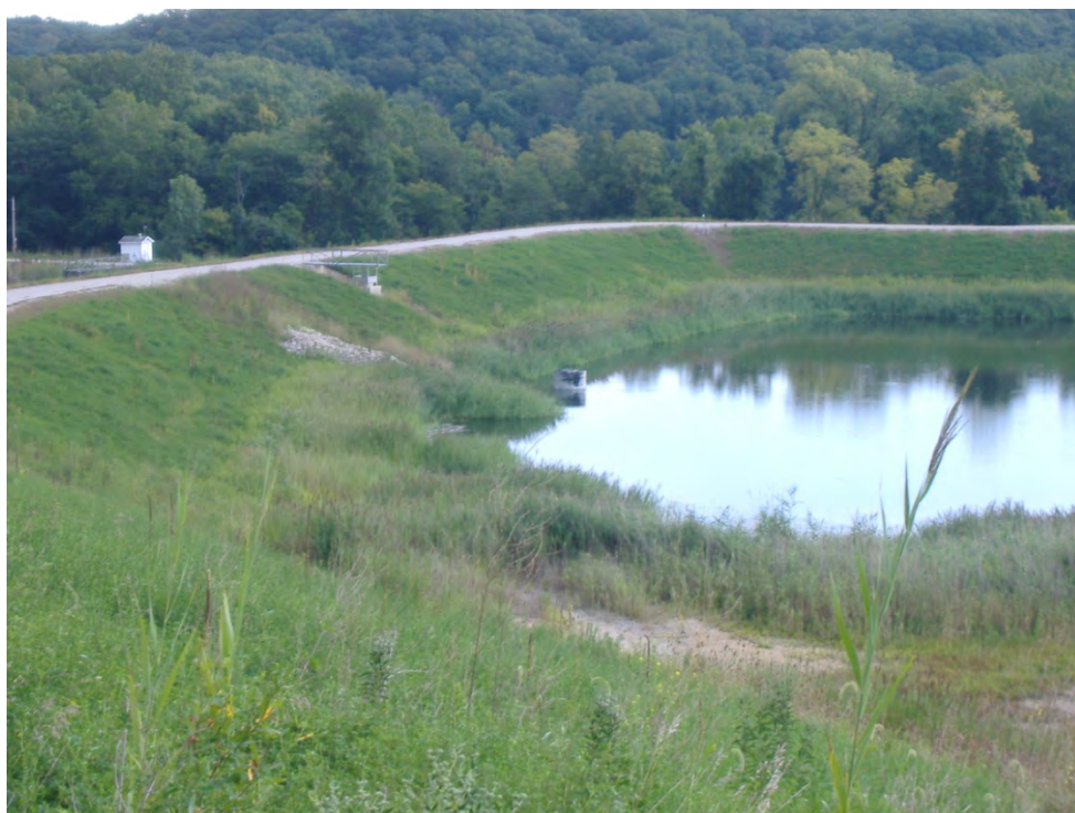
Primary Pond Typical Upstream Slope
