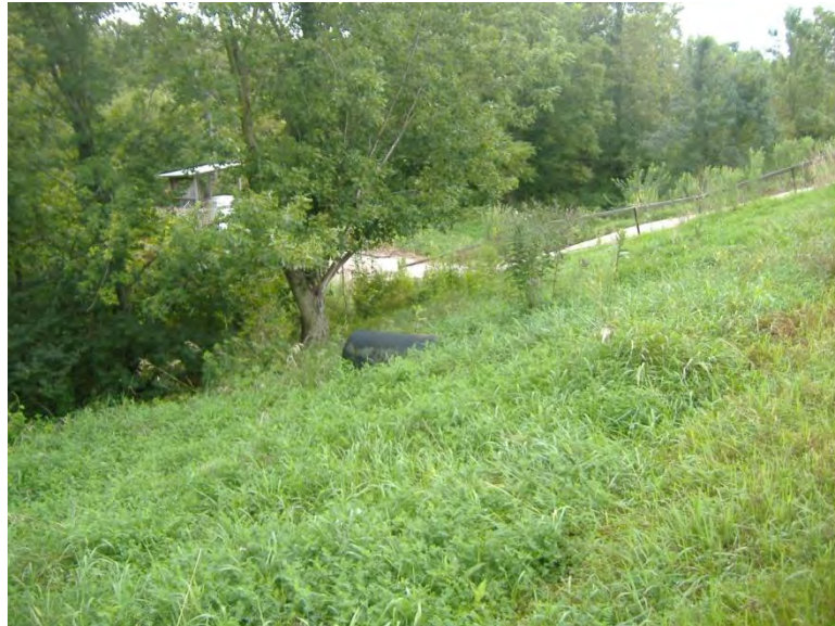
Figure 5.2.3-2: Photograph of Large Tree Near Emergency Spillway on North Ash Pond System Embankment.
