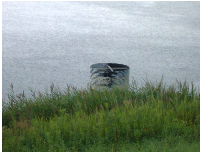
Figure 5.4.1-2: Photograph of the East Ash Pond System Primary Outfall Structure.
