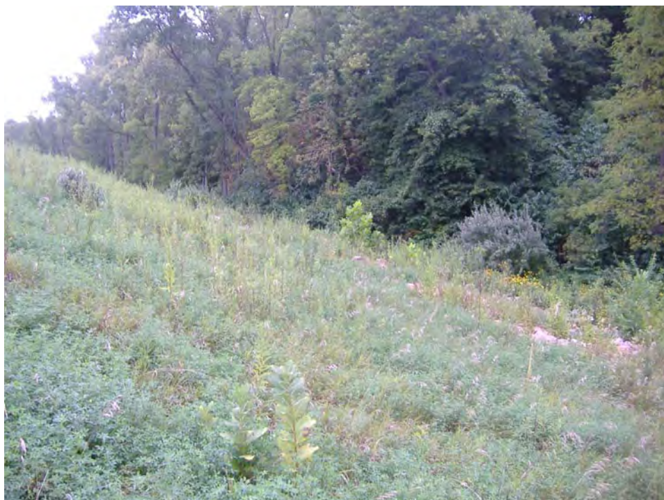
Primary Pond Typical Downstream Slope
