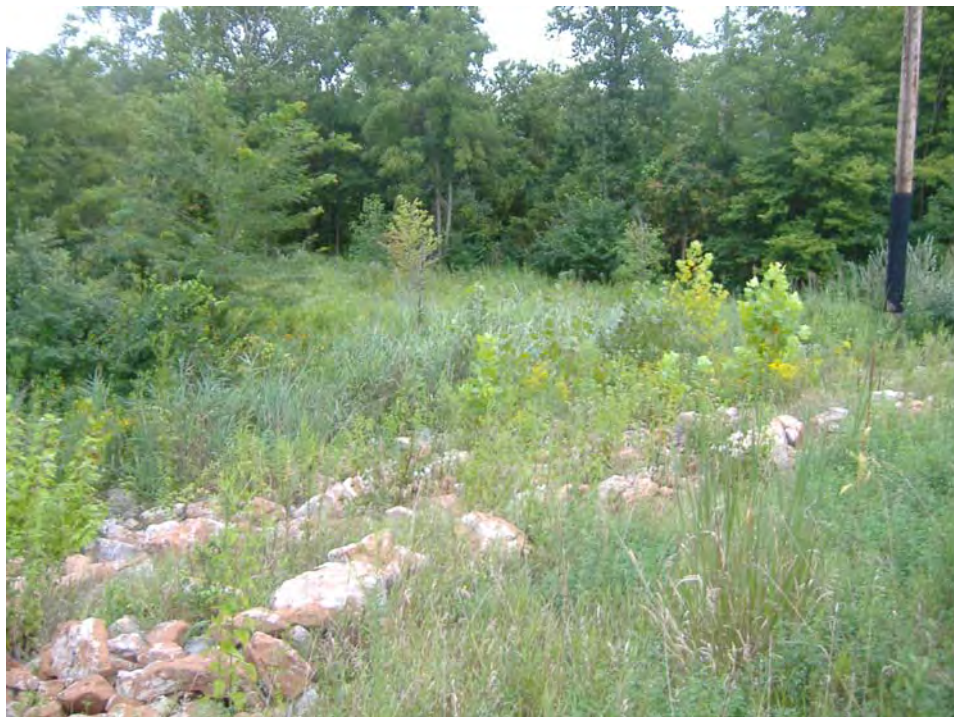
Primary Pond Rip Rap on Downstream Toe
