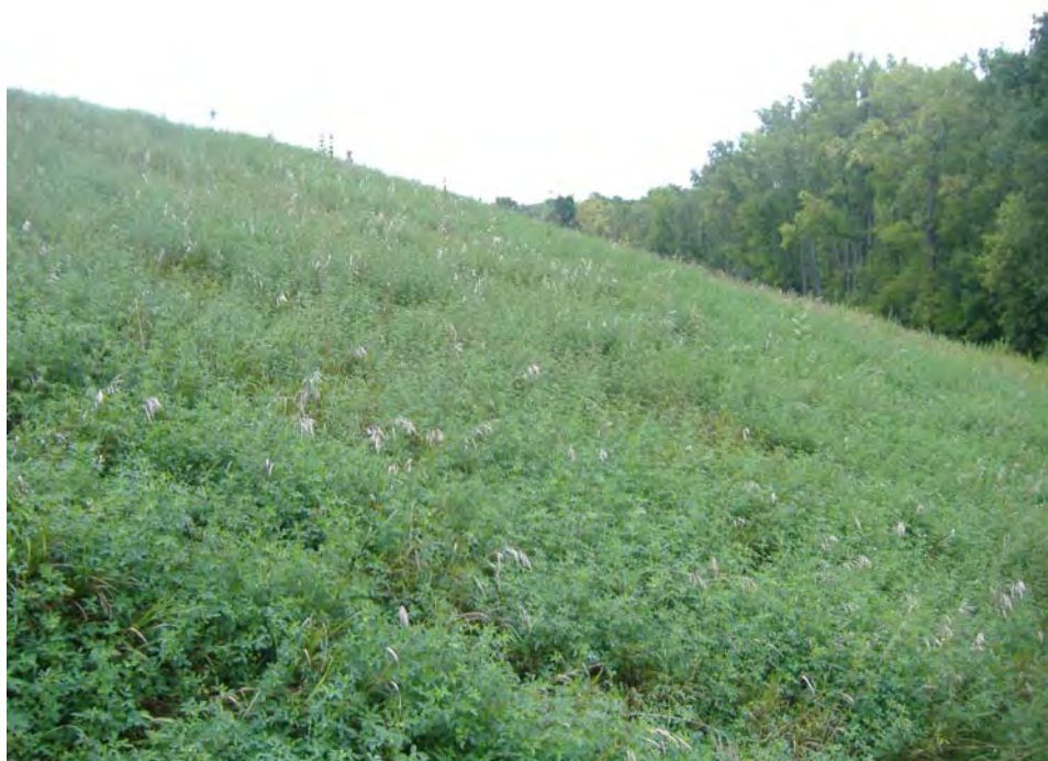
Primary Pond Typical Downstream Slope
