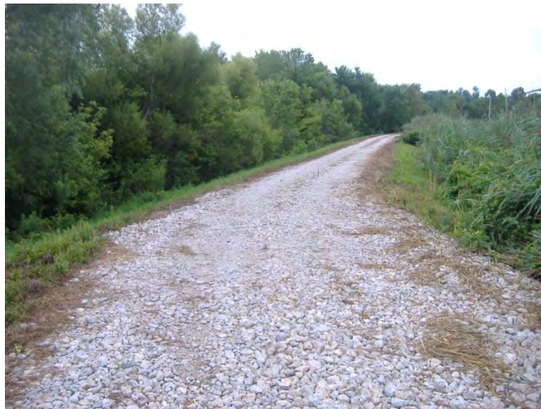
Figure 5.2.1-1: Photograph of Crest of North Ash Pond System Embankment
