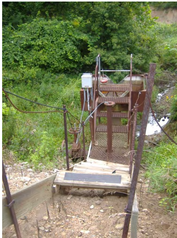
Figure 5.4.1-1: Photograph of the North Ash Pond System Overflow Structure.
