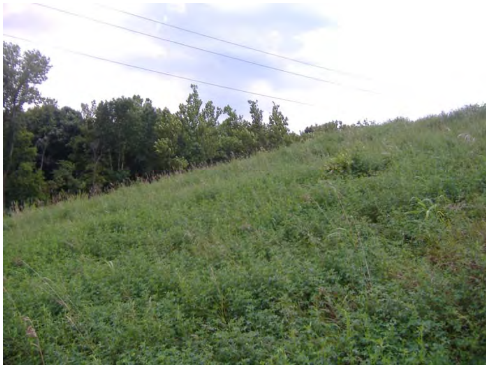
Primary Pond Typical Downstream Slope
