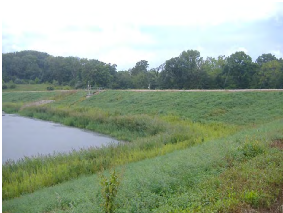
Primary Pond Typical Upstream Slope
