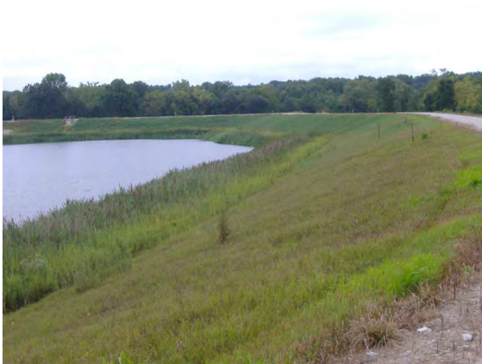
Primary Pond Typical Upstream Slope
