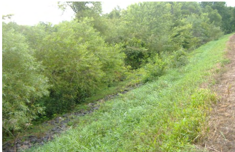
Figure 5.2.3-3: Photograph of Riprap and Dense Vegetation at the Toe of the North Ash Pond System Embankment.
