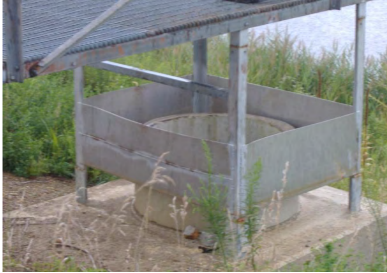
Figure 5.4.1-3: Photograph of the East Ash Pond System Emergency Outfall Pipe.
