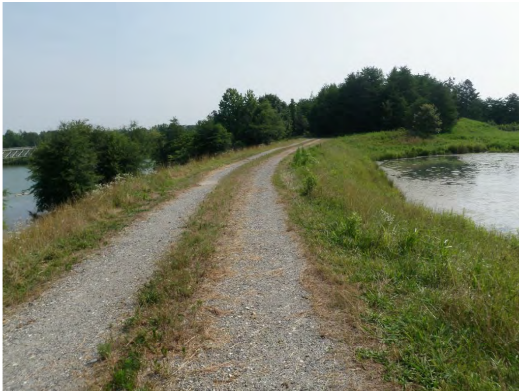
Photo 20- Divider Dike: Crest.
