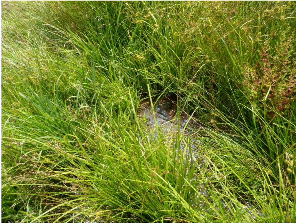
Photo 19 – Secondary Ash Basin Dam: Flowing water in seepage area.
