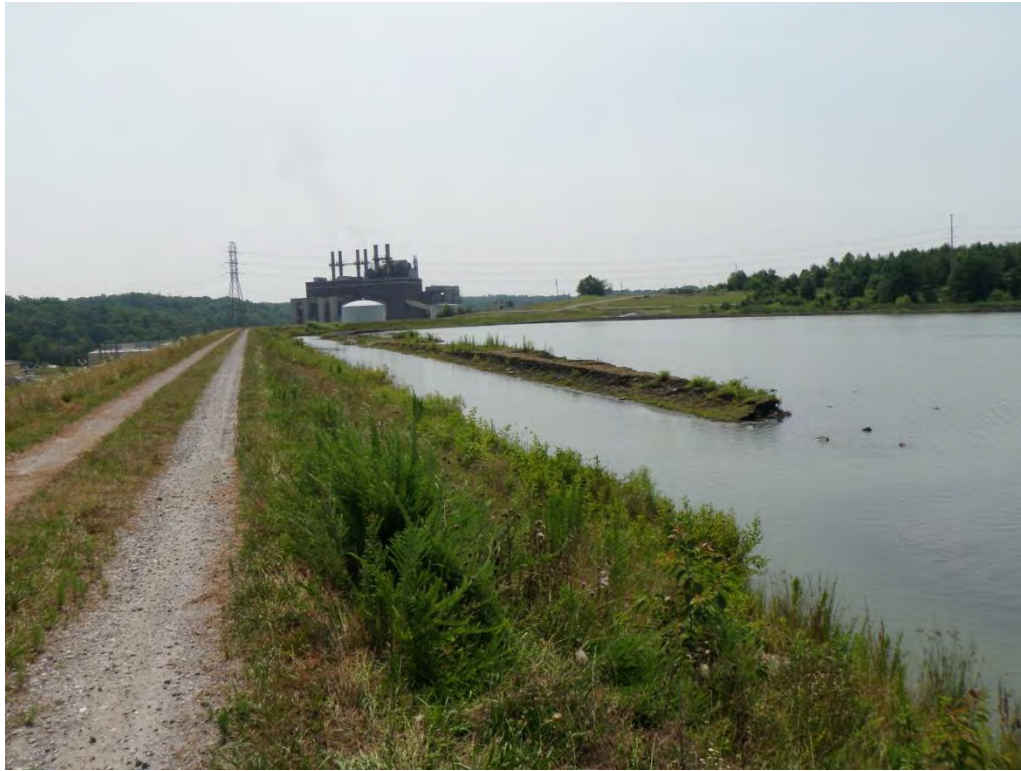
Photo 7 – Primary Active Ash Pond Dam: Upstream face and channel to decant pipe (looking east).
