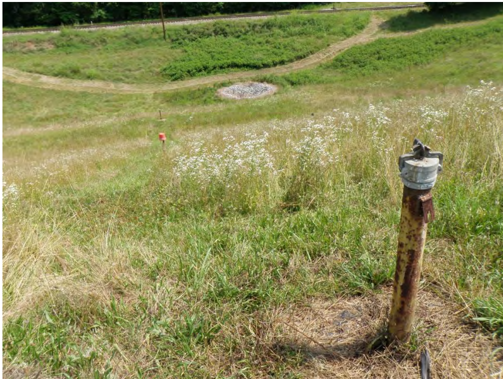
Photo 6 – Primary Active Ash Pond Dam: Piezometers L-4, L-5 and L-6 and toe drain inlet.
