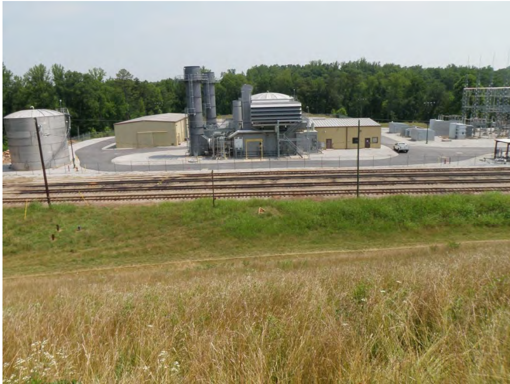
Photo 5 – Primary Active Ash Pond Dam: Plant buildings downstream.
