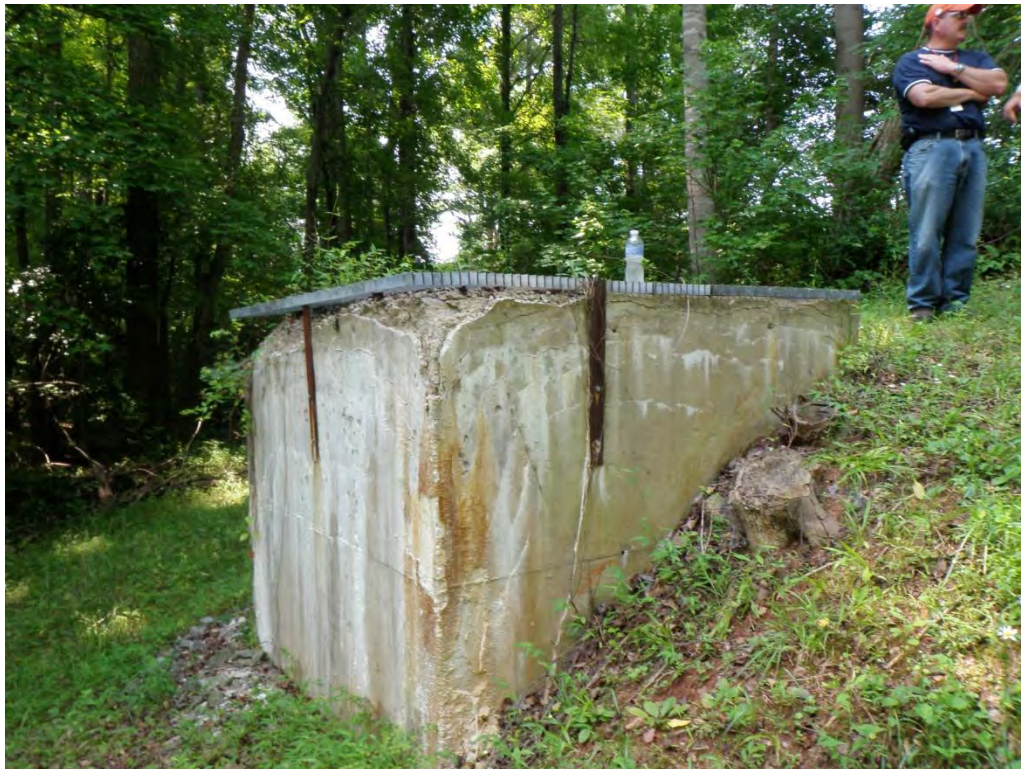
Photo 26 – Secondary Ash Basin outlet works – drop box downstream of dam. Note spalling.
