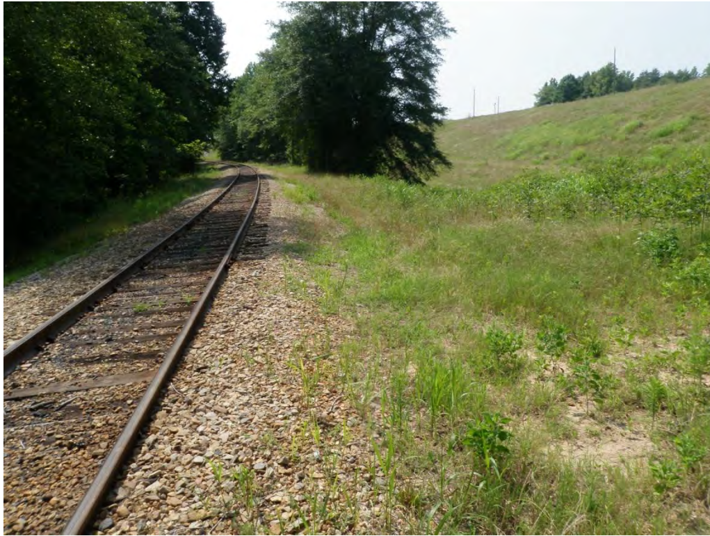
Photo 15 – Secondary Ash Basin Dam: Railroad embankment downstream of toe.
