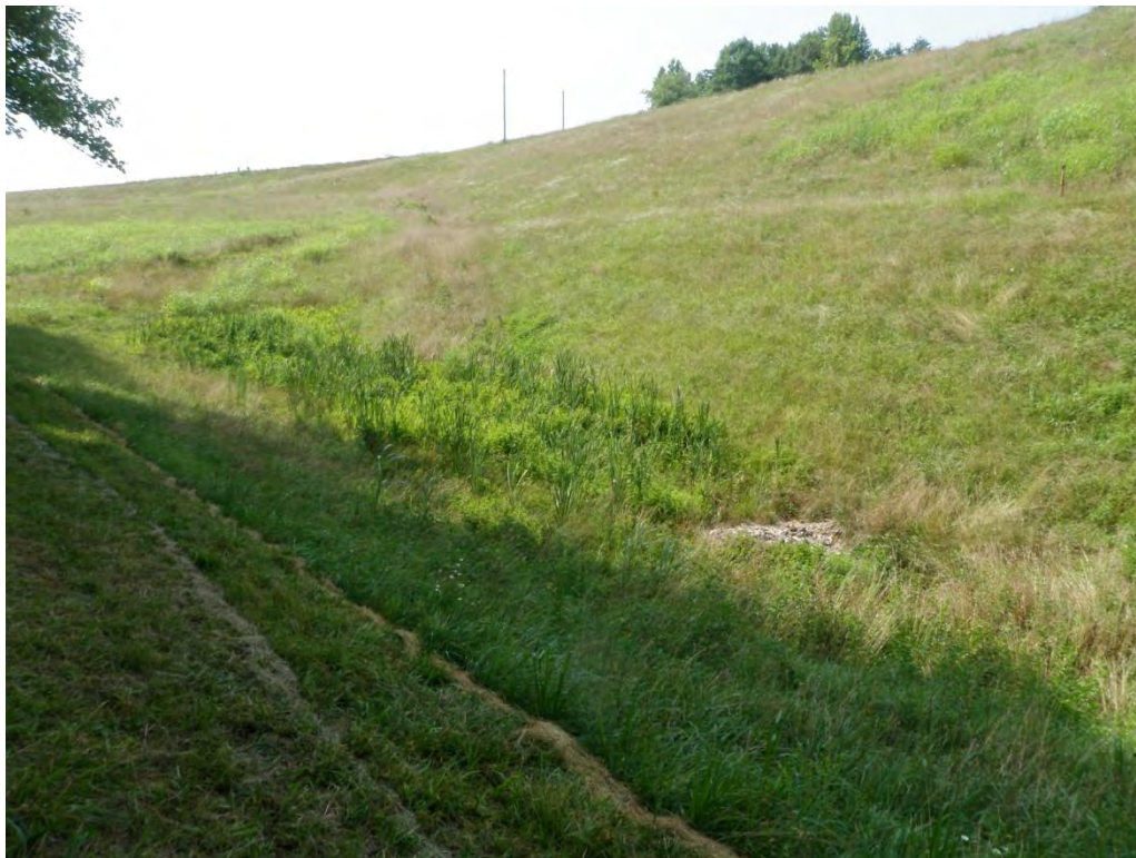
Photo 18 – Secondary Ash Basin Dam: Seepage area downstream of right abutment. Note vegetation.
