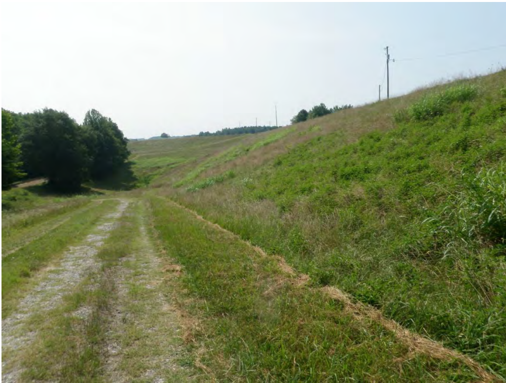
Photo 14 – Secondary Ash Basin Dam: Downstream slope from left abutment.
