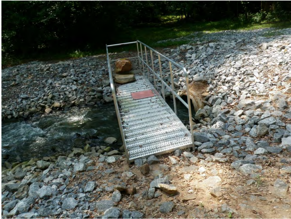
Photo 27 – Secondary Ash Basin outlet works – discharge conduit.
