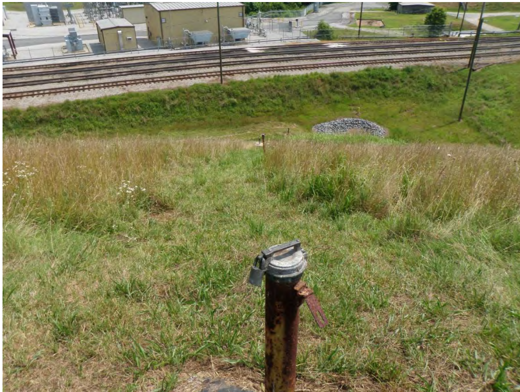
Photo 4 – Primary Active Ash Pond Dam: Piezometers L-1, L-2 and L-3 and toe drain inlet.
