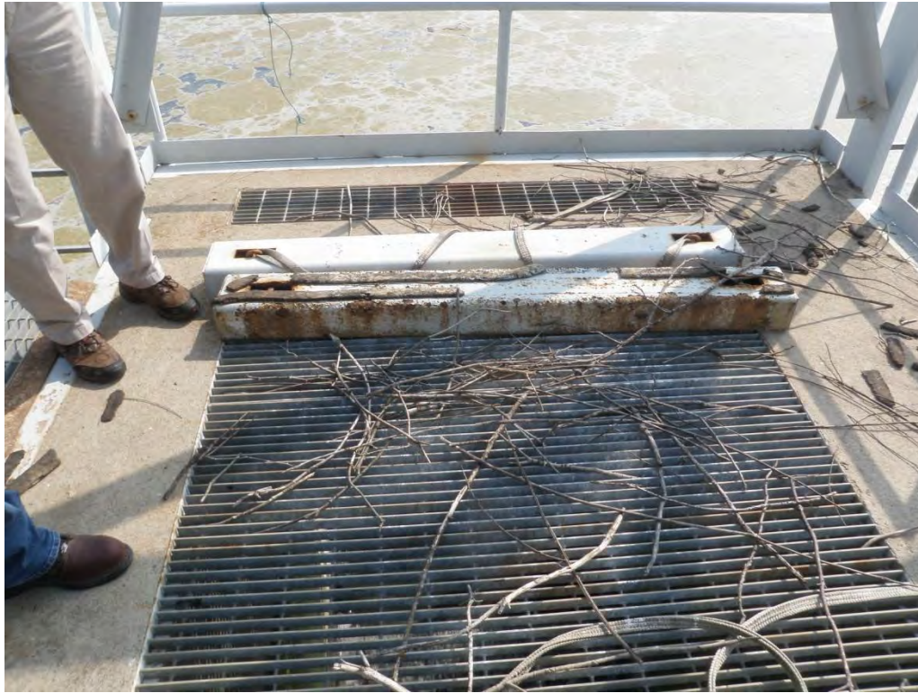
Photo 23 –Primary Active Ash Pond outlet structure – stop logs.
