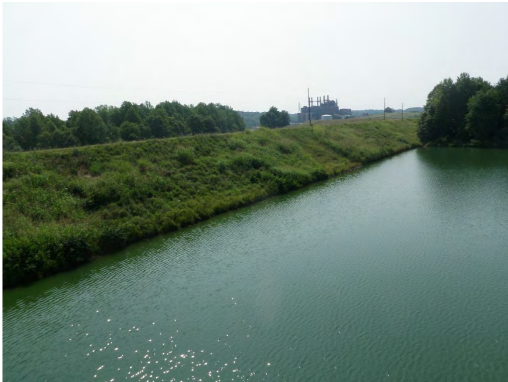
Photo 12 – Secondary Ash Basin Dam: Upstream slope looking toward right abutment.
