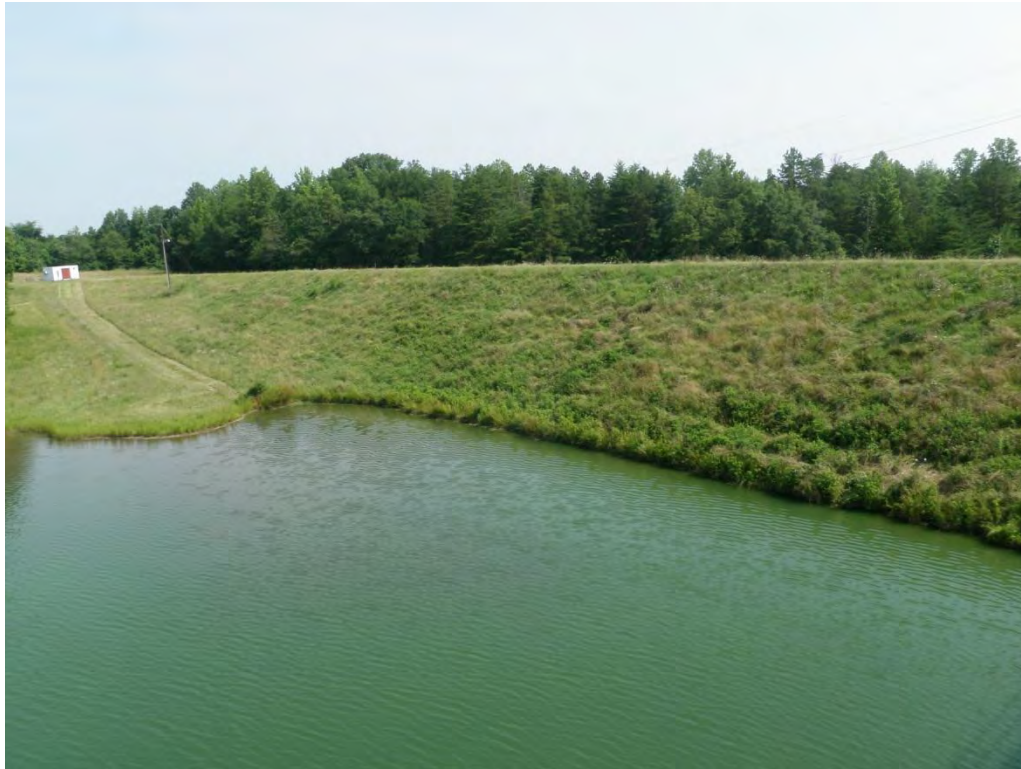
Photo 11 – Secondary Ash Basin Dam: Upstream slope and left abutment.
