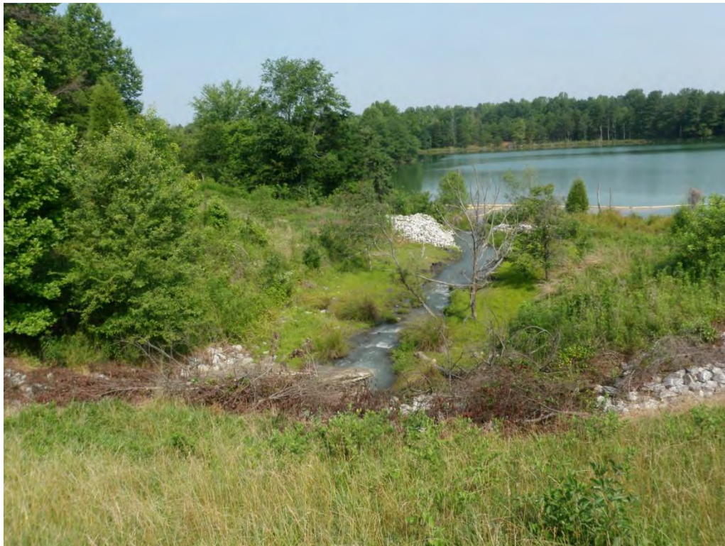
Photo 24 –Primary Active Ash Pond outlet structure – channel to Secondary Ash Basin.
