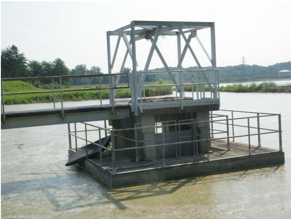
Photo 22 –Primary Active Ash Pond outlet structure.
