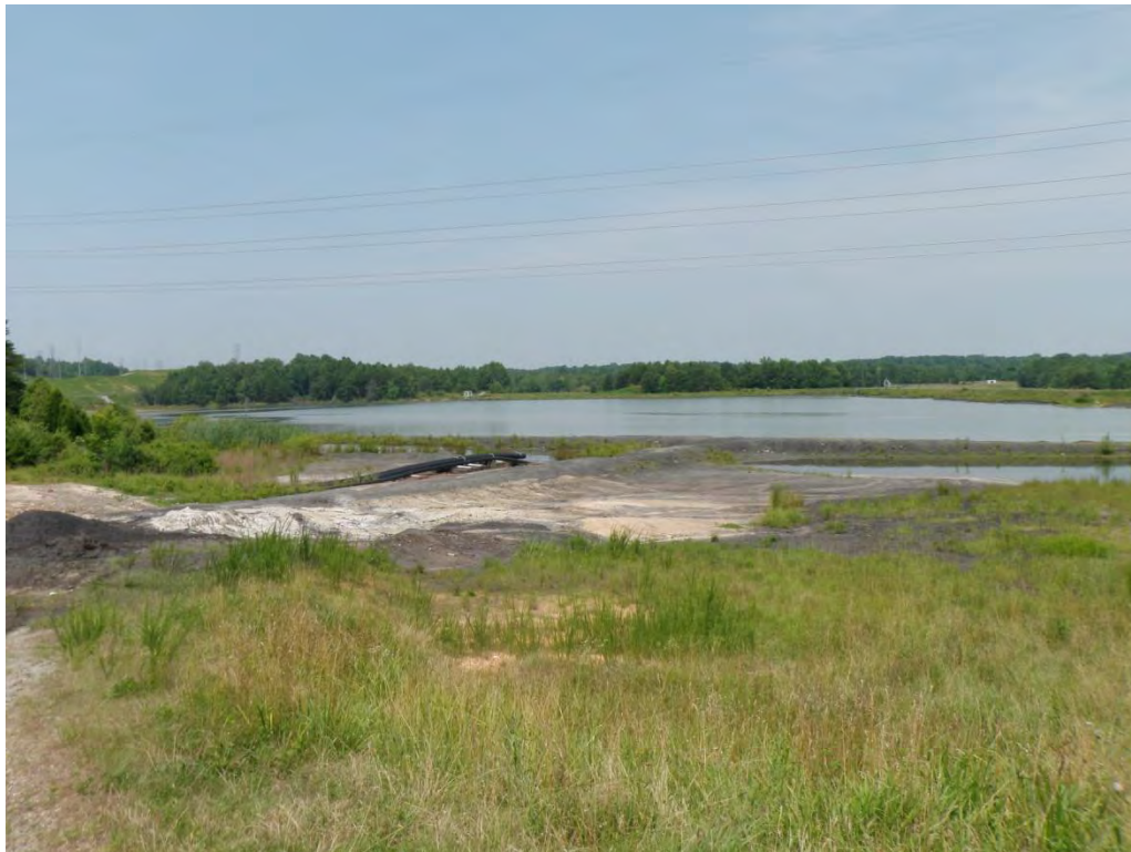
Photo 2 – Primary Active Ash Pond Dam: Overview from right abutment.
