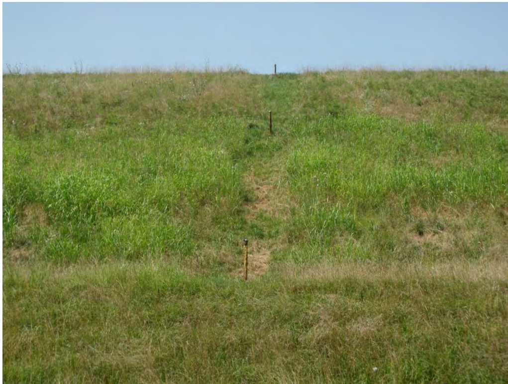
Photo 16 – Secondary Ash Basin Dam: Piezometers L-7, L-8 and L-9.
