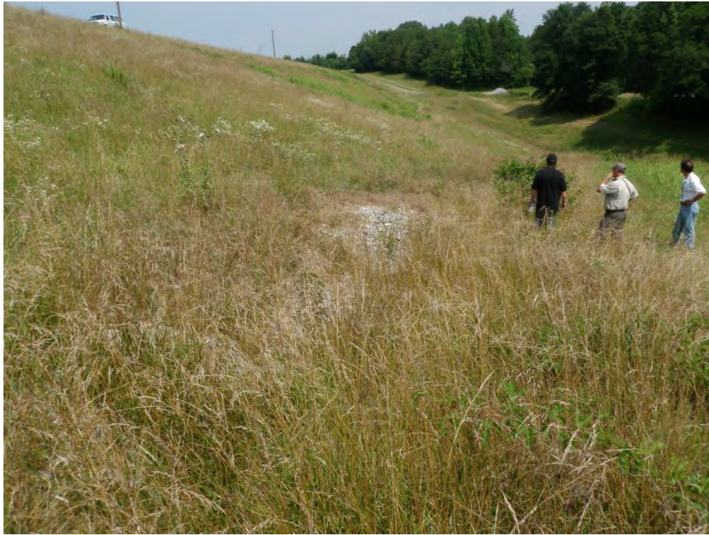
Photo 17 – Secondary Ash Basin Dam: Downstream face from left abutment. Note riprap along abutment contact.
