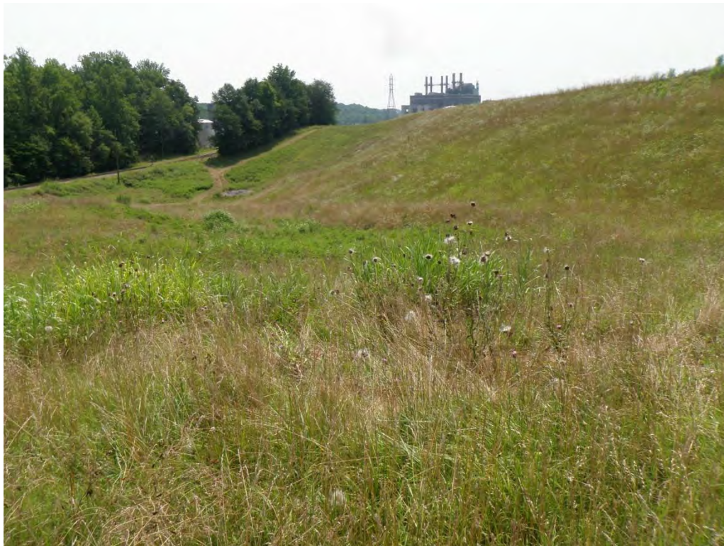
Photo 8 – Primary Active Ash Pond Dam: downstream face from left abutment.
