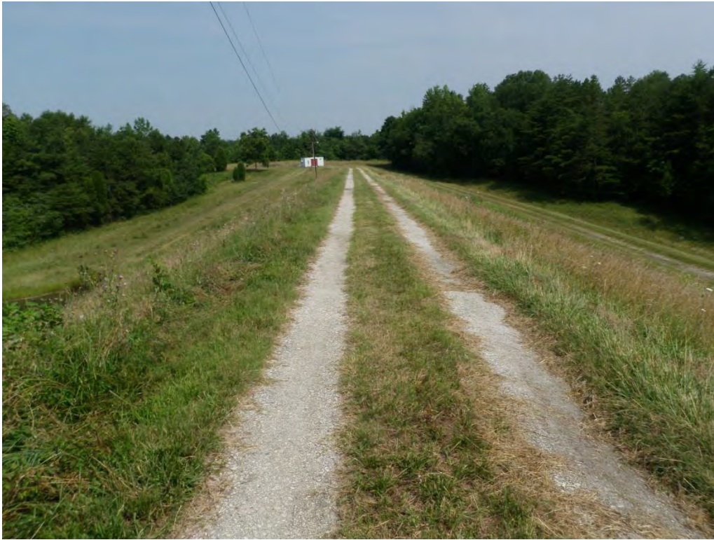
Photo 13 – Secondary Ash Basin Dam: Crest, looking west.
