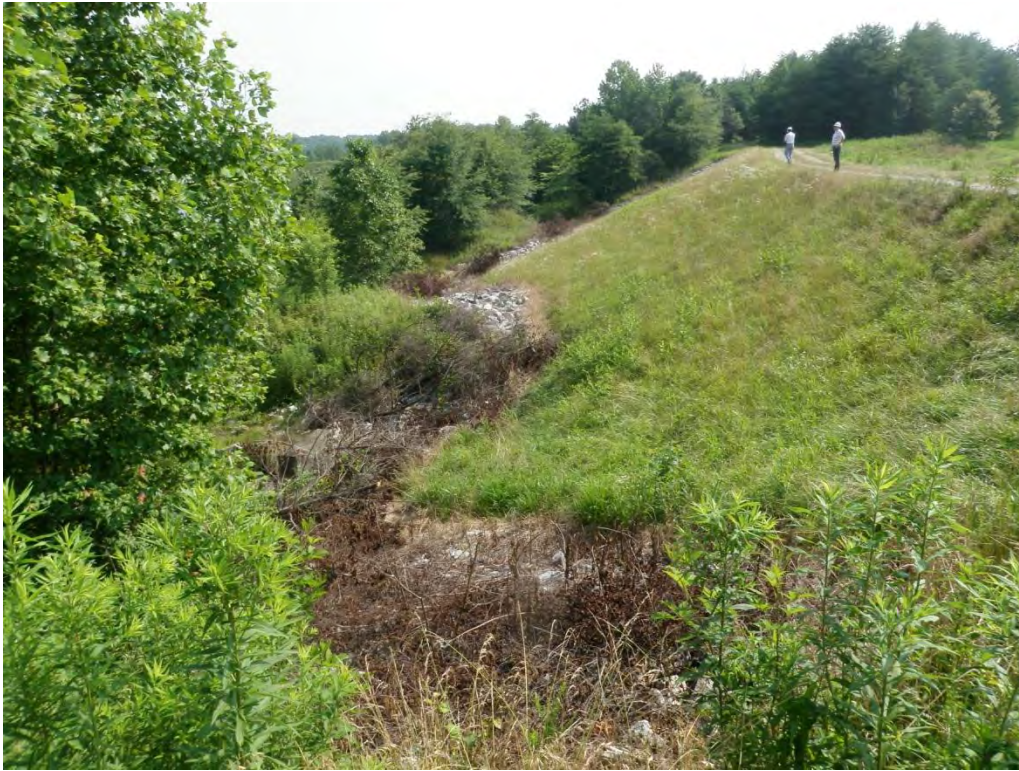
Photo 21 –Divider Dike: Downstream slope.
