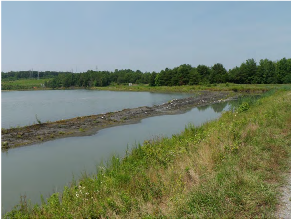
Photo 3 – Primary Active Ash Pond Dam: upstream slope and channel to decant pipe (looking west).
