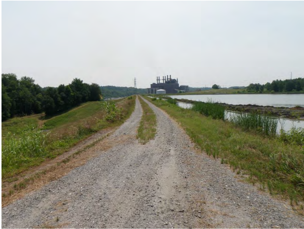
Photo 9 – Primary Active Ash Pond Dam: Crest from left abutment.
