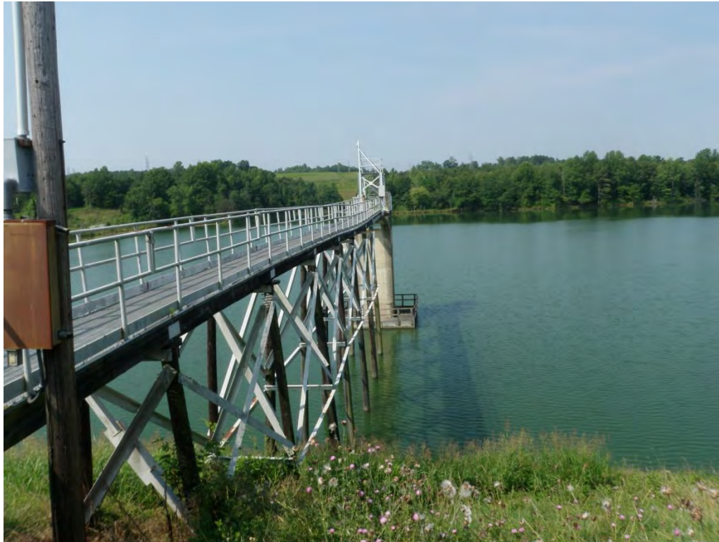
Photo 25 – Secondary Ash Basin outlet structure and bridge.
