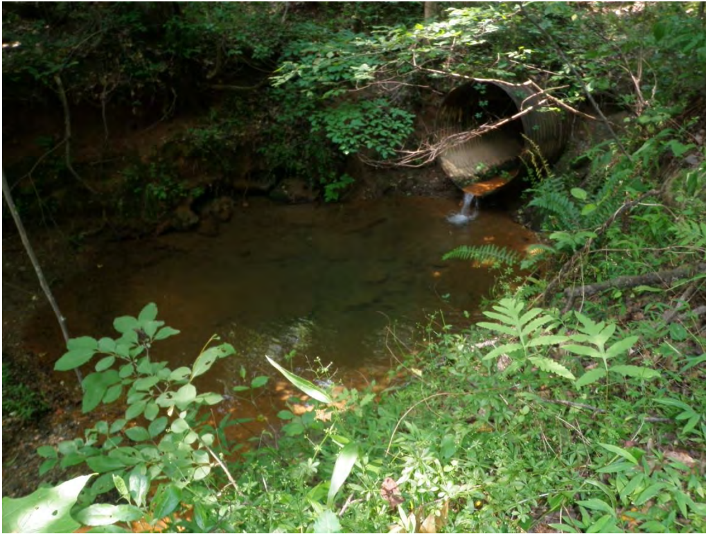
Photo 29 – Secondary Ash Basin toe drain outlet.
