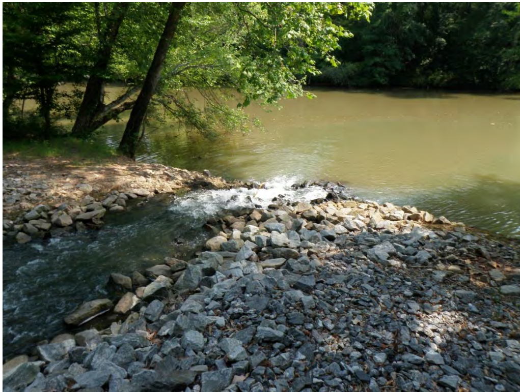
Photo 28 – Secondary Ash Basin outlet works – discharge channel to Saluda River.
