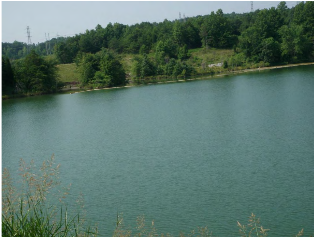
Photo 10 – Secondary Ash Basin: Looking across pond to divider dike.
