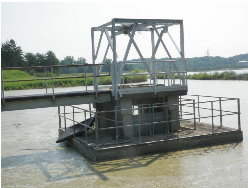
Photo 22 –Primary Active Ash Pond outlet structure.
