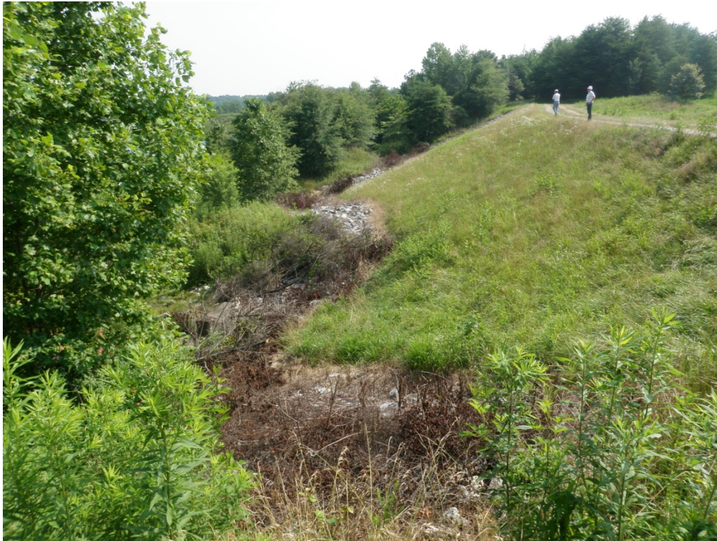
Photo 21 –Divider Dike: Downstream slope.
