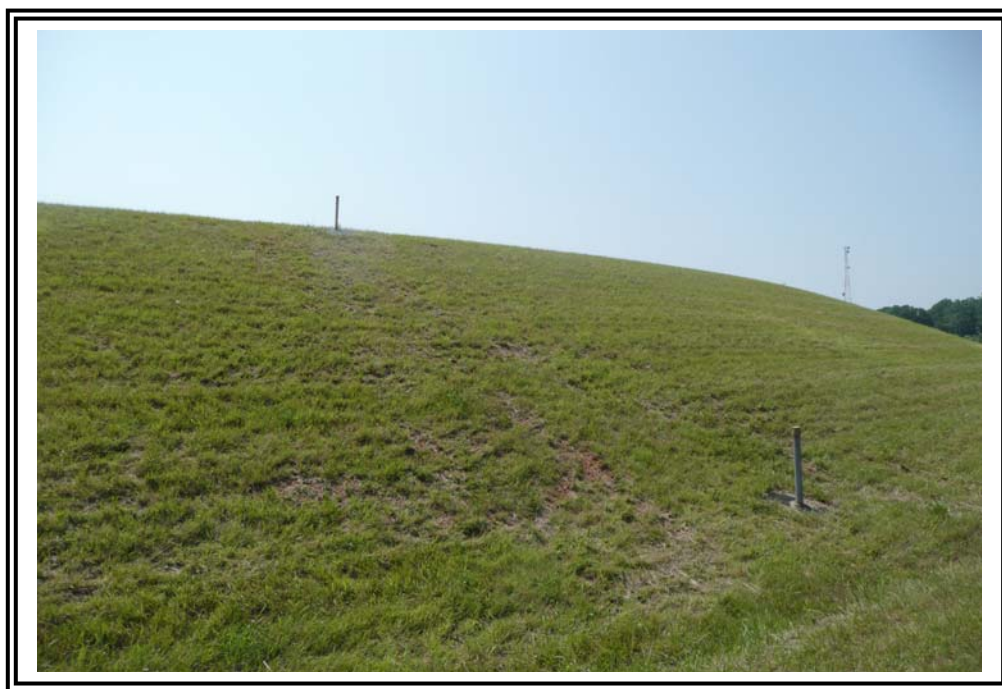
Downstream Slope of New Dike looking south. Note sparse grass coverage in some areas.
