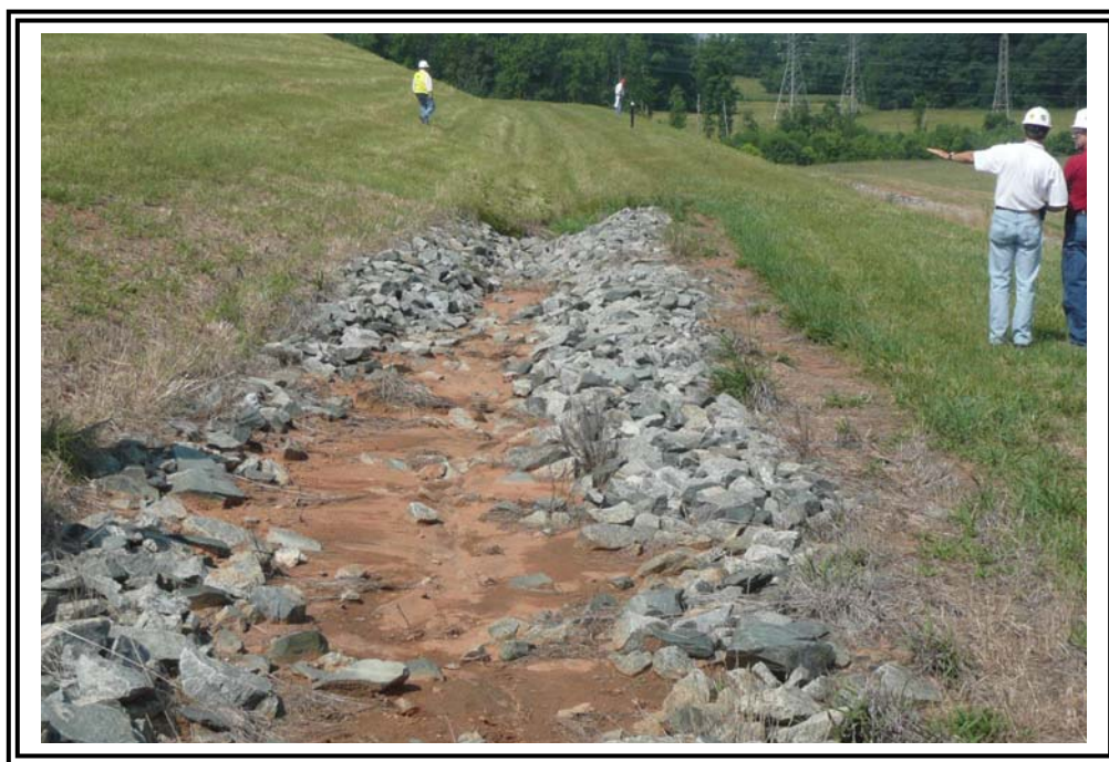
Drainage swale at north end of upper bench clogged with silt.
