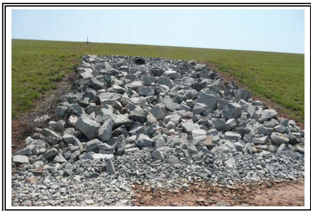
Repair area where surface runoff was causing sloughing from Upper Bench to Lower Bench. Repair was completed between 1993 and 1998 based on publically available aerial photos.
