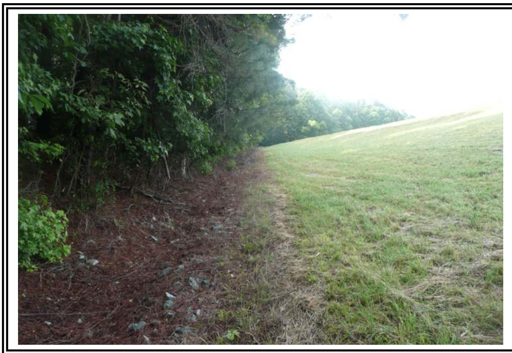
Downstream slope east of the outlet structure, looking east. Note: Rip rap is groin drainage swale. Duke Energy uses herbicide to control vegetation in rip rap.
