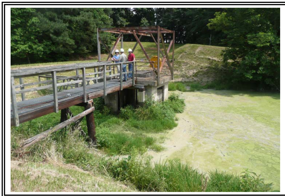
Basin 2 outlet control structure. Vegetation at base of tower and access bridge is on deposited ash.
