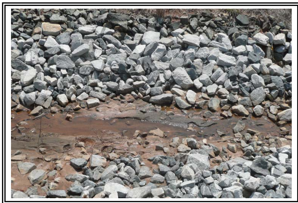
Closeup of toe drain seepage at New Dike. Water was flowing clear. Reportedly Duke Energy is in the process of discussing installation of a seepage monitoring system with an outside consultant.
