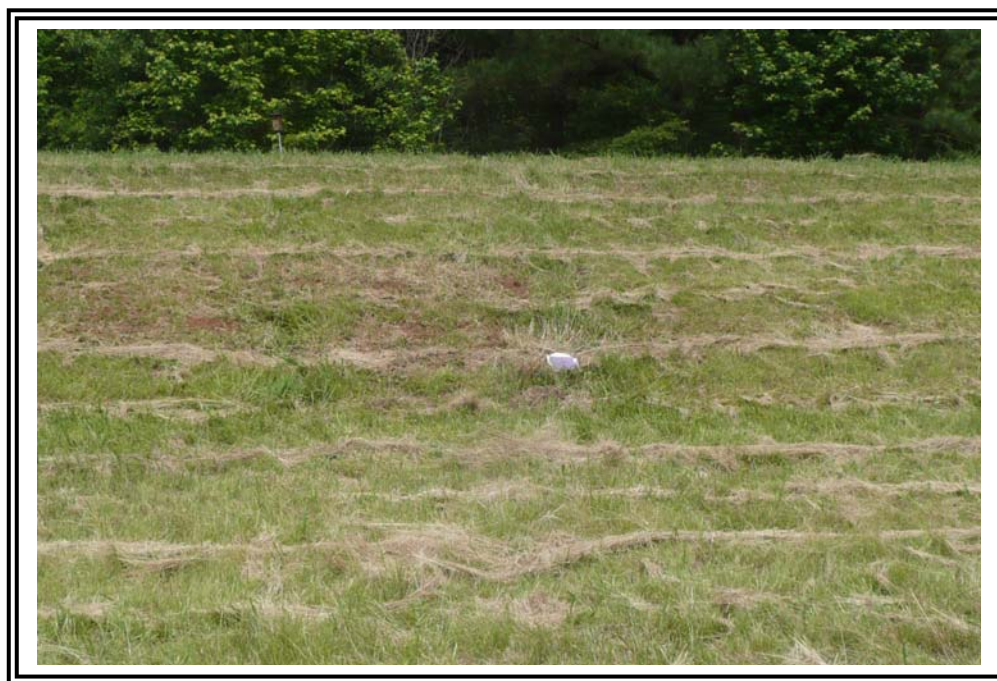
More erosion or settlement locations on downstream slope of Diverter Dike as noted by clipboard and dark green grass to left of clipboard.
