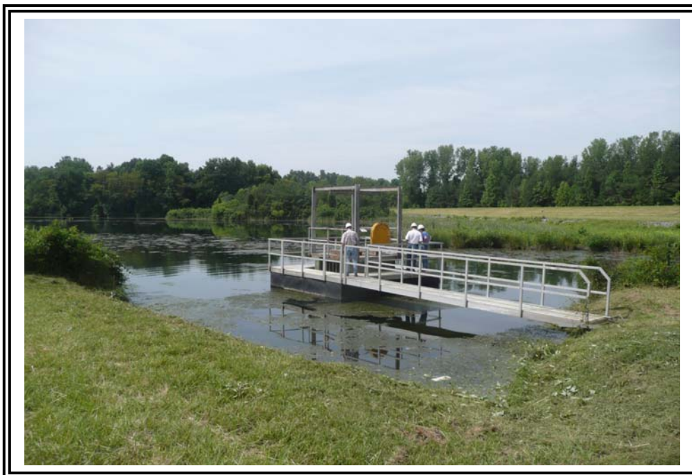
Outlet control structure in Basin 3. Structure is surrounded in Y-shaped berm system, not part of the Main Dike.
