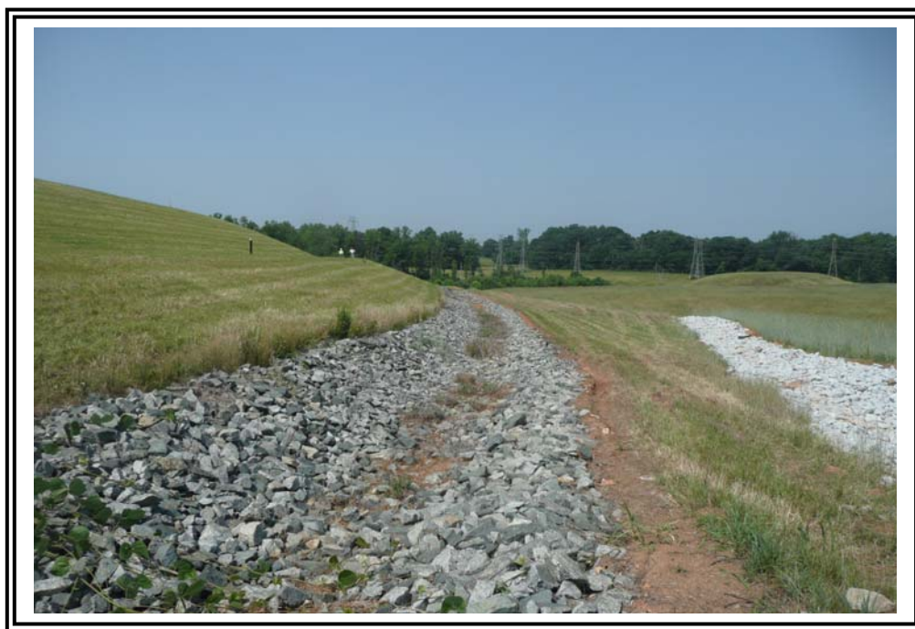
Downstream slope and toe drainage swale along northern portion of the New Dike looking southwest.
