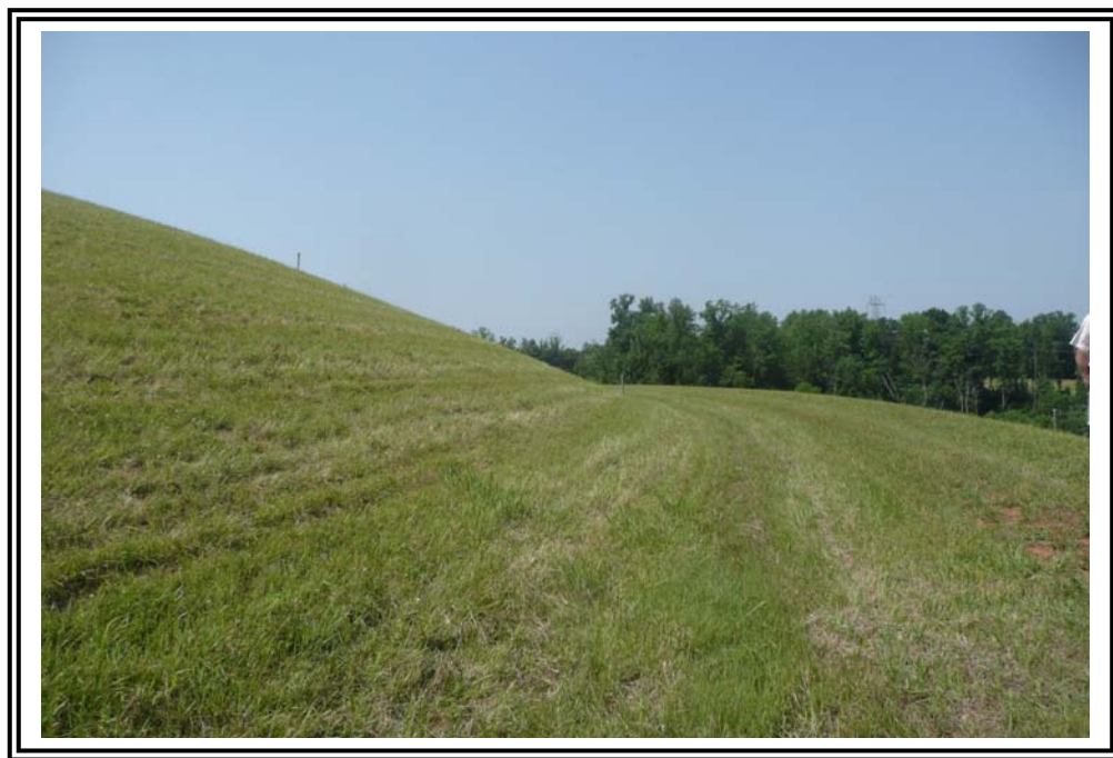
Downstream Slope at Upper Bench of New Dike looking southwest. Note occasional sparse grass cover.
