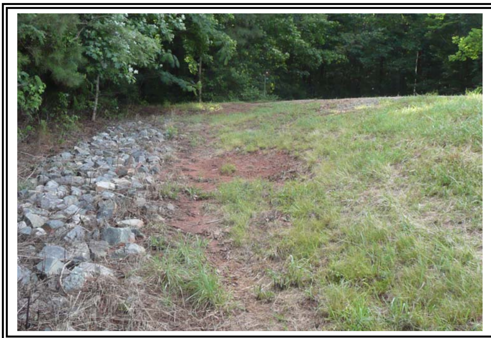
Sparse vegetation on downstream slope at east end of maintained Main Dike, looking east.
