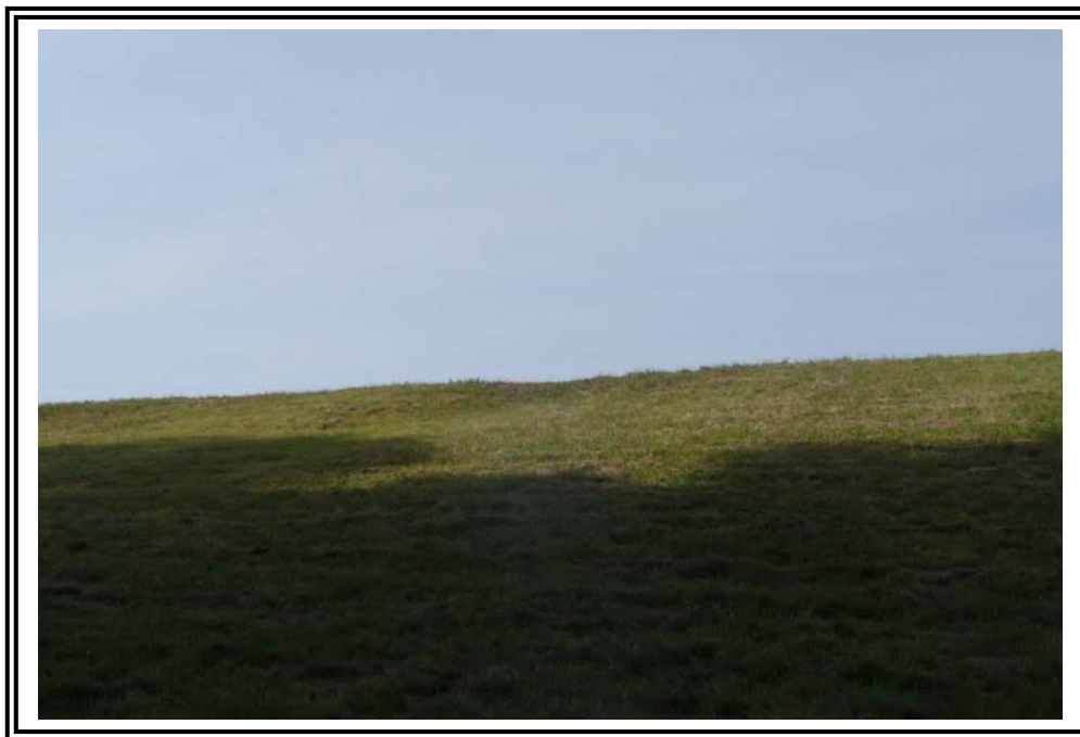
Low spot at crest, as seen from toe of Main Dike, location is adjacent to Basin 3.
