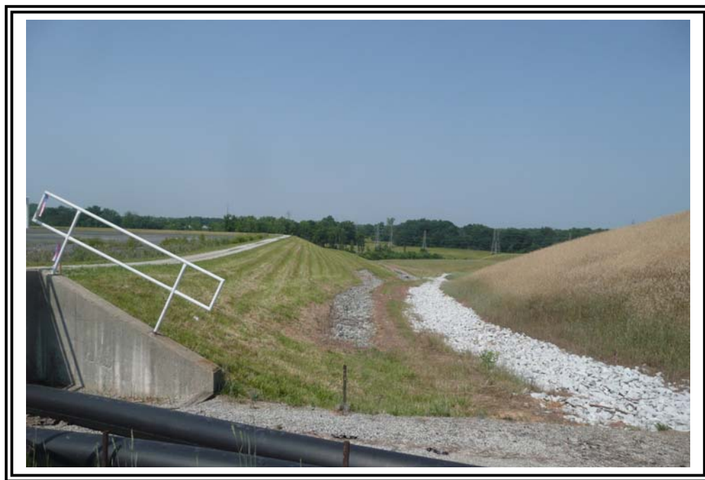
Downstream Slope looking southwest from North Abutment. Note “gray” rip rap swale is groin drainage swale associated with the New Dike, the “white” rip rap to the right is a surface drainage swale associated with the combined cycle plant currently under construction. Hill in near right of photo is a stockpile of excavated material from the combined cycle plant construction.
