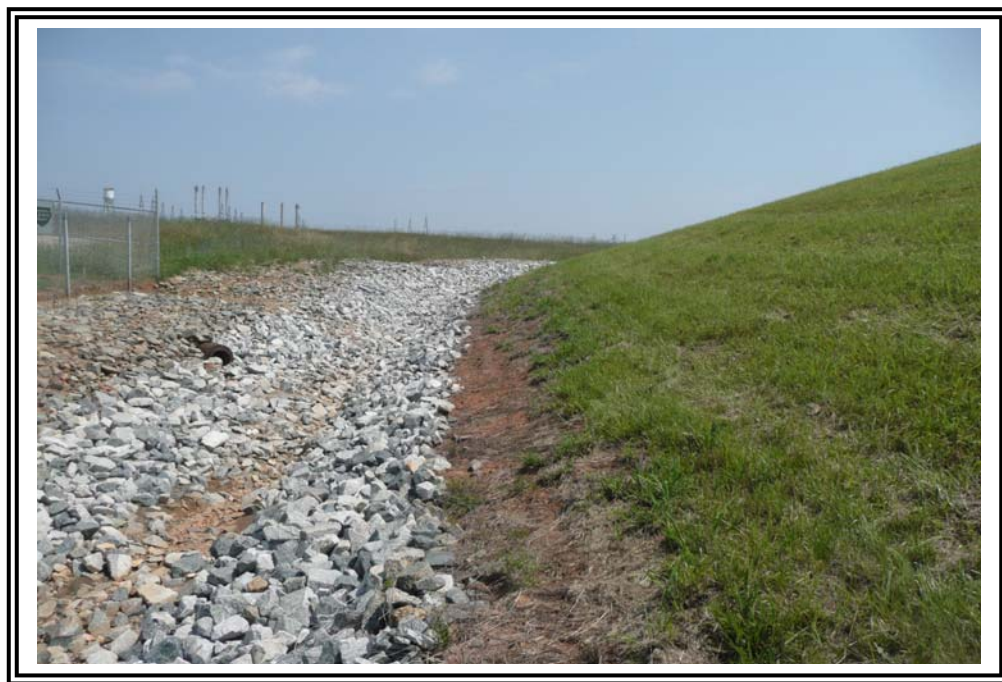
Toe swale of New Dike looking north. Note drainage pipe entering drainage swale from across access road to new combined cycle plant site. Sparse vegetation along rip rap edge likely from herbicide use to control weeds in the rip rap.
