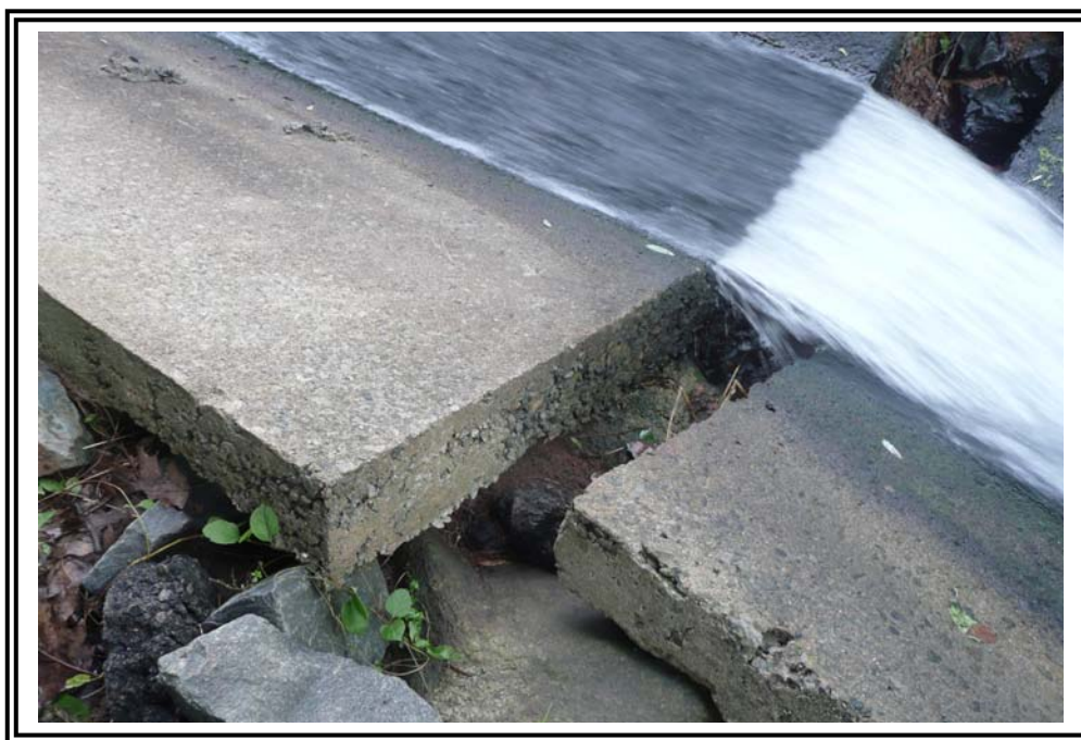
Slight undermining of concrete discharge channel at river end.
