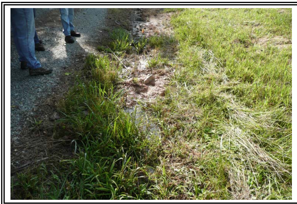
Clogged groin drainage swale on west end of Main Dike. Sediment appeared to include bentonite chips, possible runoff from poorly cleaned up drilling at “new” monitoring wells.
