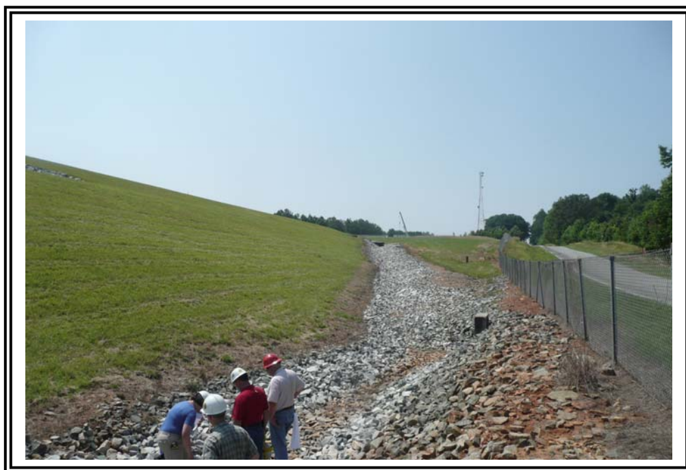
Drainage swale at toe of New Dike looking south.
