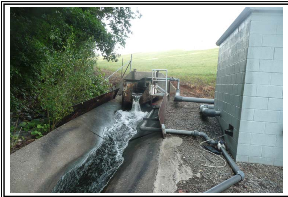
Discharge end of Basin 3 outlet.
