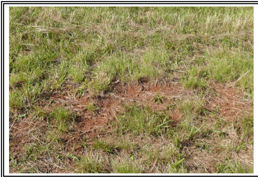
Close up of poor vegetation cover on downstream slope of Main Dike.
