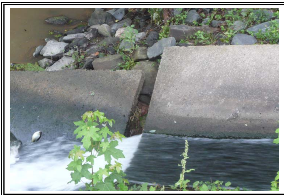
Last section of concrete channel has separated. Noted in previous inspection reports.
