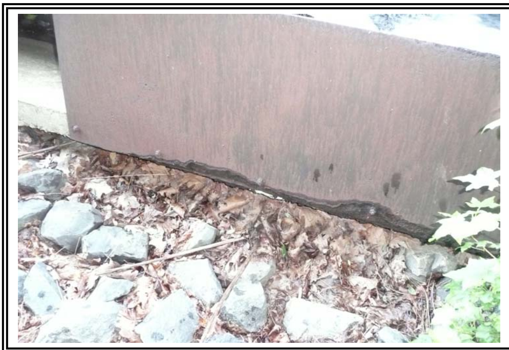
Slight undermining of concrete discharge channel at outlet structure. Baffles in place to control splash out of channel during high flows.
