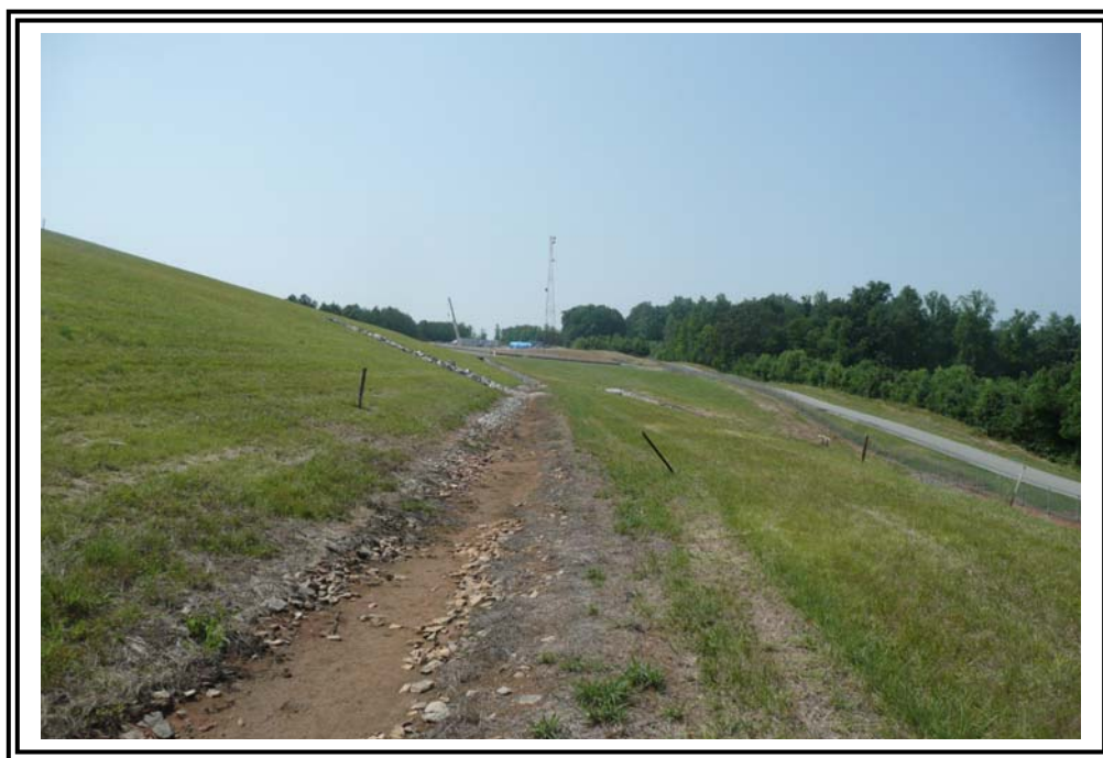
Lower Bench of New Dike looking south. Note silt deposited in drainage swale.
