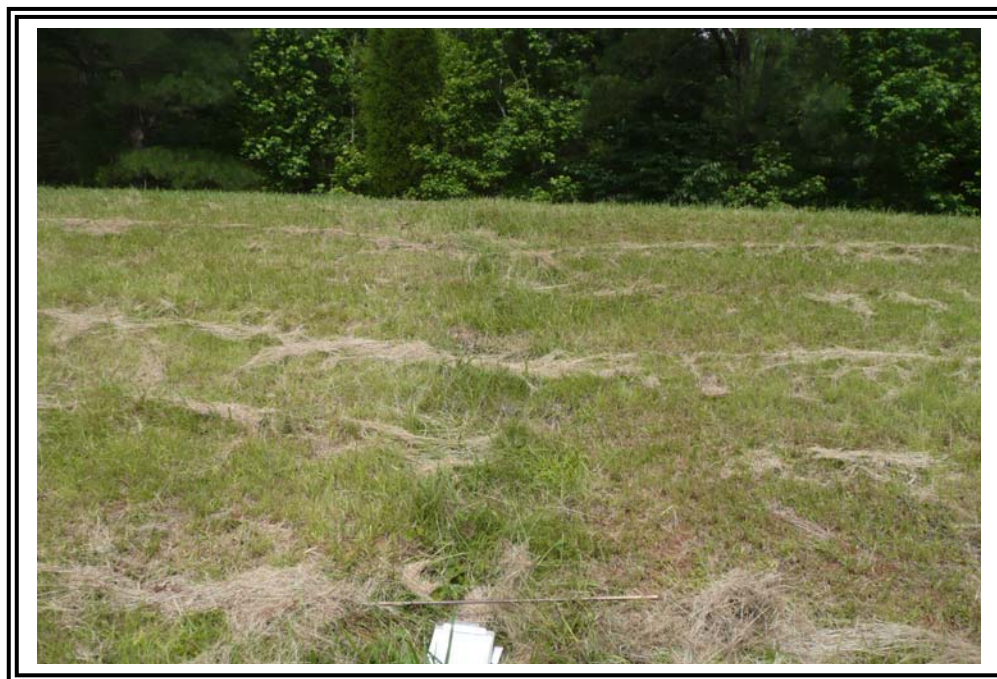
Erosion swale on downstream slope of Diverter Dike.
