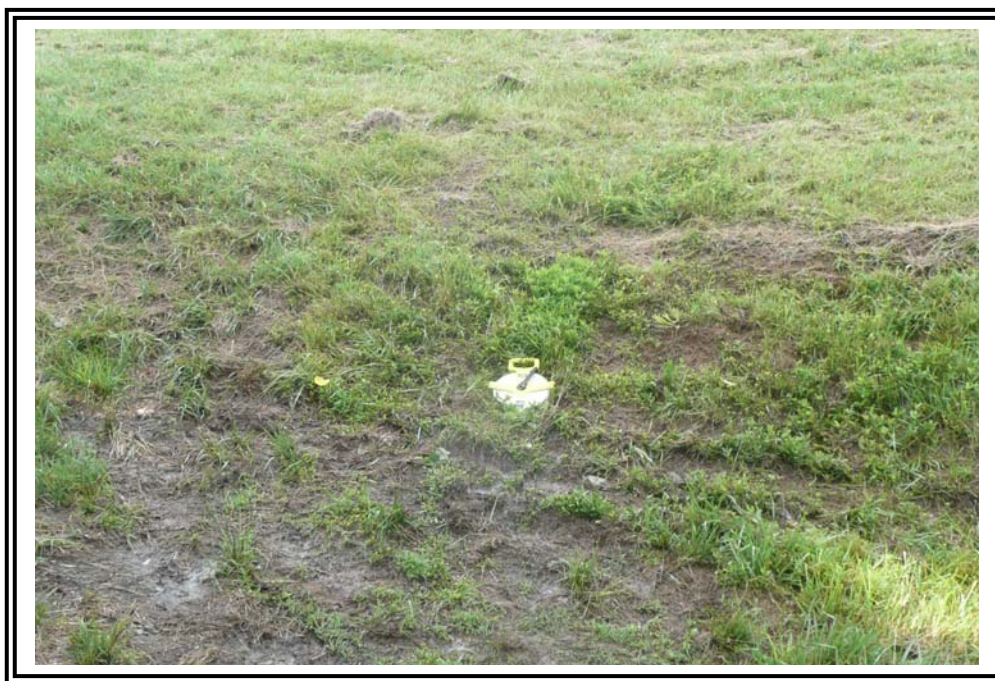
Sparse vegetation at toe of Main Dike near the outlet structure.
