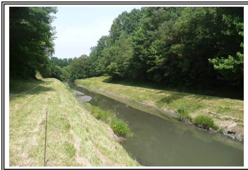
Downstream discharge channel from Basin 2 outlet. Plans indicate channel was excavated into natural ground.
