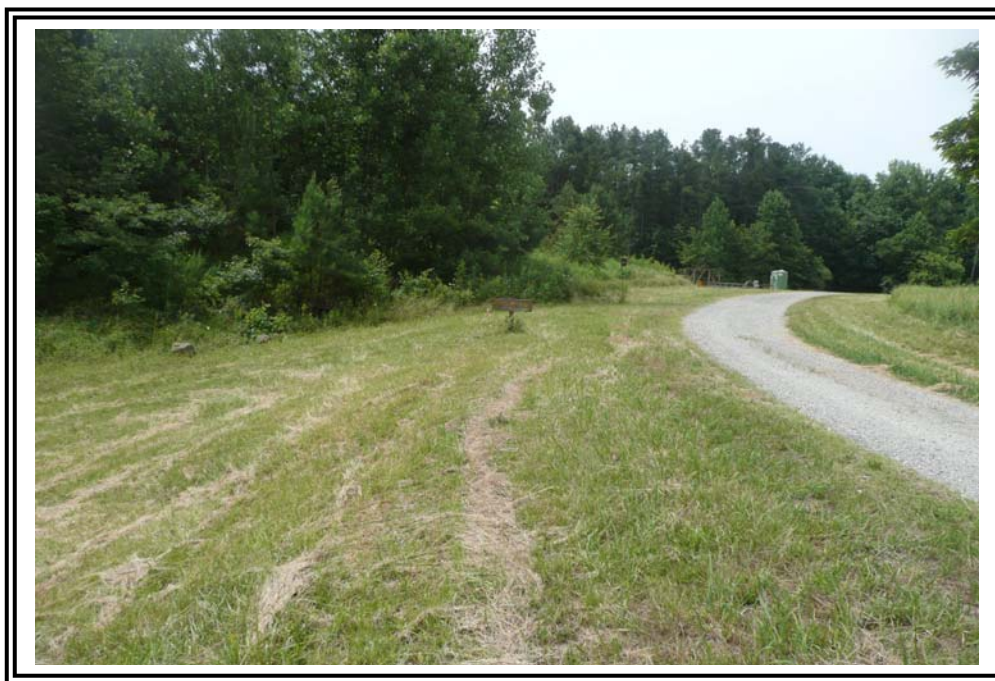
Downstream slope of Diverter Dike, looking south.
