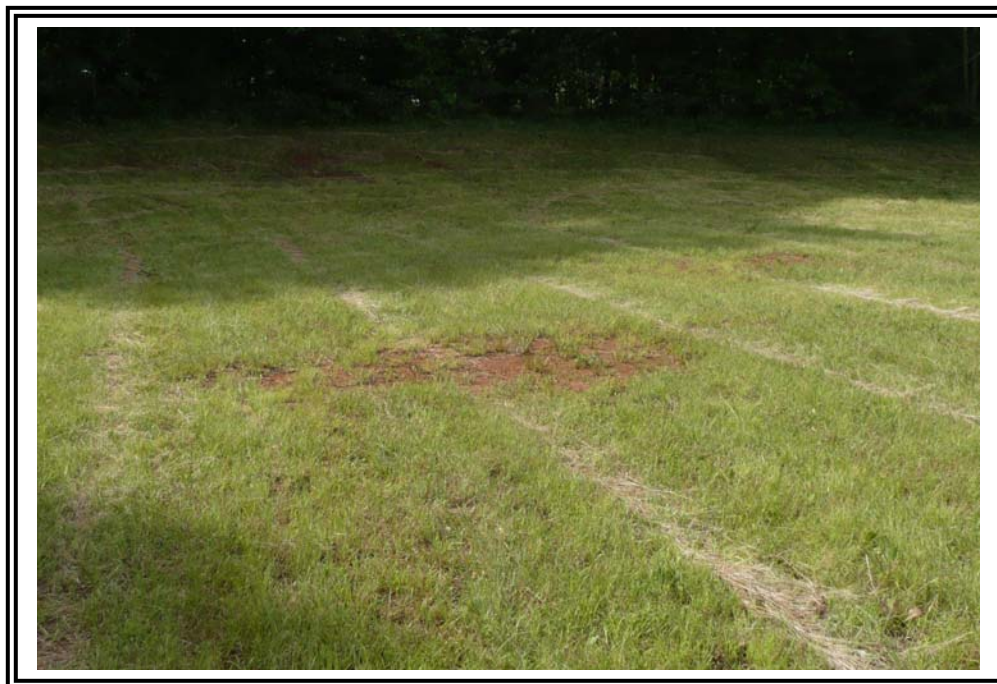
Sparse vegetation within Emergency Spillway.
