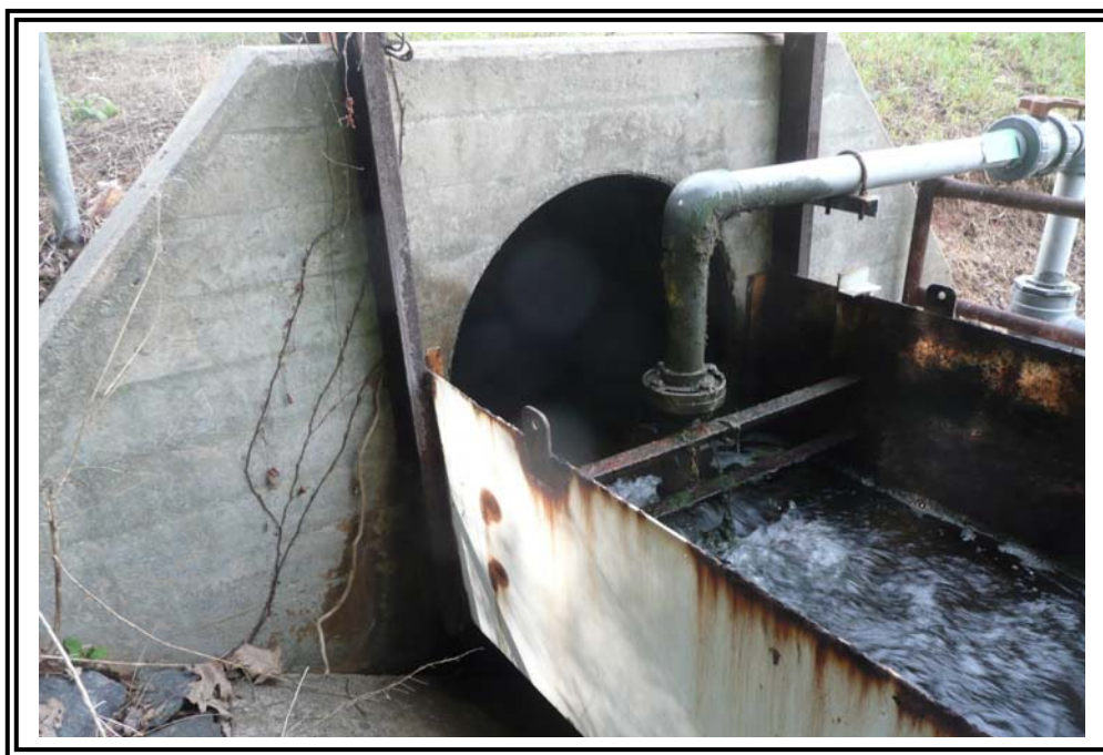
Main Dike outlet pipe headwall and pH treatment.
