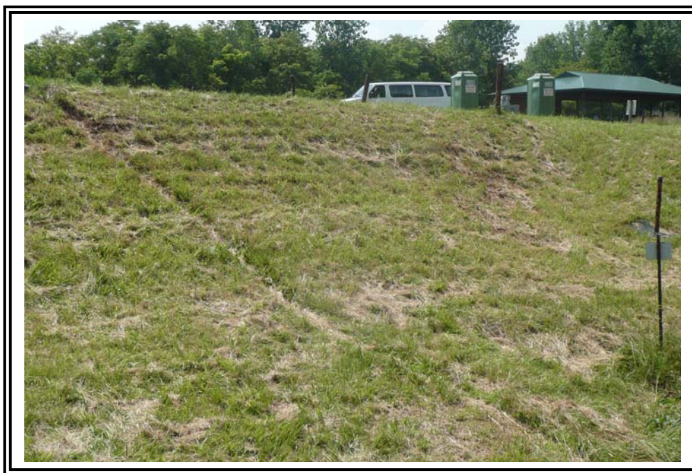
Animal trail on downstream slope of Basin 2 to Basin 3 outlet dam.
