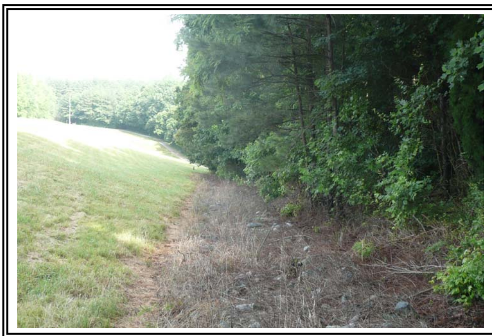
Herbicide treated vegetation in groin swale at the east end of Main Dike.
