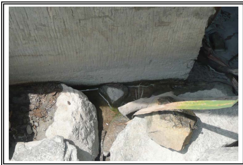
Seepage noted adjacent to downstream end of outlet pipe headwall.
