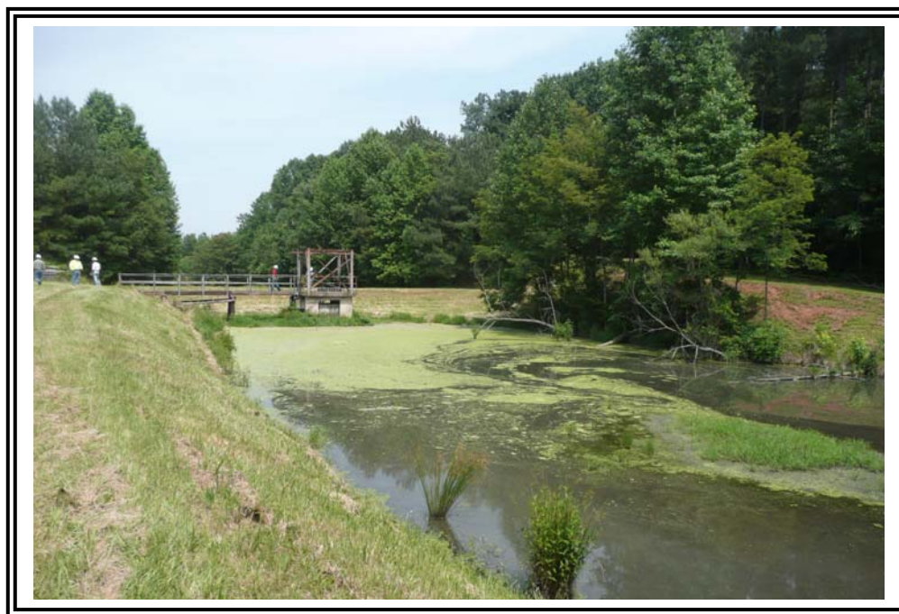
Basin 2 outlet control structure. Note: Photographer at rim of channel excavated into natural ground.
