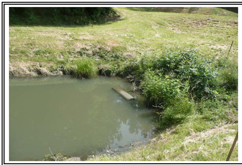
Basin 2 outlet pipe submerged on downstream end. Note: Headwall visible at water surface.
