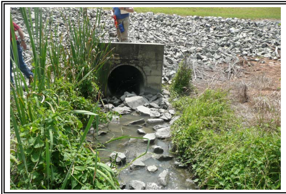
Downstream end of Basin 1 outlet pipe.
