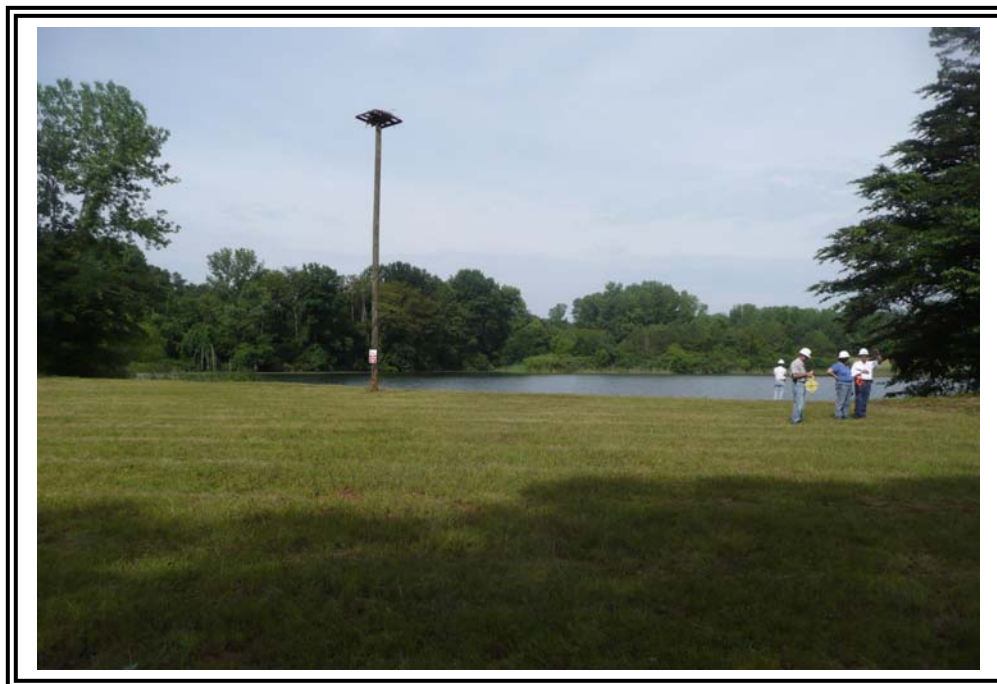
Emergency Spillway, looking west at Basin 3.
