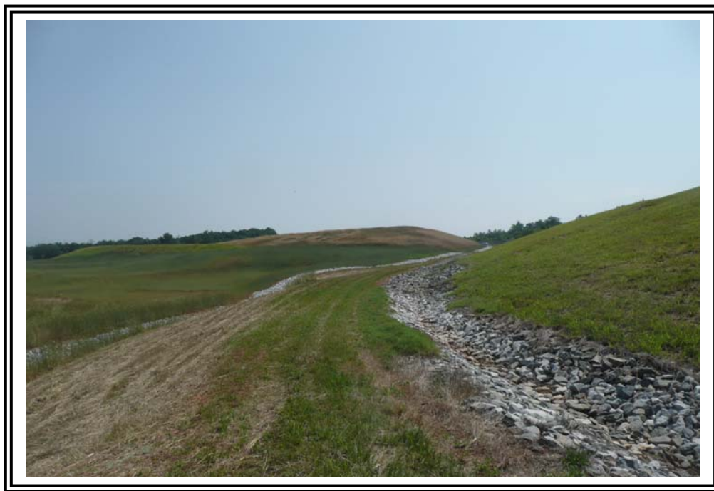
Toe of New Dike looking northeast. Toe drainage swale is in right of photo, slope down to the left is natural ground cut to new combined cycle plant site.
