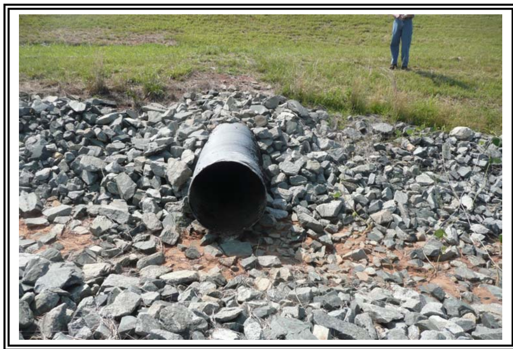
Upper bench drainage swale culvert discharging into toe swale.
