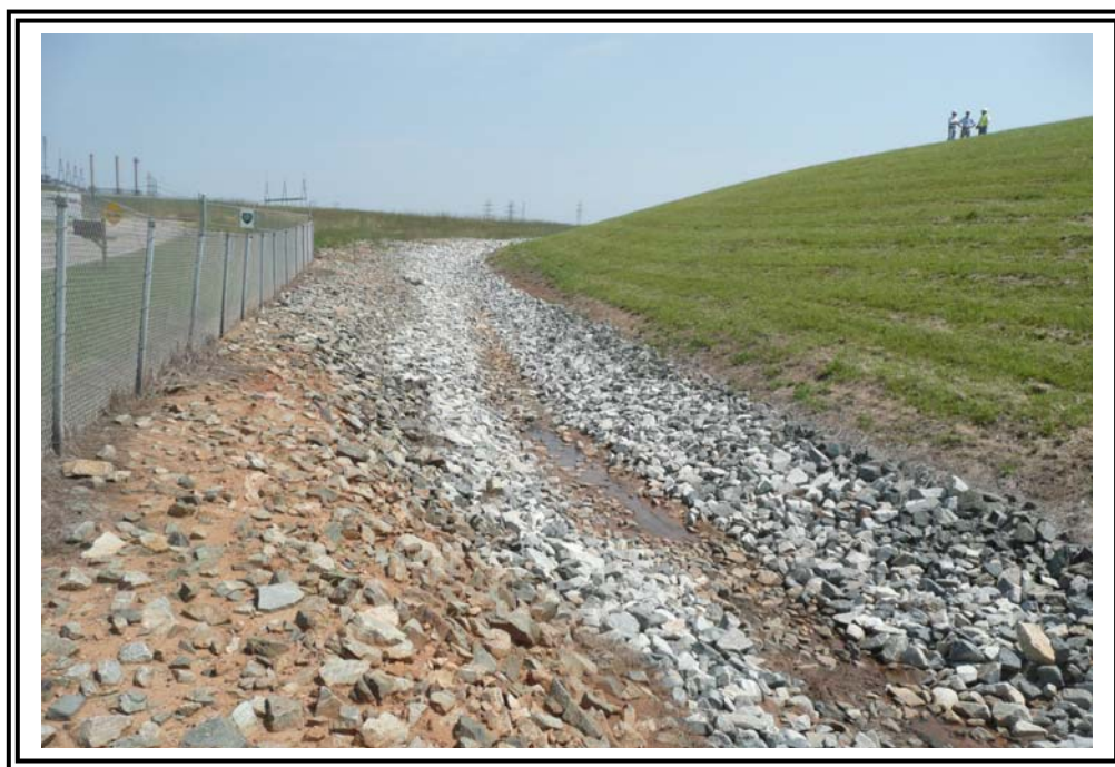
Toe swale of New Dike looking north. Area of toe drain seepage. Area starts about 100 feet north of discharge culvert under Dukeville Road.
