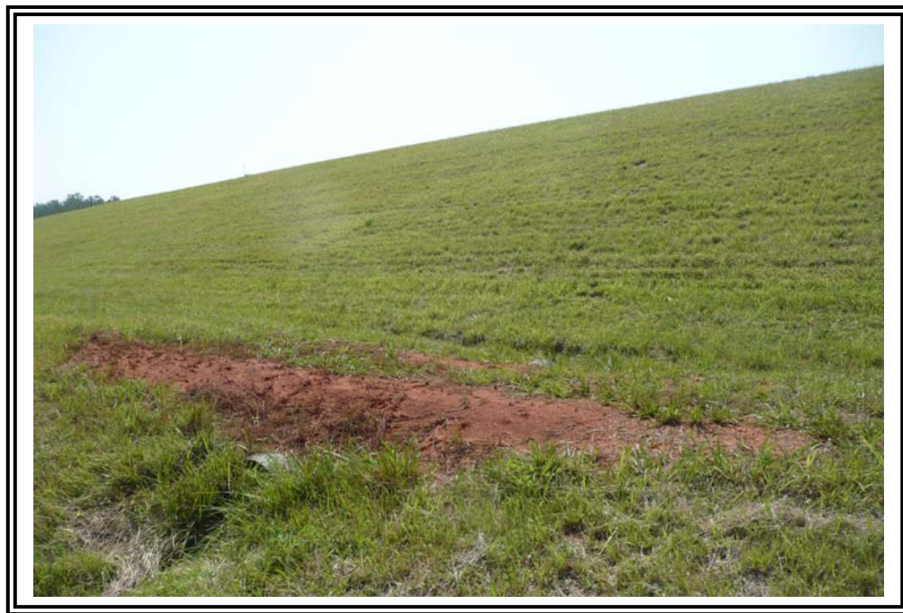
Surface drain from Upper Bench. Downstream Slope looking northeast.
