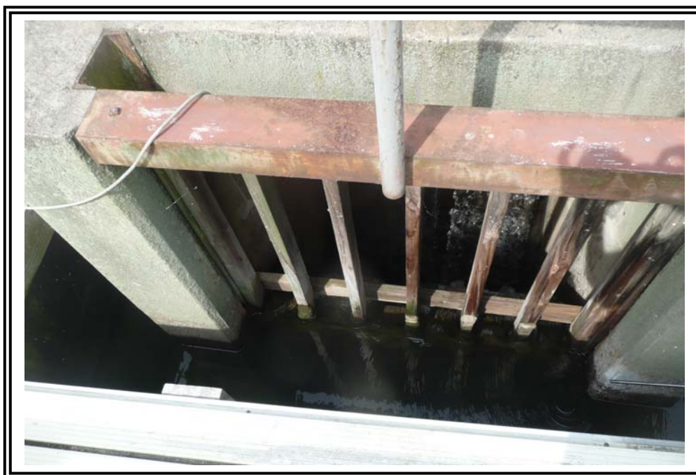
Timber trash rack sits on stop logs in Basin 3 outlet structure and can be easily removed if adjustment of stop log elevation is required.
