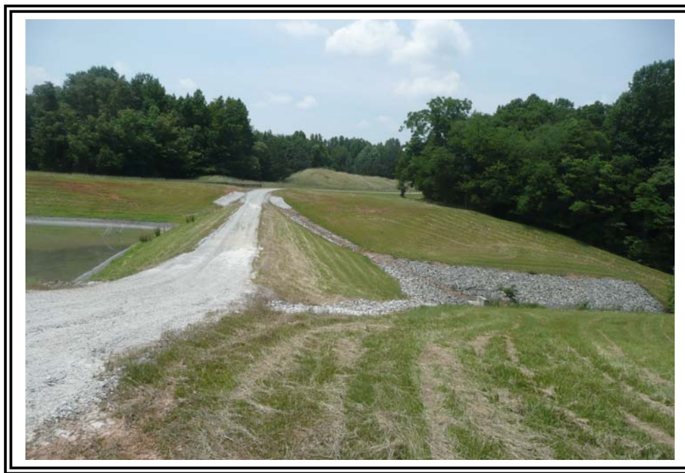
Outlet dam from Basin 1 to Basin 2 looking north. This dam is in a cut channel created to drain Basin 1 into Basin2 through a high point in the natural topography.
