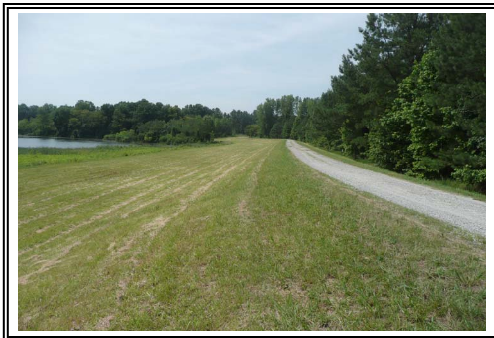
Downstream (Basin 3 side) slope of Diverter Dike, looking south. Note: Diverter Dike was constructed with a 50-foot wide bench at the Basin 3 toe of slope.
